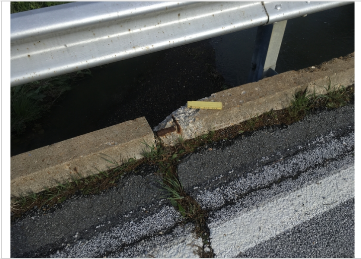
Spalling with rebar exposed on the left curb of span 2.
