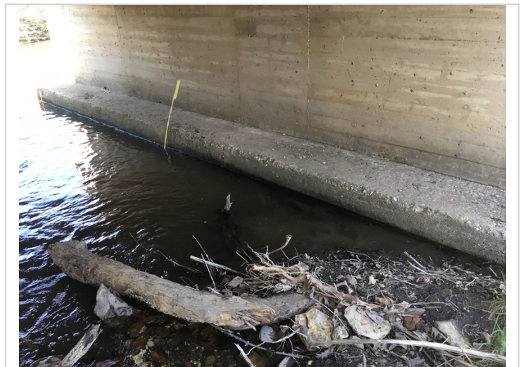
General view of the abutment #2 footing. Showing 22" of vertical face exposed.
