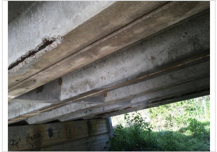
Span 1 undersurface. Showing spalling with rebar exposed.
