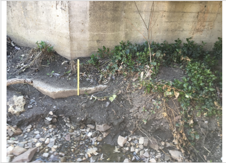
The footing is exposed at the right upstream corner of pier wall #1. With 4" of vertical face exposed for 4'.
