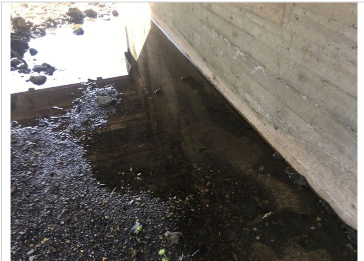
General view of the exposed footing at pier wall #2.
