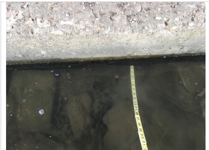
16" of undermining at the mid section of the abutment #2 footing.
