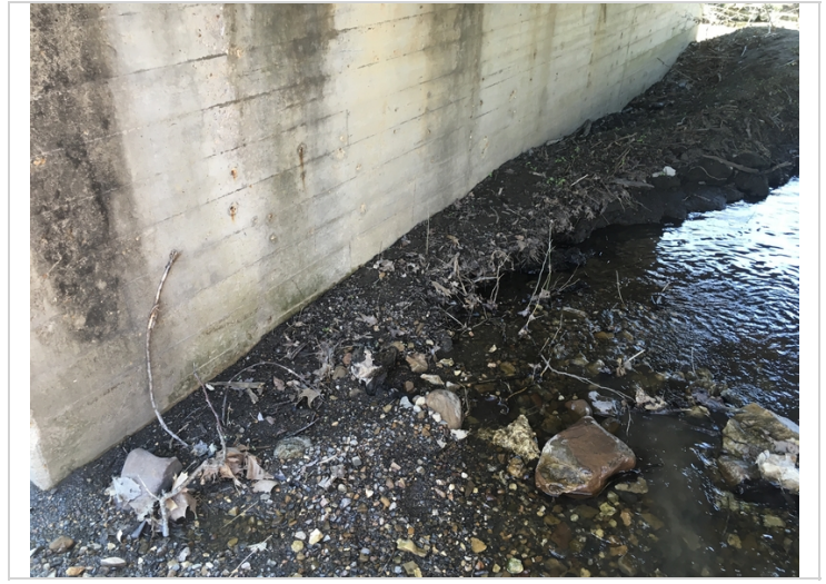
Pier wall #2 has cover over the footing.
