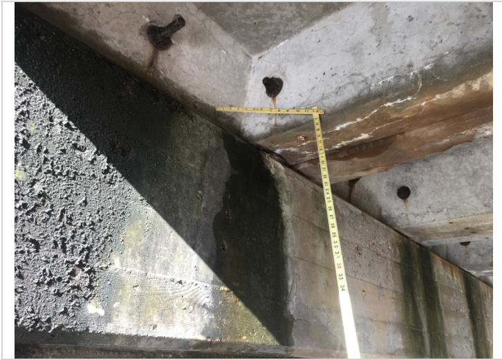
Map cracking with efflorescence on RCCB 7 at the beginning of span 2.
