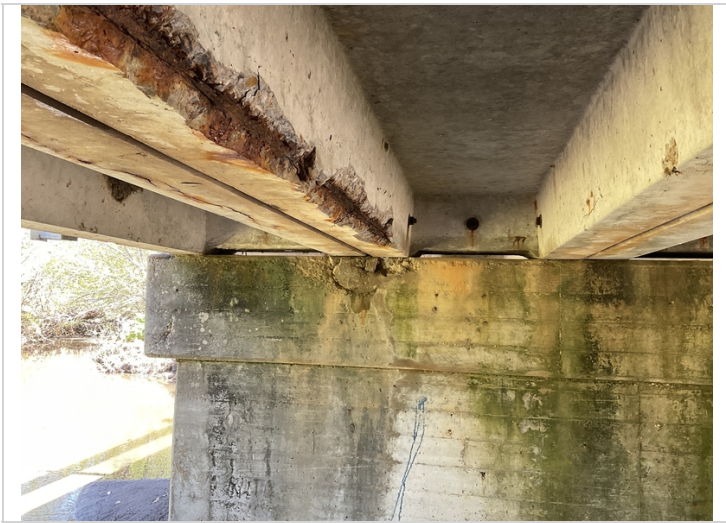
Spalling of cap at bent #1 span #1 under units #1 and #2
