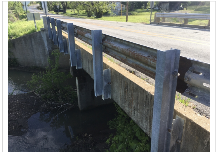
View of the corrosion on the back side of the metal railing.
