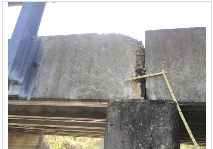
The outside face of RCCB 1 at the beginning of span 2 showing map cracking with efflorescence. Spalling with exposed rebar exists in the same footage.
