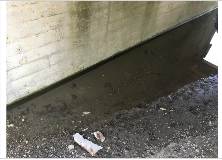
15' of the top of the footing is exposed on the span #1 side of pier wall #2.
