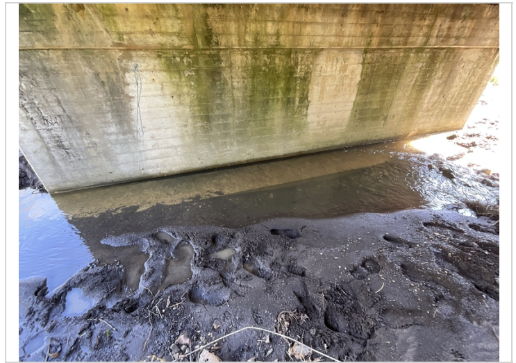
Footing at bent #1 behind side is exposed.
