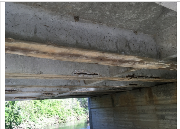
Span 2 undersurface showing spalling with rebar exposed.
