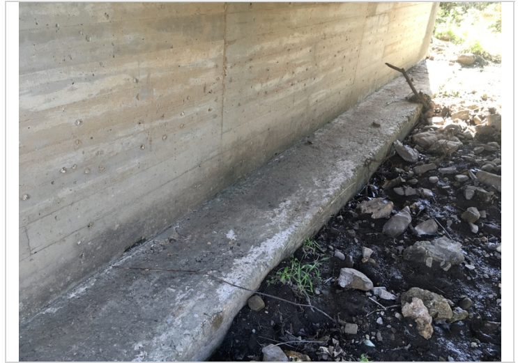
Exposed footing at abutment #2. Showing spalling on the outer edge.
