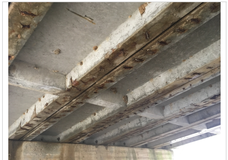
Undersurface condition in span #1.
