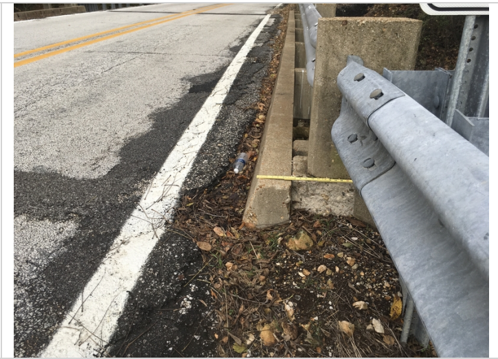
12" of concrete exposed to traffic. Typical of all 4 corners.
