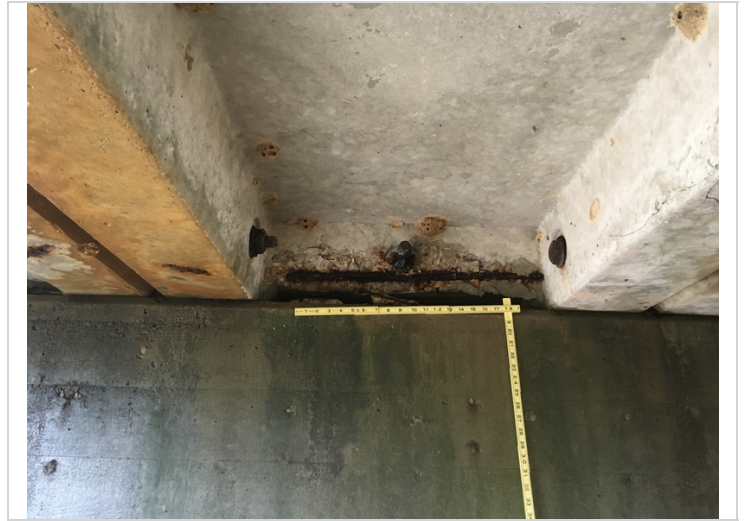
Spall with rebar exposed in the diaphragm of unit #2 at the end of span #1. Typical.
