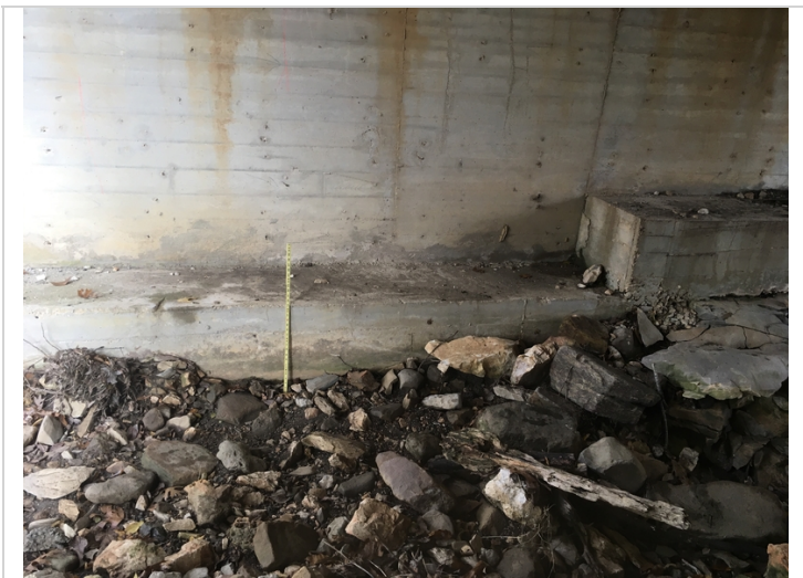
19" of vertical face of the footing exposed at abutment #2 for the length of the abutment.
