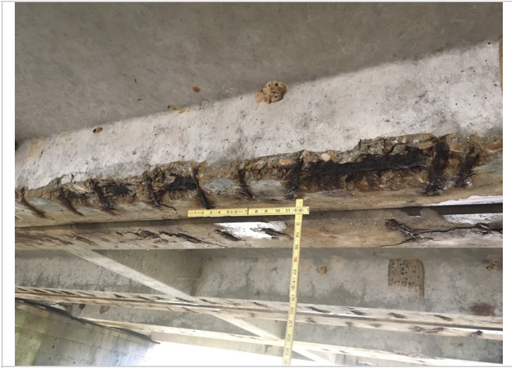
Deep spalling with exposed primary longitudinal rebar in the right stem of unit #4 in span #1. Typical of several locations.
