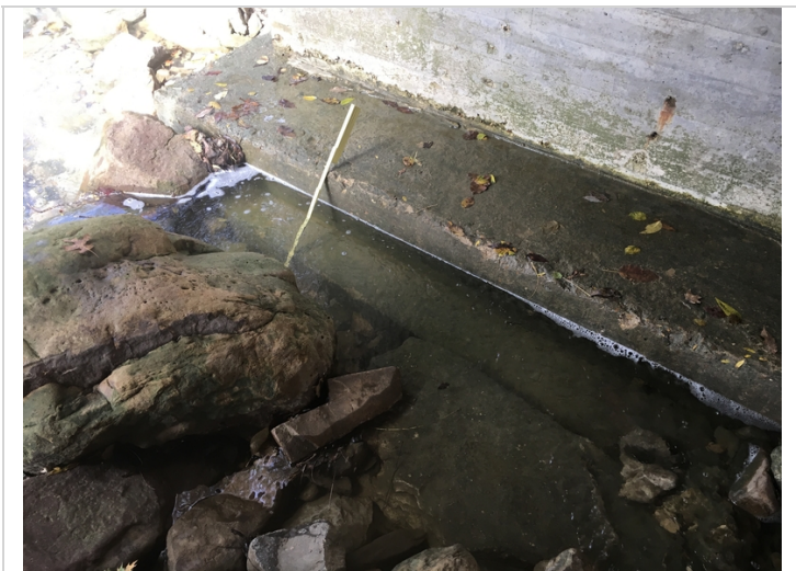
Exposed footing with 20" of vertical face exposed on the span #2 side of pier wall #2.
