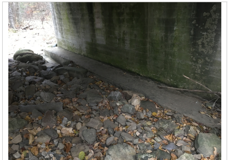
Exposed footing for the full width of pier wall 2.
