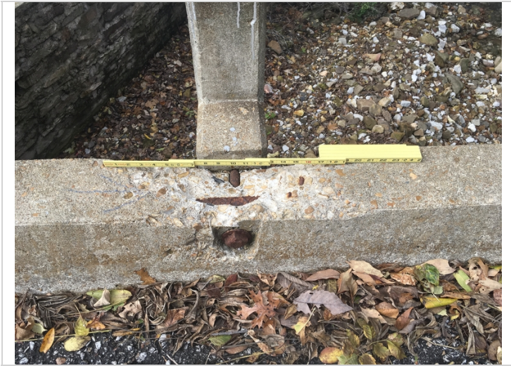
Spall with exposed rebar on the left curb at post #3.
