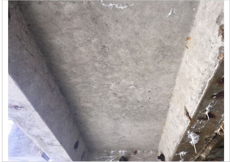
Efflorescence map cracking in the undersurface of the deck of unit #7 typical in spans #1,2,3.
