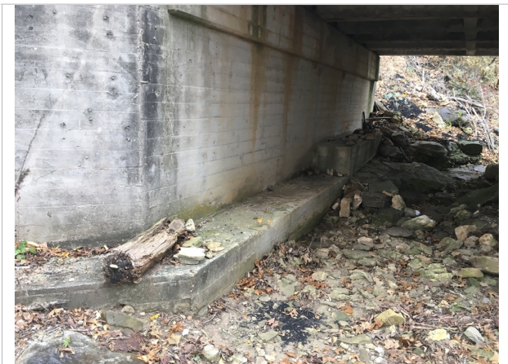
Exposed footing at abutment 2.
