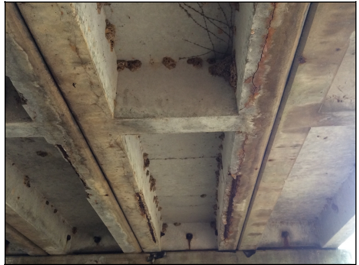
Span #2, unit #6-Spalling with exposed reinforcing steel in stems.
