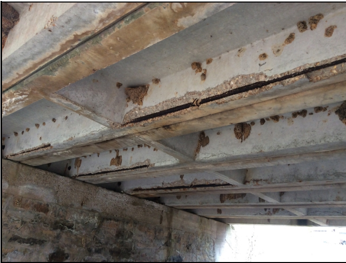
Span #3-General view of spalling with exposed reinforcing steel in stems of channel units.
