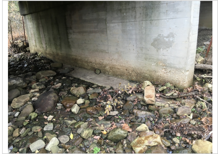
Exposed footing at pier wall 1.
