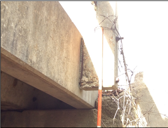
Spalling with exposed reinforcing steel to bridge railing post.
