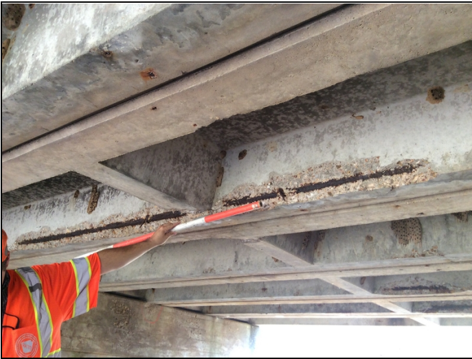
Span #1, unit #3, Right stem with spalling and exposed reinforcing steel.
