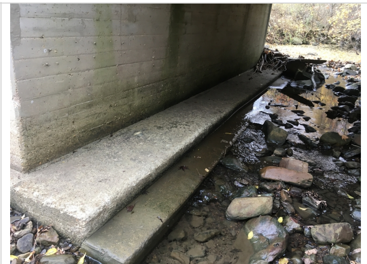
Exposed footing at pier wall 2.
