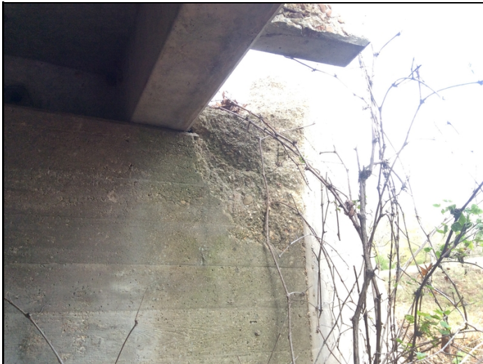
Spall on the Right side of abutment #2 breastwall.
