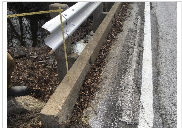
The railing end post on the right side of abutment #2 has been displaced due to collision damage and is exposing an unprotected end of the metal railing.
