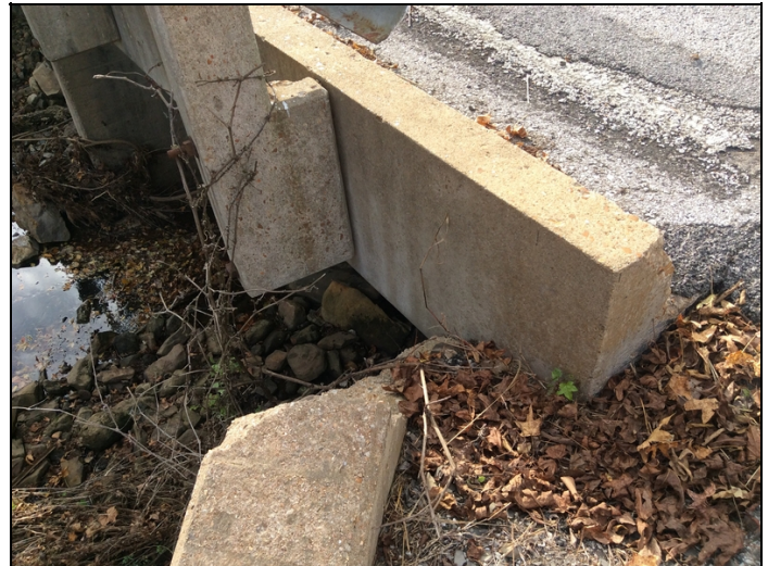
Abutment #2, Right side railing missing end post.
