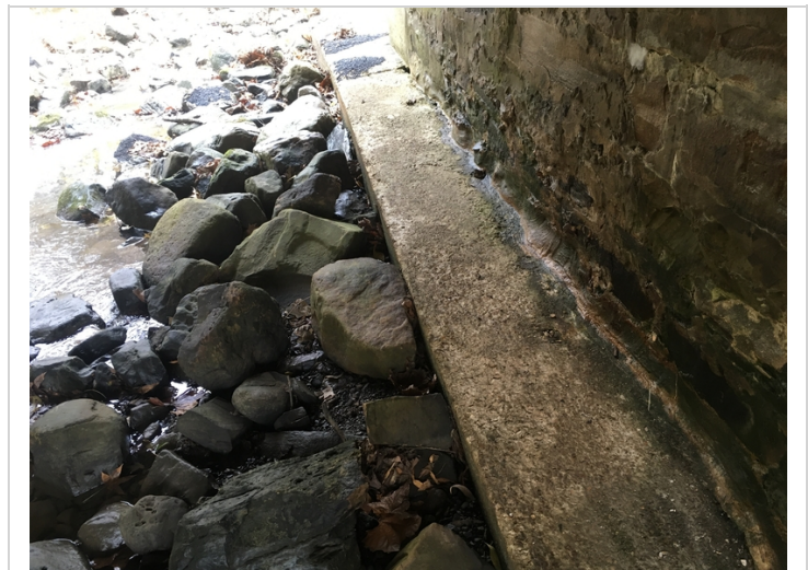
Exposed footing at abutment 2.
