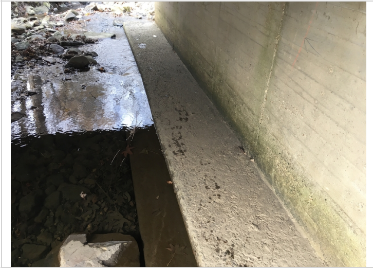
Exposed footing on the span #2 side of pier wall #2 for the length of the wall.
