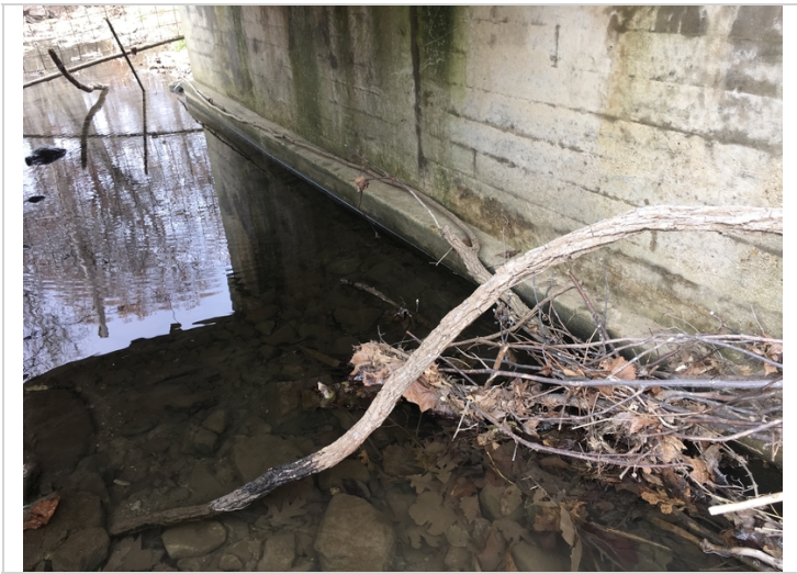
Exposed footing on the span #1 side of the pier wall.
