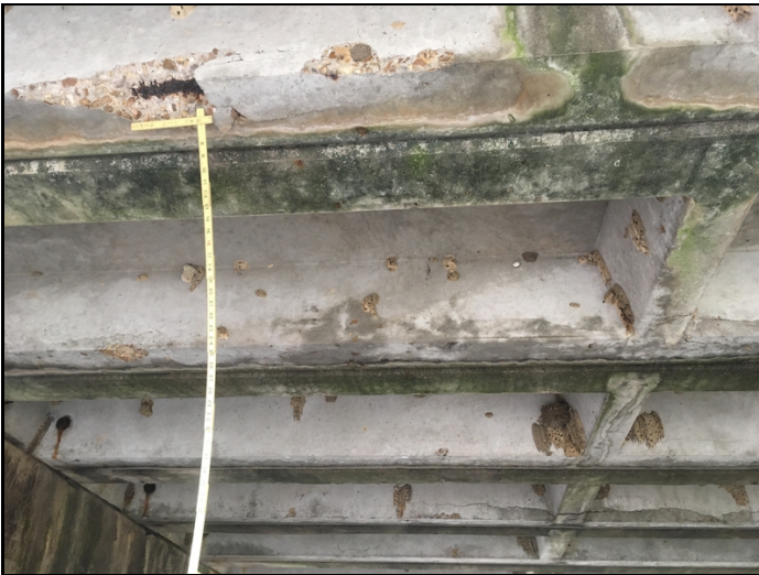
Spalling with exposed rebar on unit 1 in span 1.
