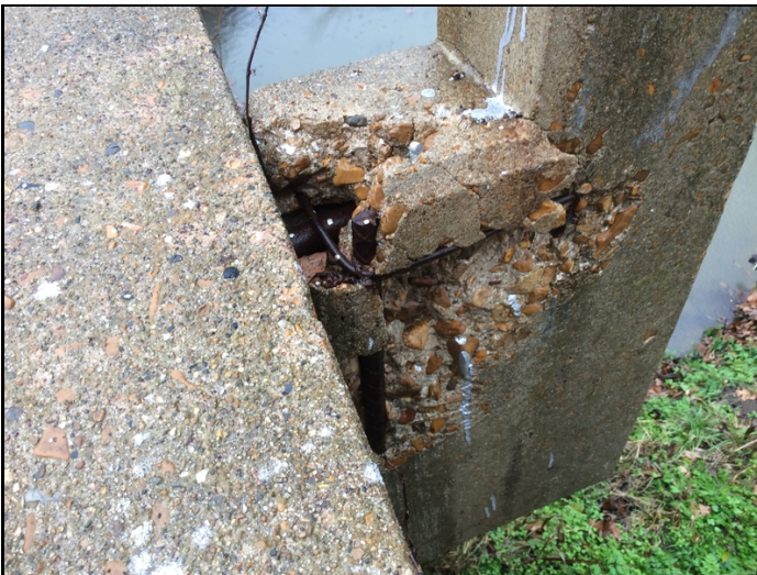
Spall with exposed rebar at post #2 at right side of span #1.
