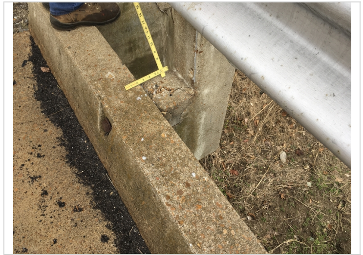
Right side post #7 has vehicle damage.
