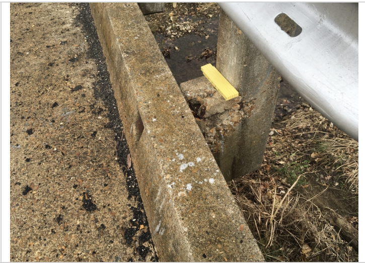
Right side post #2 has vehicle damage.
