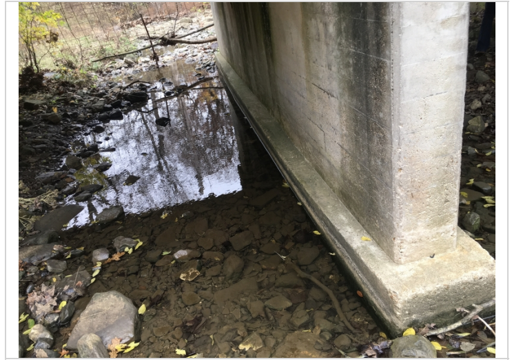
Exposed footing for the length of the pier wall on the span 1 side.
