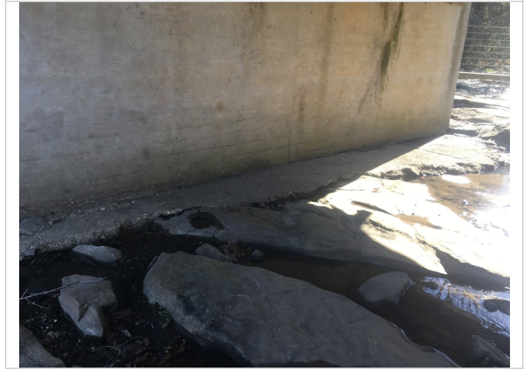
Exposed abutment #2 footing. Typical also of abutment #1.
