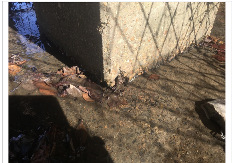
Cs3 abrasion on the extreme lower portion of column #2 of bent #2.
