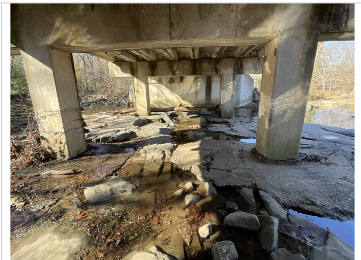
View of exposed footings at columns
