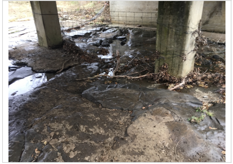
Exposed footings cast in solid rock.
