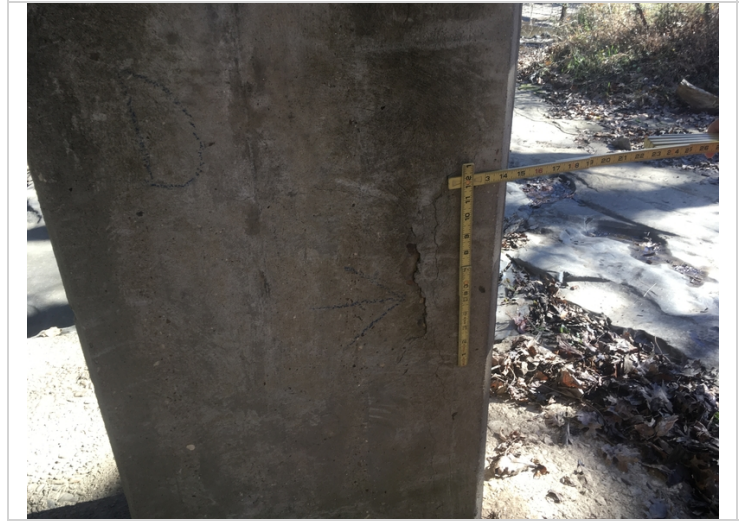
Delamination on column #2 of bent #1.
