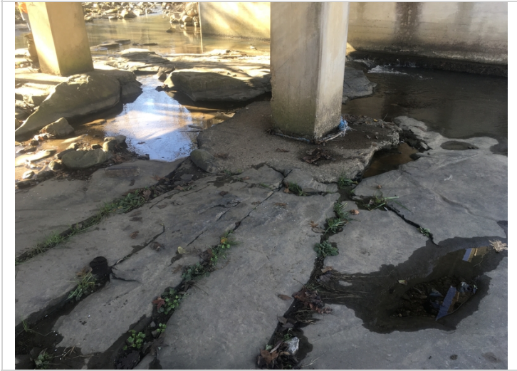
Exposed column footings. The footings are cast in solid rock. Typical view.
