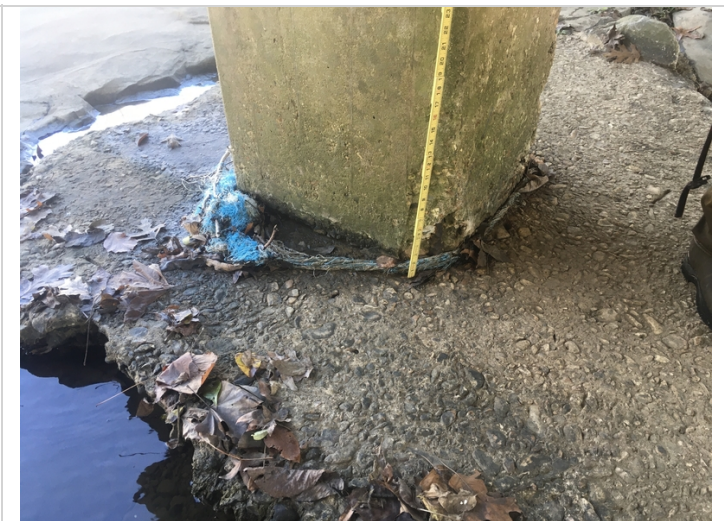
Spalling with rebar exposed on column #1 of bent #1.
