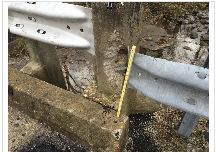
Right beginning end post has a large spall with exposed rebar.
