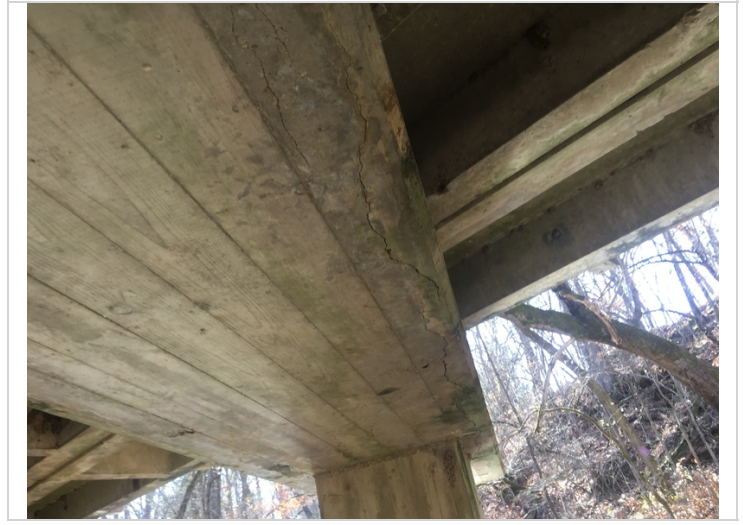
Large delamination on the under surface of the bent #3 cap.
