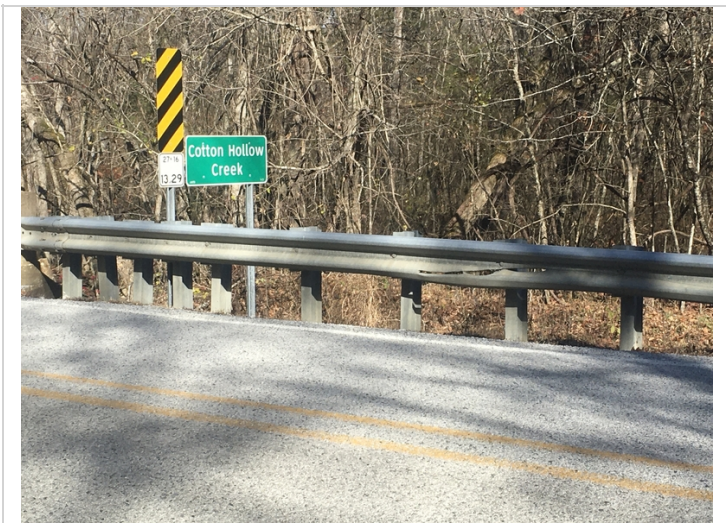
4' long tear in the face of the left ending approach railing.
