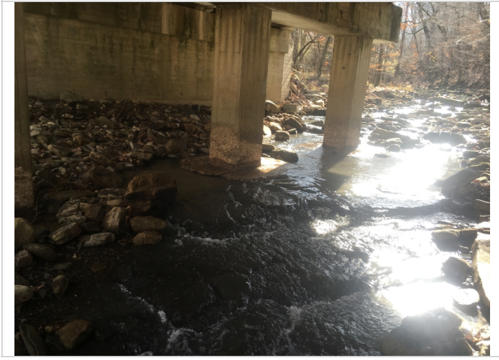
Exposed column footings at bent #3. Typical.
