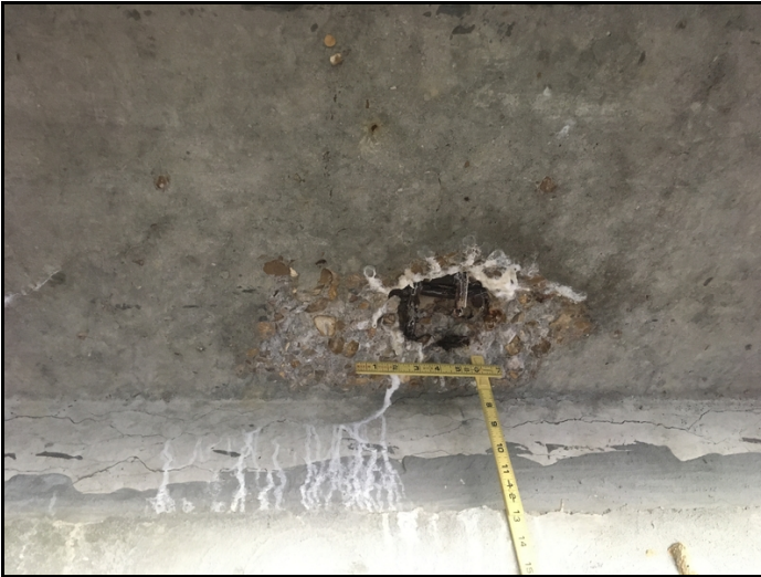
Spalling with exposed rebar in the undersurface of the deck. Typical of several locations.
