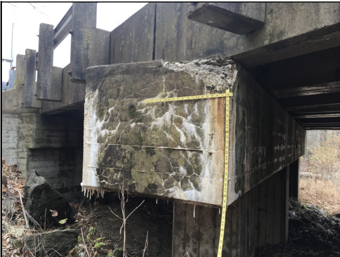
View of the right cap end of bent #1. Showing spalling and efflorescence map cracking. Typical also of the left end of the cap.
