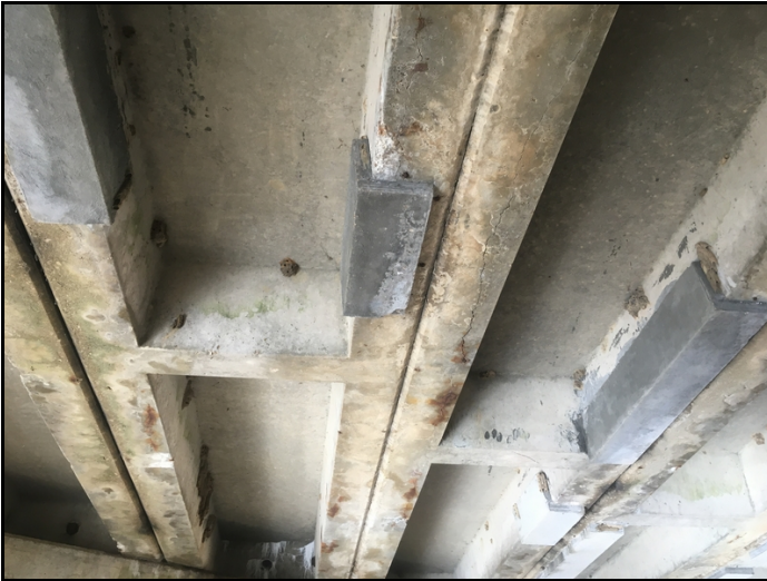
Repaired and unrepaired delamination on the channel beam stems. Typical.
