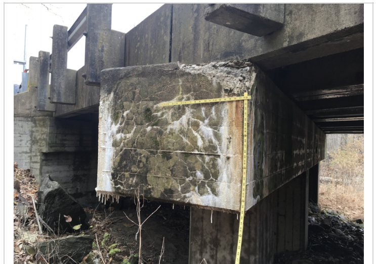
View of the right cap end of bent #1. Showing spalling and efflorescence map cracking. Typical also of the left end of the cap.
