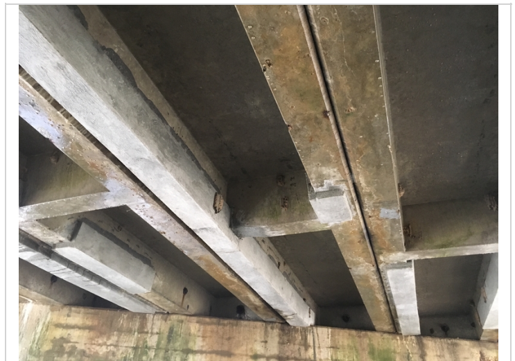
Typical view of the undersurface and repaired areas.
