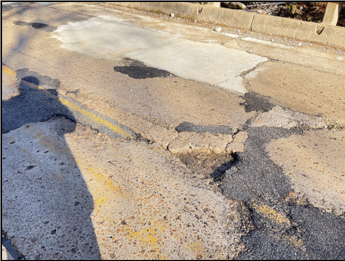
Basketball sized spall in the driving surface in span #1 end of unit #3
