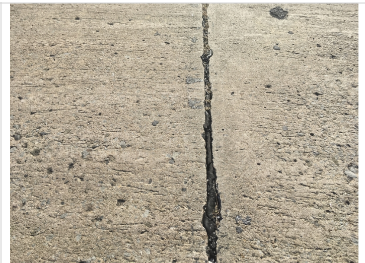
Joint seal condition over bent 2.
