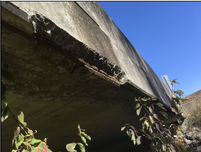
Spalling with rebar exposed at the right drip edge of span #3.
