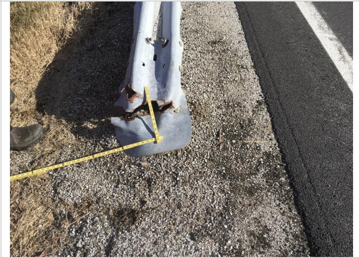
Left beginning approach railing termination has mower damage.
