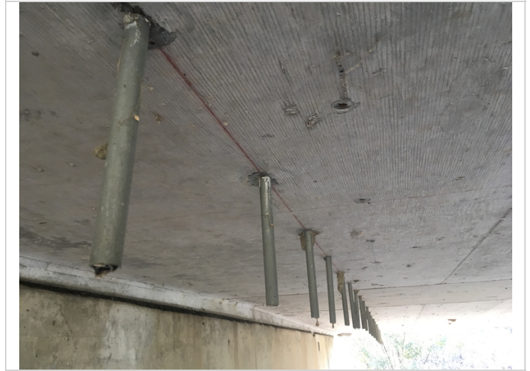
Pipes through the slab at the end of span #1.
