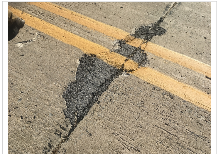
Repaired pot holes at the beginning of span 3.
