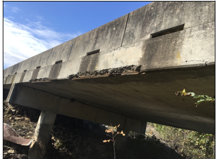
Spalling with exposed rebar at the right drip edge of span #2.
