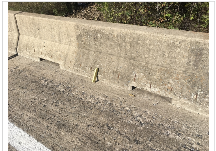
Areas of shallow exposed rebar along the bottom of the parapet walls.
