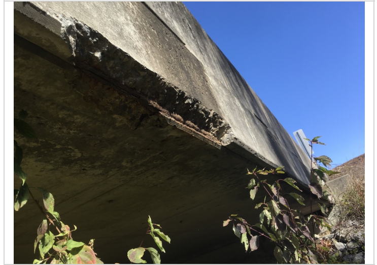
Spalling with rebar exposed at the right drip edge of span #3.
