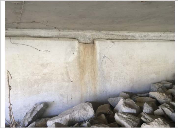
Delamination next to the left keyway at abutment 2.
