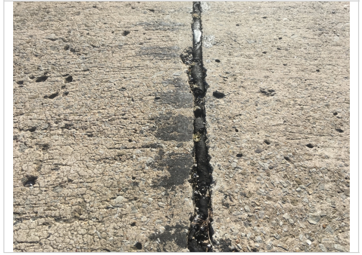
Joint seal condition over bent 1.
