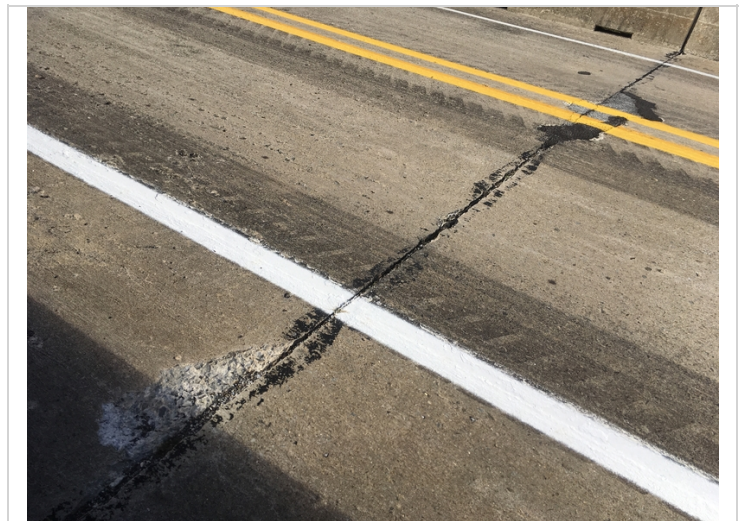
Spalling in the driving surface of the deck at the end of span #2, beginning of span #3.
