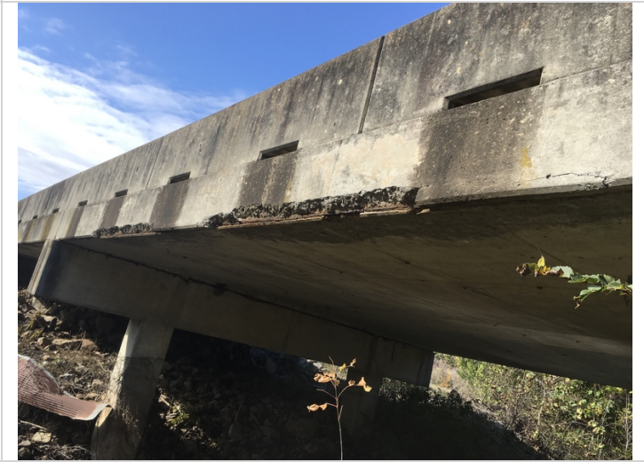
Spalling with exposed rebar at the right drip edge of span #2.
