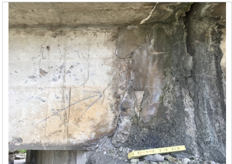
Exterior face of beam #1 at the beginning of span #4 showing 2' of spalling.
