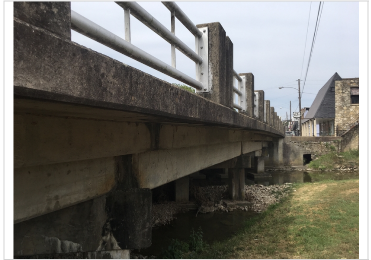
Typical view of the metal and concrete bridge railing.
