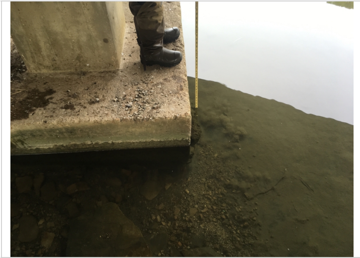
28" of the vertical face of the column footings at bent #1. Typical of all at bent #1.
