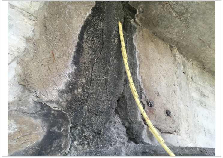
Vertical cracking at the beginning of tee beam #1 at the beginning of span #2.
