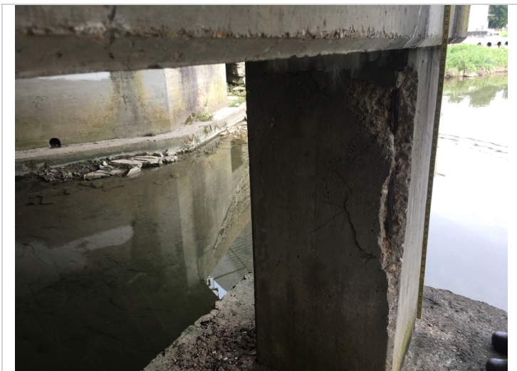
Large spall with rebar exposed on column #1 of bent #1.
