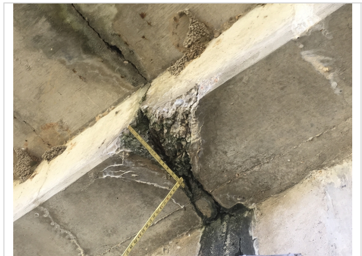
The left overhang in span #1 has a large spall with exposed rebar at the end of span.
