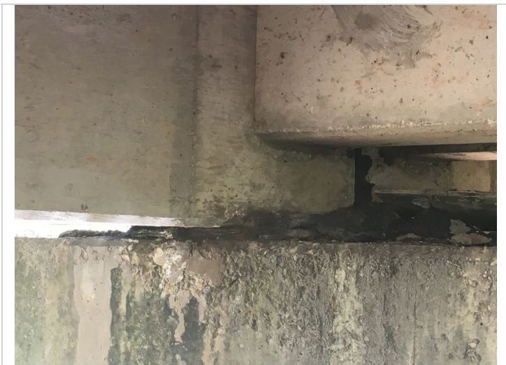
Beam #4 in span #3 bearing condition.
