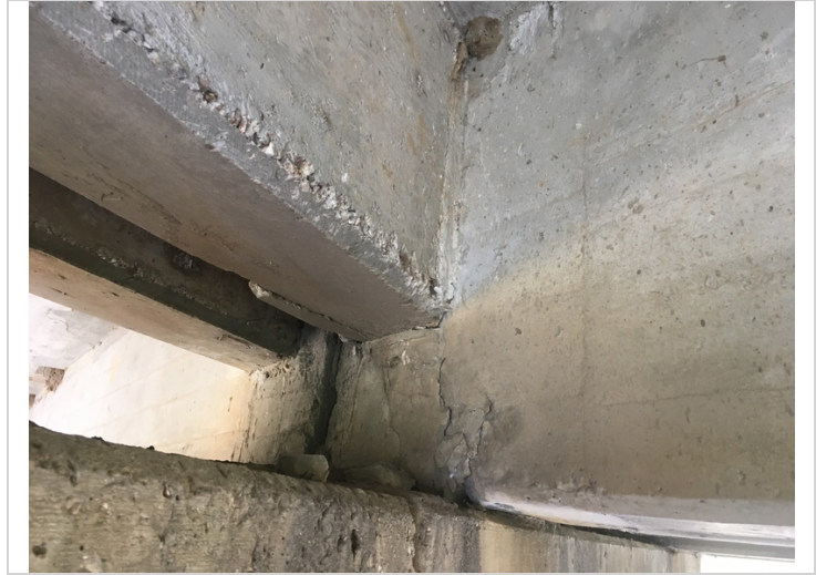
Spalling at the beginning of beam #3 at the beginning of span #3.
