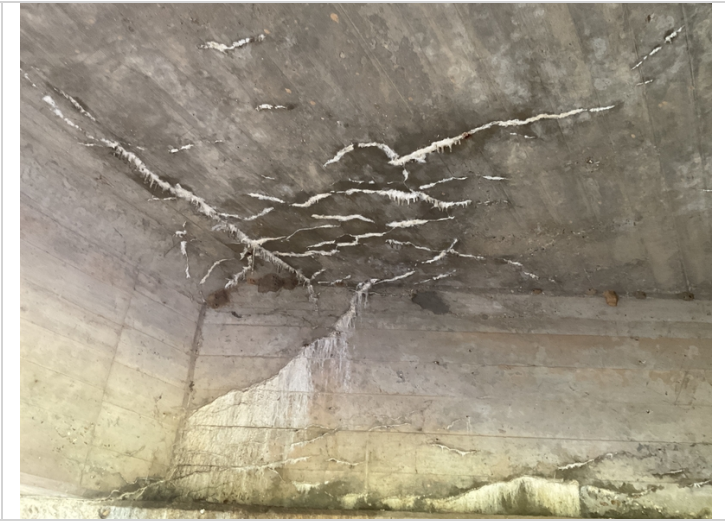
Typical cs3 map cracking with efflorescence in random locations. Bay #1 of span #3 pictured.
