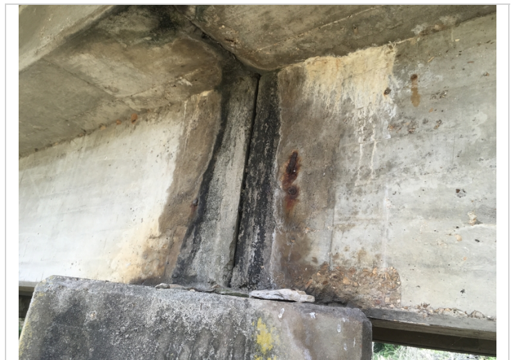
Spalling with rebar exposed at the end of beam #1 in span #2.
