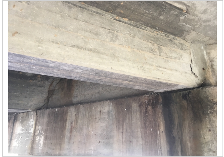
Delamination at the end of tee beams #2,3 at the end of span #1.
