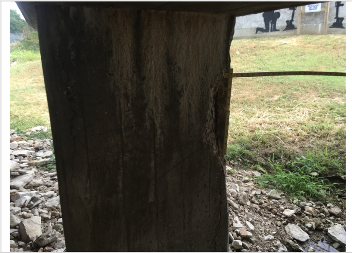
Spalling with rebar exposed on column #1 of bent #2.
