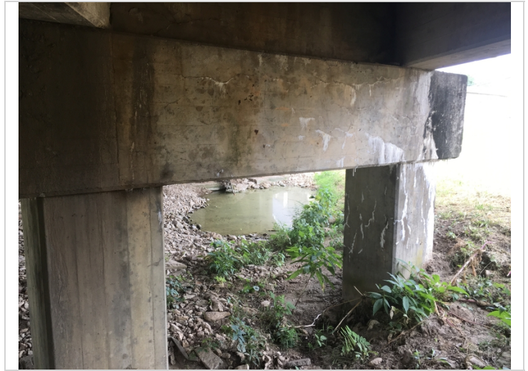
Efflorescence map cracking at the left end of bent #3 and column #1.
