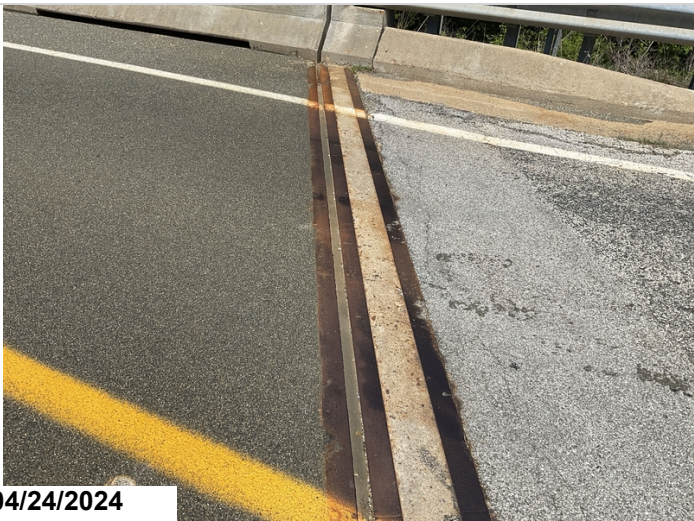
Abutment #2 seal condition. no deficiencies noted.
