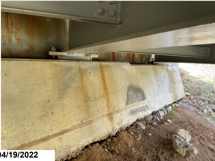
Sole plate corrosion at abutment #1.
