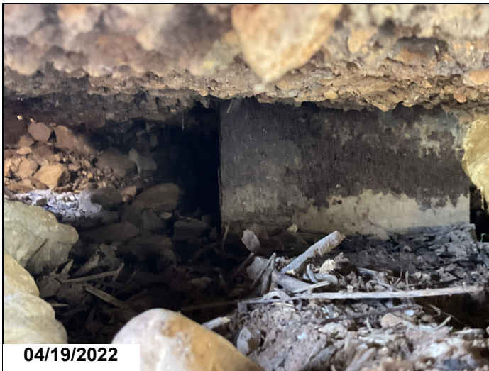
Exposed piling at abutment #1.
