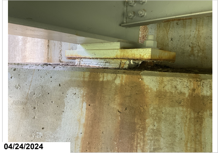
Cs3 corrosion on bearing #4 at abutment #1.
