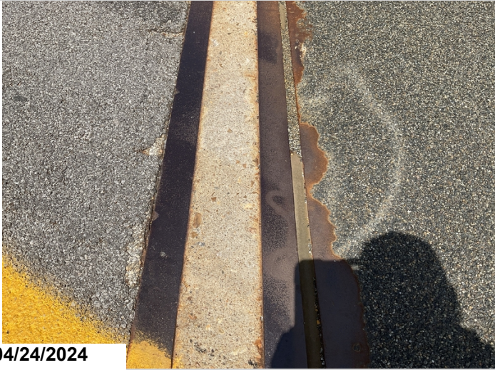
Abutment #1 pourable seal condition. no deficiencies noted.
