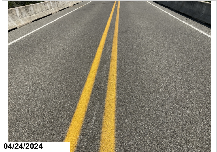
New polymer overlay condition.
