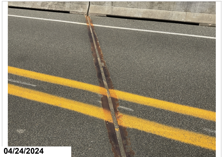
Pier #2 seal condition. no deficiencies noted.
