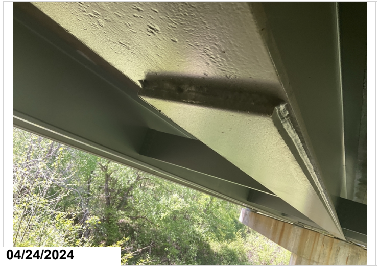
E detail. Bottom flange cover plates.
