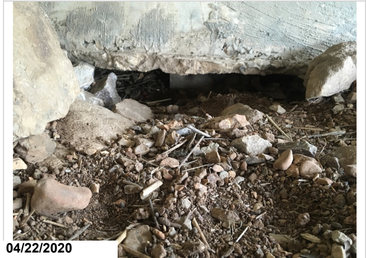
A steel pile is exposed under beam #2 at abutment #1.
