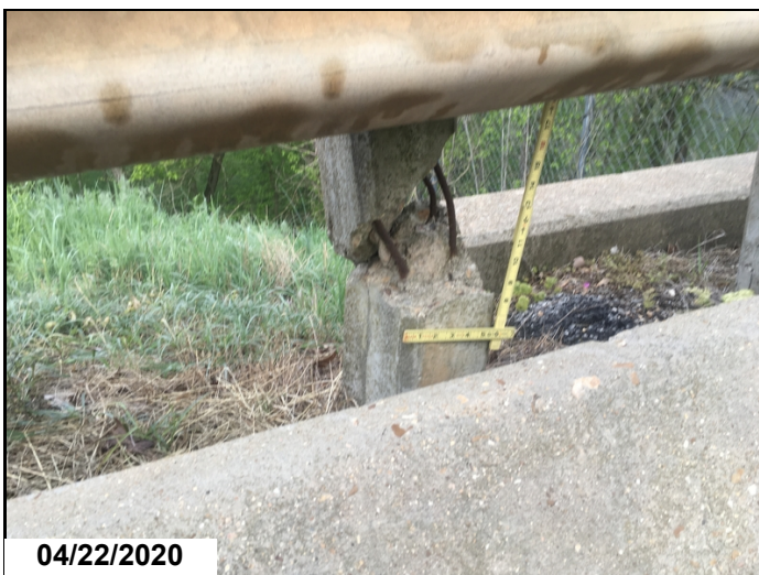
Concrete approach railing post is damaged at the left beginning of the structure.
