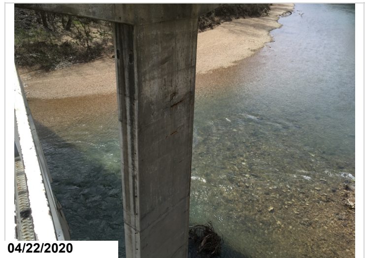
Spalling with rebar exposed on the span #3 side of pier column #2.
