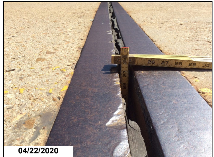
Joint seal at bents #1- #4 lose of adhesive with large portions missing.
