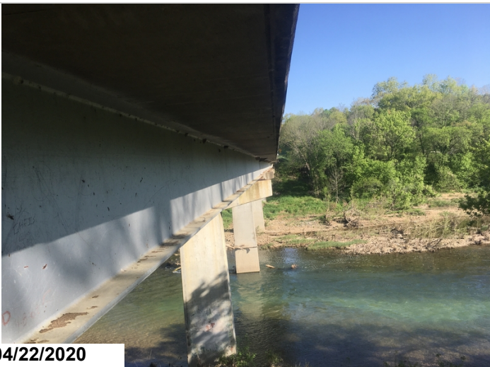
Corrosion on the top of the exterior bottom flange of beam 4 in span 1.
