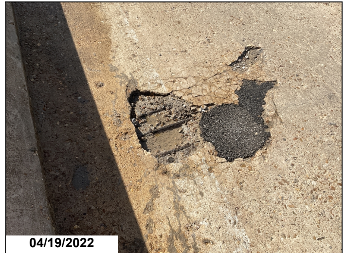
2'x1' area of pot holing with exposed rebar in span #3.
