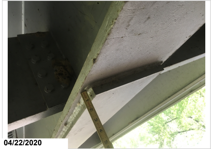
Welded cover plate detail.
