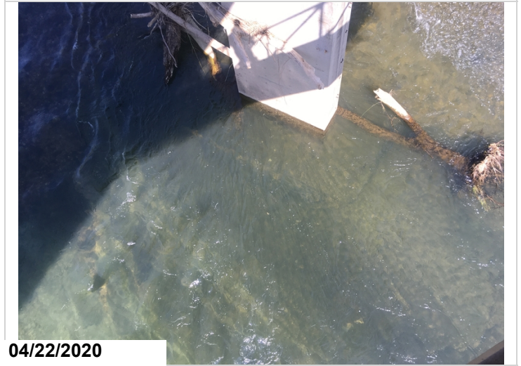
The top of the footing is exposed at pier 2. The footing is cast in solid rock.
