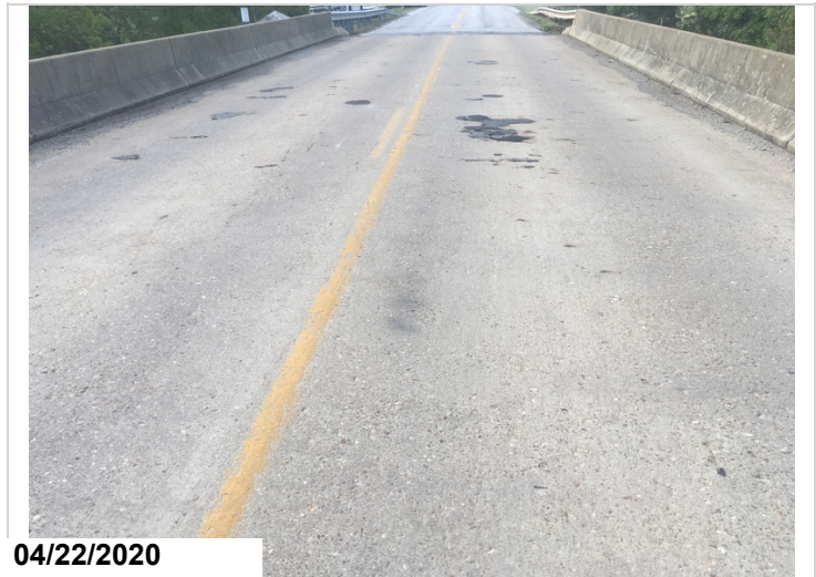
Delamination and pot holes in span 1.
