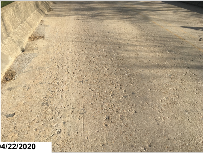
Left lane of span 5 showing scaling and delamination.
