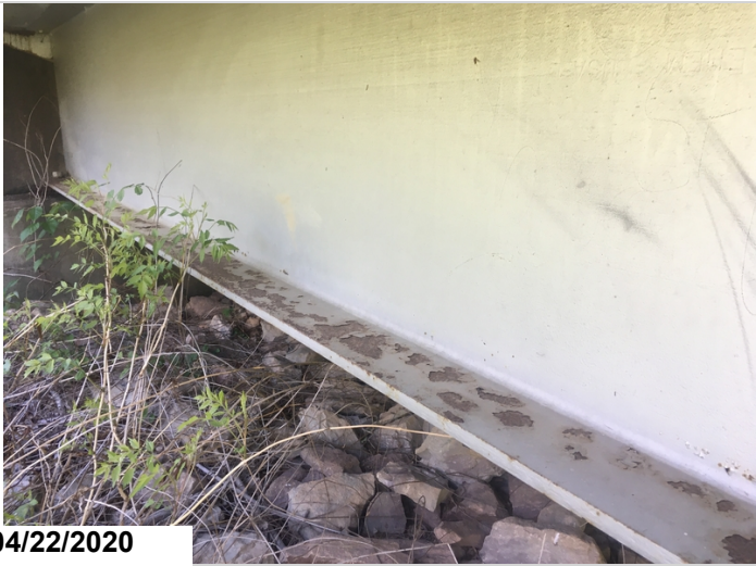
Flaking paint with minor corrosion on the exterior bottom flange of beam 1 in span 5.
