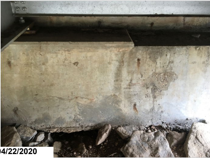
Area of map cracking with a shallow spall in bay #1 of abutment #1.
