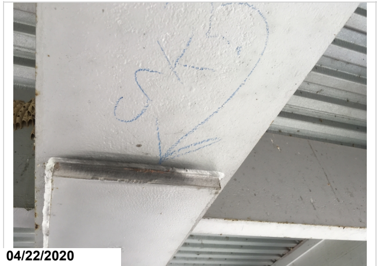
Possible crack or slag inclusion at beam #3 span #5 at the beginning of the cover plate. Will monitor.
