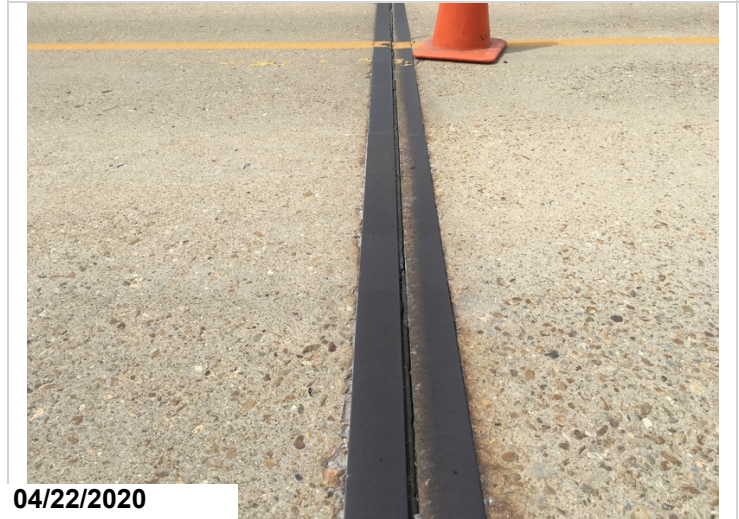
Joint seal over pier #2 is nearly adjacent.
