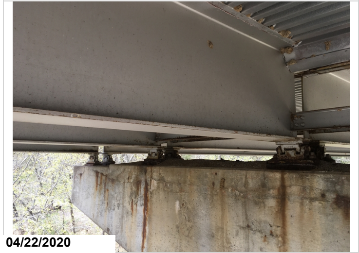
Beam end condition at pier #3.
