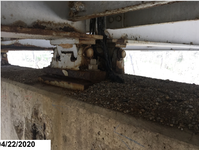
bearing condition at pier #1. Typical of all 4 moveable and all 4 fixed at this location. Note the build up on the cap due to missing joint seal.
