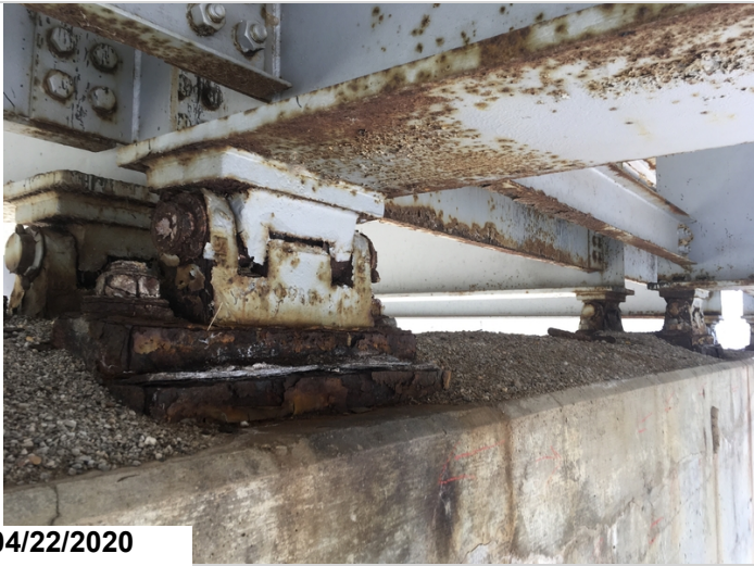
Bearing condition at pier #3. Typical of all 8 moveable bearings at this location.
