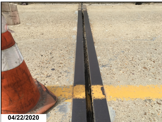
Abutment #1 joint seal condition
