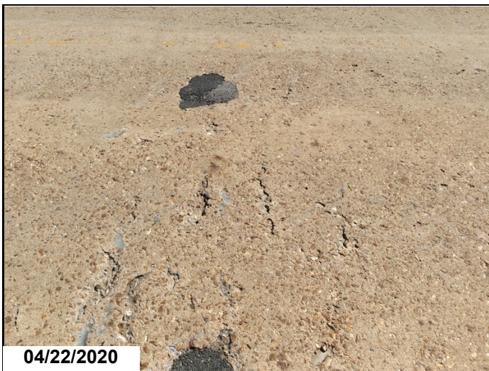
Heavy - moderate deck scaling in span #3
