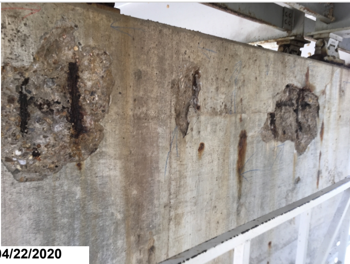
Spalling with rebar exposed on the span #1 side of pier cap #1.
