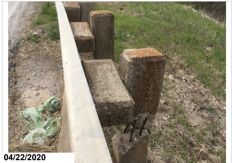
Concrete post damage at the left beginning transition railing.
