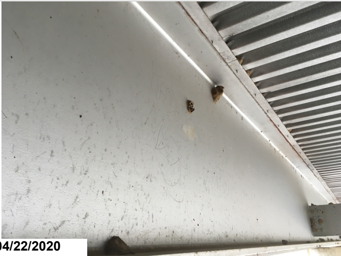
Typical paint condition of the superstructure. Loss of gloss with no chalking.
