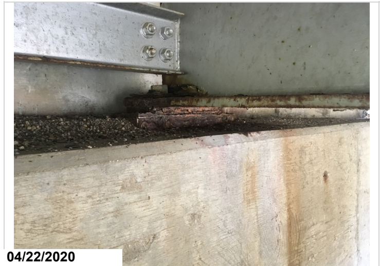
Fixed bearing condition at abutment #2. All 4 have heavy corrosion with flaking rust.
