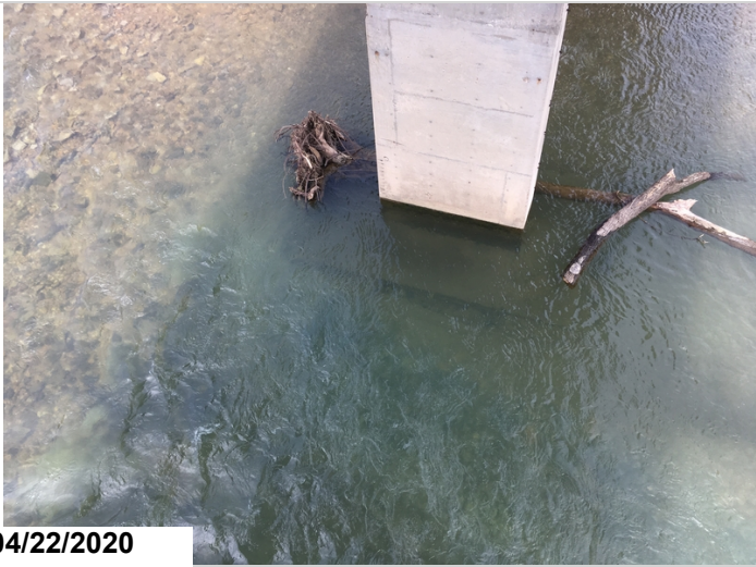
The top of the pier #2 footing is entirely exposed with 4" of vertical face exposed.
