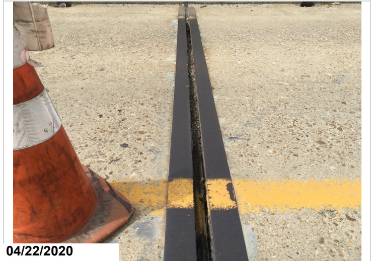
Dislodged joint seal condition. Typical over the piers.
