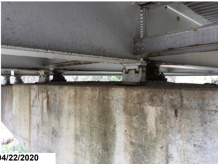
Bearing condition at pier #4. Typical of all 4 moveable and all 4 fixed bearings at this location.
