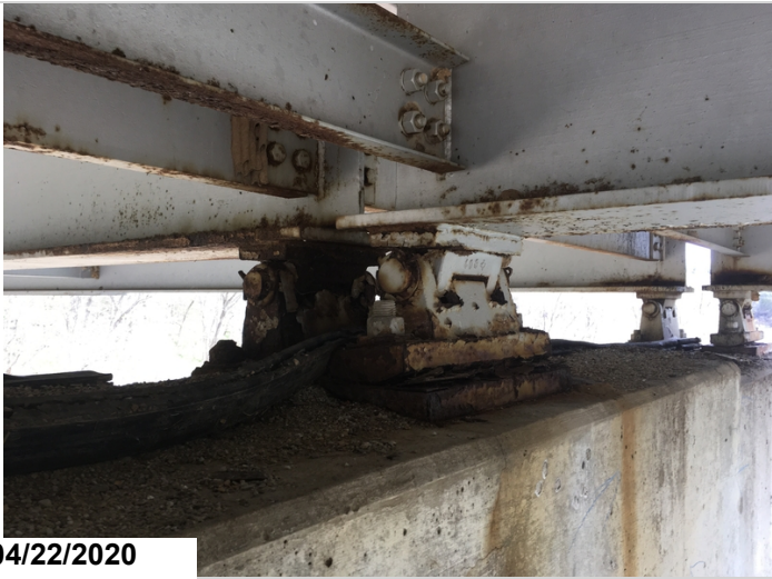
Bearing condition at pier #2. Typical of all 4 fixed and all 4 moveable bearings at this location. Note the joint seal on the cap.
