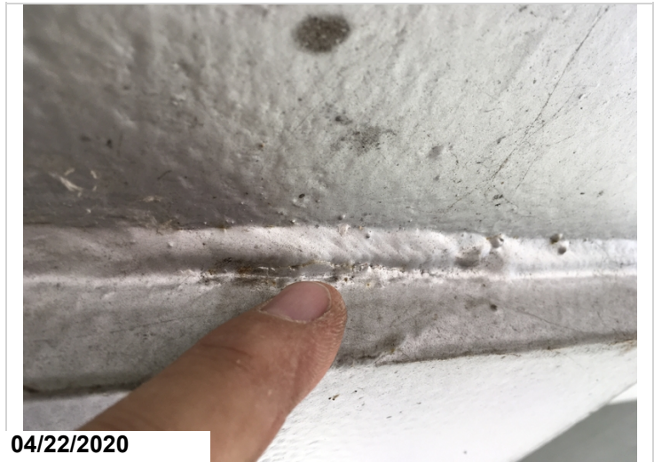
Possible crack or slag inclusion at the end of the cover plate on beam #3 span #5 at the beginning of the plate. Will monitor.
