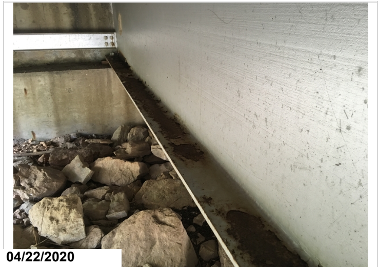
Corrosion on the top of the bottom flange of beam #2 at abutment #2 for 25'
