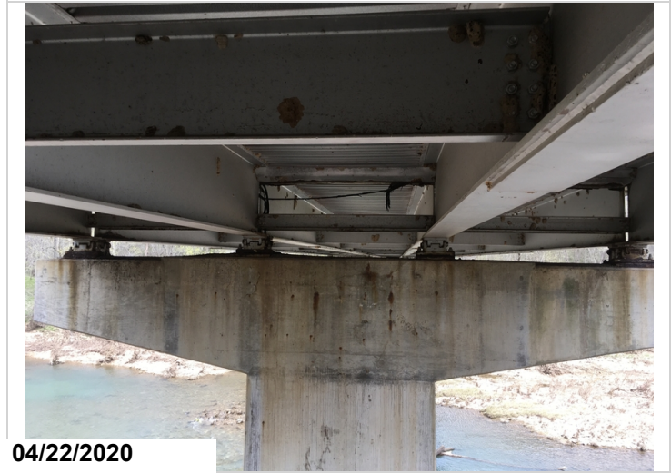
Pier #1 cap condition. Note the joint seal hanging in bay #2.
