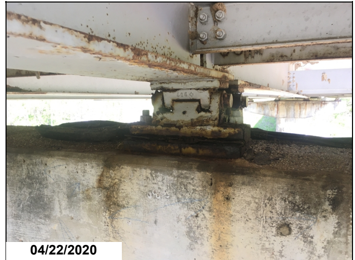
Bearing and beam end condition at pier 2. Note the joint seal and build up on the cap.
