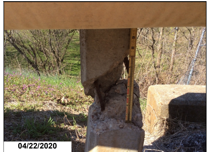
Beginning bridge 2nd guardrail post left side broken
