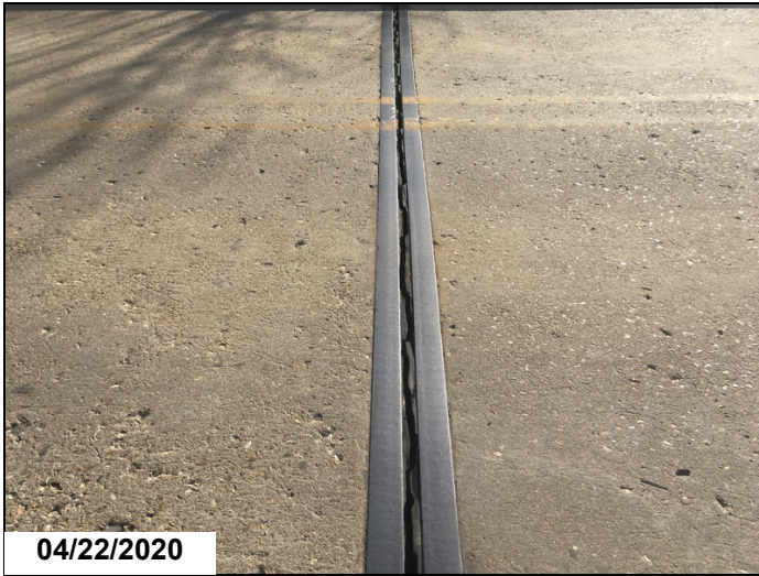
Pier 4 joint condition. Completely in cs4 leakage.
