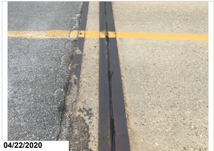
Abutment #1 compression joint seal condition. Showing cracking.
