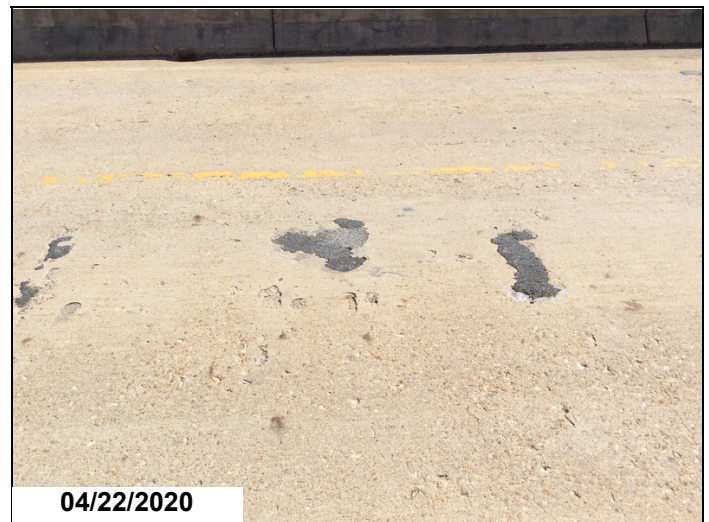
Moderate deck scaling in span #1
