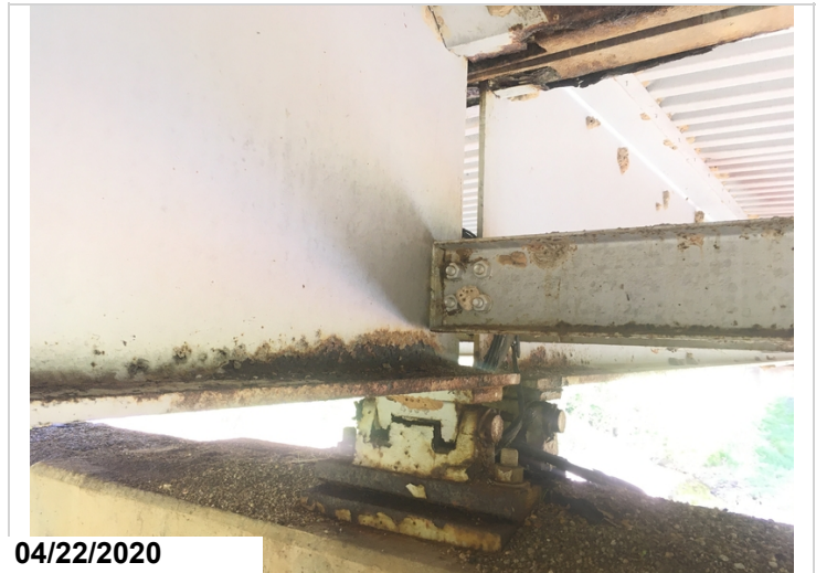
Beam end and bearing condition at pier 1
