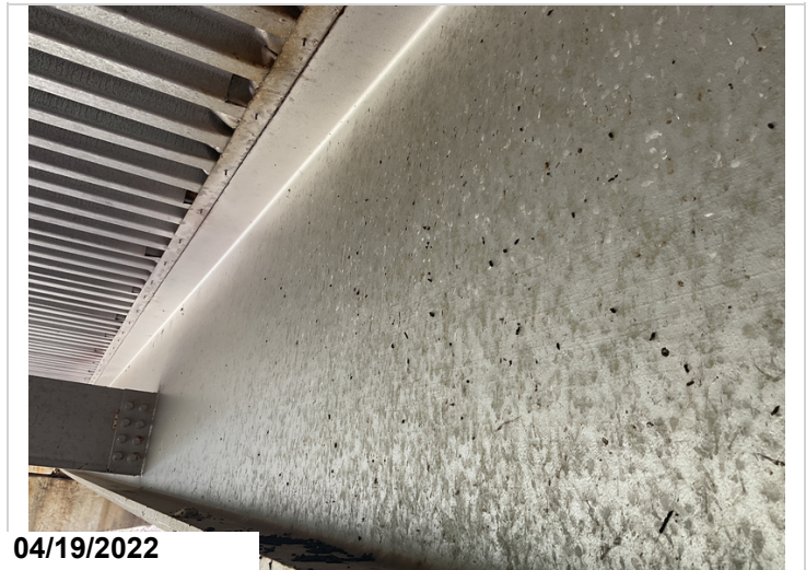
Paint condition on the interior beams.
