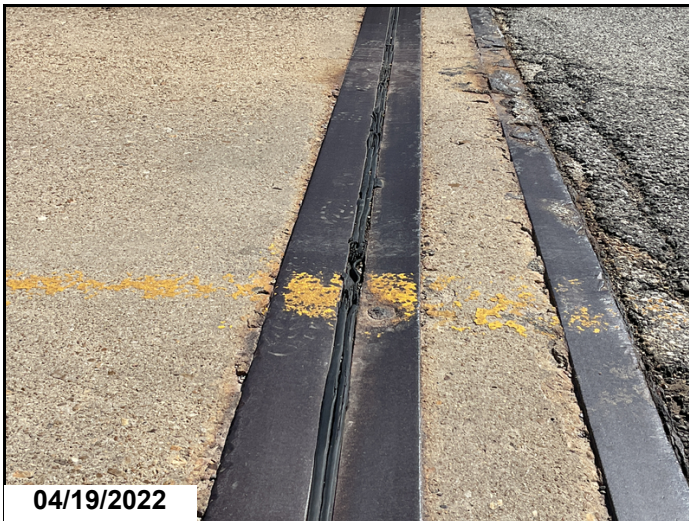
Abutment #1 joint seal condition
