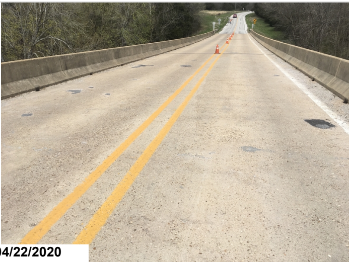
Pot holes and delamination in both lanes of span #3.
