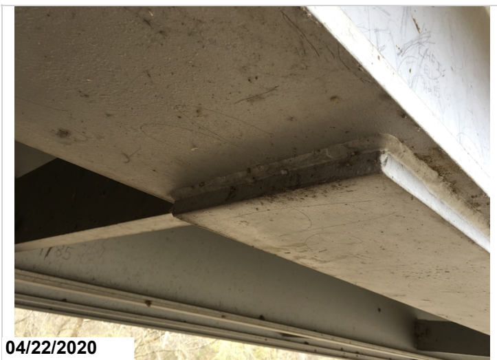
The cover plates are cut square with the bottom flange and welded in all locations.
