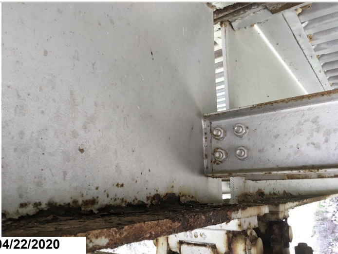
Beam end condition of beam #2 at pier #4. Typical of beams #2,3. Worst case condition at this location.
