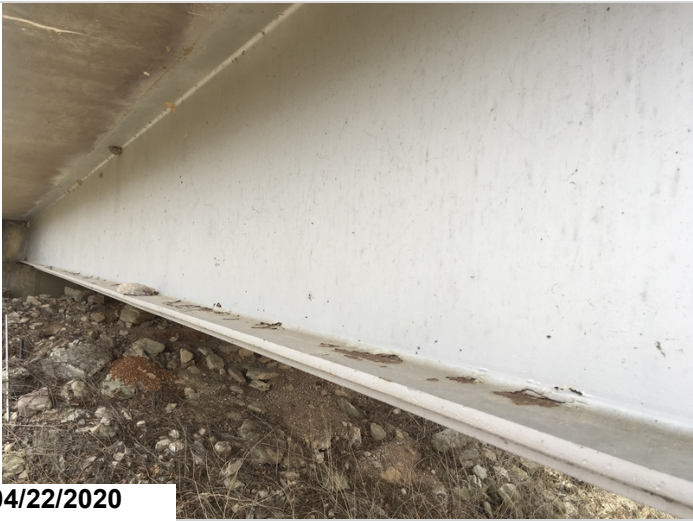
Flaking paint with general rusting on the bottom flange of beam #4 in span #1.
