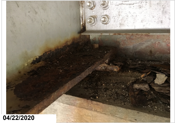
Heavy corrosion and the anchor bolt nut is missing at beam #3 abutment #2.
