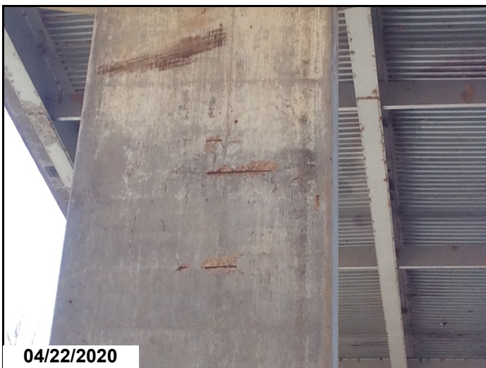
Exposed rebar back side bent #2 column
