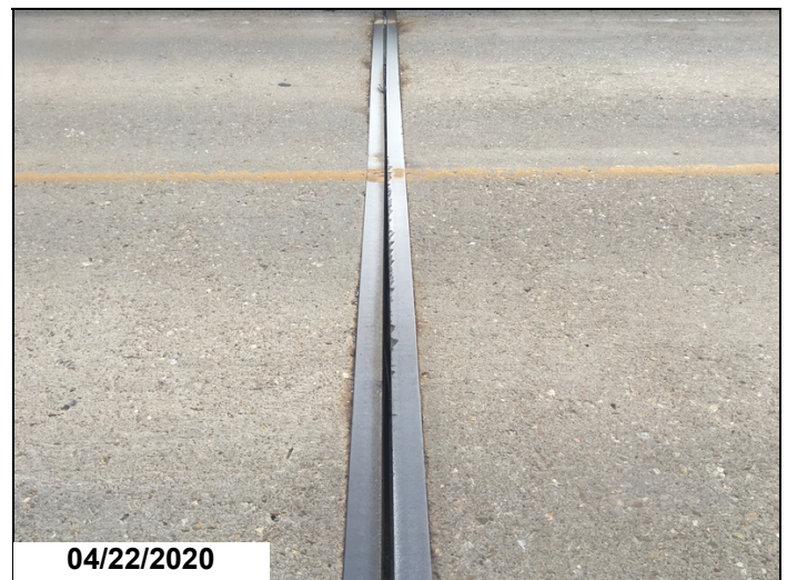
Pier 1 joint seal condition.
