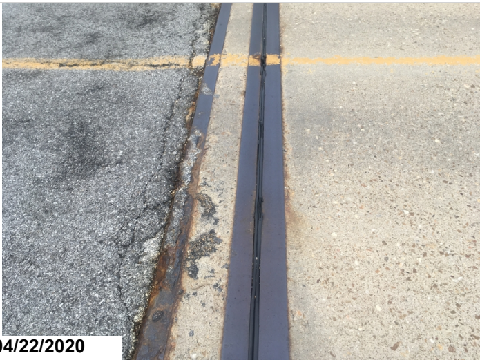
Abutment 1 joint seal condition.
