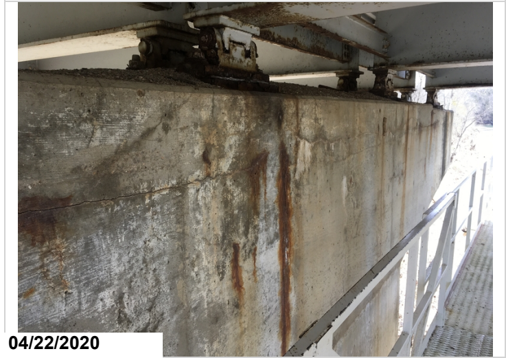
Pier cap #3 condition. Showing horizontal cracking for the full length. This area does not sound hollow under hammer blows.
