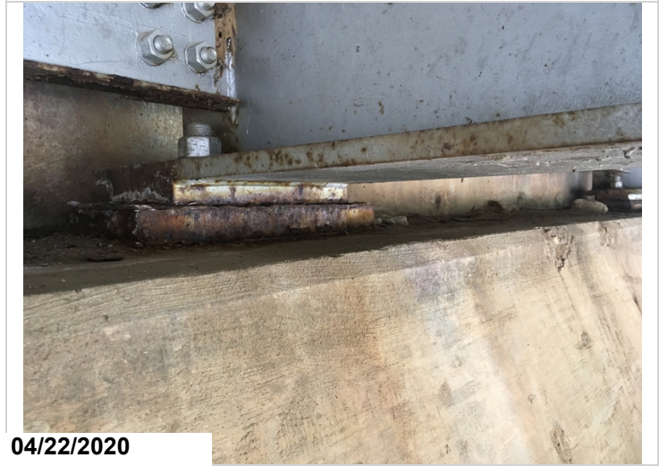
Fixed bearing condition at abutment #1. Typical of all 4 at this location.
