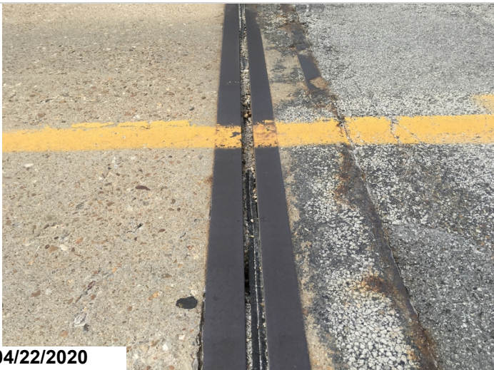
Compression joint seal condition at abutment #2. Showing loss of adhesion and debris impactation.
