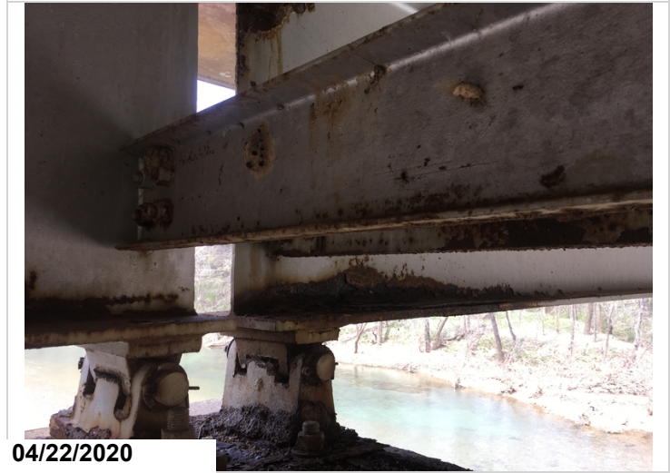
Beam end condition over pier #1. Typical of both outside beams 8' of corrosion. The inside beams have corrosion for 3'.
