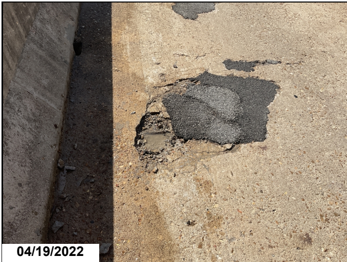
Pot hole with exposed rebar in the right lane of span #3.
