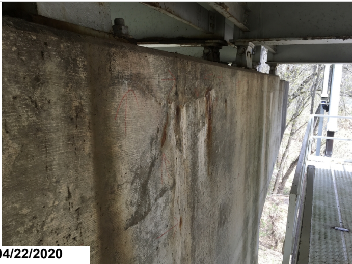
Pier #4 cap condition. Showing horizontal cracking that has begun to leach efflorescence and rust staining.
