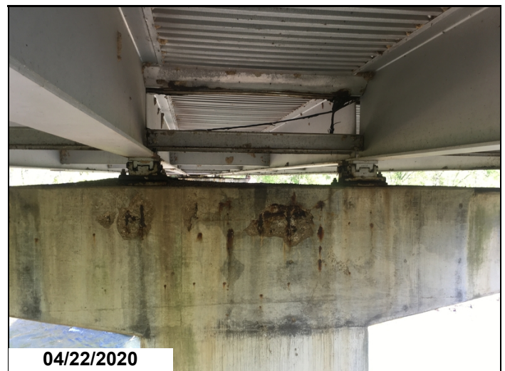
Spalling on the span 1 side of the cap with rebar exposed. Note the joint seal condition.
