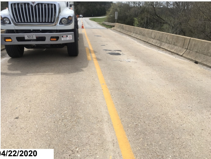
Patched areas in the left lane of span #1
