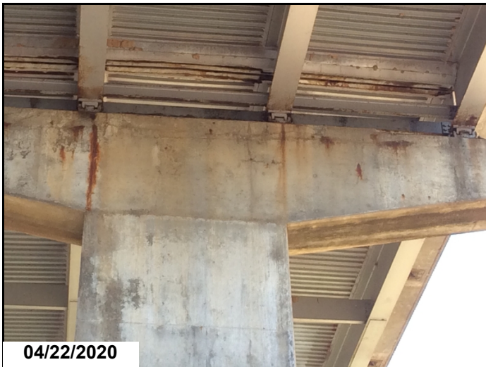
Ahead side of bent #3 cap rust stained cracking under girders #2 and #3
