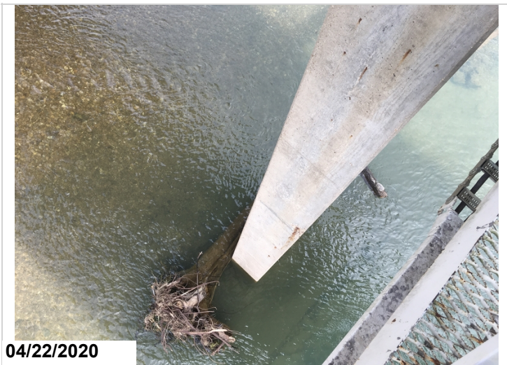
Spall with rebar exposed on the left face of pier column #2.
