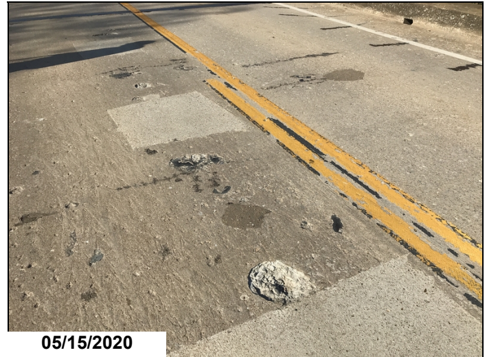
Deck span #13 left lane adjacent to centerline approximately 22' north of bent #13 basketball sized spall. Spall is approximately 2" deep at deepest point.
