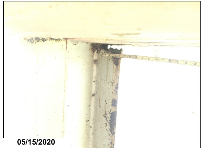
Bent #8 steel piling #3 ahead flange right side has complete section loss approximately 4" wide and 1" tall at the concrete cap juncture.
