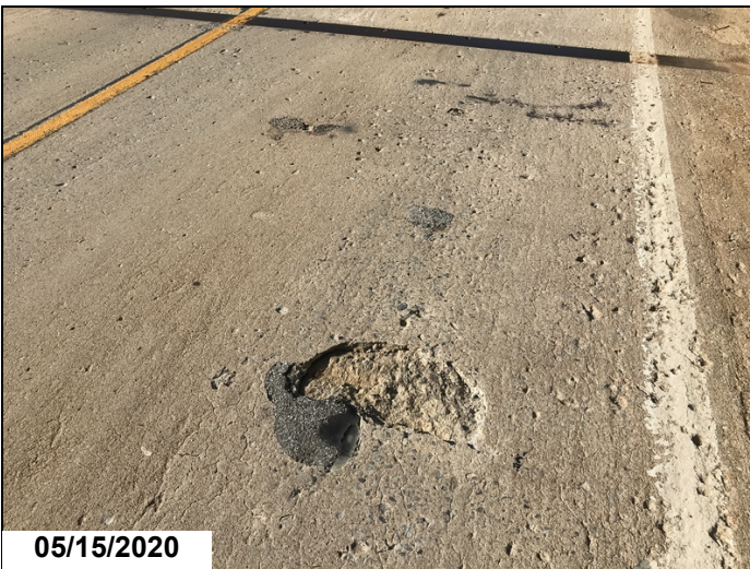
Deck Span #3 right lane spalling with steel exposed 10' north of bent #3.
