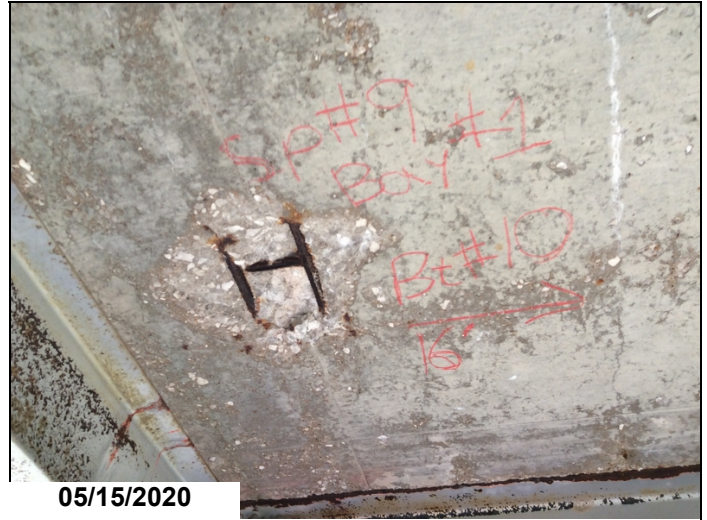
Span #9, bay #1-Spalling with exposed reinforcing steel.
