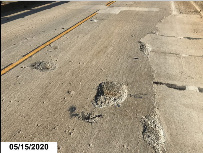
Span #2 right lane multiple spalls some with steel exposed.
