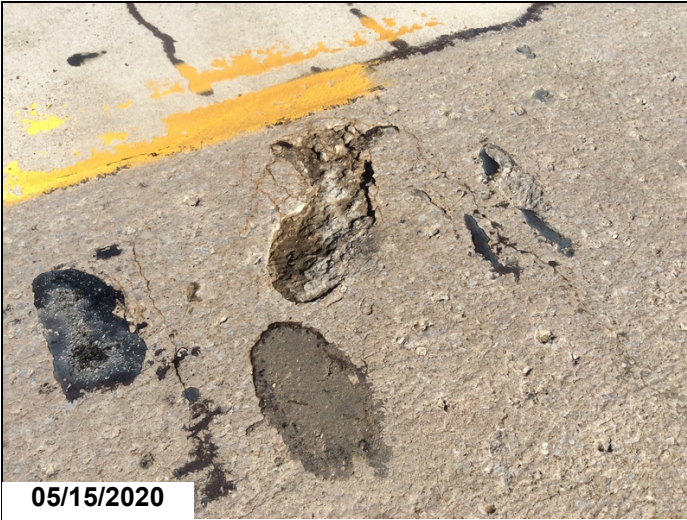
Span #7-Spalling.
