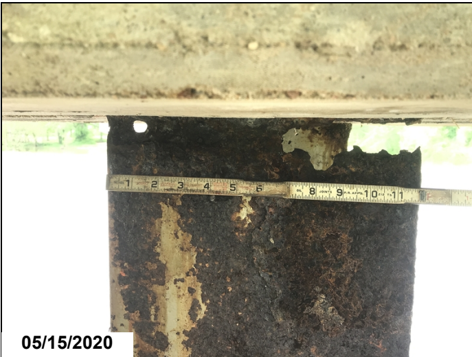
Bent #8 steel piling #4 behind flange right and left side has areas of complete section loss.
