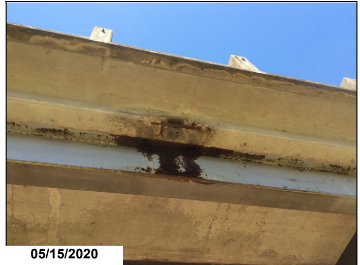
Typical spalling with steel exposed around deck drains.
