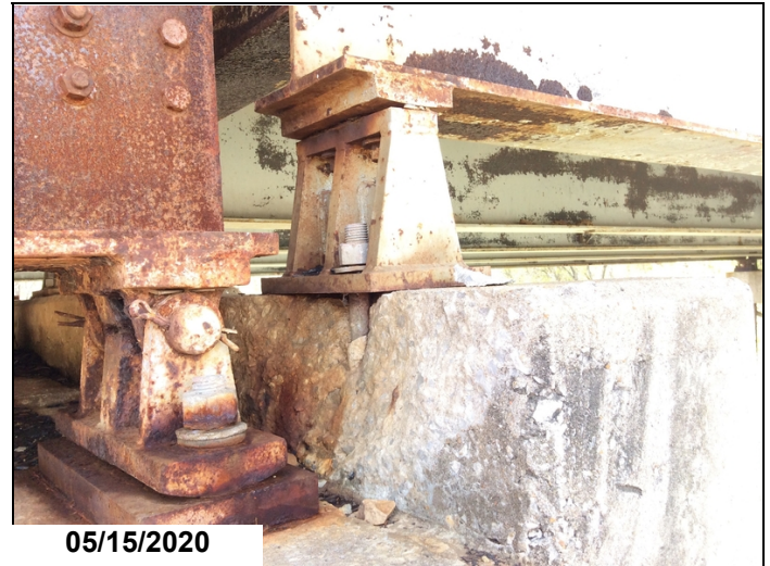
Bent #9 Span #8 bearing #1 - has loss of bearing area.
