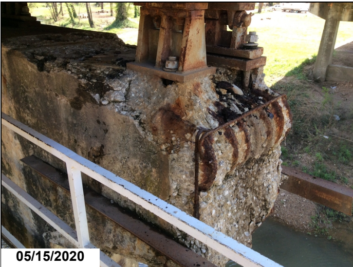
Bent #11 bearings #5 in spans #11 and #10 - have loss of bearing area and structural steel exposed.
