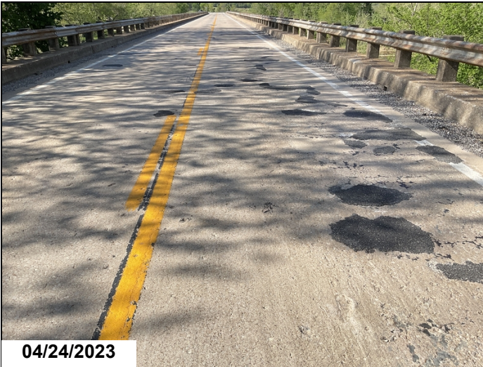
Span #6 asphalt patches
