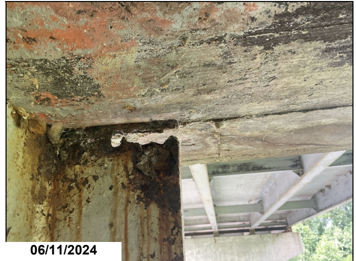
3" long by 3/4" tall rust hole at the top of pile #3 at bent #8.
