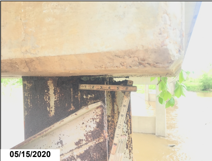
Bent #8 steel piling #5 behind flange right side complete section loss adjacent to concrete cap. Section loss area 3" x 1"
