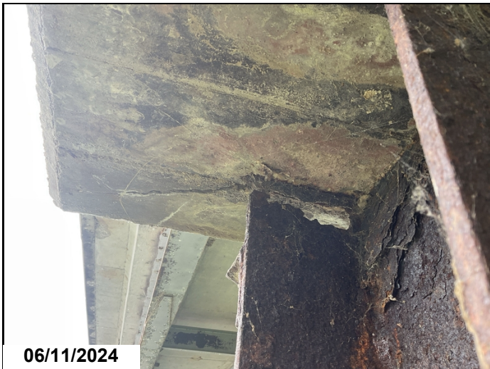
6" long by 1.5" wide rust hole on the top left flange of pile #1 at bent #8.
