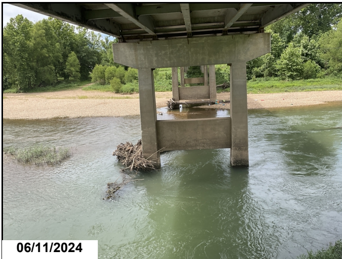
Drift accumulation on bent #9.
