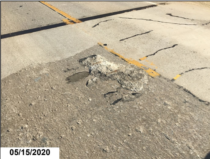
Deck span #10 left lane adjacent to centerline approximately 5' north of bent #10 large spall with steel exposed. Spall is approximately 3" deep at deepest point.
