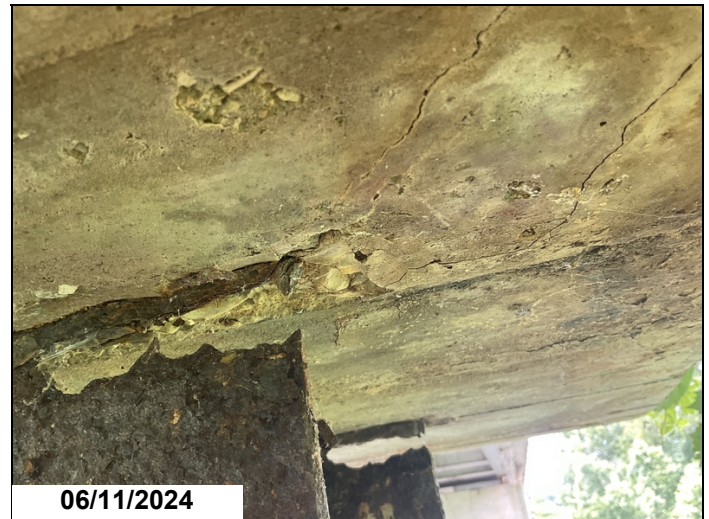
3" long by 1/2" wide rust holes at the top right side of pile #5 at bent #8 on the span #7 and span #8 sides.
