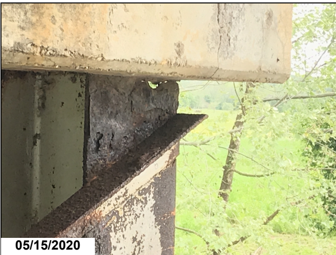
Bent #8 steel piling #1 ahead flange left side complete section loss adjacent to concrete cap. Section loss area 3" x 1"
