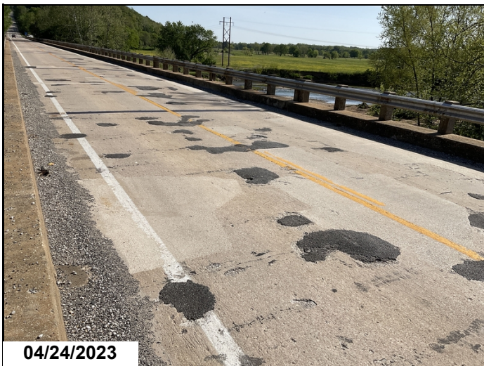
Spans #13 and #14 asphalt patches
