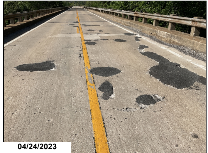
Span #2 asphalt patches
