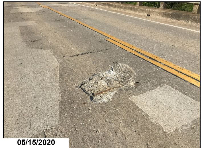
Deck span #12 left lane adjacent to centerline approximately 33' south of bent #11 large spall with steel exposed. Spall is approximately 1.5" deep at deepest point.
