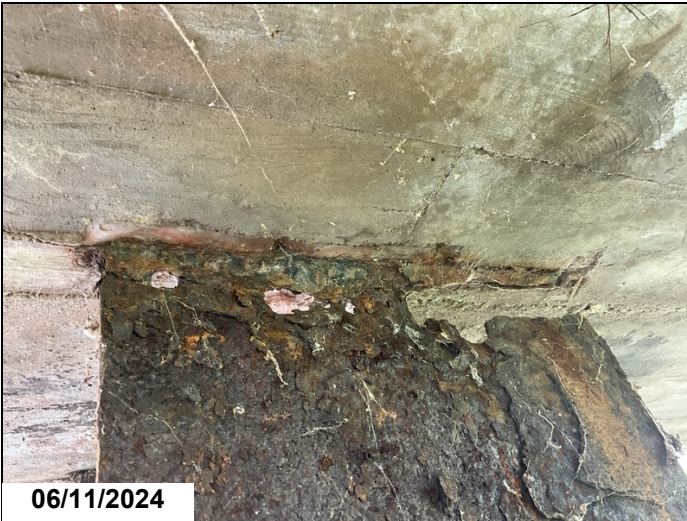
Full width flange rust hole on the span #7 side of pile #4 at bent #8.
