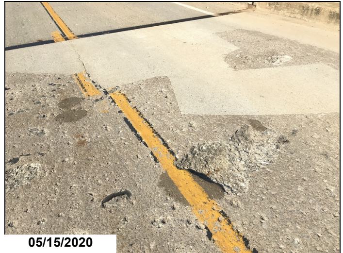
Deck Span #11 right lane adjacent to centerline spalling with steel exposed approximately 10' north of bent #3.
