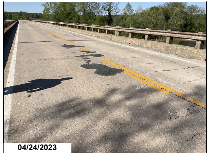
Span #8 asphalt patches
