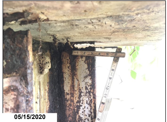
Bent #8 steel piling #5 ahead flange right side complete section loss adjacent to concrete cap. Section loss area 3" x 1"
