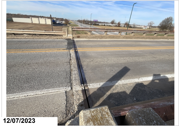
View of abutment #2 joint missing joint material
