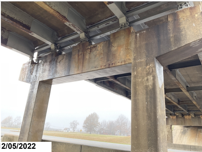
View of bent #2 cap ahead side spalling with steel exposed
