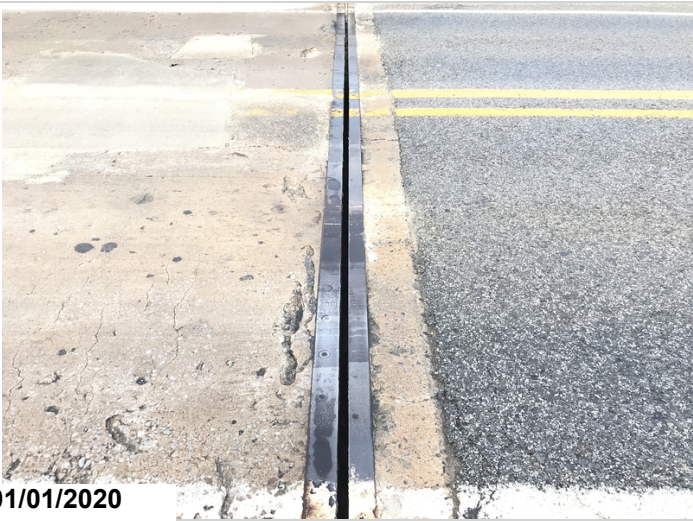
Abutment #1 expansion joint material has been displaced.
