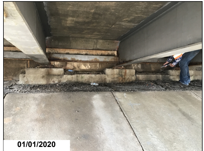
View of dirt and debris build up at abutment #2 due to open joint.
