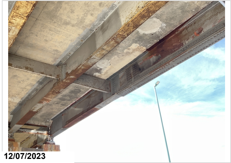
Span #2 girder #5 retrofit bolted repair
