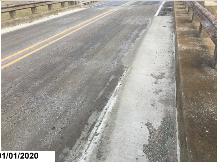
Deck Span #1 left gutterline patch repair
