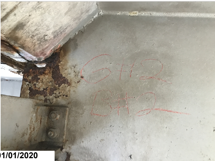
Girder #2 in span #3 over bent #2 completely section loss of web in haunch area.
