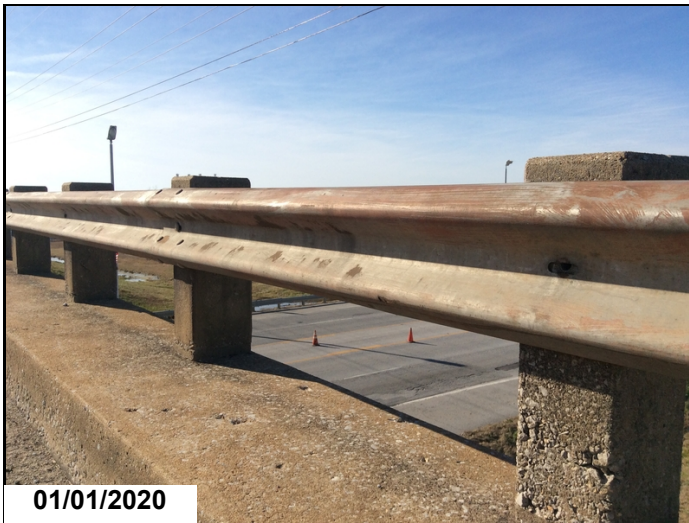
01/01/2020 Bridge rail right side span #1 - Few posts not bolted to bridge rail.
