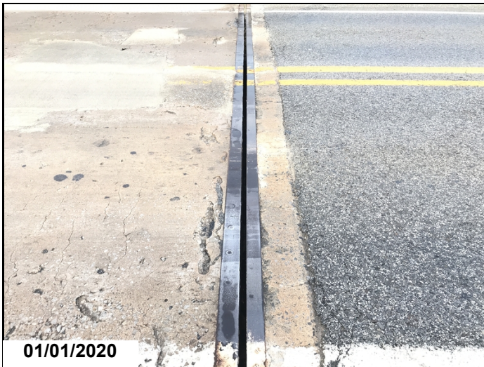
Abutment #1 expansion joint material has been displaced.
