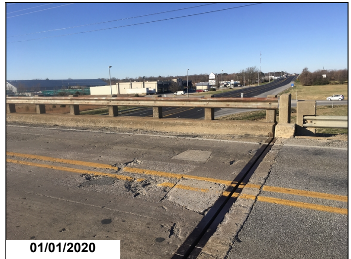
01/01/2020 3 missing bolts in guard rail span 1 right.
