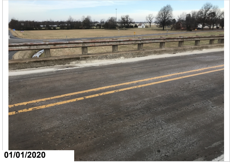
Deck Span #1 right gutterline patch repair
