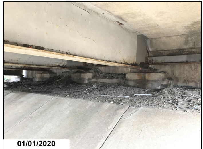
Abutment #1 dirt and debris build up.
