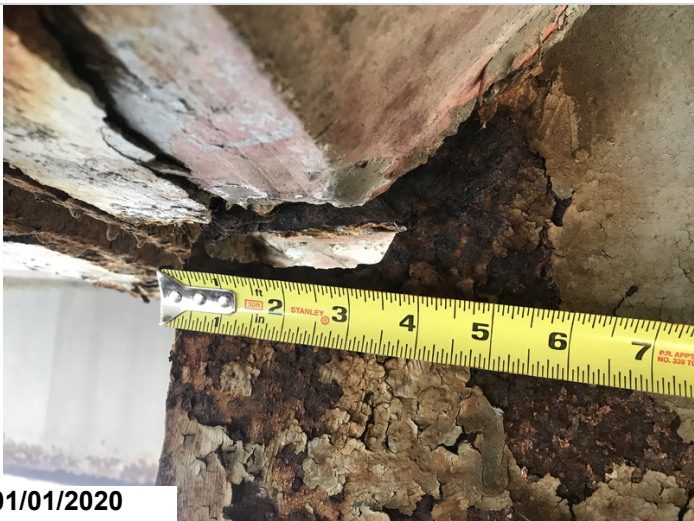
Girders #2 in span #3 over bent #2 completely section loss of web in haunch area.
