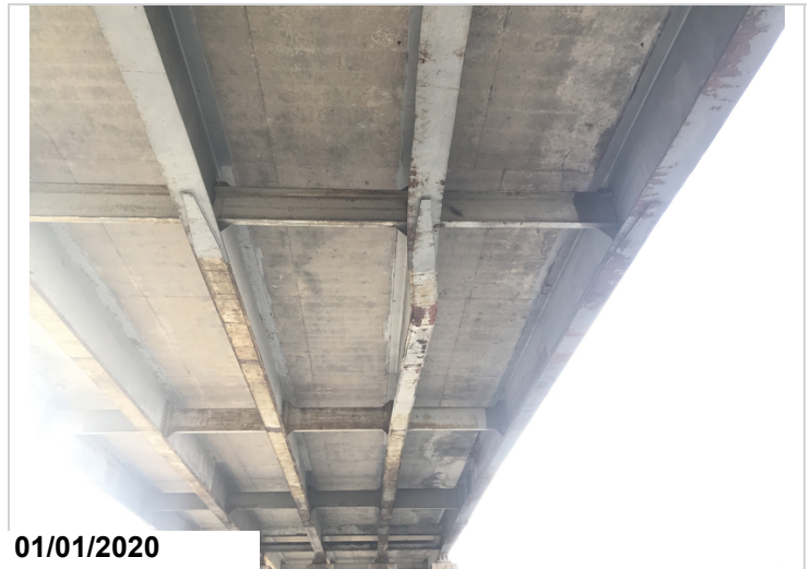
Span #2 Girder #4 out of plane bending.
