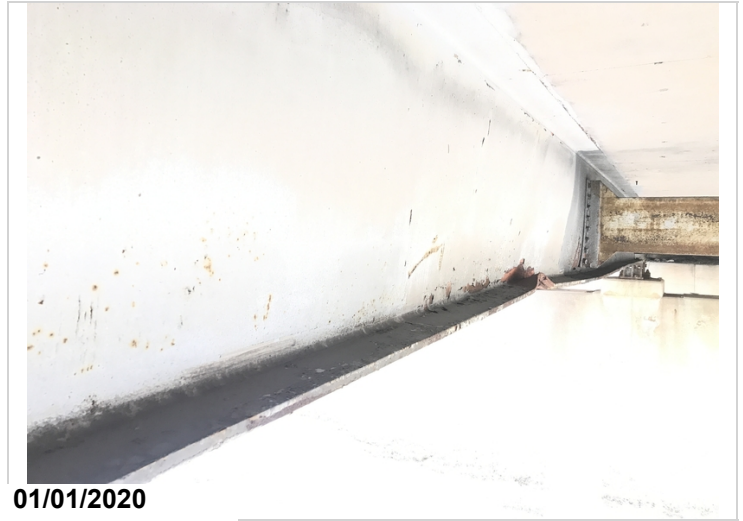
Girder #4 span #2 collision damage still exists.
