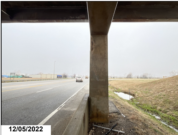
Bent #1 column #2 cracking and spalling
