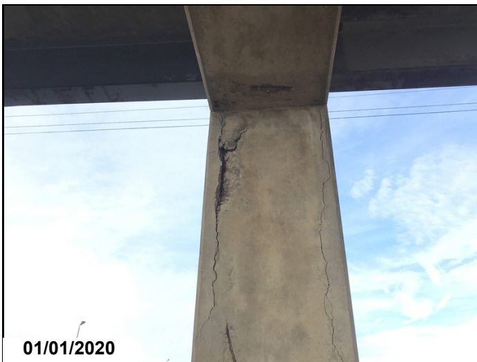
Bent #1 column #2 has spall ' with steel exposed with a vertical crack that extends down to the ground.
