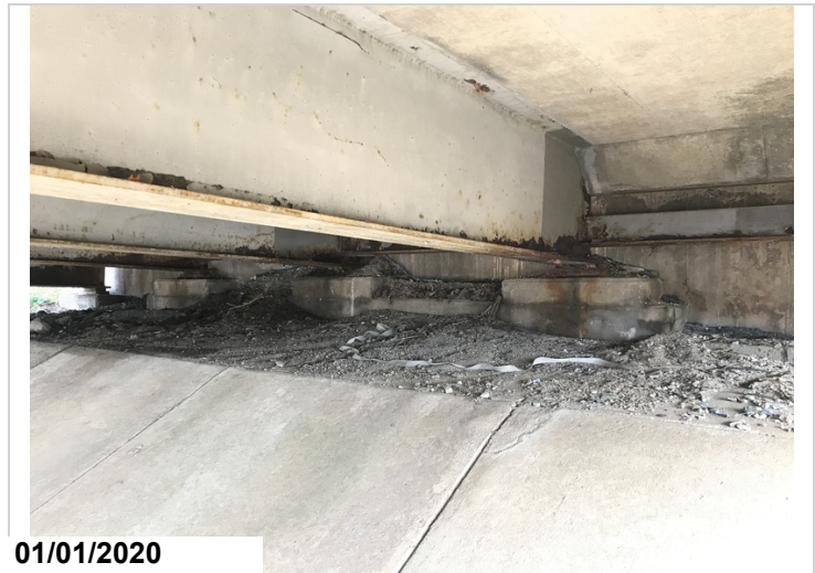
Abutment #1 dirt and debris build up.
