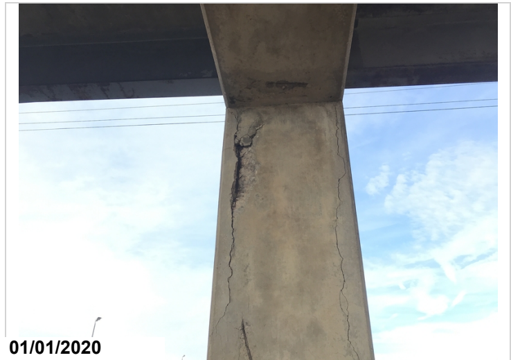
Bent #1 column #2 has spall 2' tall with steel exposed with a vertical crack that extends down to the ground.
