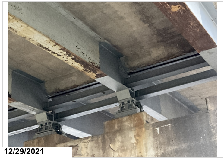
State maintenance forces have repaired haunch area with a bolted splice
