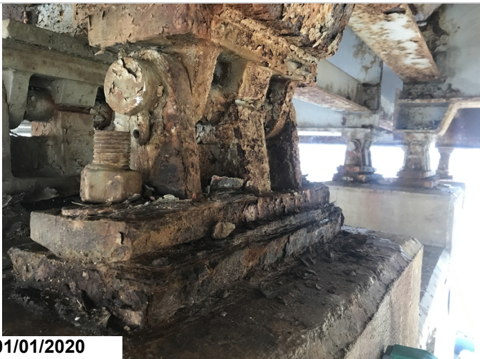
View of bearings at bent #2
