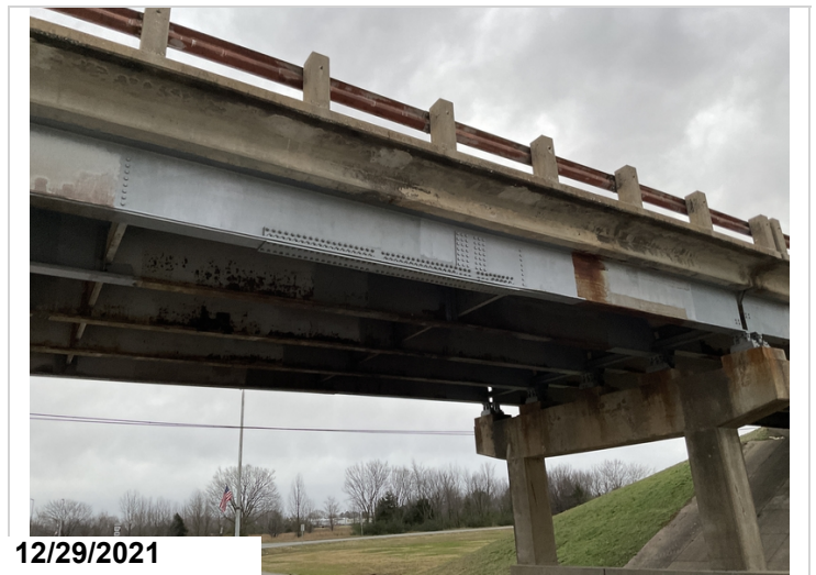
State maintenance forces have placed bolted spliced repairs
