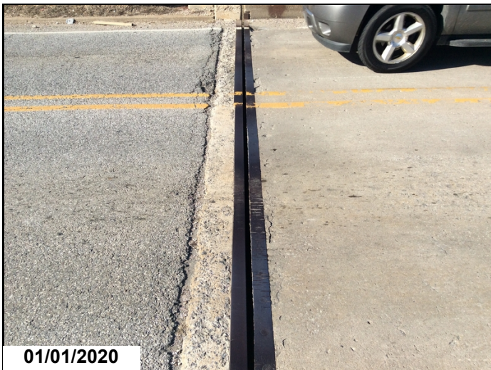
Deck bent 4 left - expansion joint missing.
