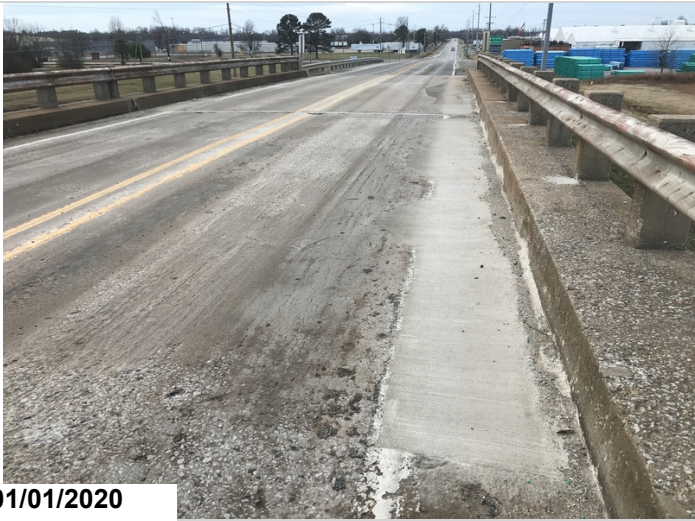
Right gutterline repairs in spans #2 and #3.
