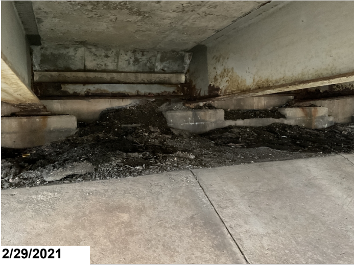
Dirt and debris accumulation at abutment #1
