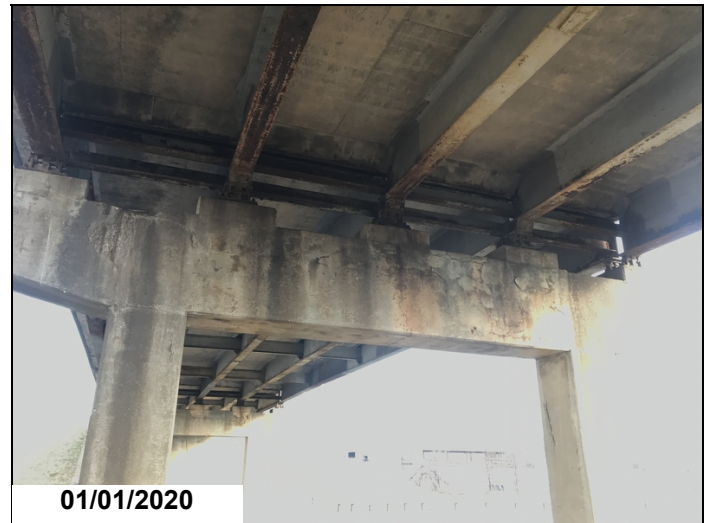
Bent #2 cap ahead side spalling steel exposed and multiple delaminated areas.
