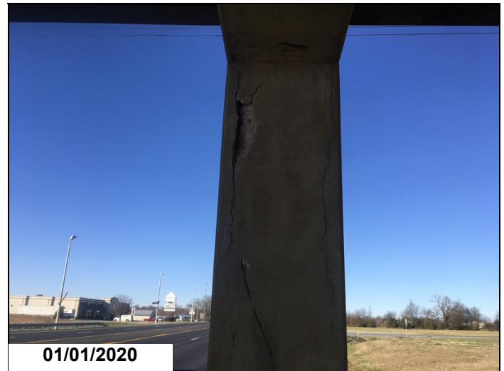
Bent 2 Column 2 spall with exposed reinforcing steel.
