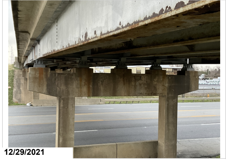
Maintenance forces have raised bridge at bearings to help combat collision to girders.
