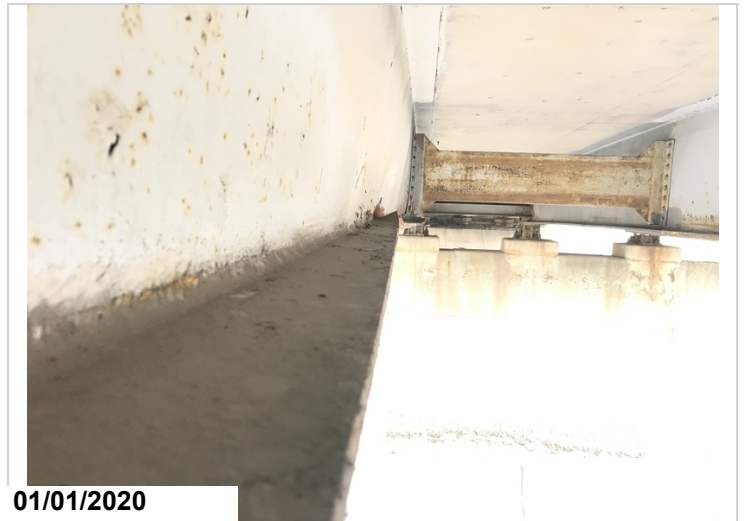
Girder #4 span #2 collision damage still exists.
