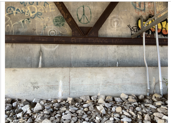
Bent 1 Efflorescence
