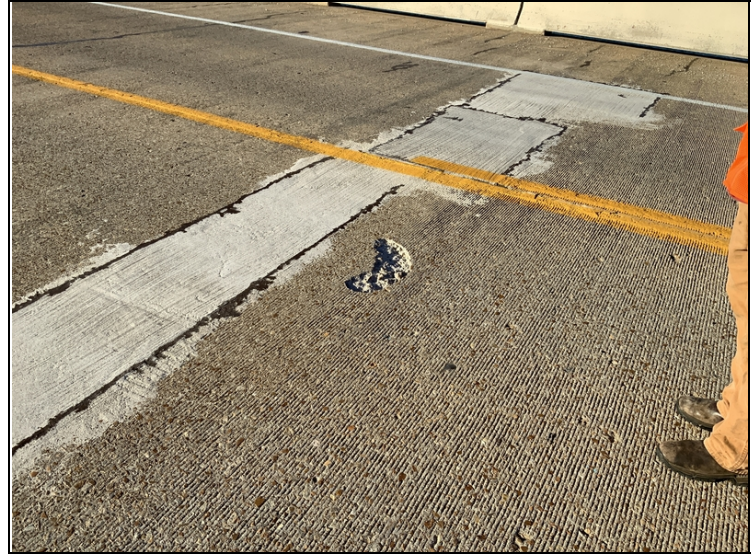
Span 12 Spalling in the right lane
