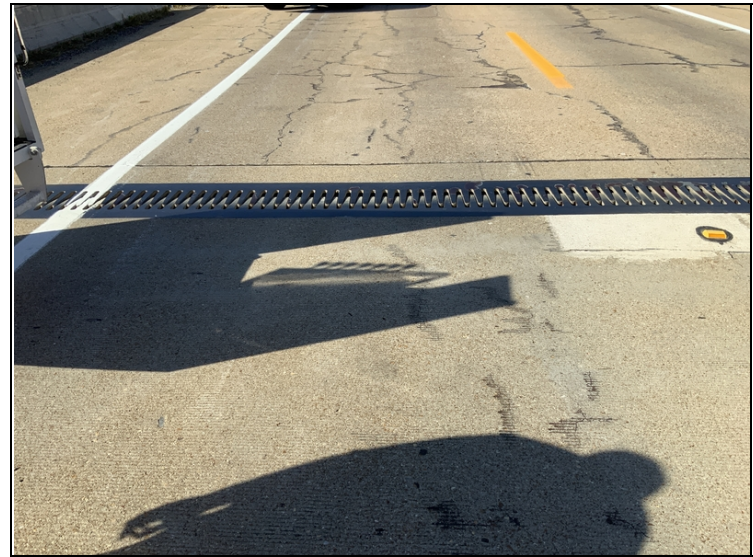
West approach finger joint raised
