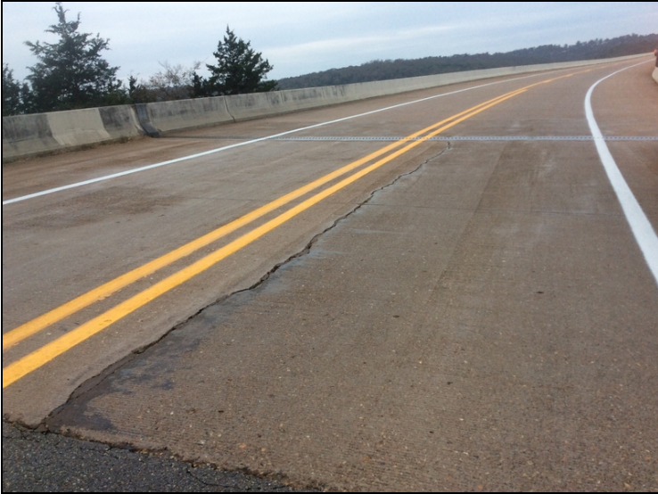
East approach longitude crack with epoxy that is cracking.
