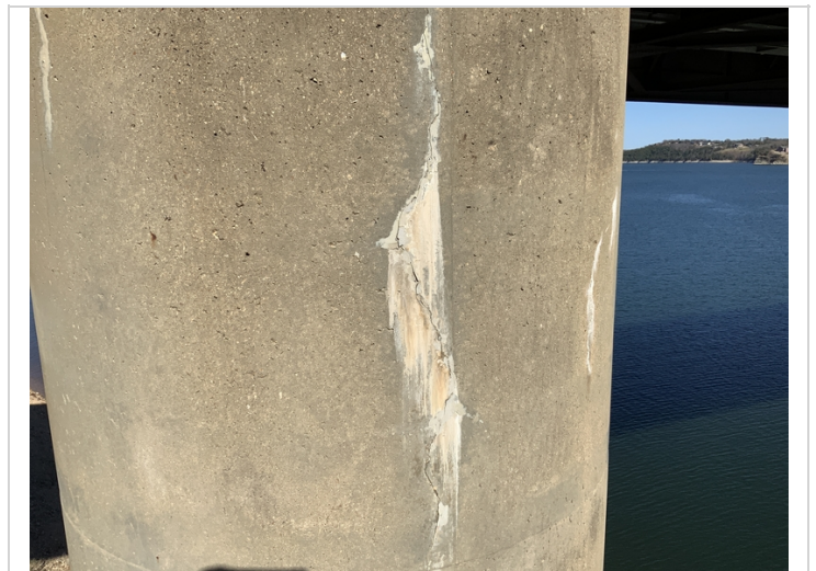
Pier 1 Crack repair failing
