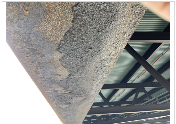
Span 8 Typical corrosion
