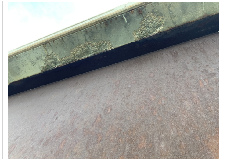
Span 3 Left and Right Spalling in undersurface
