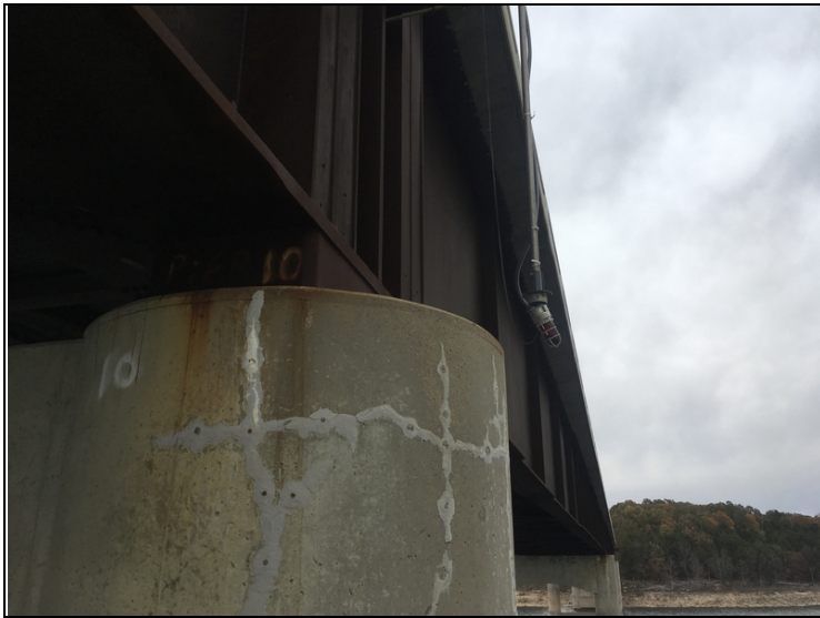
Pier 10, Right: Navigation light out.
