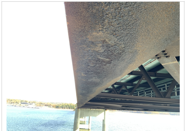
Span 3 Girder 1 Flaking rust
