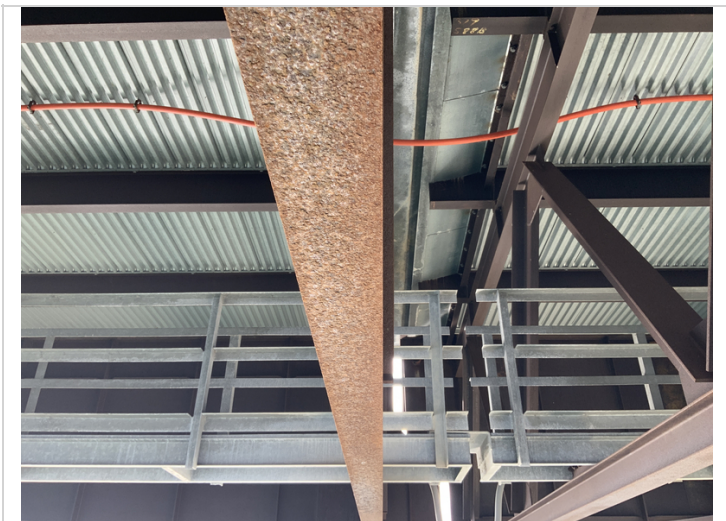
Span 8 Floorbeam 1 Bottom flange flaking rust
