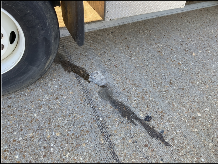
Span 14 Spalling in right lane
