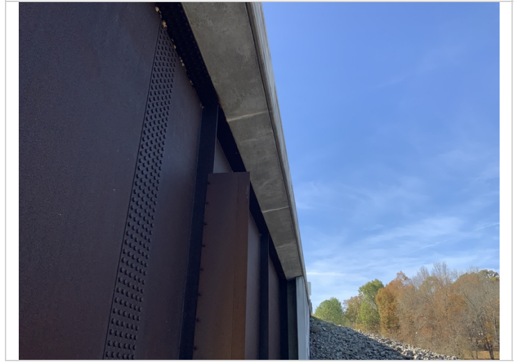
Typical efflorescence in overhangs
