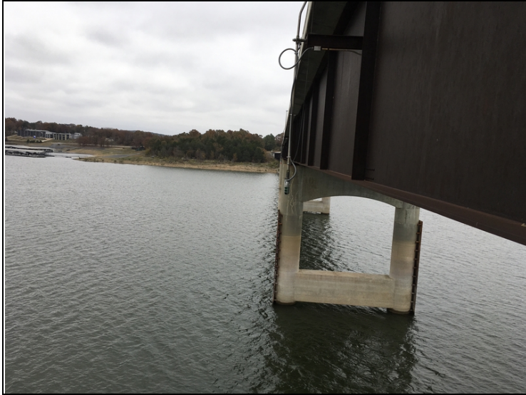
Span 9 green navigation light is out at Girder 1.
