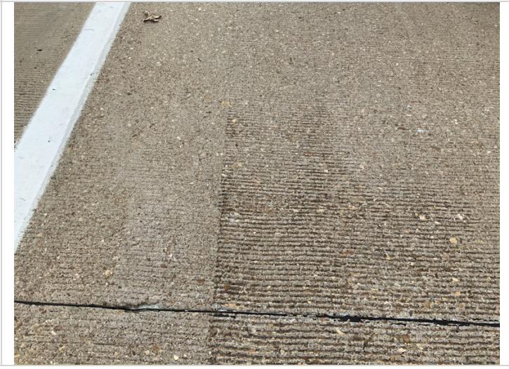
East approach sealable cracking
