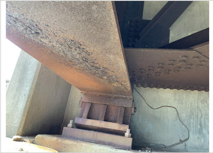
Bent 1 Girder 1 Flaking rust
