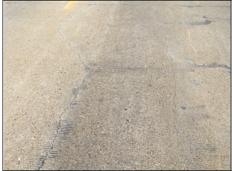
Approach Slab 1: Longitudinal cracking.
