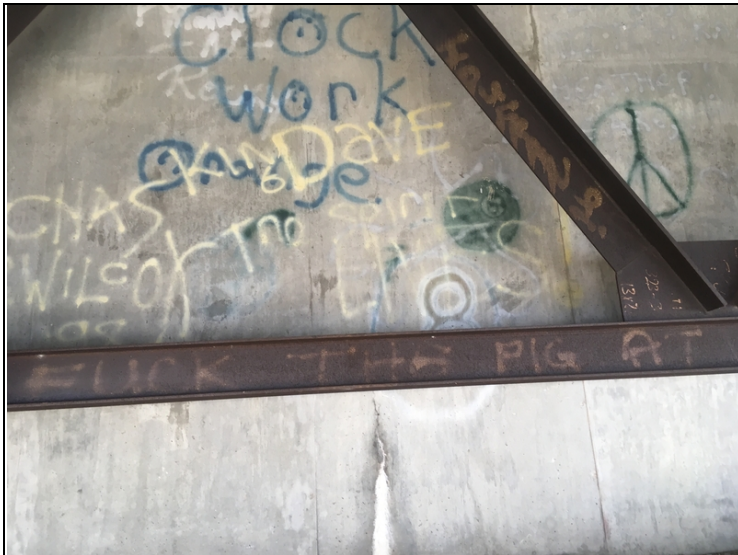
Abutment 1: Vertical cracking with efflorescence.
