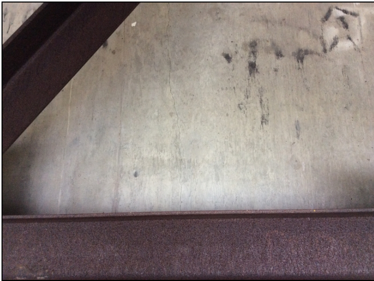
6 vertical cracks in back wall at abutment 2.
