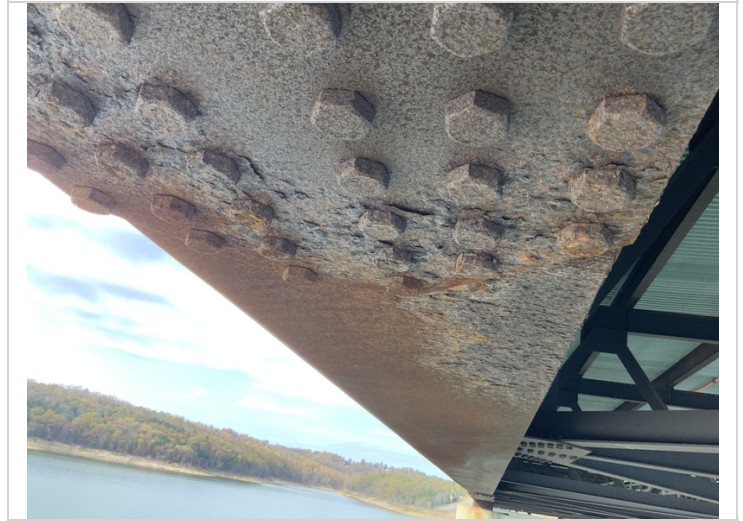
Span 9 Girder 2 Flaking rust in splice plate
