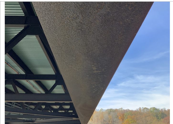
Span 2 Girder 1 Flaking rust
