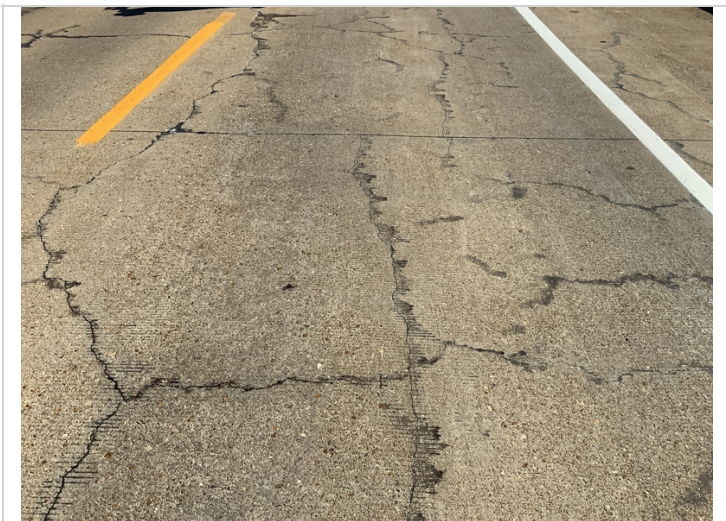
Approach slab has been sealed
