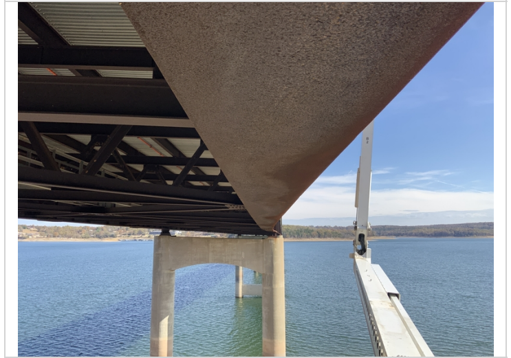
Span 1 Girder 1 Flaking rust
