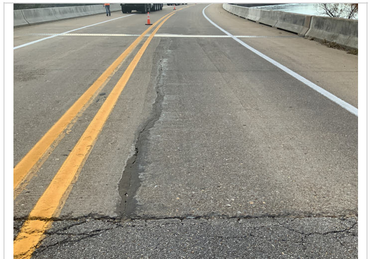
East Approach slab failing repair
