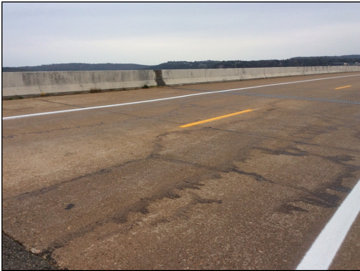
West approach has 4 longitudinal cracks
