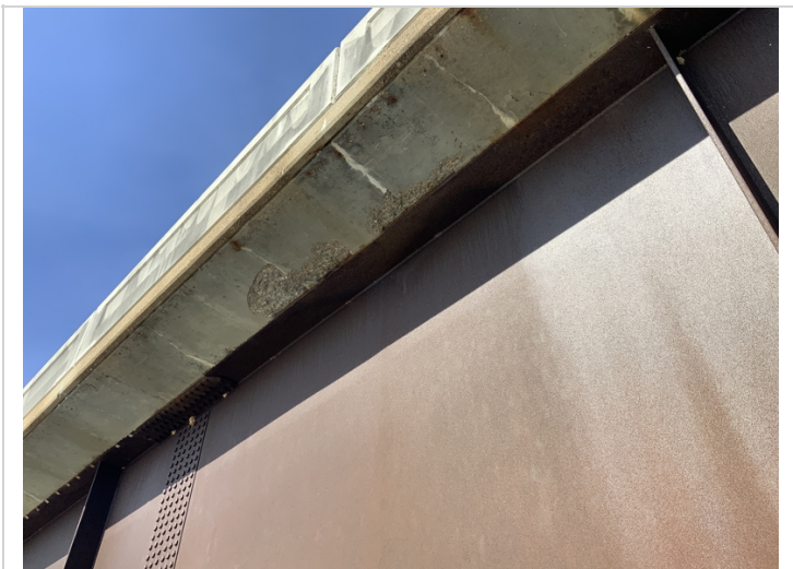
Span 1&2 right Spalling in overhangs
