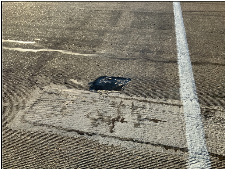
Span 6 Left lane Spalling
