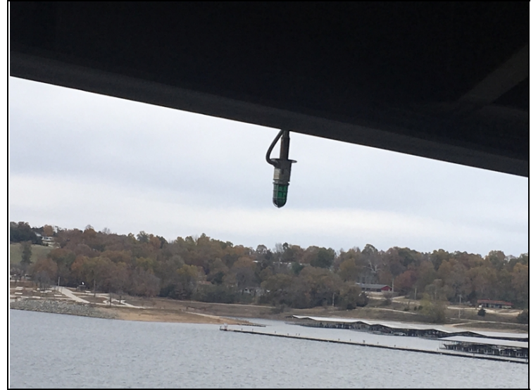
Span 9, Left: Navigation light not working.
