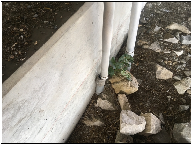
Utility conduit separating at ground level.
