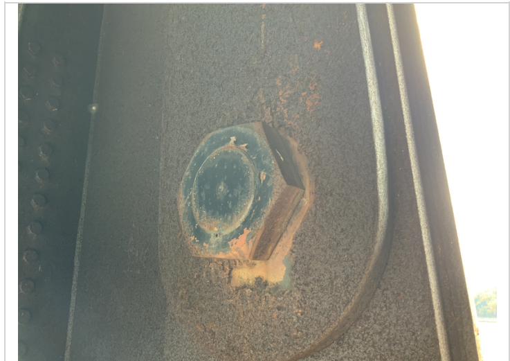
Hanger bar at bent 3 flaking rust.
