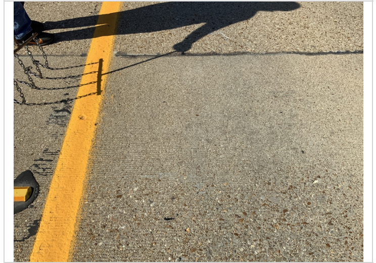
Light map cracking
