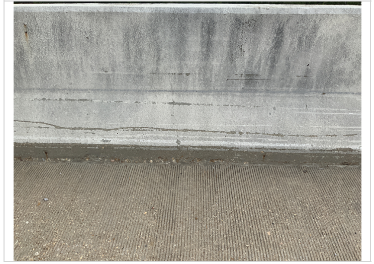
Typical vertical cracking in bridge railing
