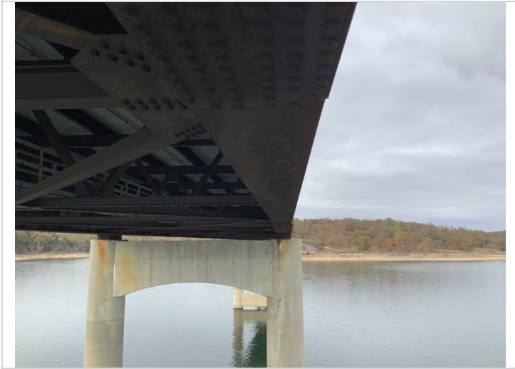
Span 7 Girder 1 Flaking
