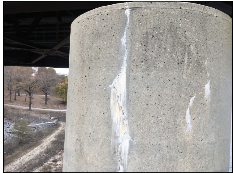
Pier 1, Column 2: Failing repairs.
