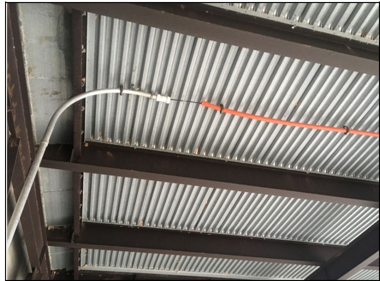
Utility conduit separating.
