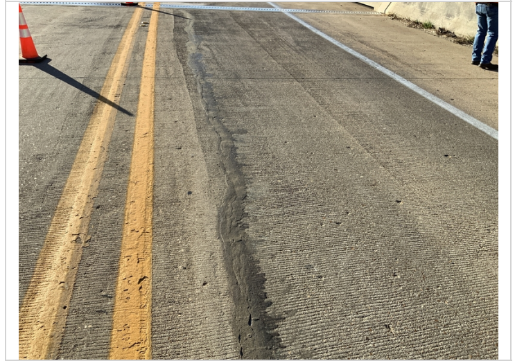
Abutment 2 Approach slab failing sealant
