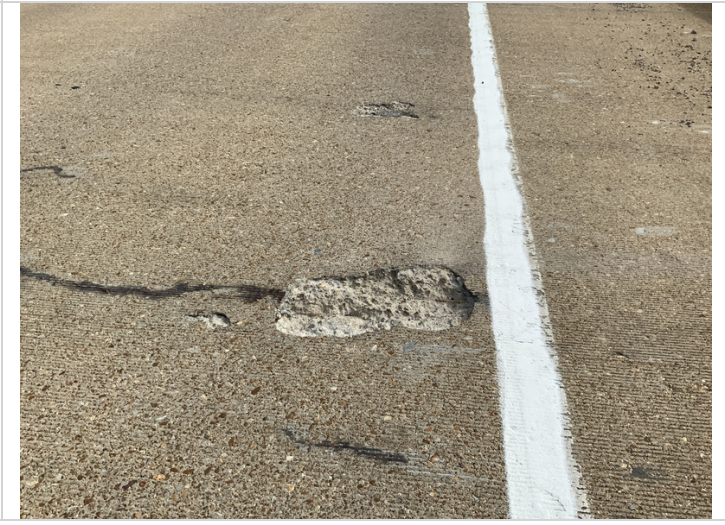
Span 5 Right lane Spalling
