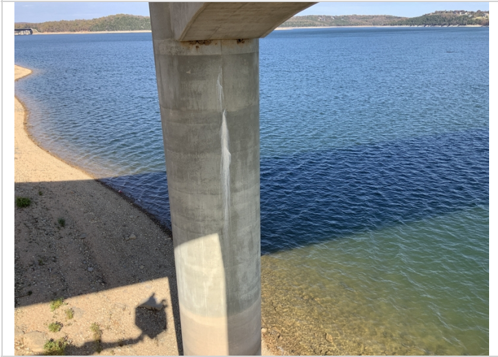
Pier 1 Column 1 Cracking with efflorescence
