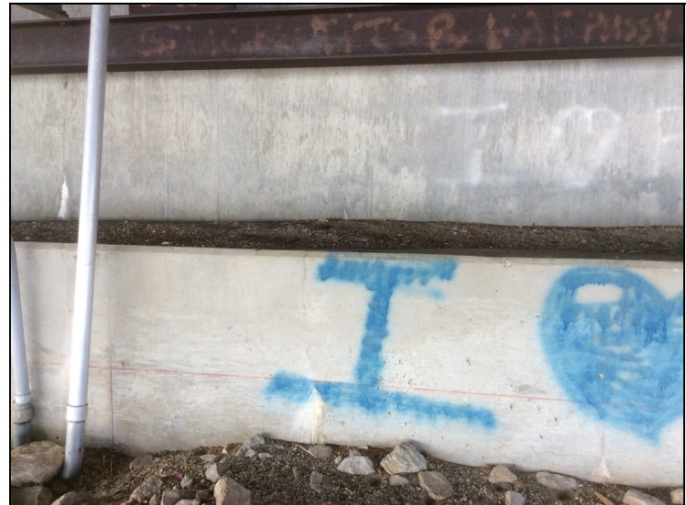
Abutment 1: 8 vertical cracks in back wall.
