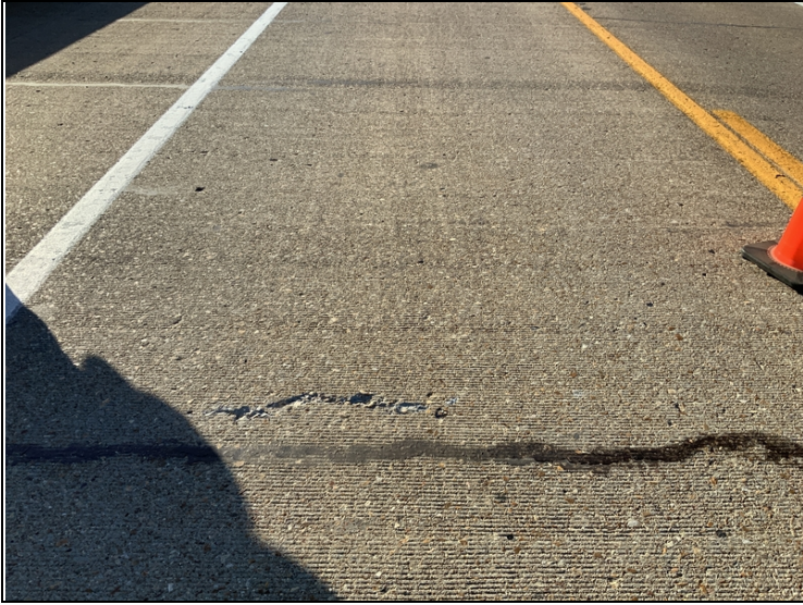
Span 13 Right lane delaminating area
