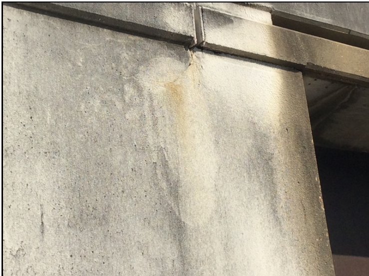
Wing wall at abutment 1 45 degree crack at the top. (Typical at all wing walls)
