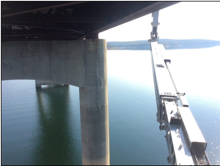
Pier 3 epoxy injection. Cracks with Efflorescence in both columns.
