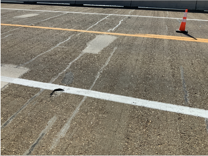
Span 2 Spalling in wheel paths
