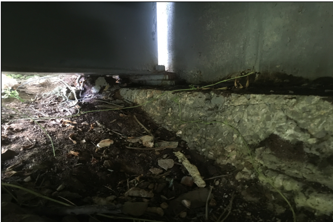
Bearing #8 at abutment #1 is partially covered with dirt and has corrosion.
