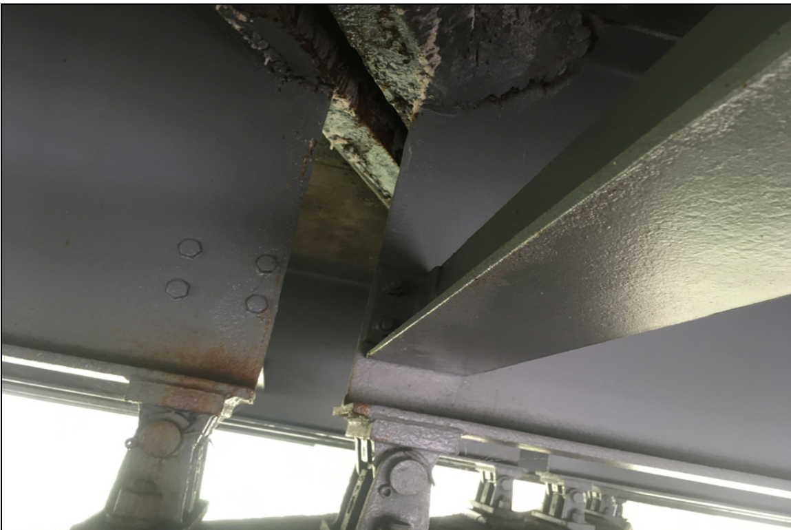
The bearings at beam #4 over pier #1 have rust staining on the paint from joint seal drainage. Typical of several locations.
