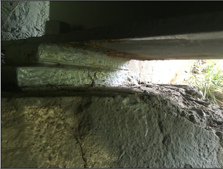
Beam #8 at abutment 2 has 1/8" of section loss on the bottom flange at the bearing area.
