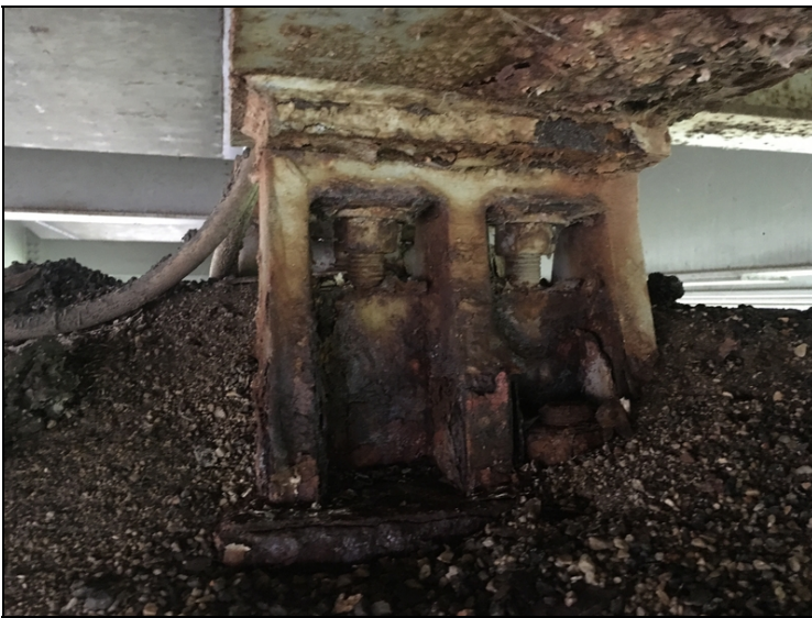
Fixed bearing condition at bent #2. Typical of bearings # 4-6.
