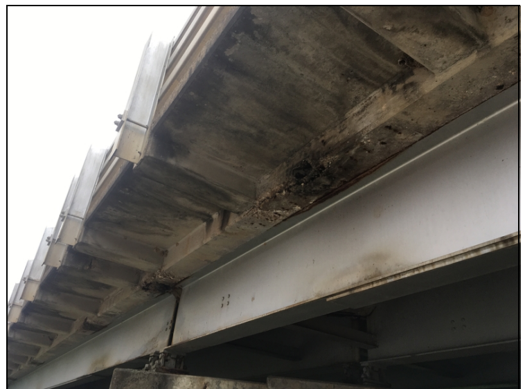
Drain area condition. Showing spalling and delamination some with rebar exposed. Typical of many locations.
