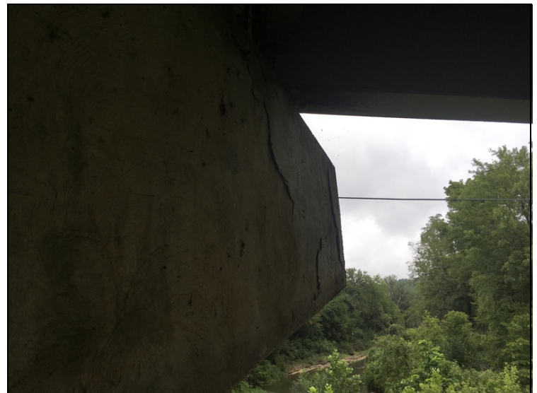
Large delaminations on the span #5 side of the bent #4 cap. Typical of the left and right sides.
