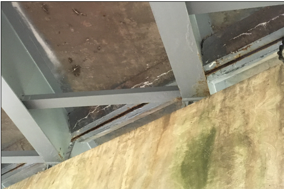
Corrosion beginning to show through the paint on beams 4,5 in span 6.
