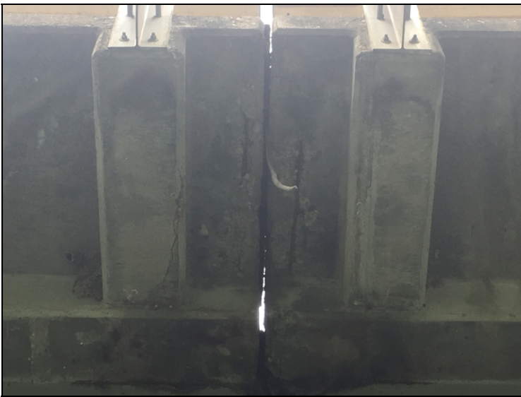
Shallow rebar exposed on the underside on the right concrete bridge rail in spans #5,6.
