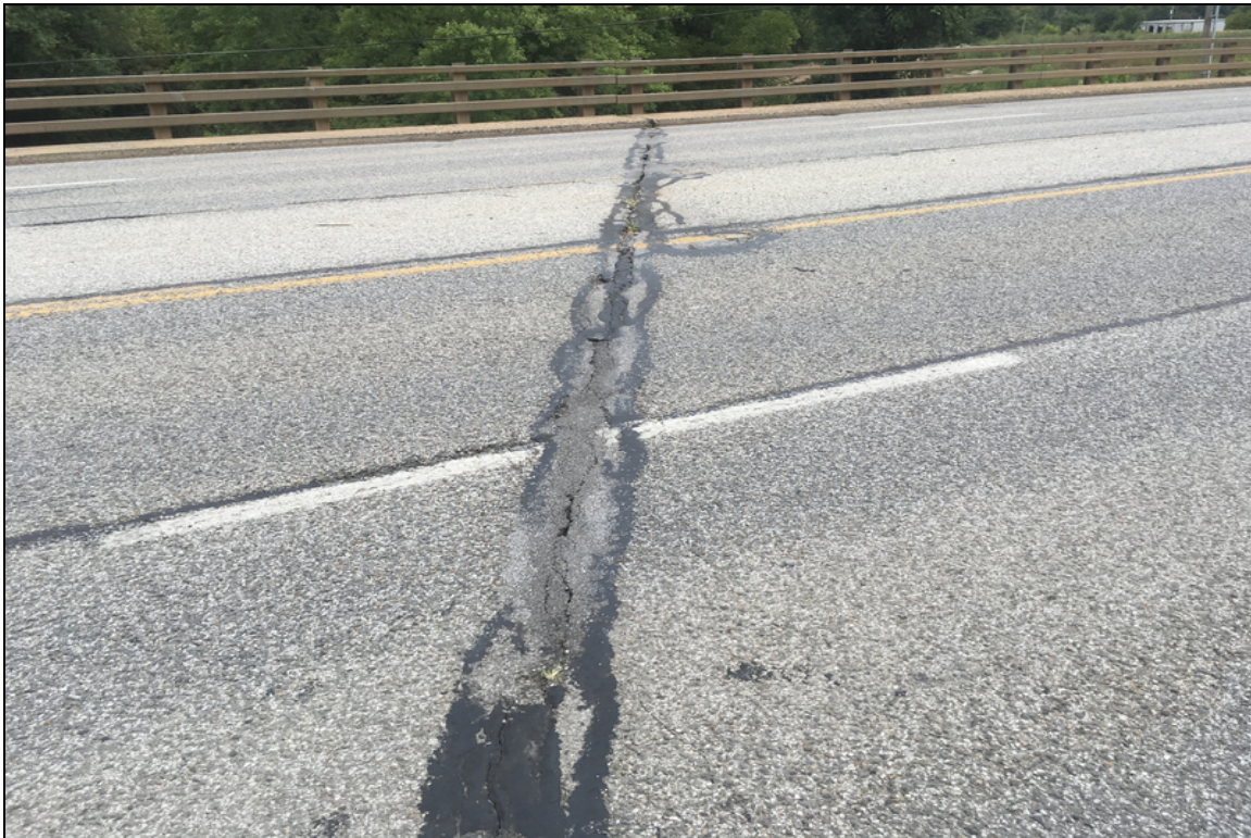
Typical view of the joint areas over the piers and abutments.
