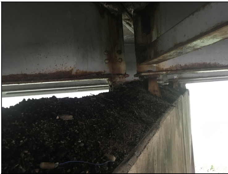
Heavy Debris build up on the bent #2 cap.
