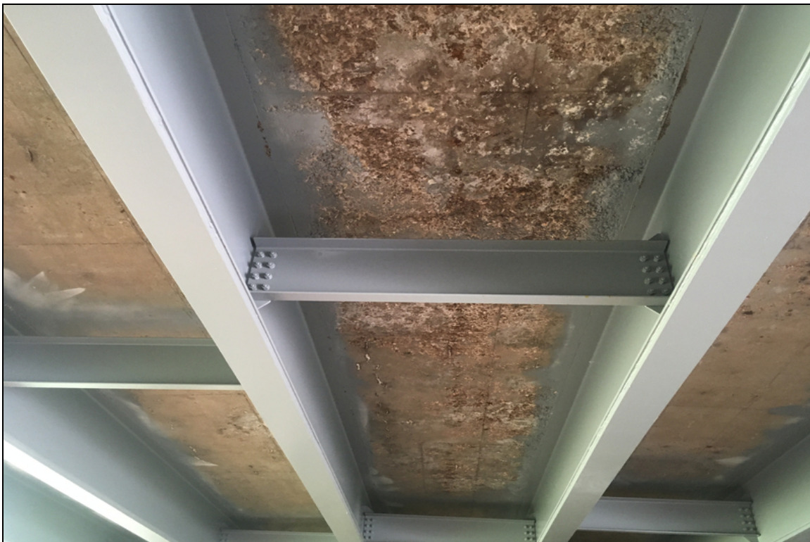
Bay #4 of span #1 showing delamination and efflorescence cracking in the deck under surface. Typical of other areas in the deck under surface.
