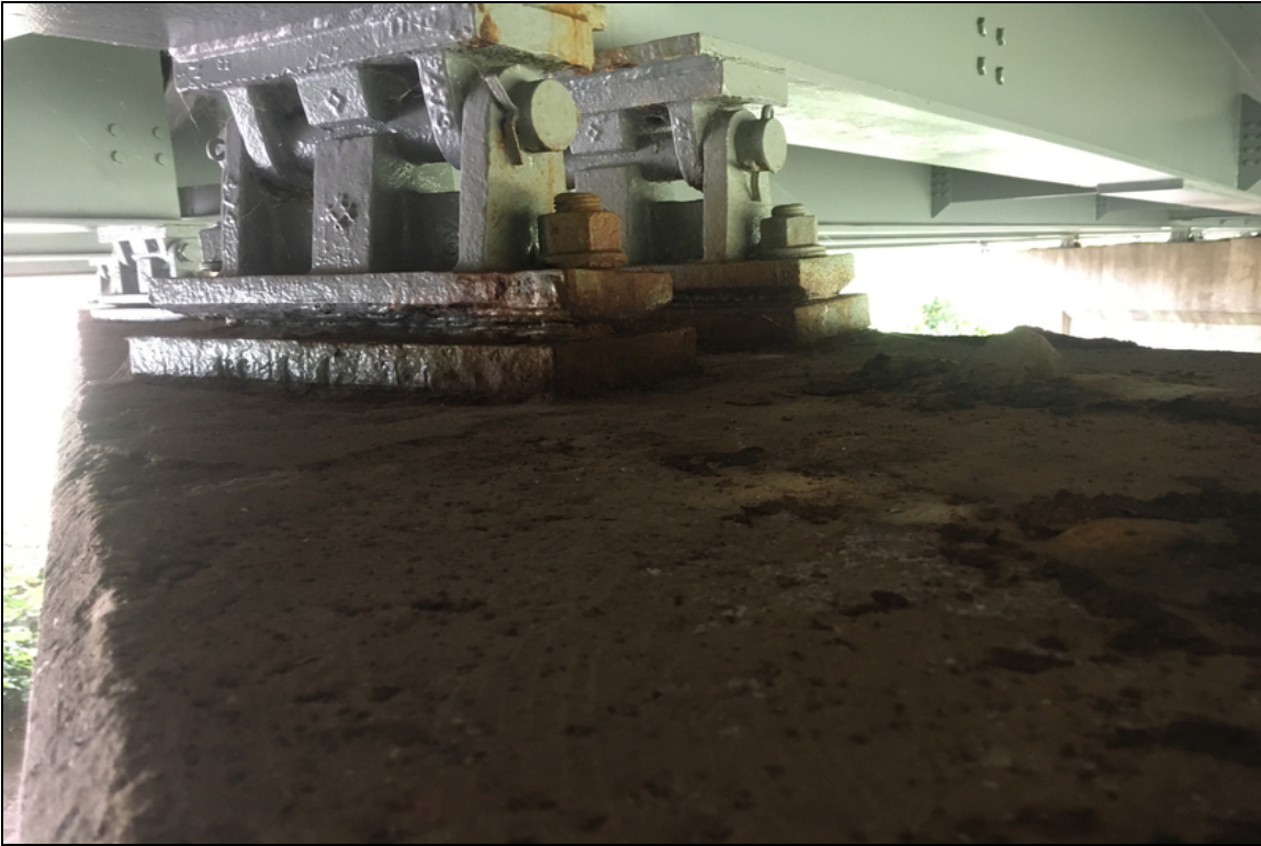
Pack rust still exists in many of the rocker areas. Typical of several locations.
