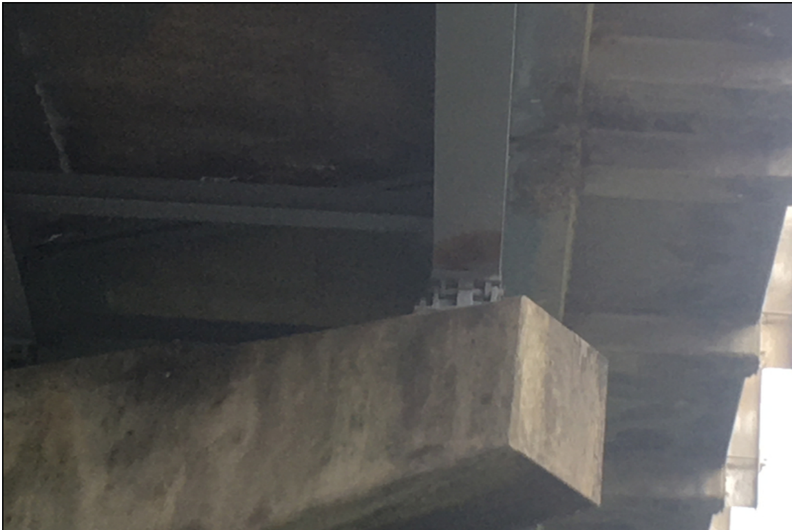
Cs2 corrosion on the bottom flange of beam 1 at the beginning of span 4.
