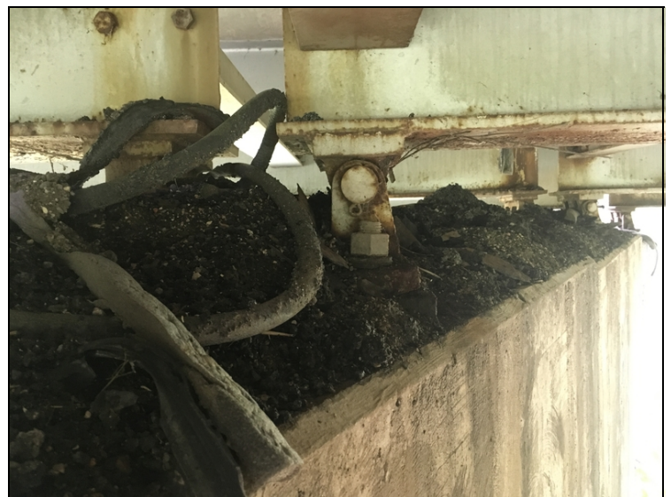
Heavy build up on the bent #5 cap.
