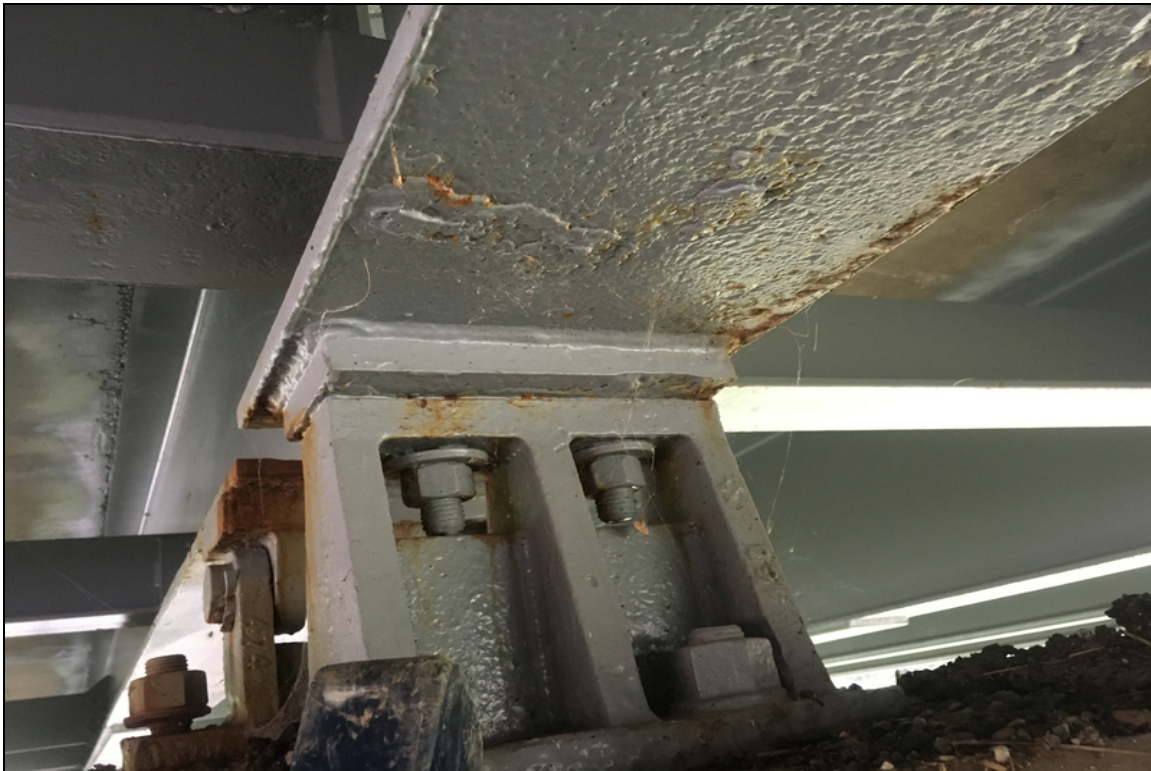
Flaking rust that has been painted over on the beams. Typical of several locations.
