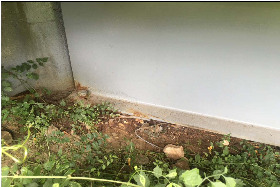
Beam 8 has 2' of cs3 corrosion on the lower web and bottom flange at the beginning of span 1 due to dirt build up.
