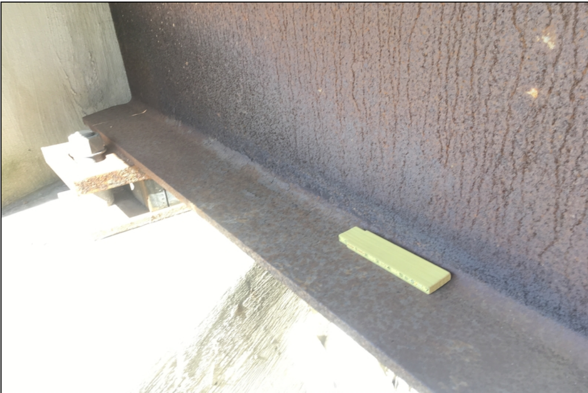
Minor corrosion of beam #5 in span #1. Typical of other locations.
