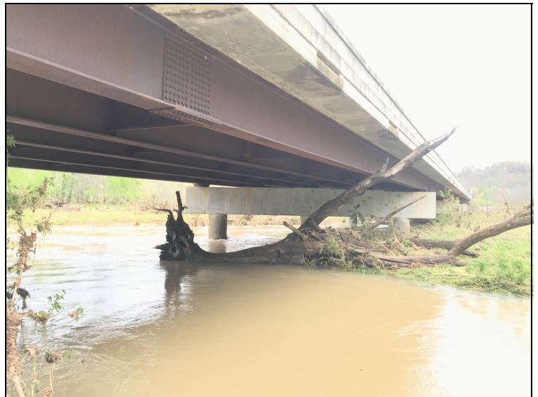
Span #2 has a large tree that has wedge against girder #5 resulting from a high water event.
