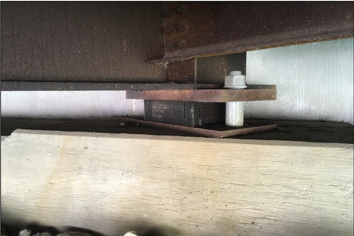
Typical view of the 5 bearings at abutment #1.
