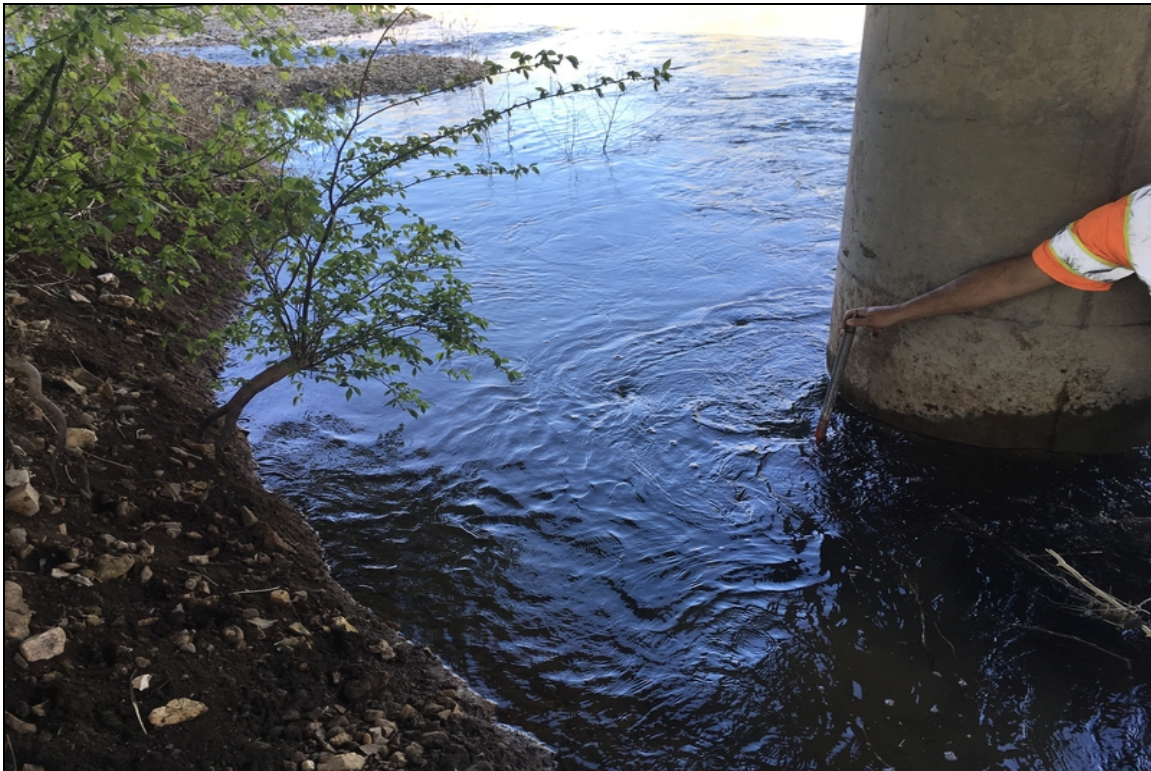
Column #1 of bent #2 showing local scour. No footing was exposed.
