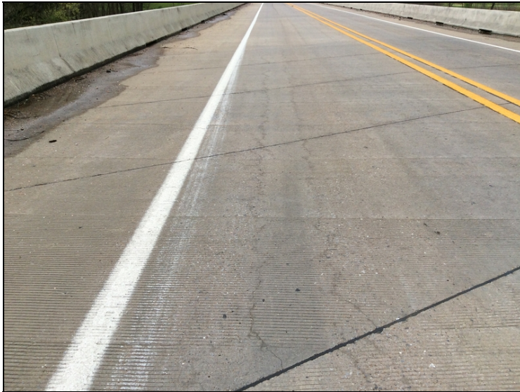
Typical longitudinal cracking.
