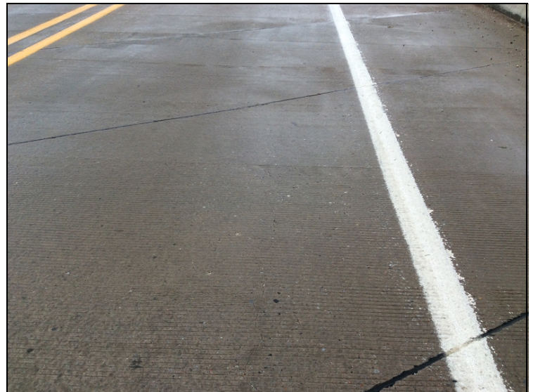
Bent 1 Left longitudinal cracking.
