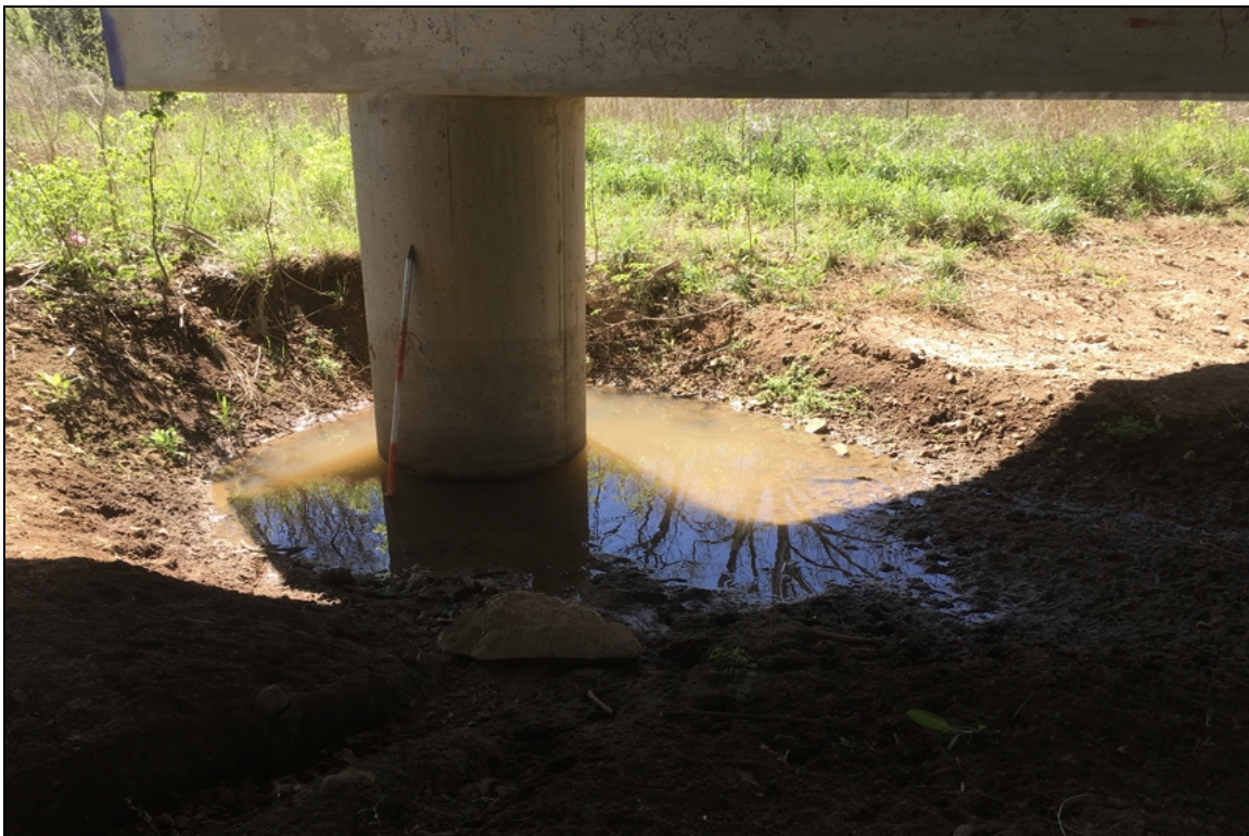
Minor local scour around column #3 of bent # 4. No footing was exposed.
