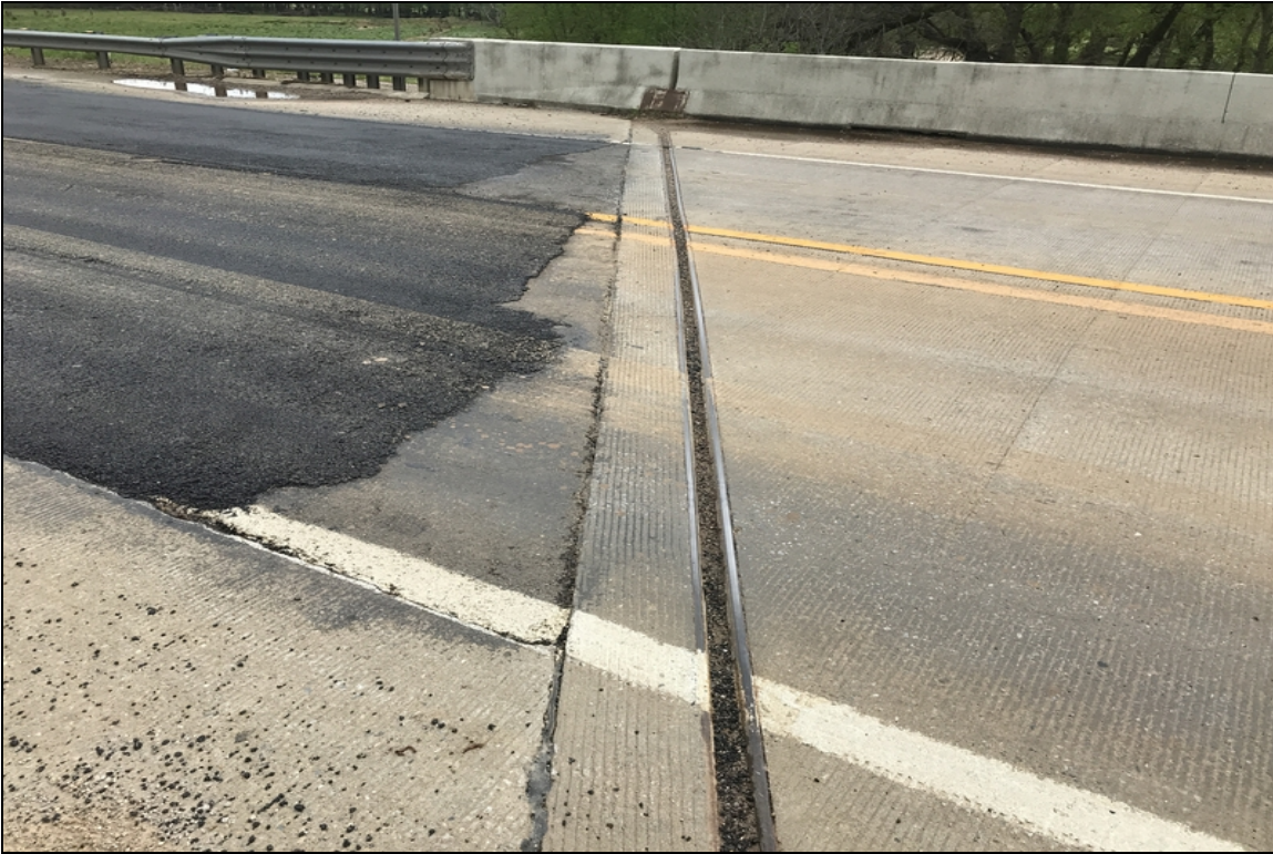
Abutment #2 expansion joint debris impact
