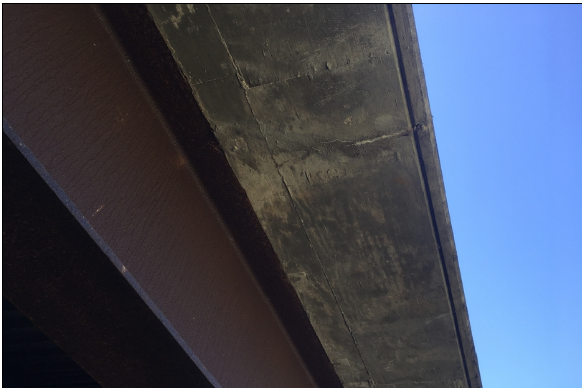
Typical efflorescence cracking in the deck over hangs.
