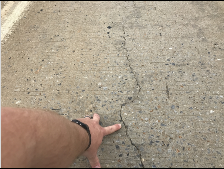
Longitudinal cracking over bent #1 in south bound lanes.
