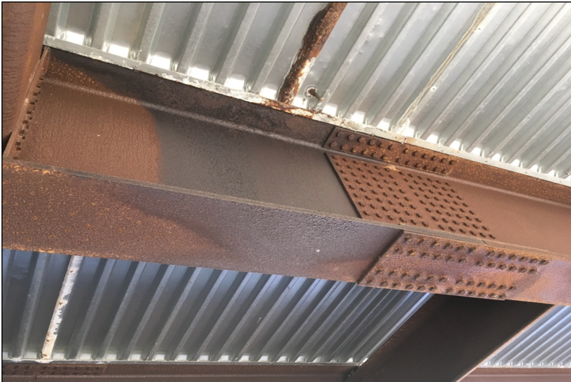
4' of corrosion with flaking rust on beam #3 in span #2 at the field splice.
