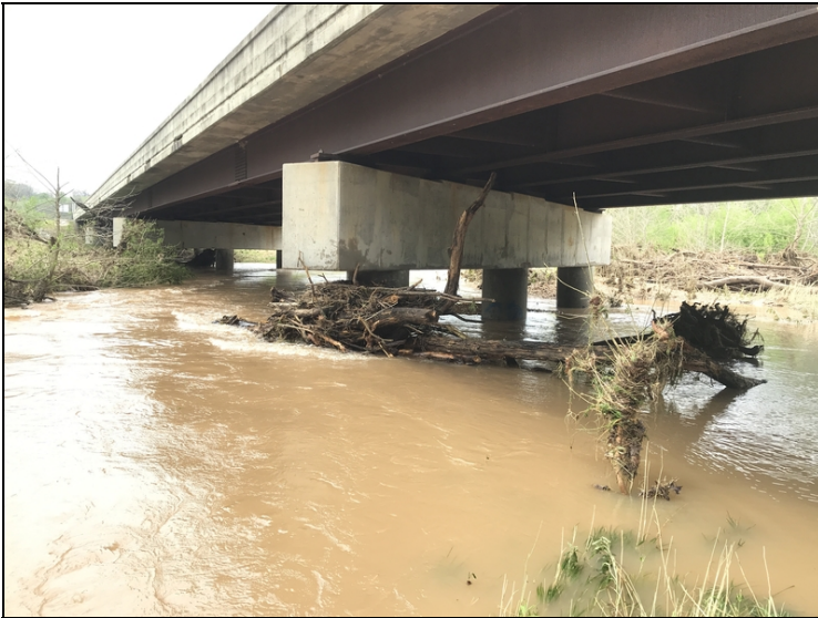
Bent #3 drift accumulation
