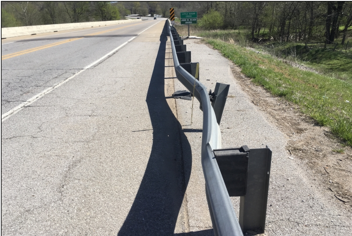
Approach guard rail damage at the right beginning of the structure.
