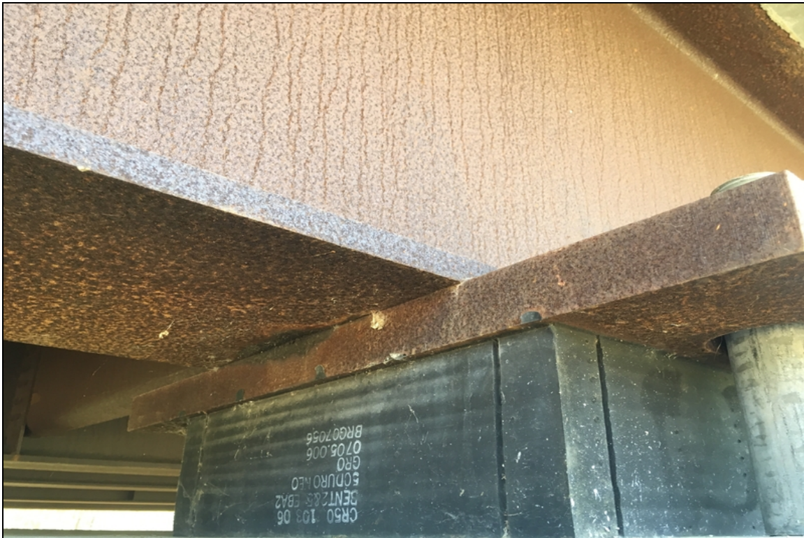
Typical bearing condition over the bents.
