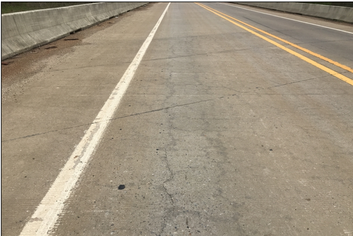
Longitudinal cracking over bent #1 in south bound lanes.
