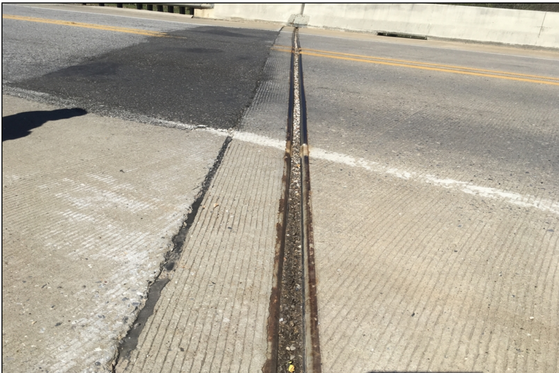
View of strip seal expansion joint at abutment #1.
