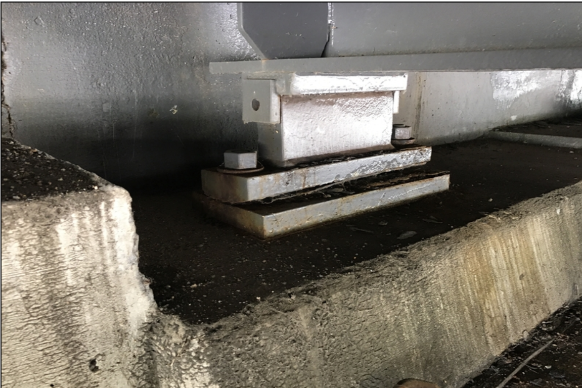
Abutment #2 bearing #5 left bolt that attaches sole plate to rocker bearing.
