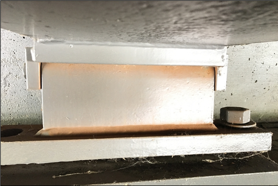
Fretting dust in the bearing area.
