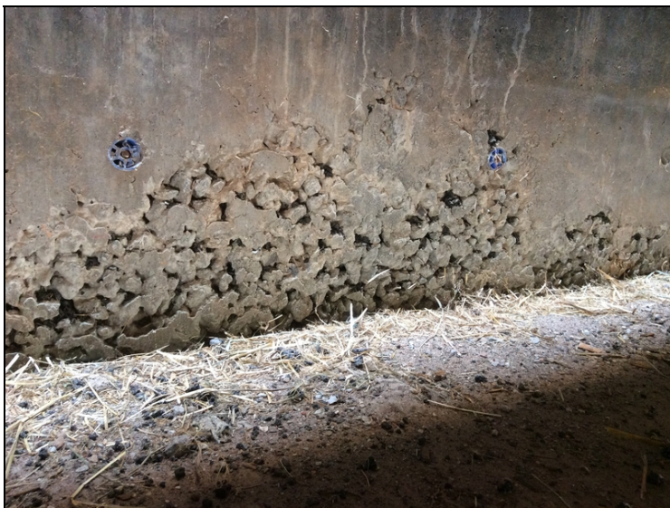
Abutment #2-Honeycombing in backwall.
