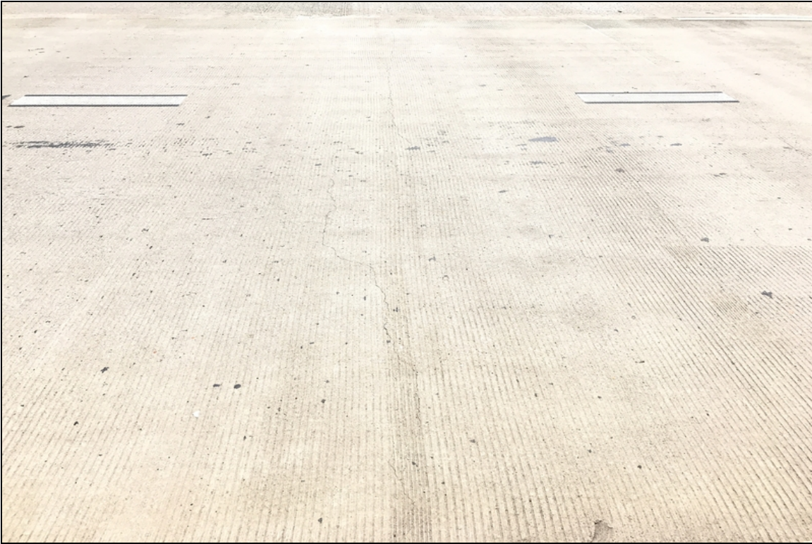
South bound lanes typical transverse cracking
