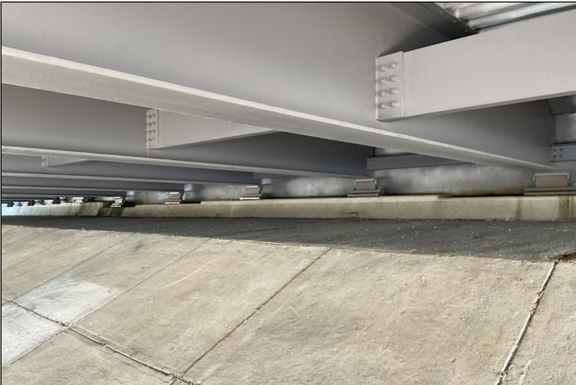
View of bent #2 bearings.
