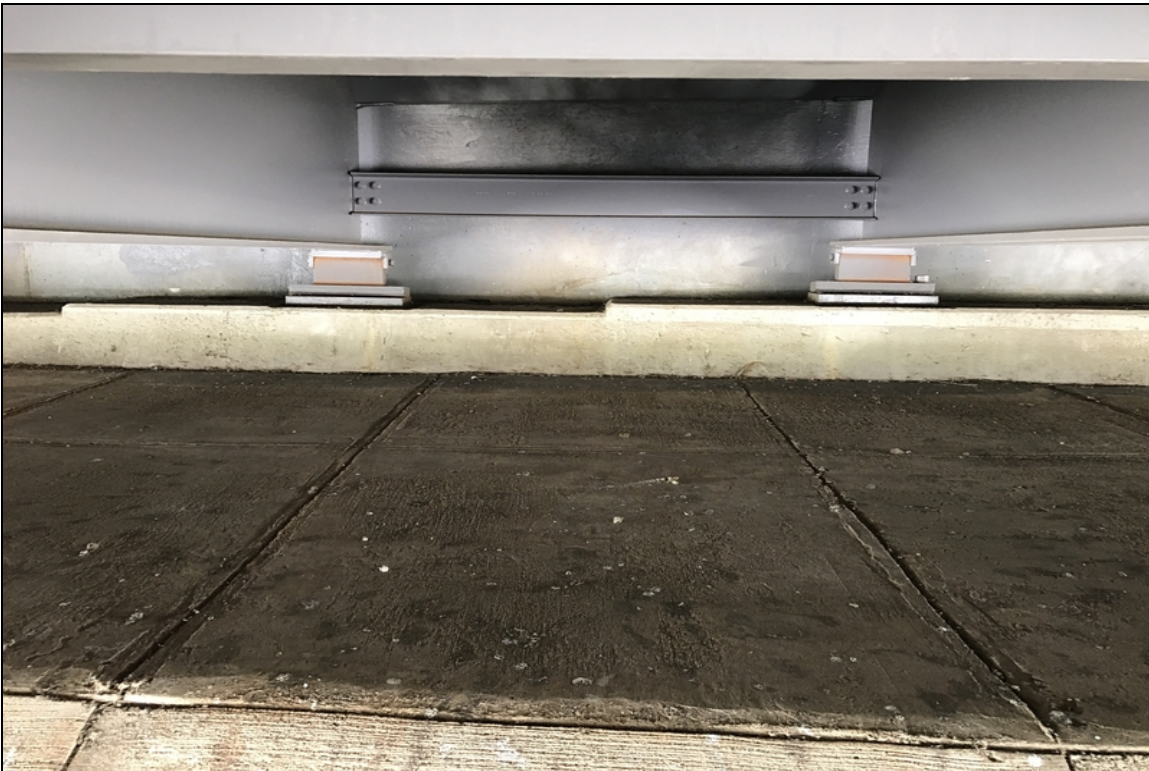
Bearings #6 and #7 at abutment #2 missing anchor bolts.
