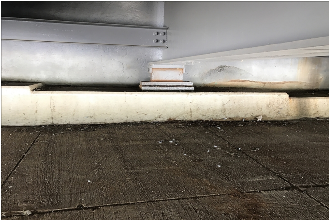
Bearing #6 at abutment #1 missing anchor bolts
