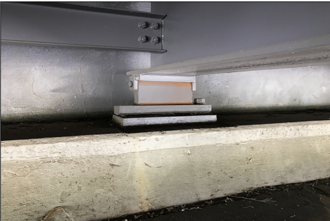
Fretting dust in the bearing area.
