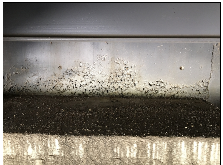
Honeycombing and un-grouted snap ties at abutment #2.
