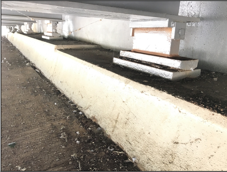
Typical view of rocker bearings at abutment #1.
