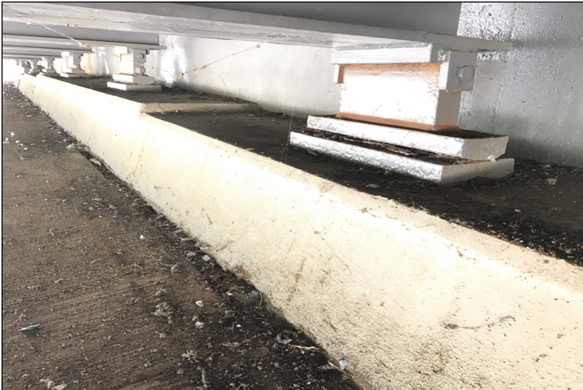
Typical view of rocker bearings at abutment #1.
