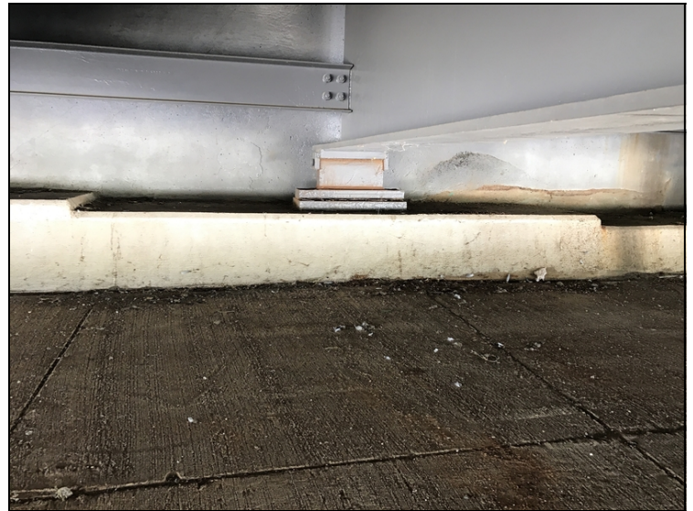
Bearing #6 at abutment #1 missing anchor bolts
