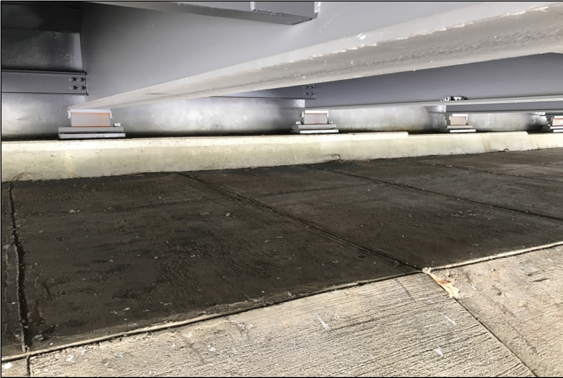
Fretting dust in the bearings
