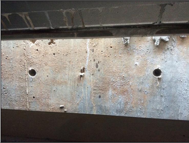
Abutment #2-Snap-tie holes ungrouted.
