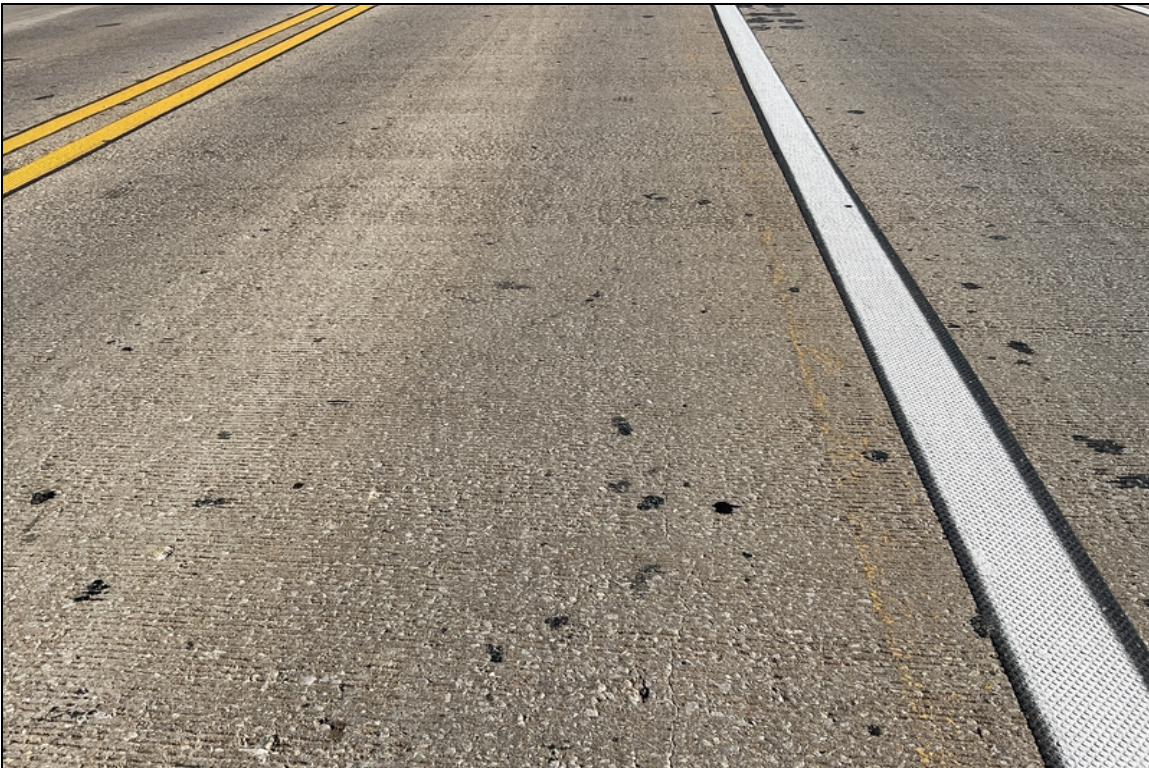
View of longitudinal cracking in older portion of bridge.
