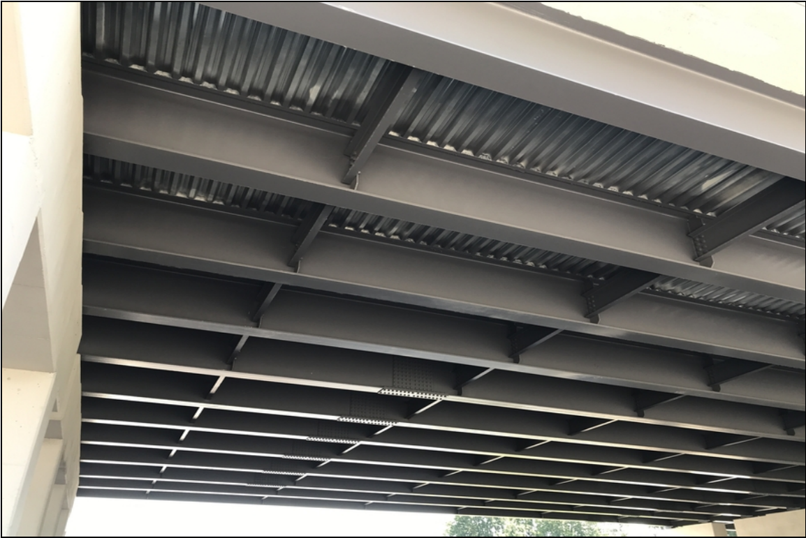
Only girders 5-10 have a second splice plate in span #2.
