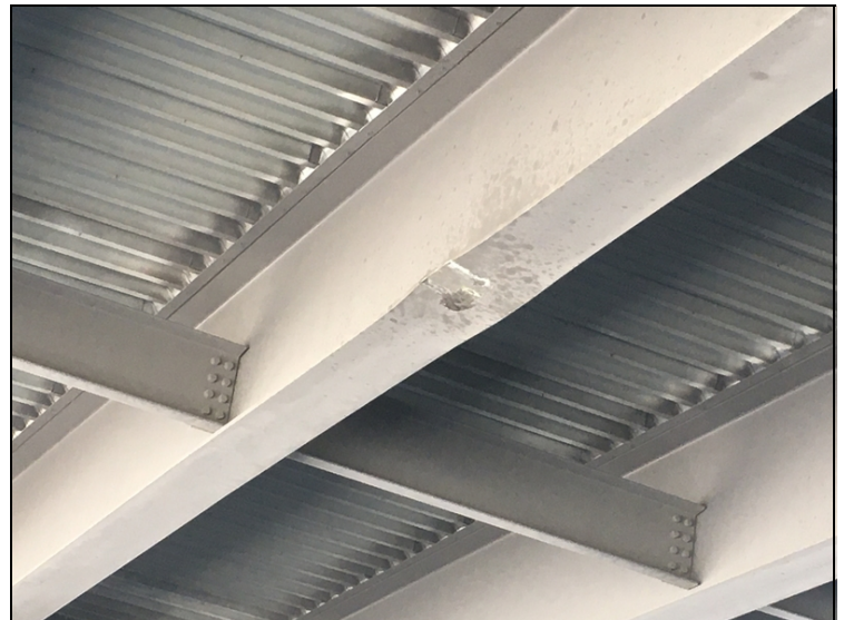
Beam #8 in span #3 has 2" of upward distortion on the bottom flange for 1'.
