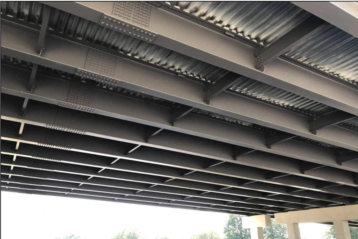
General view of span #3 superstructure.
