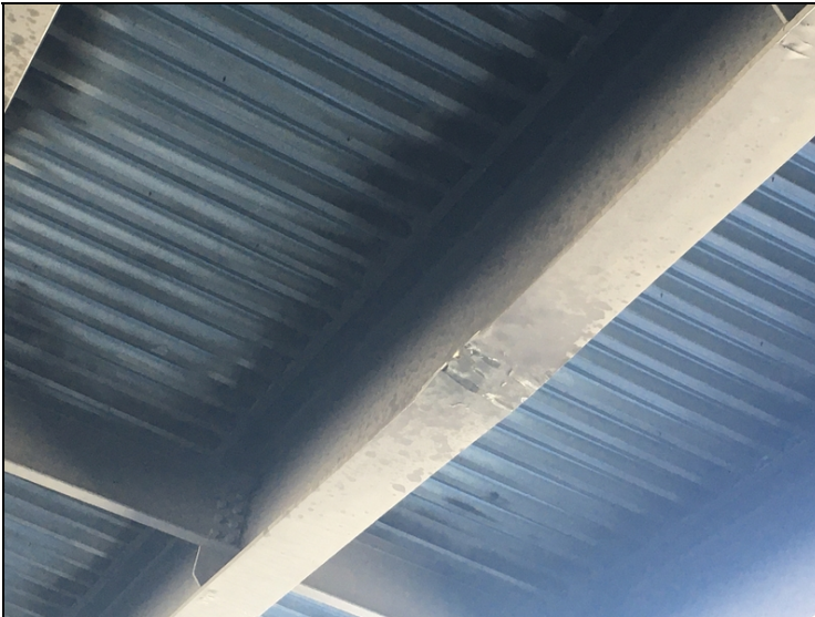
Beam #3 span #3 has 3" of upward distortion on the bottom flange for 1'. 41' ahead of bent #2.
