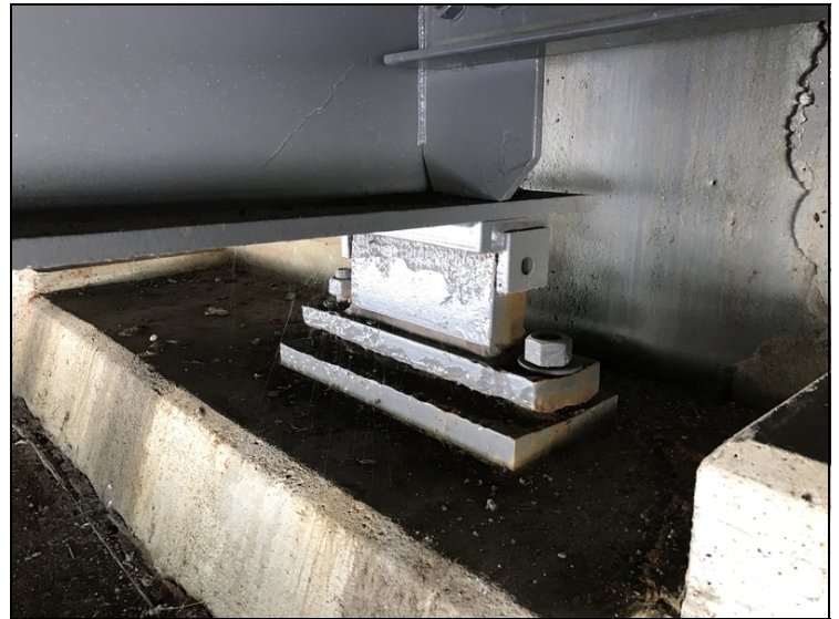
Bearing #5 at abutment #1 missing bolt that attaches the sole plate to the bearing.
