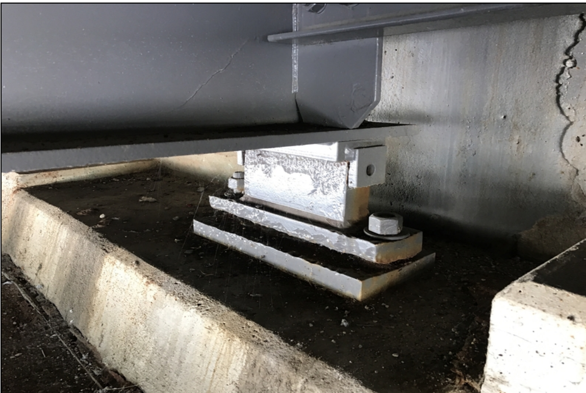
Bearing #5 at abutment #1 missing bolt that attaches the sole plate to the bearing.
