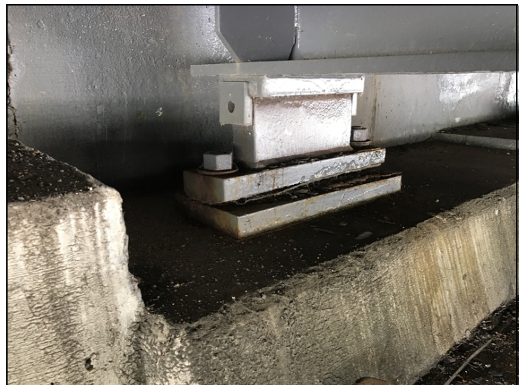
Abutment #2 bearing #5 left bolt that attaches sole plate to rocker bearing.
