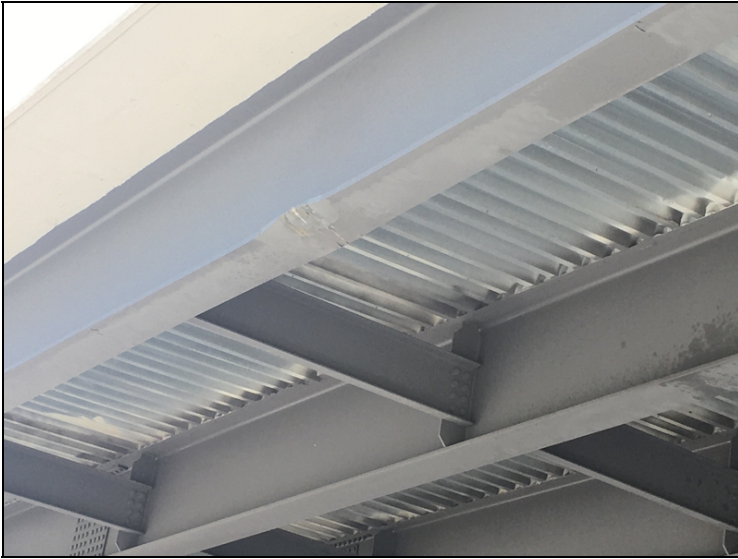
Beam #12 has 3" of upward distortion on the bottom flange for 1'.
