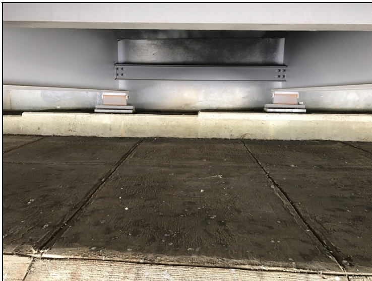
Bearings #6 and #7 at abutment #2 missing anchor bolts.
