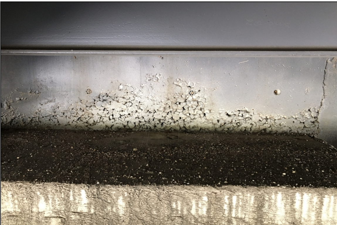
Honeycombing and un-grouted snap ties at abutment #2.
