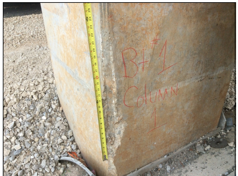
Bent #1, column #1-Spalled area.
