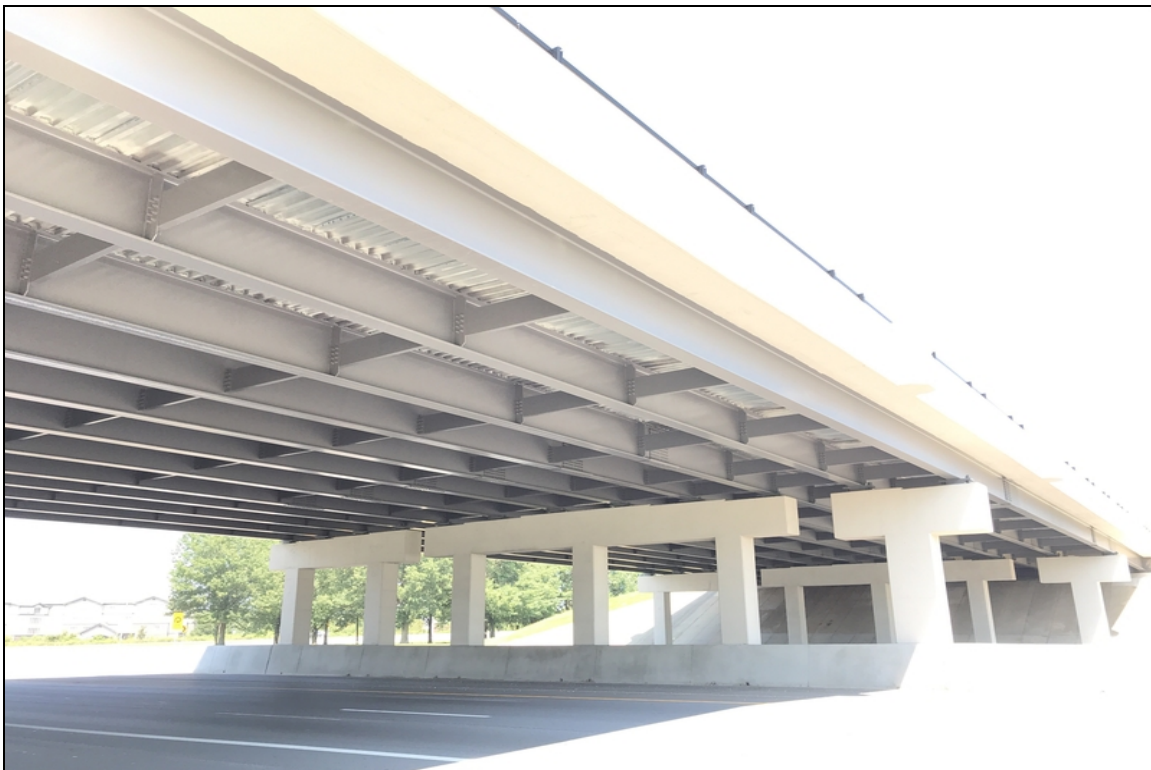
Superstructure has new steel protective coating applied since last inspection.
