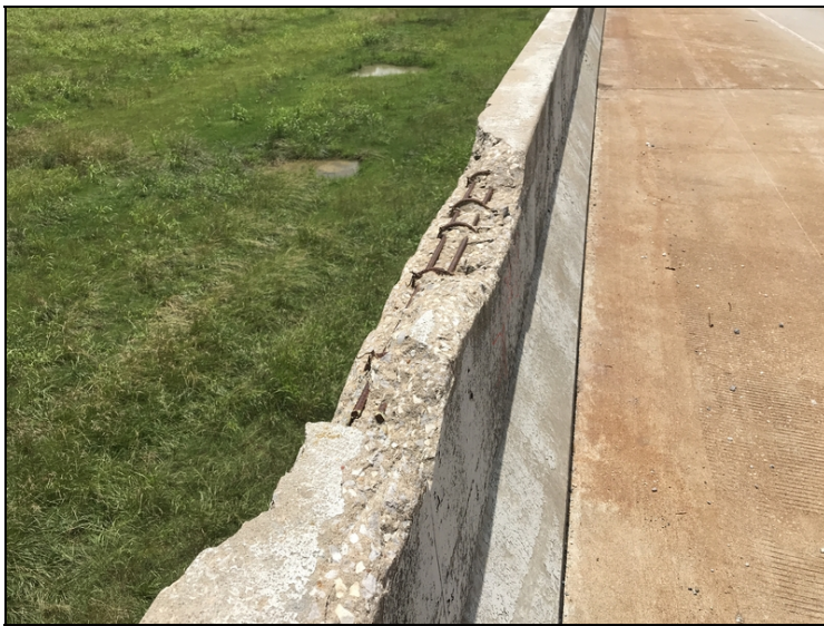
Span #8 right railing spalling with rebar exposed.
