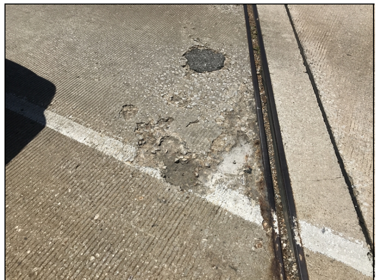
Large spall adjacent to abutment #2.
