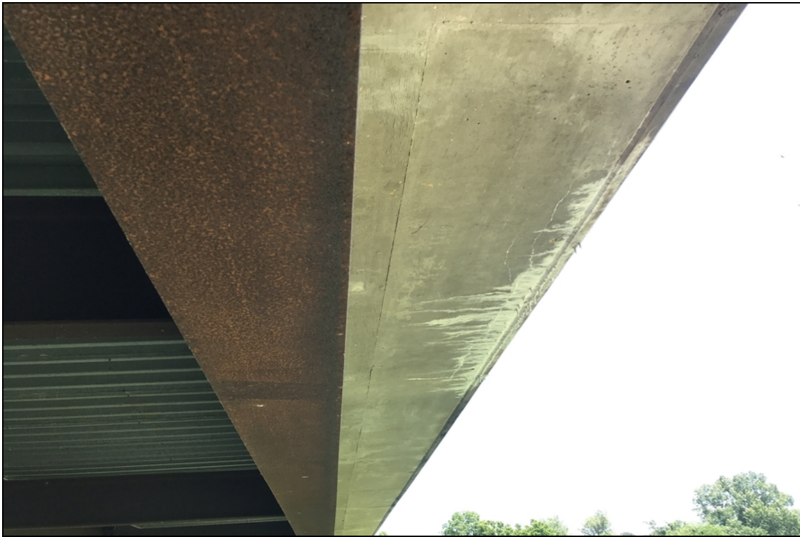
Span #11 right over hang efflorescence with cracking.
