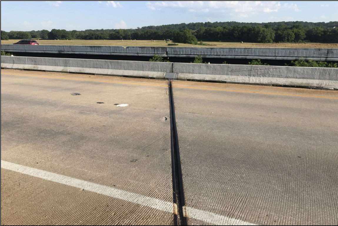
Spalling behind expansion joint at bent #4.
