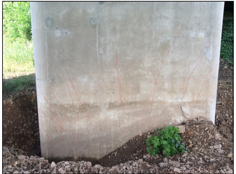
Bent #1, Span #2-Diagonal cracking.
