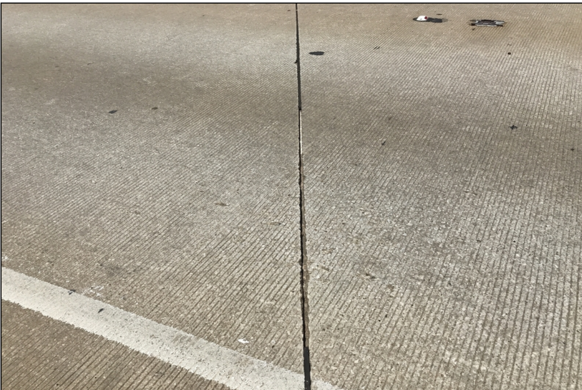
Typical displacement of pourable joint material.
