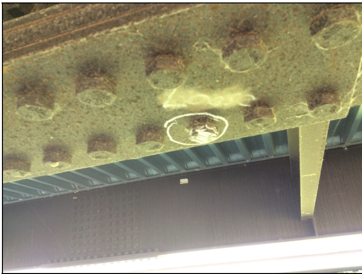
Span #15, Girder #2 has a loose bolt in the bottom flange splice plate.
