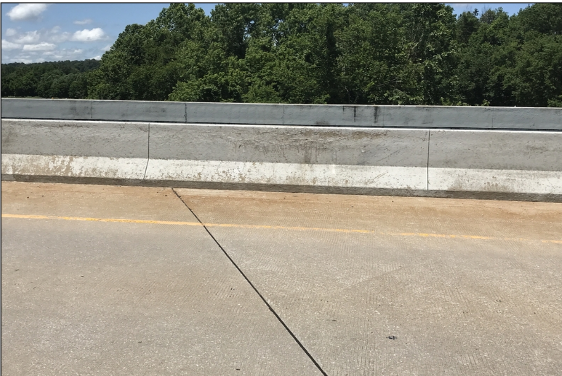
Typical efflorescence and cracking in parapet wall.
