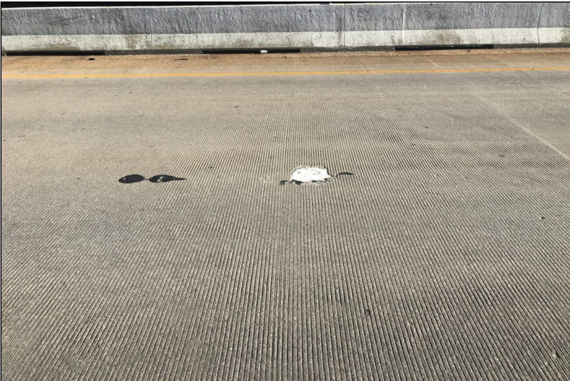
Maintenance forces have patched steel pavement markers.
