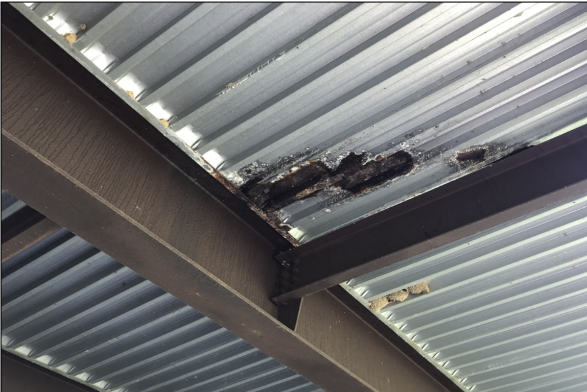
Span #2 bay #4 approximately 10' ahead of bent #1 the sip forms have active corrosion this is typical throughout undersurface.
