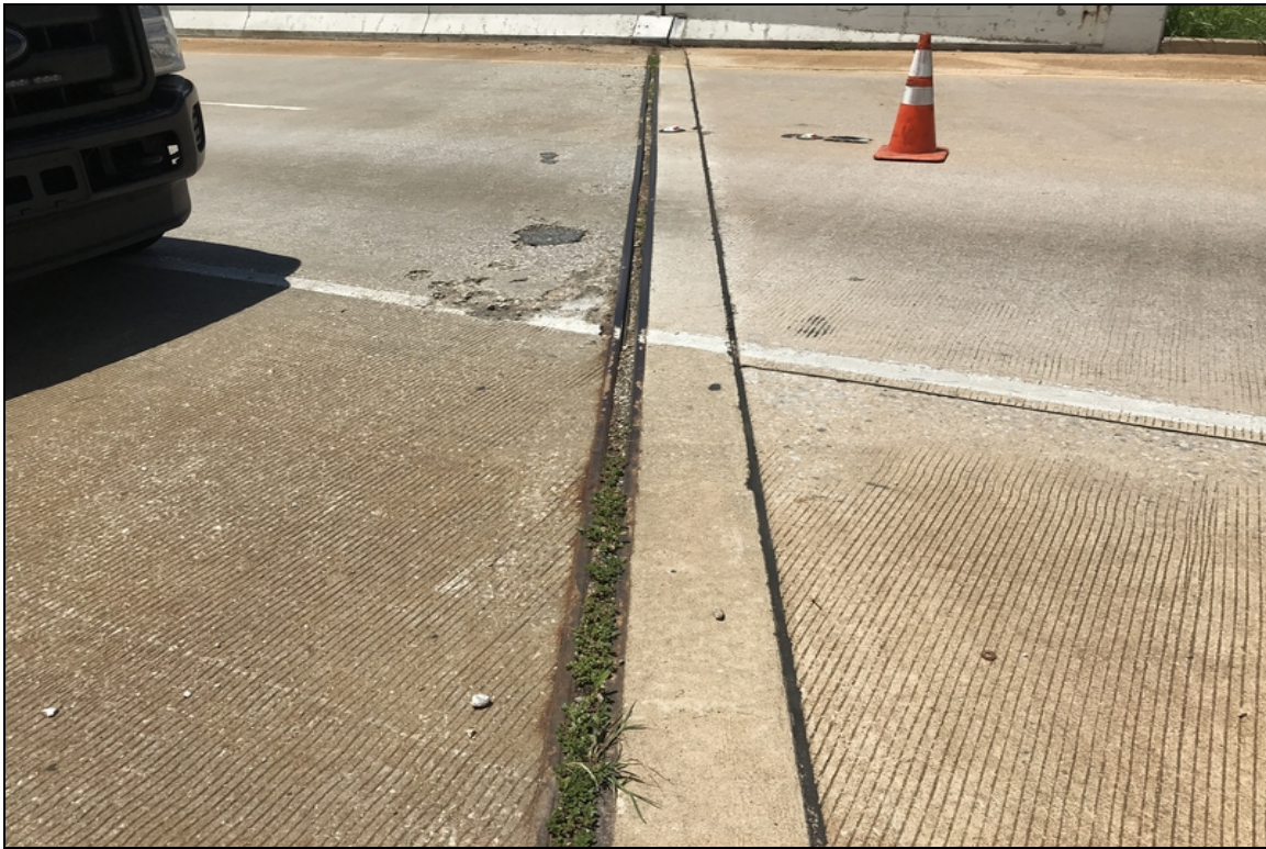
Abutment #2 debris impaction.
