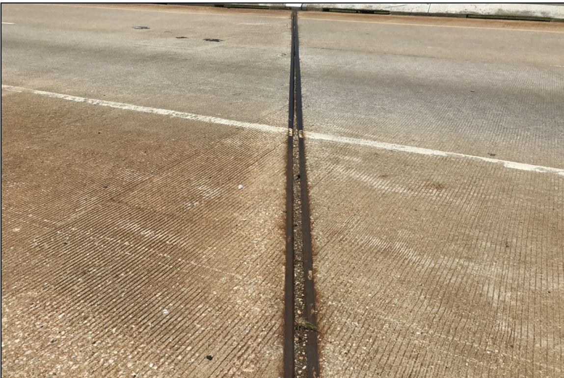
Bent #4 expansion joint debris impactation.
