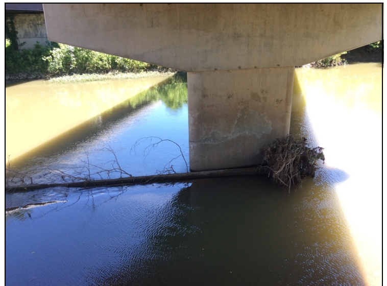
Channel-Drift at bent #17.
