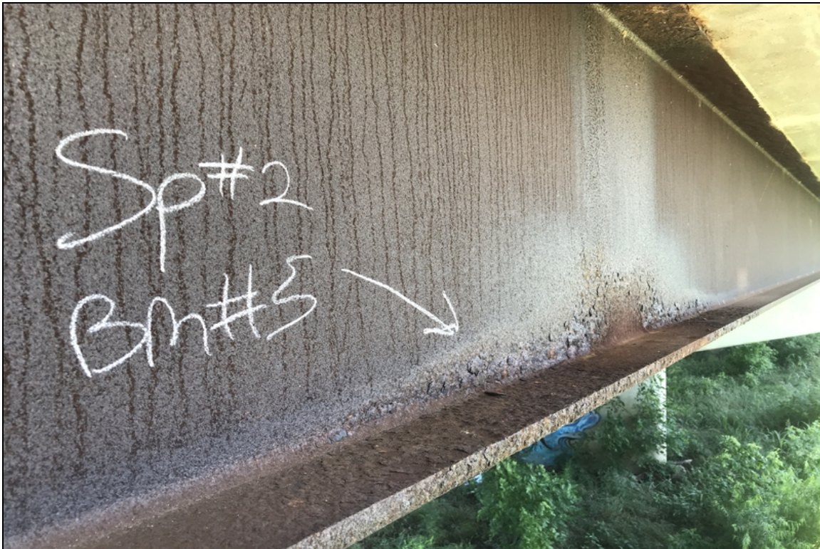
Span #2, exterior side of girder #5 has an area of corrosion with initial section loss to web and top and bottom flanges where deck cracking leaches onto superstructure.
