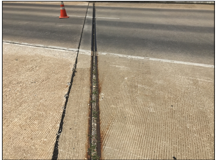
Abutment #1 minor debris impactation
