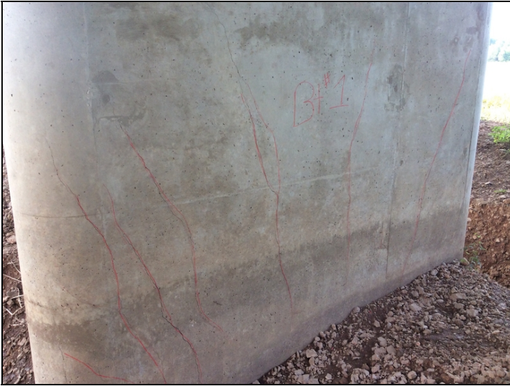
Bent #1-Diagonal cracking.
