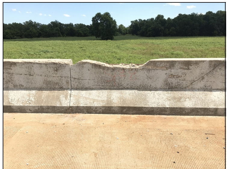
Span #8 right railing spalling with rebar exposed.
