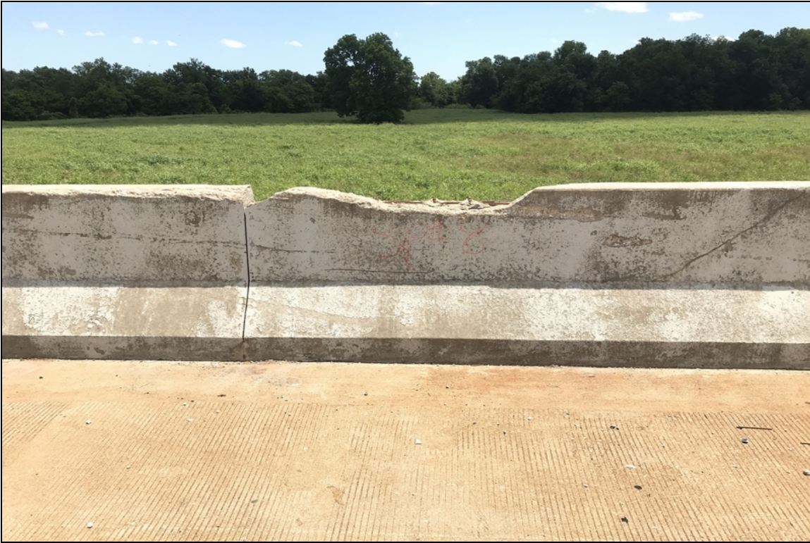
Span #8 right railing spalling with rebar exposed.
