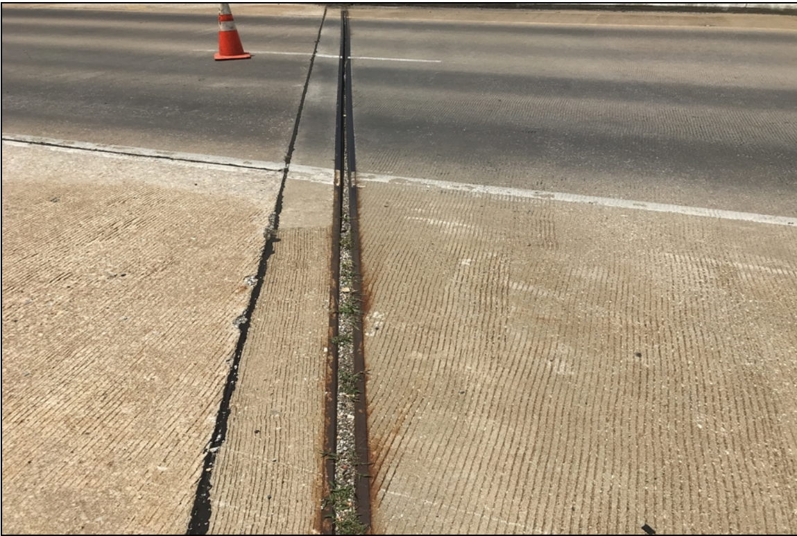
Abutment #1 minor debris impactation
