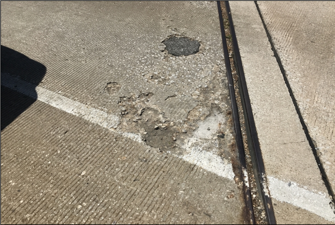
Large spall adjacent to abutment #2.
