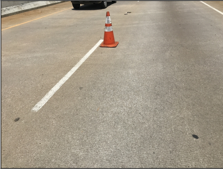
Typical view of longitudinal crack at centerline.
