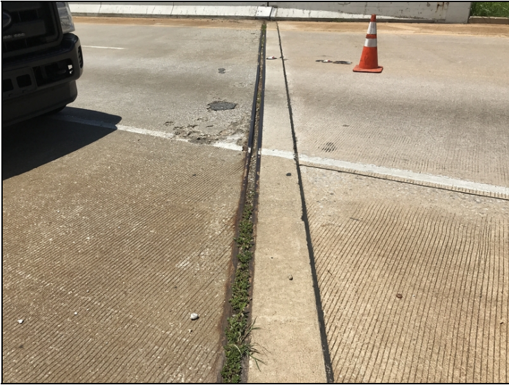
Abutment #2 debris impactation.
