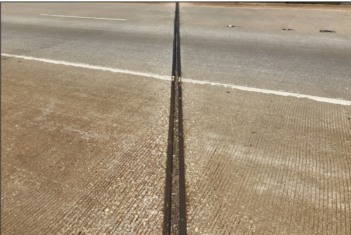
Bent #8 expansion joint debris impaction
