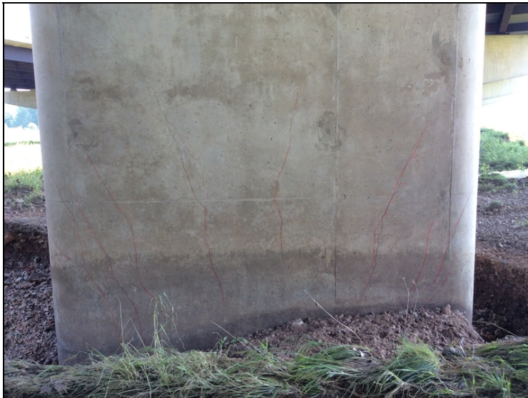
Cracking in bent #1 column. Photo #1.
