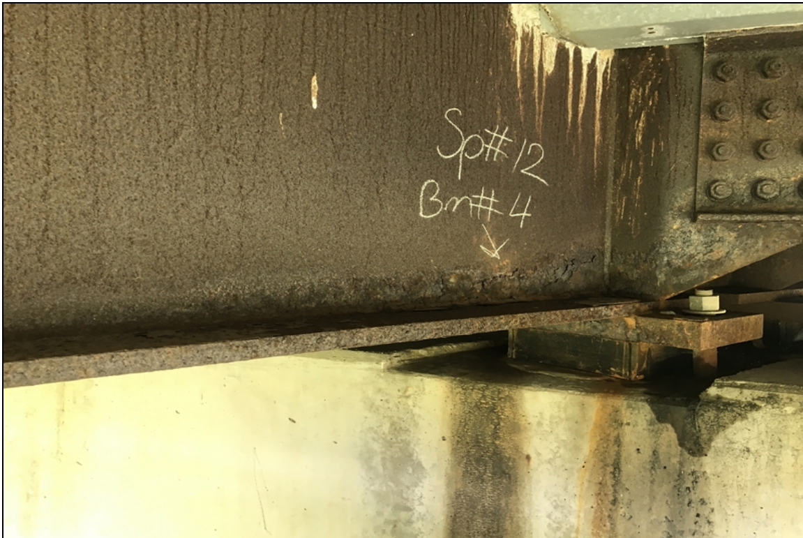
Span #12 girder #4 flaking rust at the end of girder over bent #12
