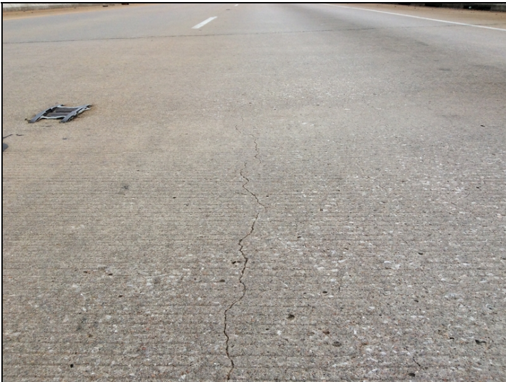
Longitudinal cracking typical, photo #2.
