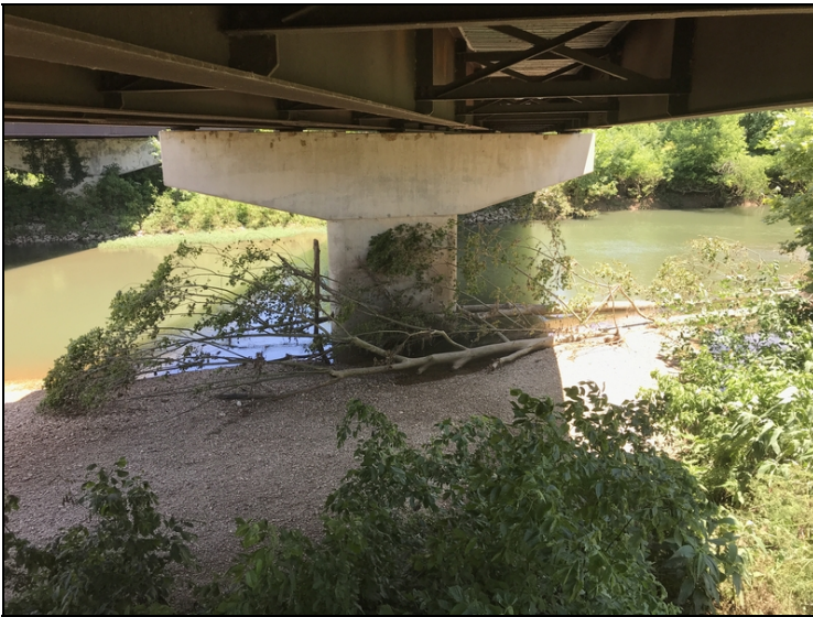
Large tree wedge against bent #17.
