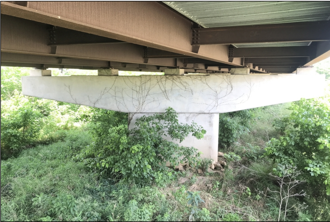
Bent #10 has concrete riser due to elevation bust.
