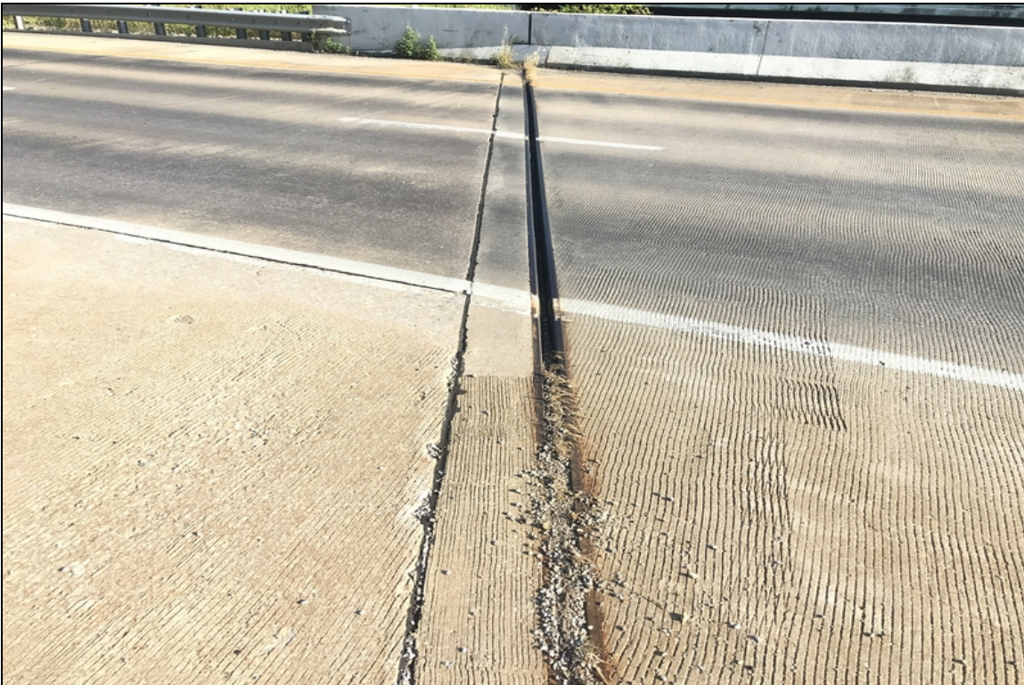
Abutment #1 expansion joint.
