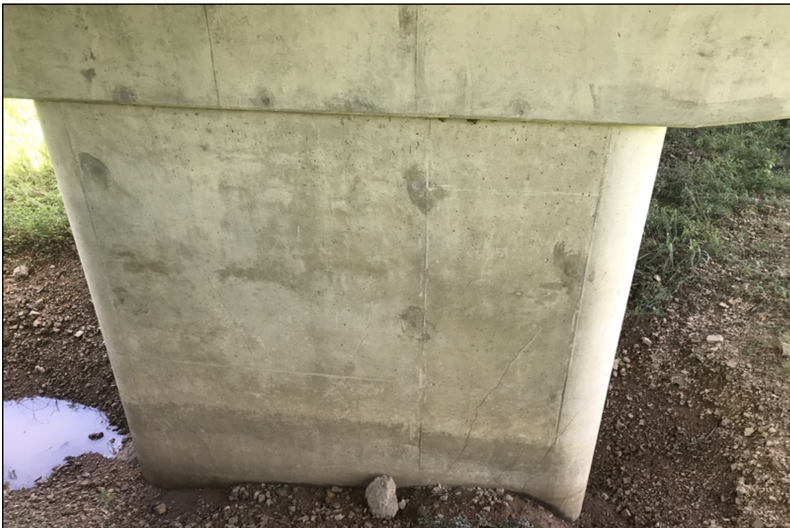
Bent #1 pier cracking in the pier.
