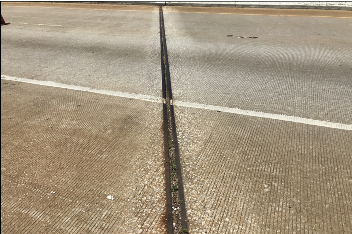
View of expansion joint at bent #16 debris impaction
