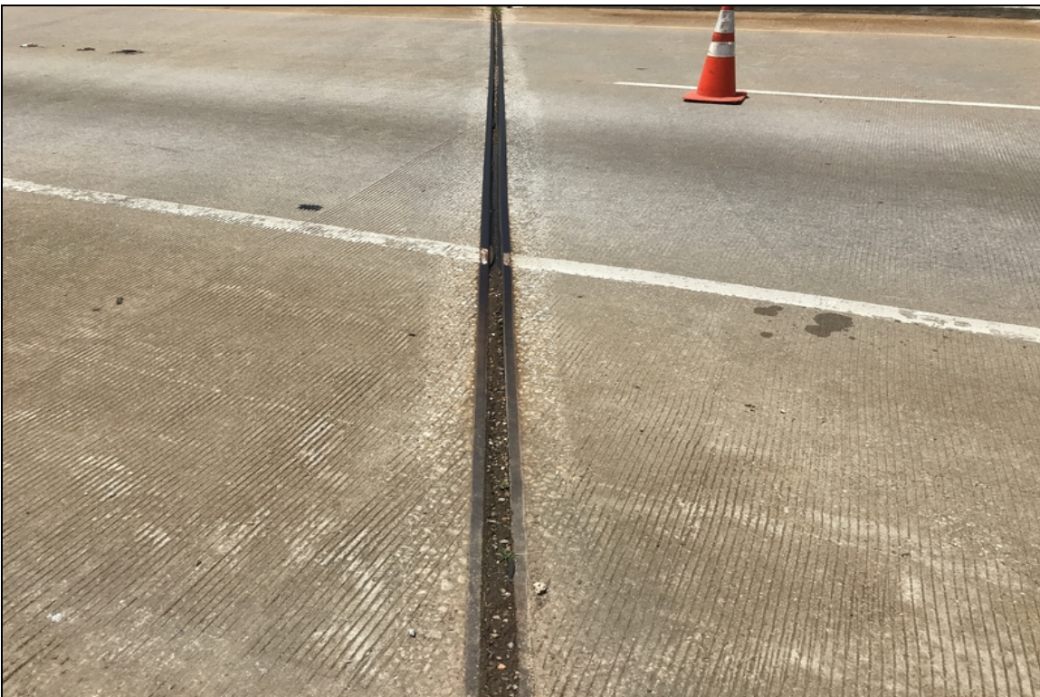
Bent #12 expansion joint debris impaction
