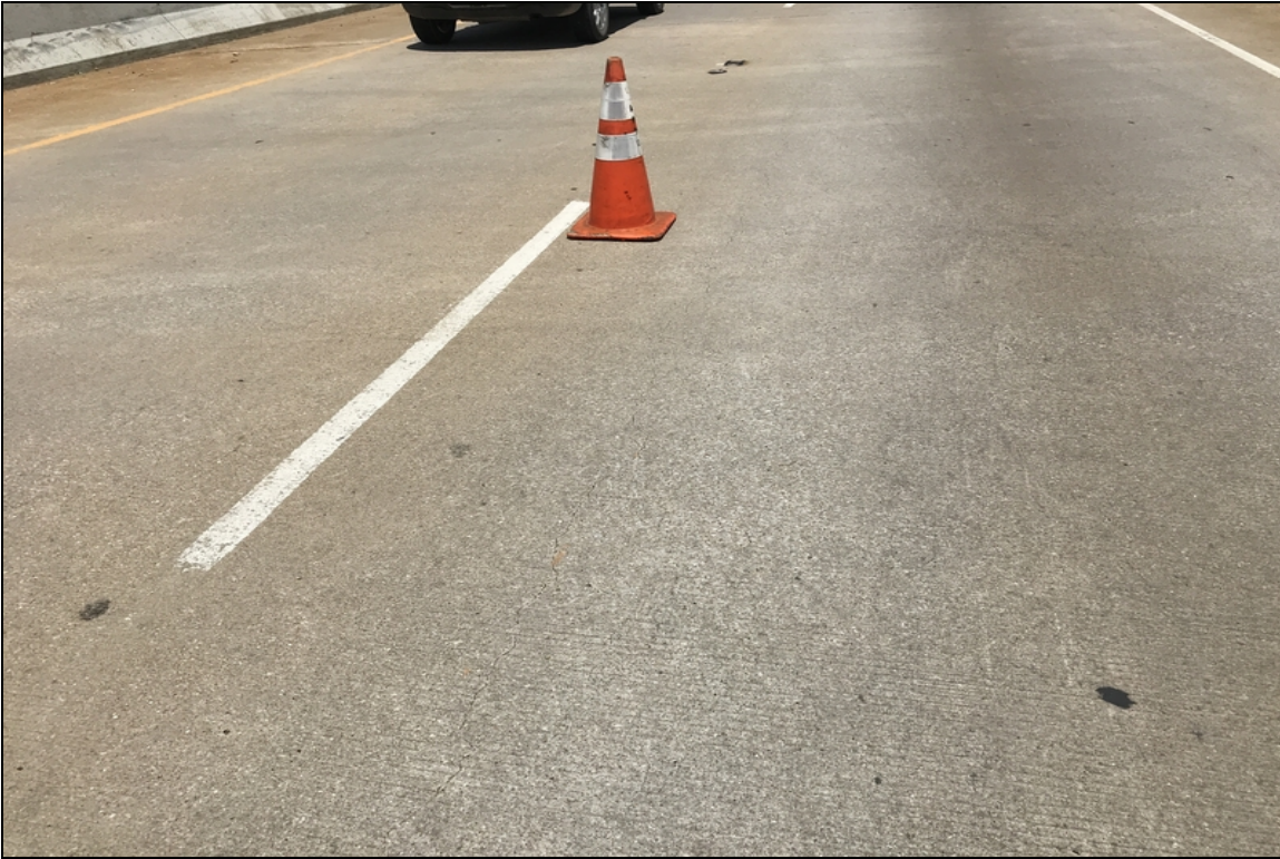
Typical view of longitudinal crack at centerline.
