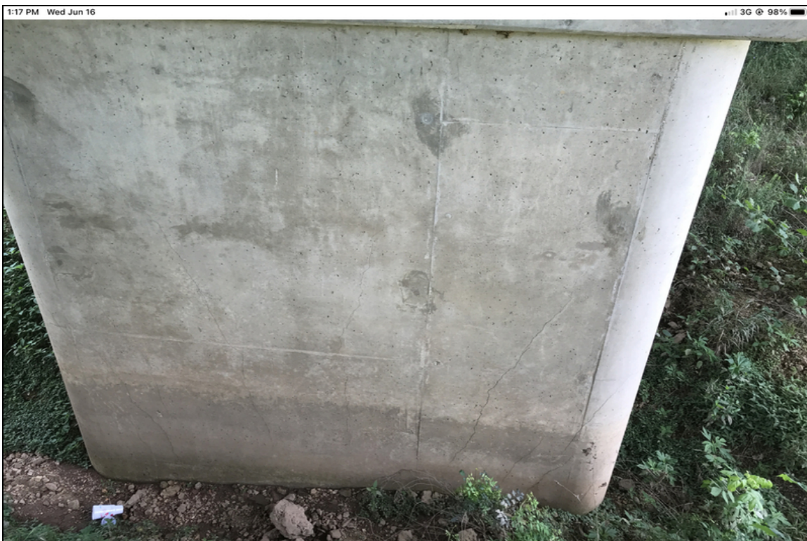
Bent #1 still has cracks present in the pier wall.
