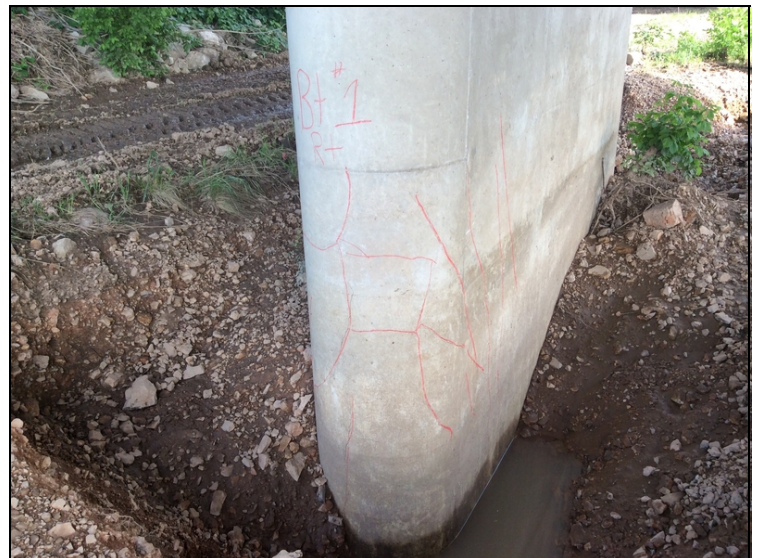
Bent #1-Cracking on right side.
