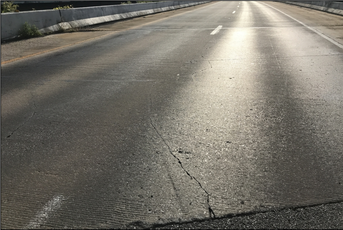
Cracking in west approach slab
