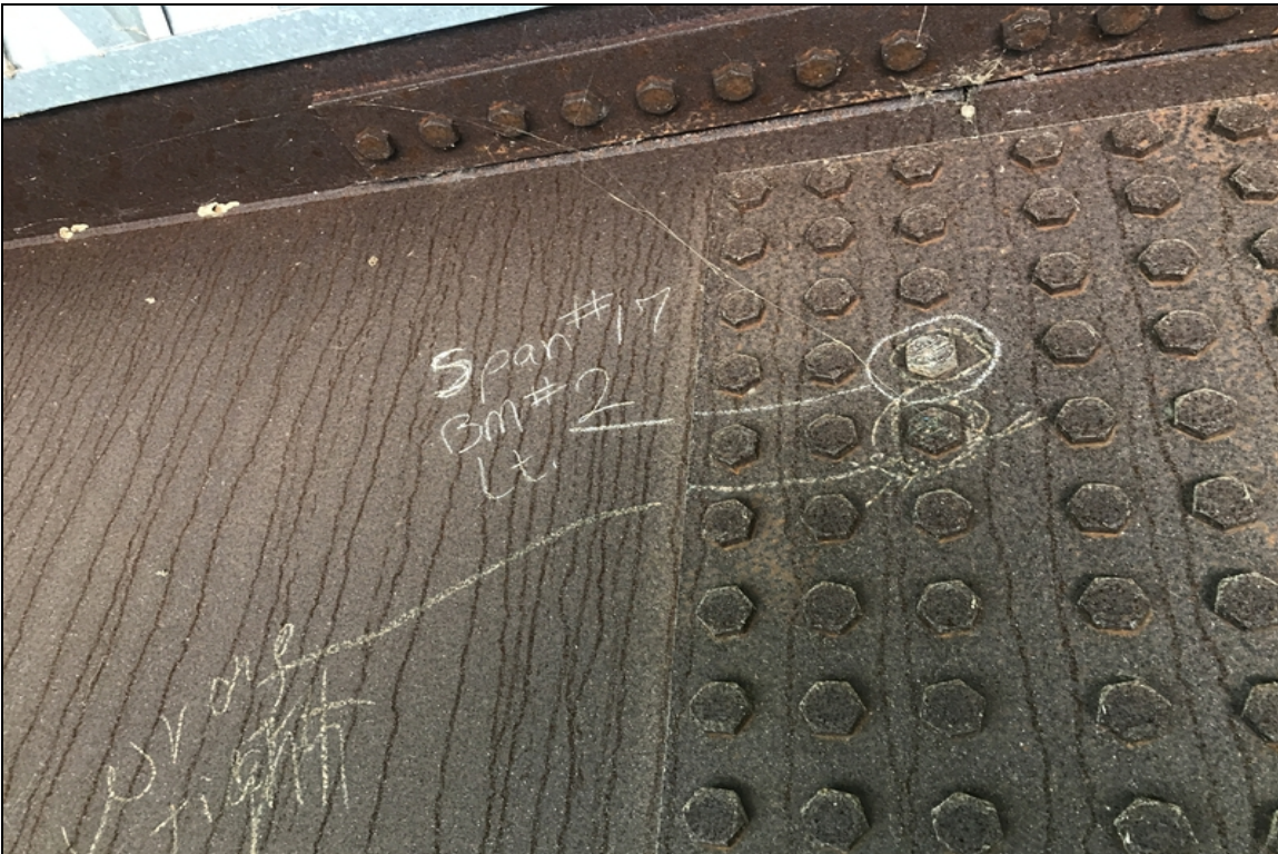
Splice bolts are still loose.
