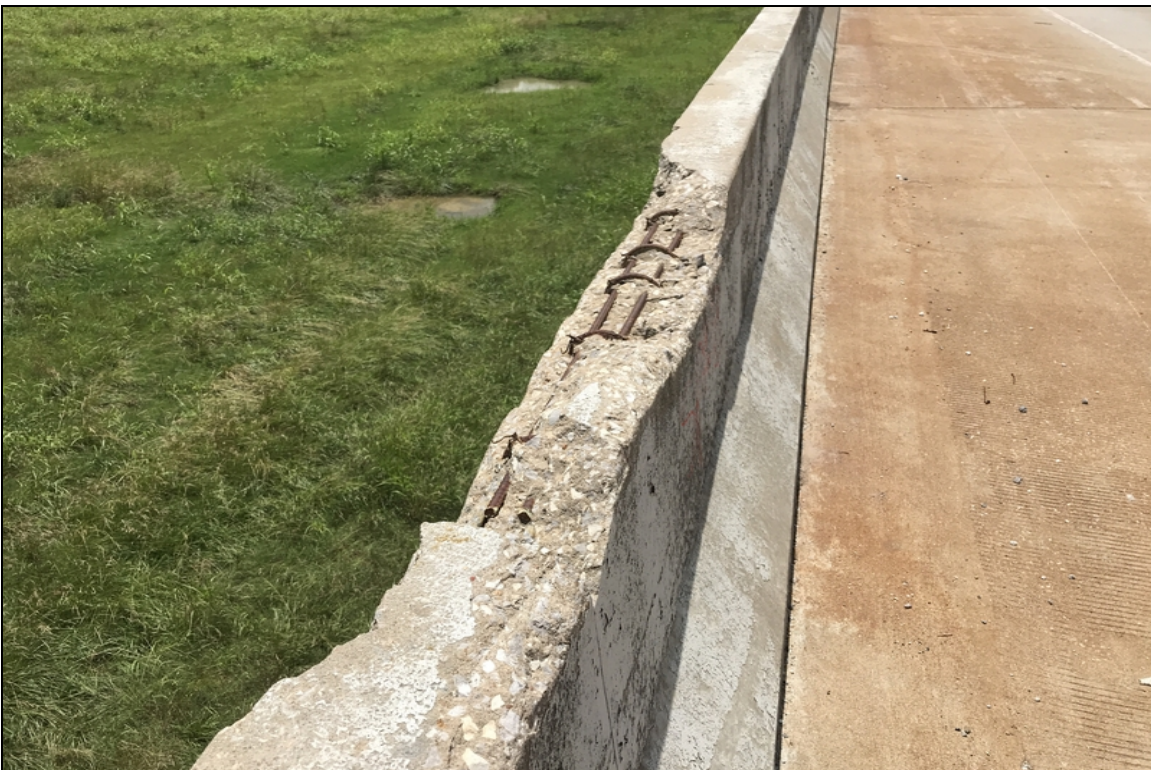
Span #8 right railing spalling with rebar exposed.
