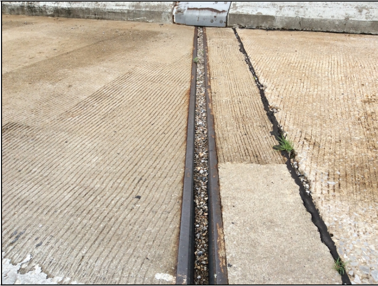
West abutment-Debris impaction.
