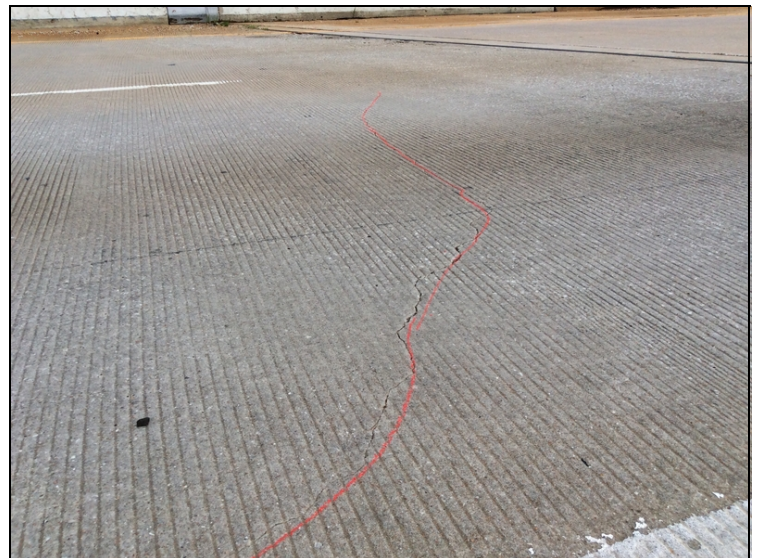
Span #19-Transverse cracking.
