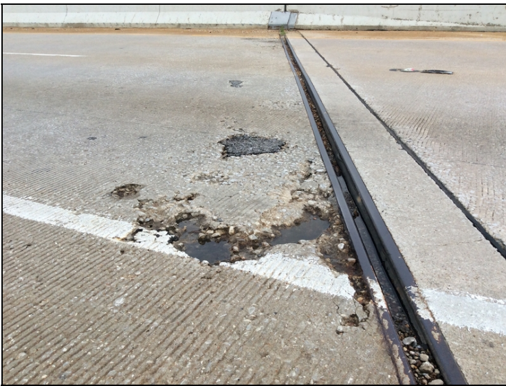
Span #19-Spalling in deck adjacent to abutment #2.
