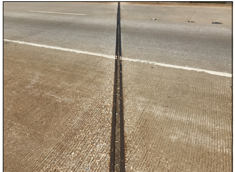
Bent #8 expansion joint debris impactation
