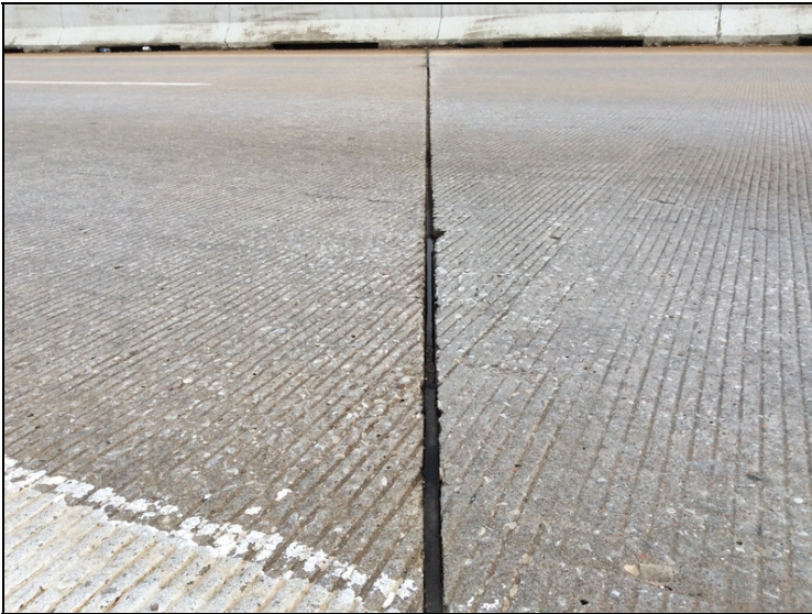
Span #10-Sawn joint material missing.
