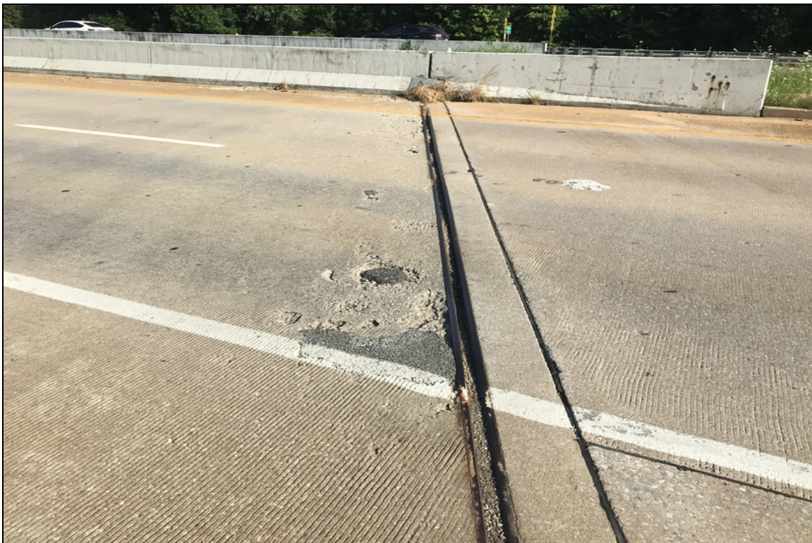
View of spalling in deck adjacent abutment #2
