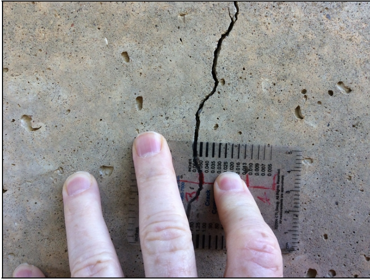
Cracking in bent #1 column. Photo #2.
