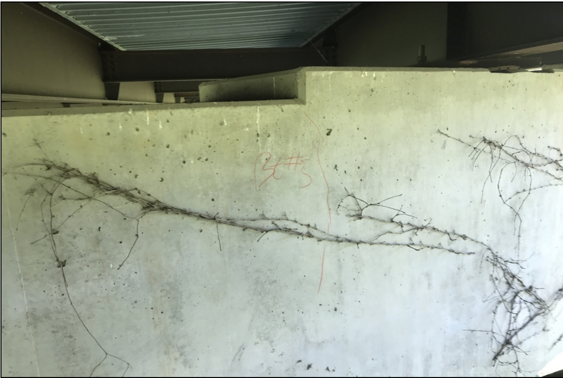
Bent #5 Typical vertical cracking in pier cap.
