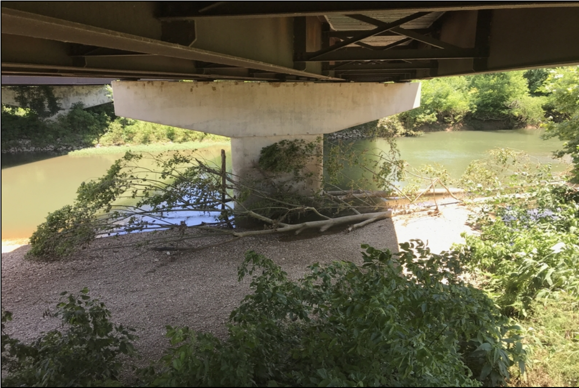
Large tree wedge against bent #17.
