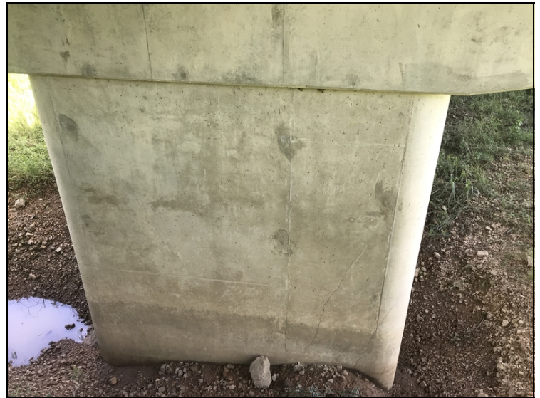
Bent #1 pier cracking in the pier.
