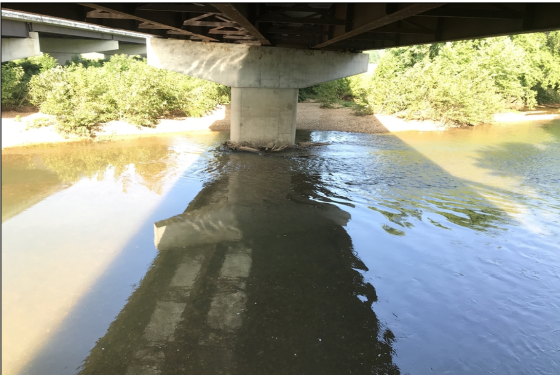
Ahead side of bent #17 - minor drift accumulation.
