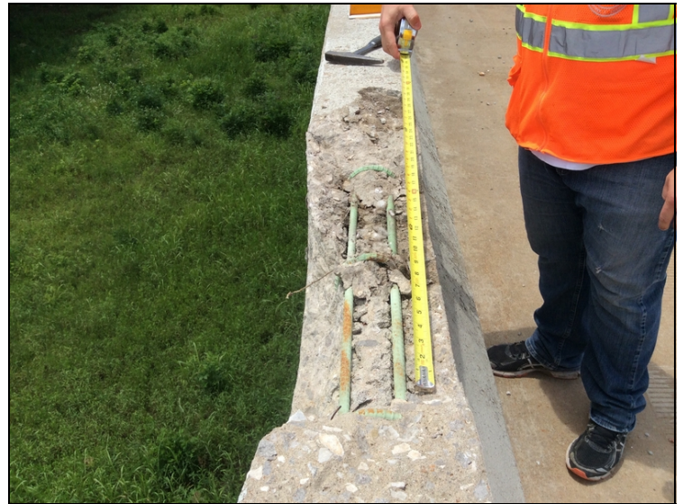
Span #4, right side-Collision damage to railing
