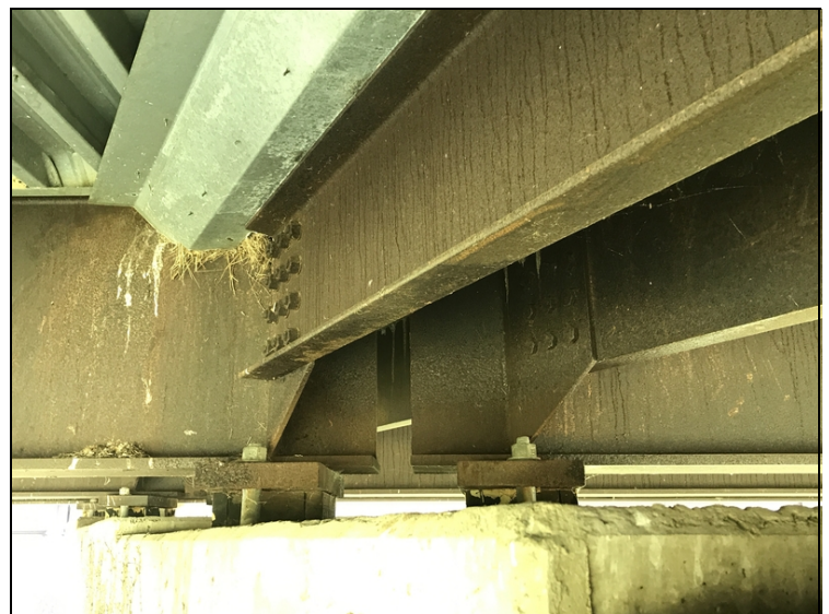
Typical Ends of Girders over bent #12 active corrosion due to leaking expansion joint.
