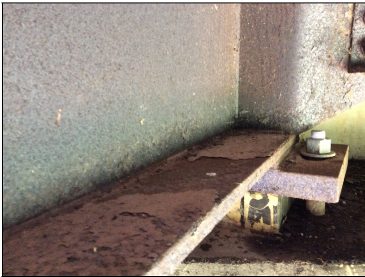
Span #17, Girder #2-Corrosion.
