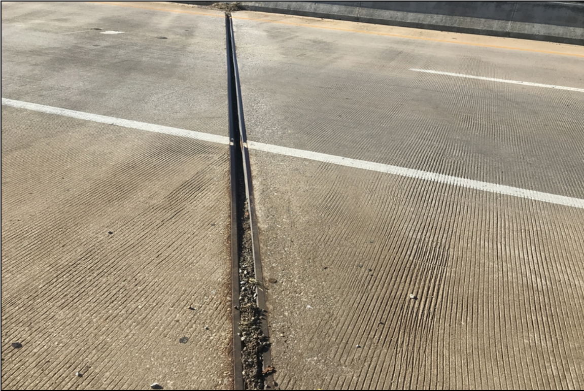
Bent #4 expansion joint
