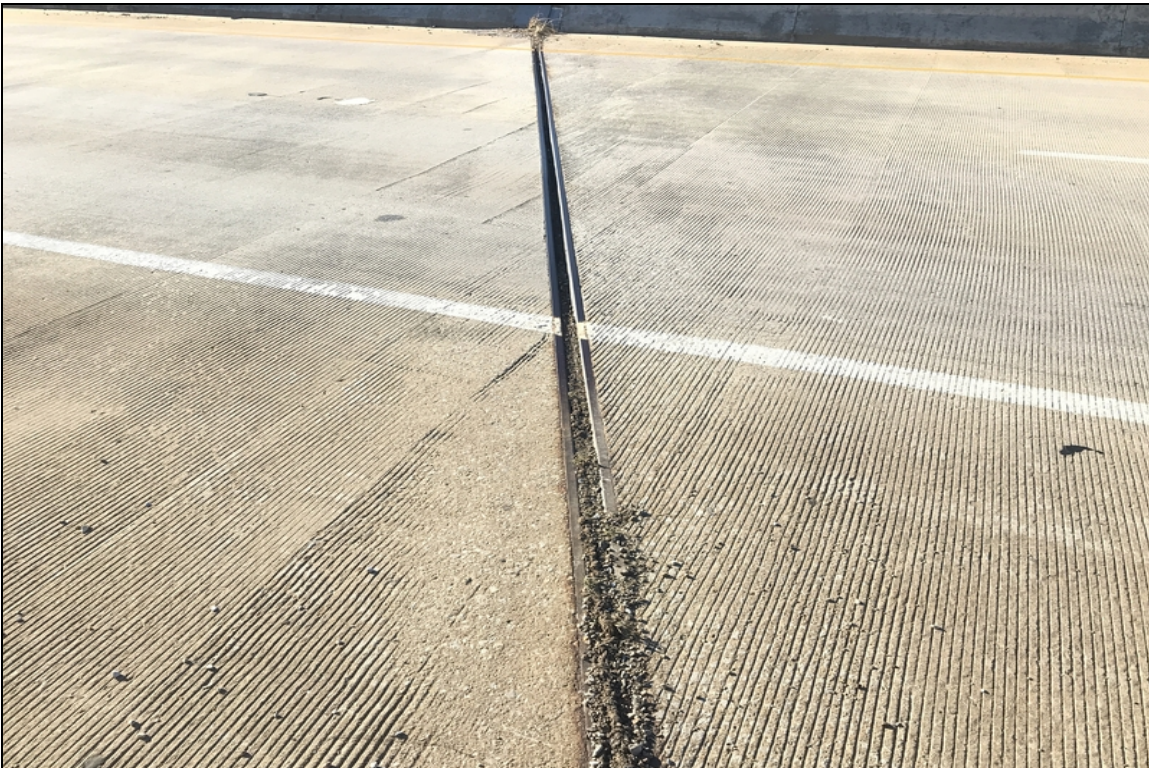
View of expansion joint at bent #12.
