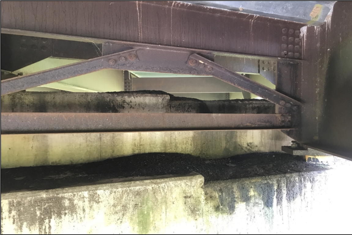
Bat droppings at bent #16 top of cap.
