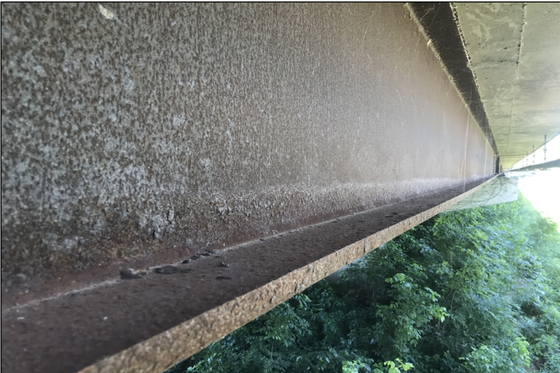
Span #16 girder #1 flaking rust
