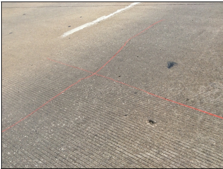
Span #19-Transverse and longitudinal cracking in driving surface.
