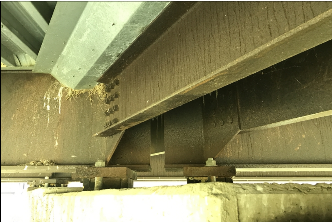
Typical Ends of Girders over bent #12 active corrosion due to leaking expansion joint.
