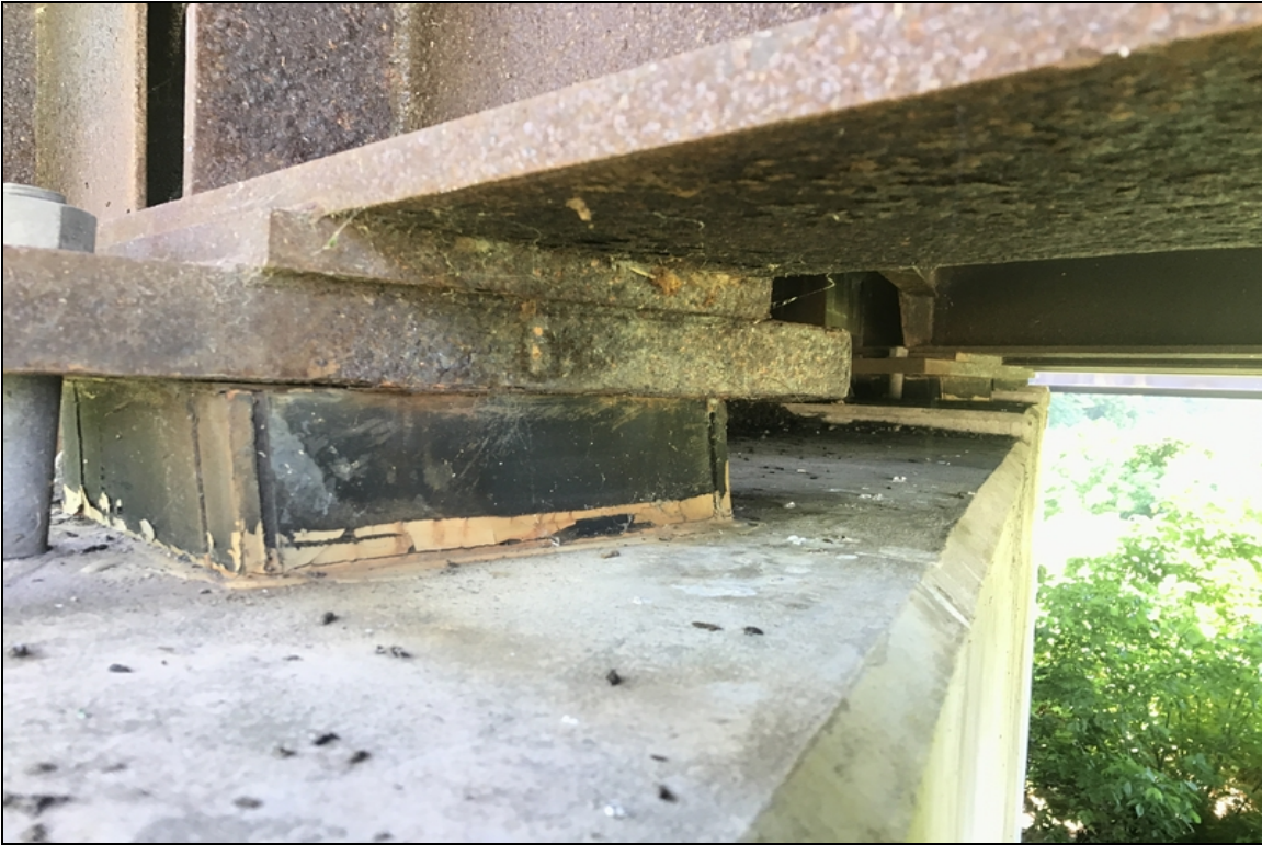
Bearing #1 at bent #16 flaking rust
