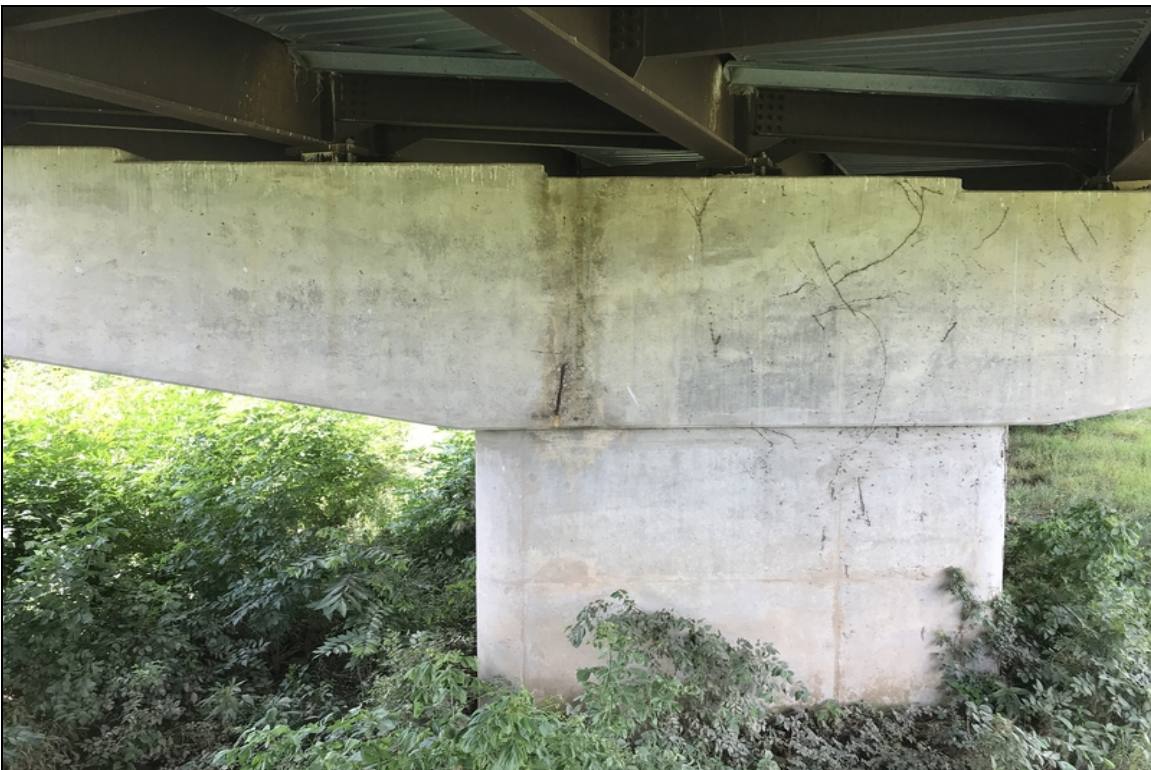
Bent cap #4 ahead side has large spall with steel exposed with minor section loss.
