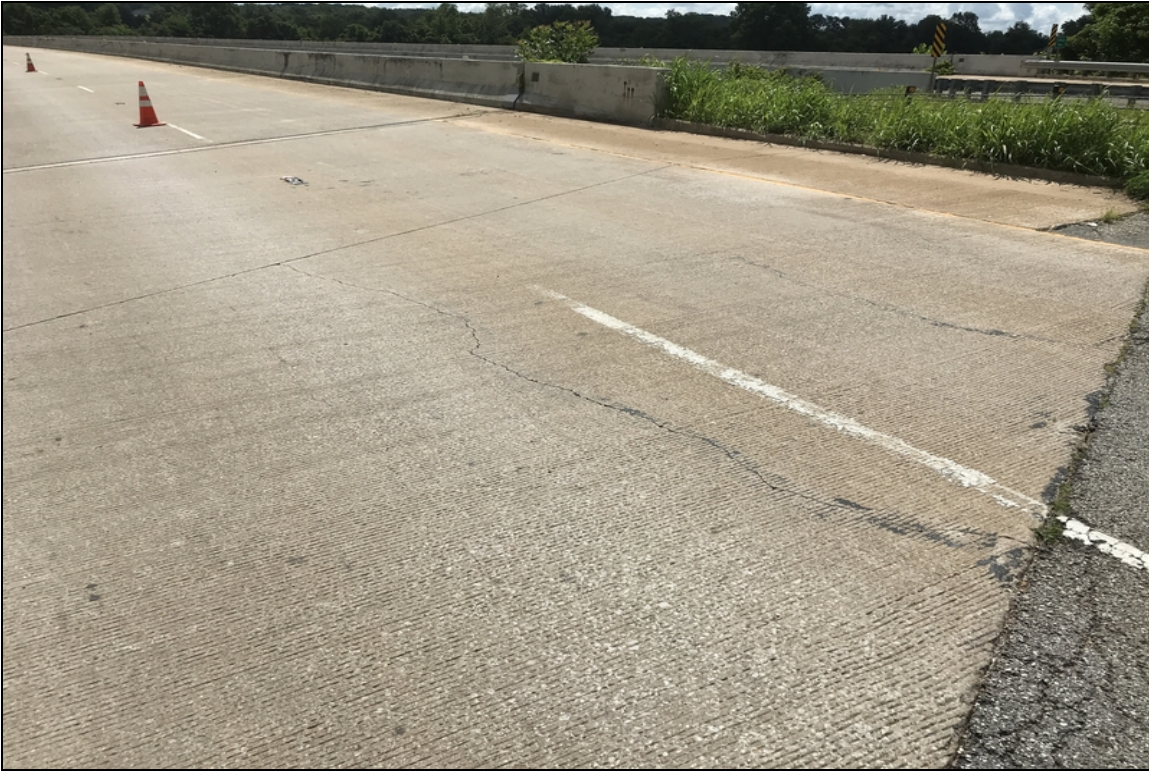
West approach slab cracking
