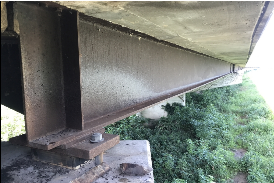
Typical of exterior girders - failing of the patina adjacent to compression joints.
