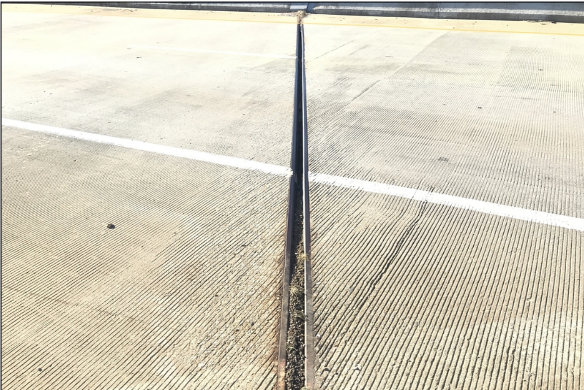
View of expansion joint over bent #8.
