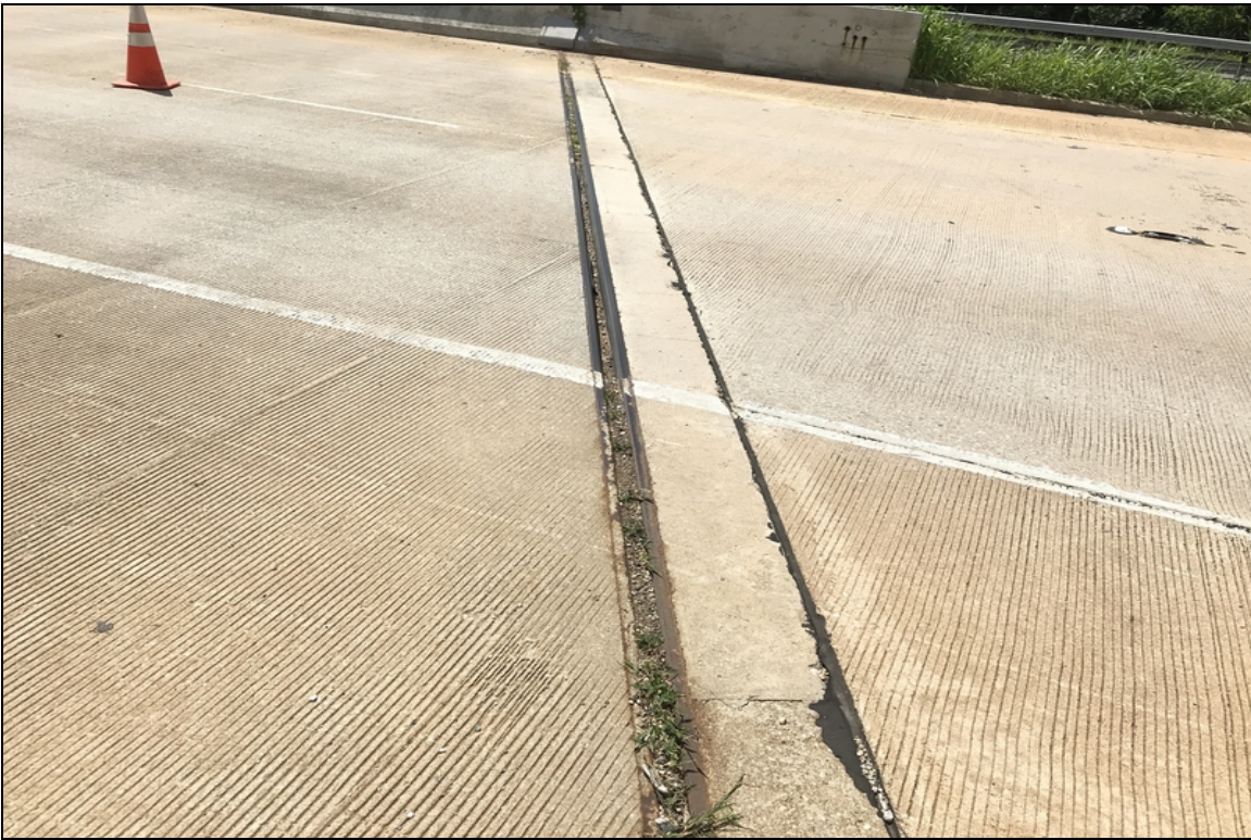
Abutment #1 expansion joint debris impact.
