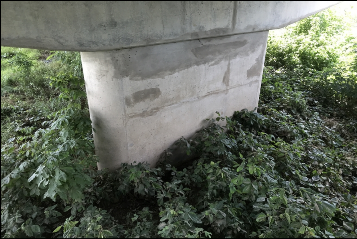
Bent #5 behind side of pier has diagonal cracking.
