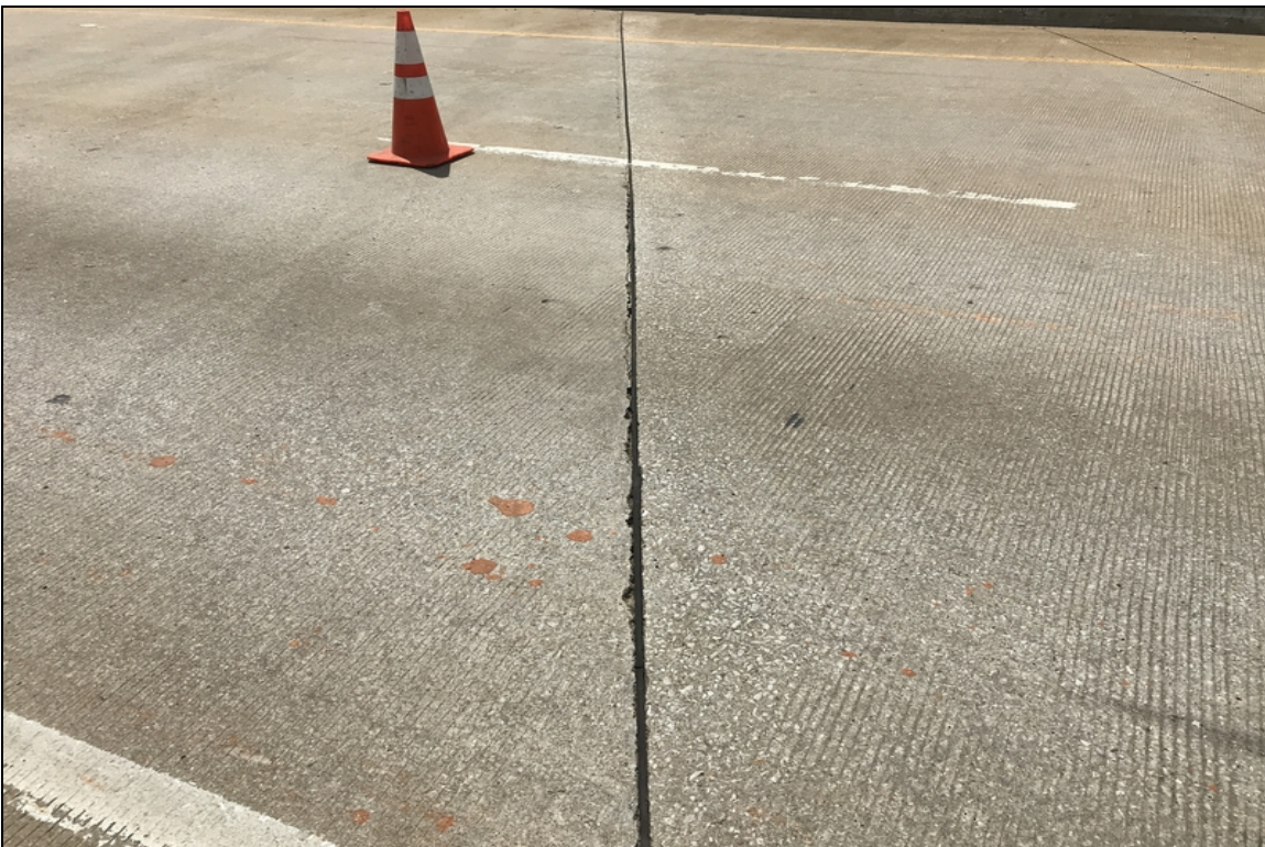
Joint material for sawn joints loss of adhesion due to spalling.
