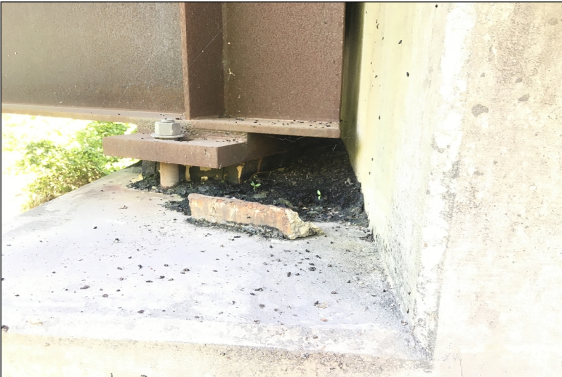
Large amounts of bat Feces accumulated on top of bent #16.
