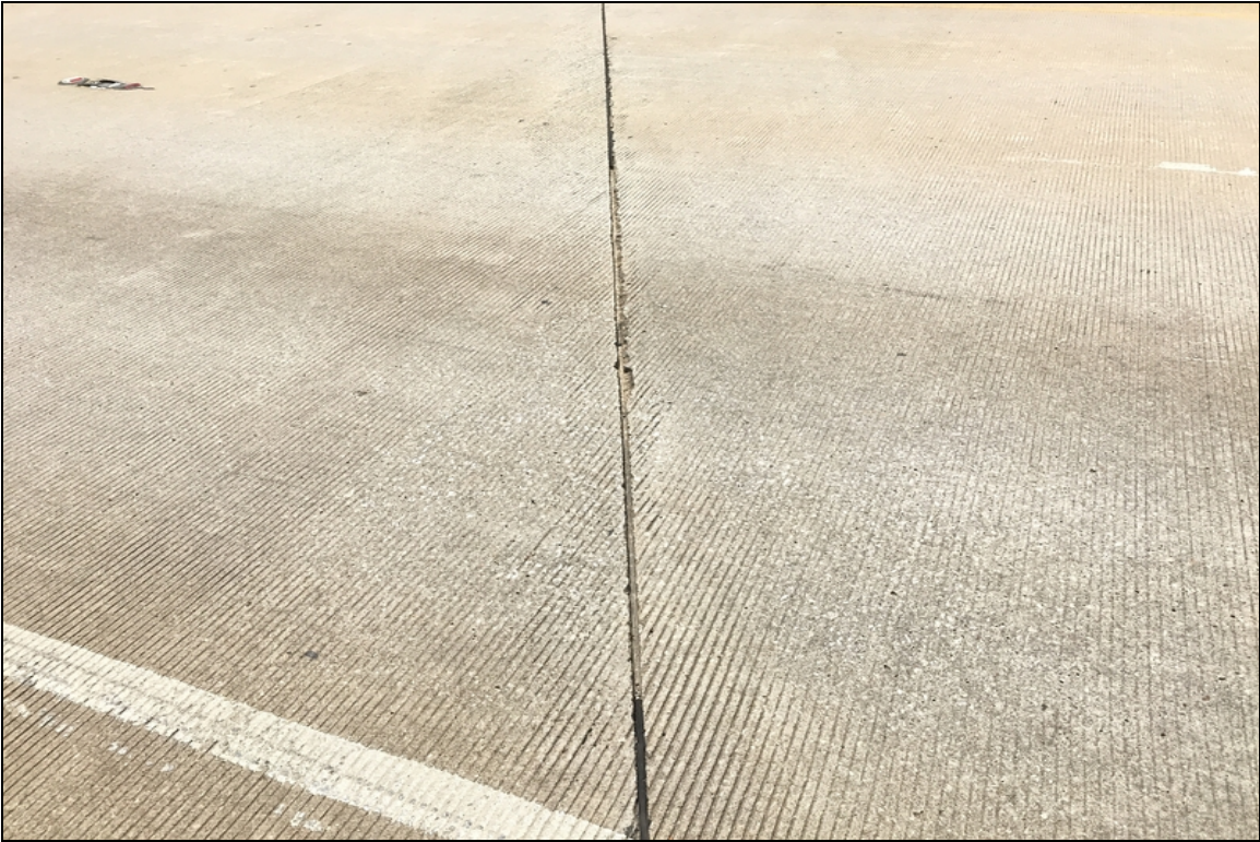
Typical - Joint material for construction joints have bent displaced in random locations.
