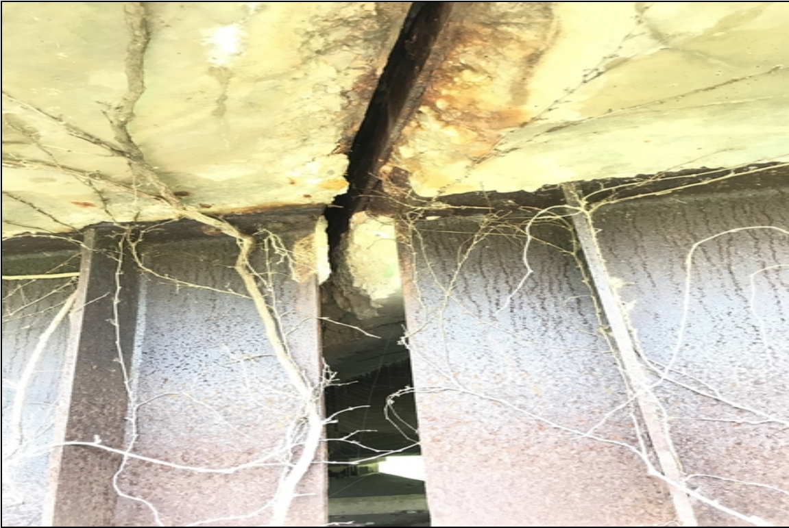
Spalling over bent #12 left epoxy coat steel exposed at the bottoms of haunch area.
