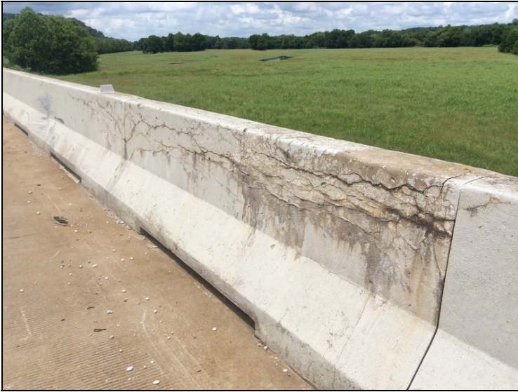
Span #7-Mapcracking in left bridge railing.
