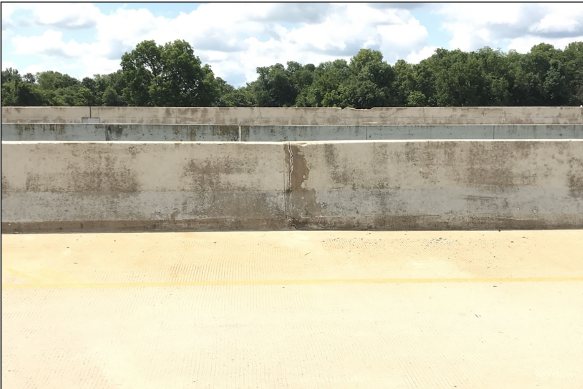
Parapet right span #8 large crack adjacent sawn joint.
