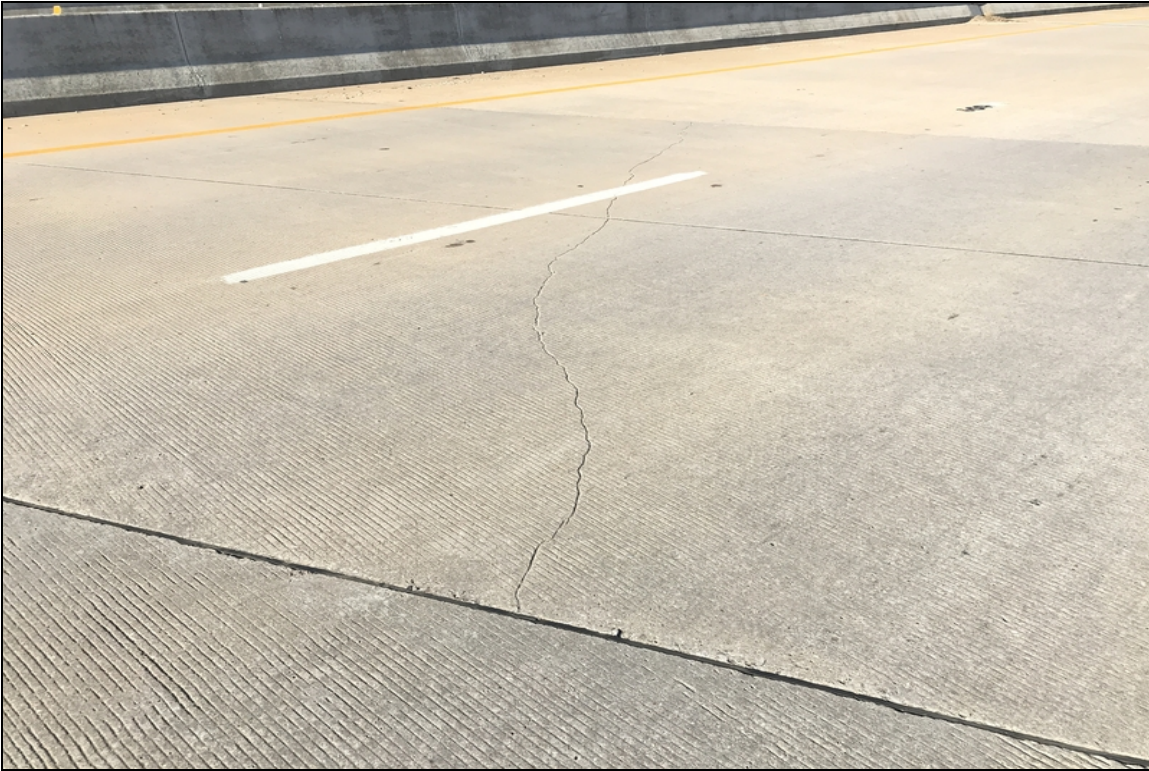
Large diagonal crack over bent #5.
