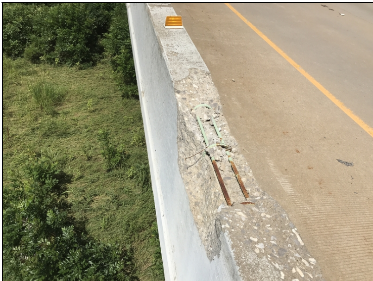
Span #4 right parapet approximately 10' behind bent #4 spalling in parapet.
