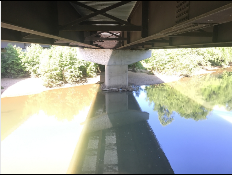
Drift still exists at bent #17
