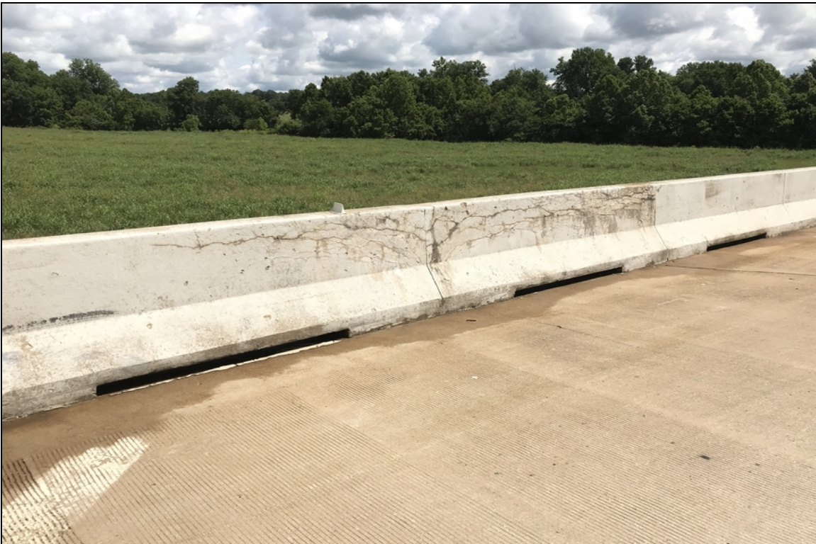
Typical cracking and efflorescence in parapet.
