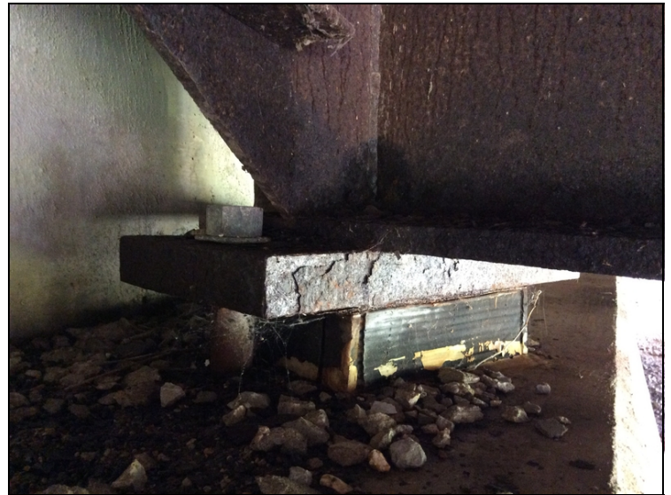
Bearing corrosion.
