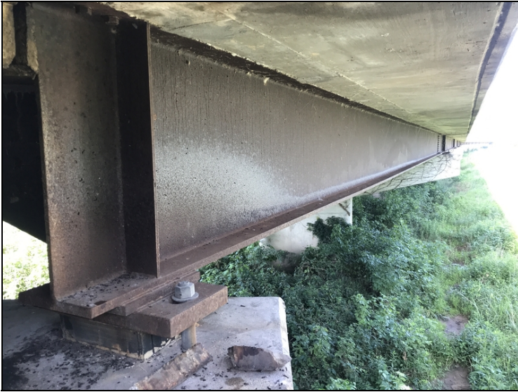
Typical of exterior girders - failing of the patina adjacent to compression joints.
