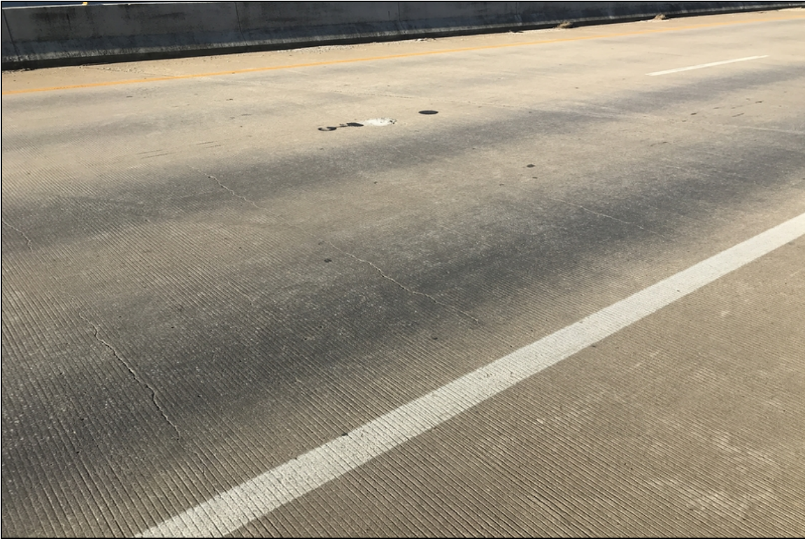
Typical cracking in deck over bent #18
