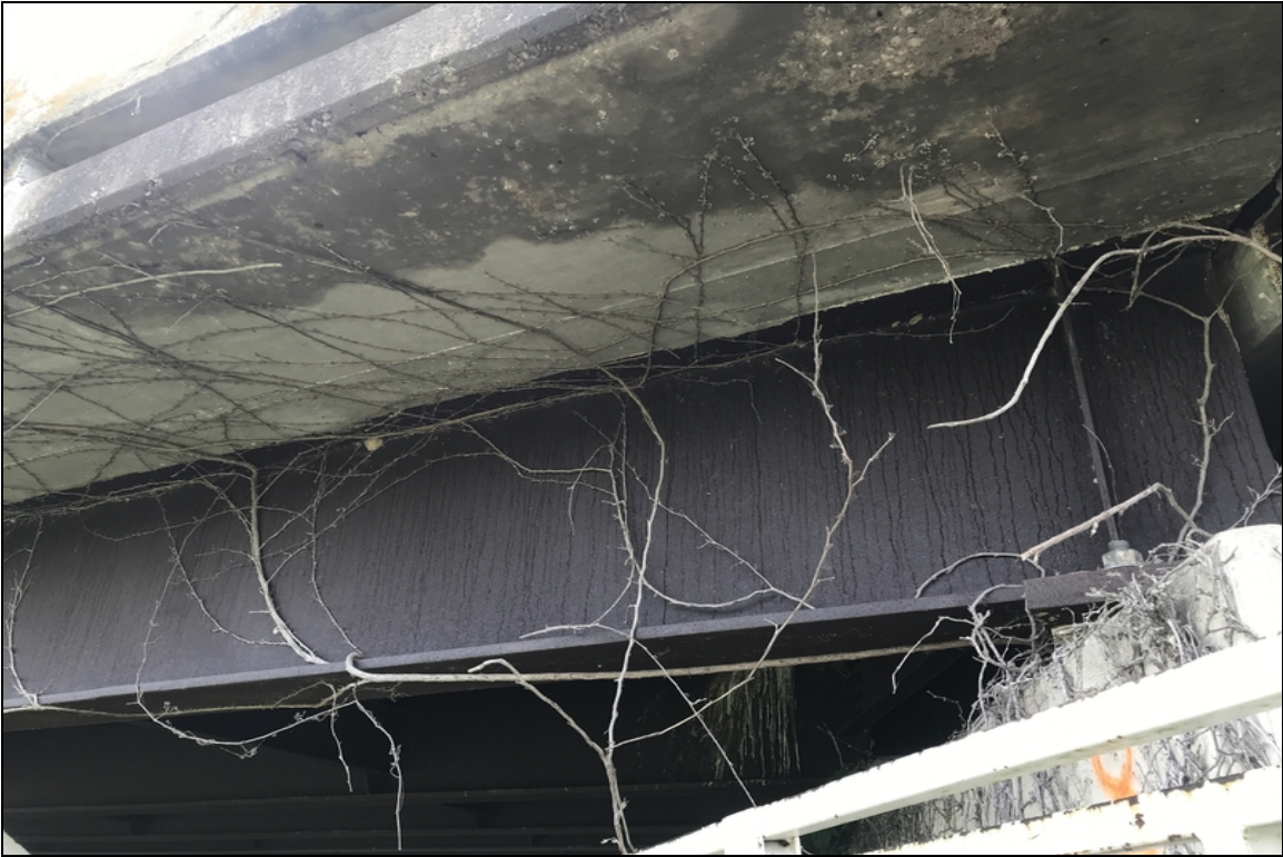
Span #9 left overhang & ahead of bent #8 honeycombed area with steel exposed.
