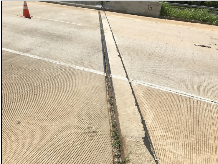
Abutment #1 expansion joint debris impactation.
