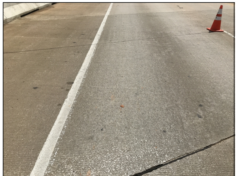
Typical cracking over bents.
