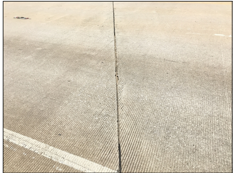
Typical - Joint material for construction joints have bent displaced in random locations.
