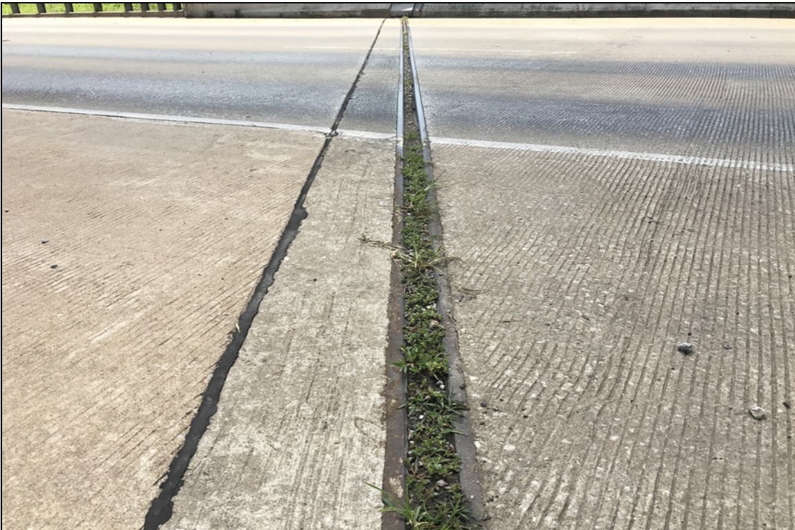
Abutment #2 expansion joint material debris impaction.
