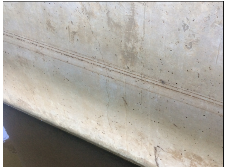
Bent #6-Vertical and diagonal cracking in column.
