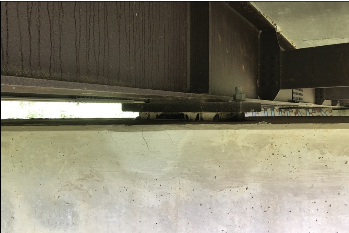
Bent #1 cap ahead side under girder #2 repaired area is cracking.
