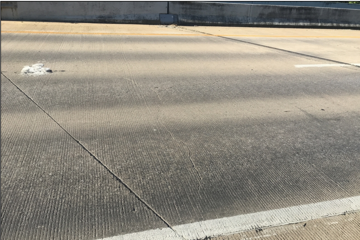
Cracking in east approach slab
