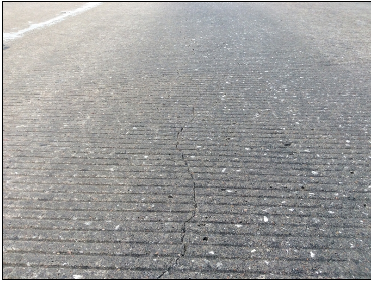
Longitudinal cracking in driving surface.
