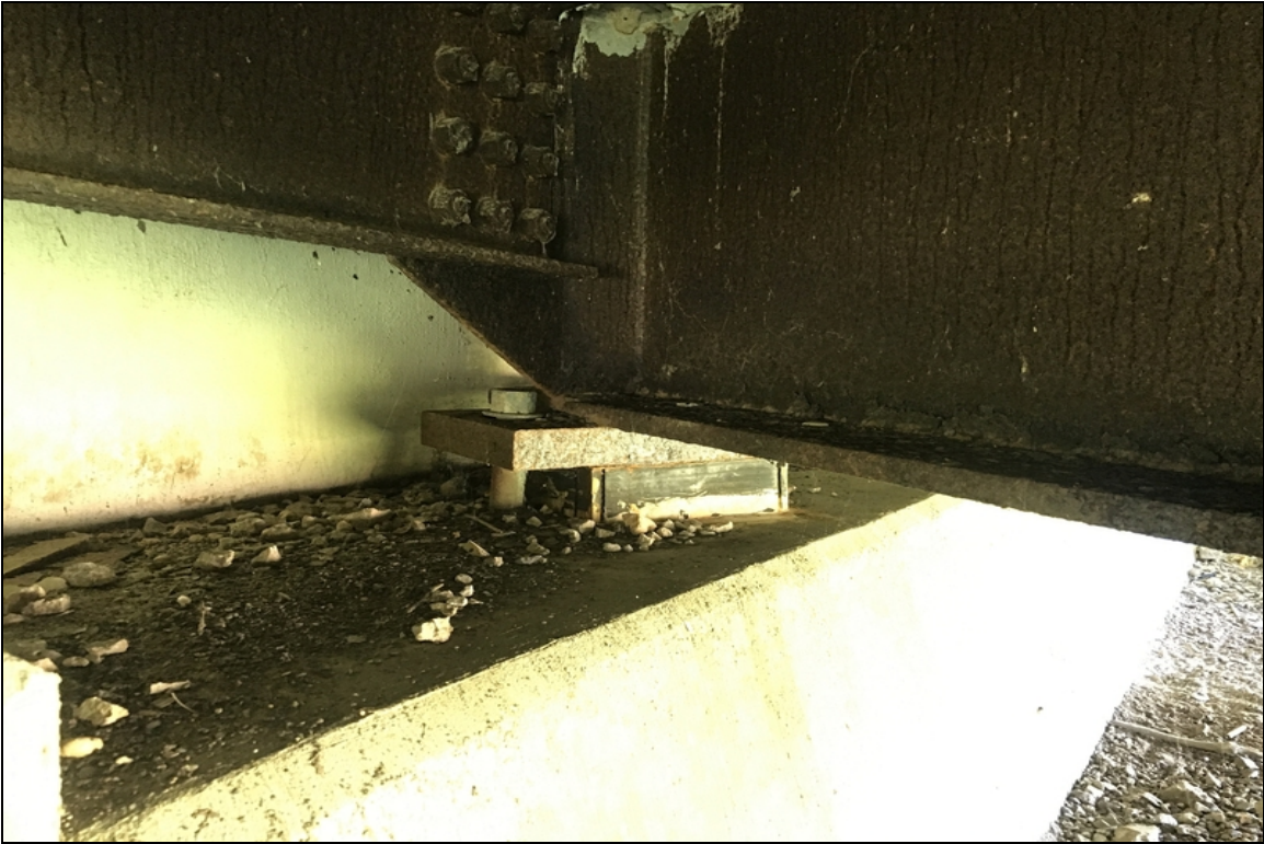
Typical flaking rust at abutment #1 for bearings and girders.
