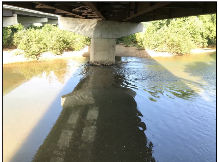
Ahead side of bent #17 - minor drift accumulation.
