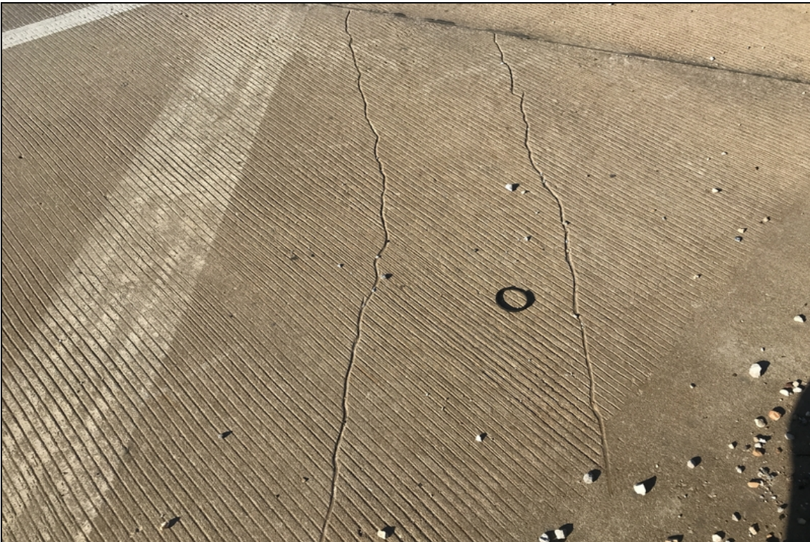
Additional diagonal cracking at bent #5 cracking repairs are not holding as of this inspection
