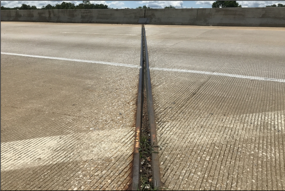
Bent #7 expansion joint minor debris impaction.
