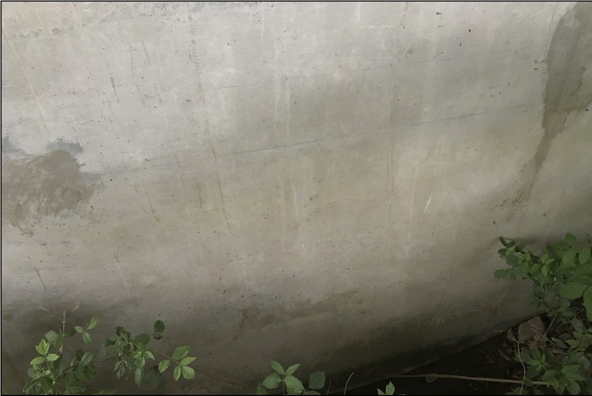
Bent #10 base of column has 3 narrow short duration vertical cracks. Visible from the ahead side.
