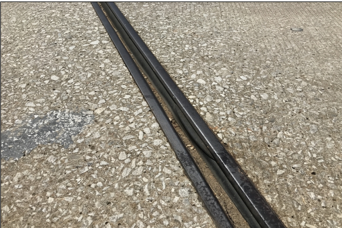
Typical view of expansion joint material coming loose from connection allowing leakage.
