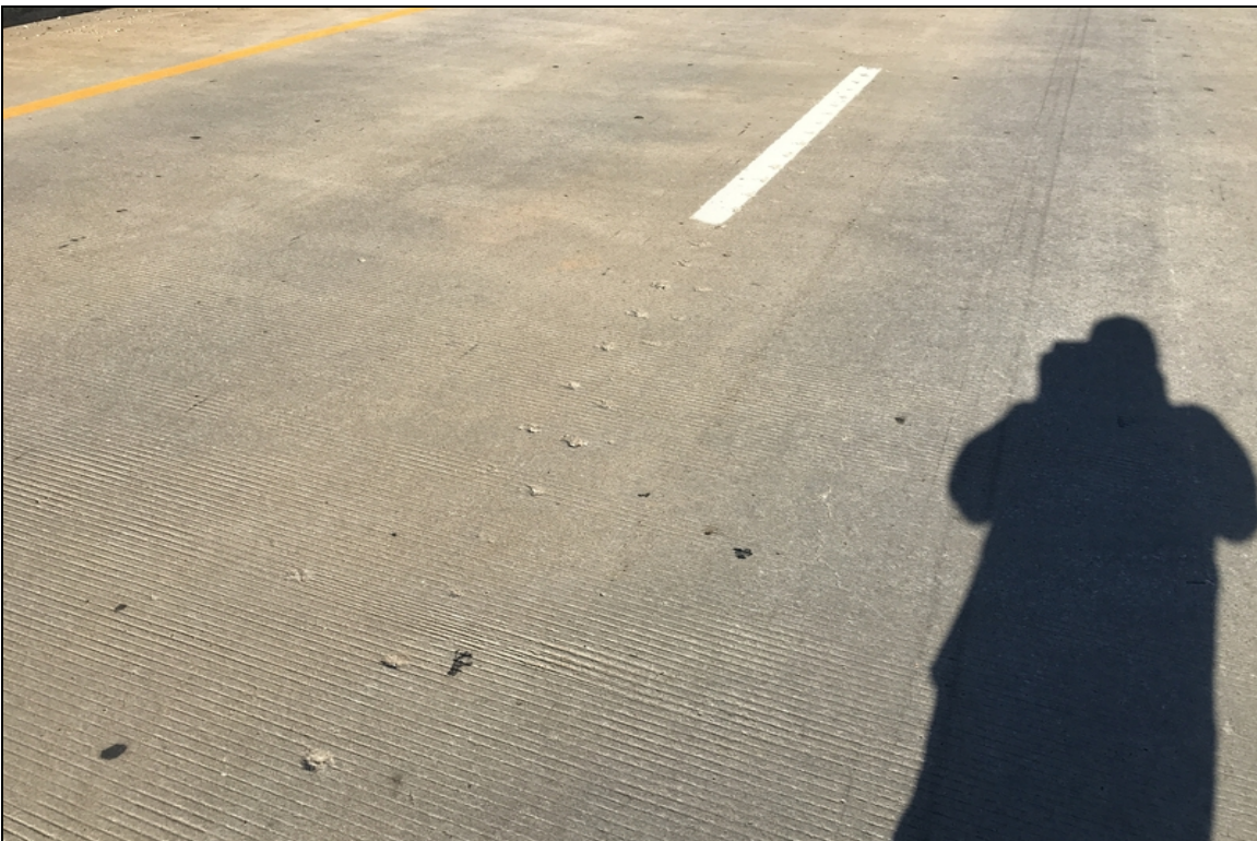
Limited cover over shear pins has caused multiple pop outs.
