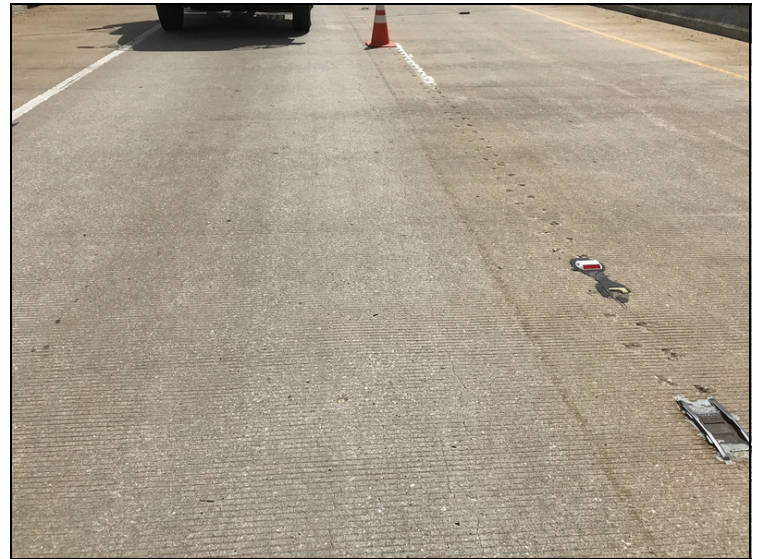
Span #3 typical longitudinal cracking.
