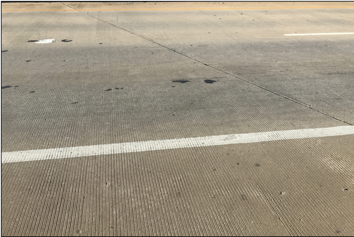
View of diagonal cracking propagating from construction crack over bent #14.
