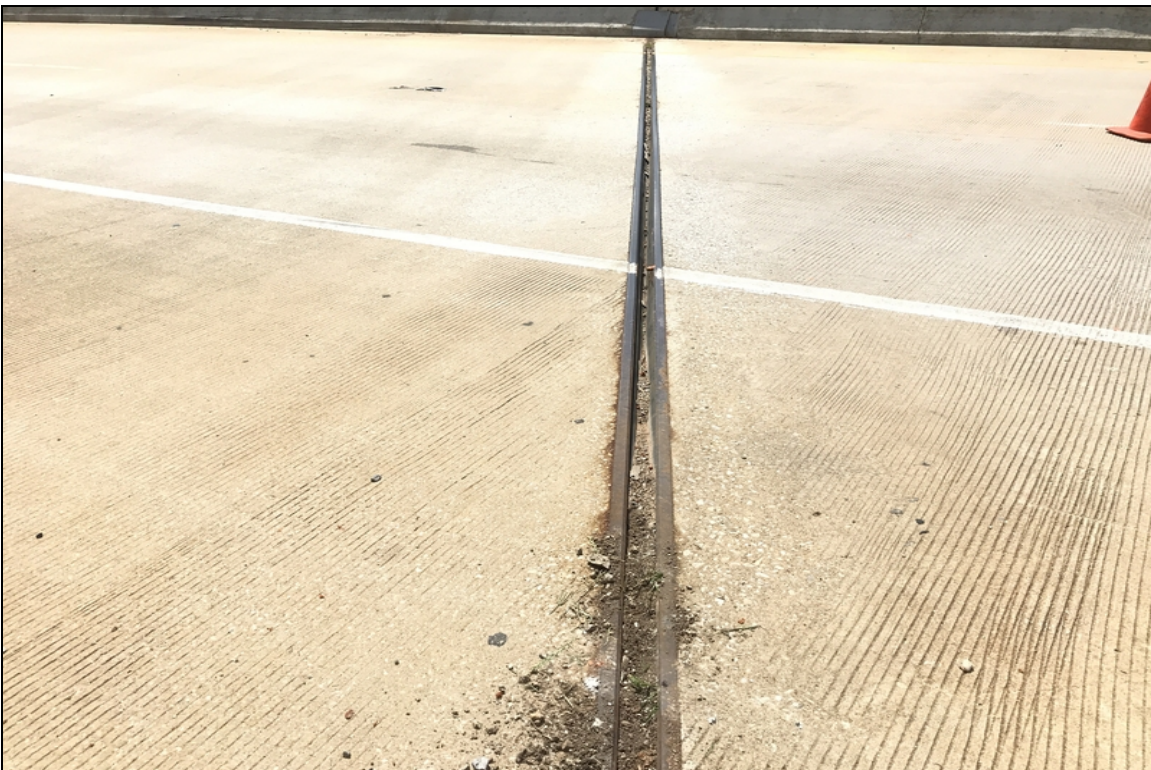
Expansion joint over bent #4 debris impact.
