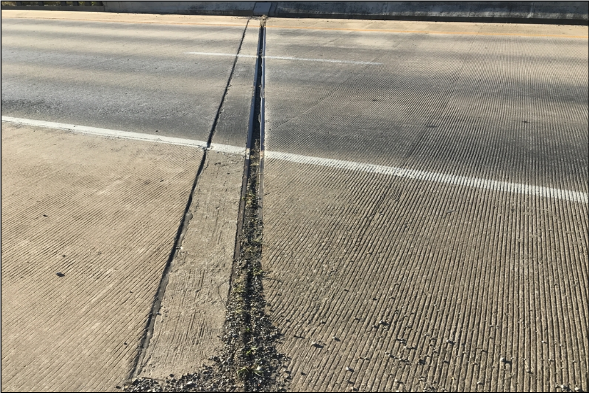
View of abutment #2 expansion joint
