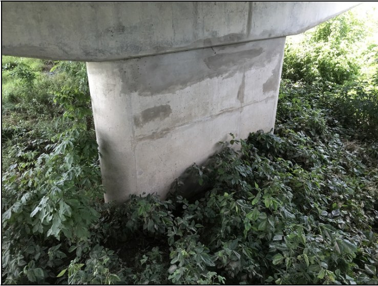
Bent #5 behind side of pier has diagonal cracking.
