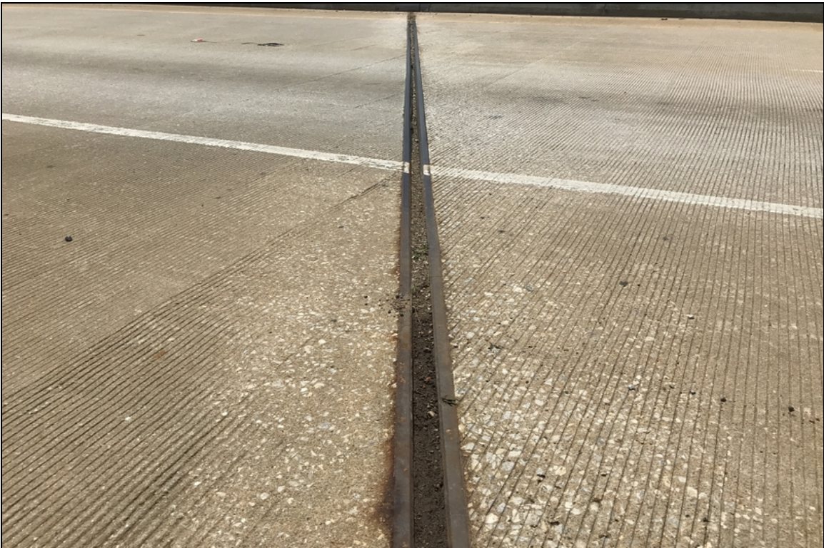
Expansion joint over bent #12 debris impaction.
