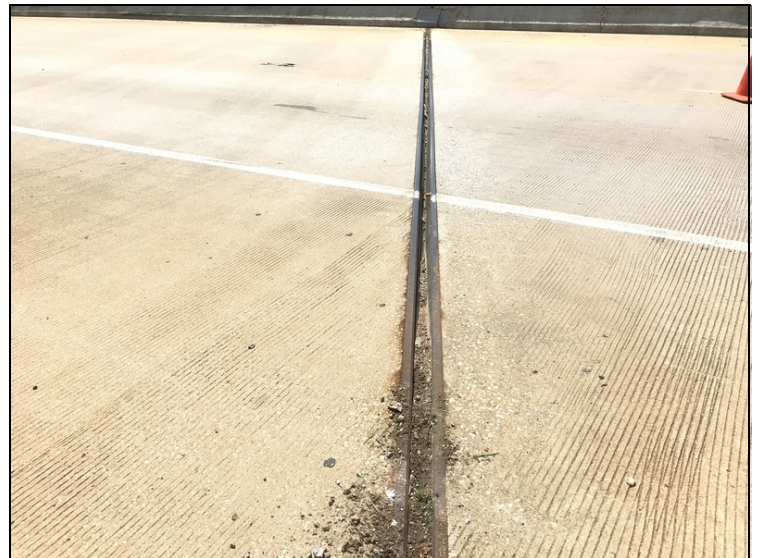
Expansion joint over bent #4 debris impactation.
