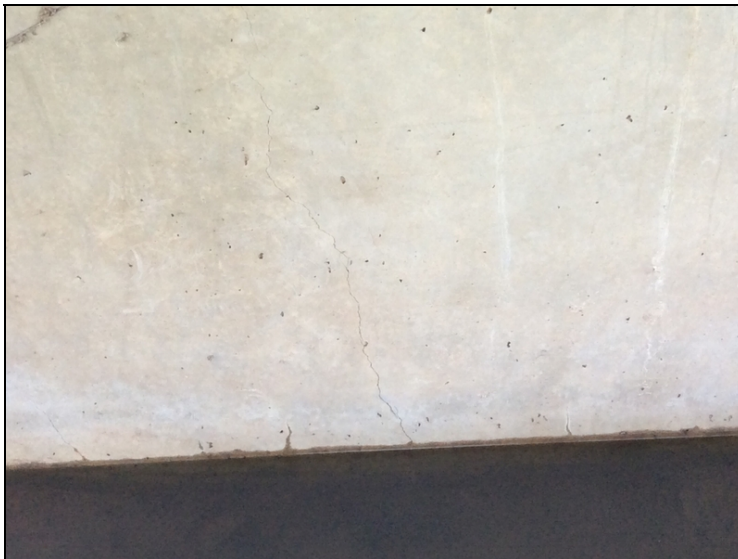
Bent #9-Vertical cracking.
