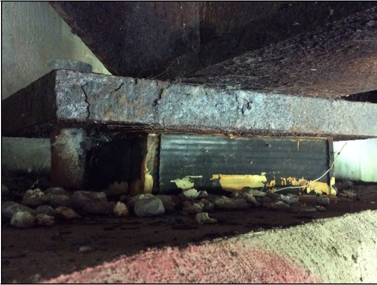
Abutment #1, bearing #3-Corrosion with flaking rust.
