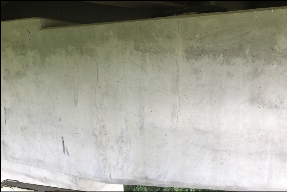
Ben #7 cap ahead side - tall hairline vertical cracking at random locations throughout the cap.
