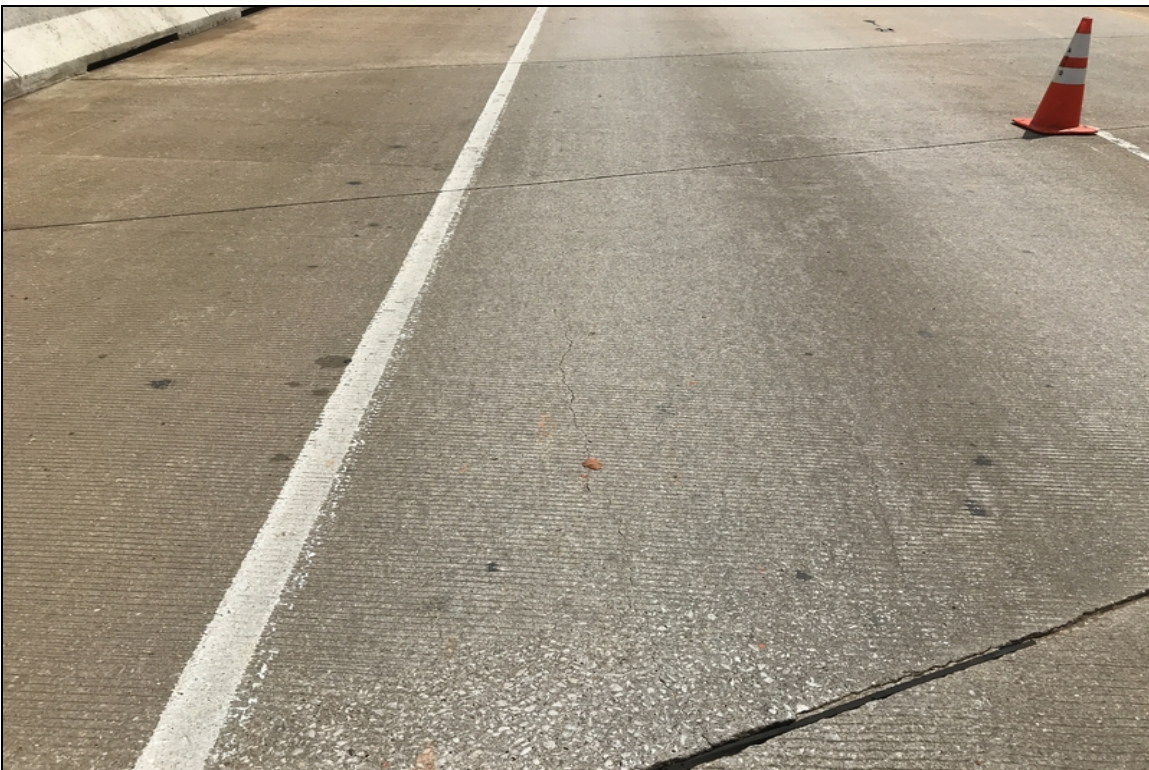
Typical cracking over bents.
