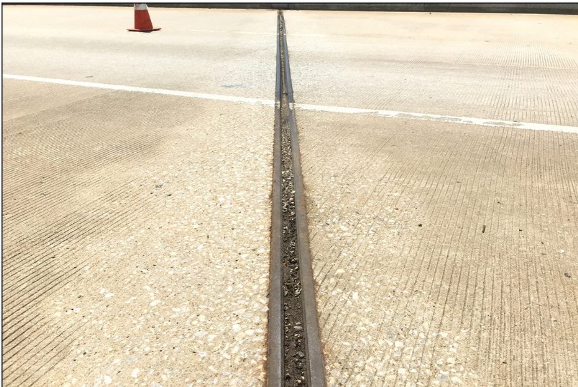
Expansion joint over Bent #16 debris impaction.
