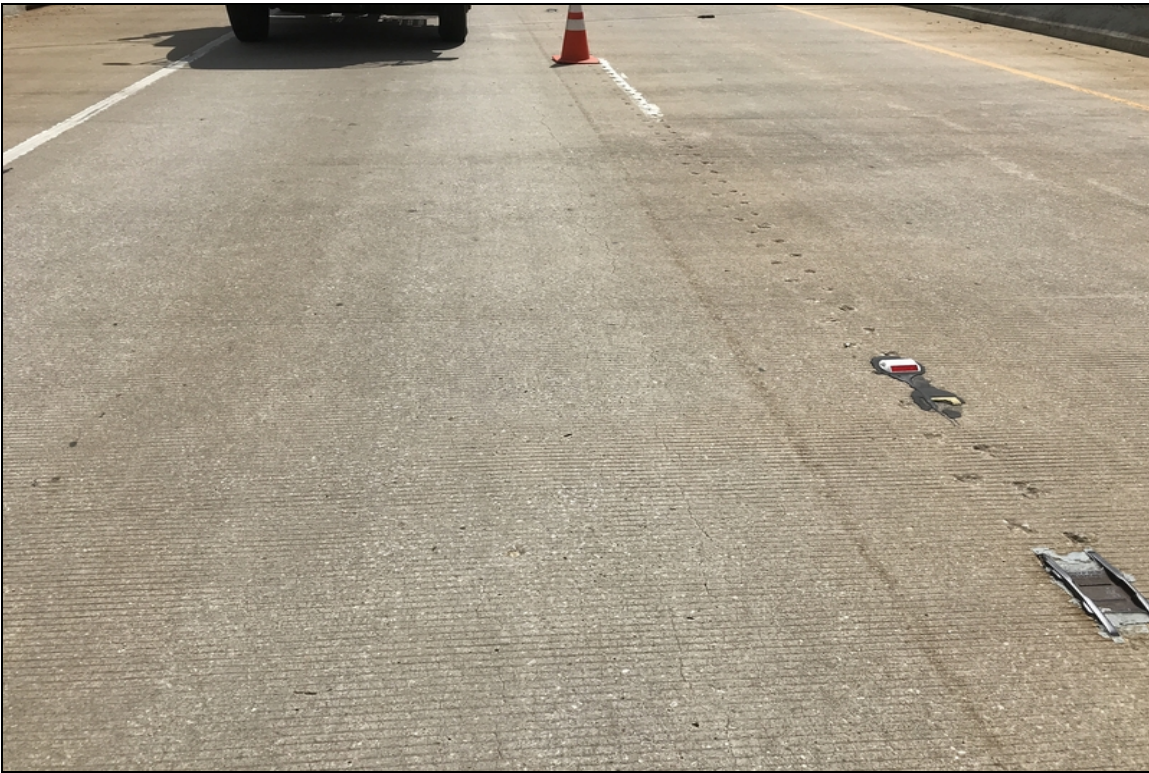
Span #3 typical longitudinal cracking.
