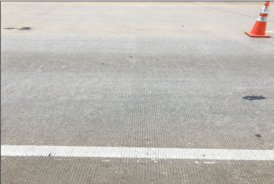
Span #17 left typical transverse cracking.
