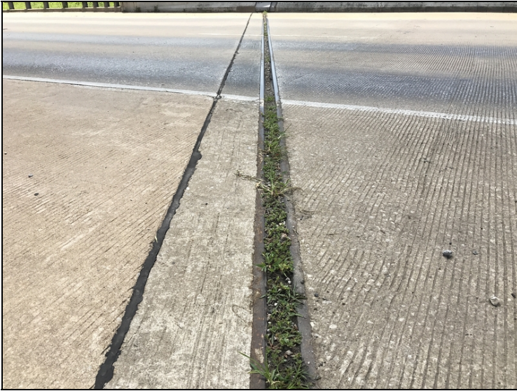
Abutment #2 expansion joint material debris impaction.
