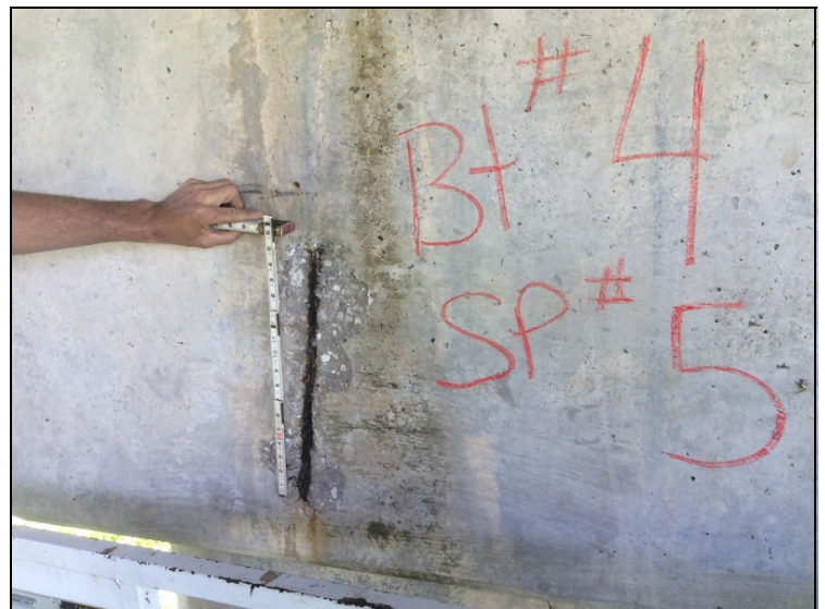
Bent #4 cap-shallow spalling with exposed reinforcing steel.
