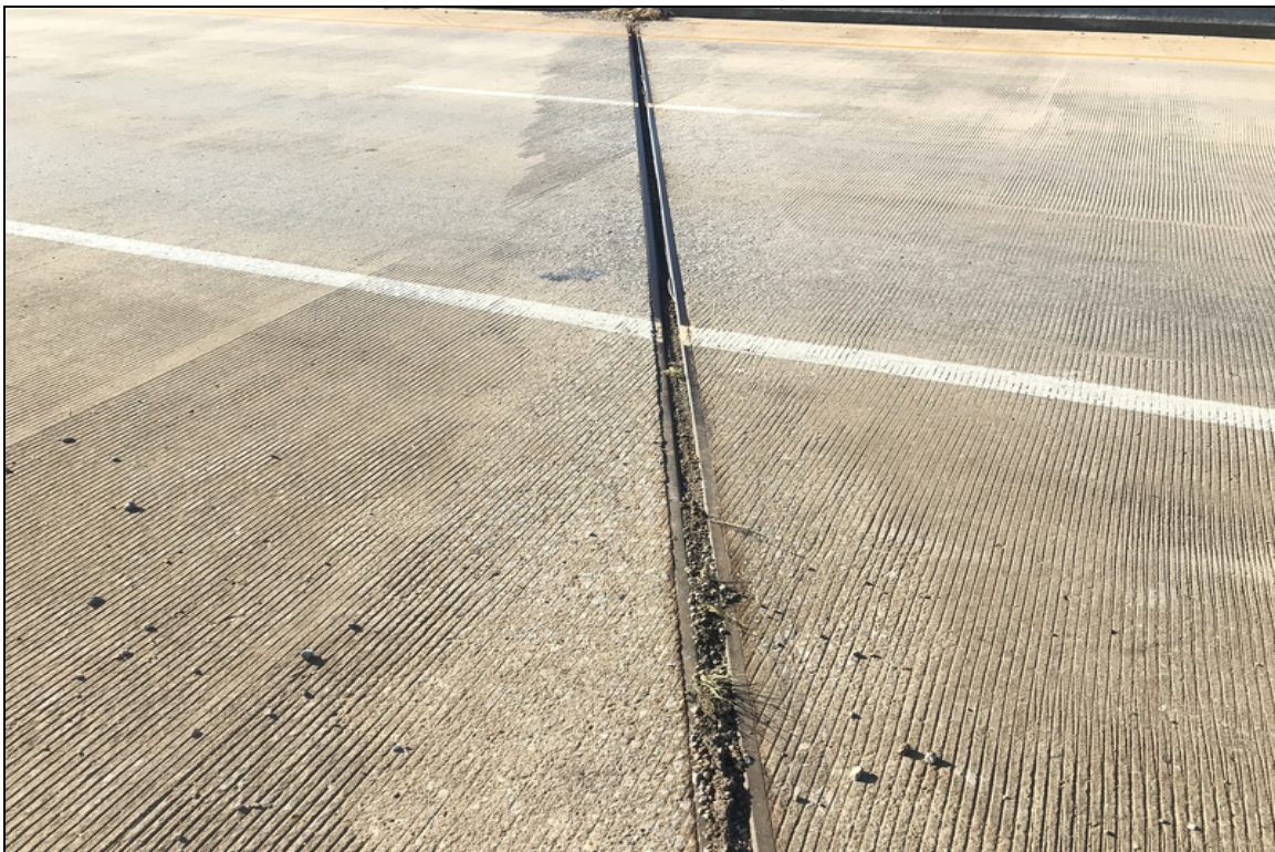
View of expansion joint at bent #16
