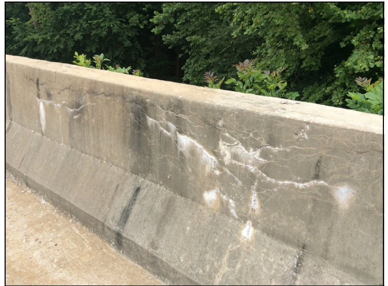
Span #1, right side-Mapcracking with efflorescence.
