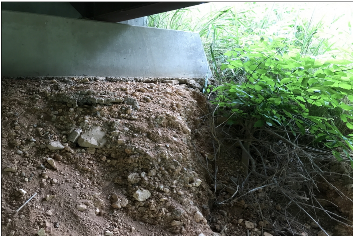
Right side of abutment #2 erosion.
