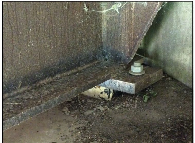
Abutment #2, beam #4-Corrosion due to leaking expansion joint.
