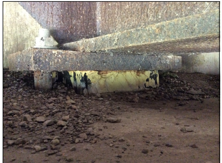
Excessive corrosion due to leaking expansion joint.
