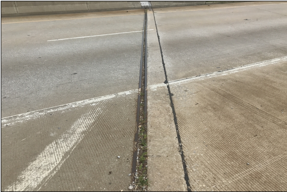
General view of abutment #2 compression joint debris impact.
