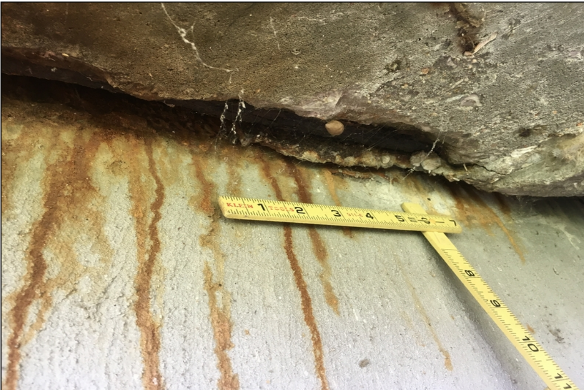
Spalling with rebar exposed on the deck undersurface at the left corner at the end of span #3
