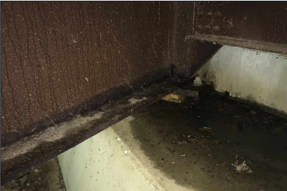
Girder #3 over abutment #1 active corrosion due to leaking compression joint.
