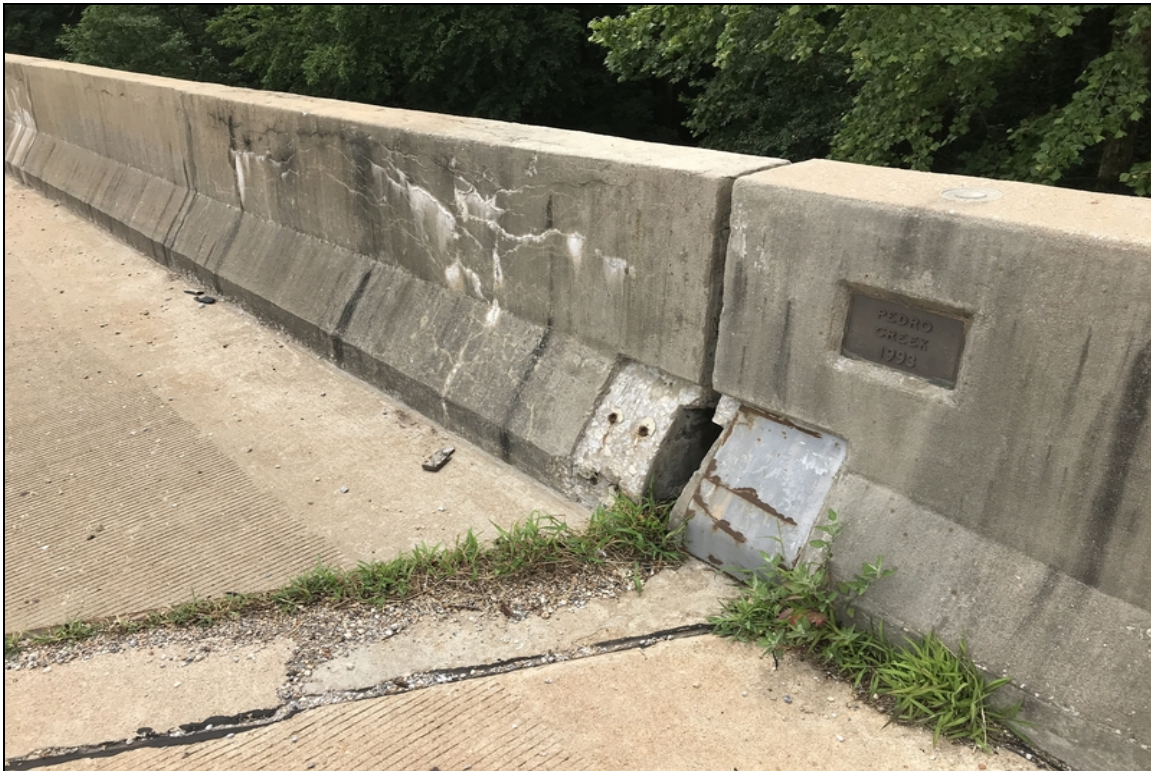
Expansion plate on right parapet missing.
