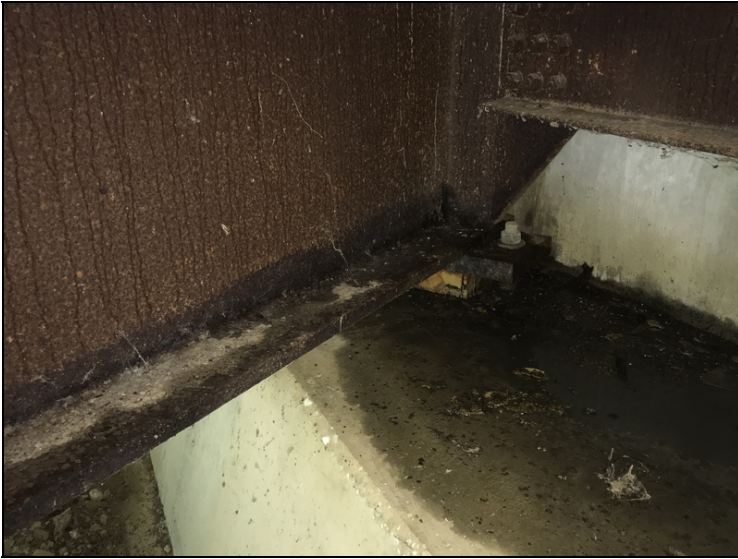
Girder #3 over abutment #1 active corrosion due to leaking compression joint.
