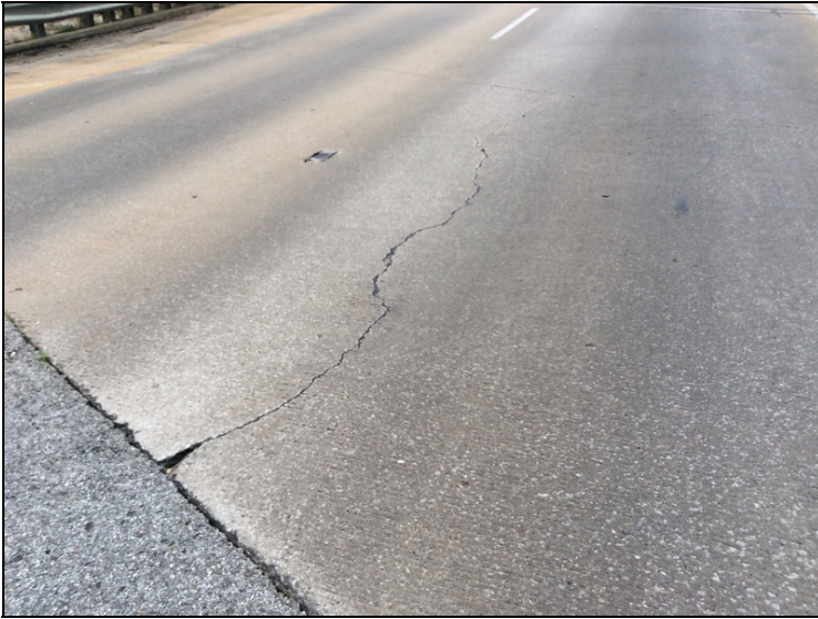
West approach slab-Longitudinal cracking.
