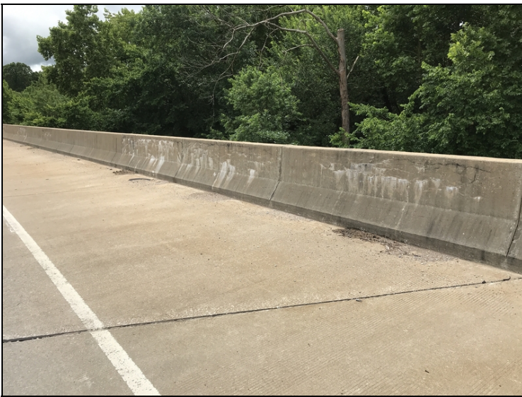
Typical cracking and efflorescence of parapet.
