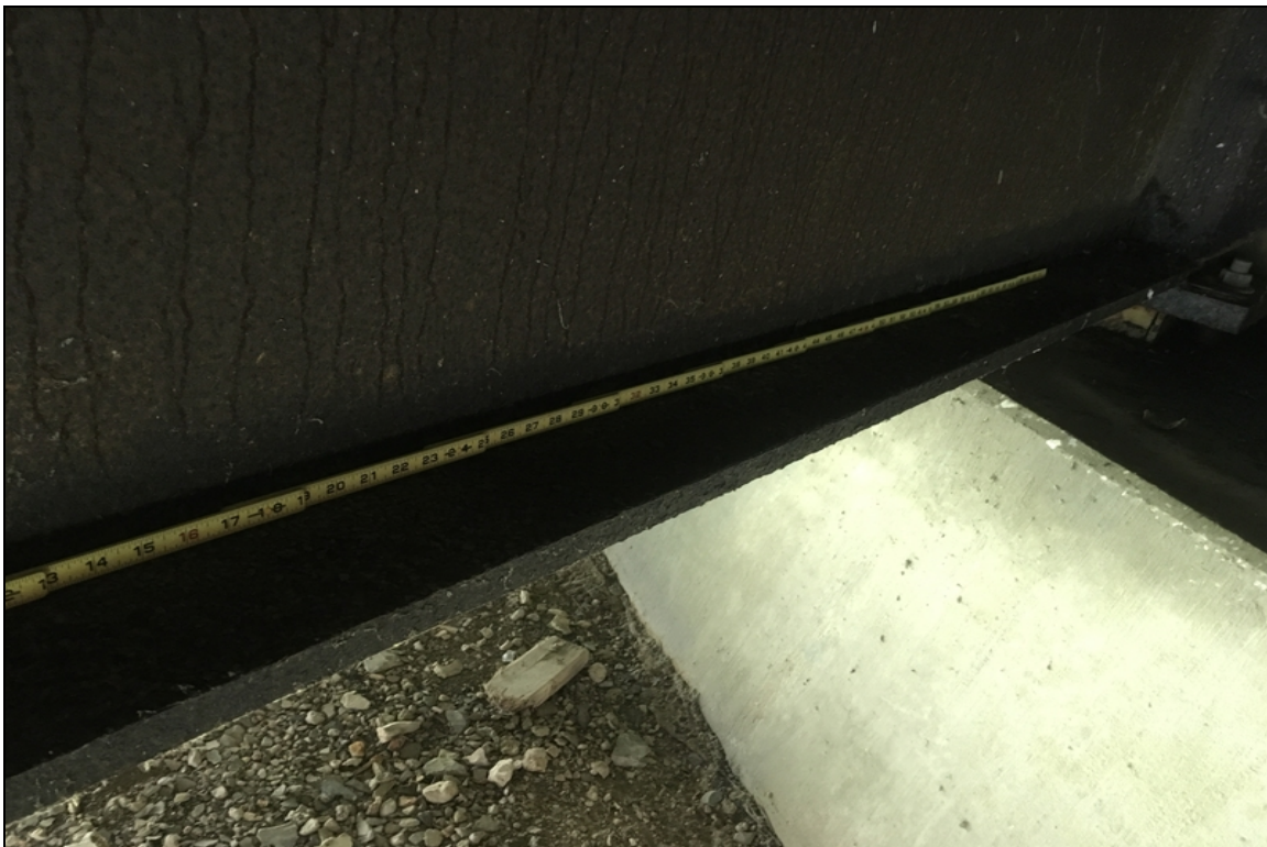
Cs3 corrosion on beam #3 in span #1.
