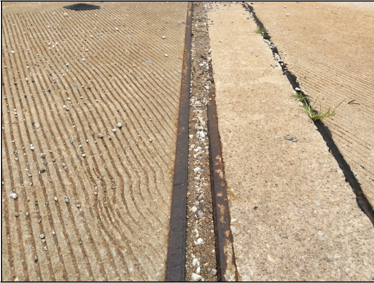
Abutment #1-Debris impact in expansion joint.
