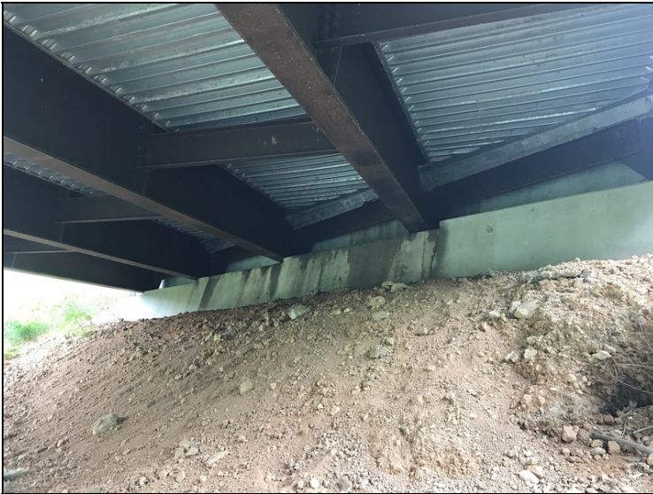
Leakage on bridge seat from leaking compression seal.
