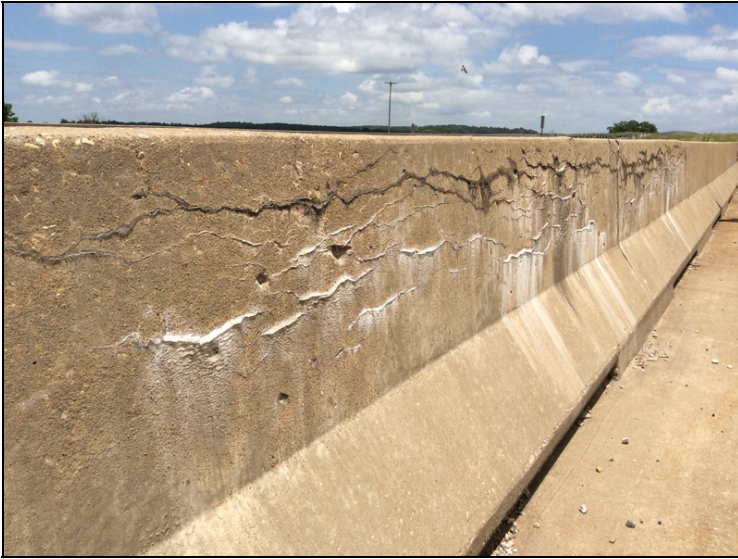
Left parapet-Mapcracking with efflorescence.
