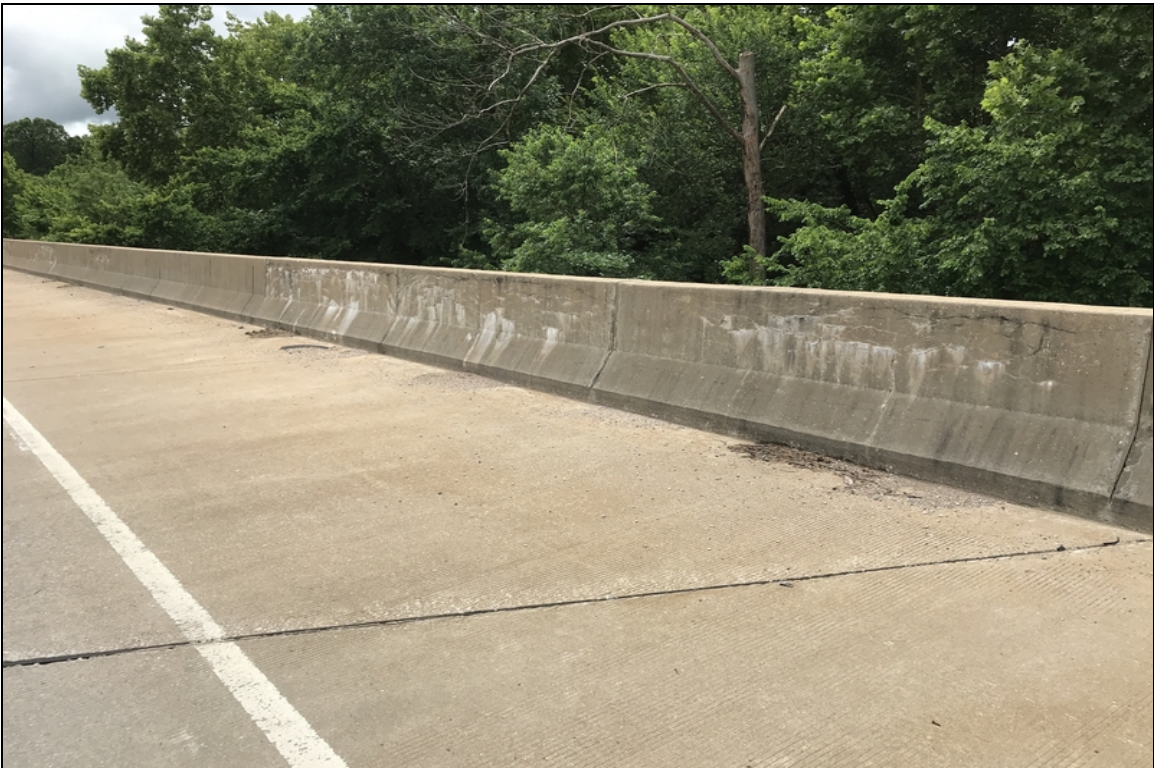
Typical cracking and efflorescence of parapet.
