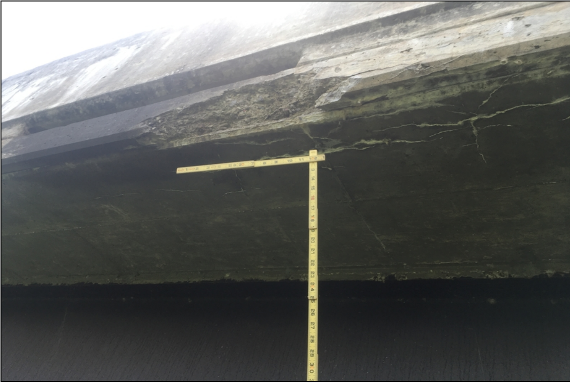
2' of cs3 spalling with no rebar exposed on the left outer overhang of span #1.
