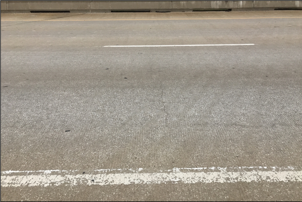
Typical transverse cracking in bridge deck.
