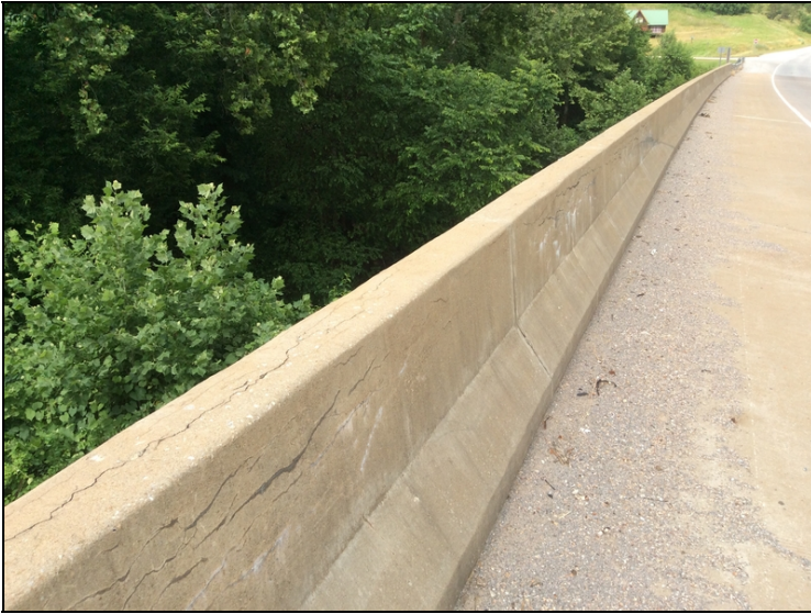
Parapet wall has map cracking with efflorescence
