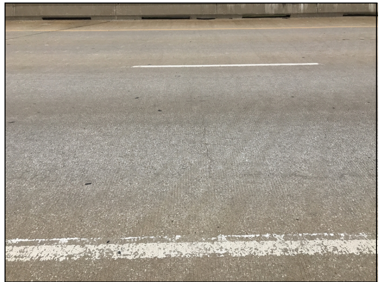
Typical transverse cracking in bridge deck.
