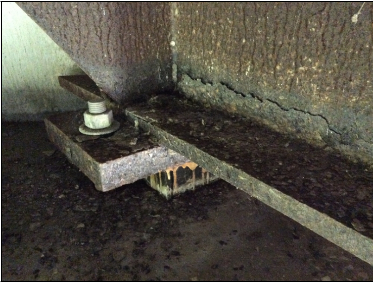
Abutment #1, beam #3-Corrosion to bottom flange and web due to leaking expansion joint seal.
