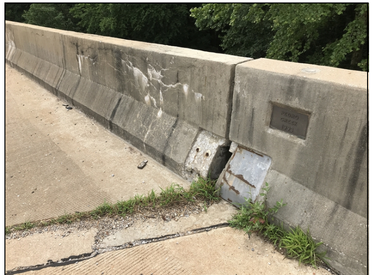
Expansion plate on right parapet missing.
