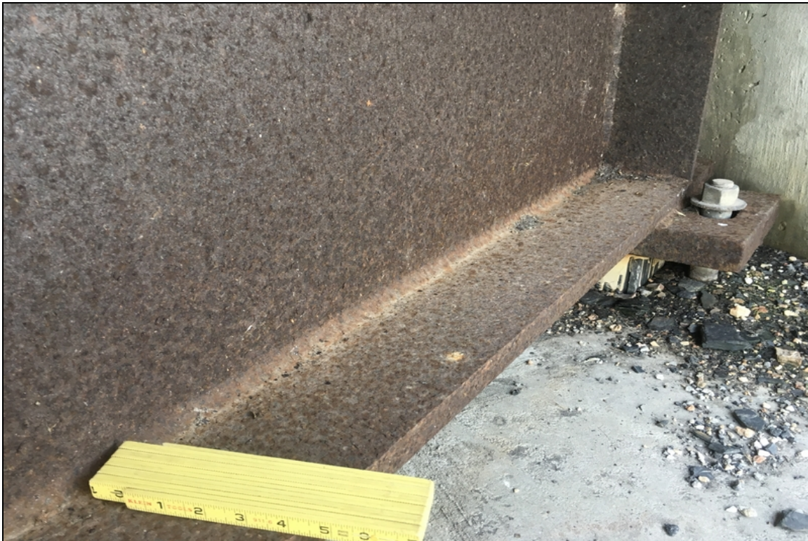
Cs2 corrosion on beam #1 at the beginning of span #1.
