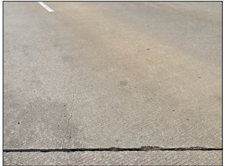
Deck-Typical of diagonal cracking.
