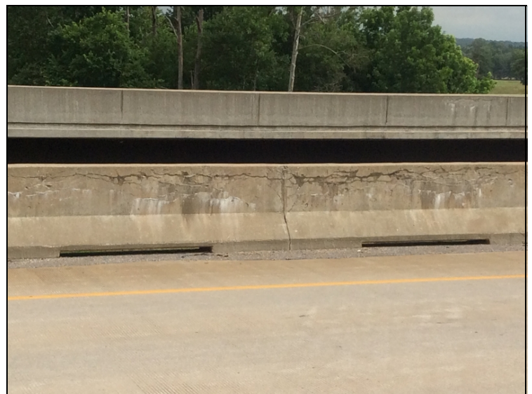
Map cracking in parapet wall
