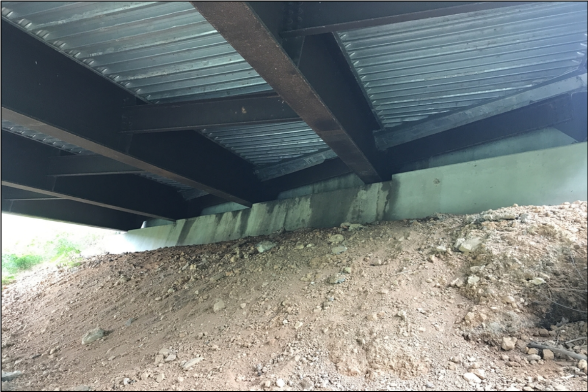
Leakage on bridge seat from leaking compression seal.
