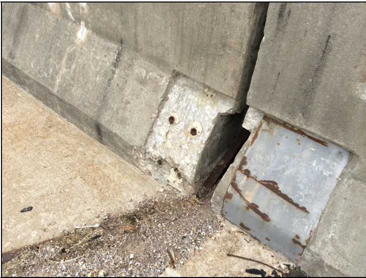
Abutment #1, right side-Missing sliding plate on parapet.
