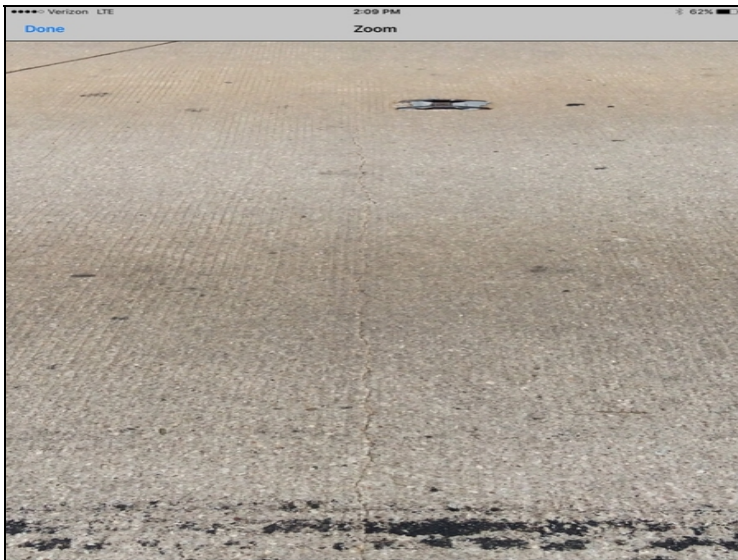
Transverse deck cracking.
