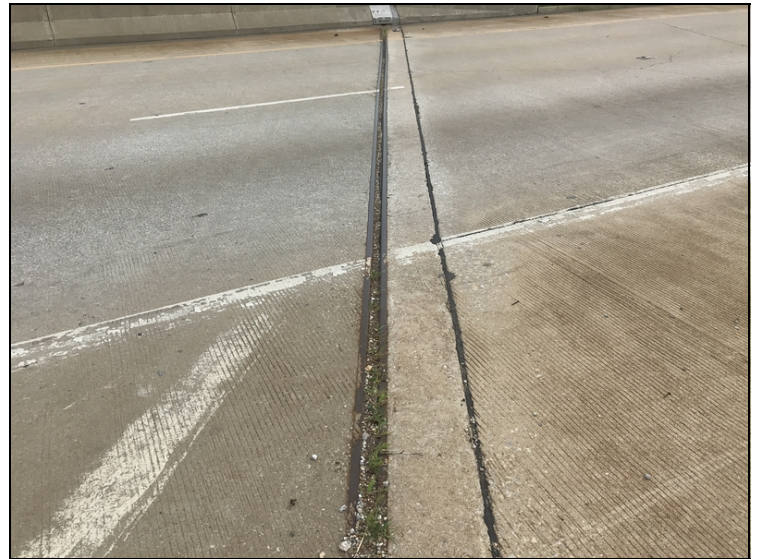
General view of abutment #2 compression joint debris impact.
