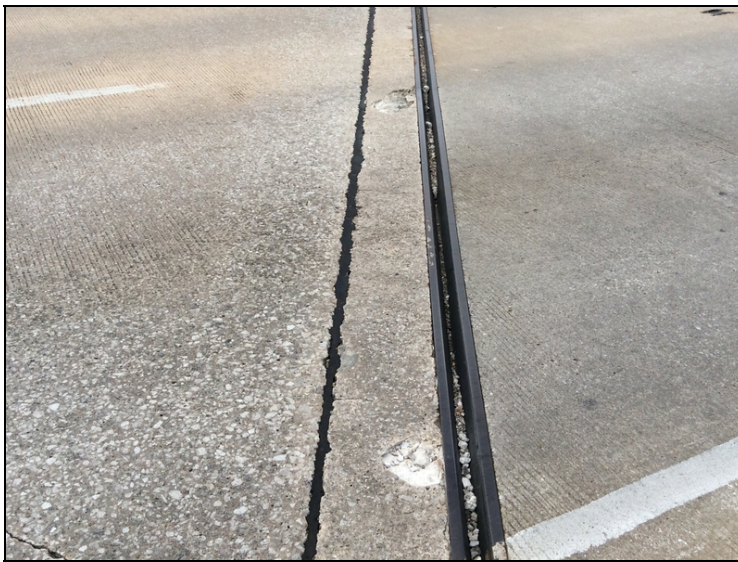
Spalling in top of East abutment backwall.
