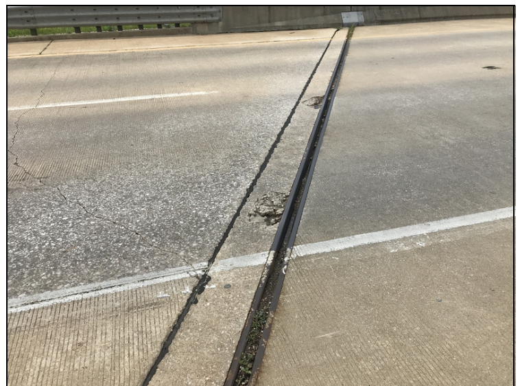
Abutment #2 spalling
