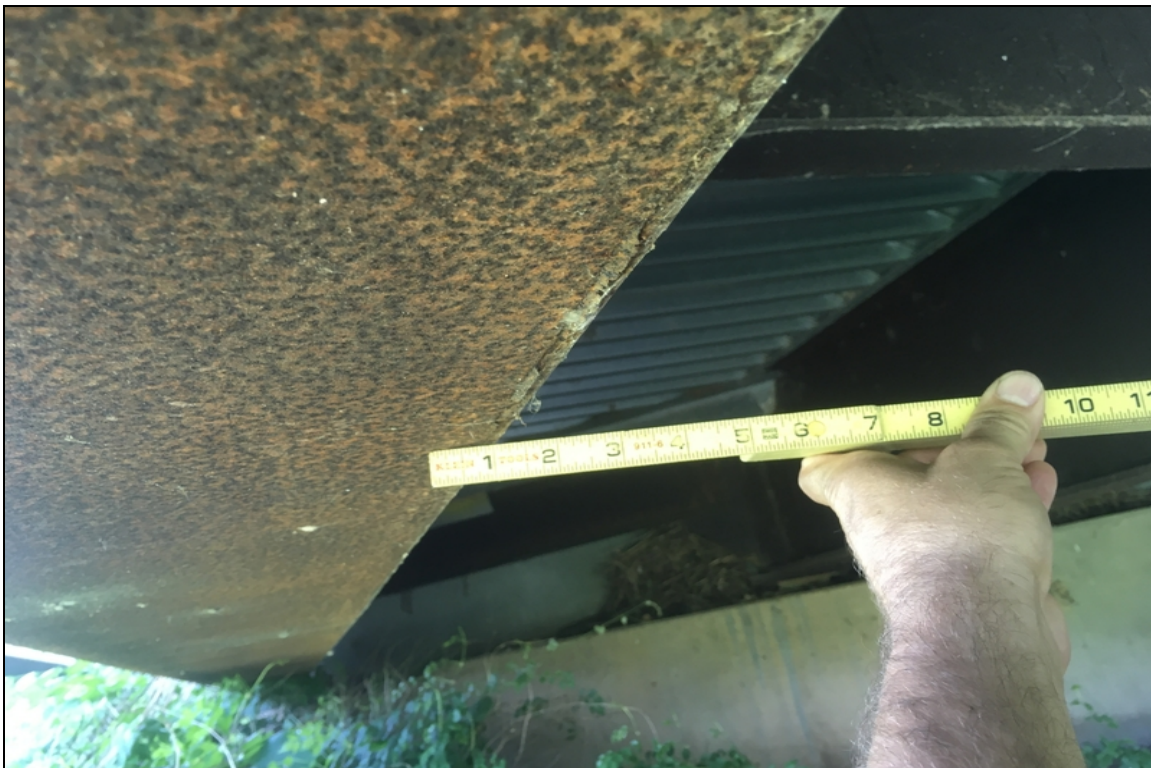
Factory defects on the bottom flange of beam #1 in span #3.
