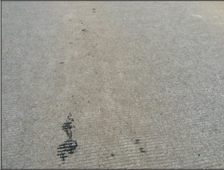
Sealable longitudinal deck cracks located in the driving surface.
