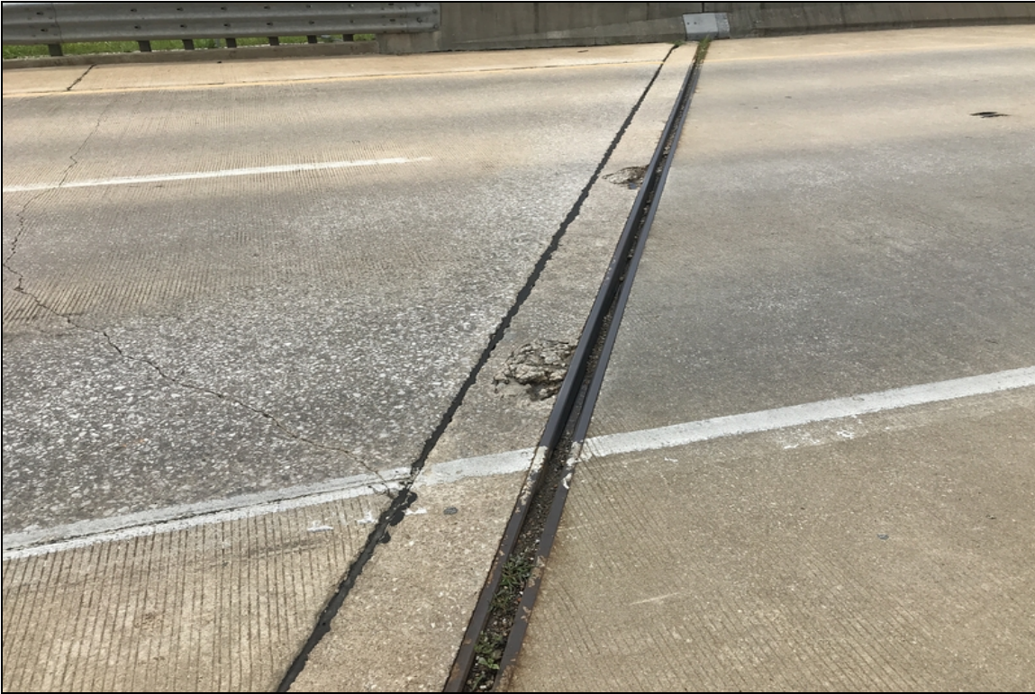
Abutment #2 spalling
