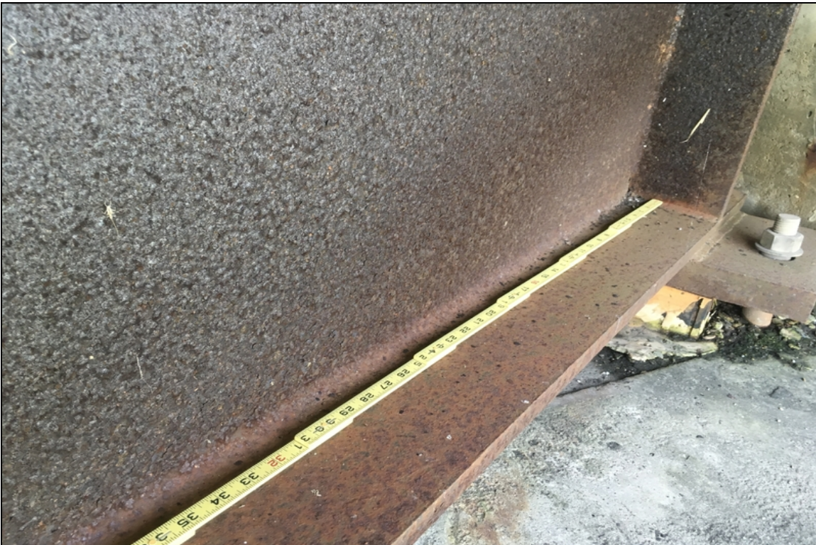
4' of cs2 corrosion on the exterior web of beam #1 in span #1.
