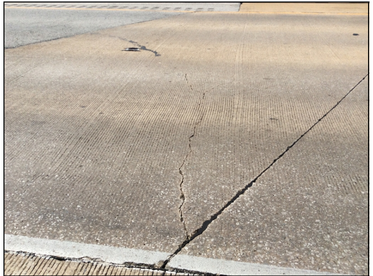
East approach slab-Cracking.
