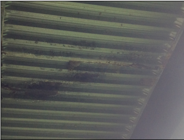
Span #1 bay #5 active corrosion to SIP forms.
