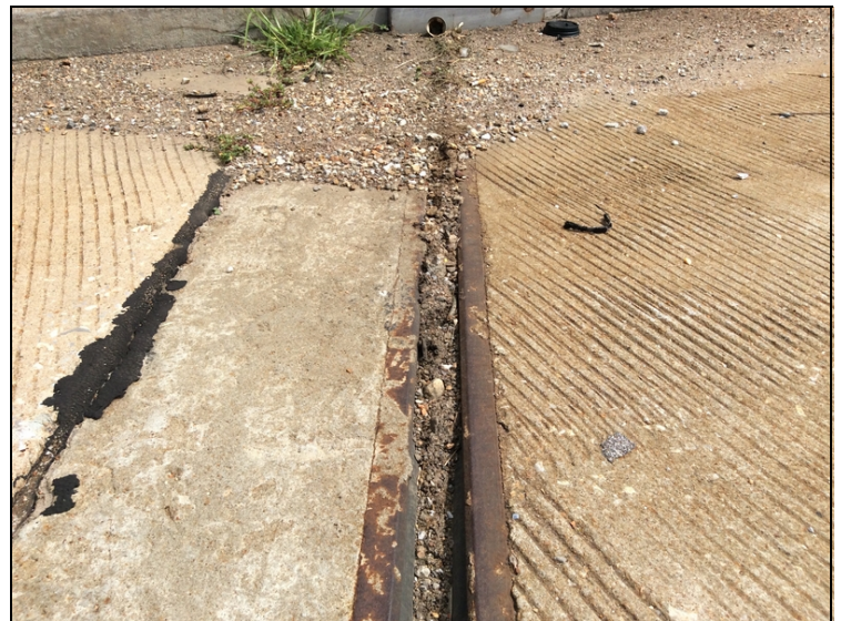
Abutment #1-Debris impaction in expansion joint.
