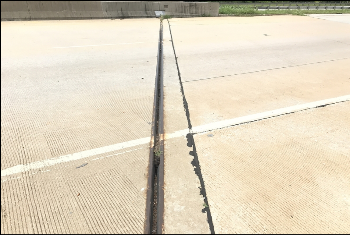
View of abutment #1 compression joint.
