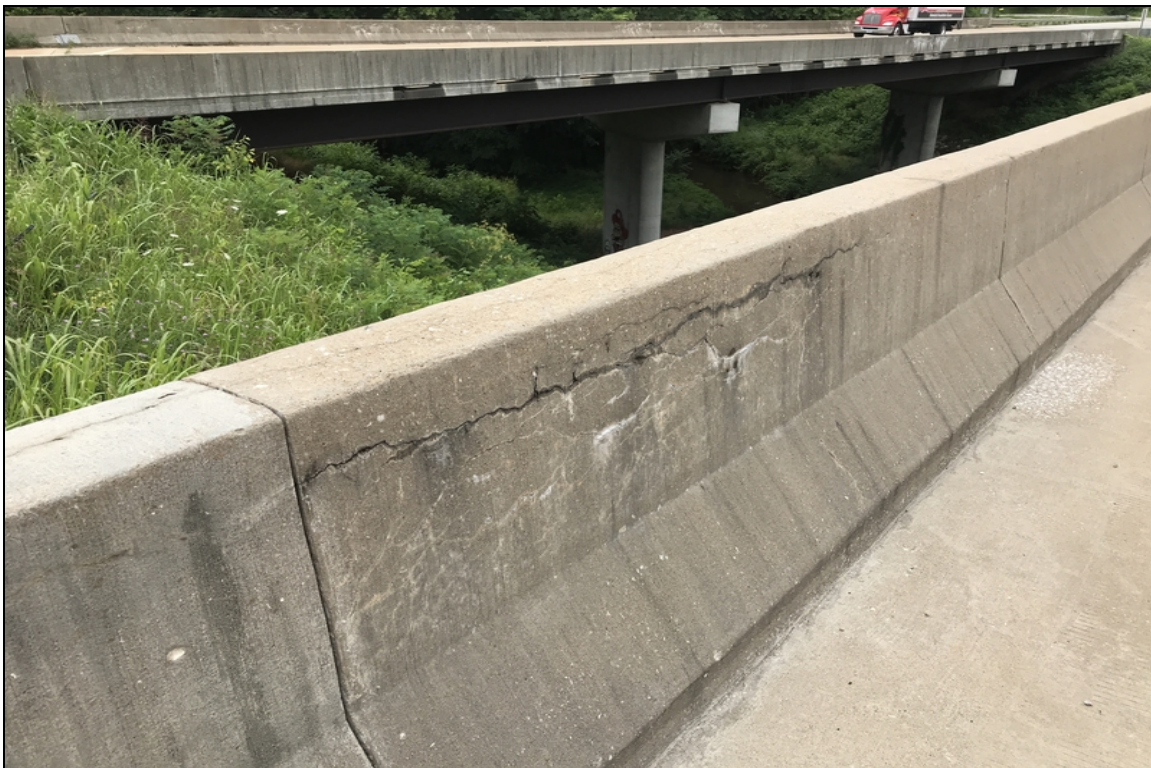
Railing right cracking with efflorescence.
