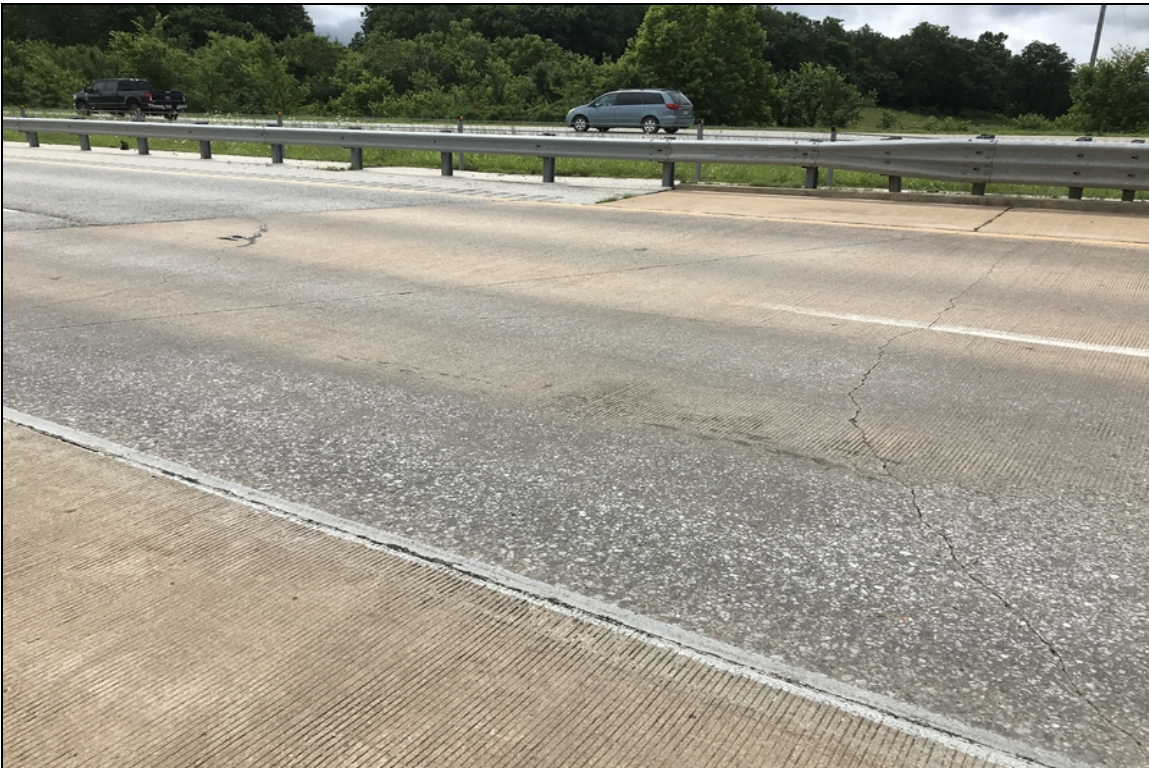
East approach slab cracking.
