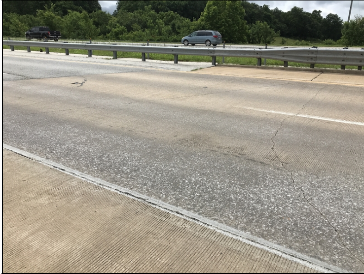
East approach slab cracking.
