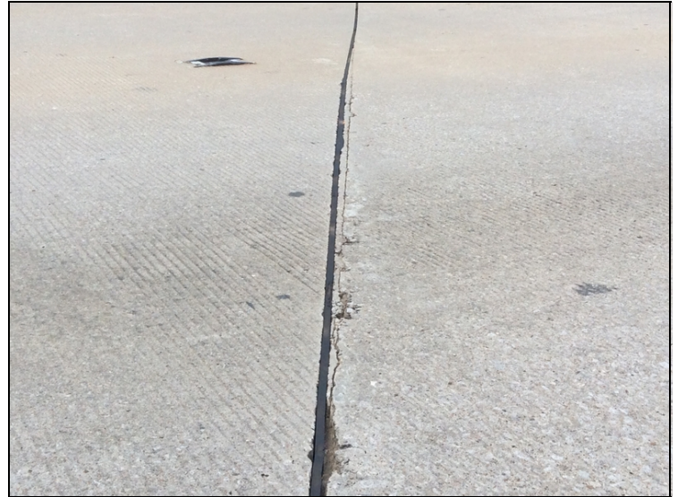
Cracking along sawn joints
