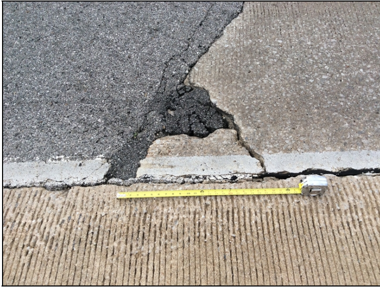
East approach slab-Spalling.
