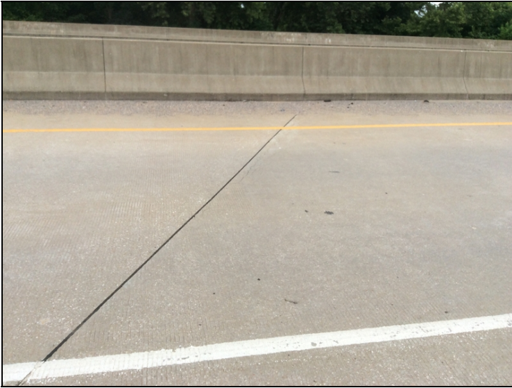
Span #1 right transverse crack adjacent to saw joint
