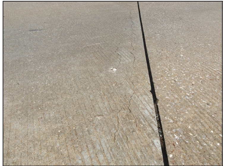
Cracking along sawn joints
