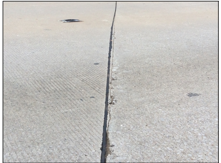
Cracking along sawn joints.
