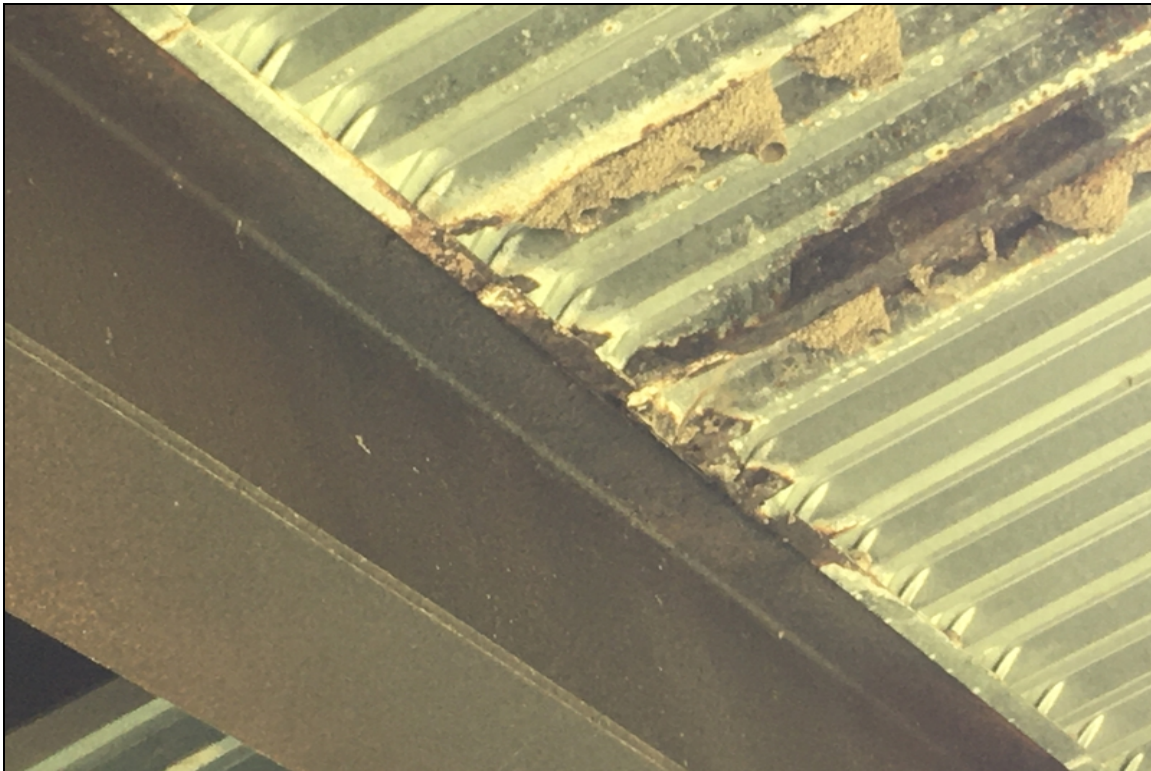
Typical view of cs3 corrosion beneath the construction joints.
