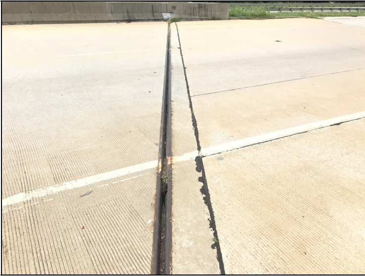
View of abutment #1 compression joint.
