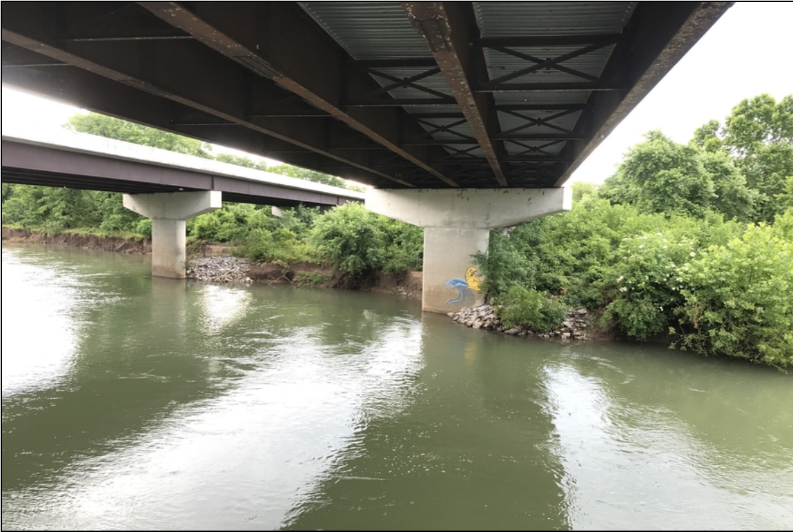
Localized scour at #2 bent of A and B bridge.
