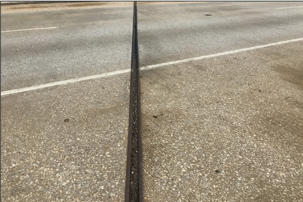
Bent #4 expansion joint debris impaction.
