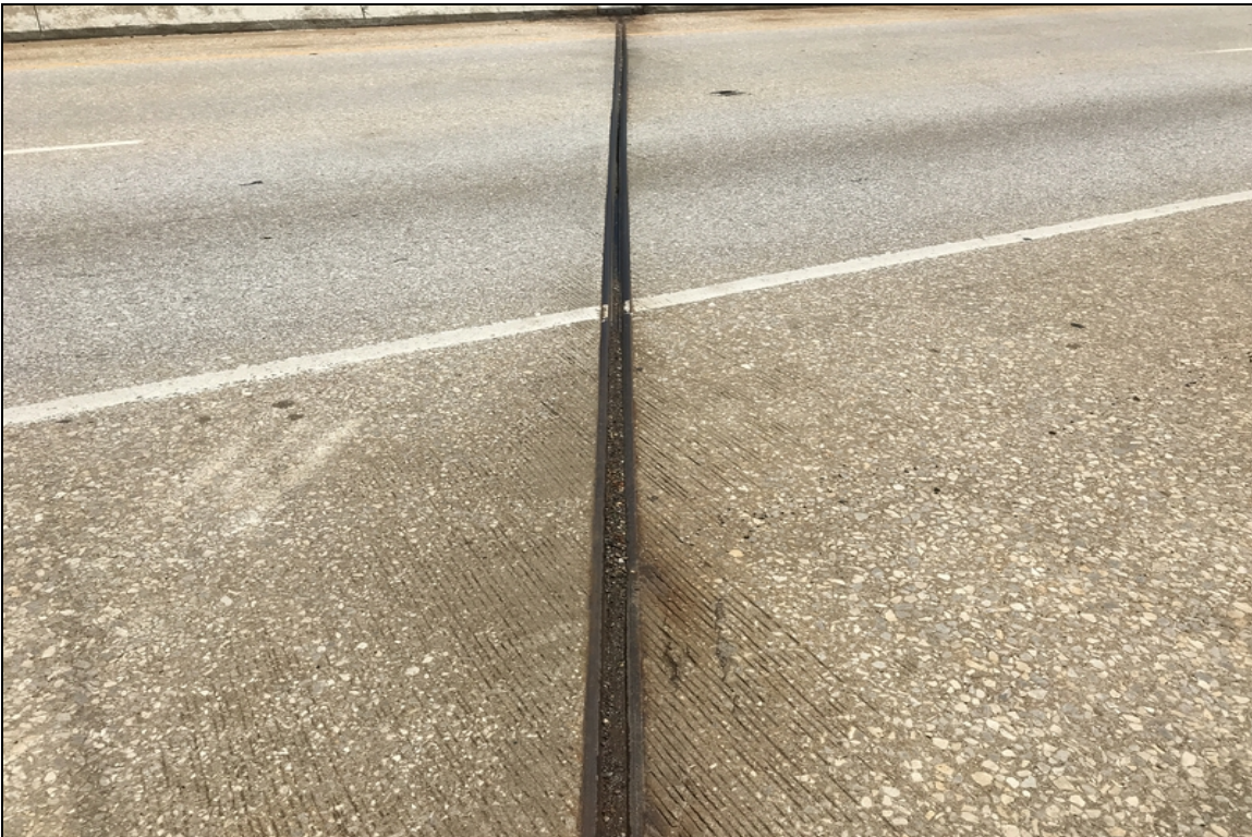
Expansion joint at bent #16 debris impaction.
