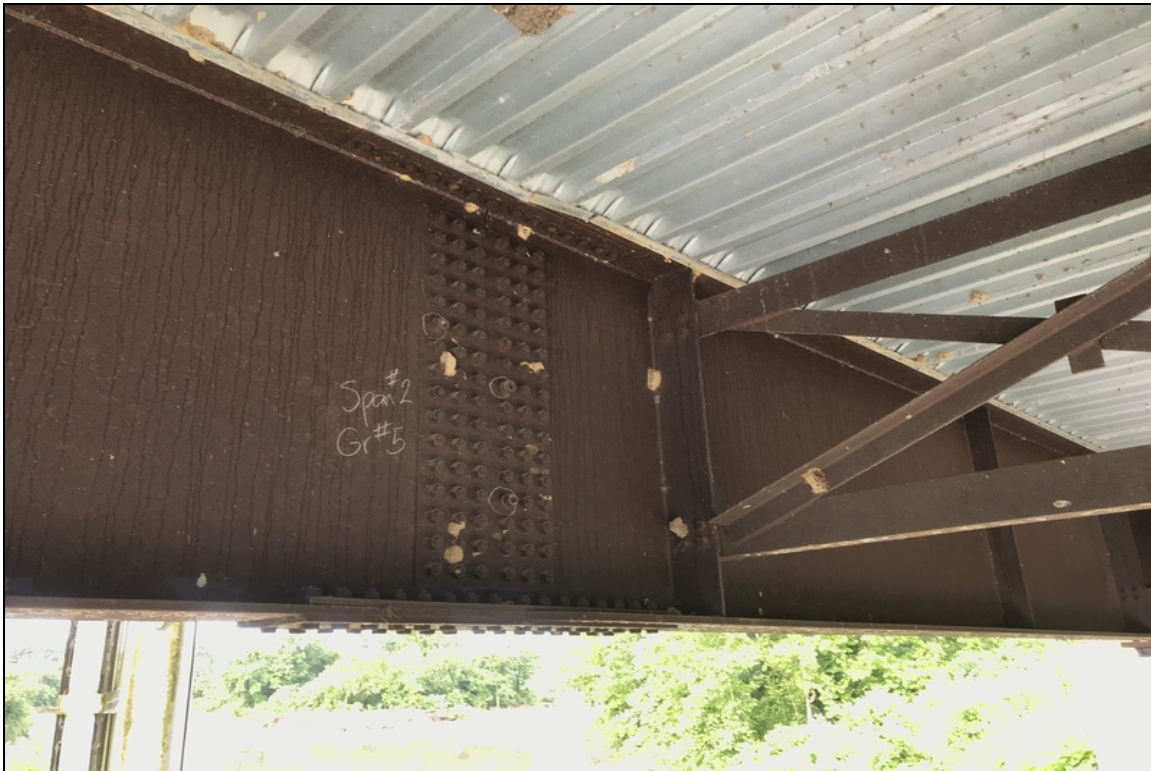
Typical Loose bolts still present from last inspection.
