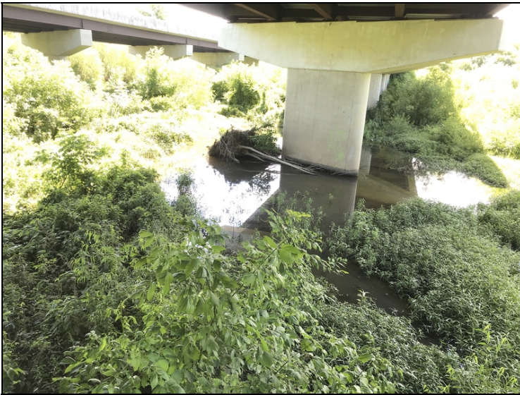
Drift accumulation adjacent to bent #14.
