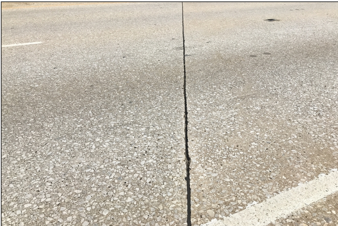
Typical View of pourable joint material displaced from construction joints.
