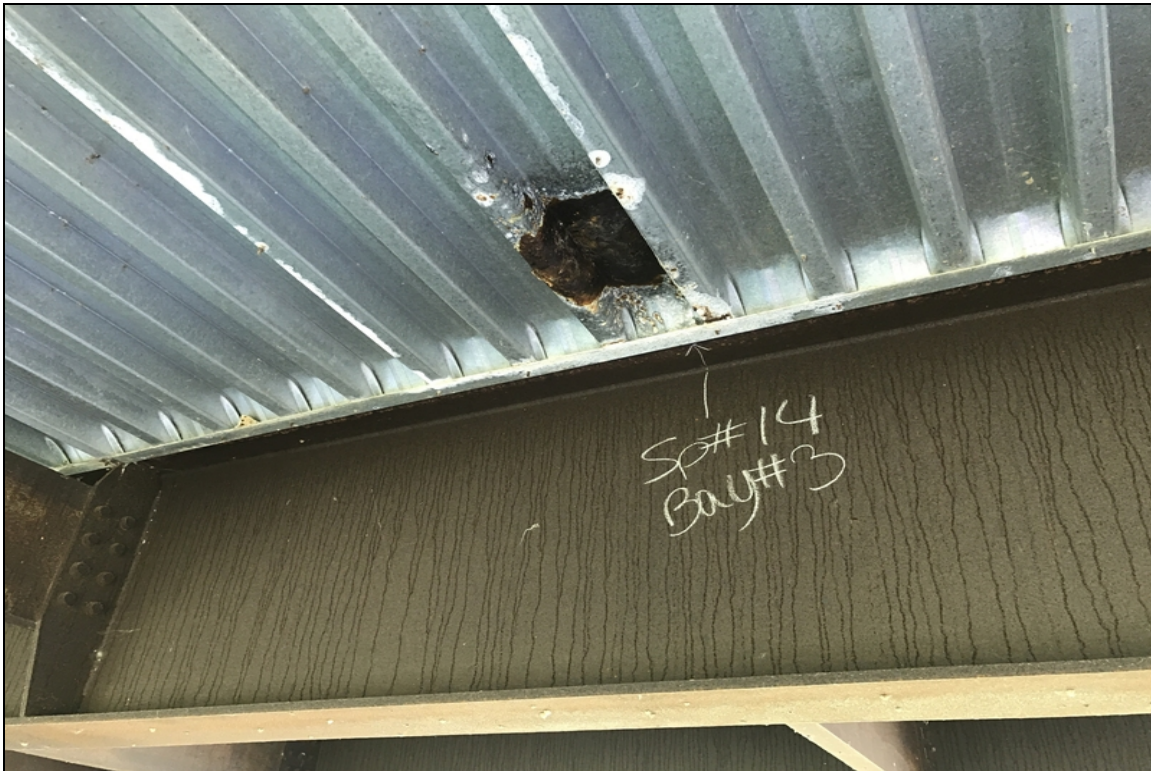
Span #14 bay #3 adjacent girder #4 active corrosion to SIP forms.
