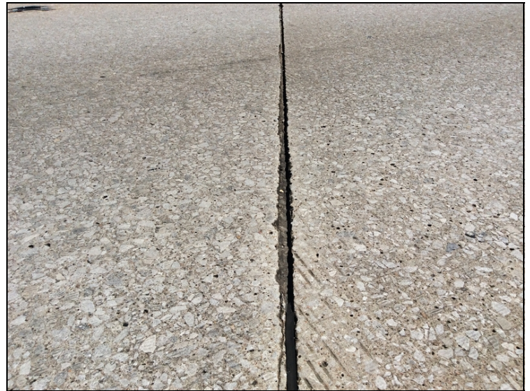
Sawn construction joint sealant missing.
