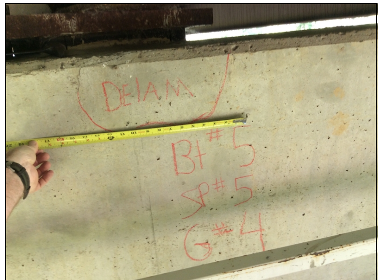
Span #5, bent #5-Delaminated area under Girder #4.
