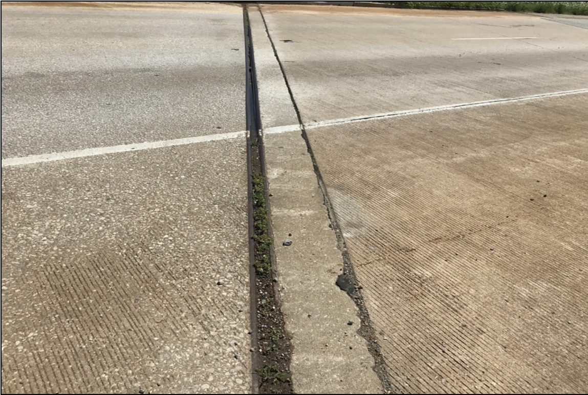
General view of abutment #2 expansion joint material debris impaction
