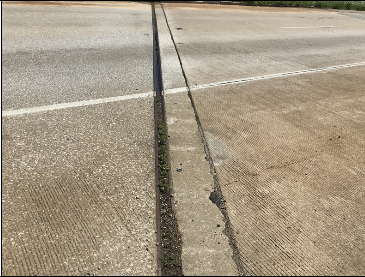
General view of abutment #2 expansion joint material debris impaction
