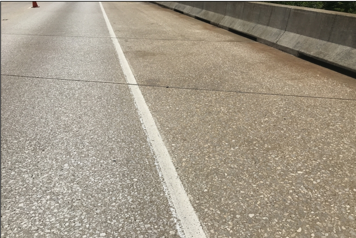
Entire deck surface appears to have been milled down.
