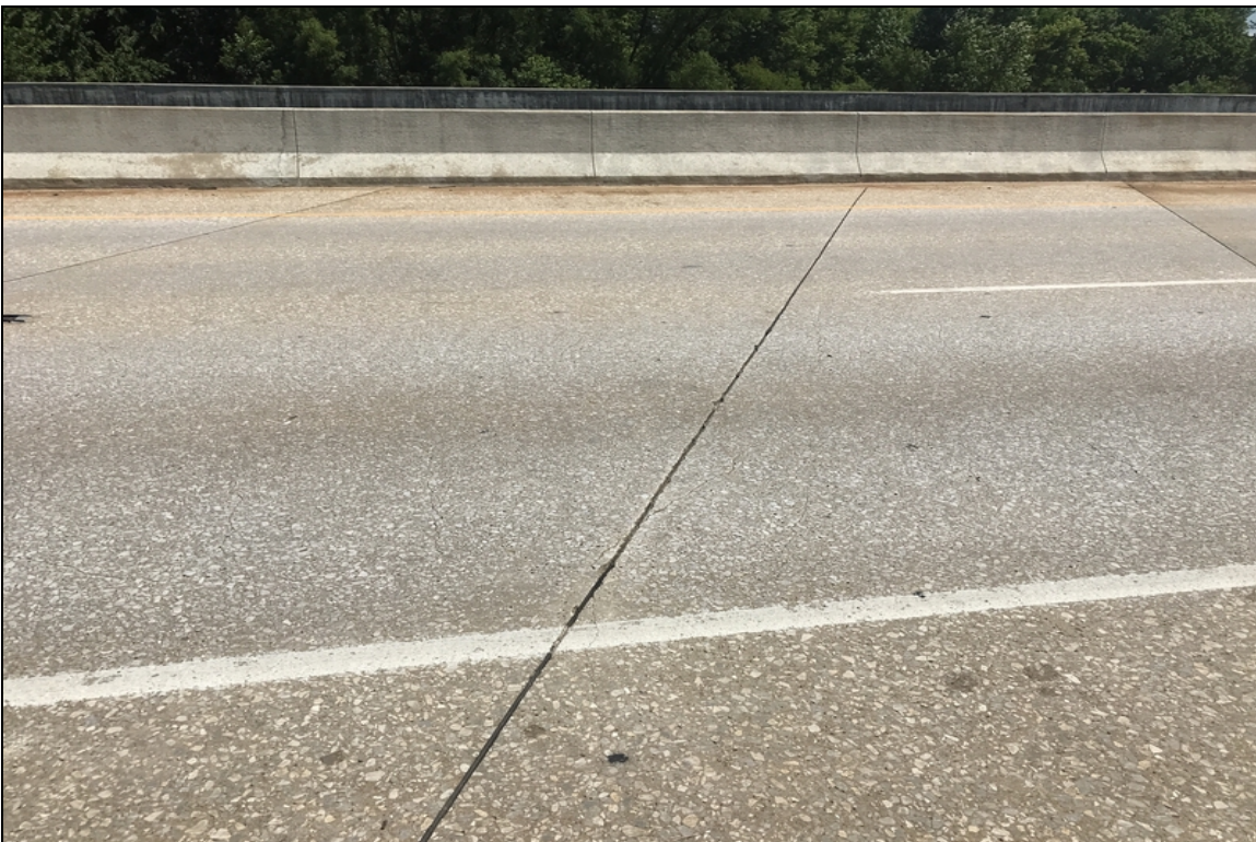
Area of map cracking over bent 11
