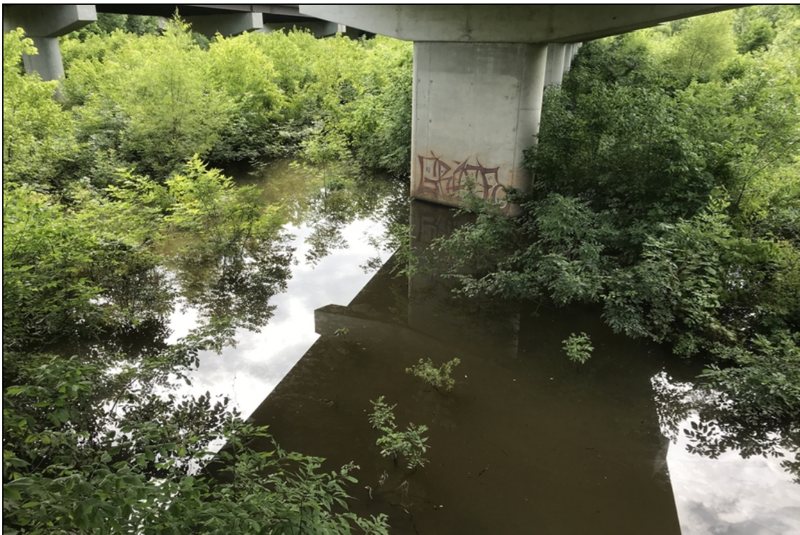
Majority of channel under structure has approximately 2' of trapped flood water.
