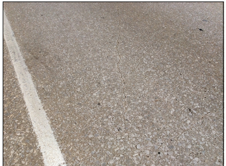
Span #11, outside lane-Wide cracking.
