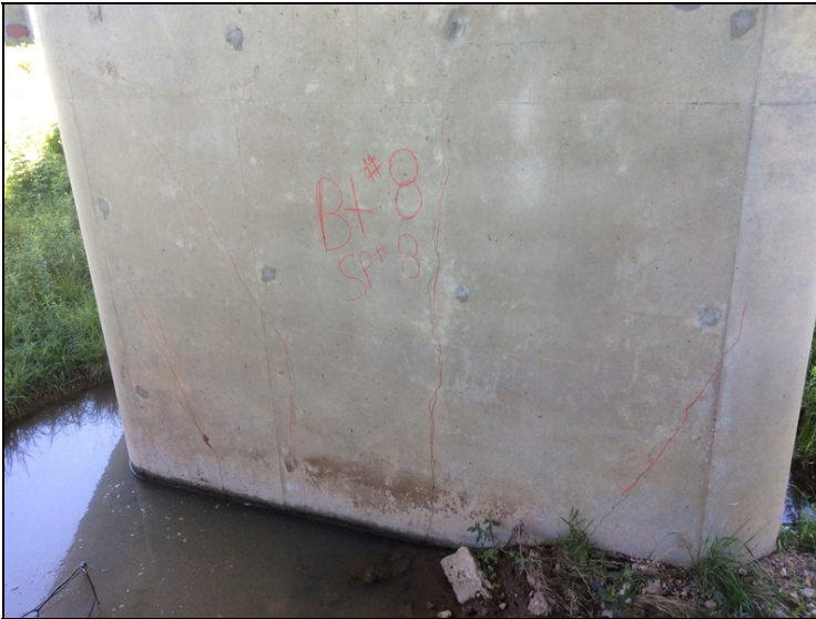
Bent #8-Wide cracking in column. Photo #2.
