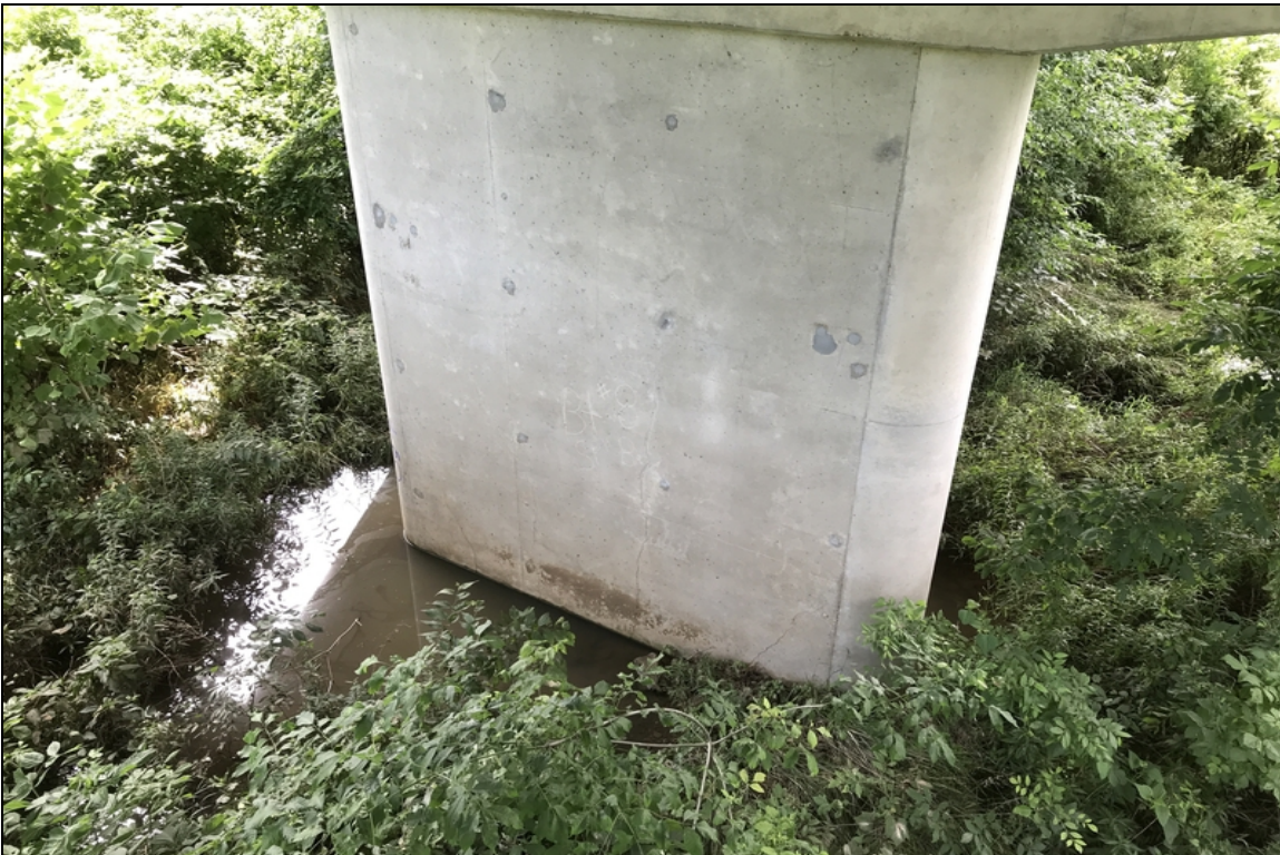
Bent #8 pier vertical and diagonal cracking are still present.
