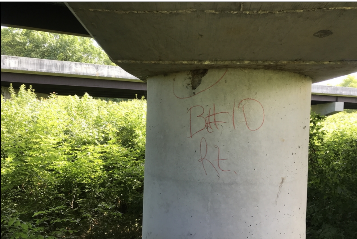
Bent #10 right side of pier baseball sized spall.
