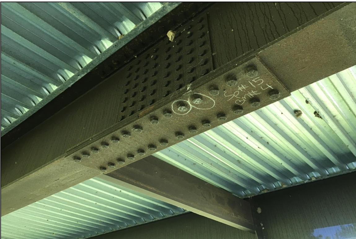
Span #15 Girder #4 has two loose bolts.
