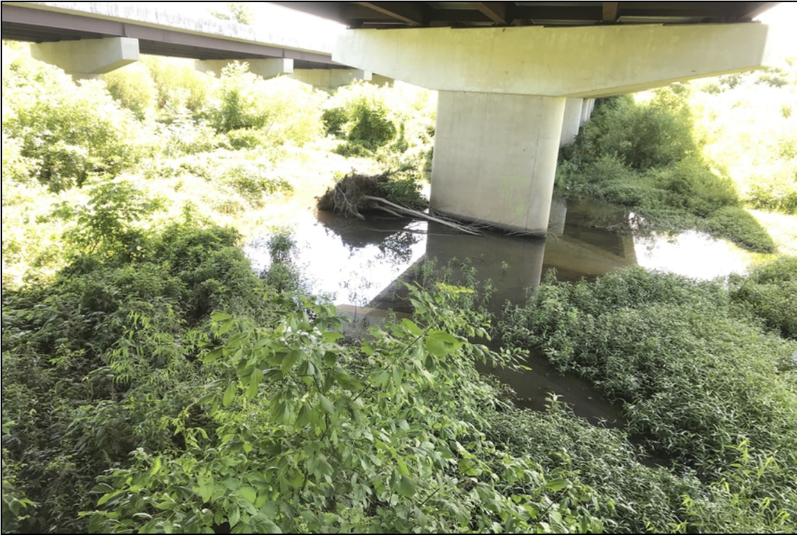
Drift accumulation adjacent to bent #14.
