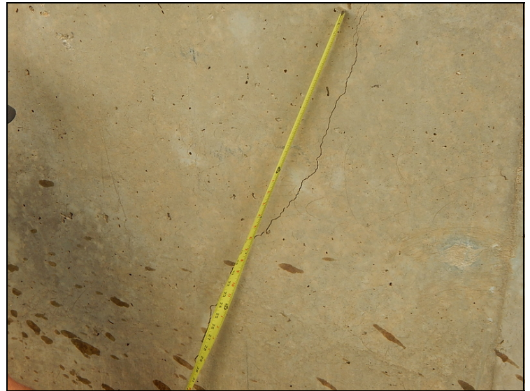
Vertical crack at bent #9 column
