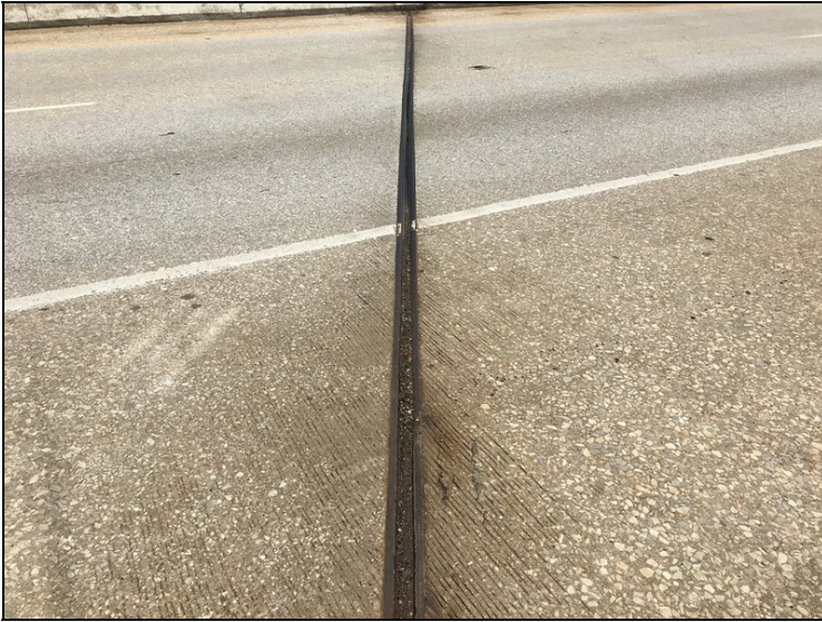
Expansion joint at bent #16 debris impaction.
