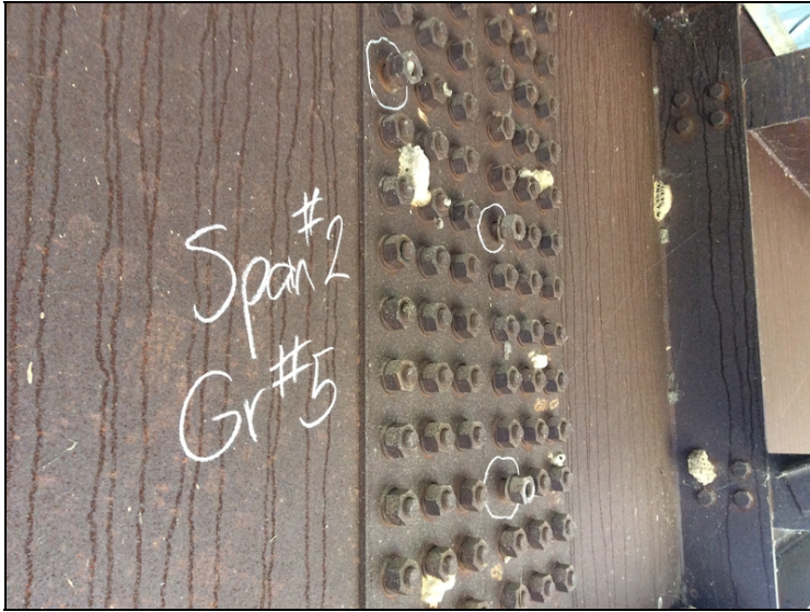
Span #2, girder #5 splice #1 has 3 loose bolts.
