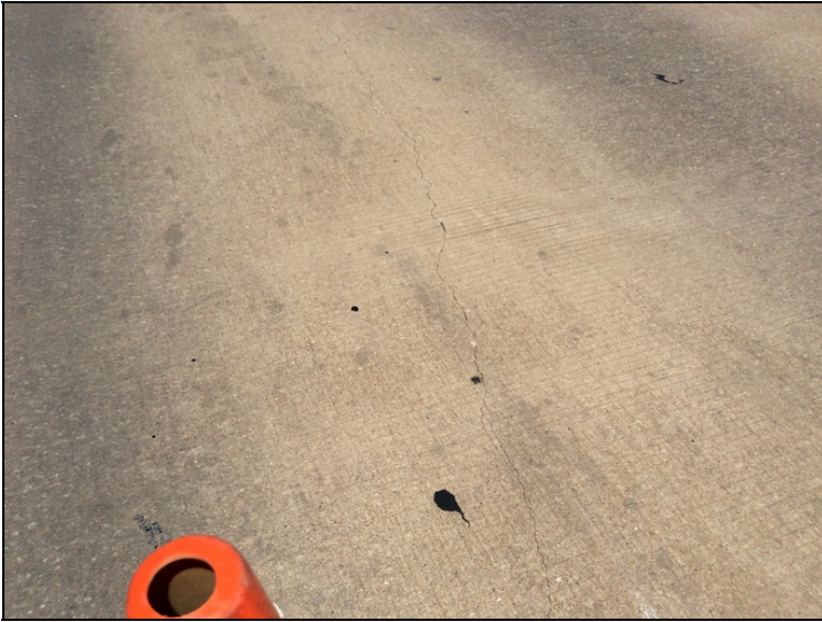
West approach slab-longitudinal cracking.
