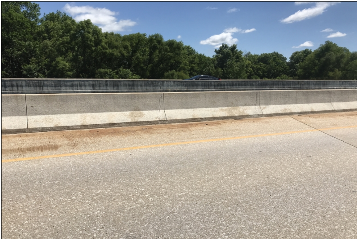
Typical cracking in parapet wall.
