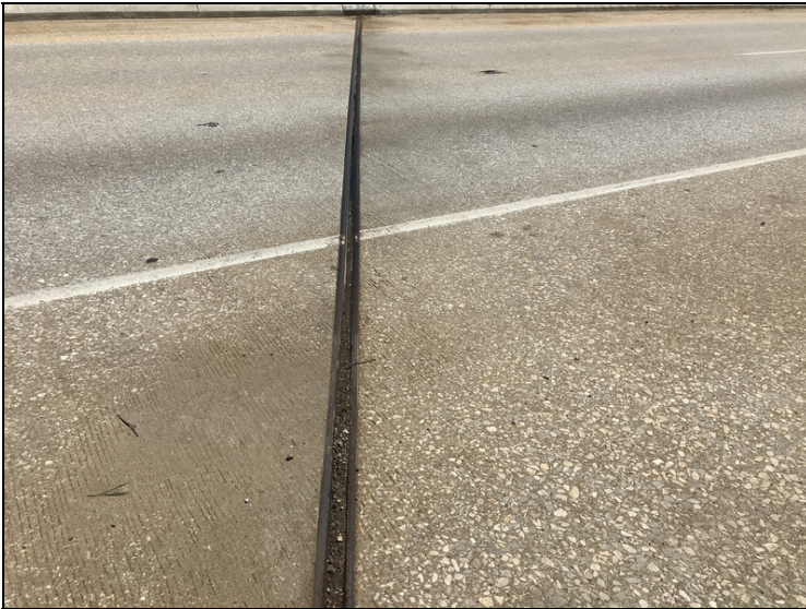
Bent #8 expansion joint.
