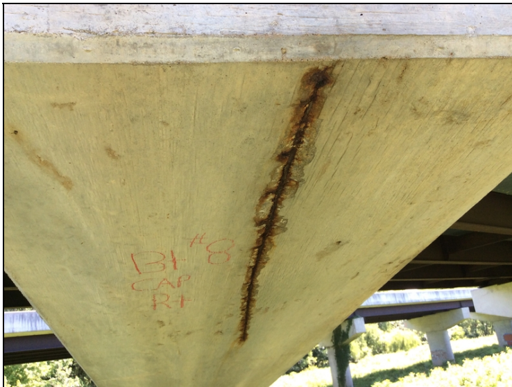
Bent #8 cap-Shallow spalling with exposed reinforcing steel in undersurface.
