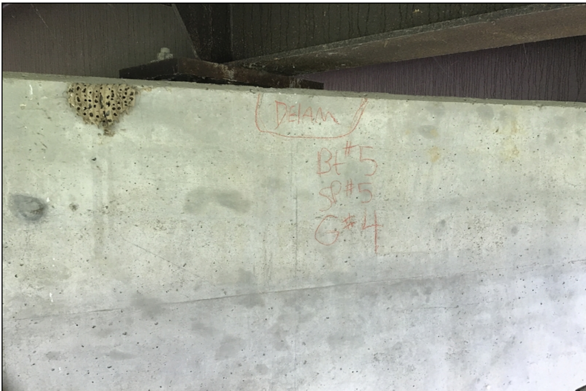
Delaminations at Bent #5 are still present from last inspection.
