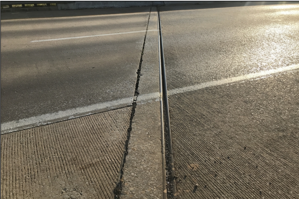
View of abutment #1 expansion joint
