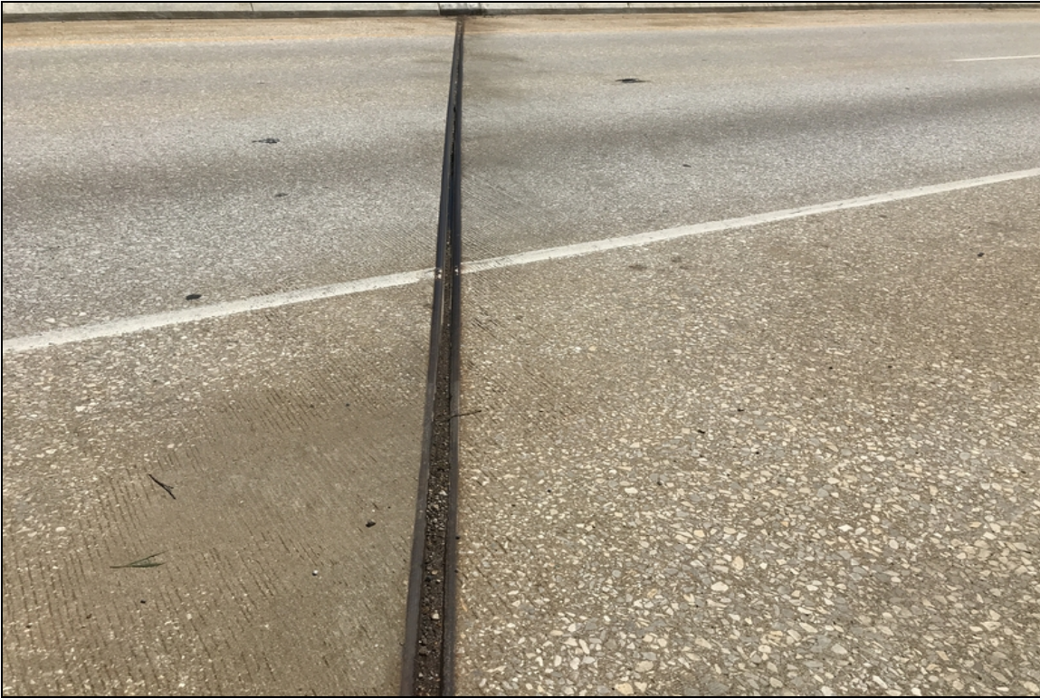
Bent #8 expansion joint.
