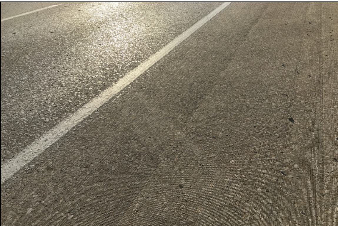
Mill work on deck surface and traffic abrasion has removed the Tyne wearing surface.
