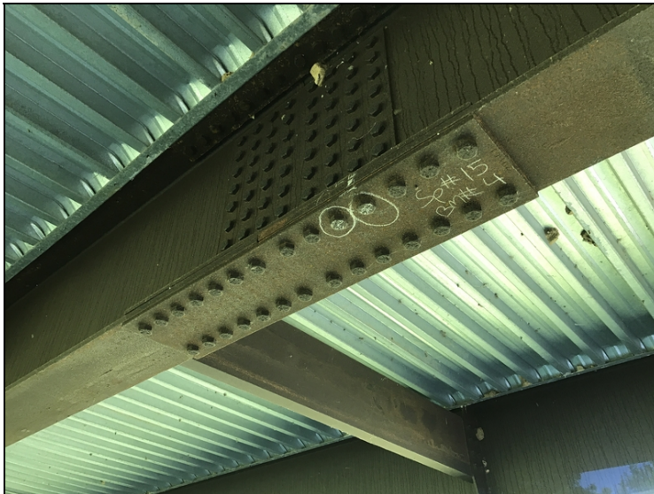
Span #15 Girder #4 has two loose bolts.
