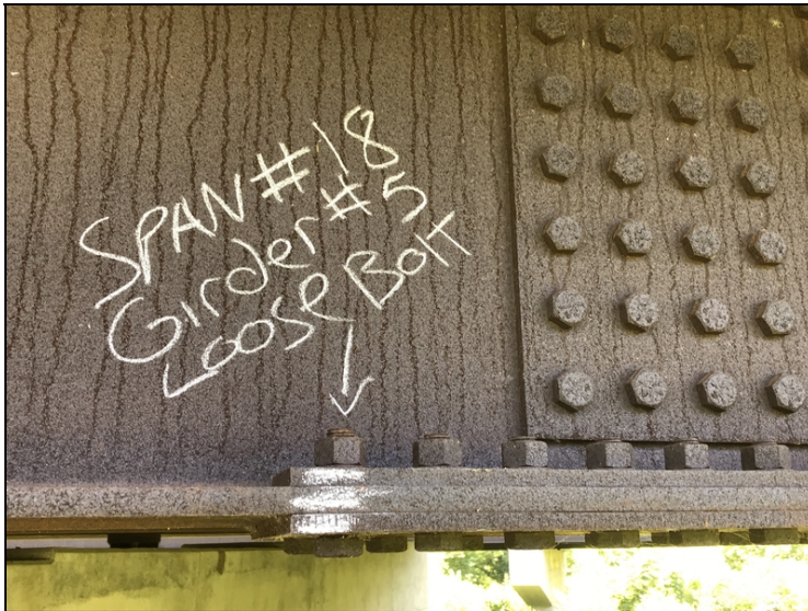
Span #18 Girder #5 has one loose bolt.
