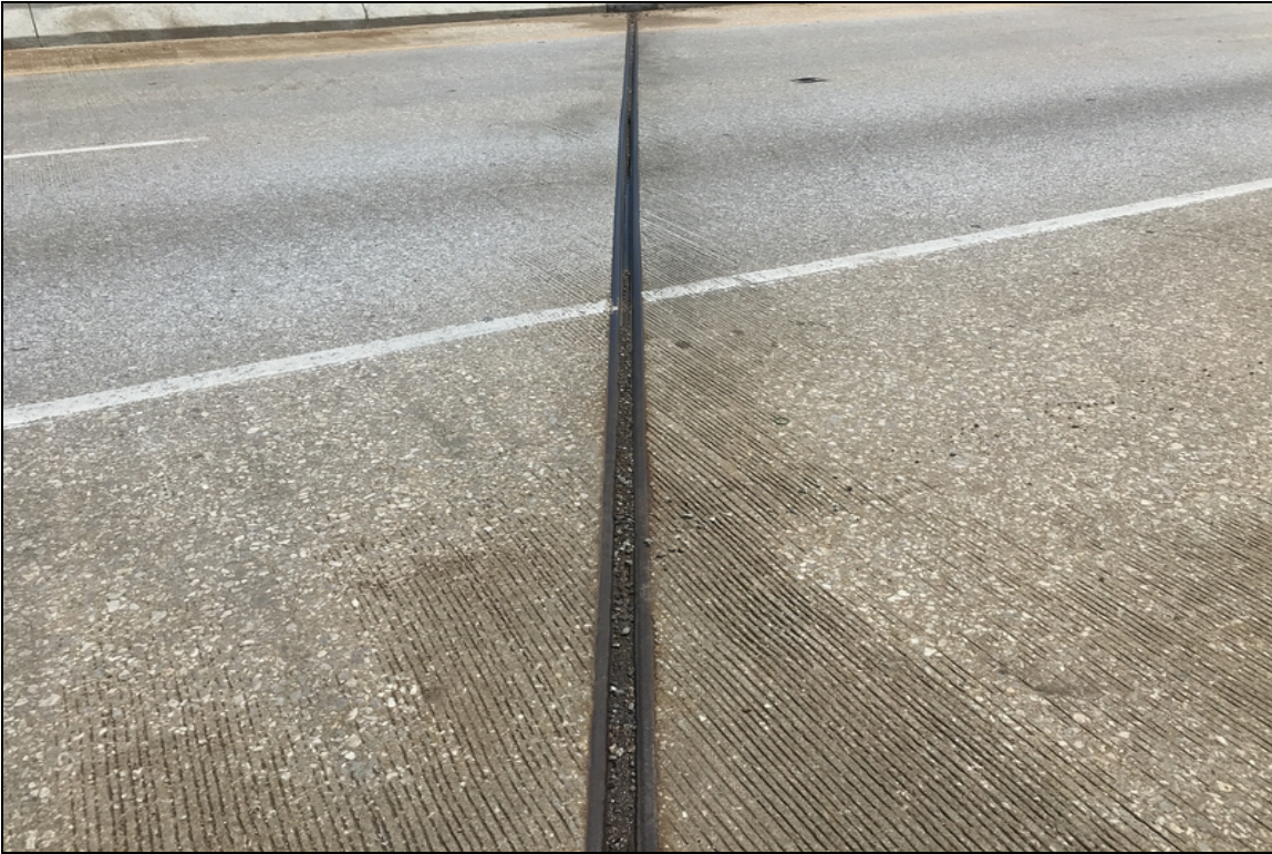
Bent #12 expansion joint debris impaction
