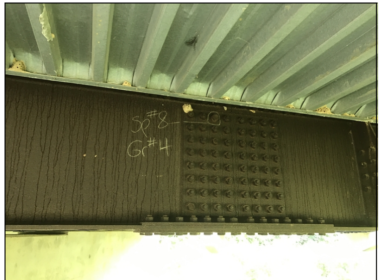
Loose bolts still present from last inspection.
