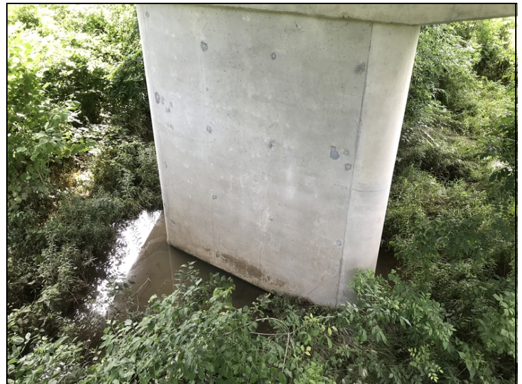
Bent #8 pier vertical and diagonal cracking are still present.
