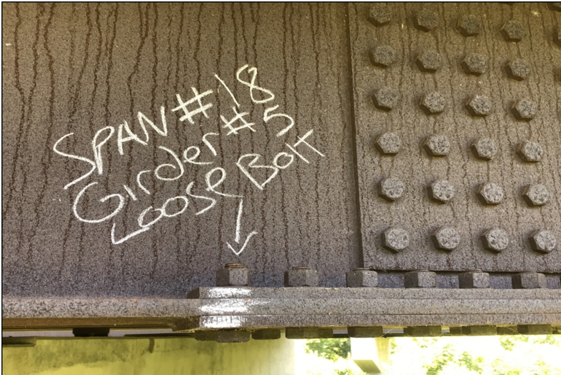
Span #18 Girder #5 has one loose bolt.
