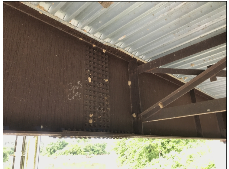
Typical Loose bolts still present from last inspection.
