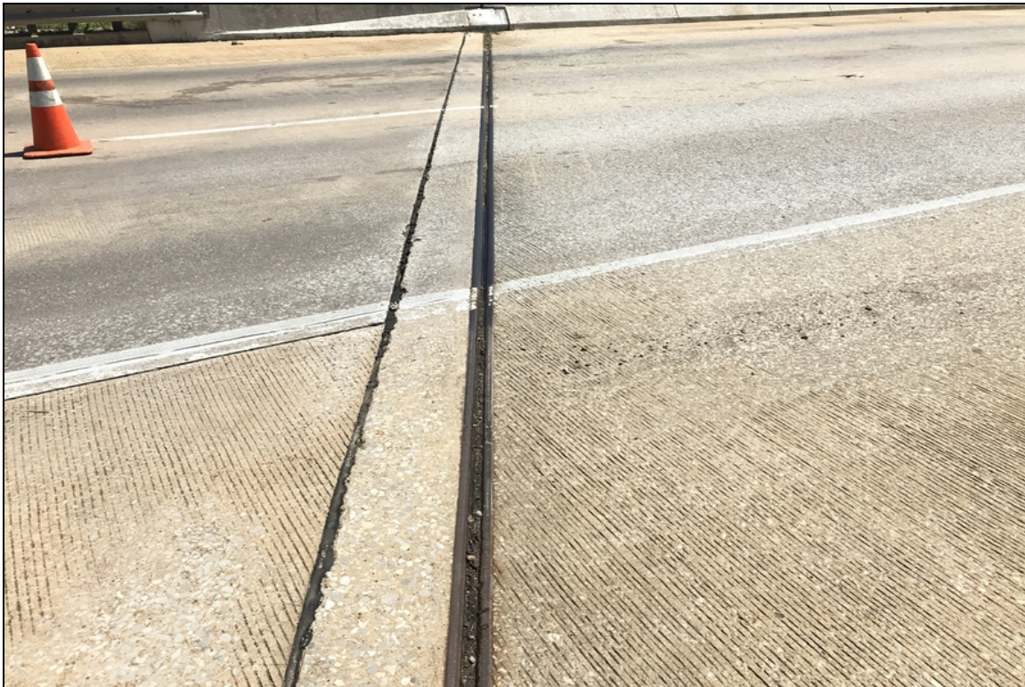
Abutment #1 expansion joint debris impaction.
