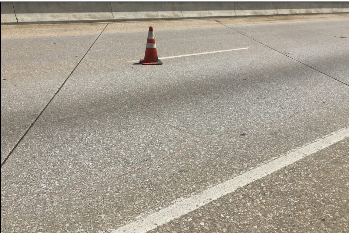
Typical transverse and longitudinal cracking of the deck.
