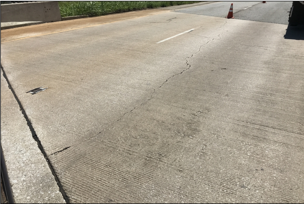
East approach slab cracking.
