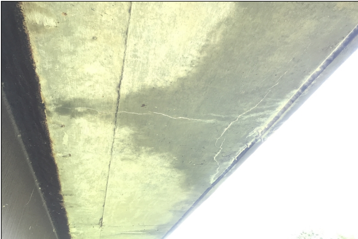
Span #10 right overhang approximately 7' ahead of bent #9 efflorescence with cracking.
