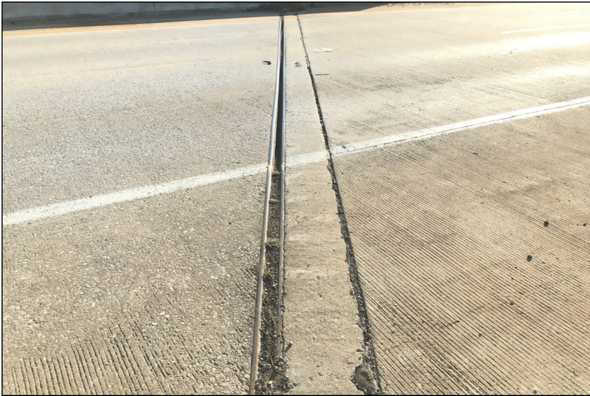
View of expansion joint at abutment #2.
