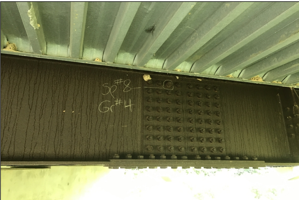
Loose bolts still present from last inspection.
