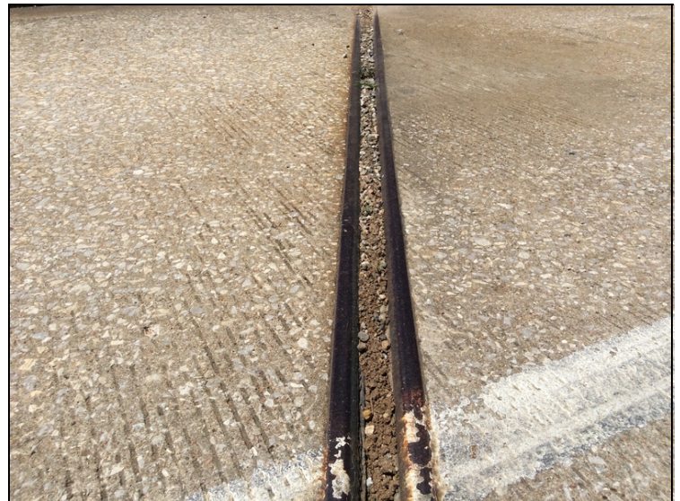
Strip seal expansion joint-Dirt and debris compaction.
