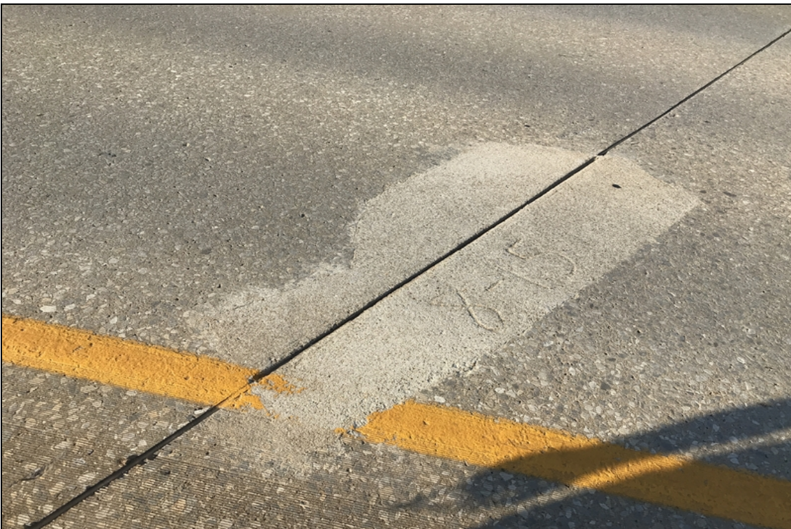
Deck surface concrete patch span #13 on the adjacent bent #13.
