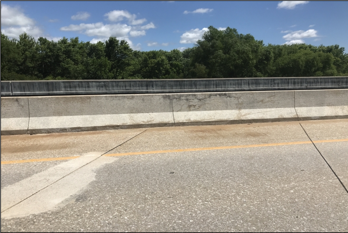
Cracking with efflorescence in parapet wall typical.
