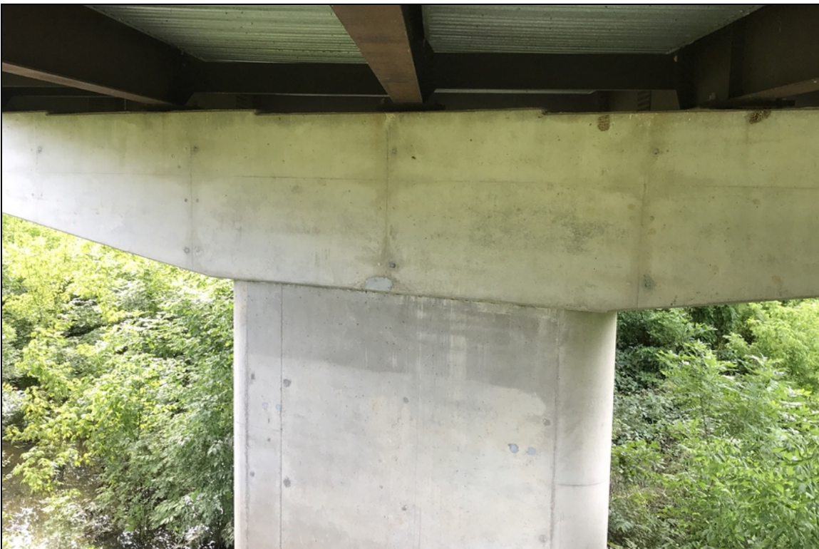
Bent #6 cap behind side has a 1&rsquo; wide patch at the bottom of cap near centerline.
