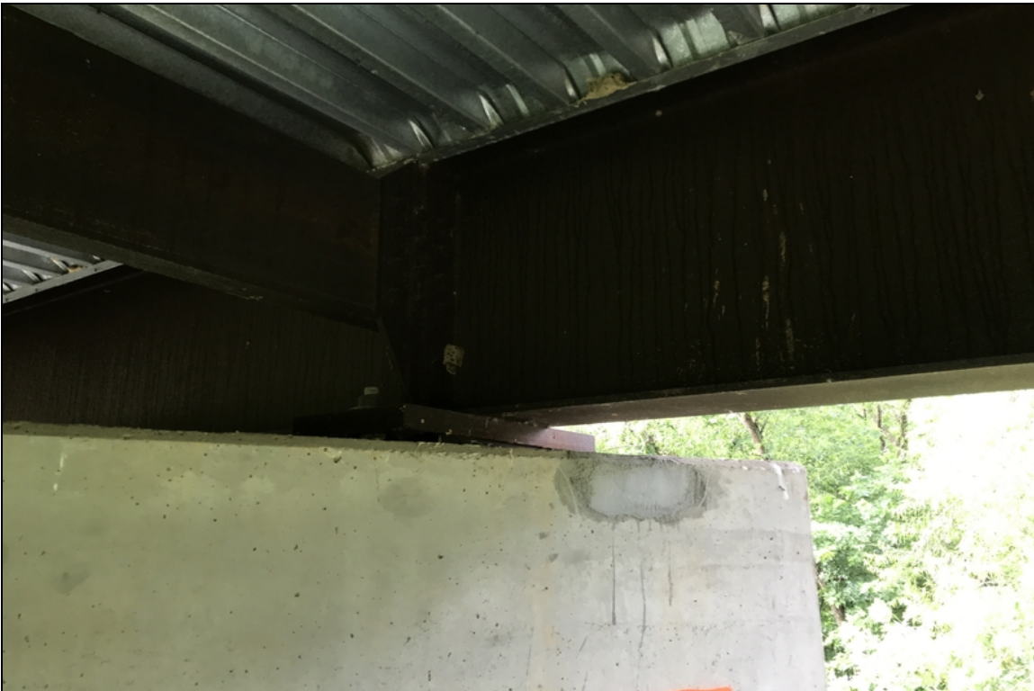
Repaired spall bent #5 pier cap under girder #5
