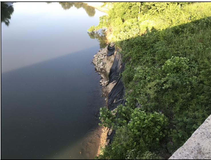
Erosion of the southwest embankment.
