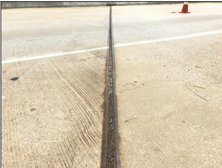
Bent #8 debris in expansion joint.
