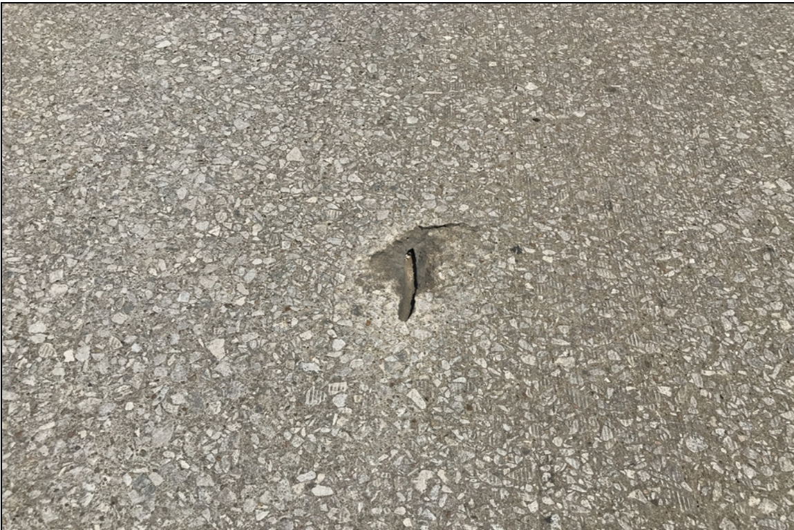
Spall in the left lane in span #8 no steel exposed
