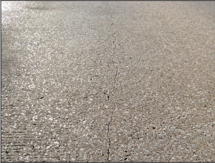
Longitudinal cracking over bent #2.
