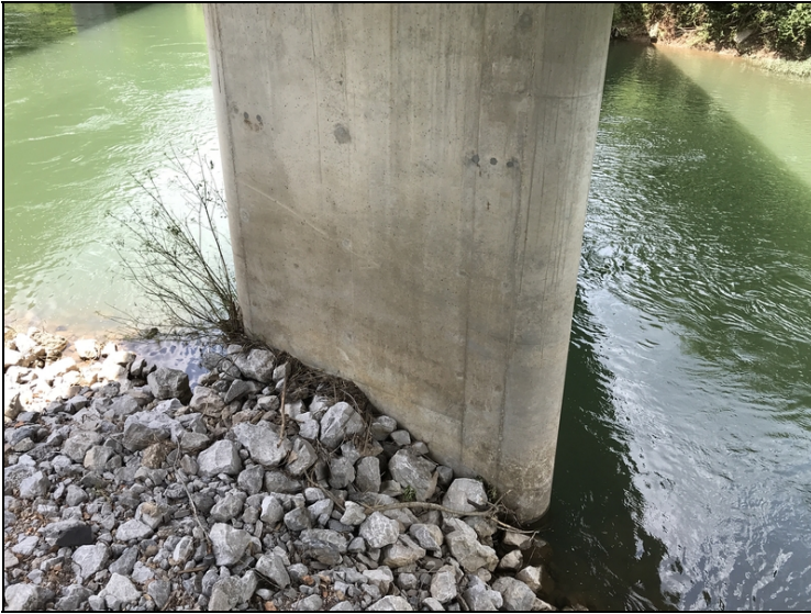
Bent #2 Vertical and diagonal cracking in pier.
