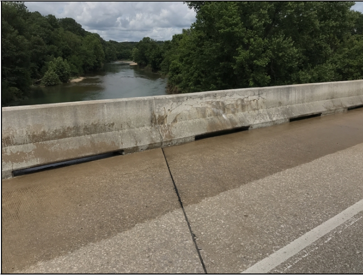
Typical cracking in parapet wall.
