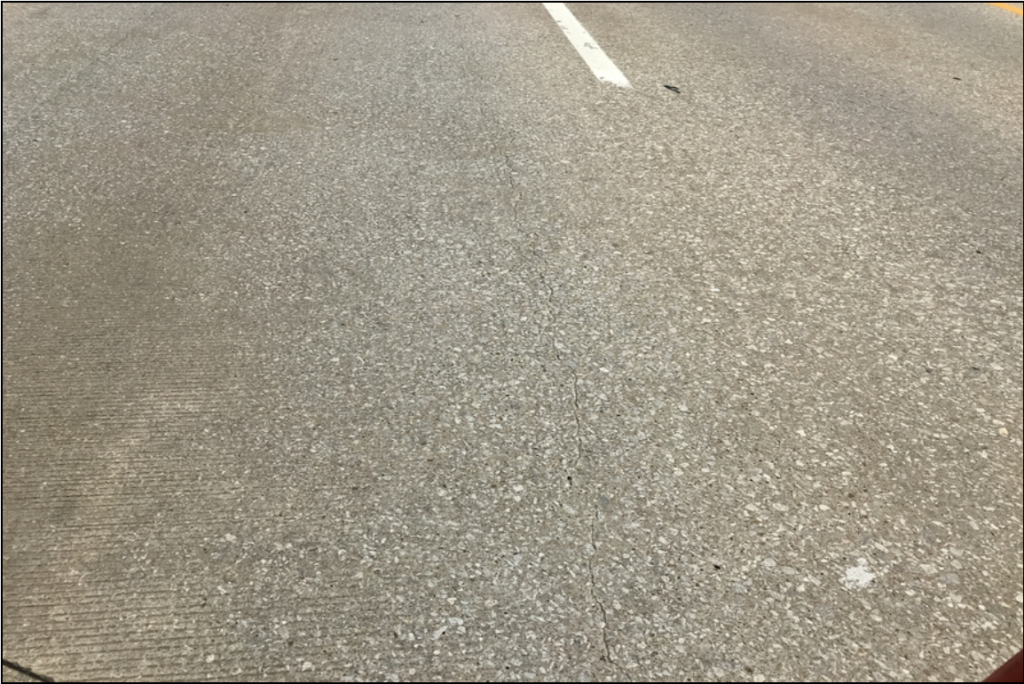
Typical longitudinal cracking in span #3 over bent #2.
