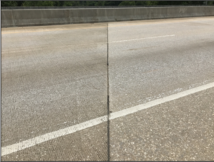
Pourable joint material for construction joints has been displaced.
