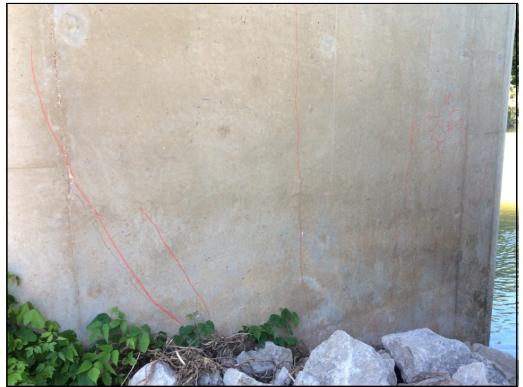
Bent #2-Diagonal cracking in column.
