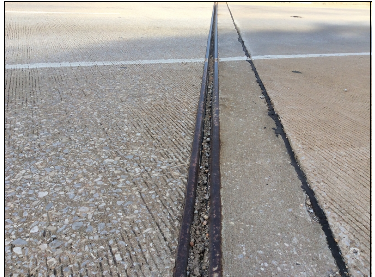
Abutment 1-Debris impaction.
