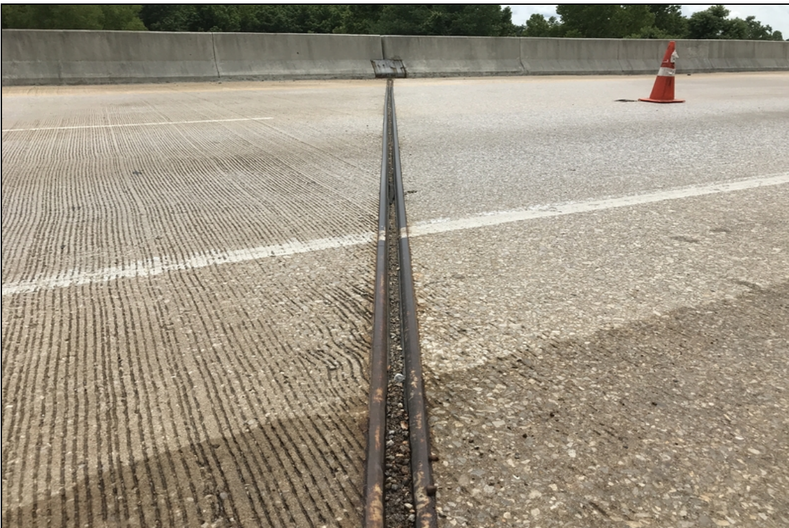
Bent #4 expansion joint debris.
