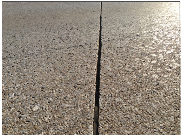
Missing joint sealant.
