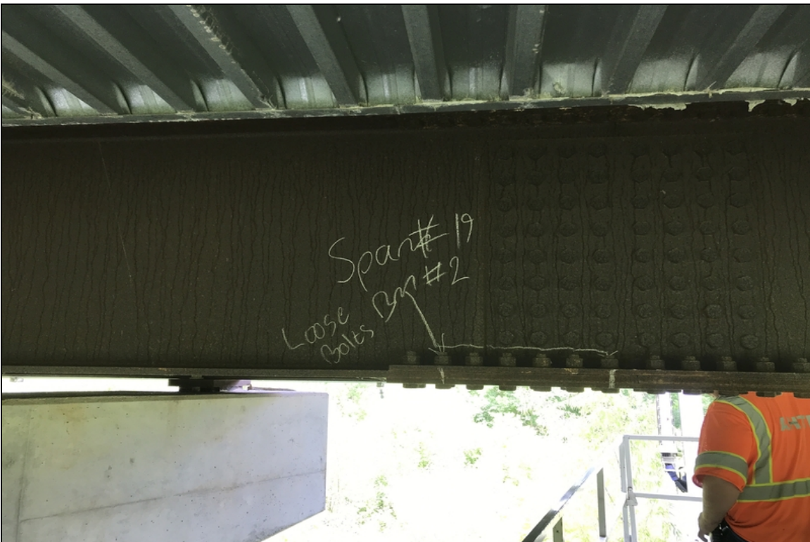
Span #19 Girder #2 has 2 loose bolts.
