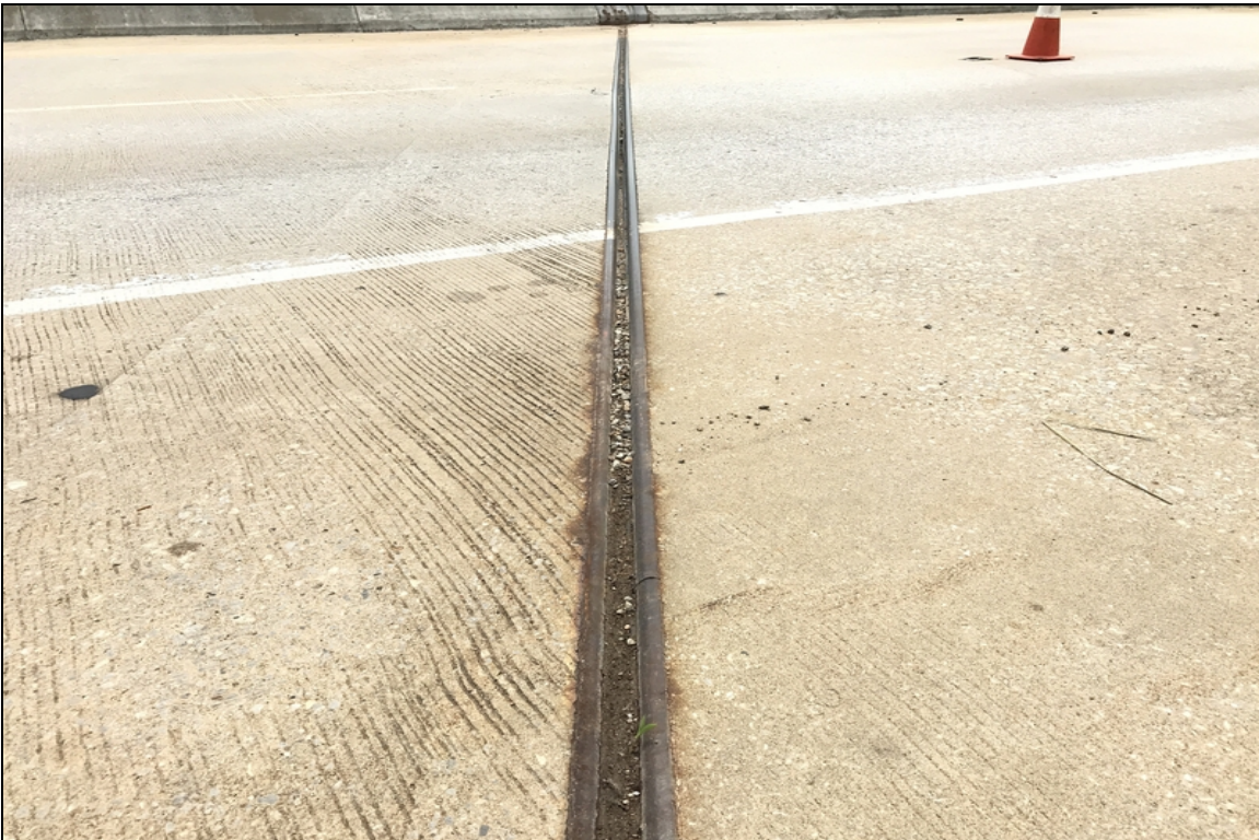
Bent #8 debris in expansion joint.
