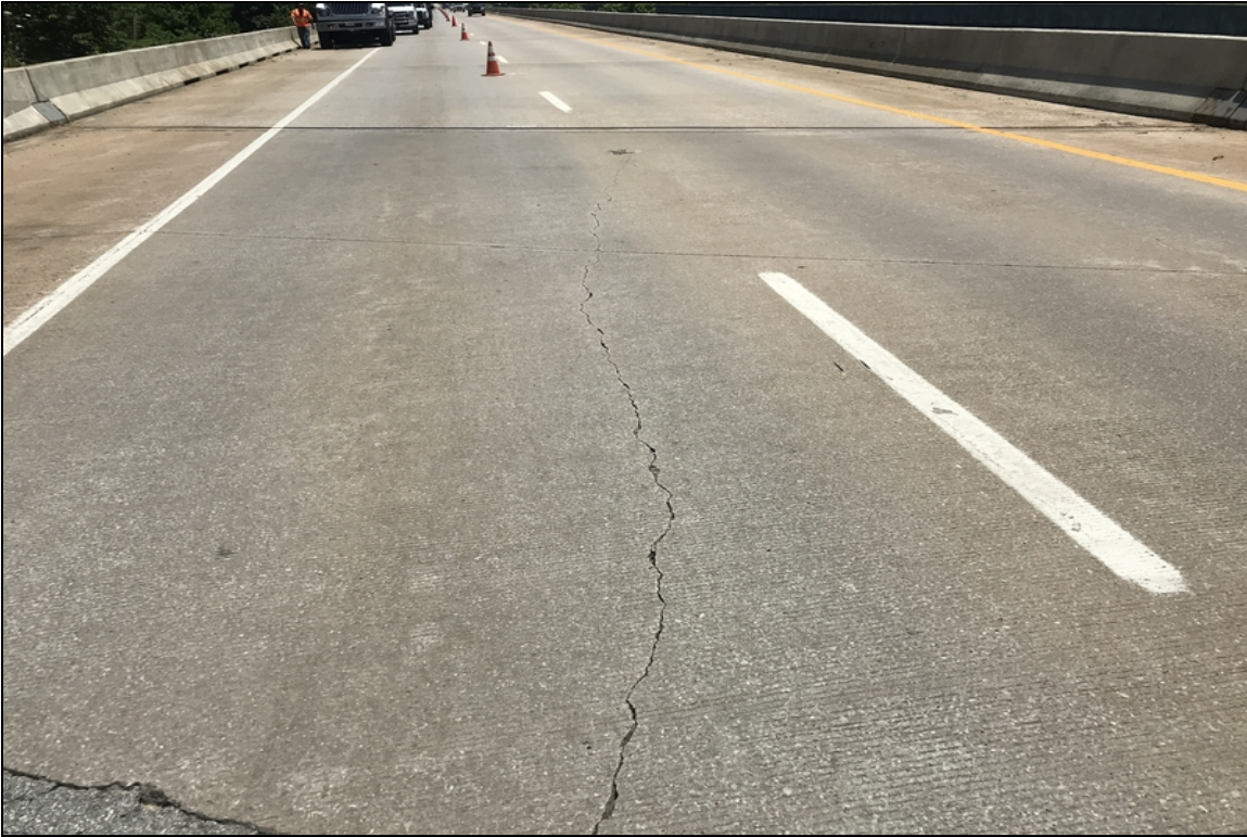
Cracking in the west approach slab.
