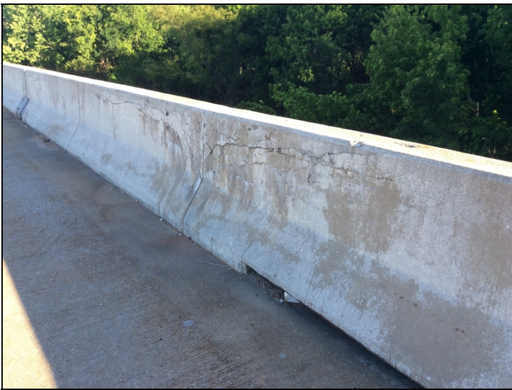
Span 9 parapet wall left typical cracking.
