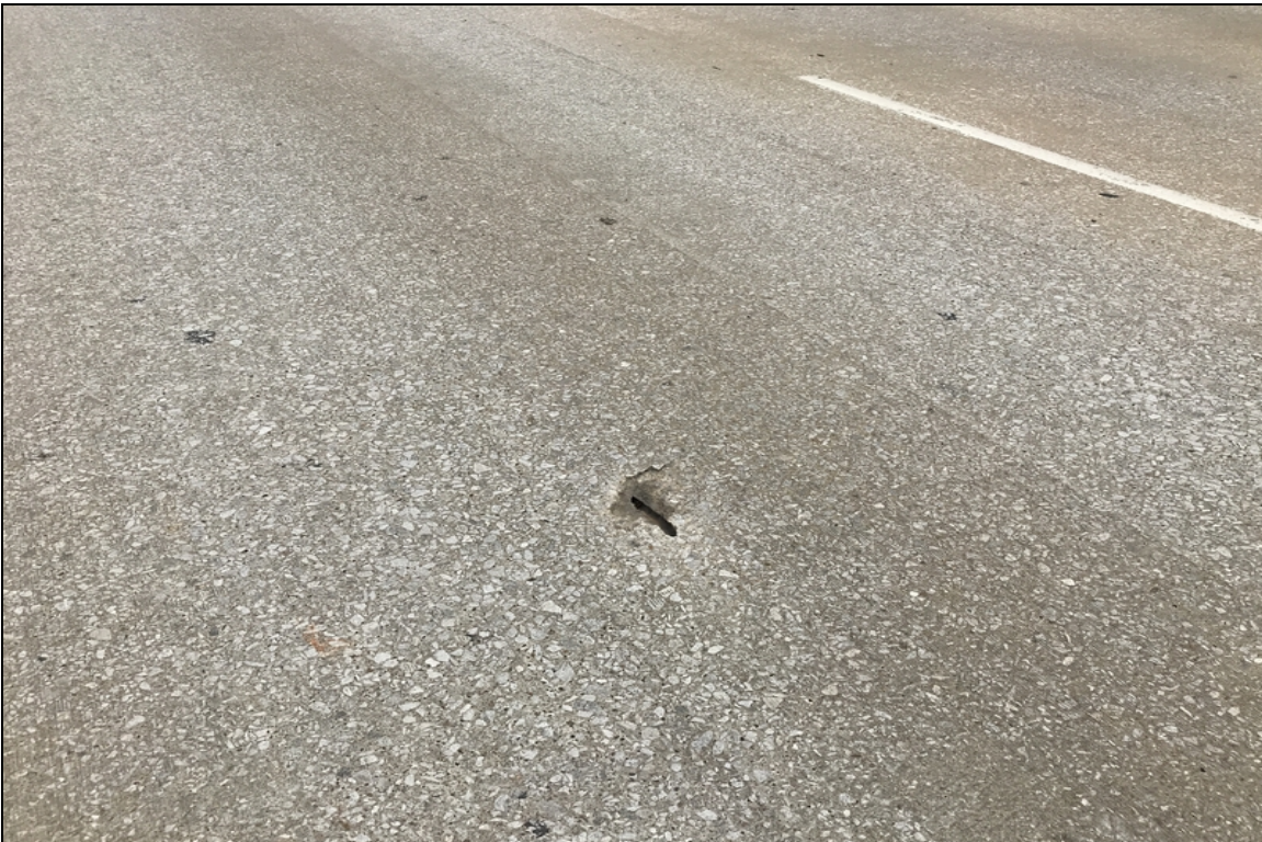
Span #9 softball sized spall.
