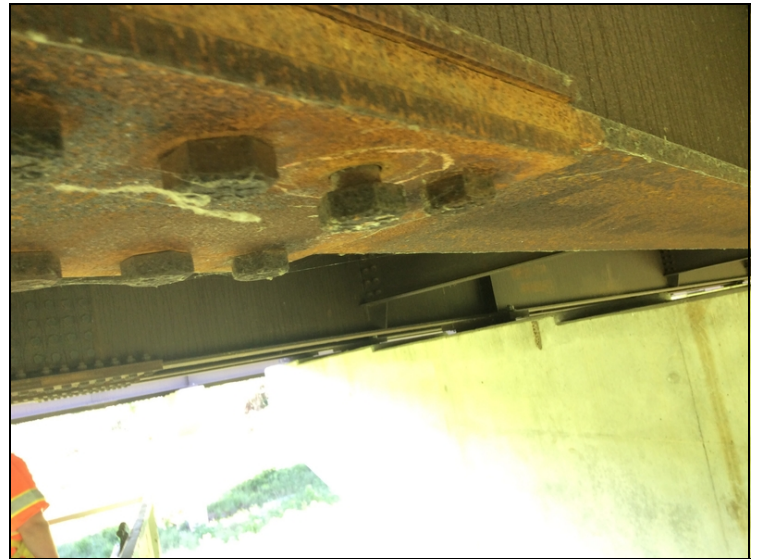
Span #11, Girder #2-Loose splice connection bolt.
