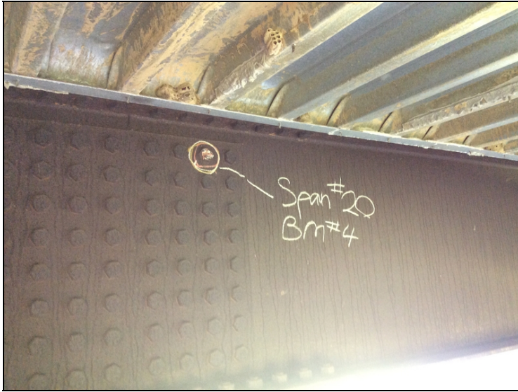
Span #20, Girder #4 has loose splice connection bolt.
