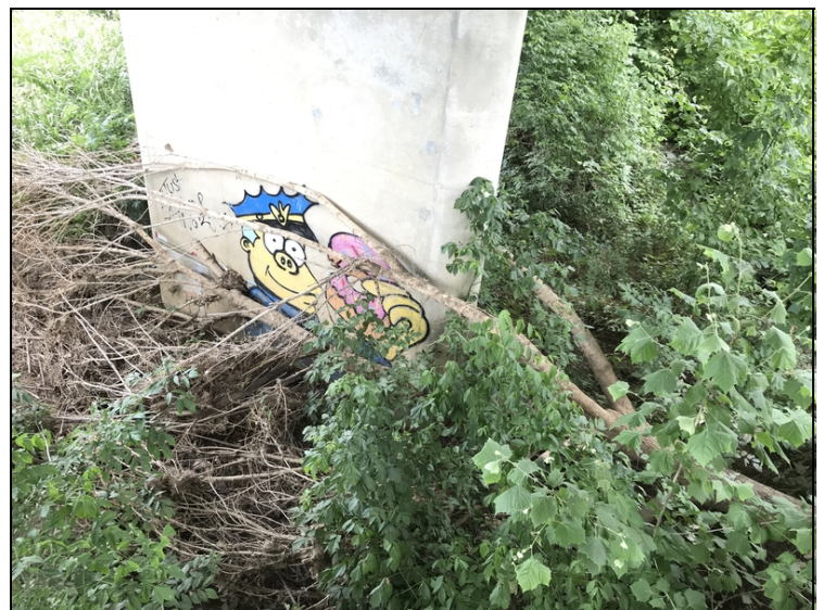
Bent #5 has a tree lodged against Pier.
