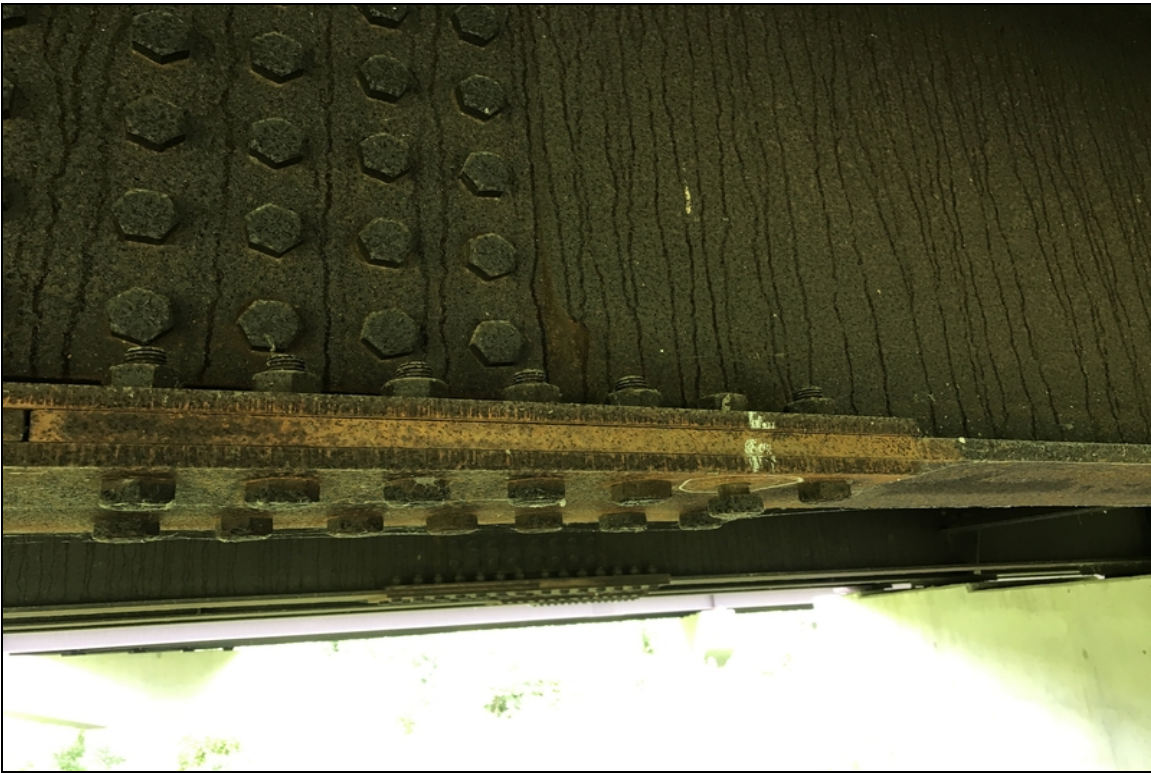
Span #11 Girders #2 loose bolt
