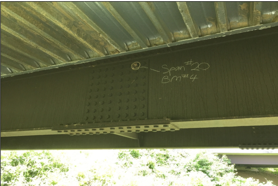
Span #20 girder #4 loose bolt in splice plate.
