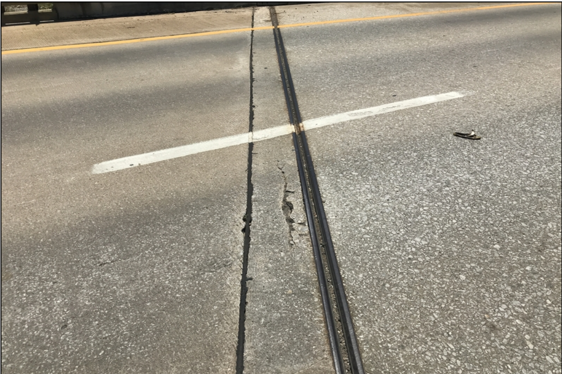
Spalling in the top of abutment #2 breastwall.
