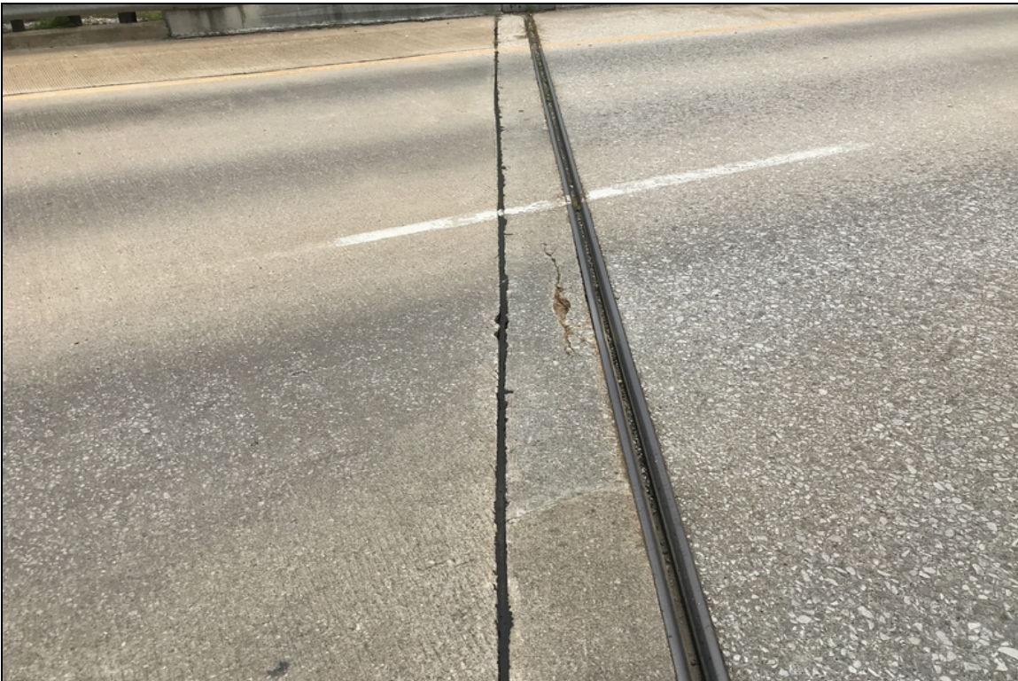
Abutment #2 cracking and spalling.
