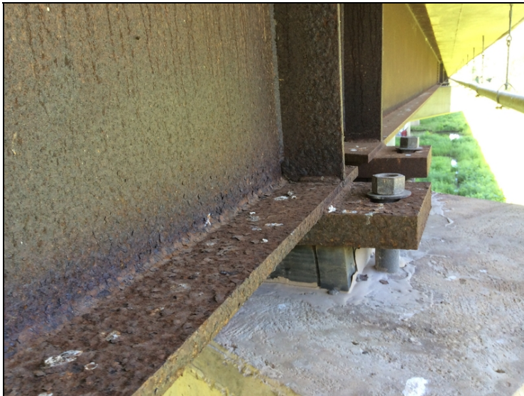
Span #13, end of Girder #1 over bent #12 has an area of corrosion approximately 4' long due to leaking expansion joint.
