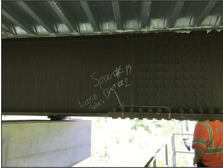
Span #19 Girder #2 has 2 loose bolts.
