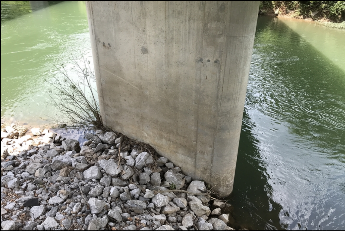
Bent #2 Vertical and diagonal cracking in pier.
