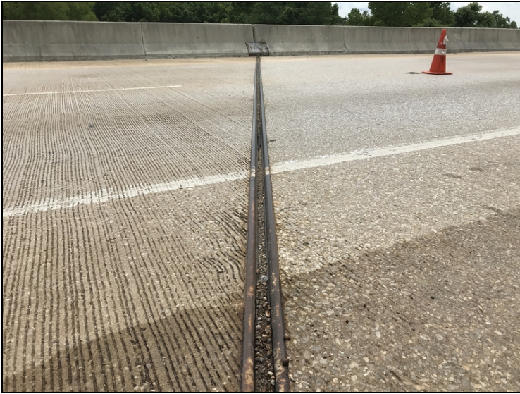
Bent #4 expansion joint debris.
