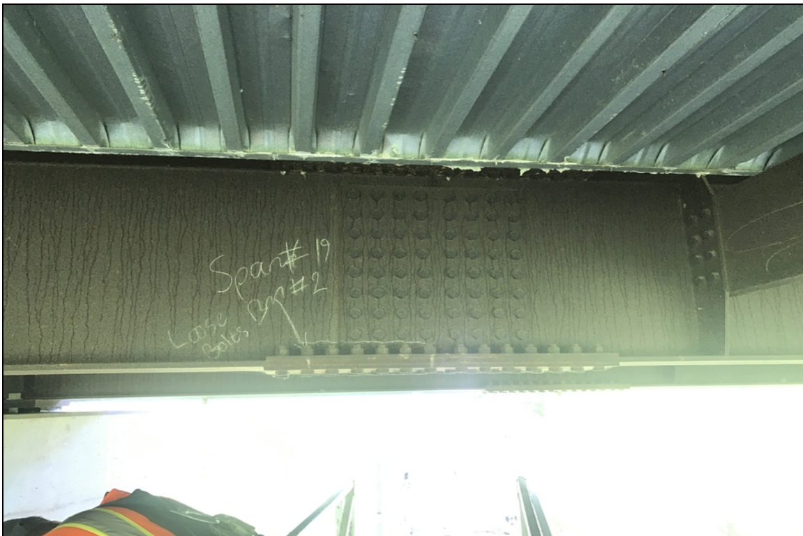
Bolts still loose as of this inspection.
