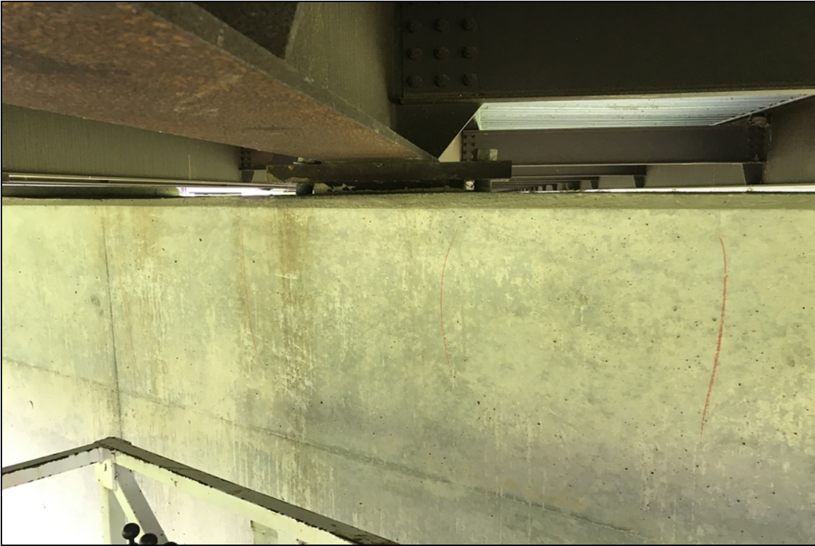
Typical hairline cracking in the tops of pier caps.
