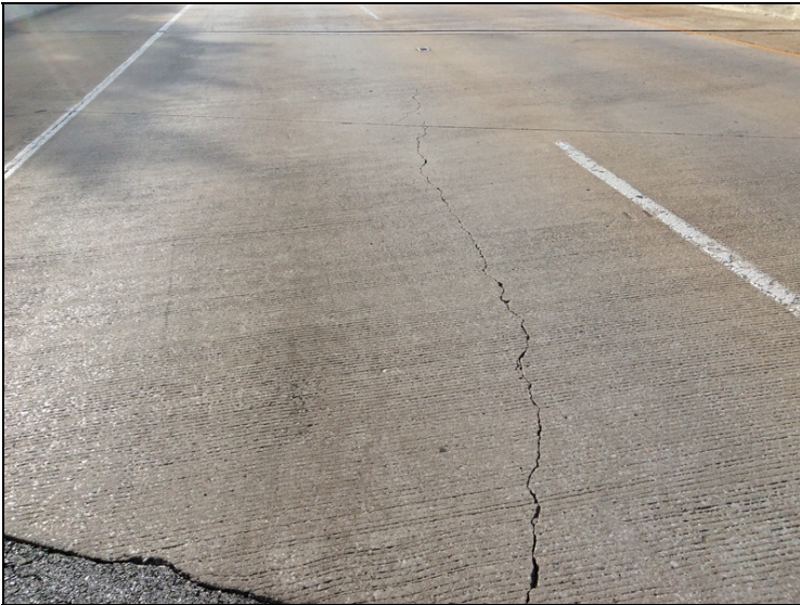
West approach slab-Wide longitudinal cracking.
