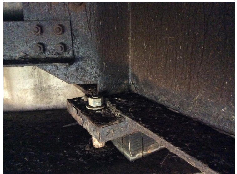
Span #1, Girder #2 at abutment #1-Corrosion due to leaking expansion joint.
