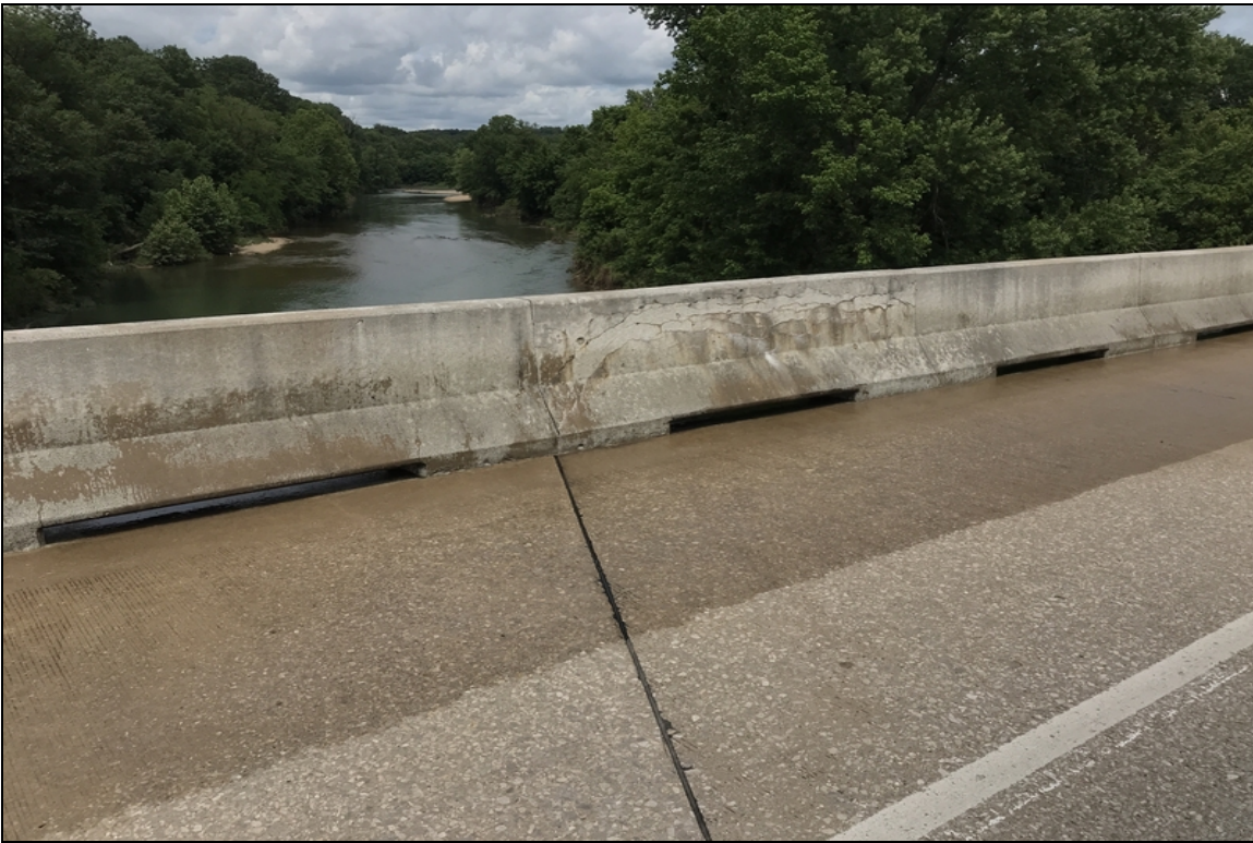
Typical cracking in parapet wall.
