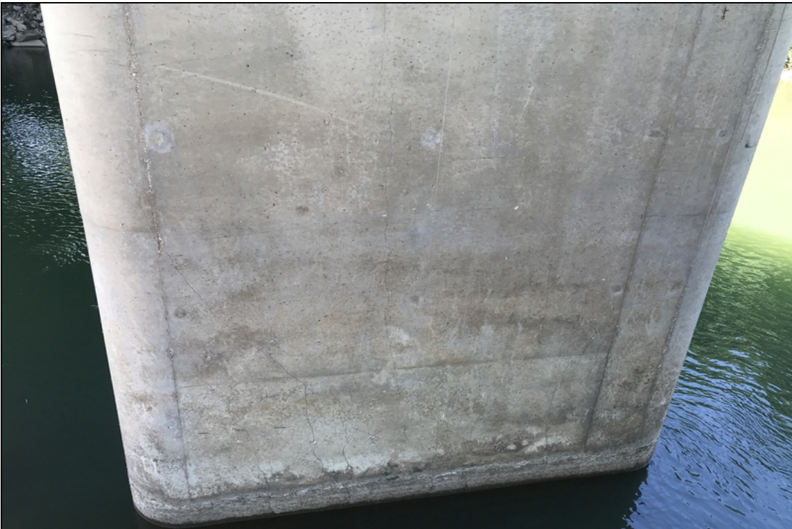
Cracking in pier #2 ahead side still exists.
