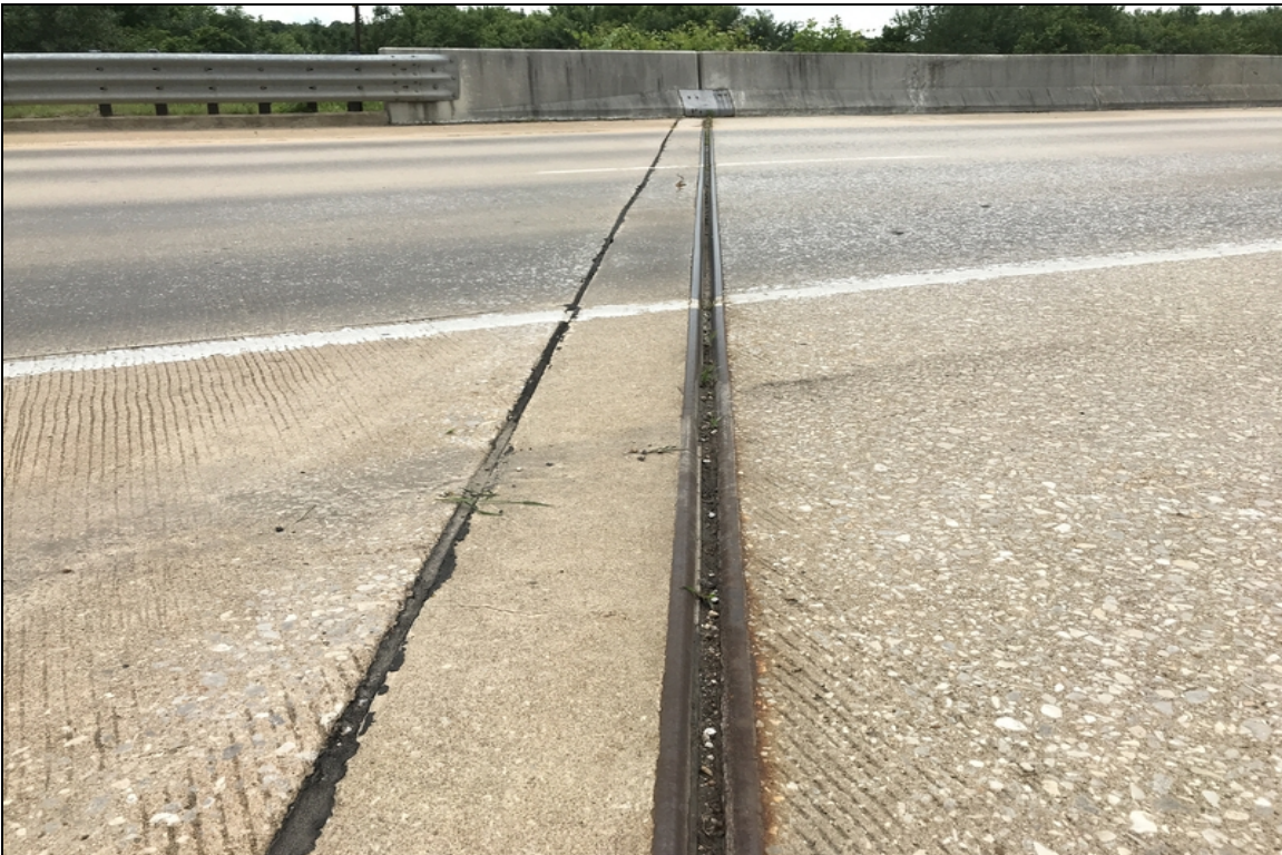
Abutment #2 expansion joint material debris impaction.
