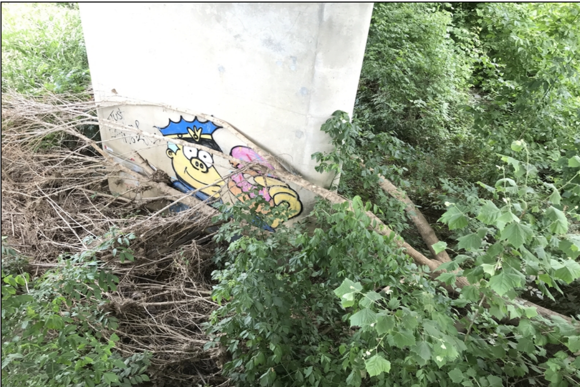
Bent #5 has a tree lodged against Pier.
