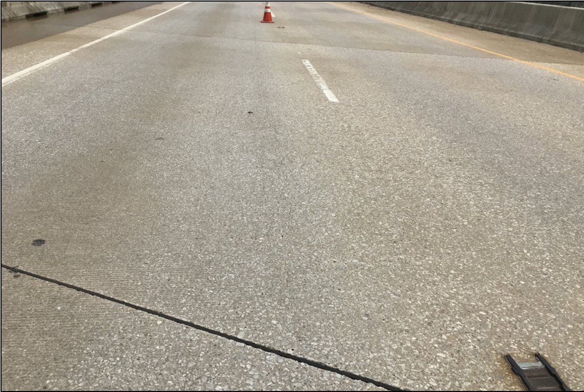
Typical longitudinal cracking.
