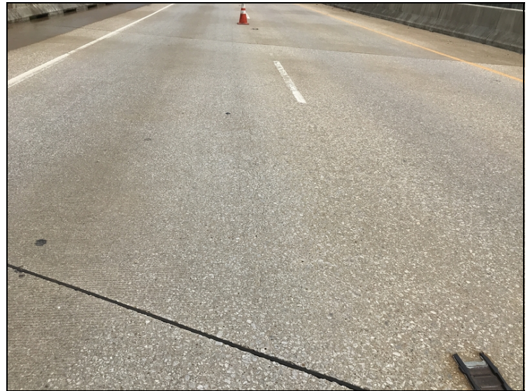
Typical longitudinal cracking.
