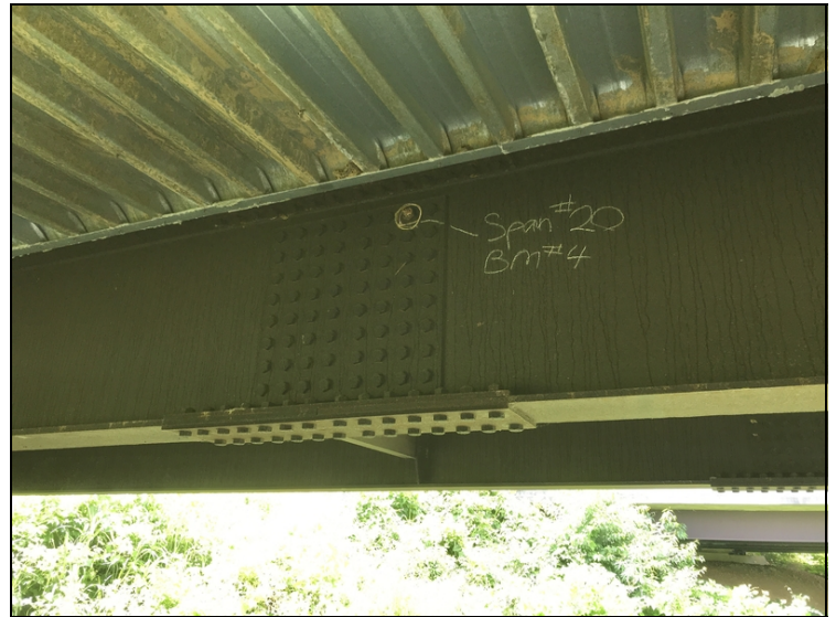
Span #20 girder #4 loose bolt in splice plate.
