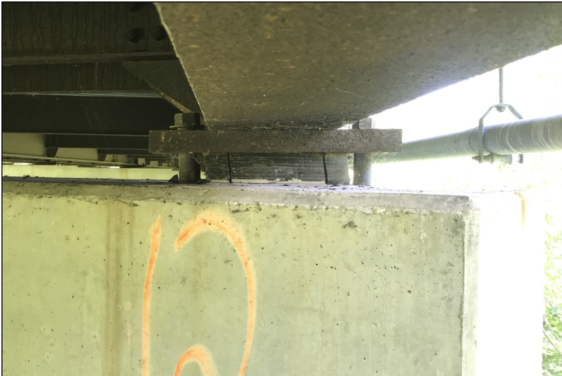
Elastomeric bearing #1 in span #13 over bent #12 is skewed out of plum.
