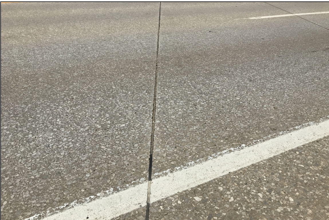
Pourable joint material has been displaced in multiple locations.
