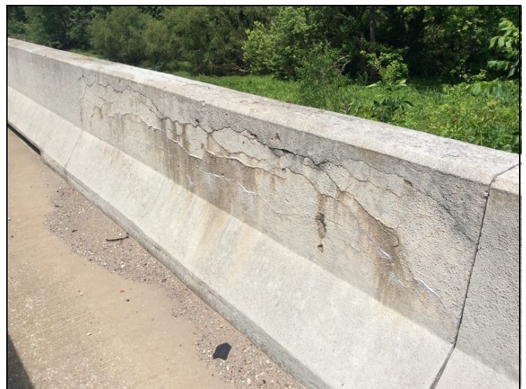
Span #20, left bridge railing-Cracking.
