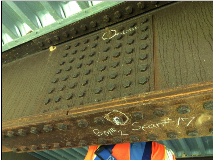
Span #17, Girder #2-Loose splice plate connection bolts.
