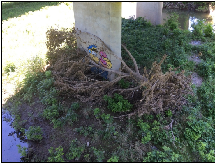
Bent #5-Tree lodged against bent.
