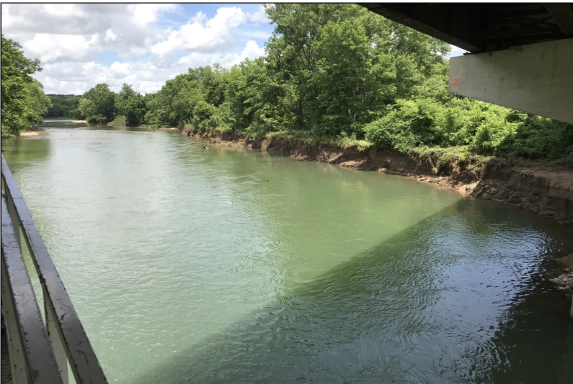
East side of upstream channel has bank erosion.
