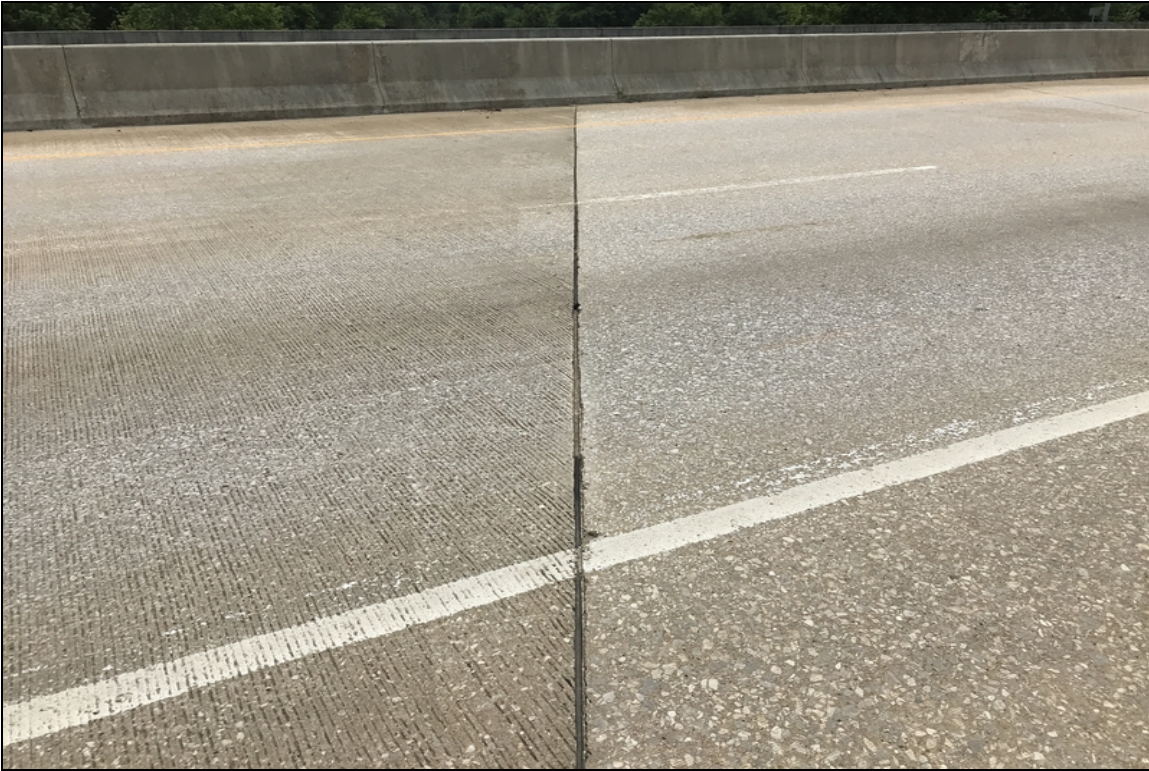
Pourable joint material for construction joints has been displaced.
