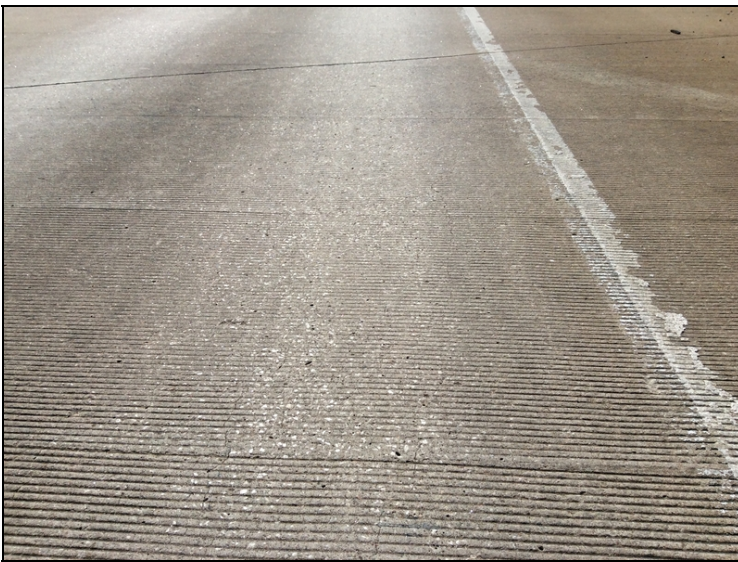
Typical of sealable deck cracking.
