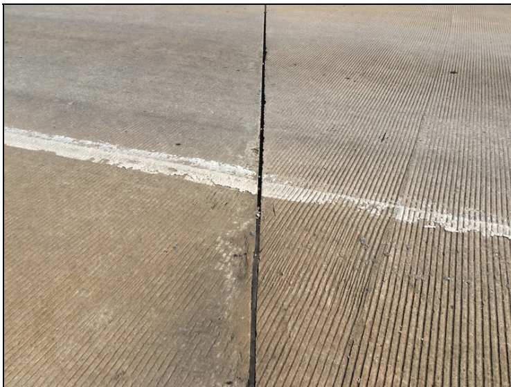
Typical of pourable joint material in the construction joints right lane.
