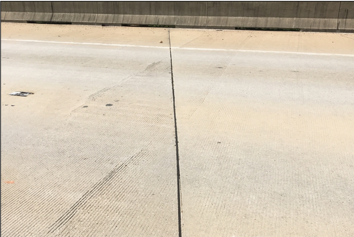
Loss of pourable joint material typical.
