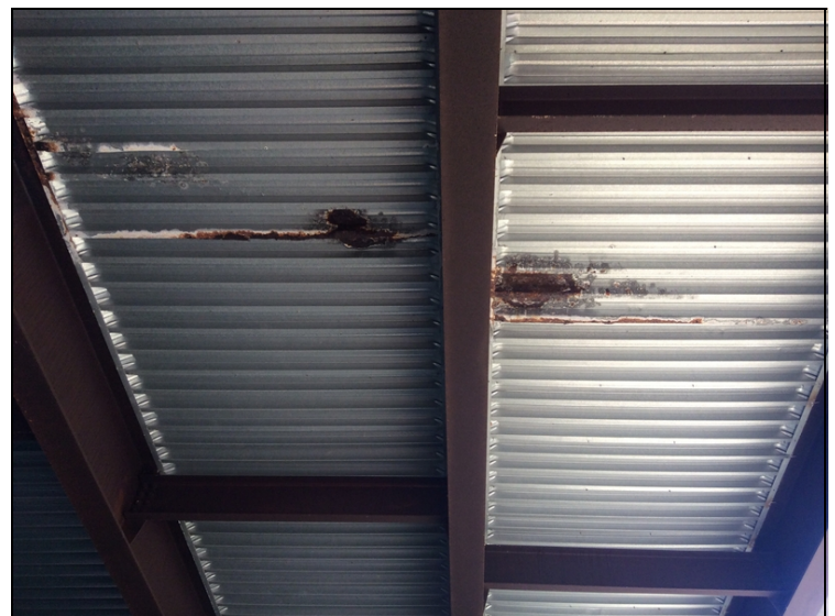
Span #1, bays #1 and #2-Corrosion to SIP forms.
