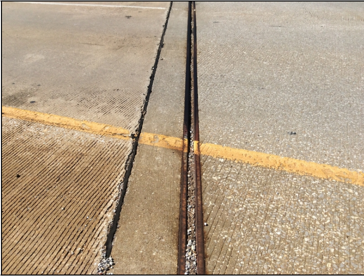
Typical - compression joint seals have debris impaction.
