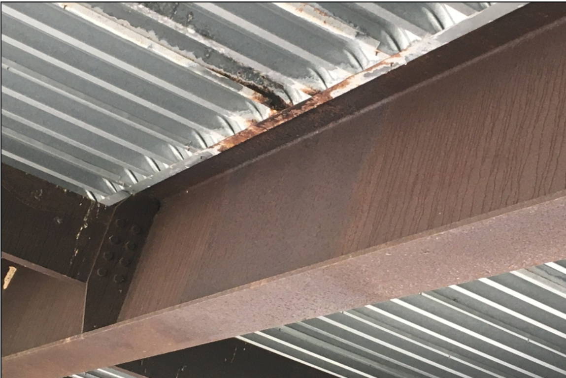
4' of corrosion on beam #3 in span #1.
