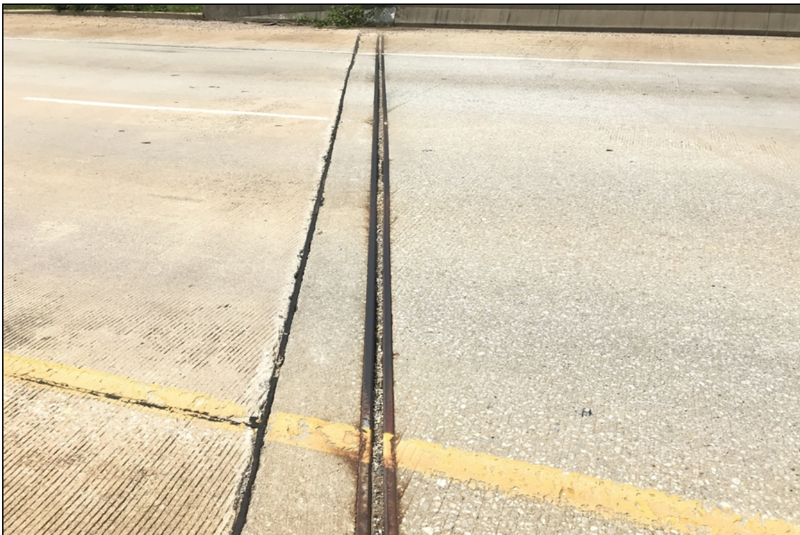
Abutment #2 joint material debris impact and loss of adhesion.
