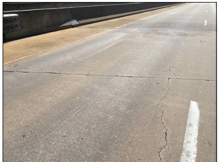
Typical cracking in the right lane of west approach slab.
