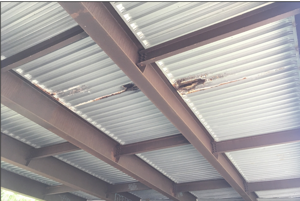
Span #1 bays #1 & #2 active corrosion of SIP forms.
