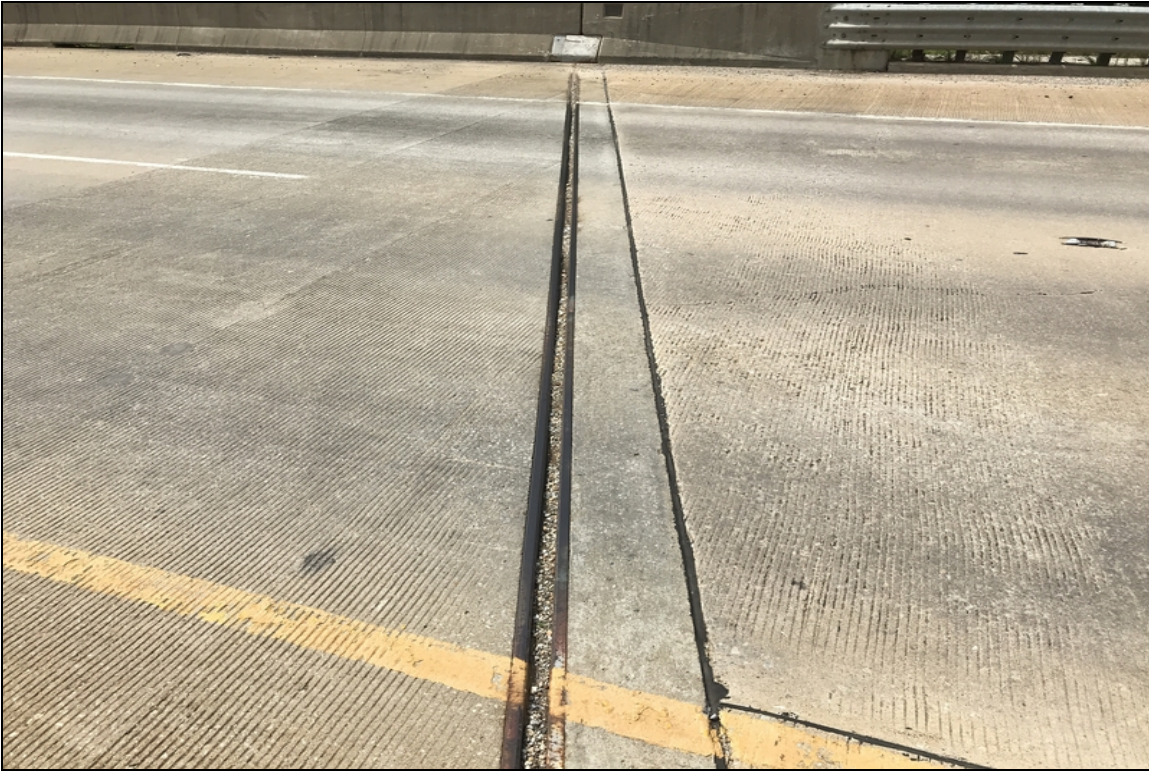
Abutment #1 joint material debris impaction and loss of adhesion.
