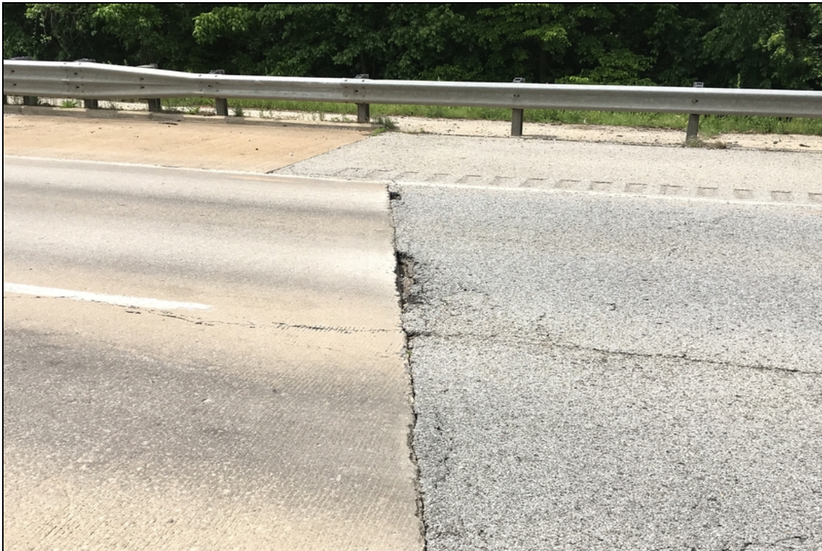
West approach roadway adjacent to west approach slab right lane potholes.
