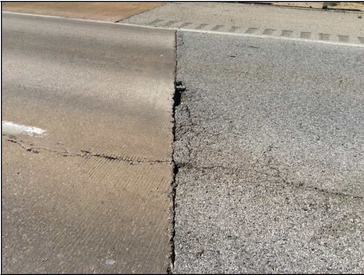
Approach roadway at Right lane of west approach roadway - pothole.
