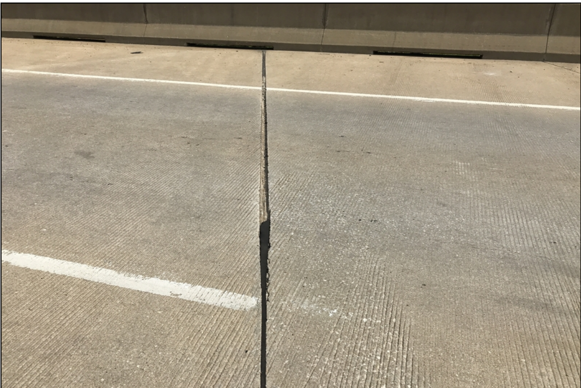
Construction joint pourable material missing. Typical
