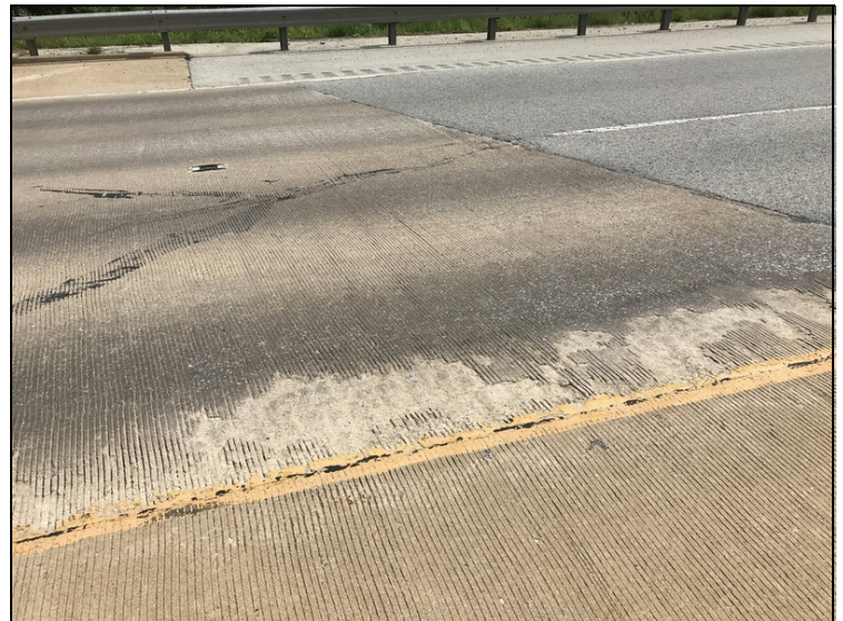
East approach slab minor spalling adjacent yellow line.
