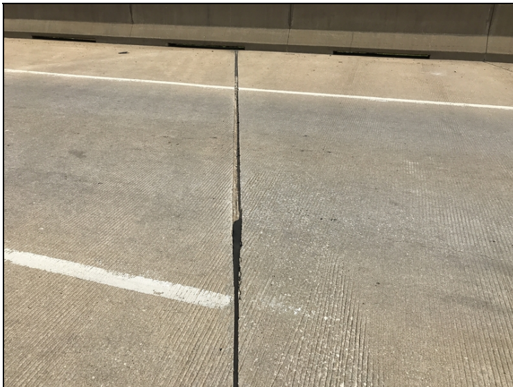
Construction joint pourable material missing. Typical
