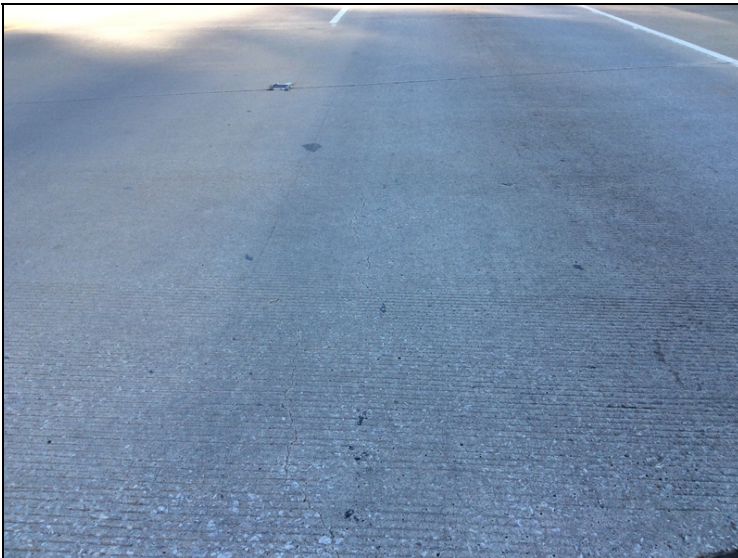
Deck Left lane over bent 2 longitudinal cracking.
