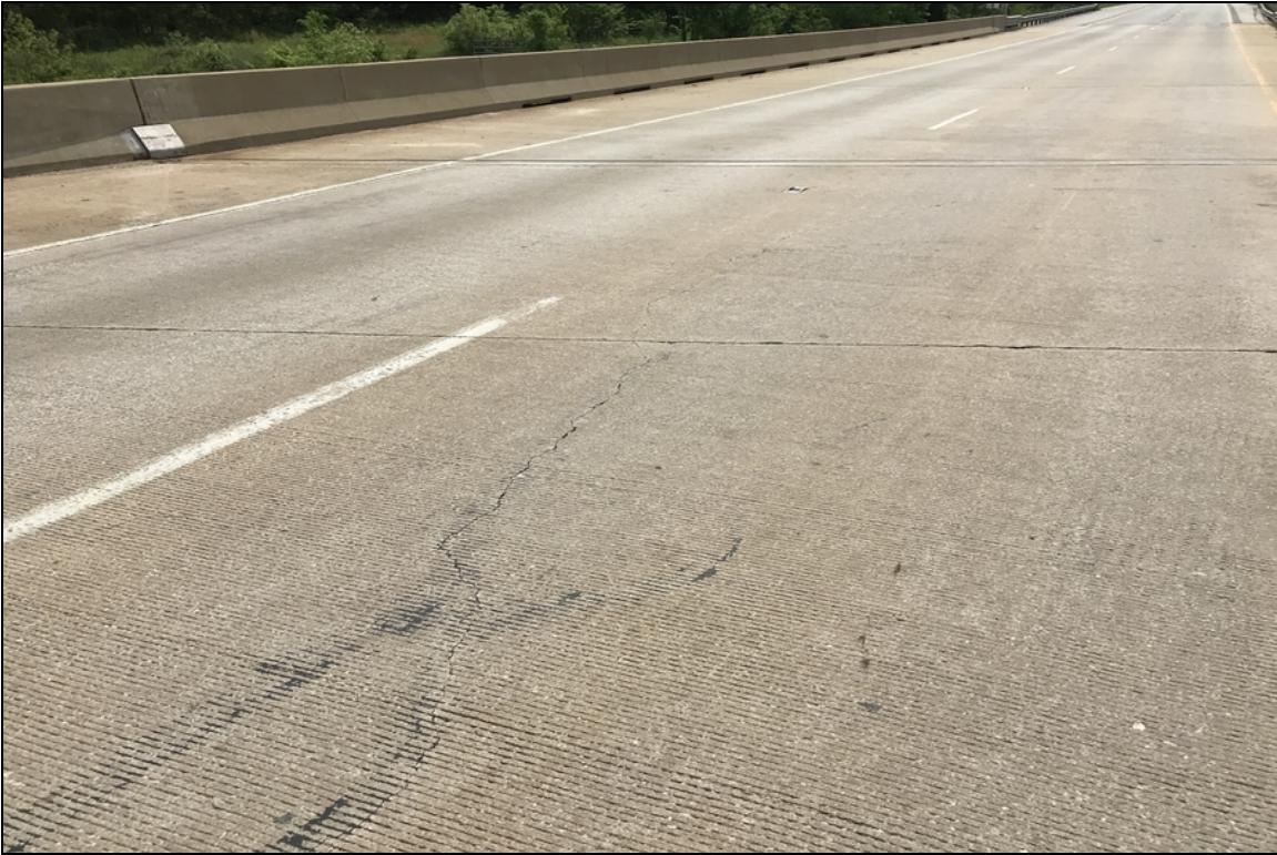
Large cracking in west approach slab.
