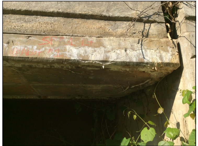
Span #1, Left side-Delaminated area with cracking and efflorescence.
