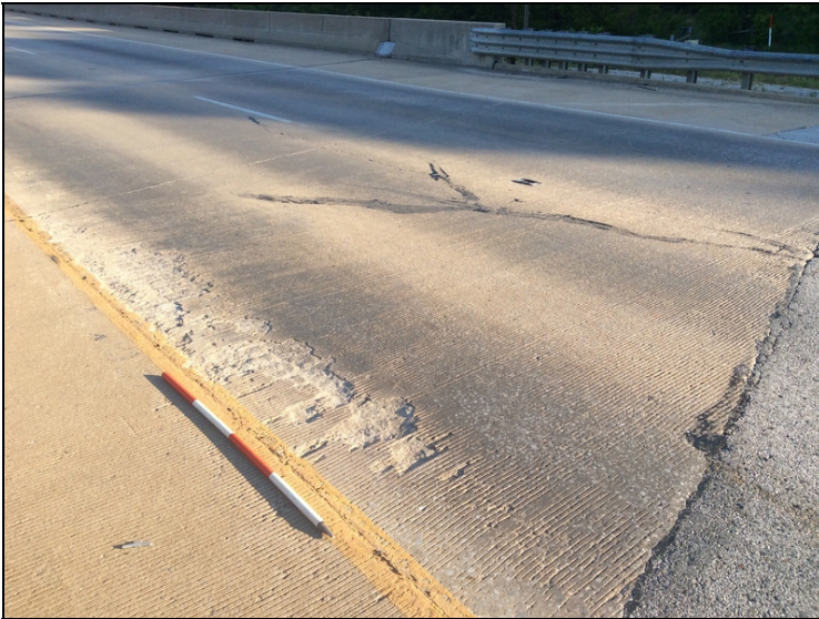
East approach slab has cracking and spalling.
