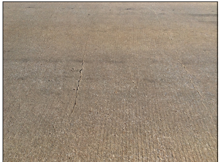
Span #1, outside lane-Transverse cracking.
