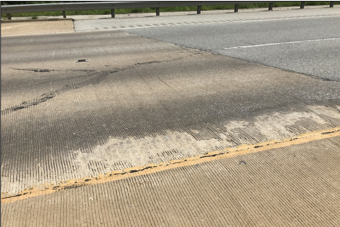
East approach slab minor spalling adjacent yellow line.
