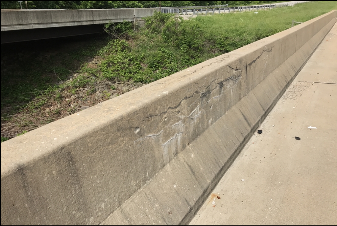
Parapet Railing right cracking with efflorescence.
