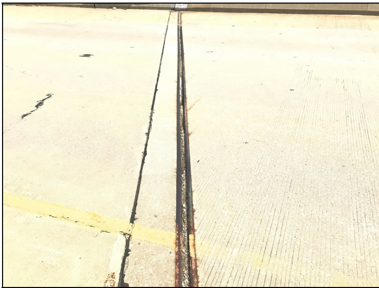
Abutment #1 joint material has debris impaction and loss of adhesion
