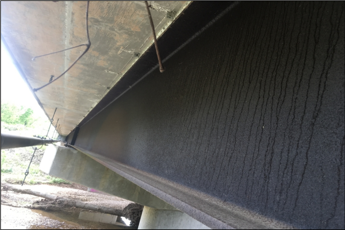
Areas of cs2 corrosion on the exterior of beam #1 in all 3 spans.
