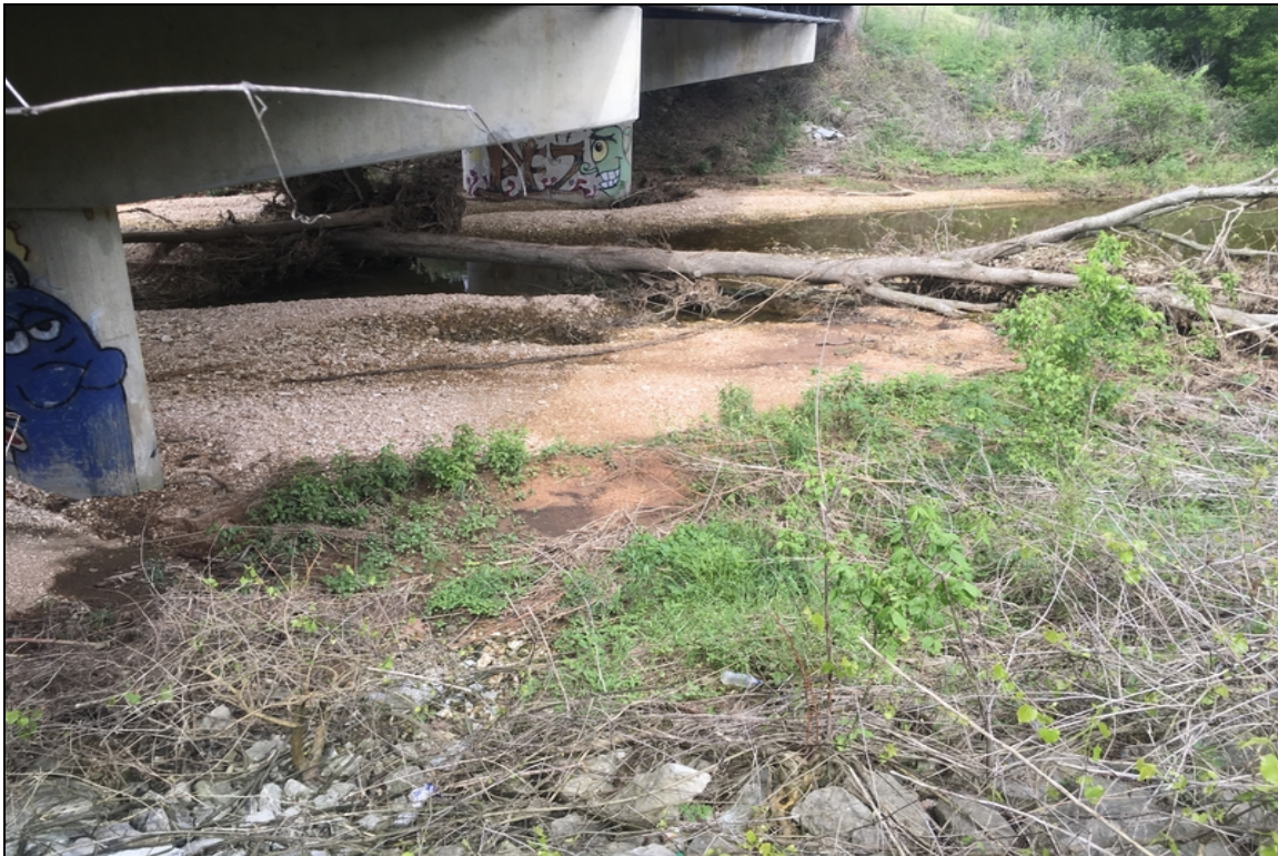
Span #2 has a large tree in the channel.
