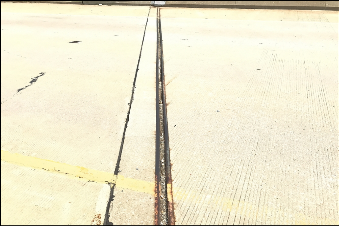
Abutment #1 joint material has debris impaction and loss of adhesion
