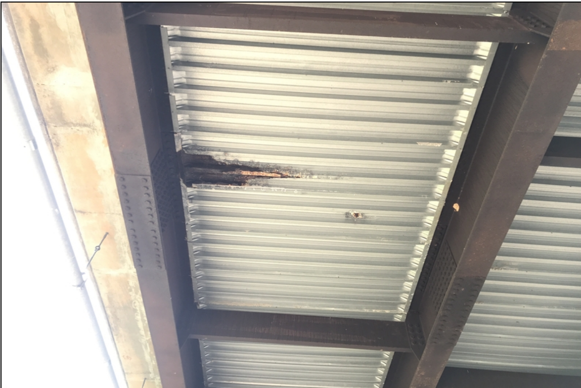
Span #2 bay #1 approximately 13' behind bent #2 corrosion of SIP form.
