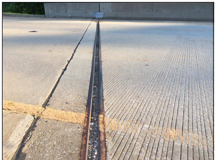
Abutment 1 compression joint seal- debris impaction.
