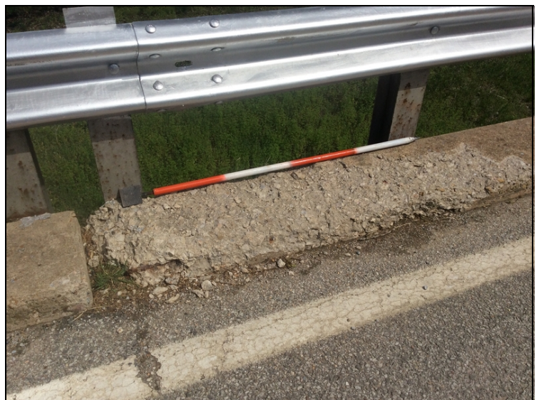
Deterioration at the left curb of structure typical of several locations.
