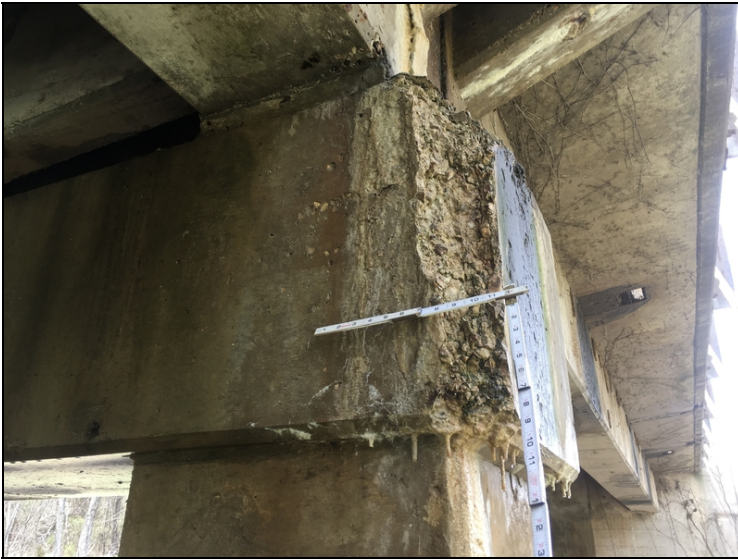
The left cap end of bent #1 showing deterioration for 1'.
