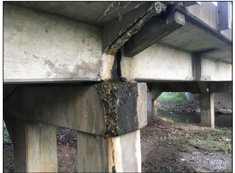
Left end of bent cap 2 showing spalling with rebar exposed.
