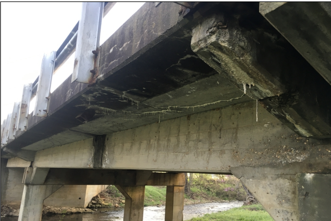
Efflorescence in the right overhang of span 2.
