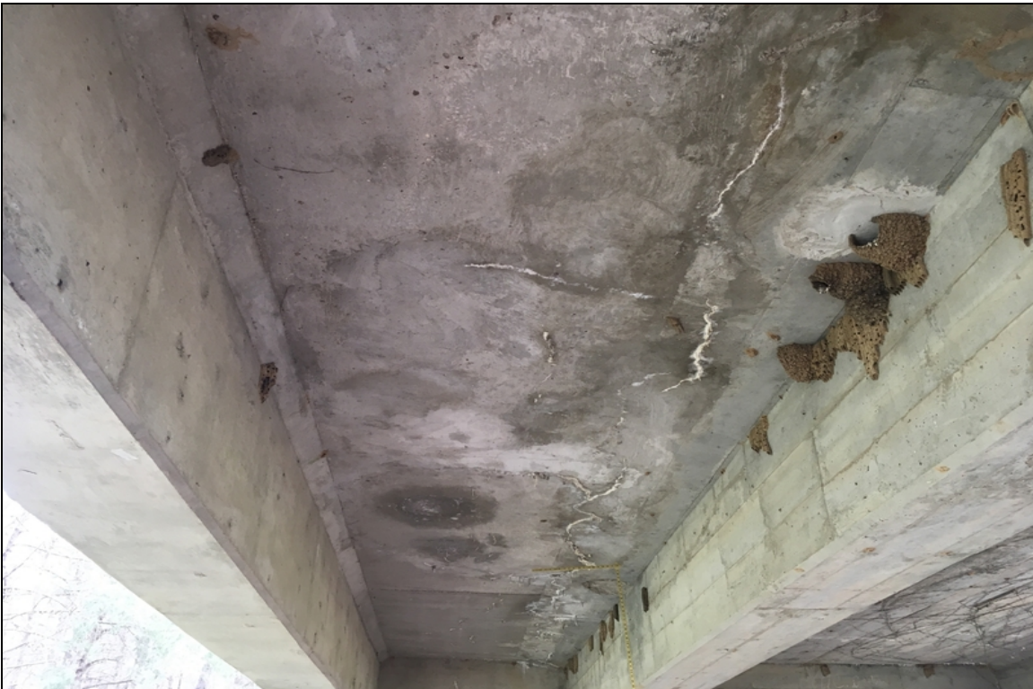
The deck soffit in span #2 bay #1 has heavy efflorescence cracking with rust staining between tee beams #1 and #2
