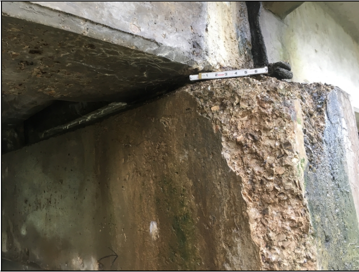
Map cracking with efflorescence on the underside of tee beam #1 at the beginning of span #3. The tee beam was sound under hammer blows.
