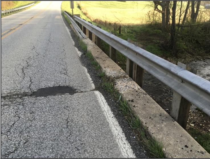
Deterioration in the left curb section.
