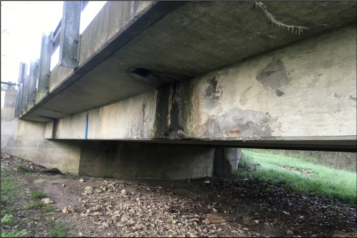
General condition of beam 1 in span 3. Showing spalling with rebar exposed and delamination.
