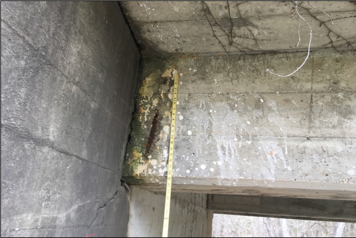
Tee beam #3 has a shallow exposed rebar at the beginning of span #1.
