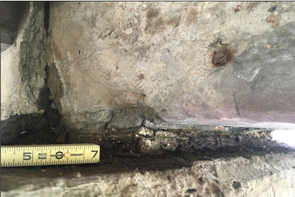
Steel bearing under beam #1 at pier #2. Typical of both.
