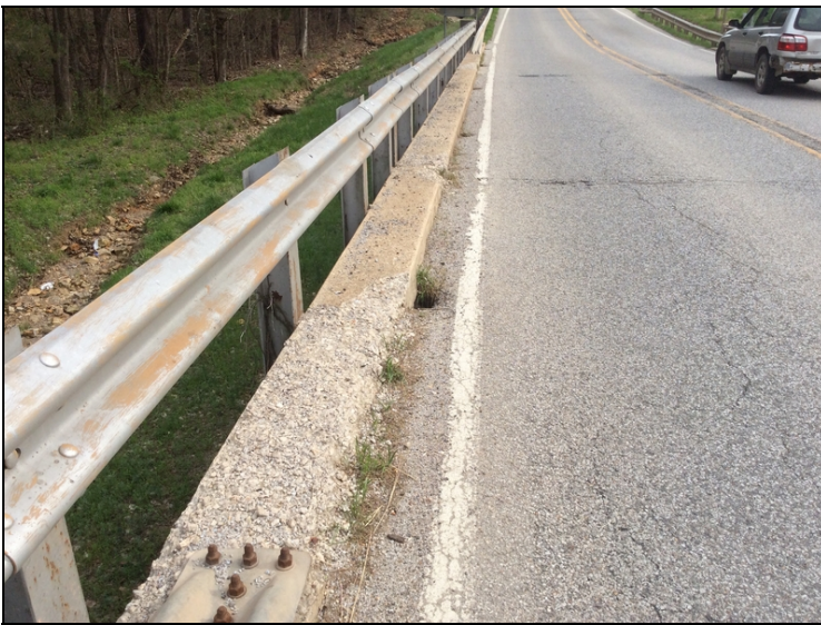
Deteriorated curb areas at left side of structure
