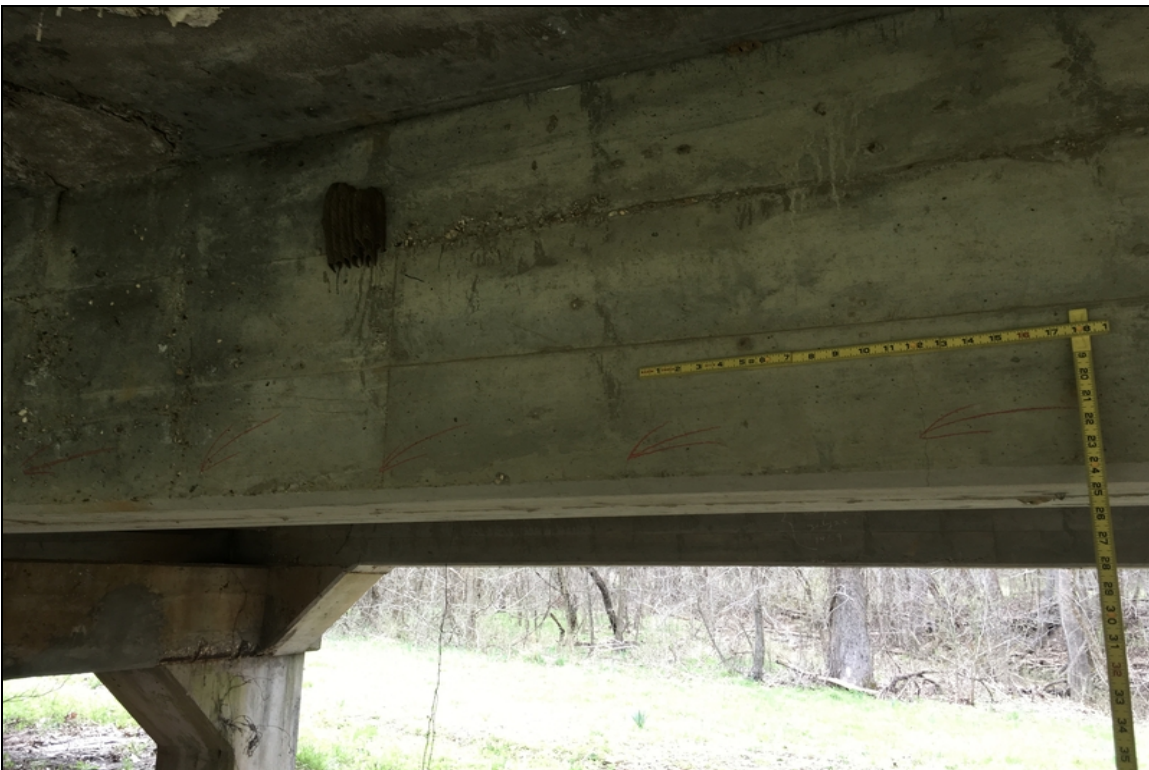
Flexure cracking in beam #2 in span #2. Approximate spacing of 12".
