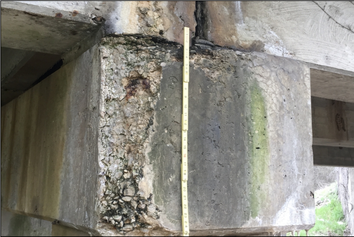
The left cap end of bent #1 has large areas of deteriorated concrete, these areas have not yet affected the bearing area
