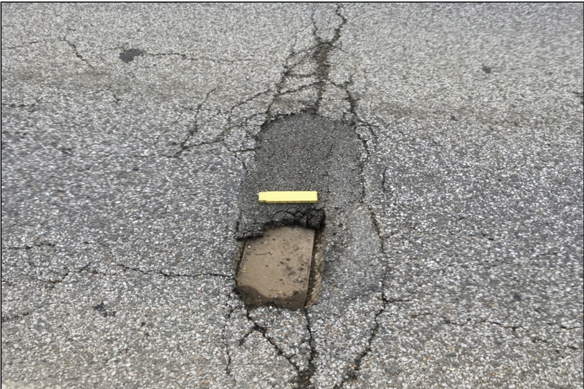
Pot hole in the right driving lane over the joint area.
