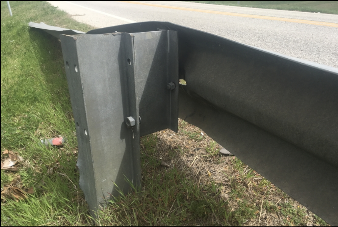
Connection bolt has pulled through the metal railing at the first post of the right side approach railing
