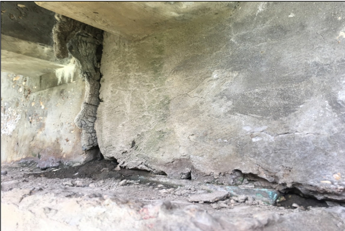
Original brass Bearing condition under beam #3 over bent #2.
