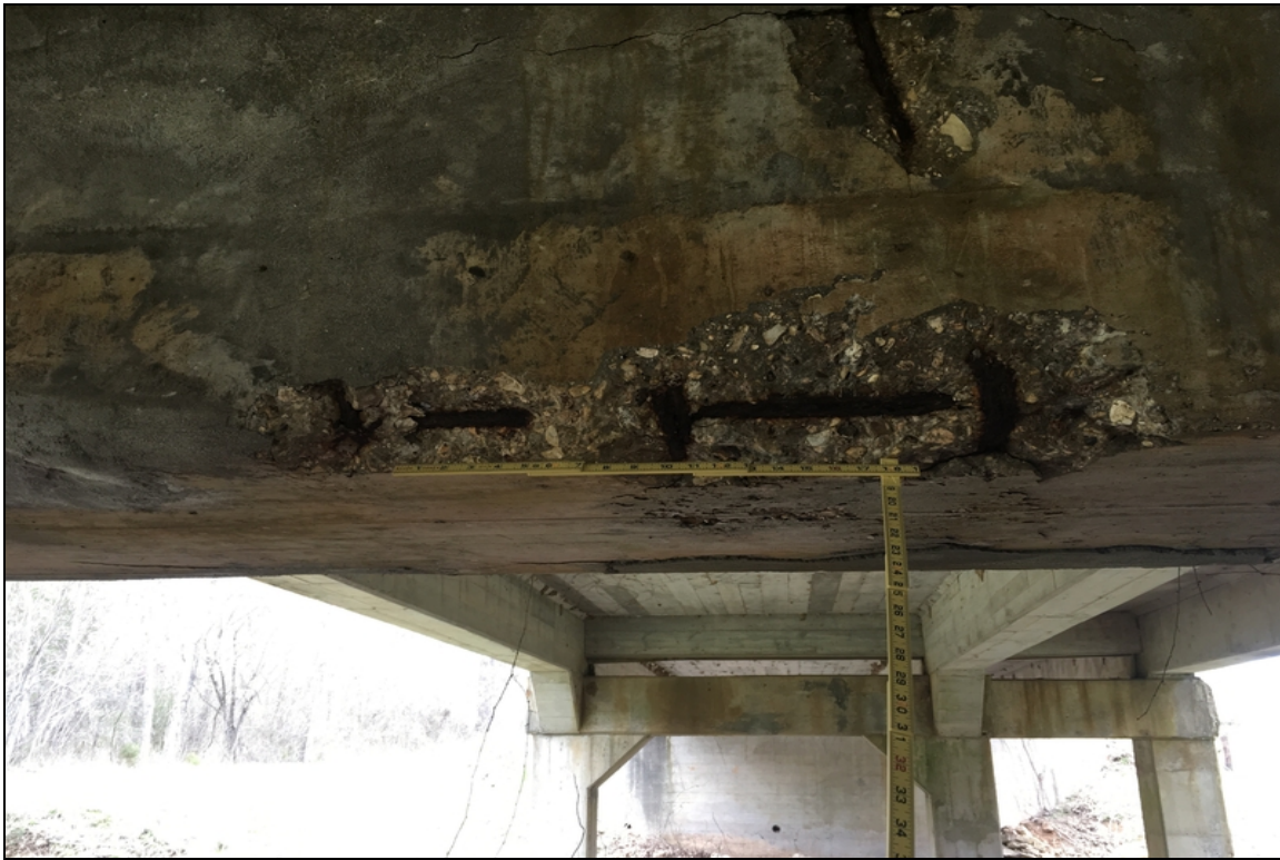
Spalling with rebar exposed on bent #2 cap.
