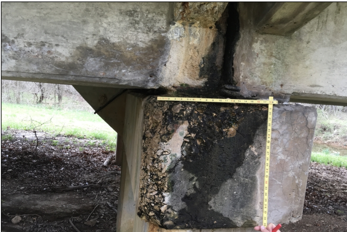
The left cap end of bent #2 has large areas of deteriorated concrete, these areas have not yet affected the bearing area
