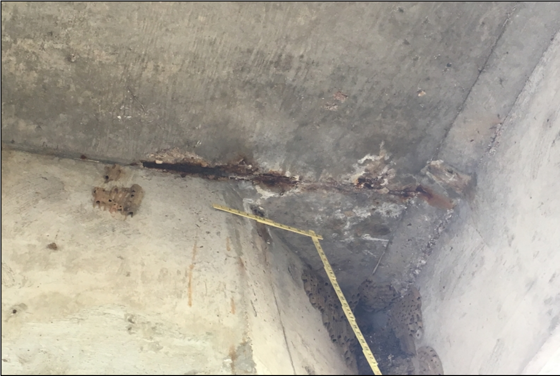
Spall with rebar exposed between beams #1 and 2 in span #1.
