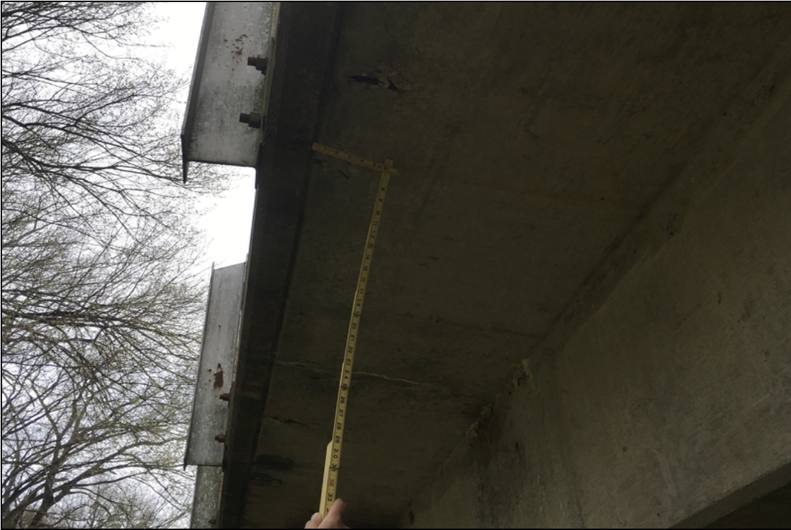
The deck soffit in the left and right overhangs of span #1 and span #2 has deep spalling with exposed rebar.
