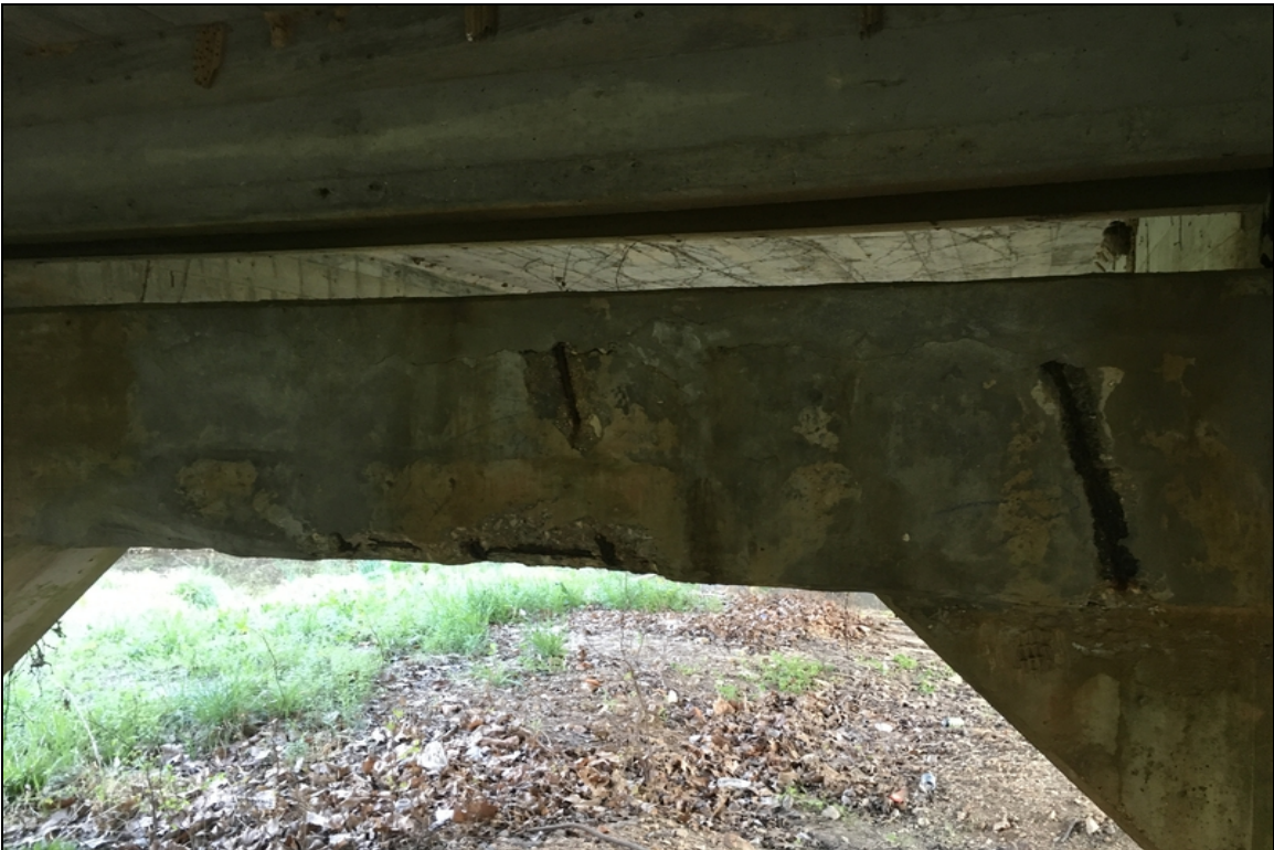
Spalling with rebar exposed on the span 3 side of the bent 2 cap.
