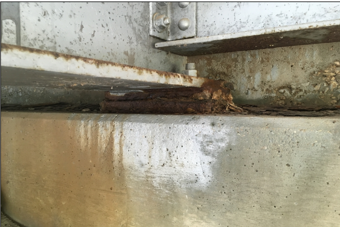
Abutment #1 bearing corrosion. Typical except bearing #4.
