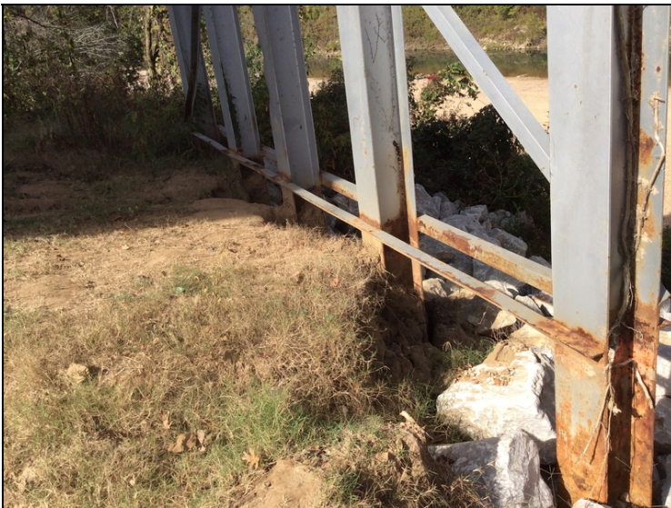
General view of erosion to bent #5 piling.
