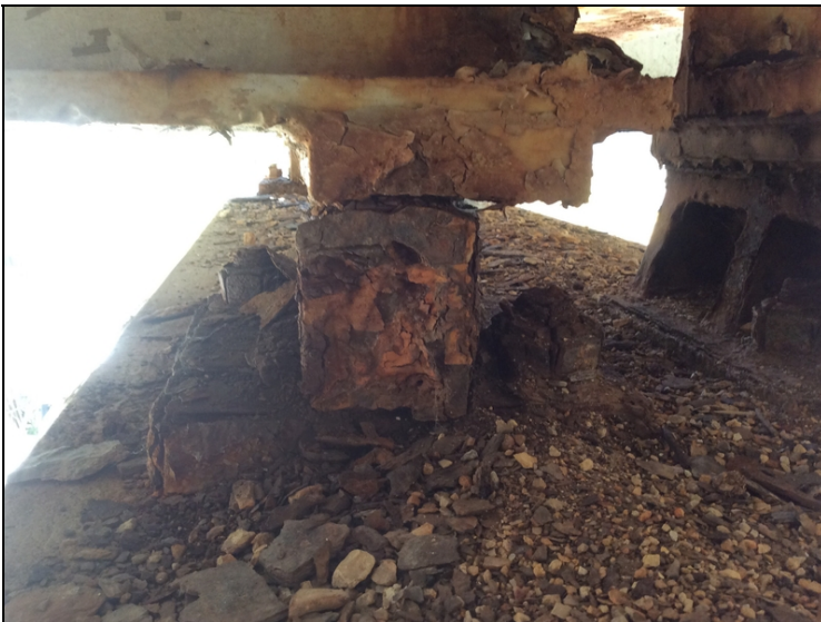
Bent #5, bearing #2-Out of position.
