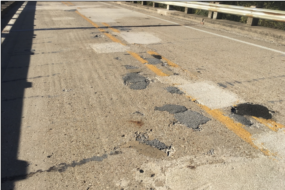
Typical spalling and delamination in the deck near the patched areas.
