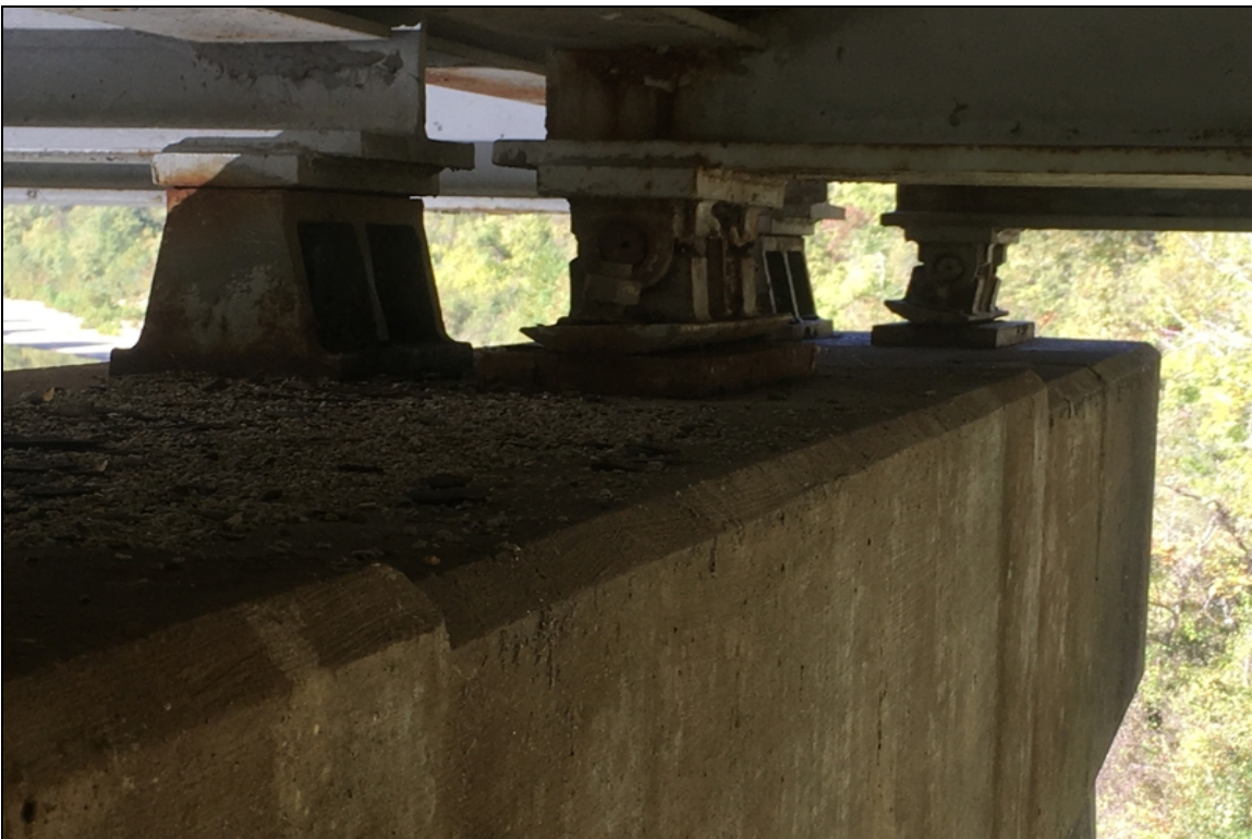
Bearing 5 tilt at the end of span #1.
