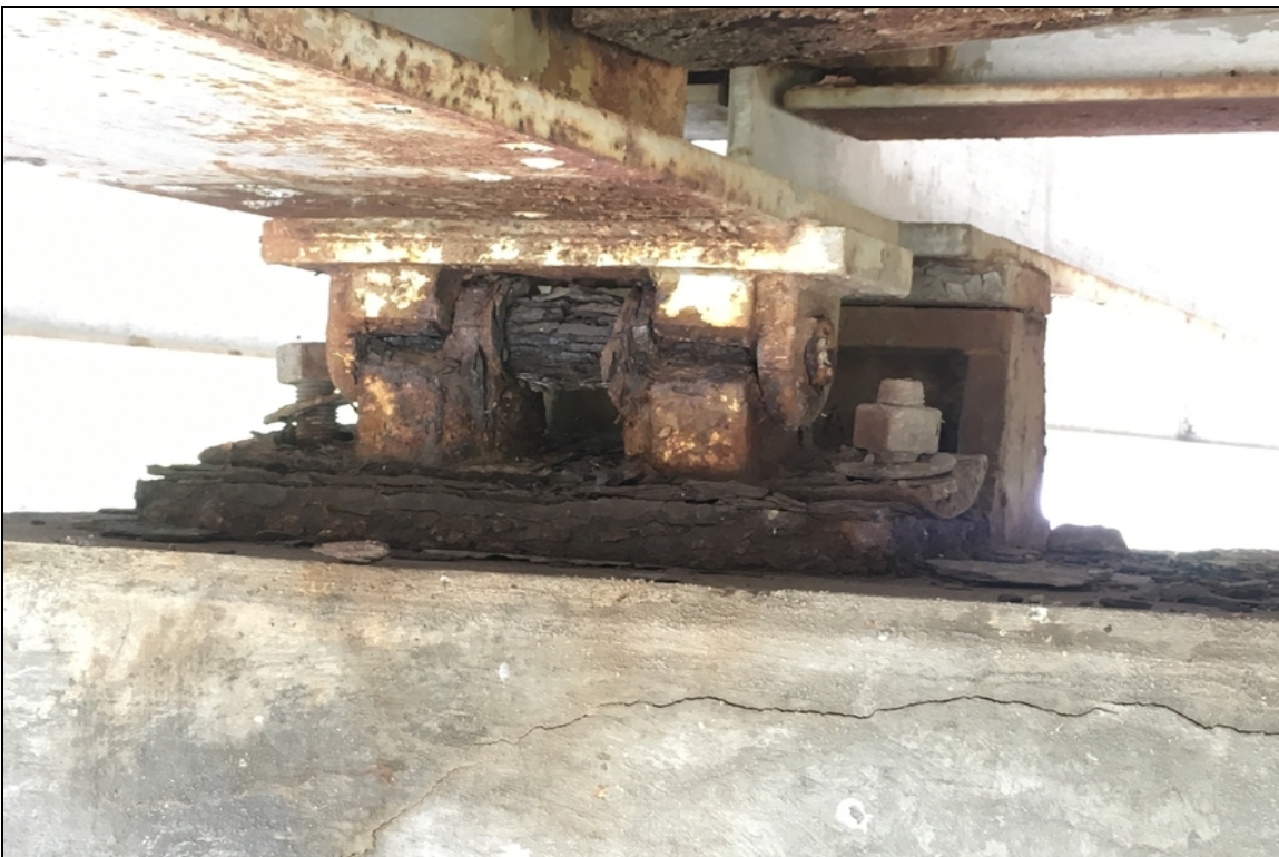
Movable bearing #2 condition over pier #3. Typical also of bearings #3,4 at the same location.
