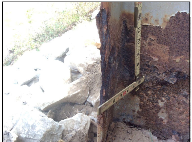
Bent #5, pile #4-Section loss.
