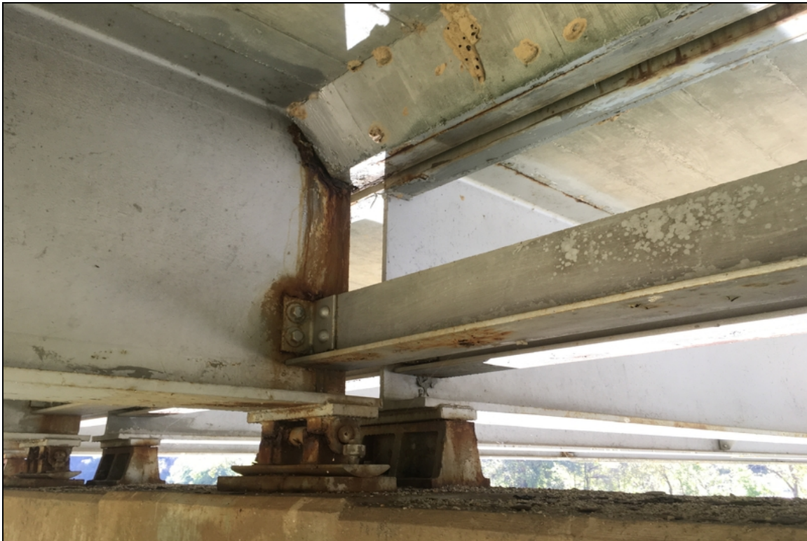
Beam end and bearing corrosion at the end of span #1.
