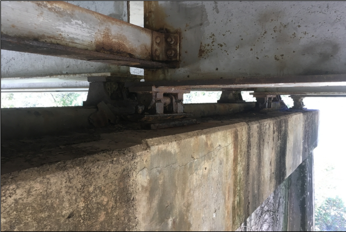
Pier #4 bearing condition. Showing corrosion that has been needle scaled and section loss.
