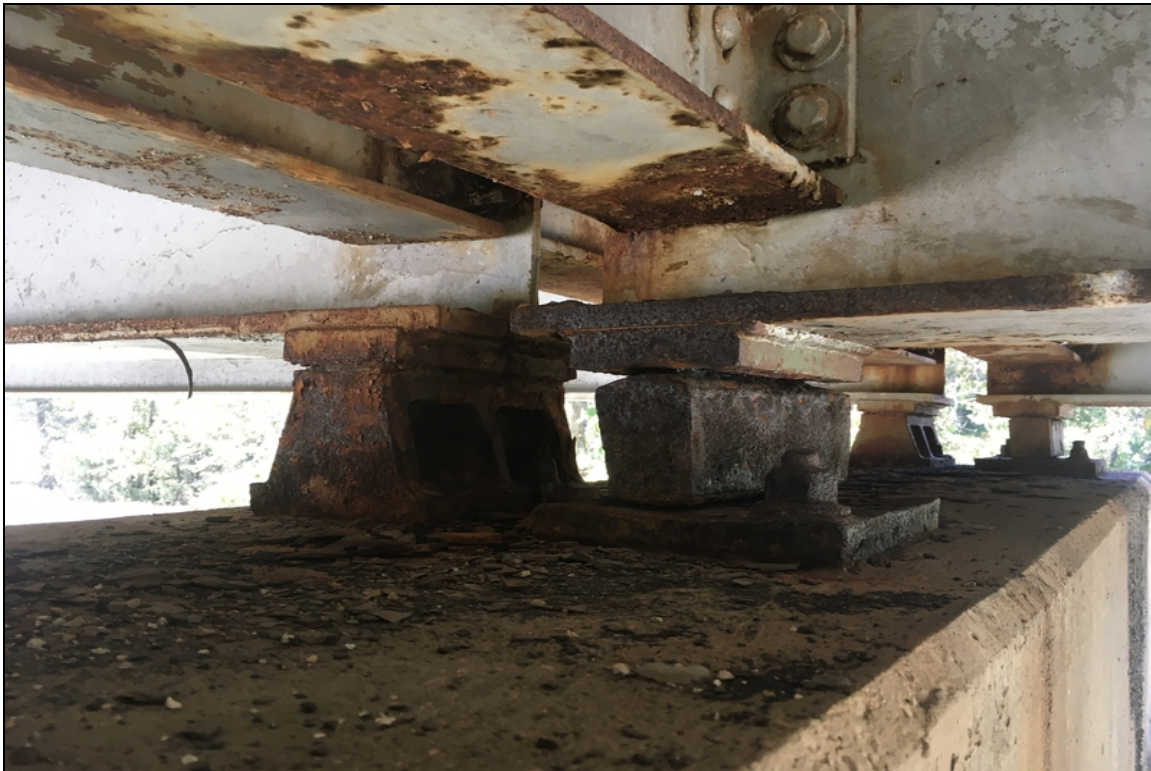
Section loss on movable bearing #4 over steel bent #4.
