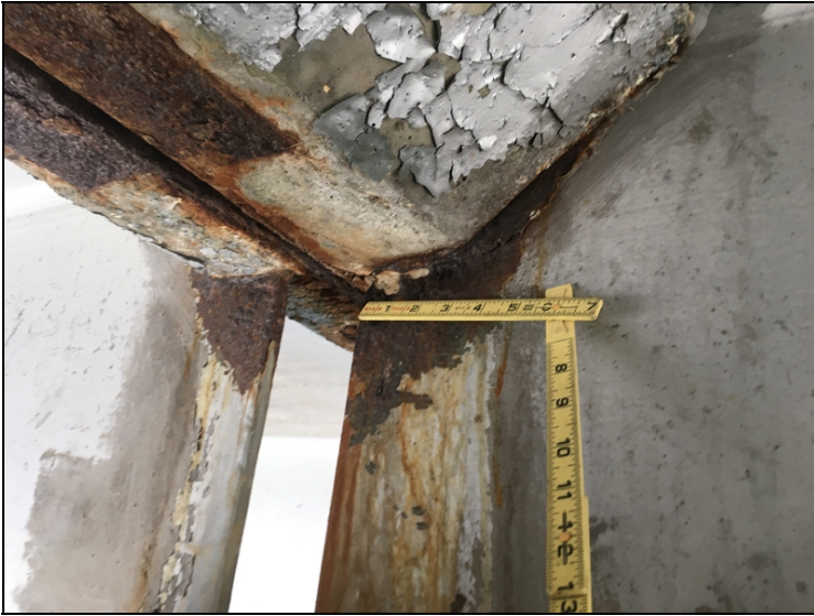
2" rust hole in the upper portion of the web at the end of beam #3 in span #5.
