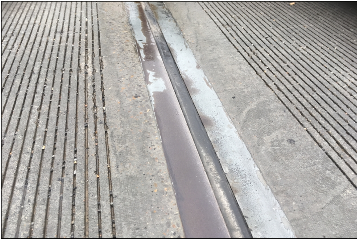
Adhesion loss at the pier #7 seal.
