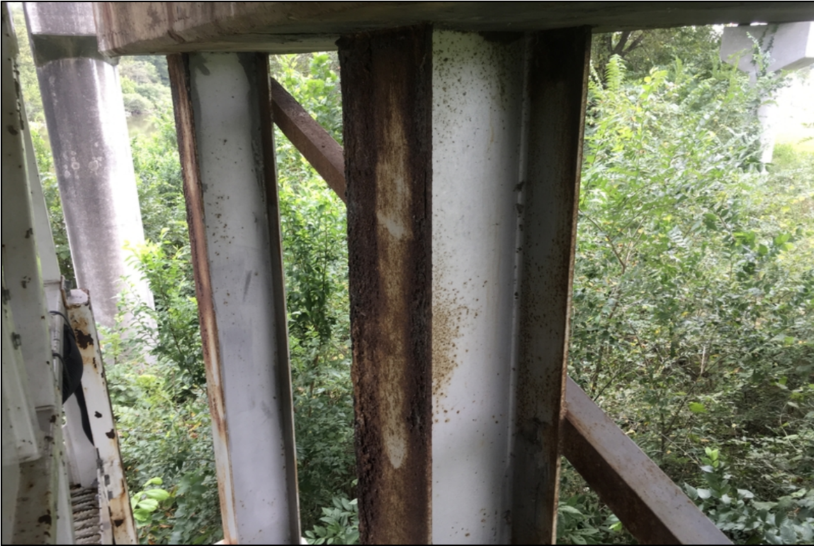
Corrosion with minor section loss at the tops of piles #1,2 at pile bent #4
