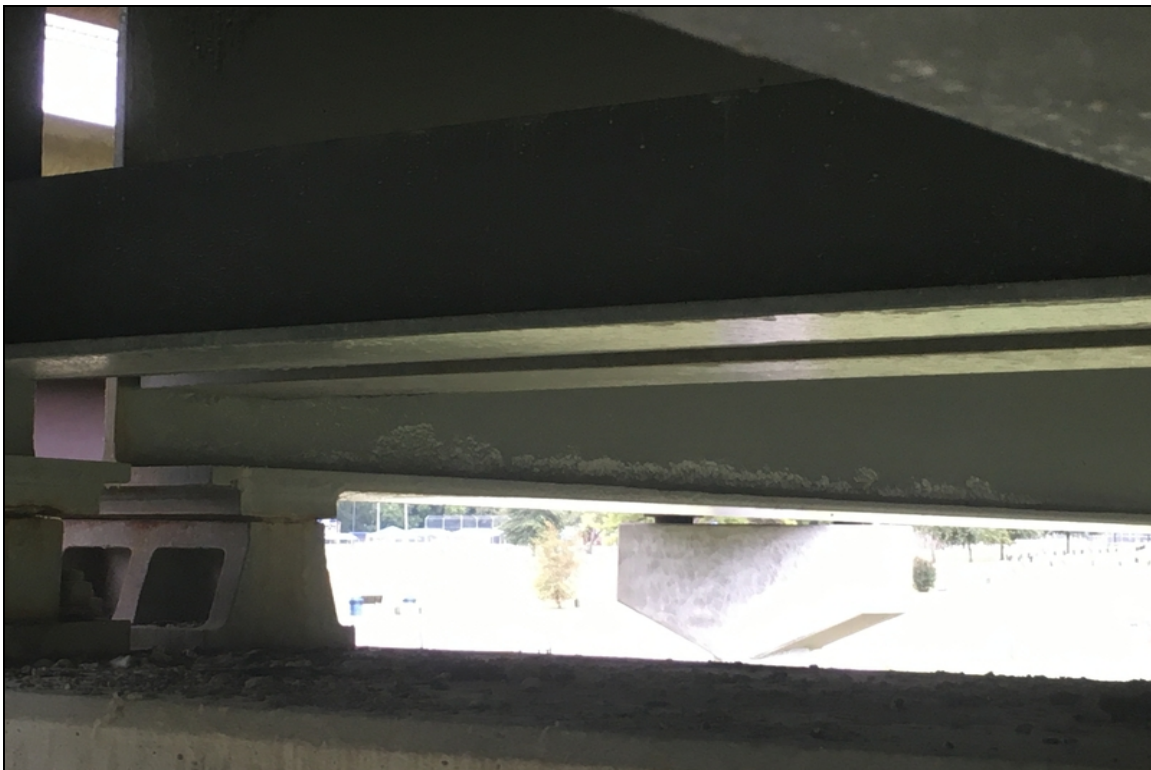
Shallow pitting on the interior lower web of beam #1 in span #6.
