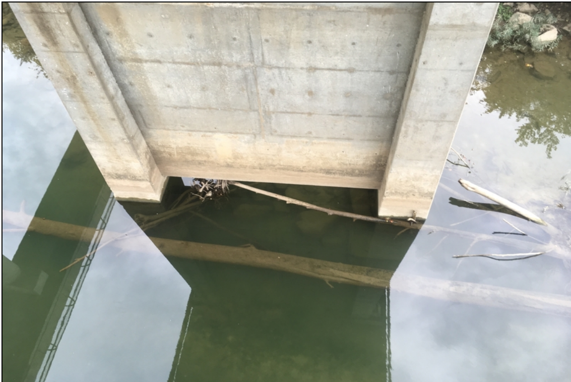
Footings exposed at pier #3.
