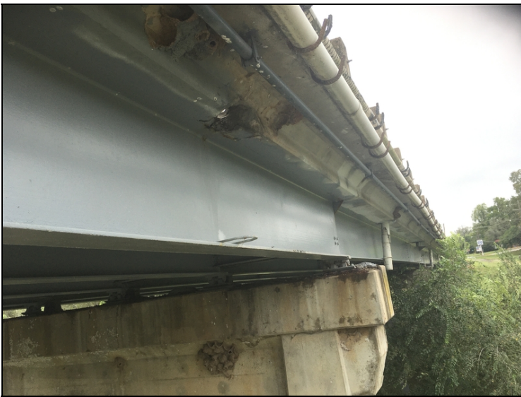
Missing drain pipe on the right side of span #3.
