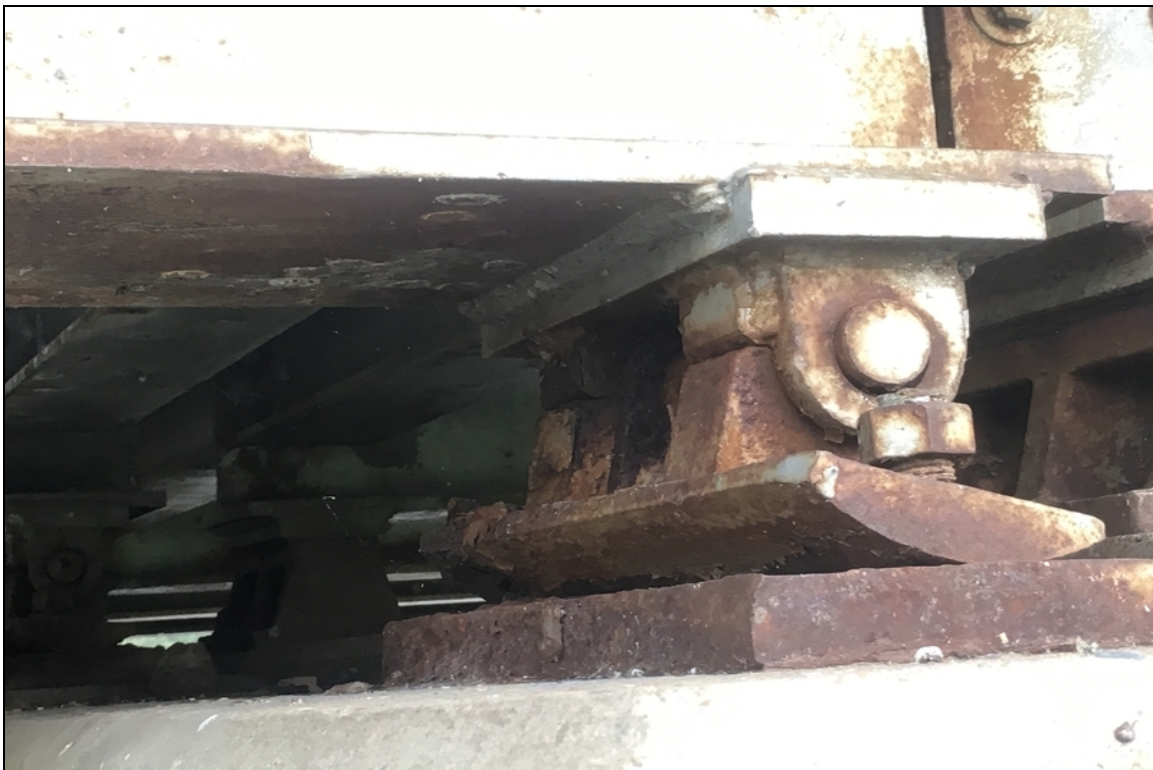
Tilted bearings at the span #3 side of pier #3. # 1,2,4,5 are tilted #3 is not.
