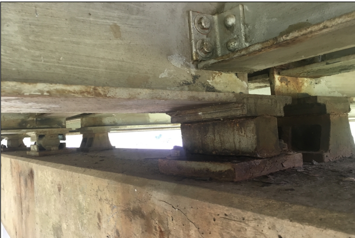
Bearing condition at pile bent #6.
