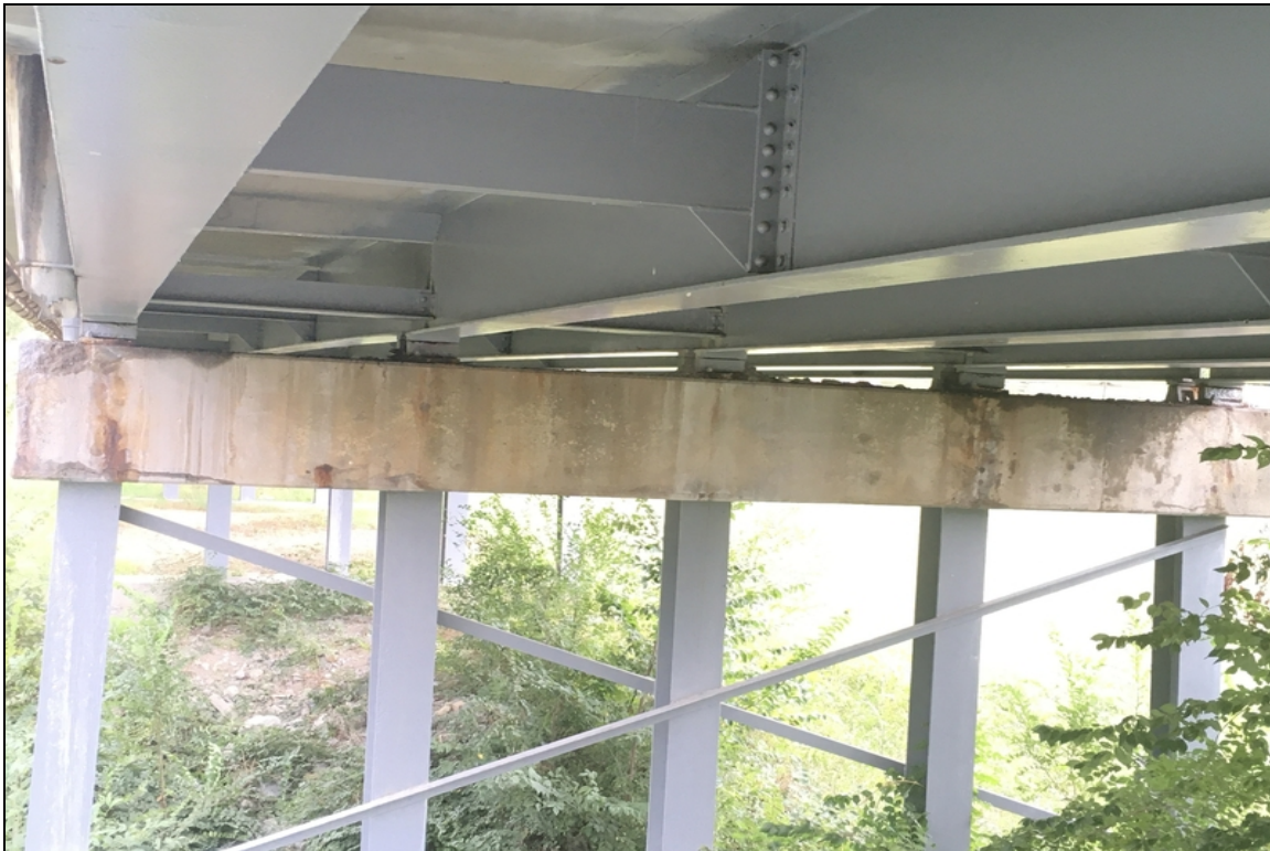
Bent #4 bearing condition. Showing corrosion.
