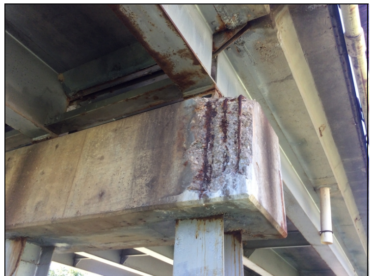
Spall with rebar exposed at left cap end of bent #3
