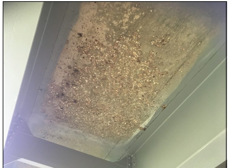
5' by 5' area of shallow delamination in the undersurface of span 8 in bay #4.
