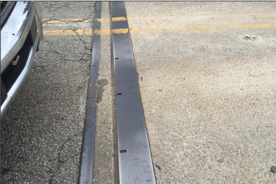
Assembly joint at abutment #1.
