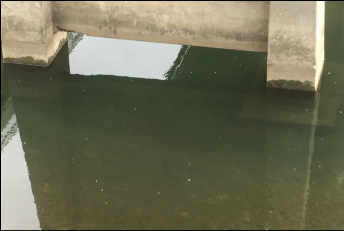
Exposed footings at bent #2.
