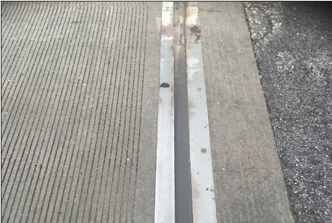
Abutment #1 joint seal condition. New. No deficiencies noted.
