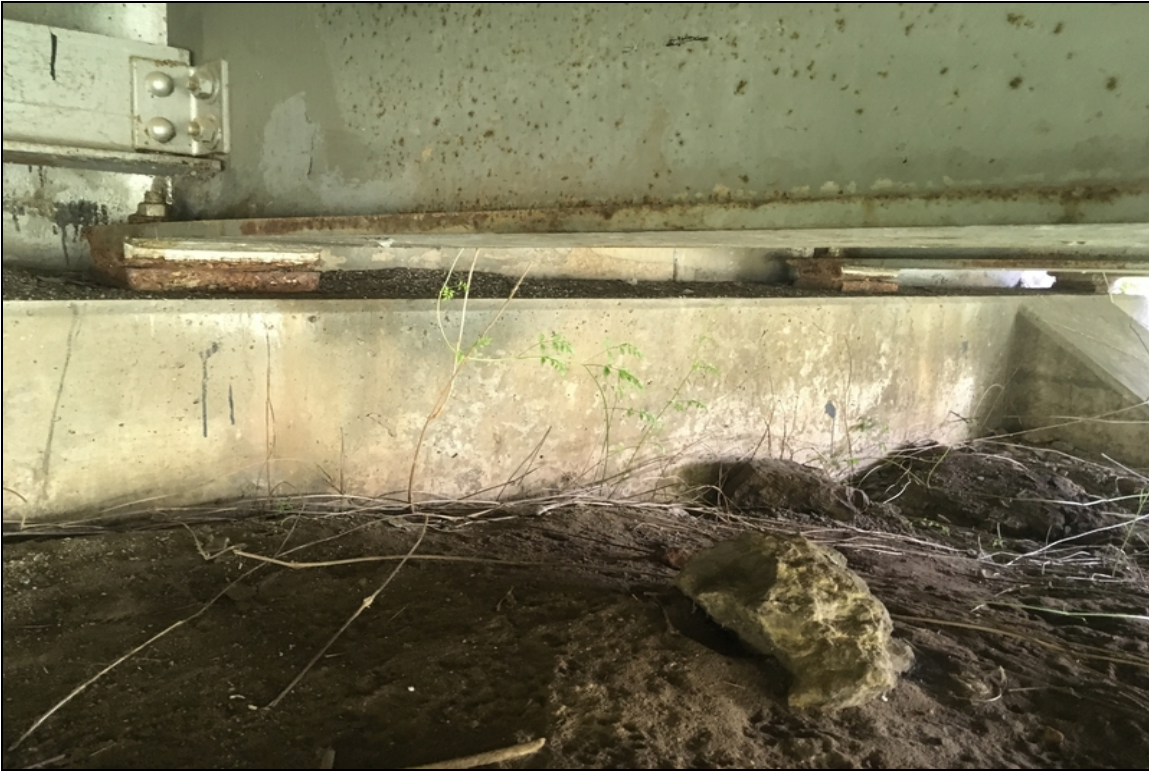
Bearing condition at abutment #2.
