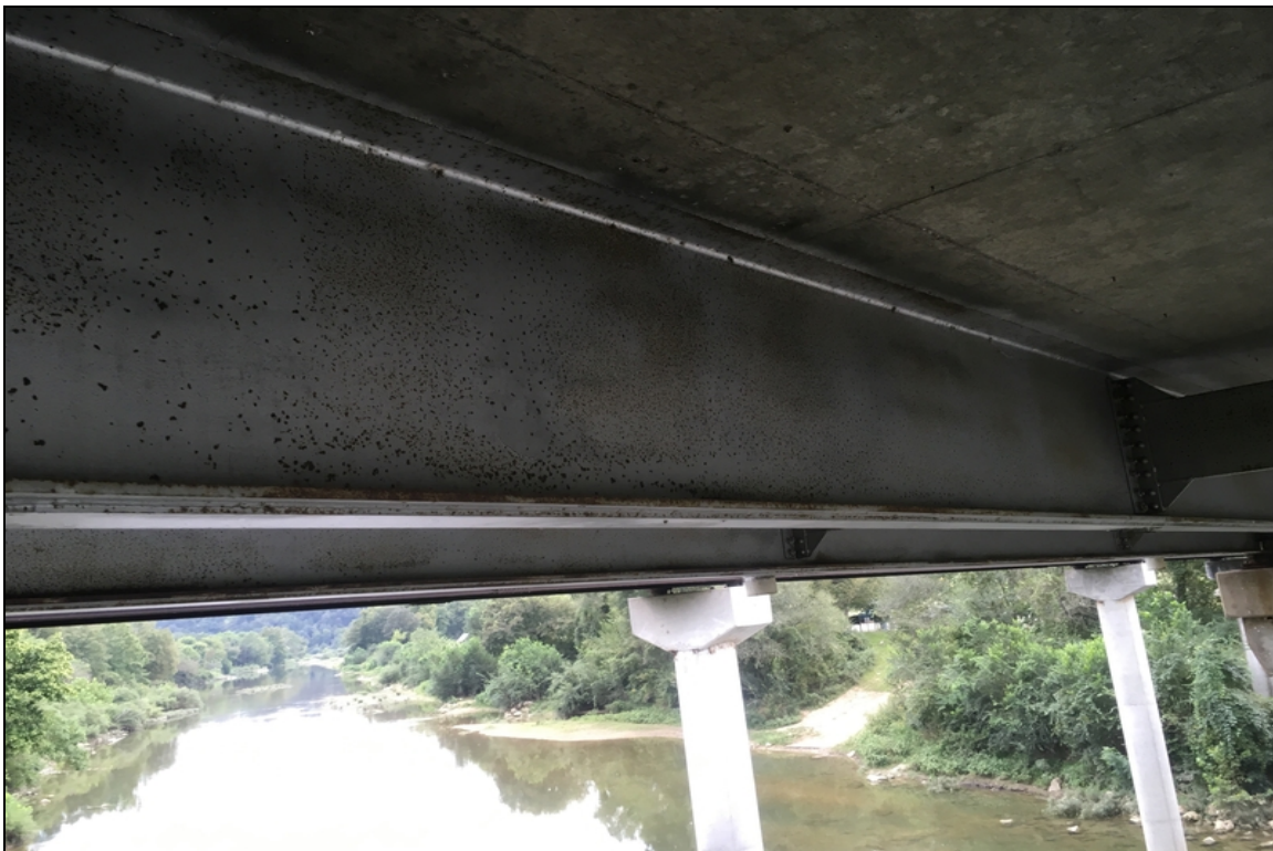
Large areas of pin point rusting in span #2.
