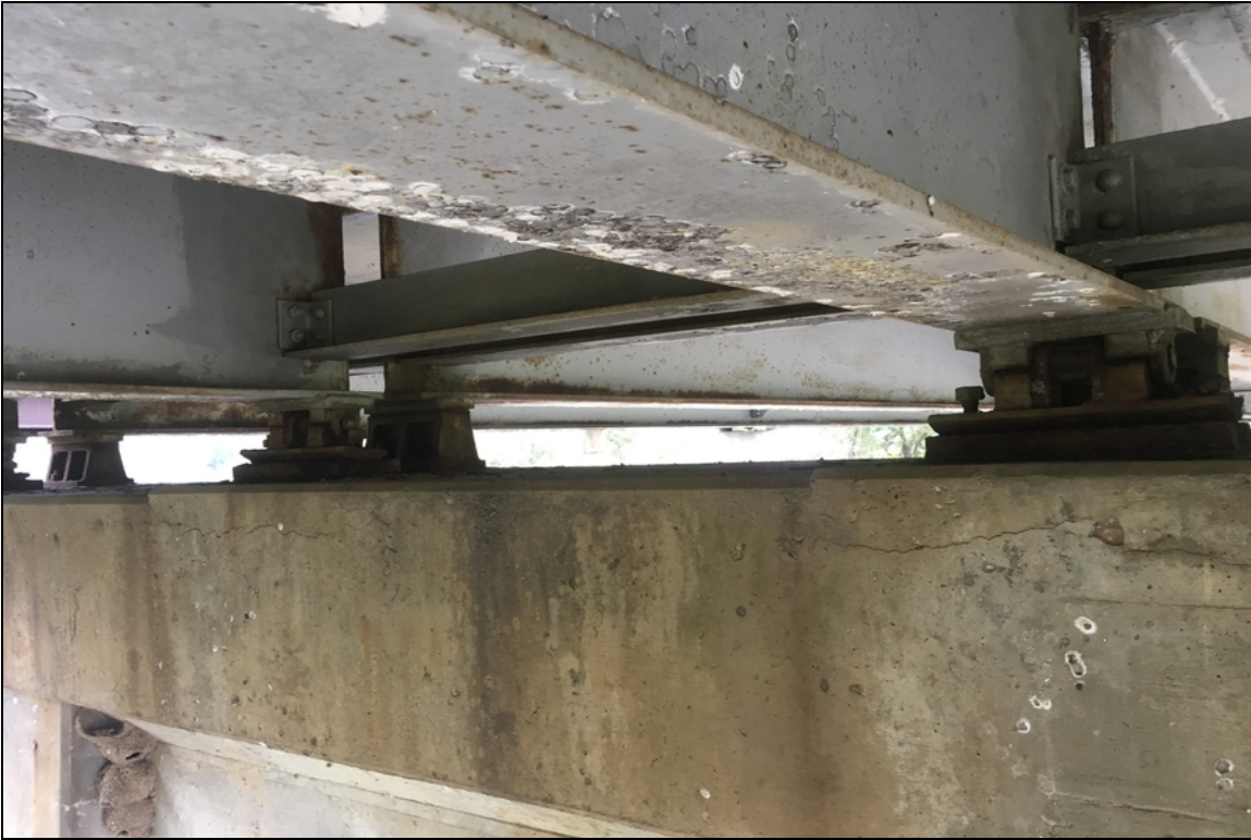
Bearing condition at pier #2. Note the delamination on the pier cap.
