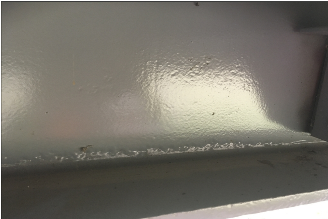
9' of shallow section loss with arrested corrosion on the interior lower web of beam #1 in span #5
