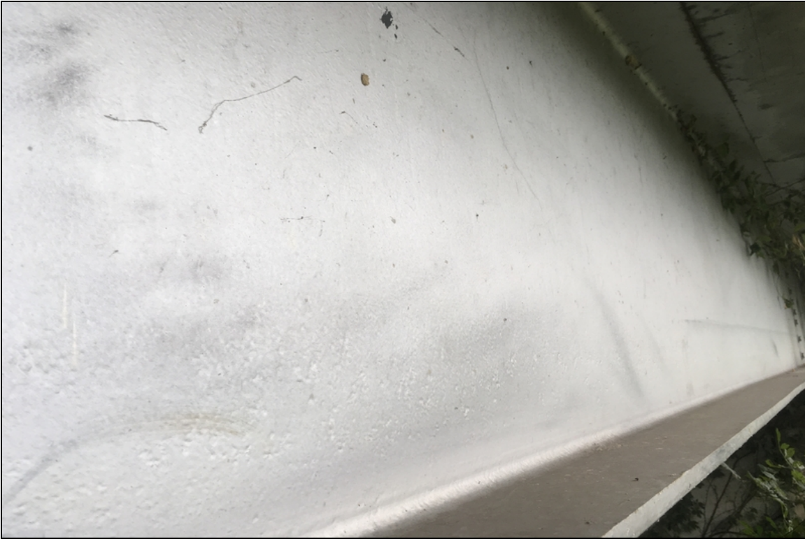
Typical beam paint condition of the exterior of beam #5.
