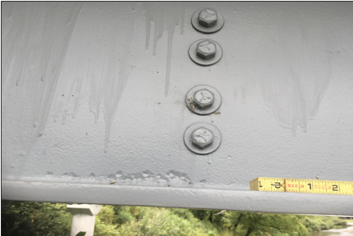
1' area of arrested corrosion on the exterior lower web of beam 5 in span #2.
