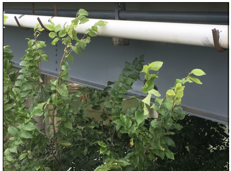
Partially missing drain pipe on the right side of span #4.
