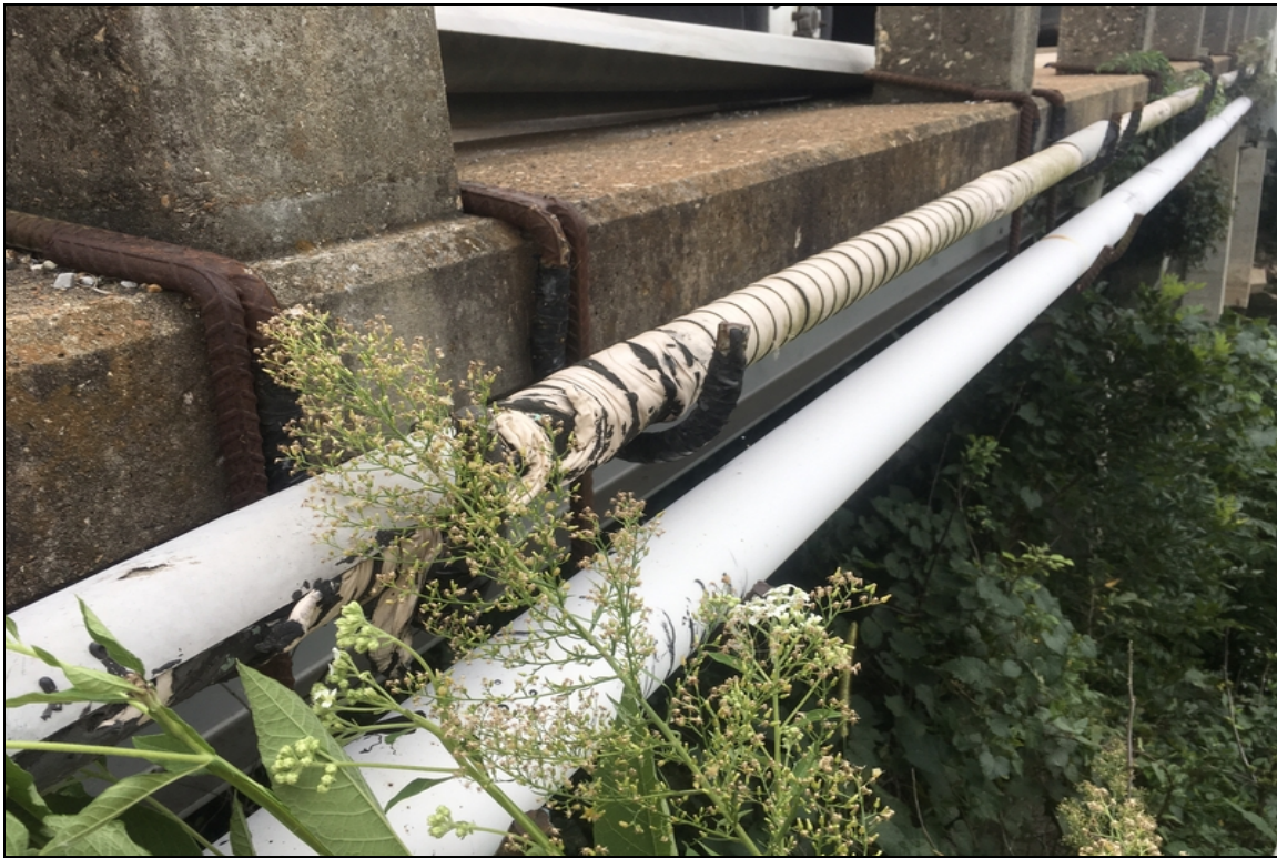
Utility attachment on the right side of the structure.
