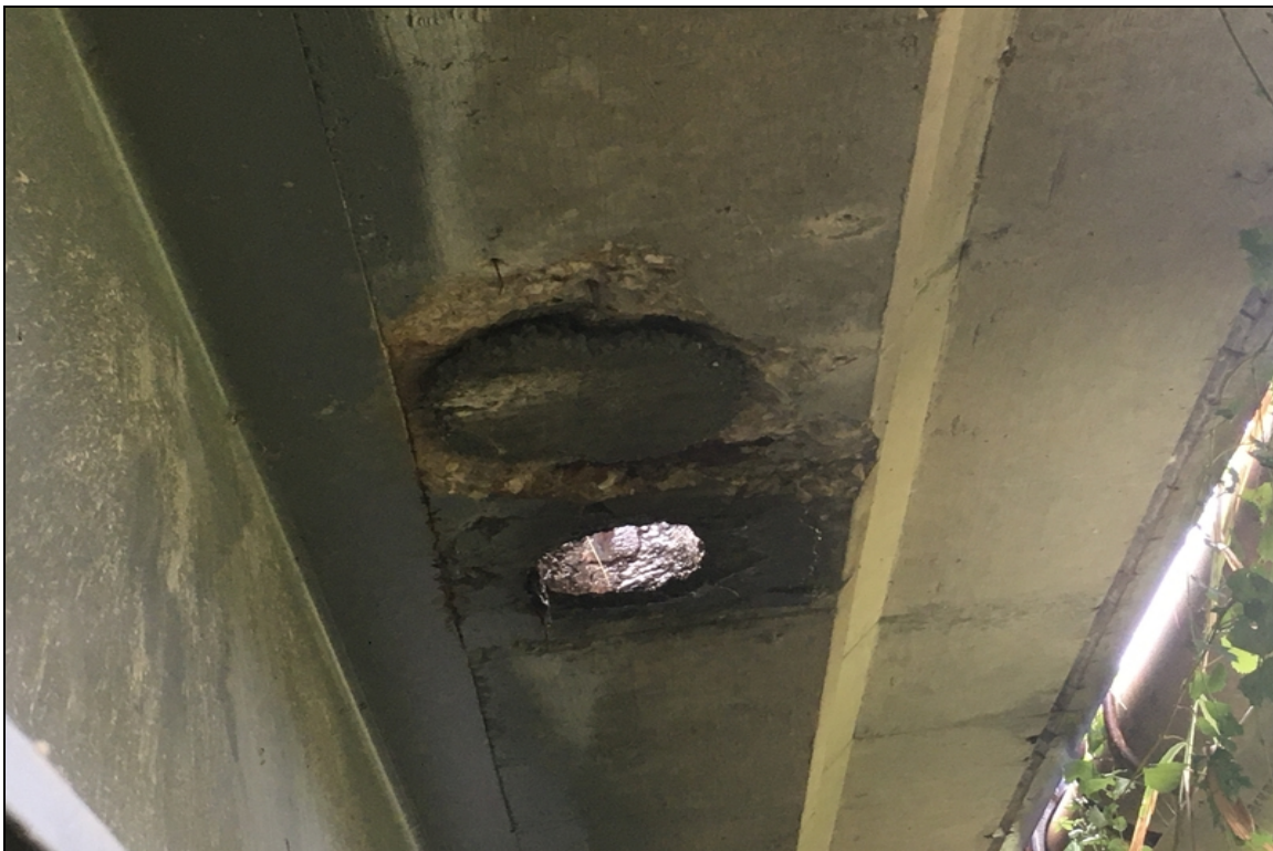
Spalling with exposed rebar at the left drain of span #1.
