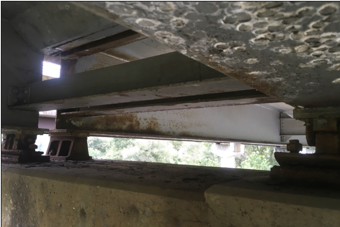
Beam end corrosion at the beginning of span #3.
