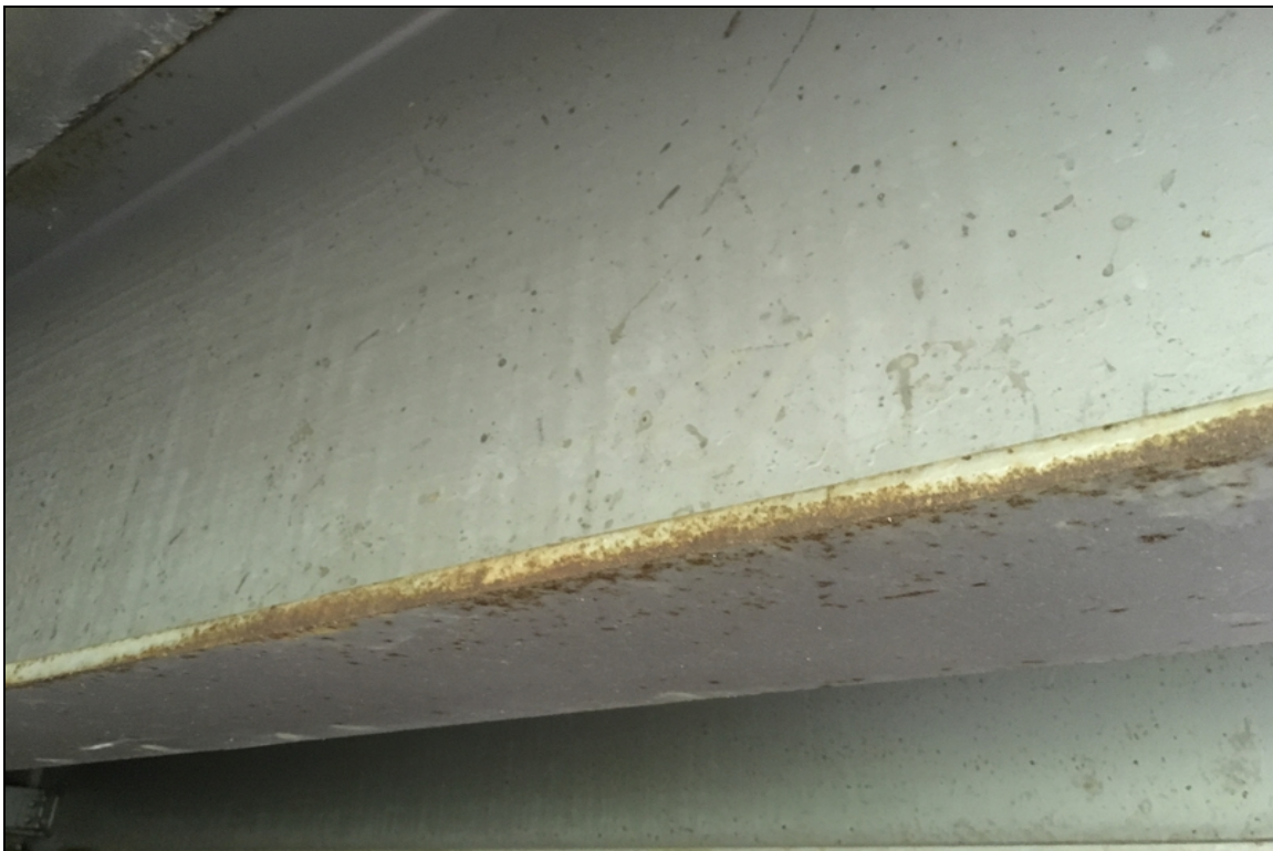
Pin point and general corrosion typical of many locations.
