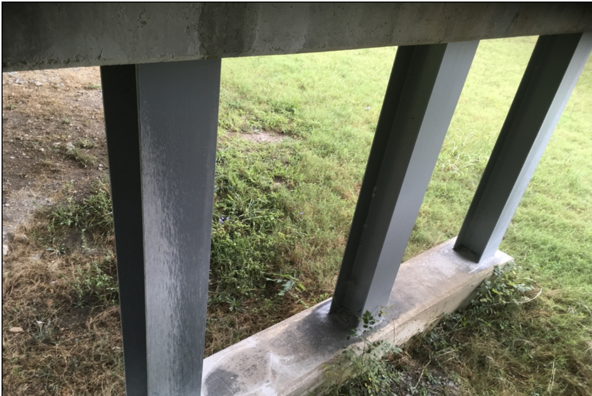
Repainted steel pile columns.
