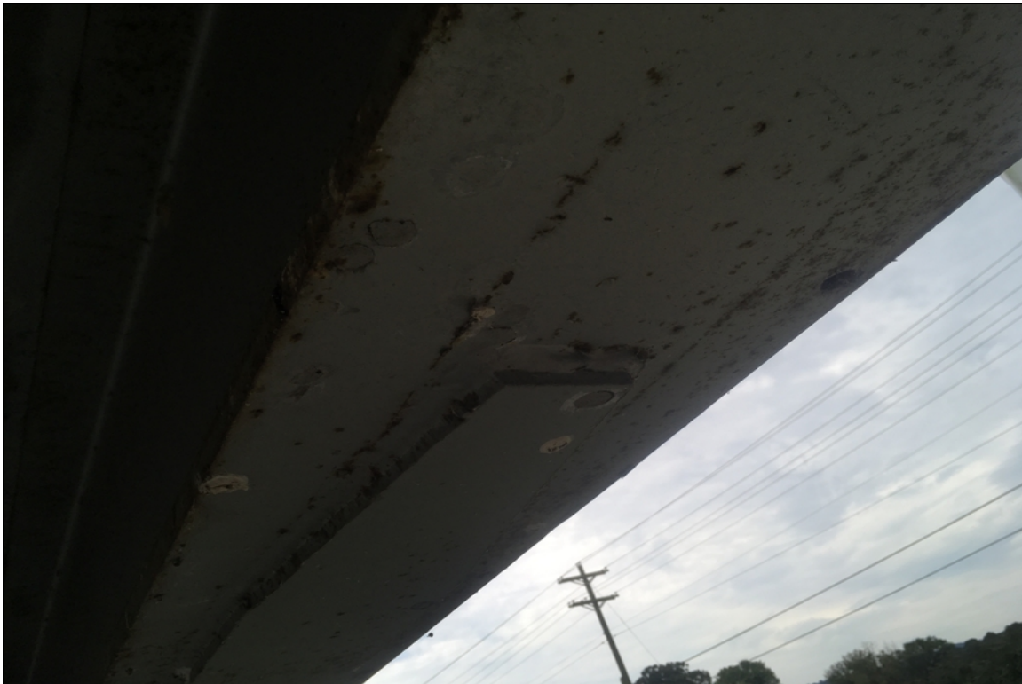
Longitudinal factory defect in the bottom flange of beam #5 in span #3 at the beginning of the cover plate.
