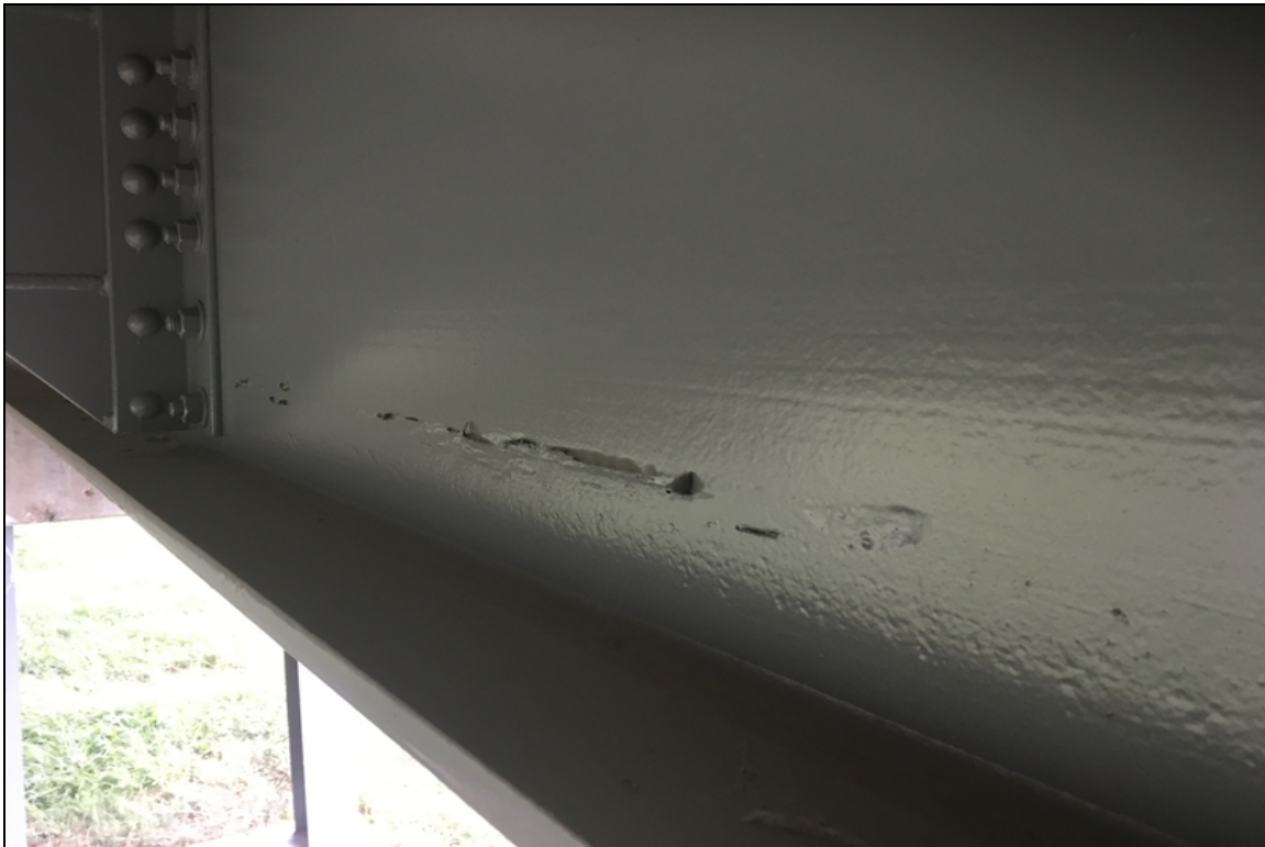
Superficial factory defect in the web of beam #4 in span #6.
