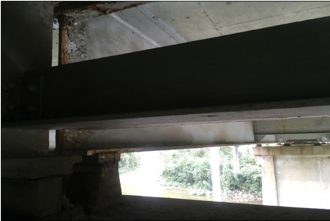
Corrosion on the bottom flange and beam ends in span #2.
