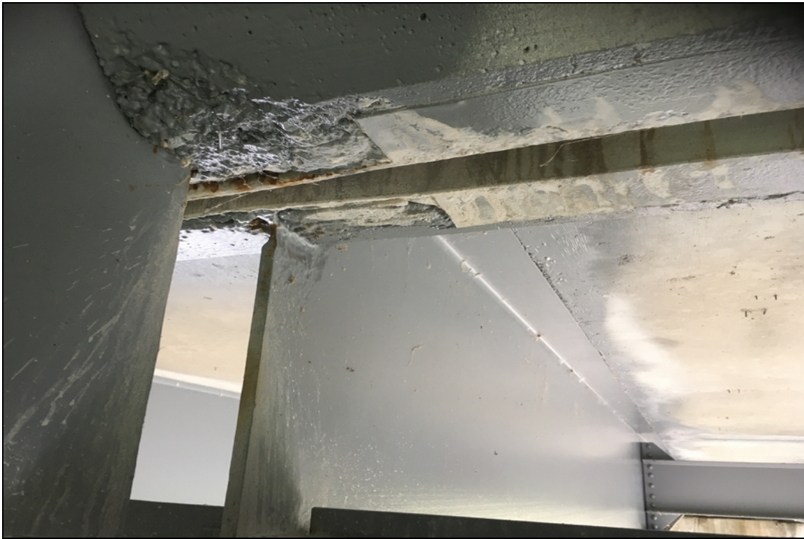
Small areas of section loss and arrested corrosion on the upper web of the span #3 beams.
