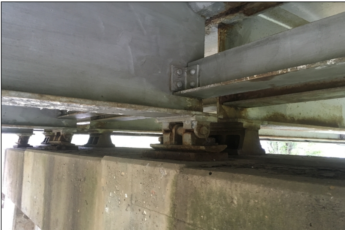
Bearing condition at pier #3.
