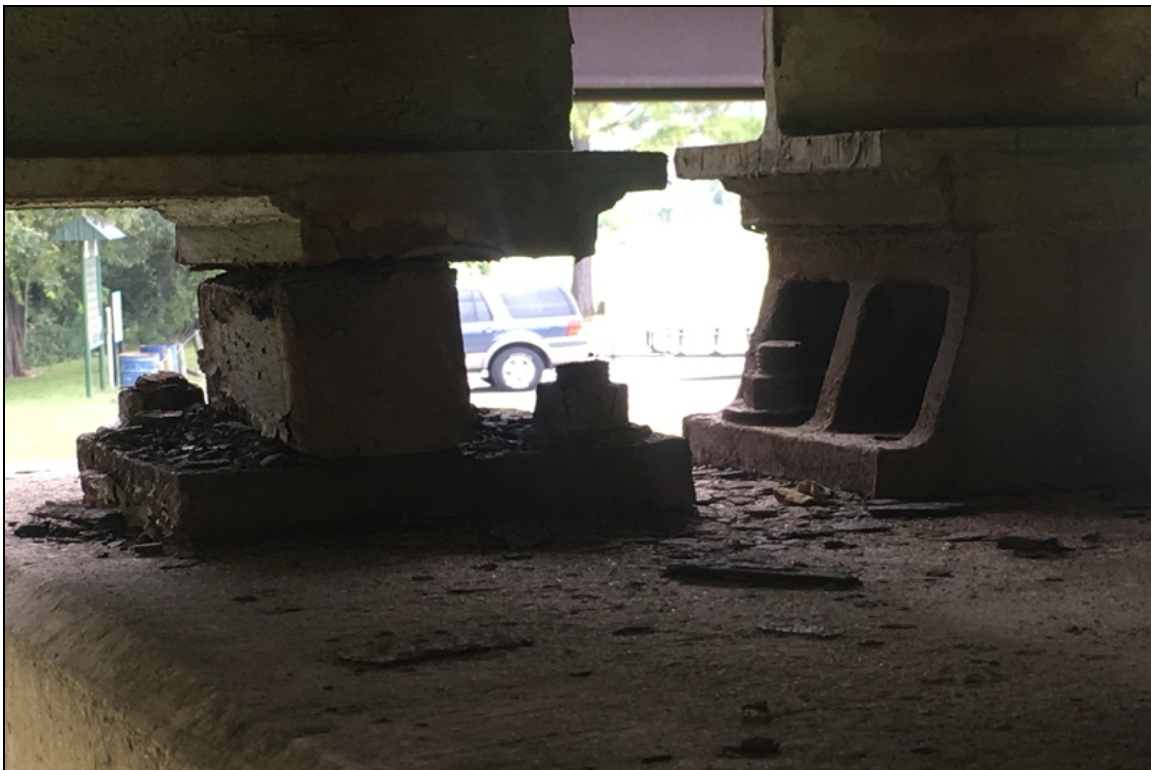
Bearing #1 and #5 are no longer centered beneath the sole plate at bent #6.
