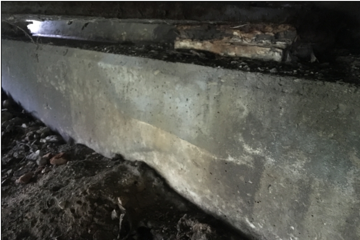
Bearing condition at abutment #1. Typical of all 5 at this location.
