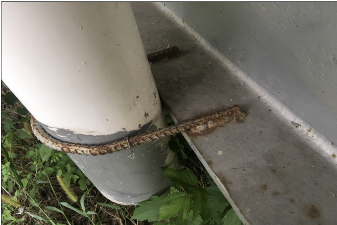
Typical welded detail of the drain extensions on the bottom flange of the fascia beams.
