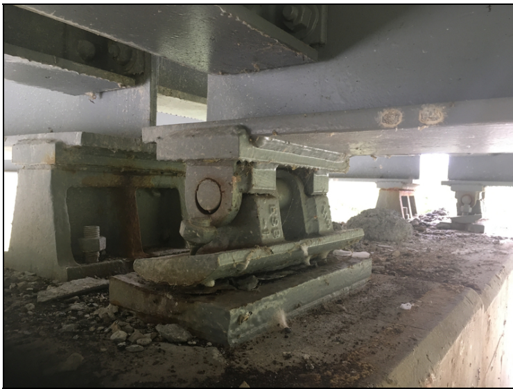
Section loss on the anchor bolt studs at pier #2.
