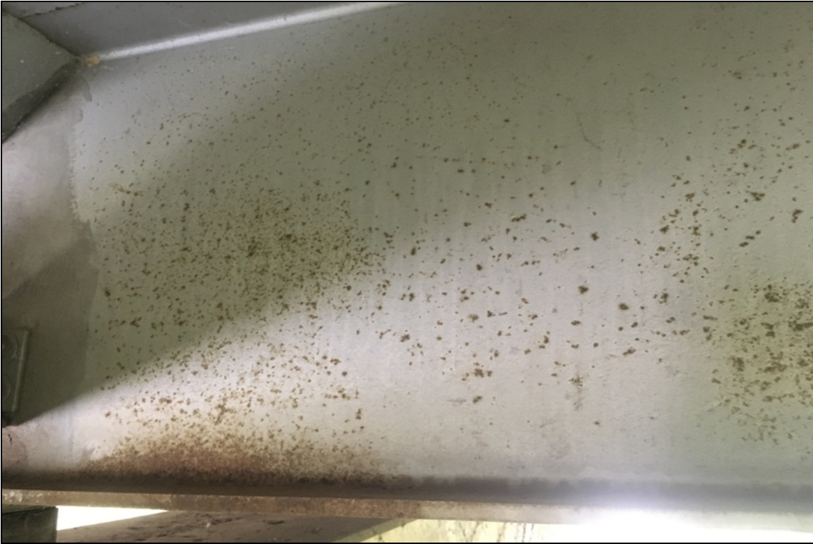
Pin point rusting at the beam ends in span #1.
