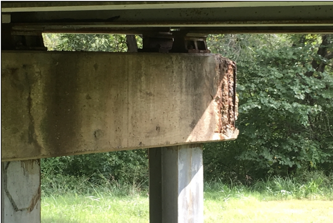
Spalling with rebar exposed on the left cap end of bent #6.
