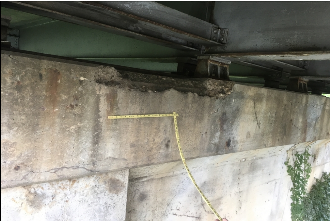
Spalling with rebar exposed on the span #2 side of the pier #1 cap. Note the delamination also.
