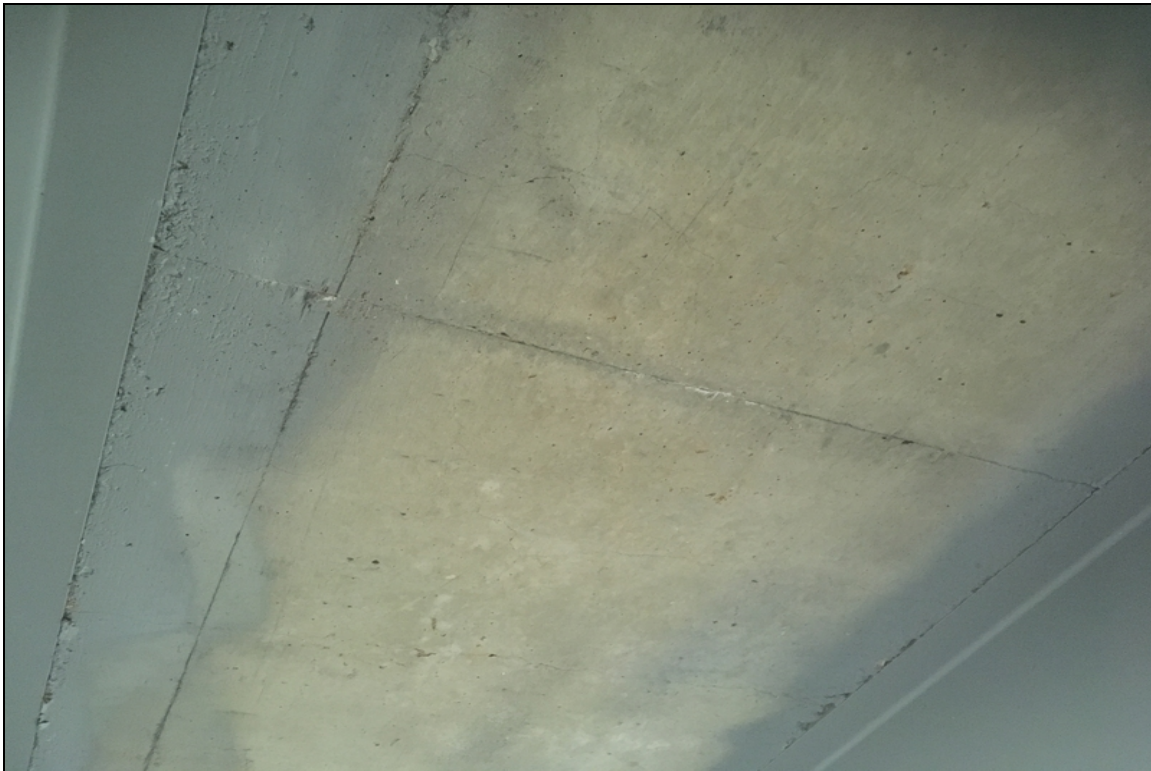
Deck cracking in the undersurface. Showing cs2 efflorescence.
