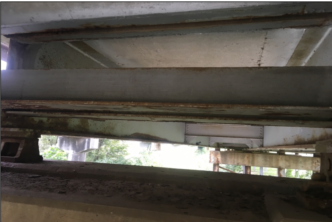
Beam #1 at the beginning of span #4 showing heavy corrosion on the bottom flange and lower web.
