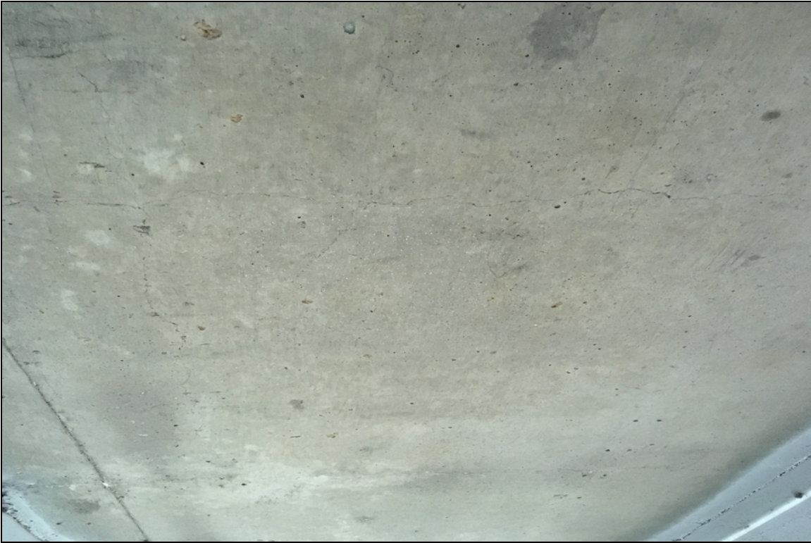
View of the deck undersurface. Showing transverse hairline cracking.
