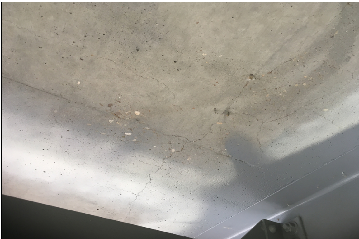
Deck cracking in the undersurface. Typical. 0.016" wide.
