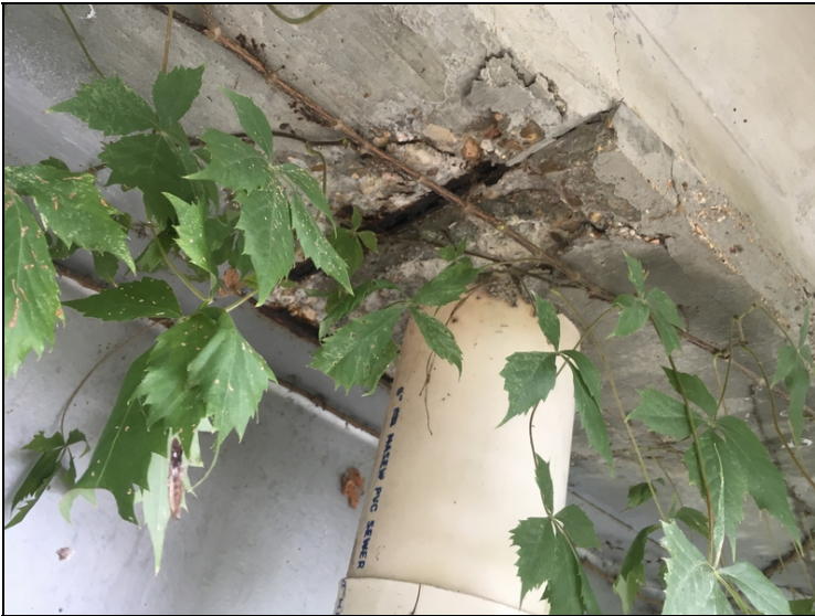
Spalling with rebar exposed in the right overhang of span #1.
