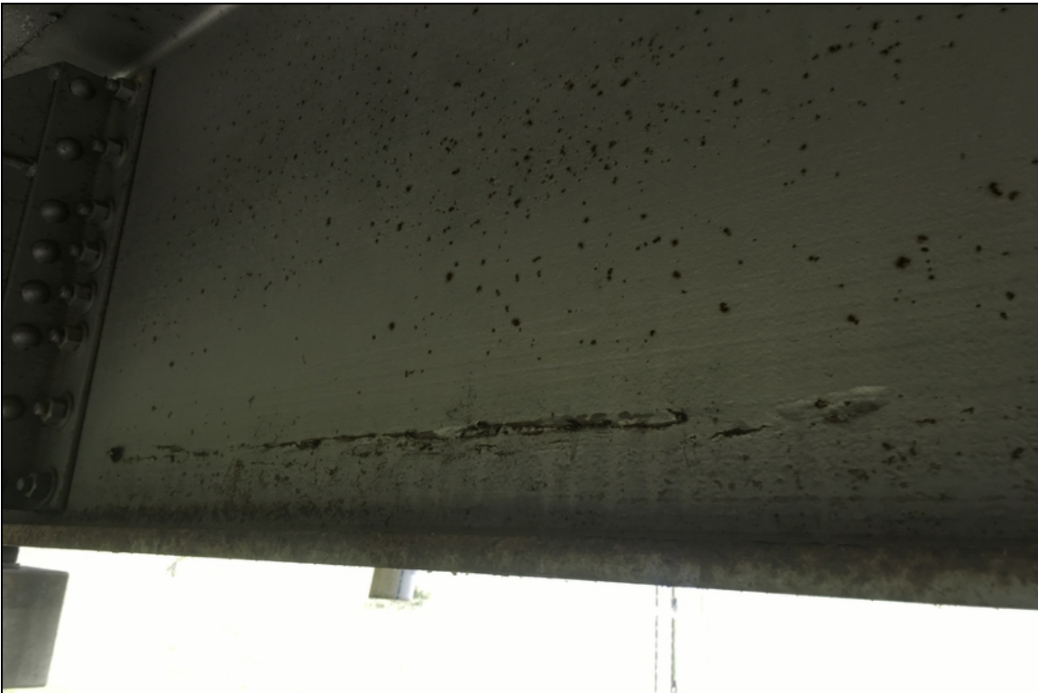
2' long longitudinal factory defect in the lower web of beam #4 in span #6.
