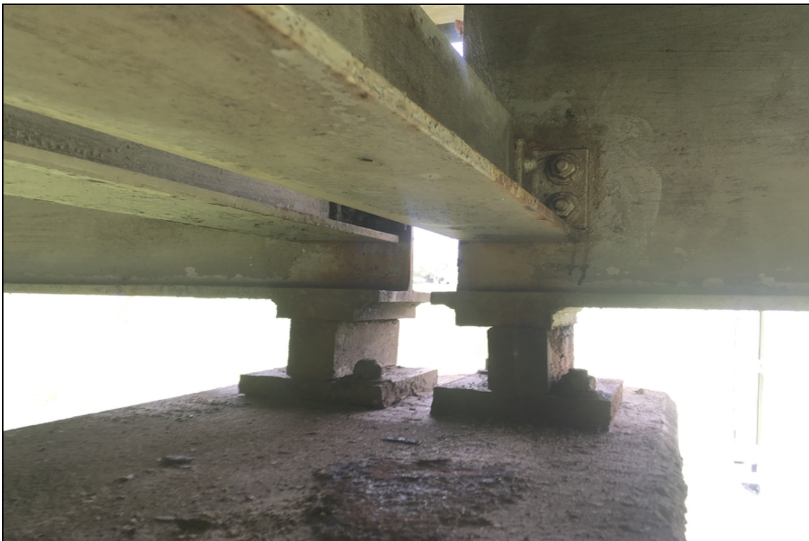
Bearing #5 at bent #7 is not centered beneath the sole plate.
