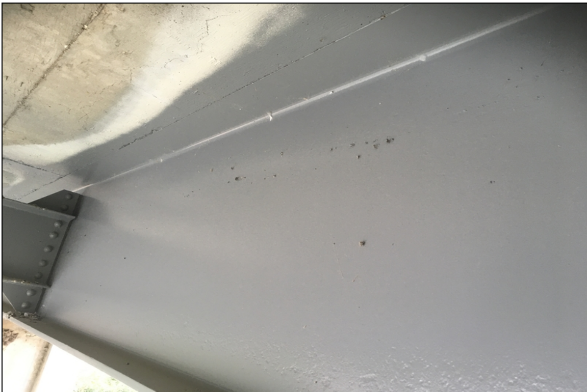
Factory defects in the web of beam #3 in span #3.
