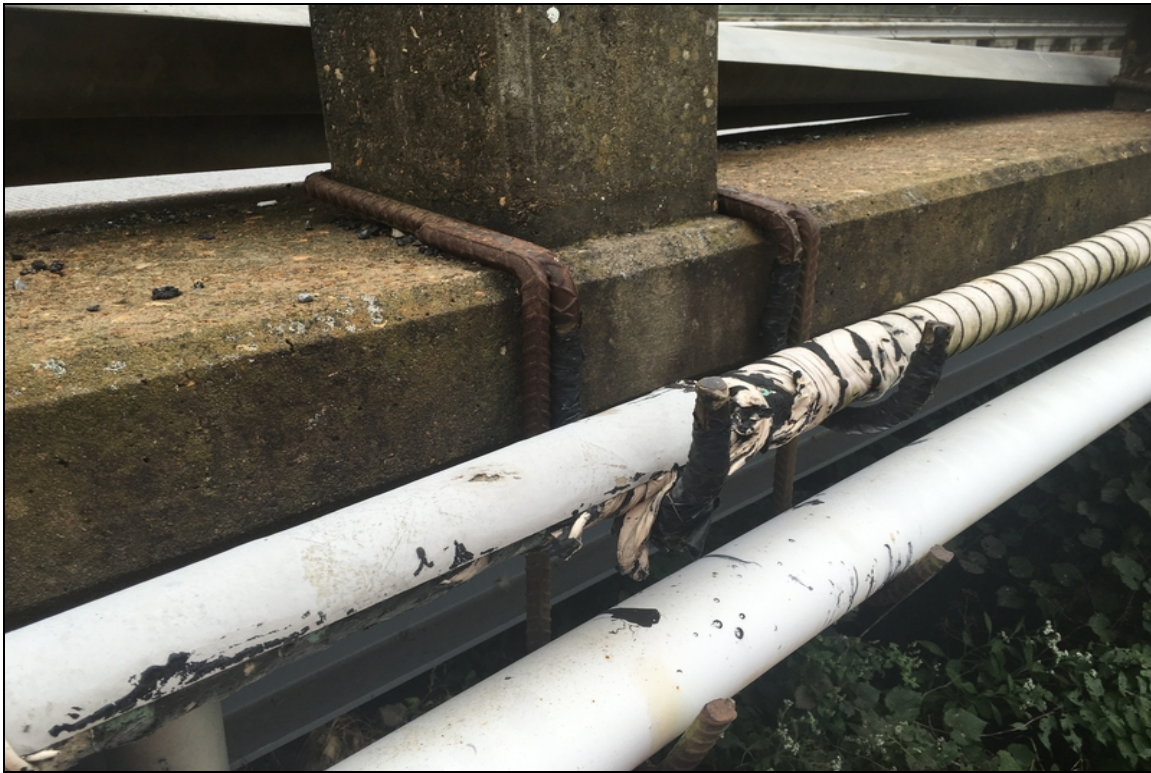
Typical utility attachment on the right side of the structure.
