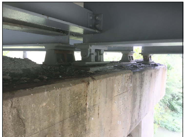
Missing anchor bolt studs at pier #3 movable bearings.
