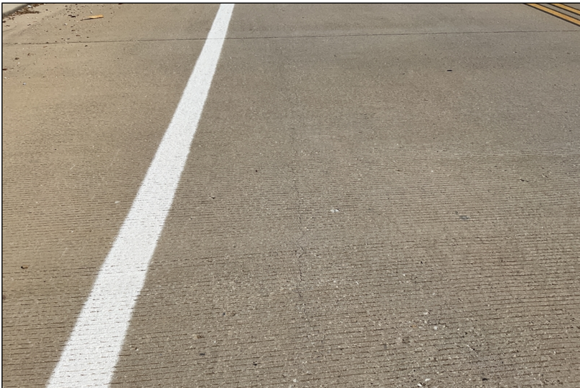
Typical full length longitudinal cracking.
