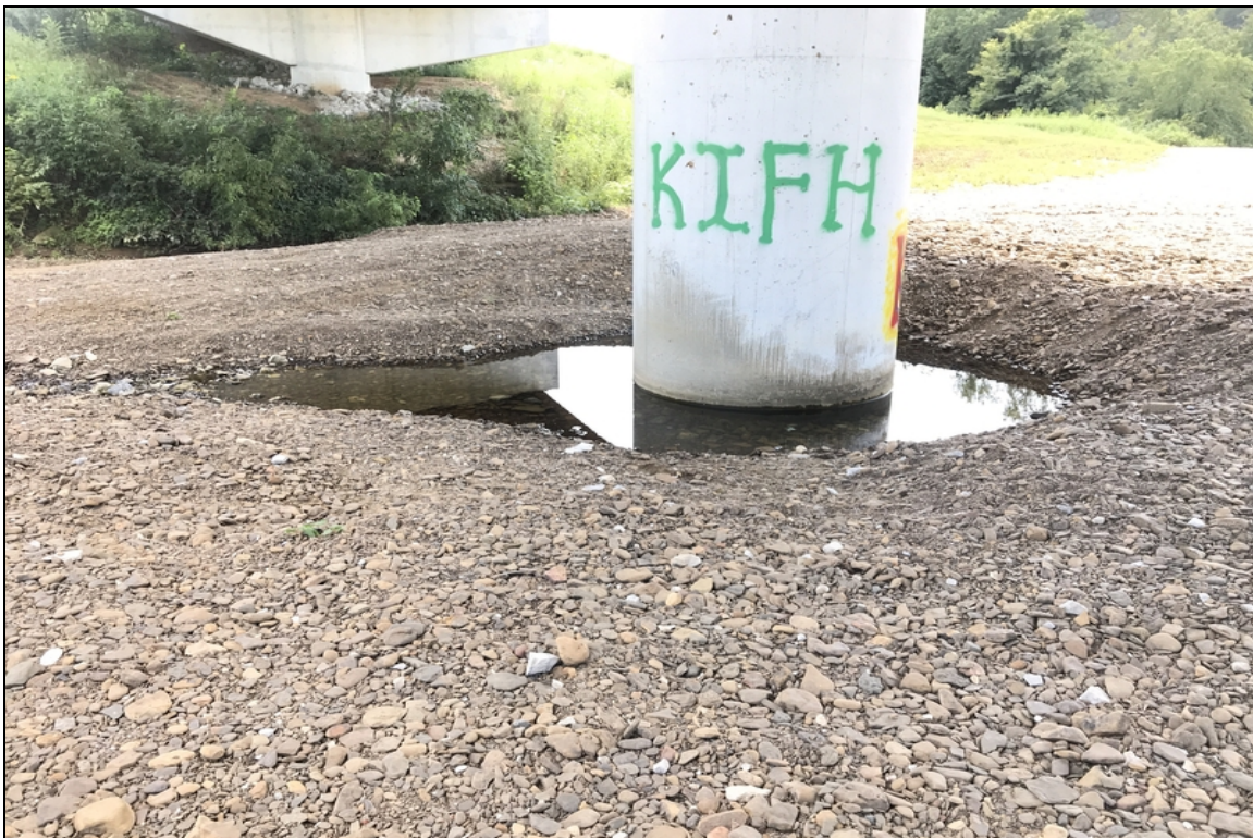
Typical scour hole around bents
