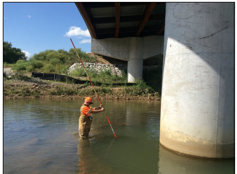
Bent #4 - localized scouring approximately 4'. photo #1.
