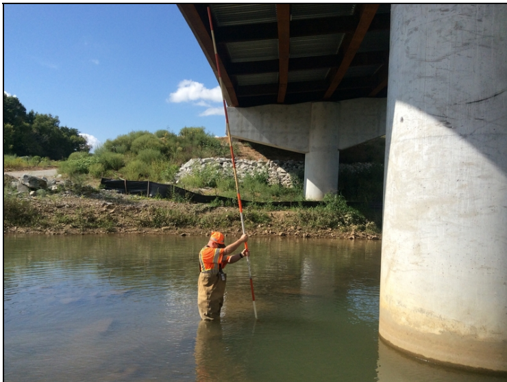
Bent #4 - localized scouring approximately 4'. photo #2.
