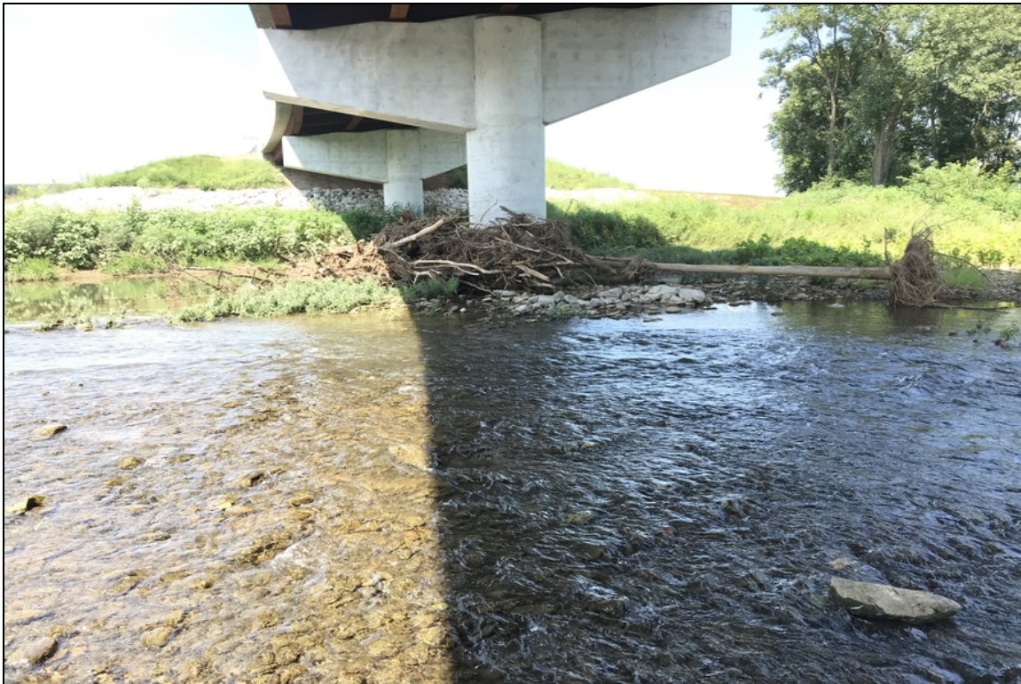
Drift accumulation against bent #4.
