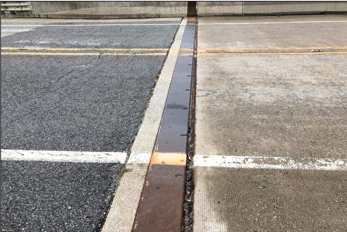
Abutment #1 joint assembly
