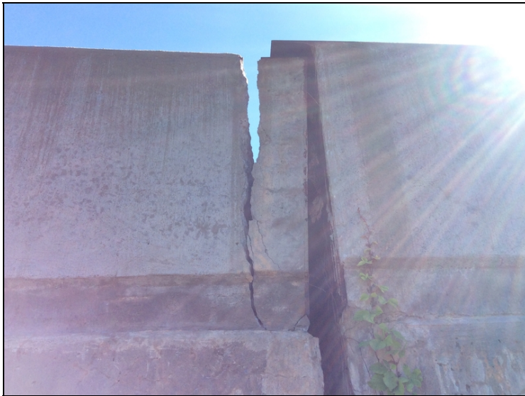
Span #1, Left side at abutment #1-Fractured concrete bridge railing.
