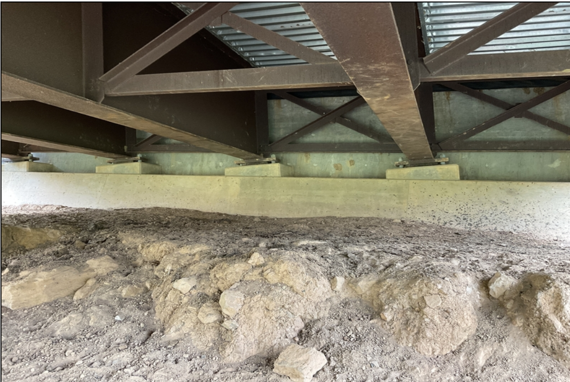
View of bearings at abutment #1
