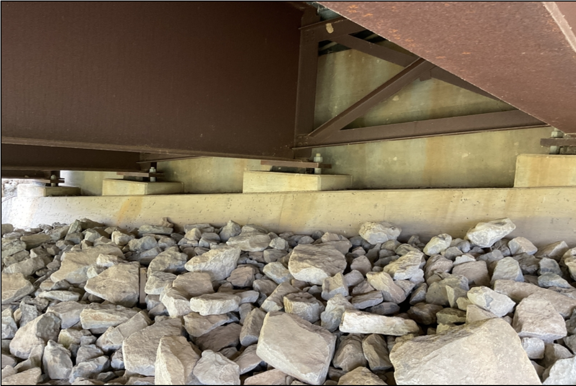
View of bearings at abutment #2.
