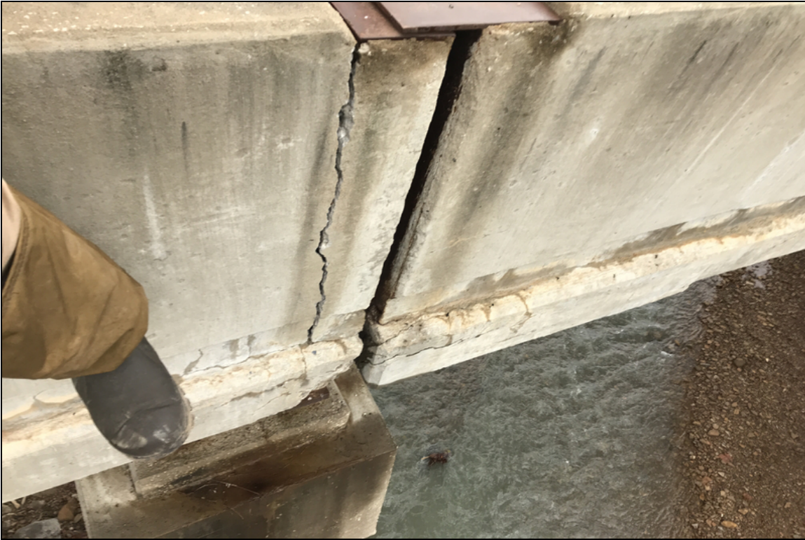
Left parapet over bent #4 complete fracture.
