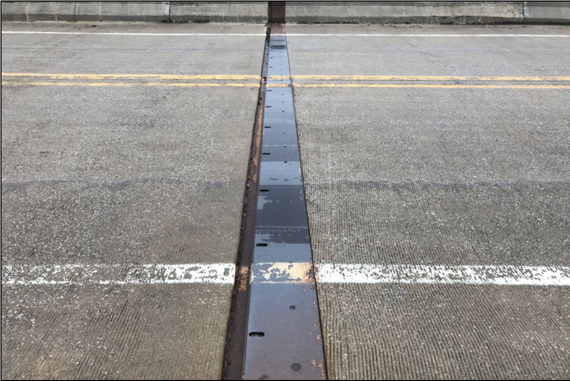
Joint assembly at bent #2
