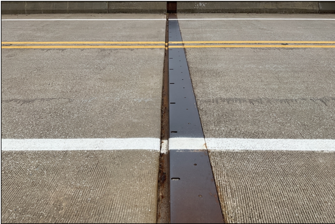
Bent #2 sliding joint.
