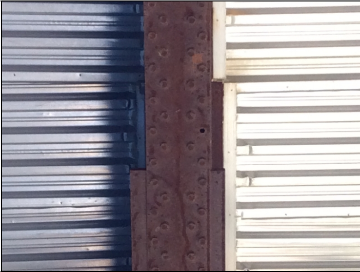
Span #1, Girder #3-Missing bolt in bottom flange splice plate.
