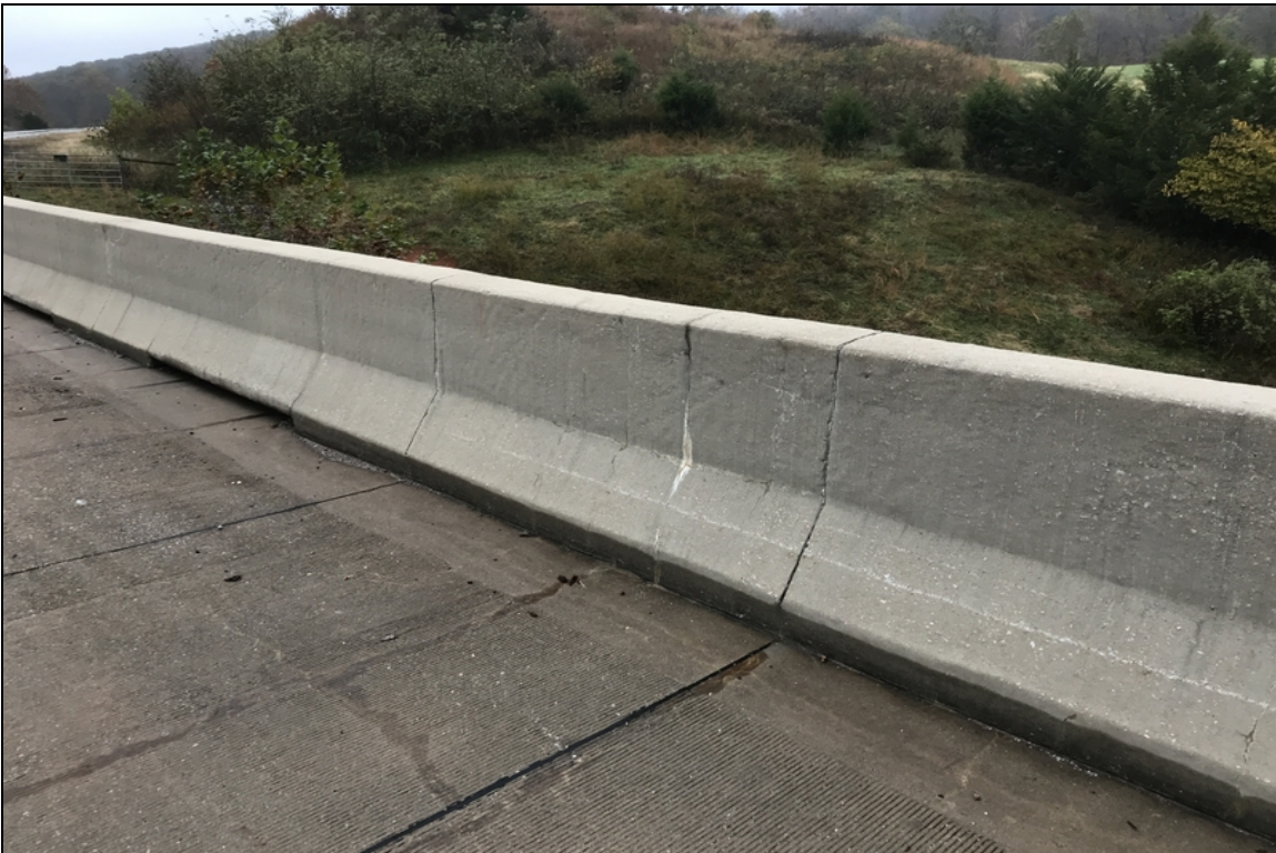
Typical cracking in parapet wall.
