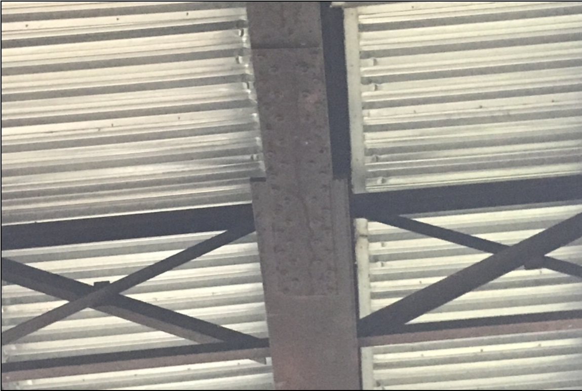
Span #1 girder #3 splice plate bottom flange - Bolt still missing
