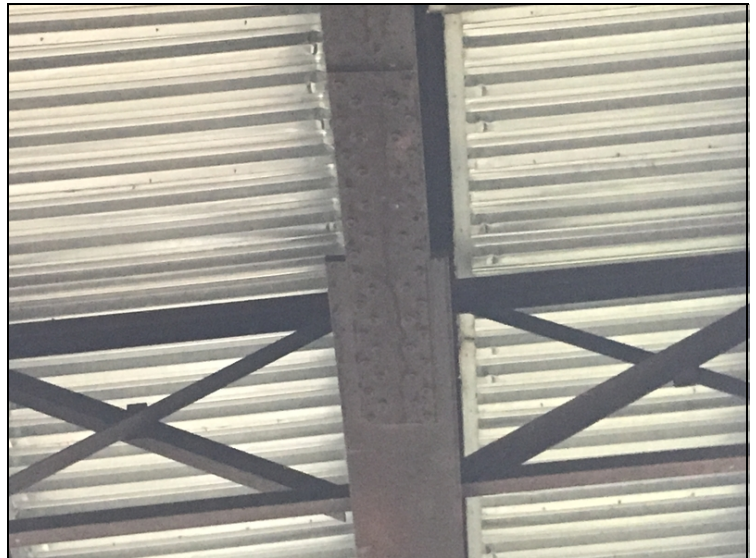
Span #1 girder #3 splice plate bottom flange - Bolt still missing
