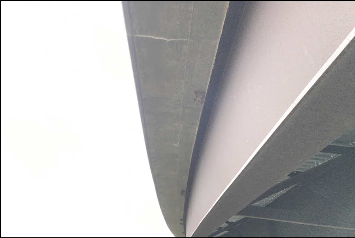
Right overhang typical transverse efflorescence and cracking.
