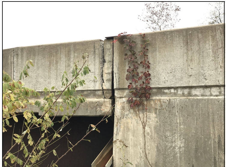
An area of the left bridge railing at abutment #1 has an area approximately 6" long and full height of the railing that is completely fractured under the vertical portion of the sliding plate assembly at abutment #1.
