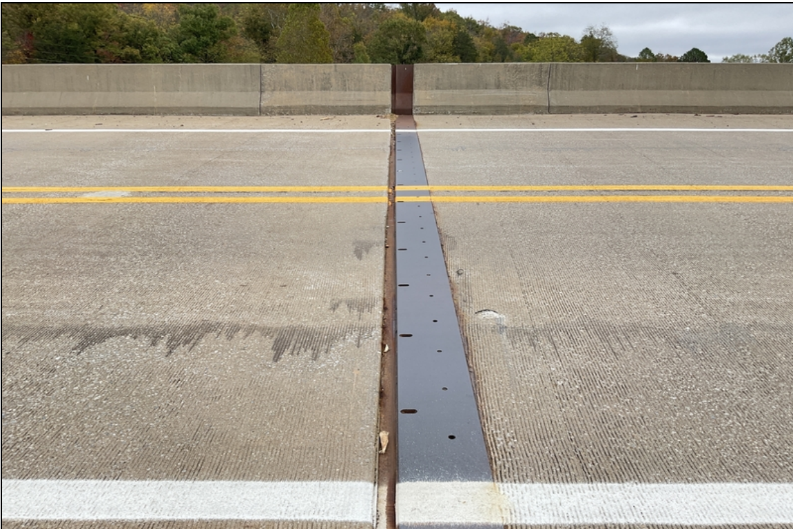
Bent #4 sliding plate.
