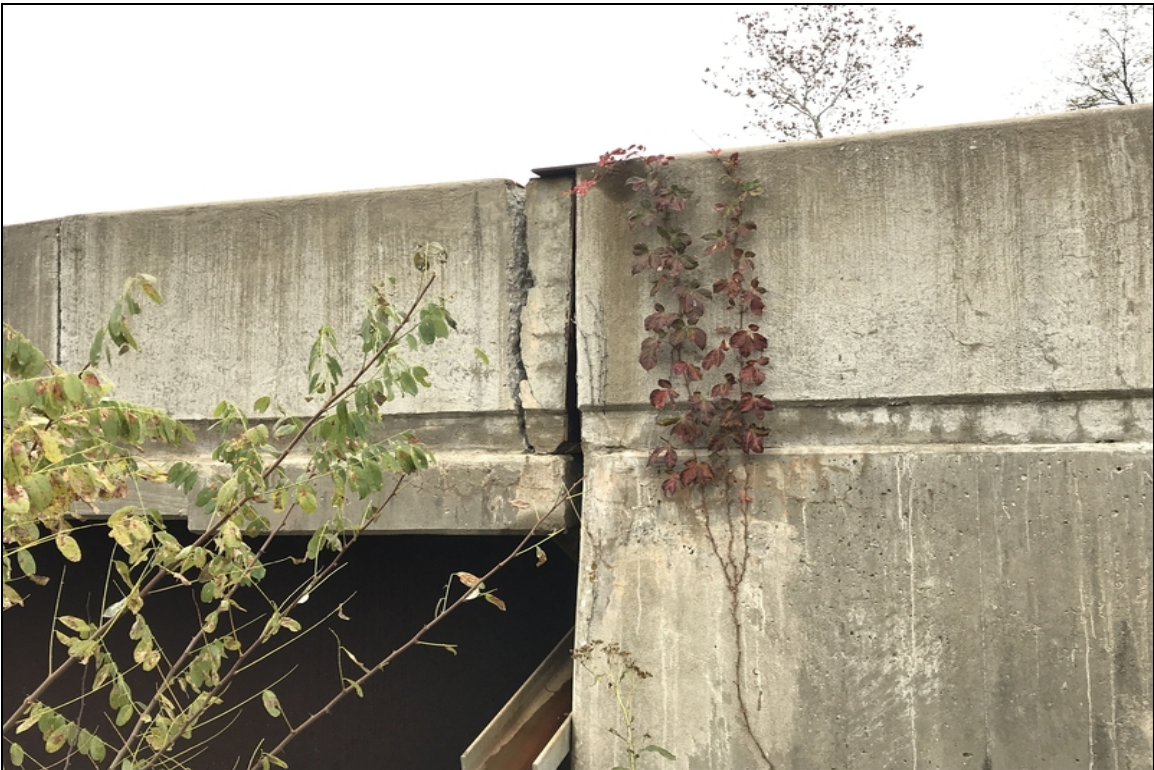
An area of the left bridge railing at abutment #1 has an area approximately 6" long and full height of the railing that is completely fractured under the vertical portion of the sliding plate assembly at abutment #1.
