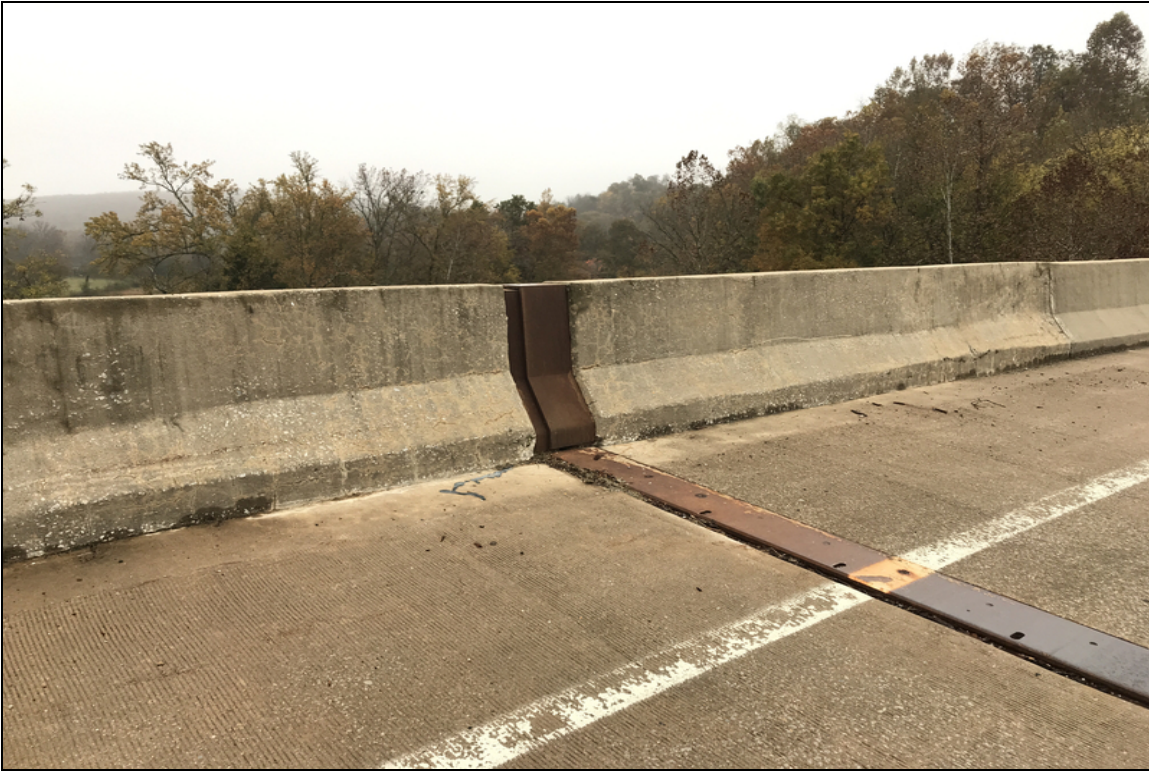
Right parapet map cracking at bent #2.
