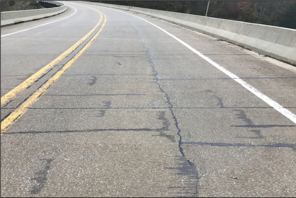
Typical sealed cracking northbound lanes
