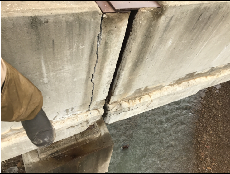
Left parapet over bent #4 complete fracture.
