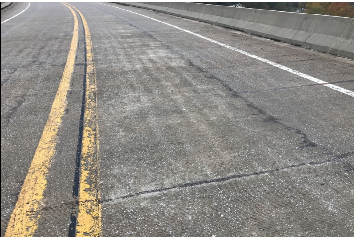
Longitudinal cracking has been sealed typical throughout deck surface
