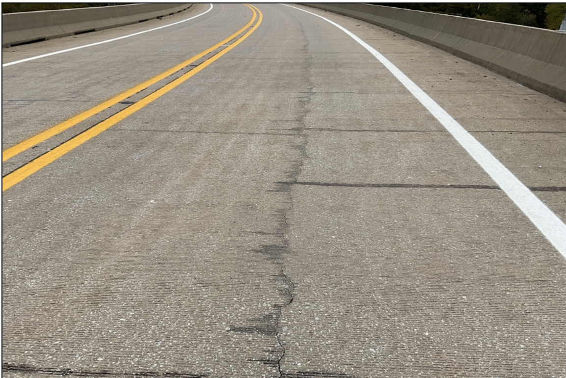
Large full length longitudinal cracking in the right lane of bridge deck.
