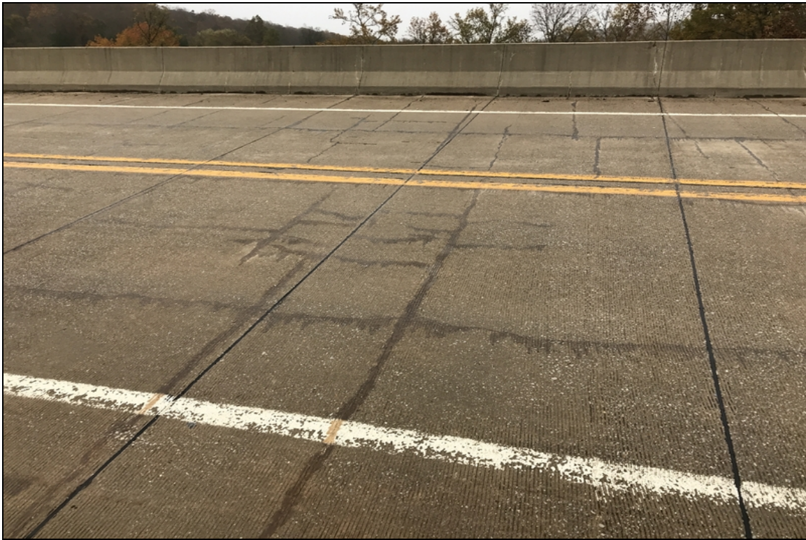
Sealed transverse deck cracking over bent #1
