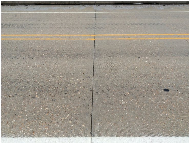
Concrete deck at construction joints Leakage thru deck
