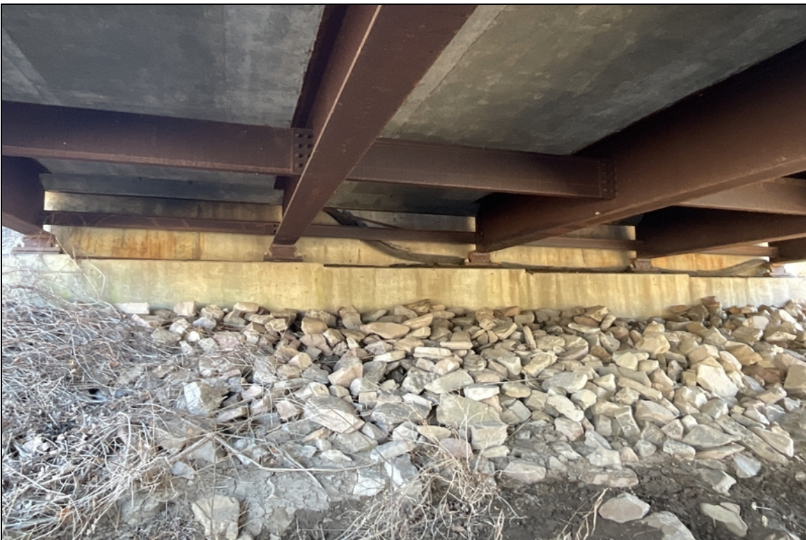
View of joint material at abutment #2.
