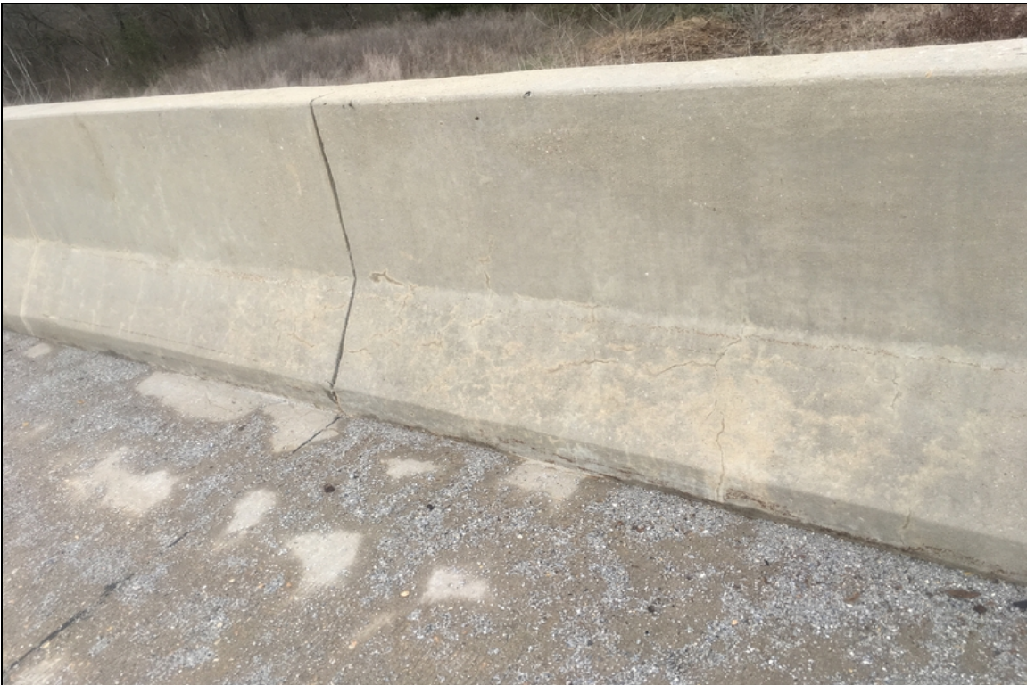
Map cracking on the parapet wall.
