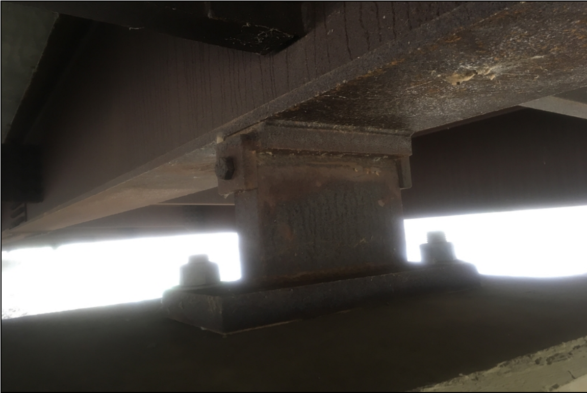
Typical bearing condition at bents #1,2,3.
