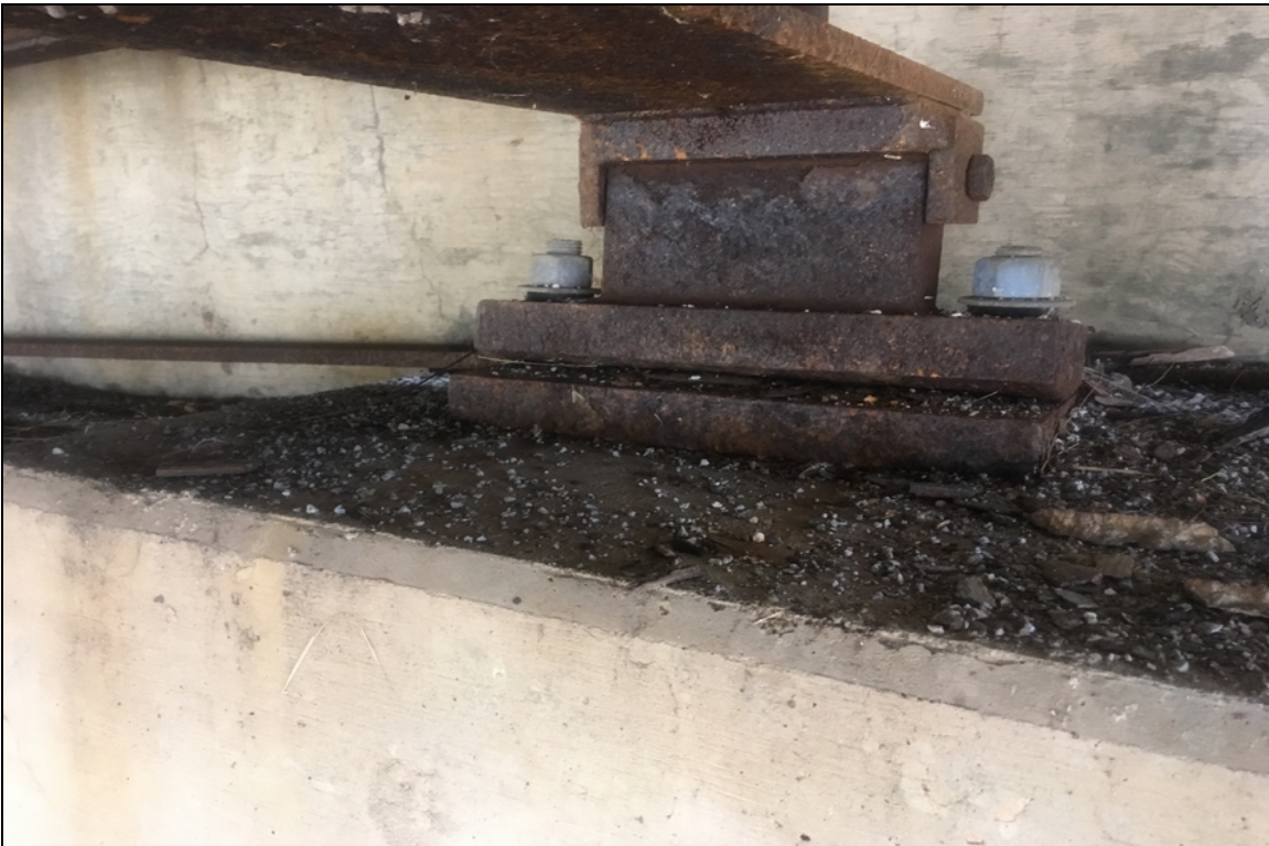
View of typical bearing corrosion at abutment #1.
