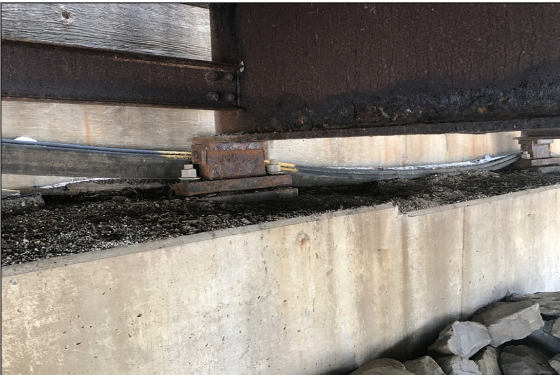
Compression joint material is still displace at abutment #2 allowing water and debris to flow freely onto bridge seat.
