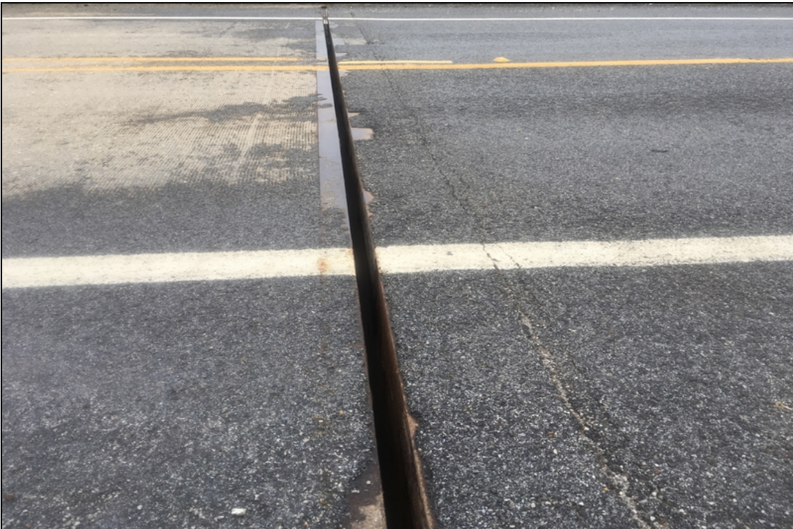
Abutment #2 compression joint seal condition.
