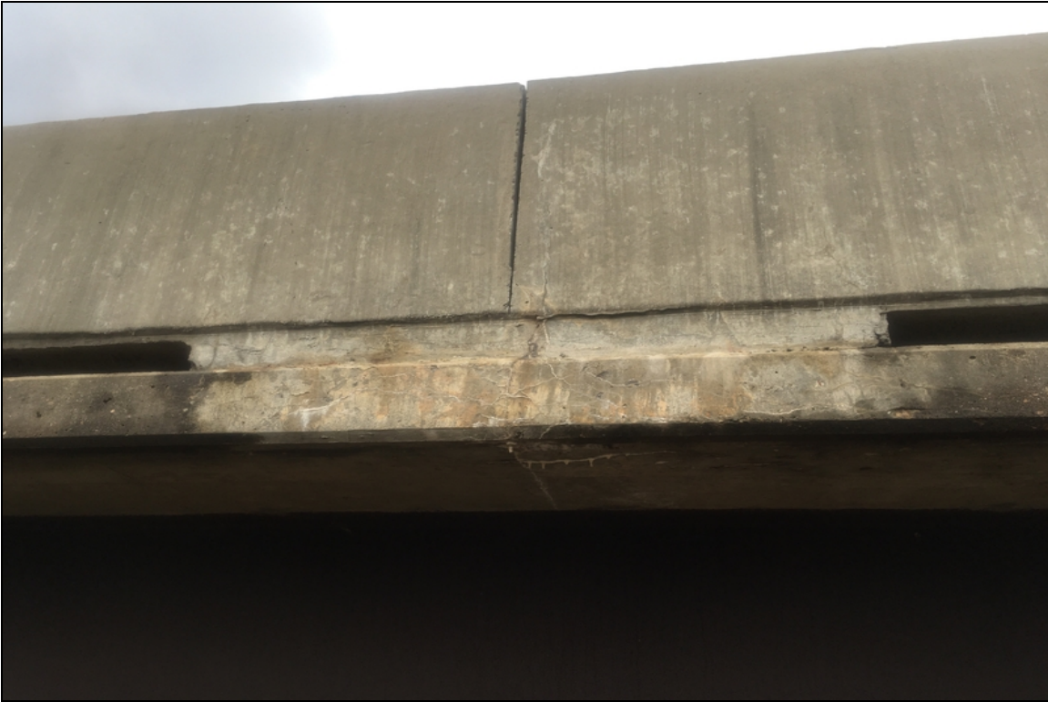
Efflorescence map cracking in the right and left deck edge. Typical.
