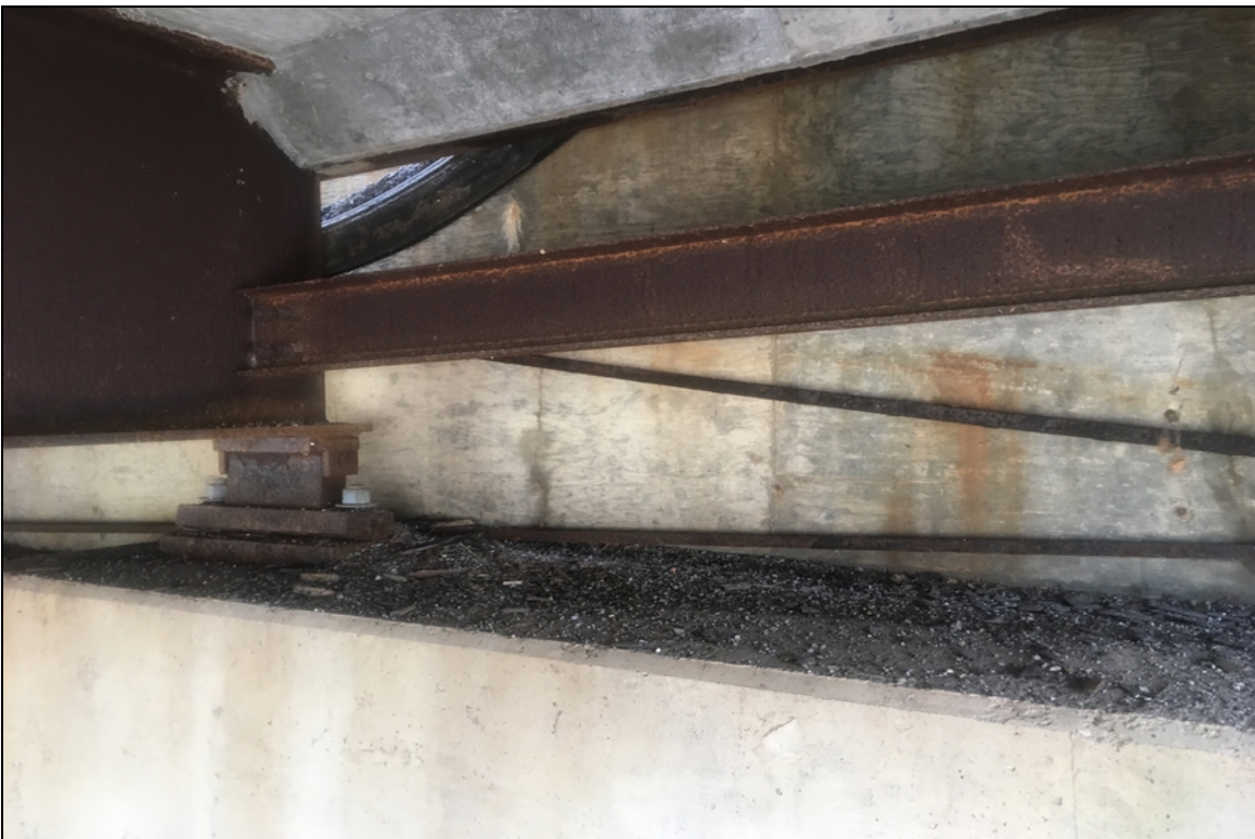
The retaining steel has become unattached at abutment #1 allowing the compression joint seal to drop out of position.
