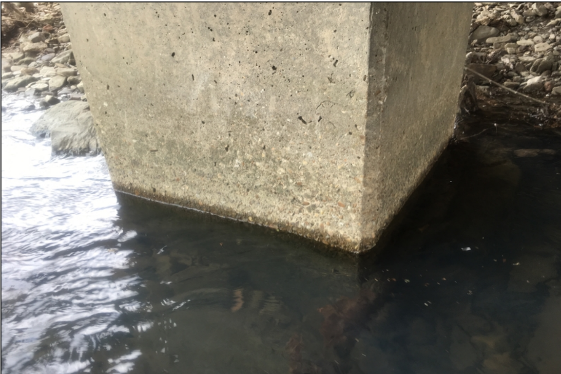
Minor abrasion at the left column of bent #3.
