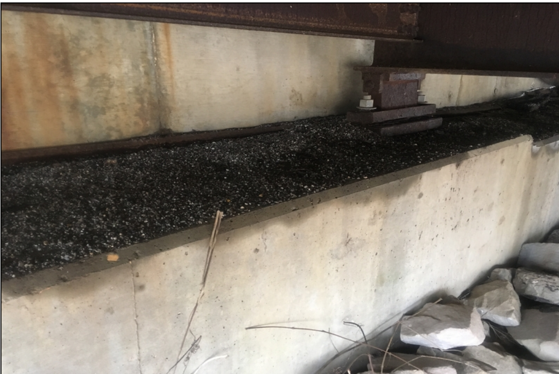
Build up on the abutment #2 bridge seat.
