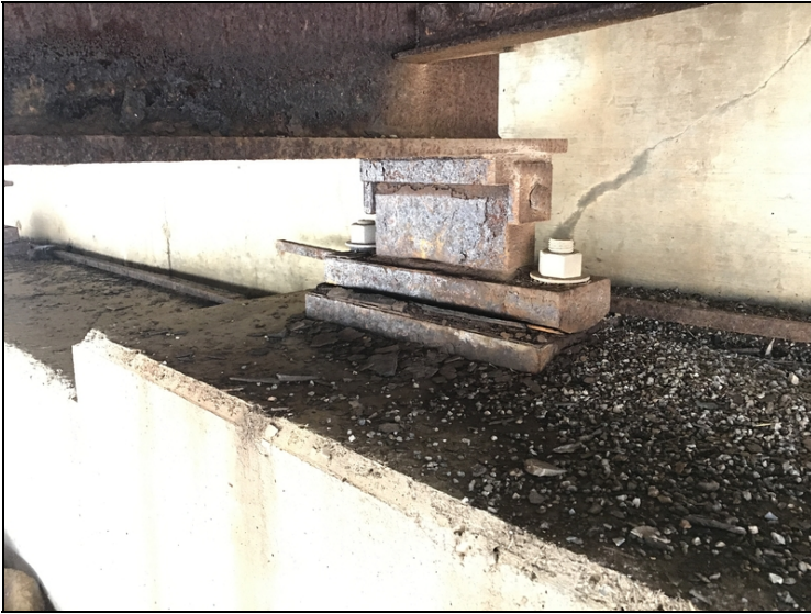
Bearing #3 at abutment #1 flaking rust due to leaking joints.
