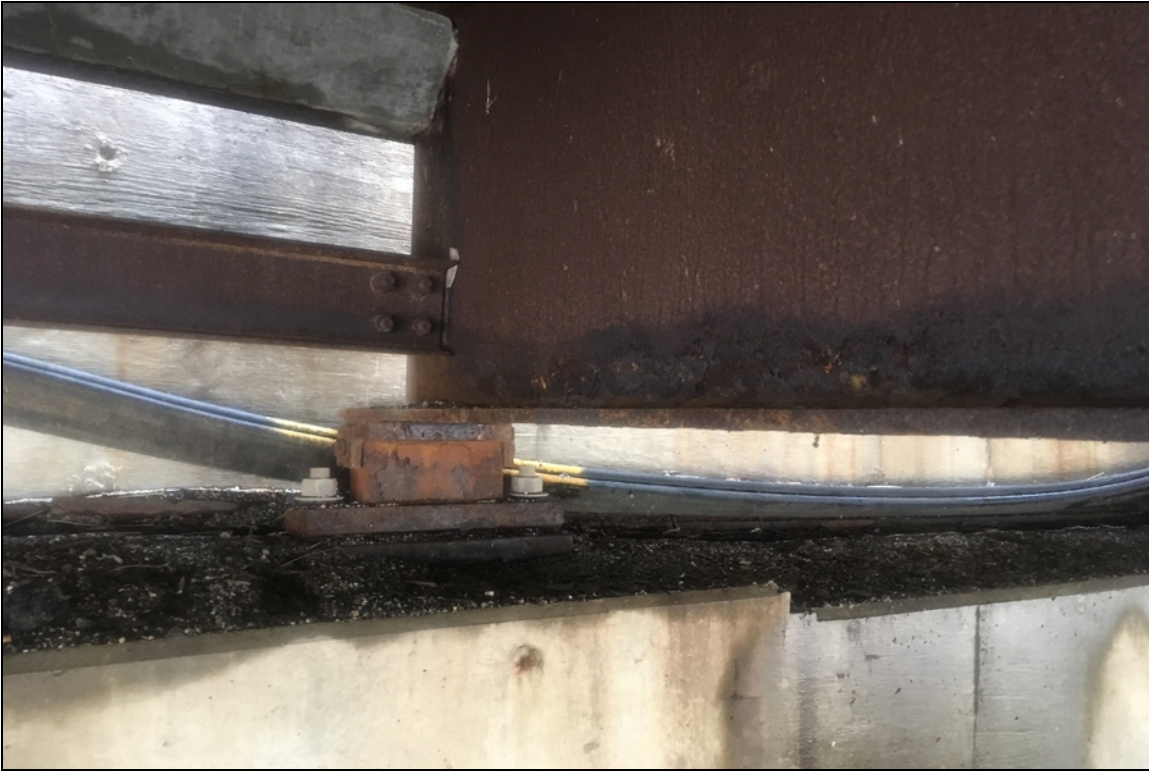
Beam end and bearing condition of beam #3 at abutment #2.
