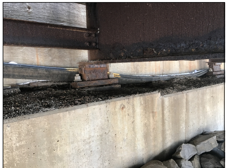
Compression joint material is still displace at abutment #2 allowing water and debris to flow freely onto bridge seat.
