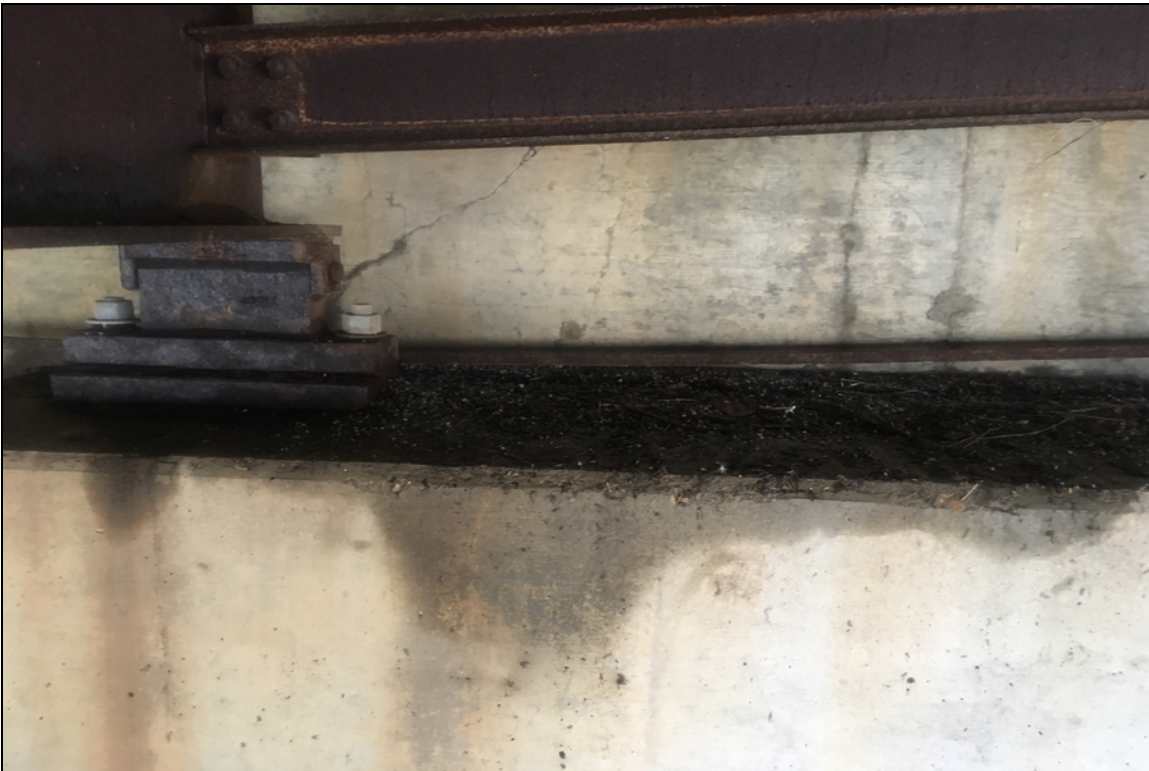
Build up on the bridge seat at abutment #1 below the missing joint seal area is promoting corrosion of the bearings.
