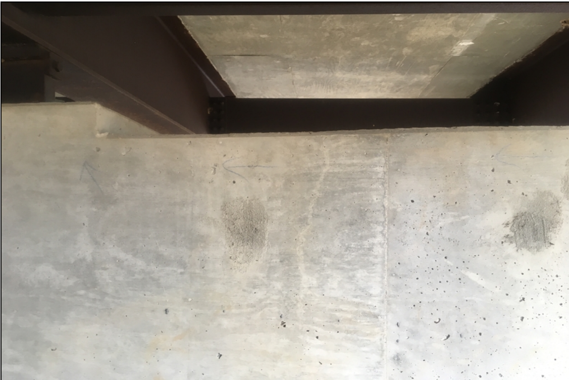
View of hairline cracking in the pier caps. Typical.
