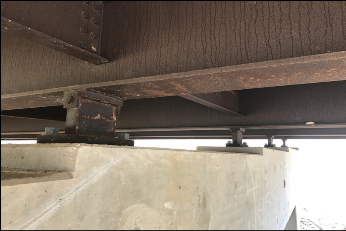
View of bearings at bent #2
