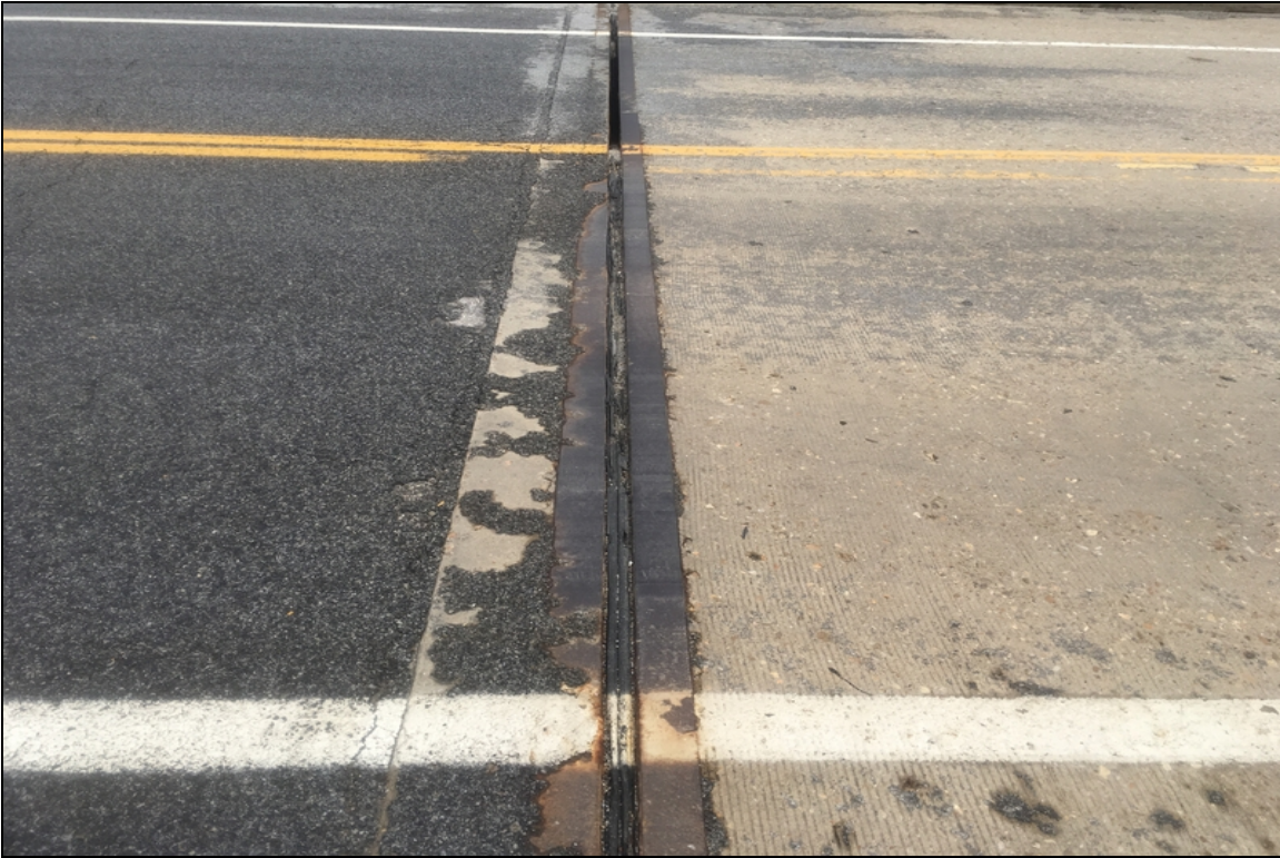
Abutment #1 compression joint seal condition.
