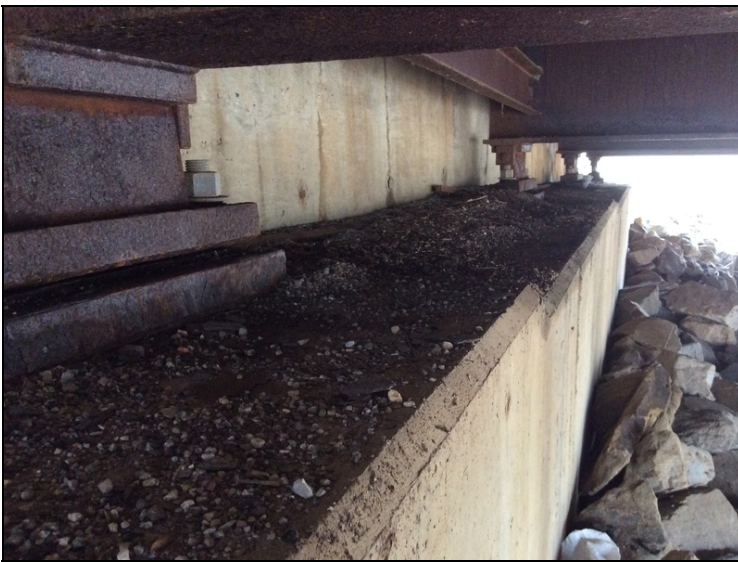
Bent #5 concrete cap- gravel and debris buildup
