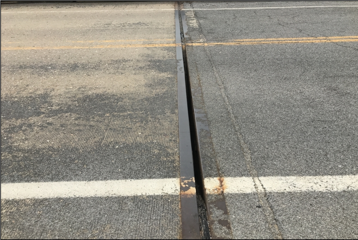
Joint seal failure at abutment #1
