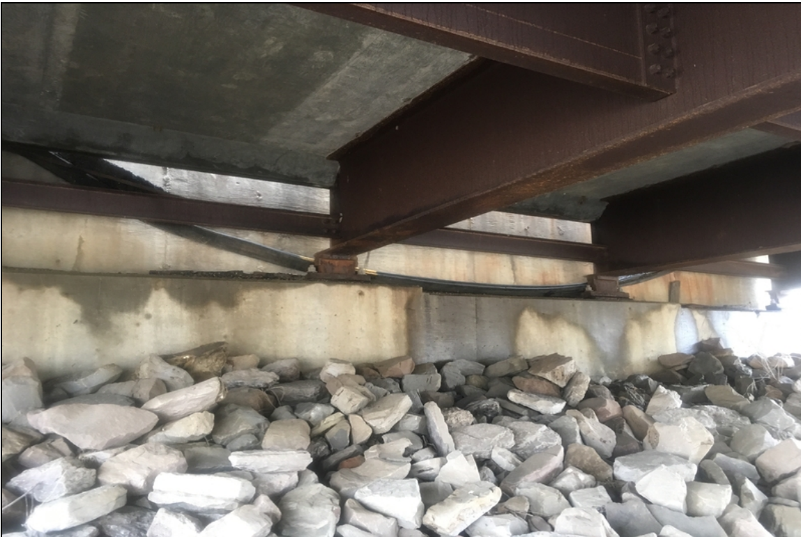
General view of abutment #2. Note the compression joint seal.
