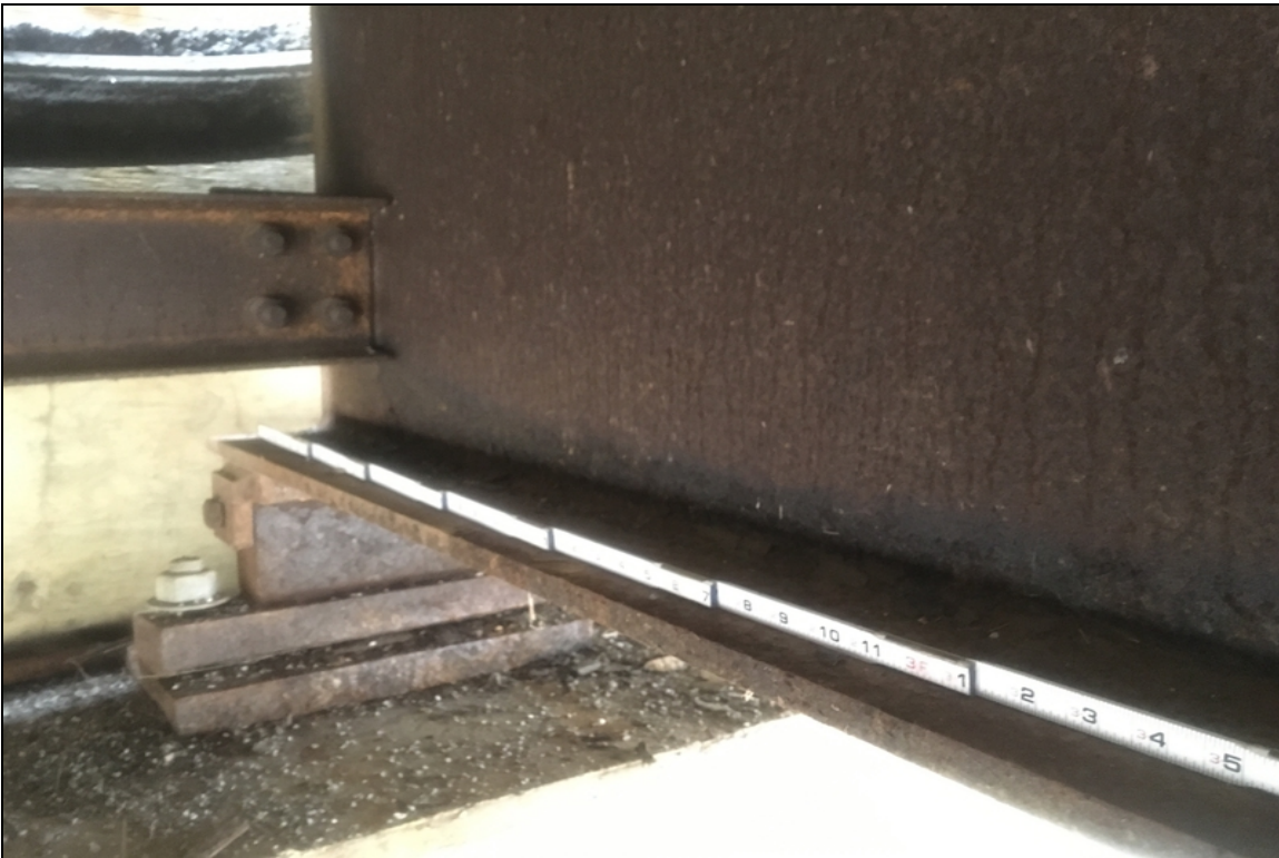
4' of Minor corrosion on the top of the bottom flange and lower web at beam #2 at abutment #1.
