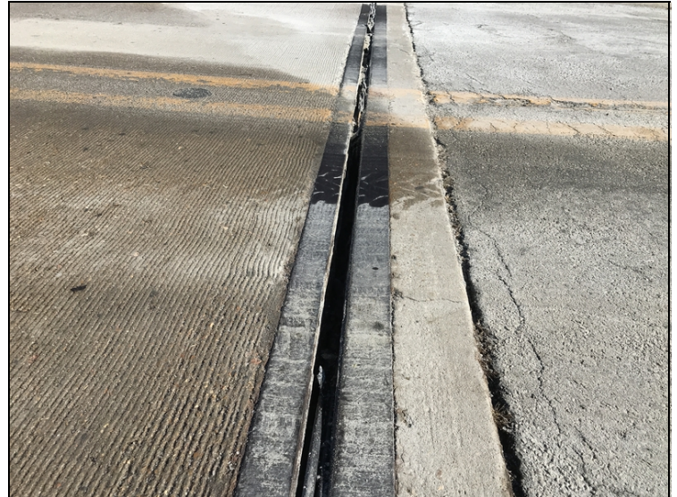
Abutment #1 expansion joint material lost adhesion.
