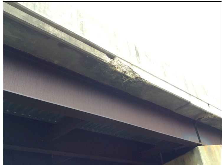
Soffit Span 3 right - spall with exposed reinforcing steel.
