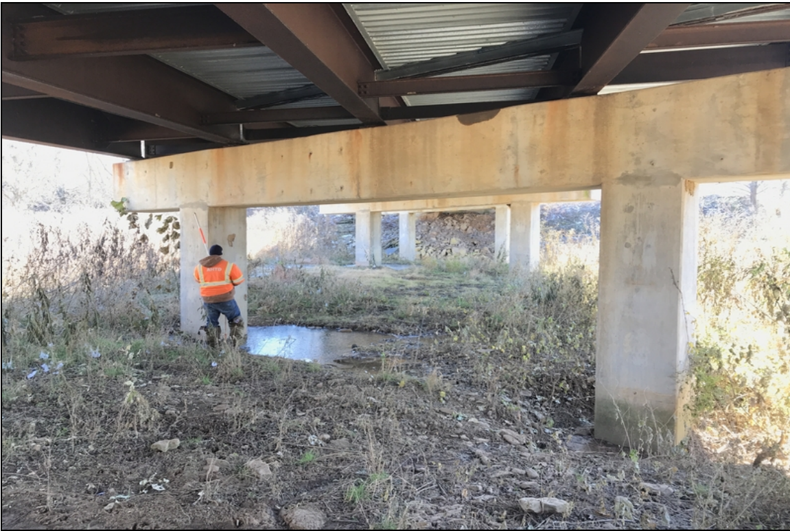
Localized scouring at bents 2 and 3
