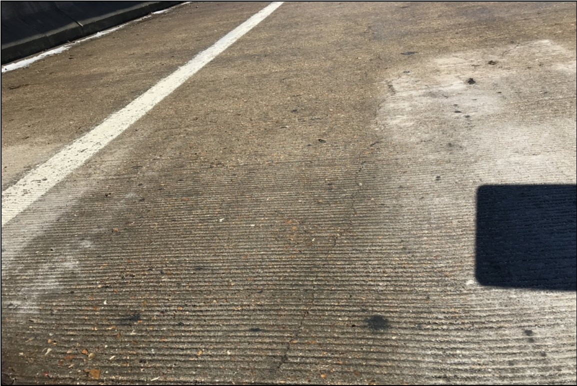
Span #2 left lane typical longitudinal cracking
