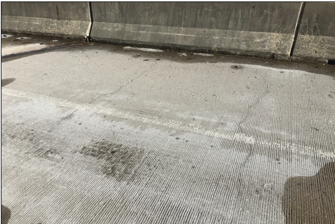
Span #3 right transverse cracking.
