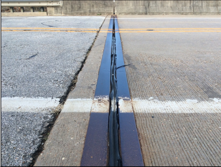
Abutment #1-Compression seal deteriorated.
