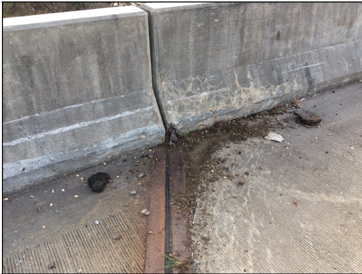
Deck bent #1 right spalling adjacent to joint and parapet.
