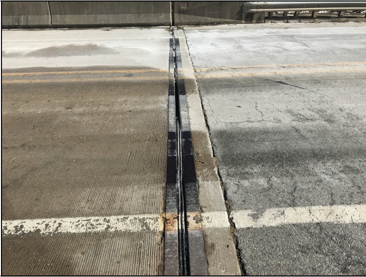
Abutment #1 expansion joint material lost adhesion.
