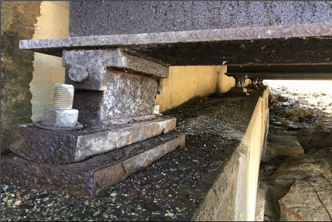
Typical condition of bearings at abutment #1.
