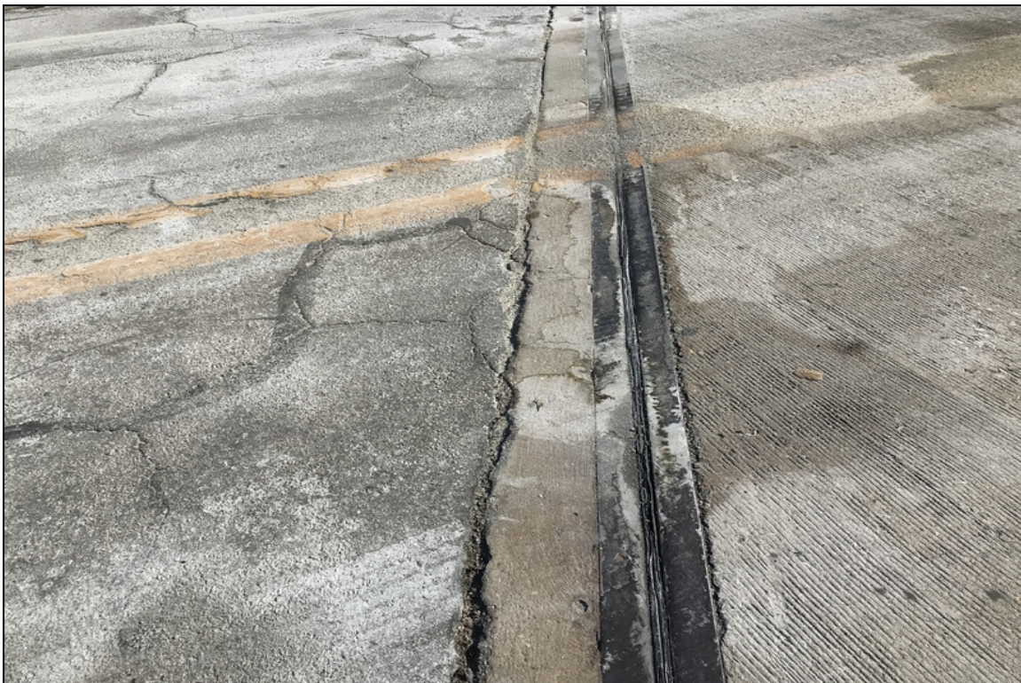
Abutment #2 top of abutment backwall cracking and minor spalling.
