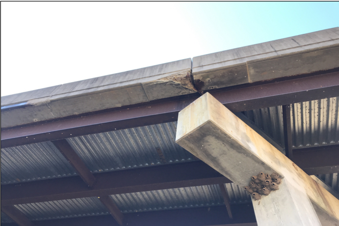
Deck span #1 overhang right spalling with steel exposed.
