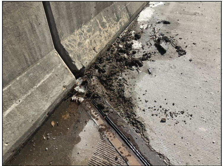
Span #1 at Bent #1 right spalling adjacent to road iron.
