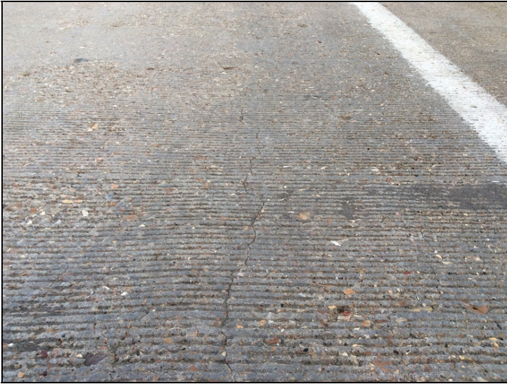
Span #1, right lane longitudinal cracking.
