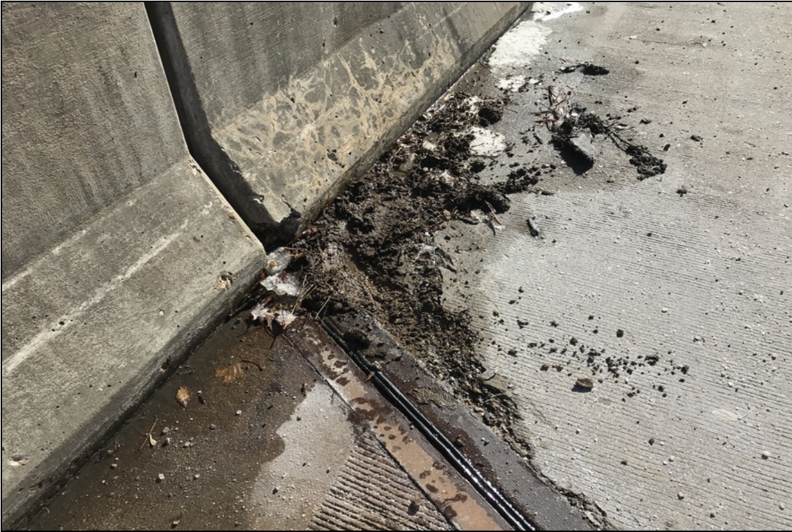
Span #1 at Bent #1 right spalling adjacent to road iron.
