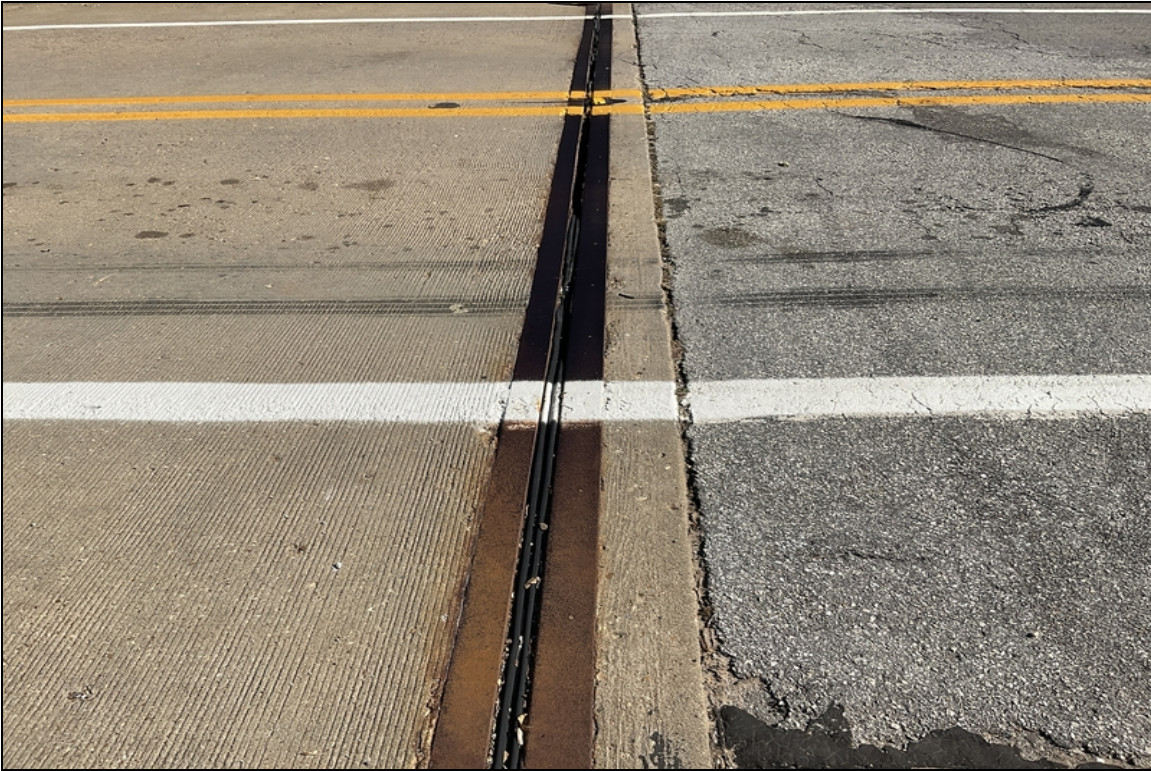
View of joint at abutment #1
