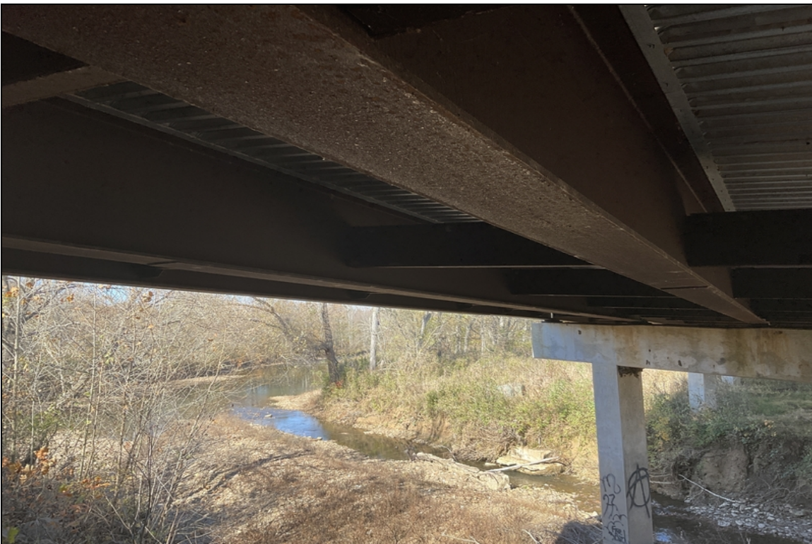
span #1 girders bottom flange #1 - #3 have welded cover plates varying in size.
