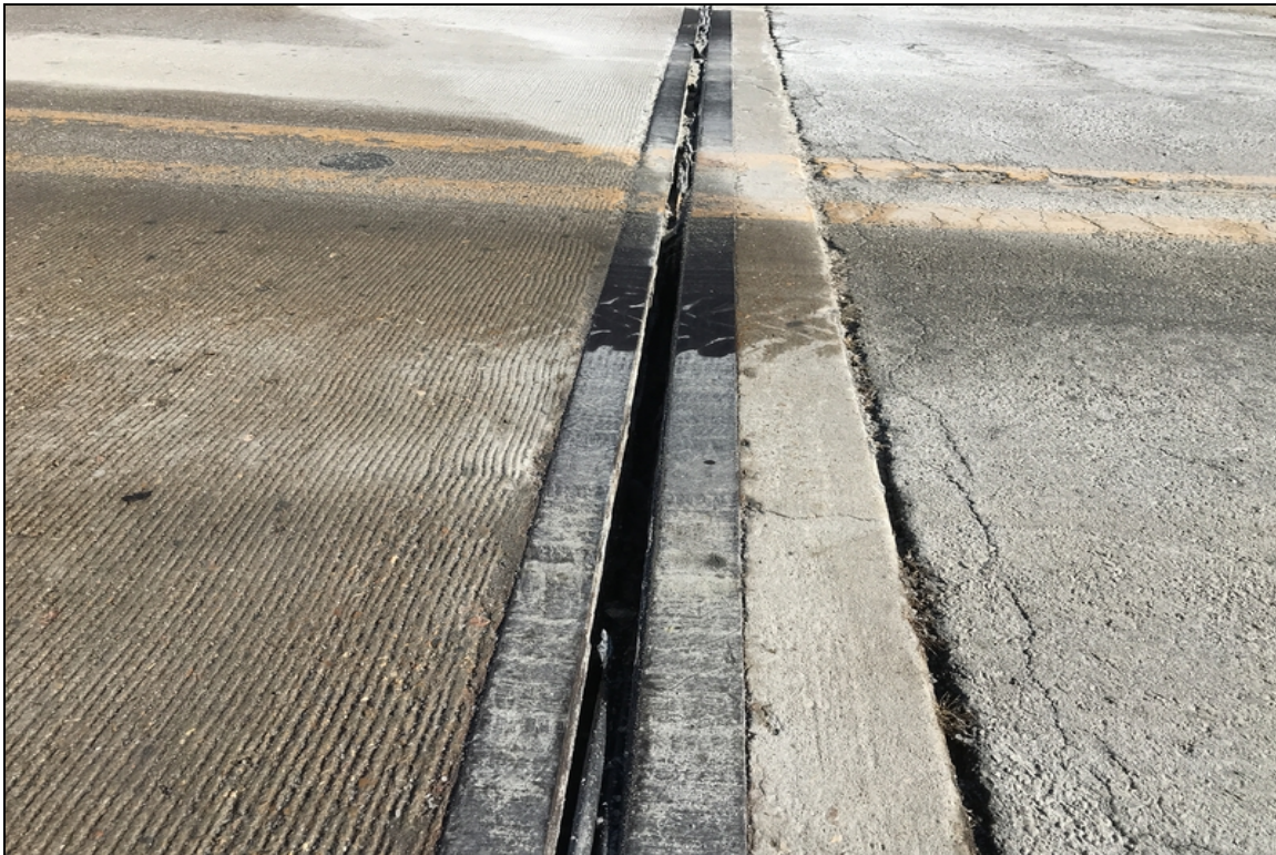
Abutment #1 expansion joint material lost adhesion.
