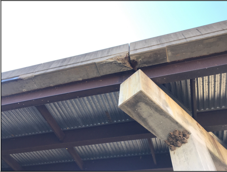
Deck span #1 overhang right spalling with steel exposed.
