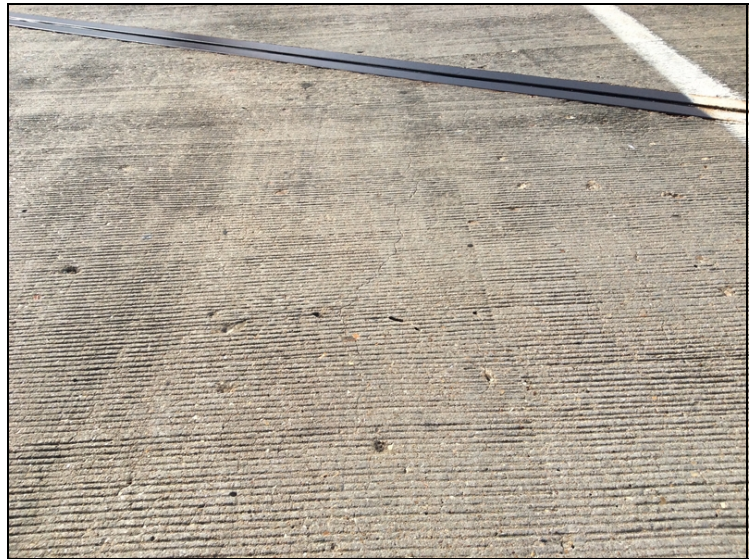
Span #3 Left lane adjacent to bent #2 looking South typical deck cracking.
