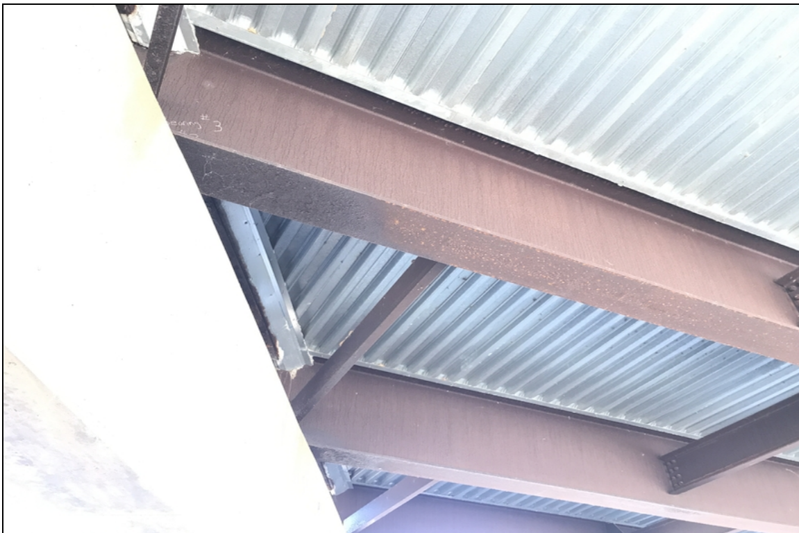
Span #3 typical flaking rust to bottom flange of girders at intermediate bents.
