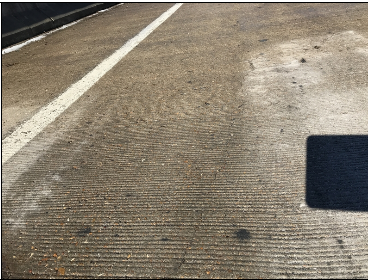
Span #2 left lane typical longitudinal cracking
