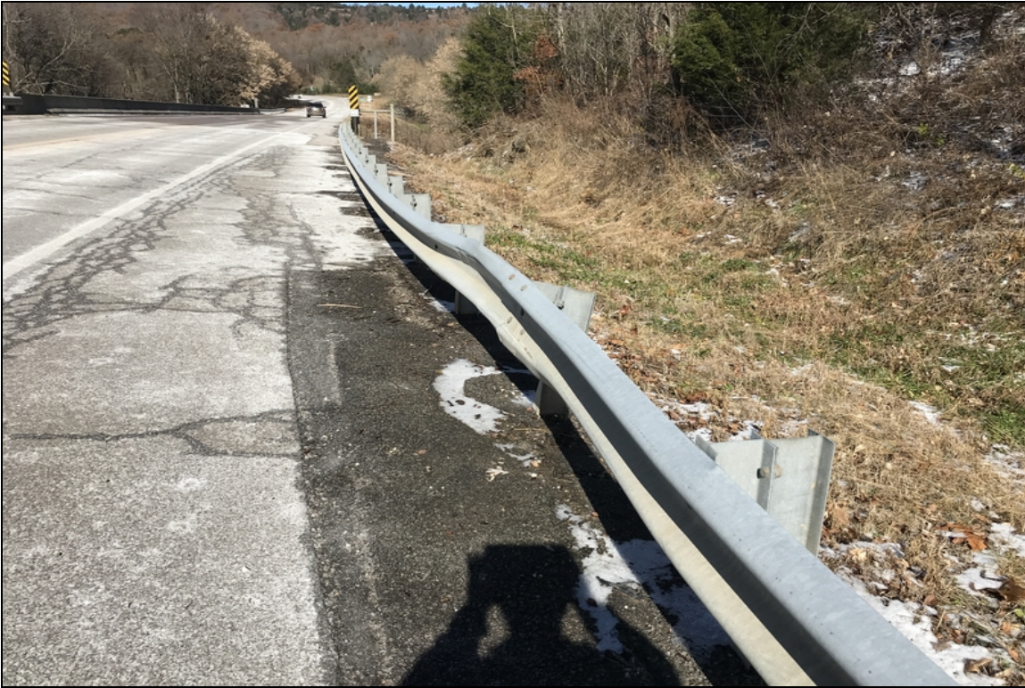
Southeast approach railing has collision damage that has caused out-of-plane bending to approximately 12° of the railing and twisted one of the railing post.
