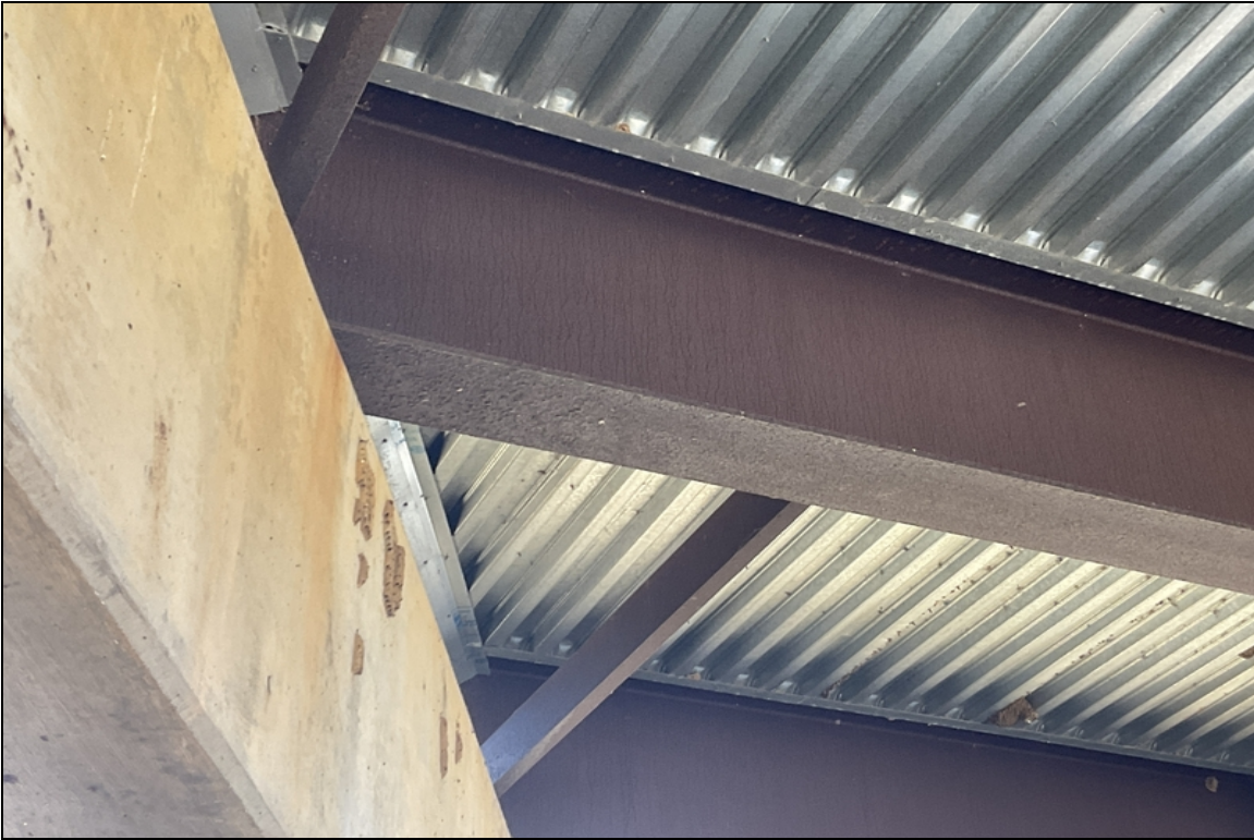
Typical flaking rust at girder ends
