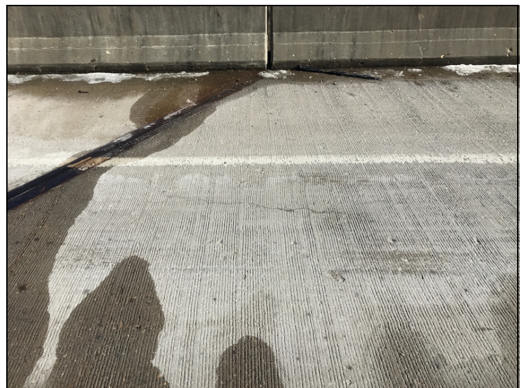
Span #2 right lane typical diagonal cracking.
