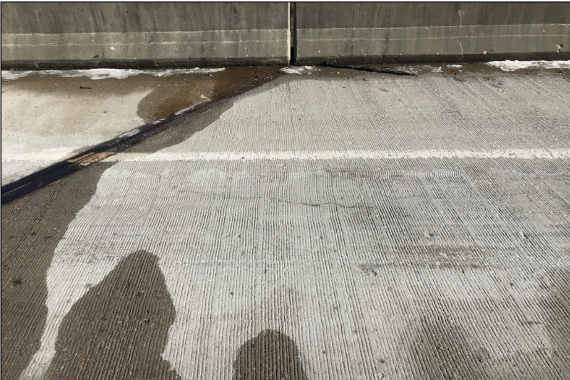
Span #2 right lane typical diagonal cracking.
