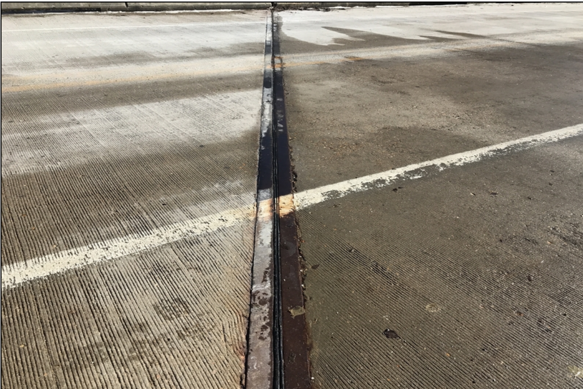
Bent #1 joint material condition
