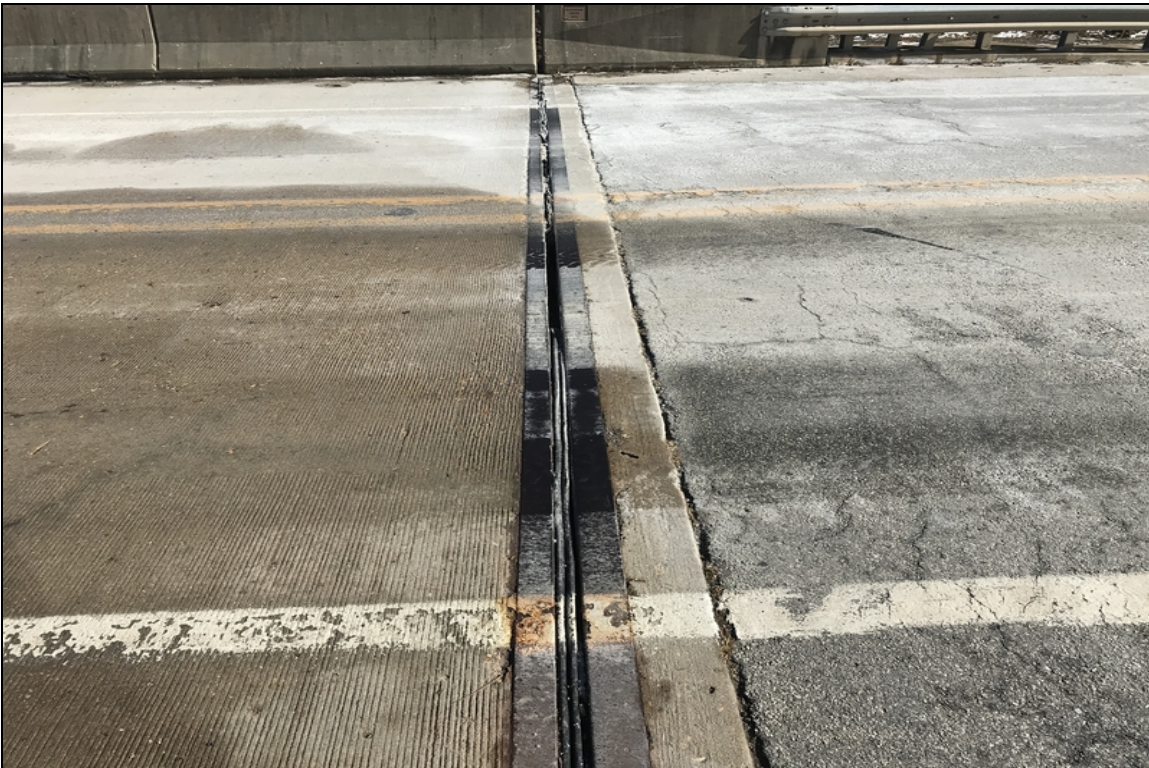
Abutment #1 expansion joint material lost adhesion.
