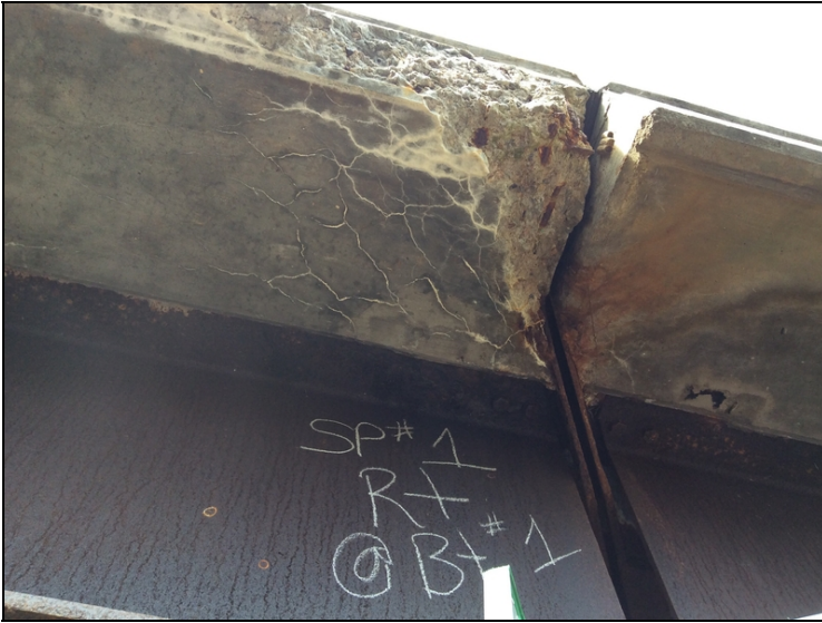
Span #1, right side over bent #1-Spalling / delaminated area with exposed reinforcing steel.
