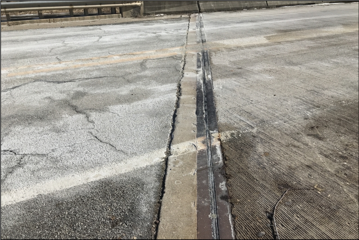
Abutment #2 joint material condition
