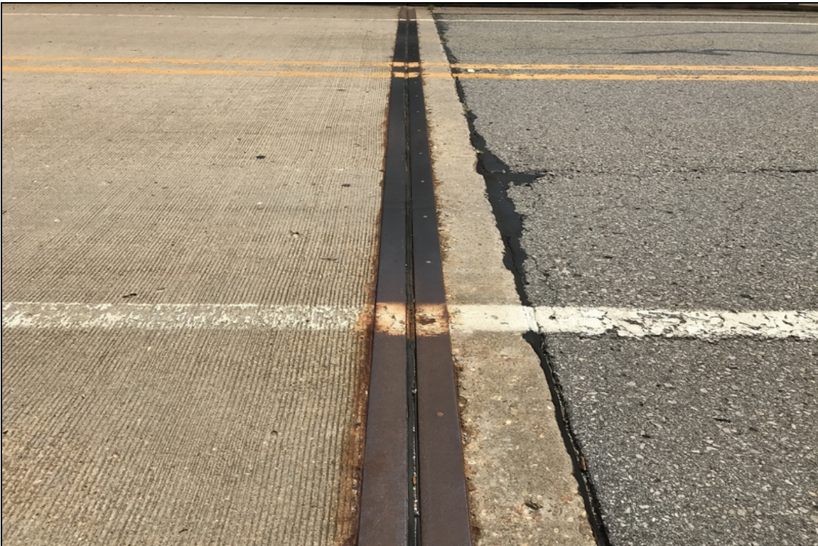
Abutment #1 expansion joint.
