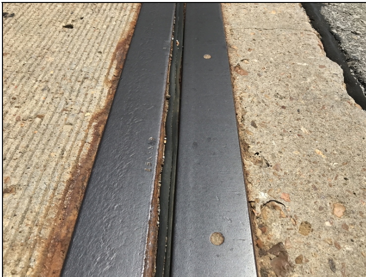
Abutment #1 road irons pack rust causing adhesion failure
