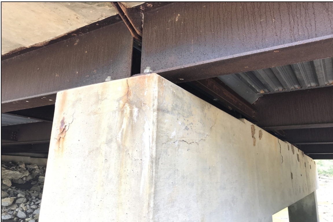
Substructure - The left side of bent #2 cap has a delaminated area on the back face that is approximately 3' long and propagates diagonally under bearing #1.
