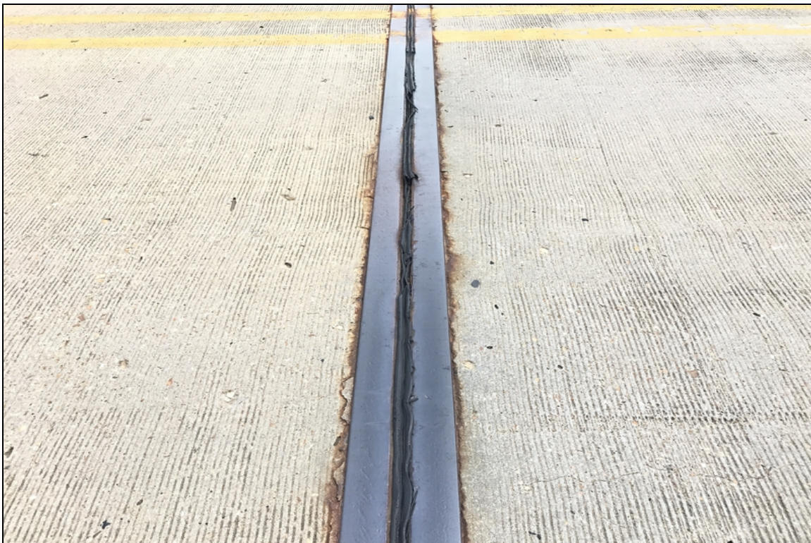
Bent #2 expansion joint material is cracking and tearing largely due to vehicle impactation.
