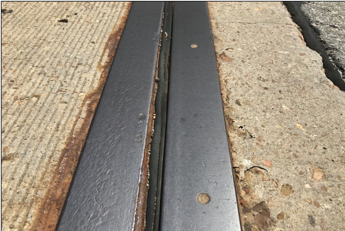
Abutment #1 road irons pack rust causing adhesion failure
