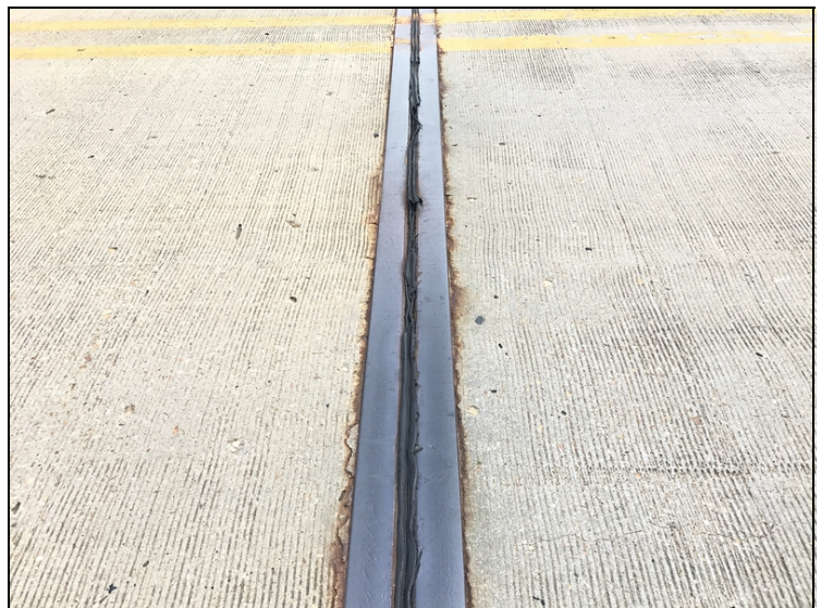
Bent #2 expansion joint material is cracking and tearing largely due to vehicle impact.
