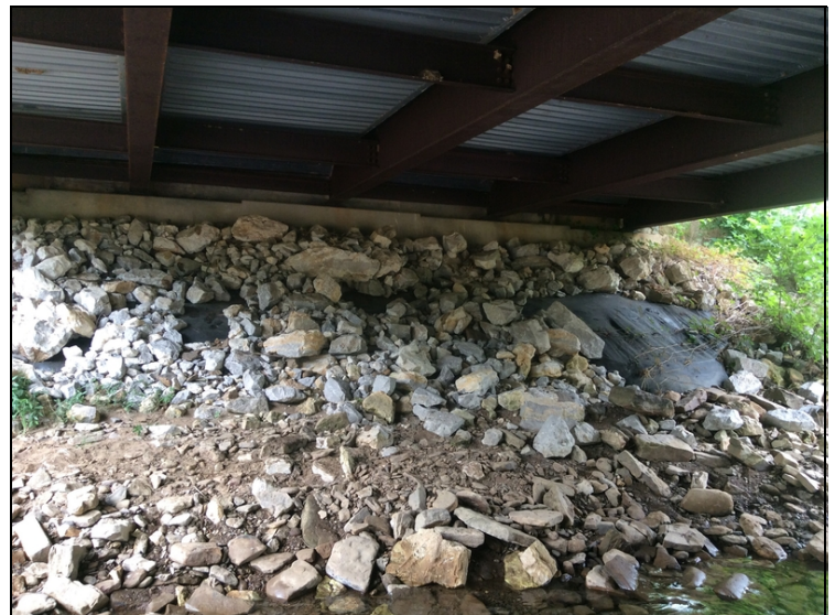
North embankment-Rip-rap displacement.
