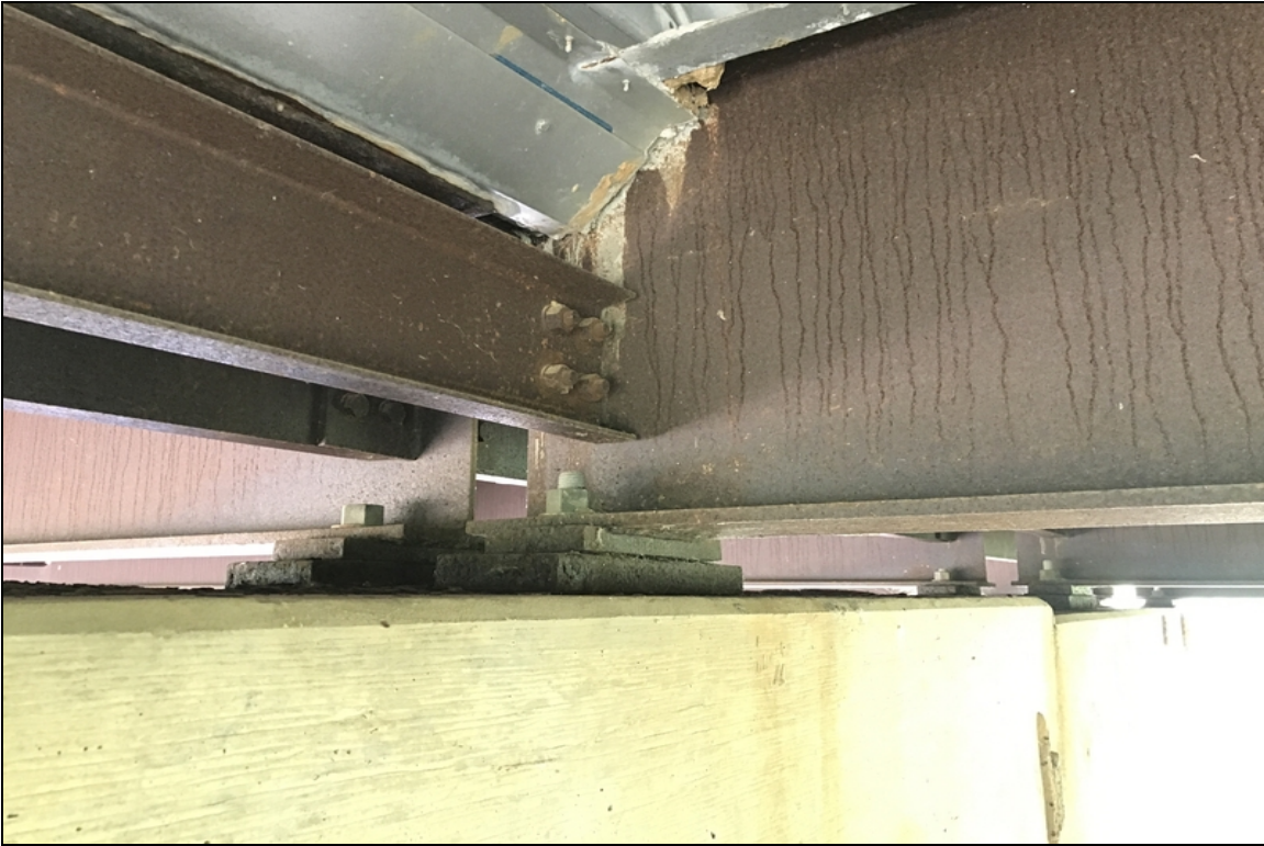
Bent #1 span #1 Typical minor typical minor flaking rust to bearings.
