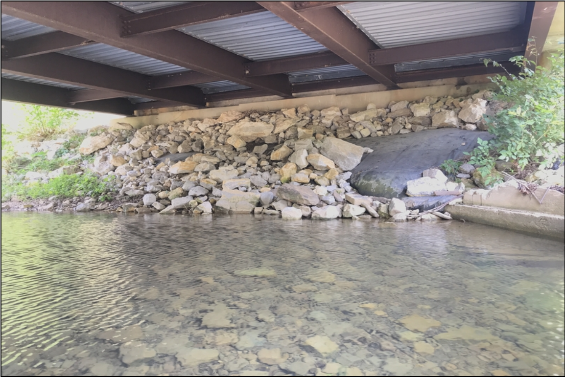
Embankment adjacent to abutment #2 has rip rap that has been displaced.
