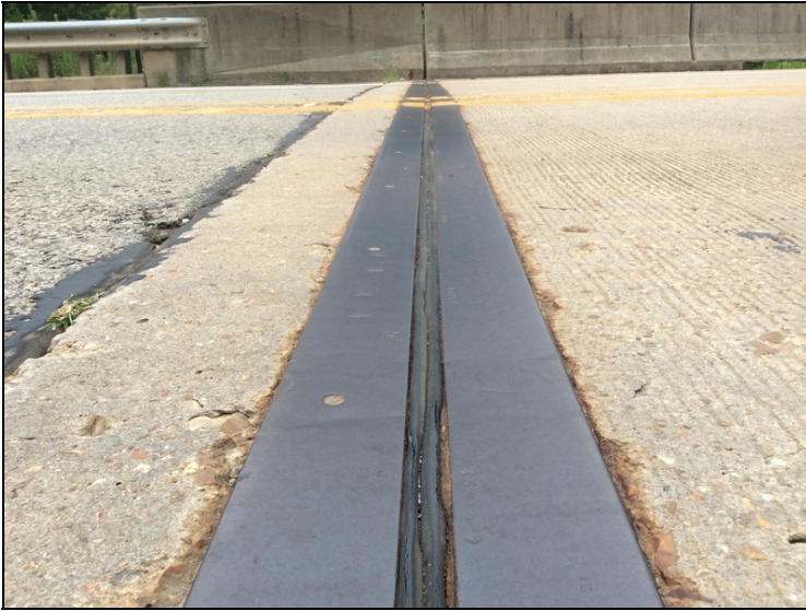
Abutment #1-Deteriorated compression joint seal.
