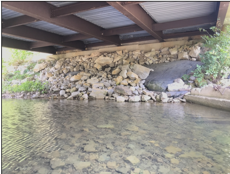
Embankment adjacent to abutment #2 has rip rap that has been displaced.
