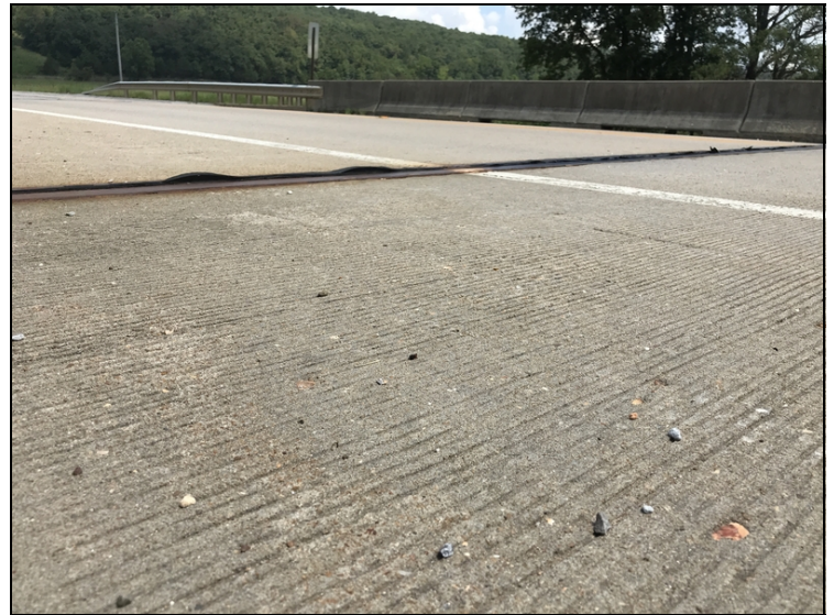
Bent #2 expansion joint is backing out.
