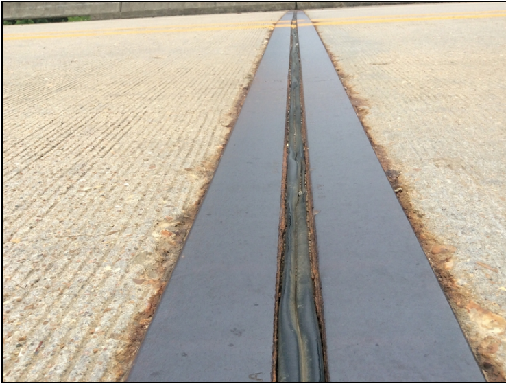
Pack rust in compression joint assembly.
