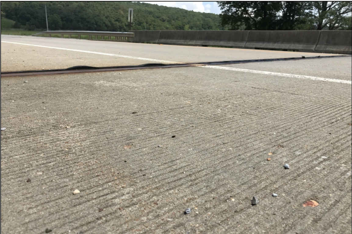
Bent #2 expansion joint is backing out.
