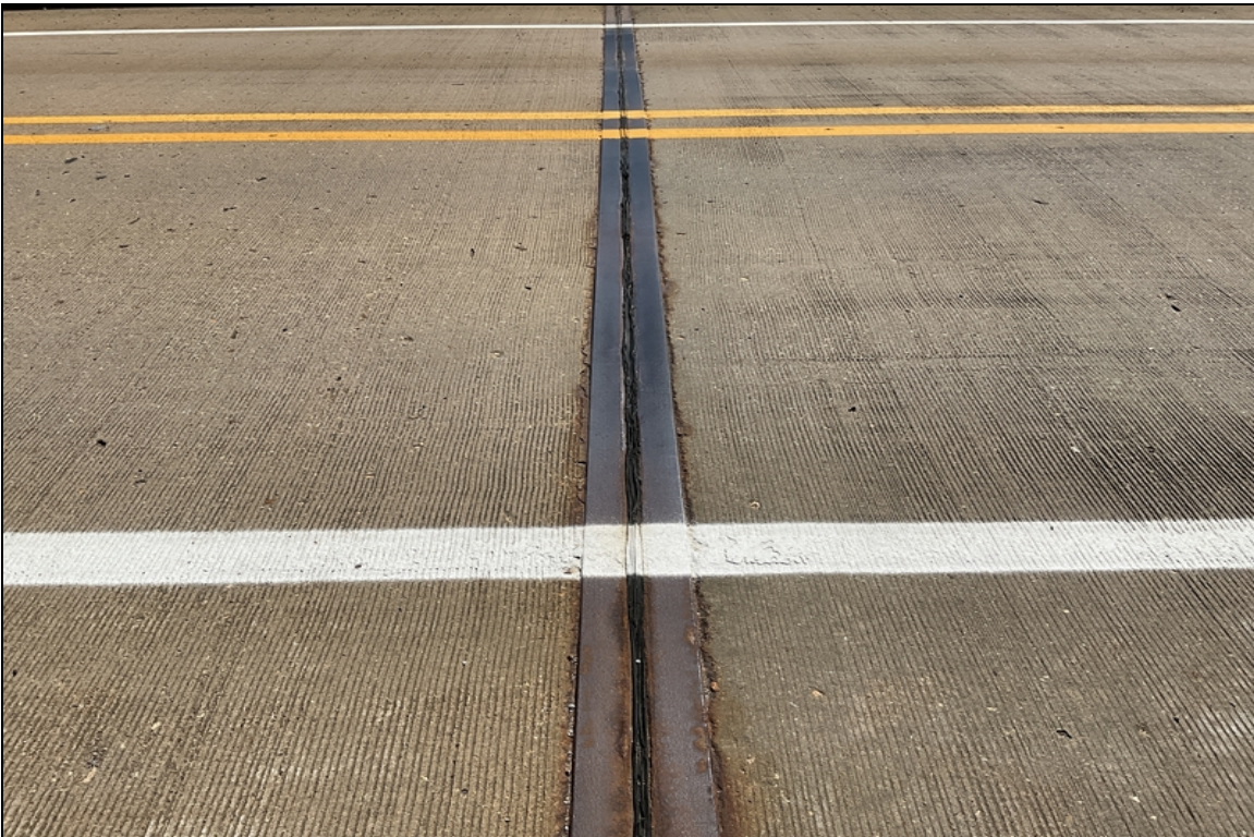
View of joint at bent #2.
