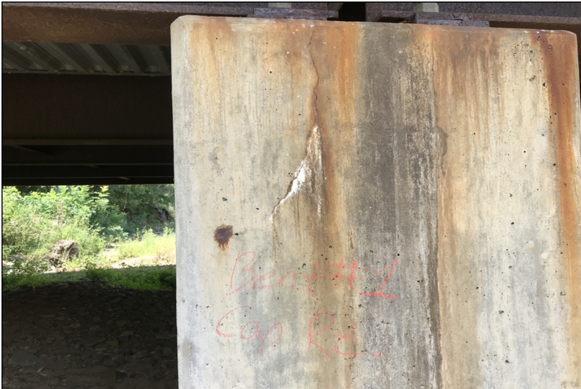
Bent #1 cap right has a vertical crack with minor efflorescence accumulation.
