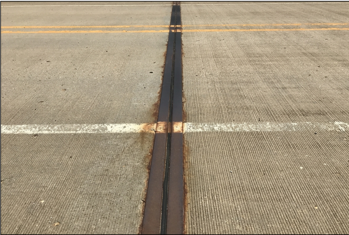
Bent #1 expansion joint.
