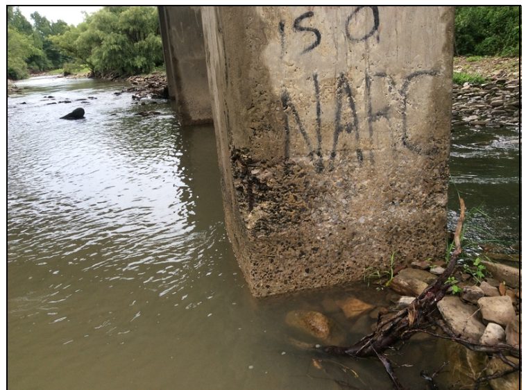
Bent 2 Column 1 ahead side spalling with steel exposed.
