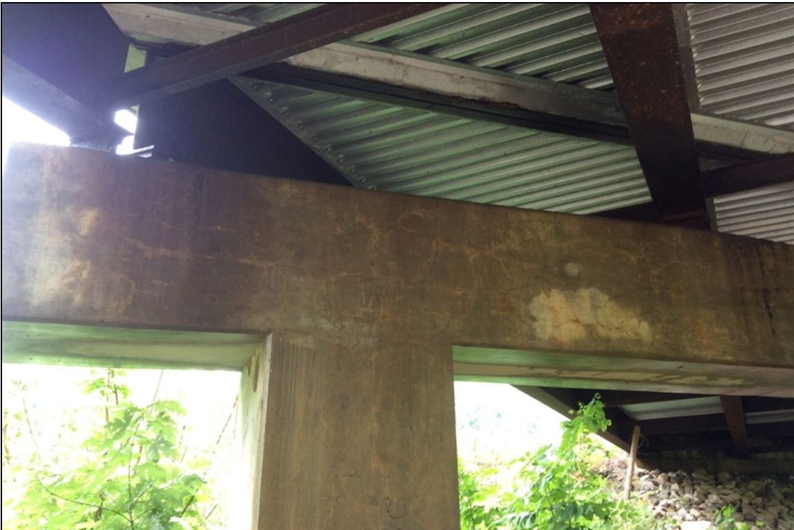
Bent 4 cap mapcracking.
