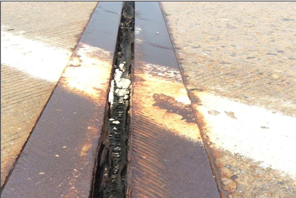
Bent 2 joint material lose of adhesion and flaking rust on road irons.
