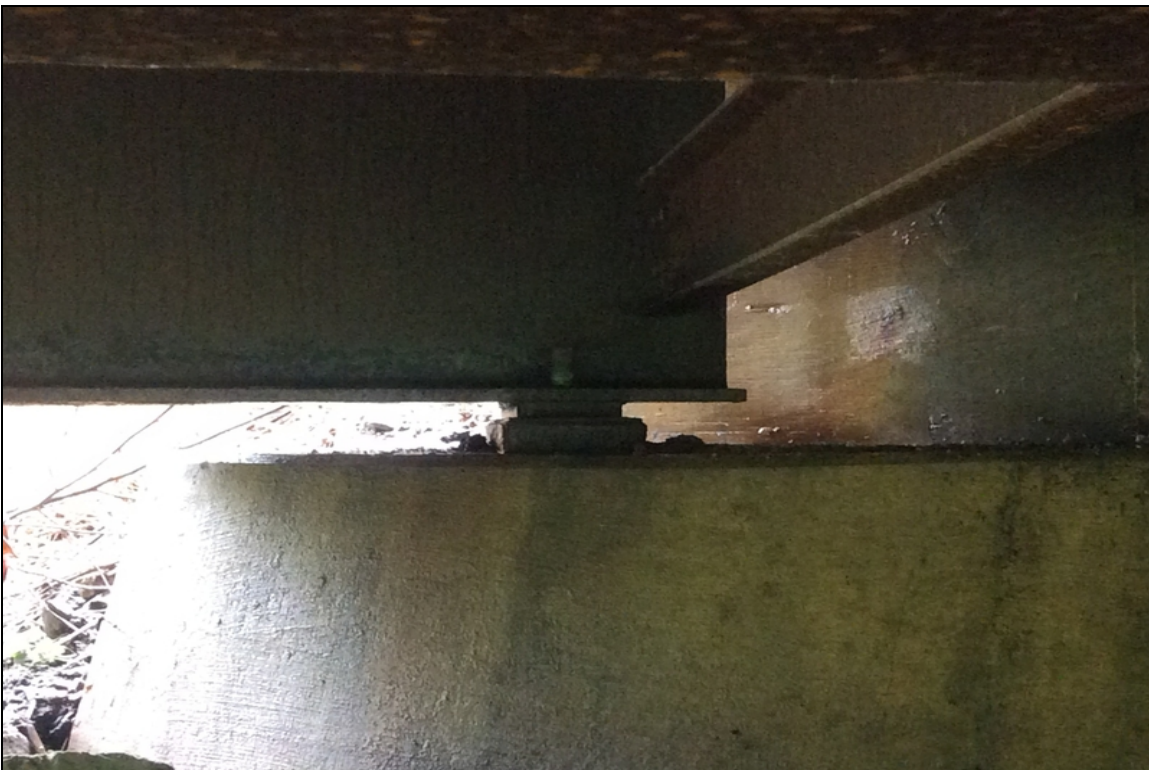
Span 5 abutment 2 girder 1 nut is missing.
