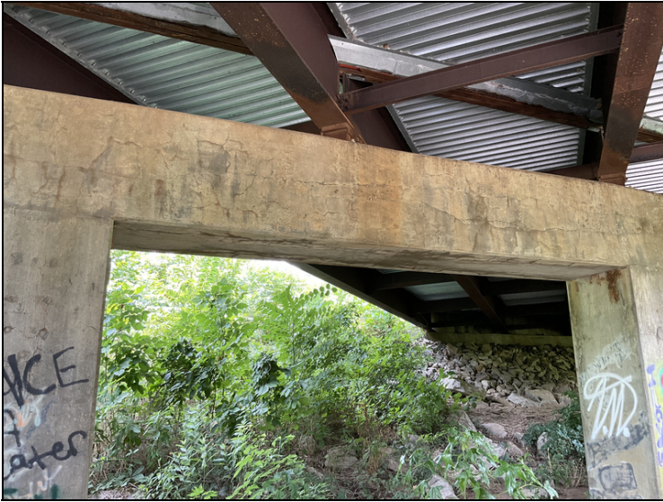
Cracking in cap the behind side of bent #4
