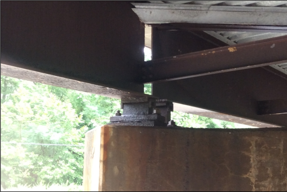
Span 1 Bent 1 Bearing 1 - Typical condition of bearings with active corrosion.
