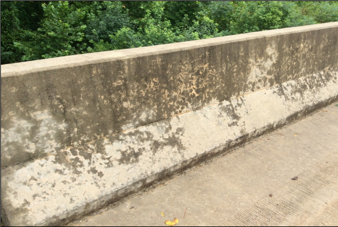
Railing Right typical view of cracking in parapet wall.
