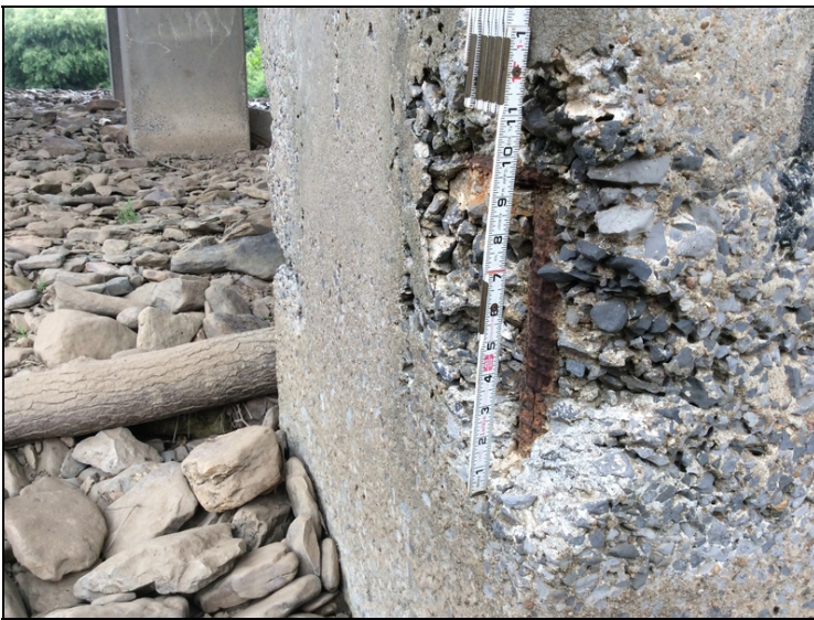
Exposed rebar column #1 of bent #2
