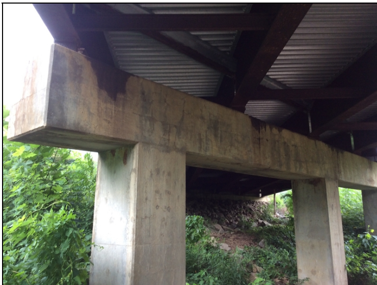
Typical map cracking to all bent caps.
