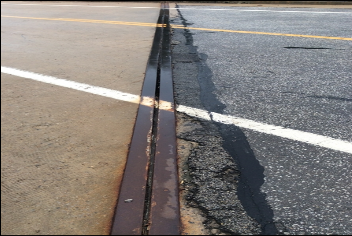
Abutment 1 joint material displaced and top of abutment back wall has spalls.
