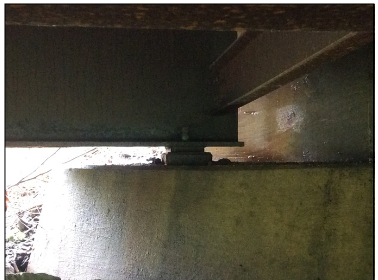
In span #5 abutment #2 girders #1 has nut is missing for the anchor bolt.
