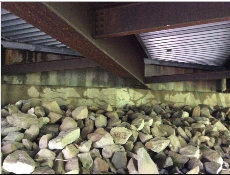
Map cracking to face of abutment #2
