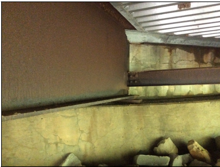
In span #5 abutment #2 girder #2 has nut is missing for the anchor bolt.
