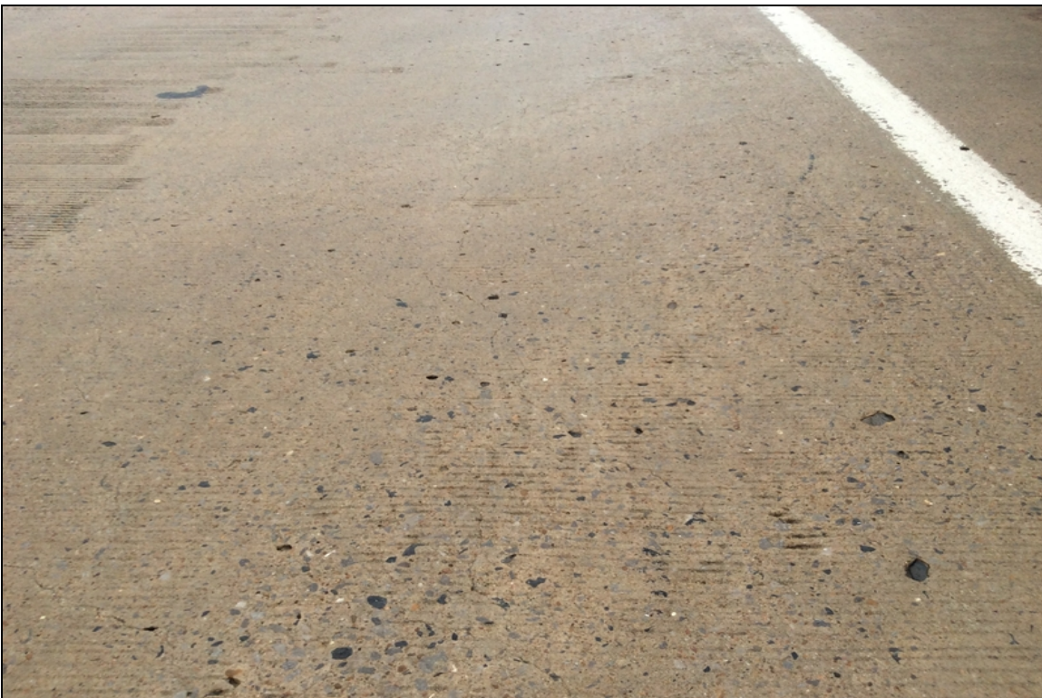
Span 1 typical map cracking.
