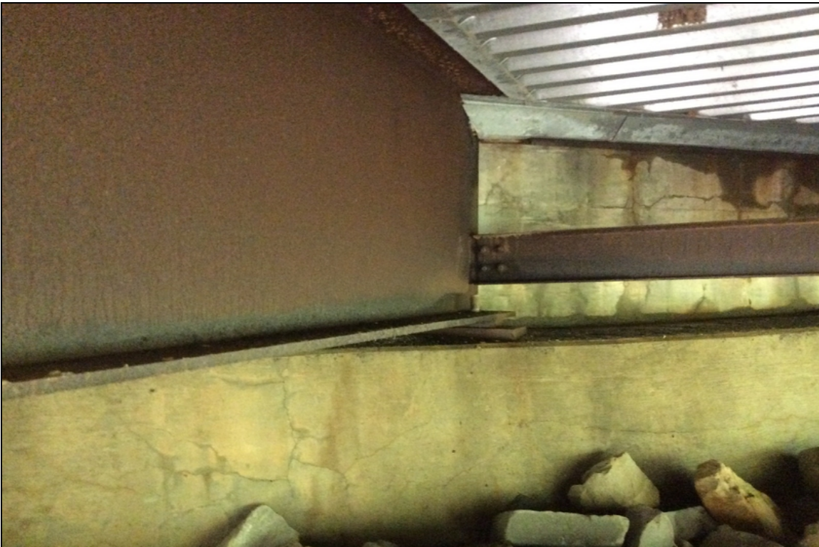
Span 5 abutment 2 girder 2 nut is missing.
