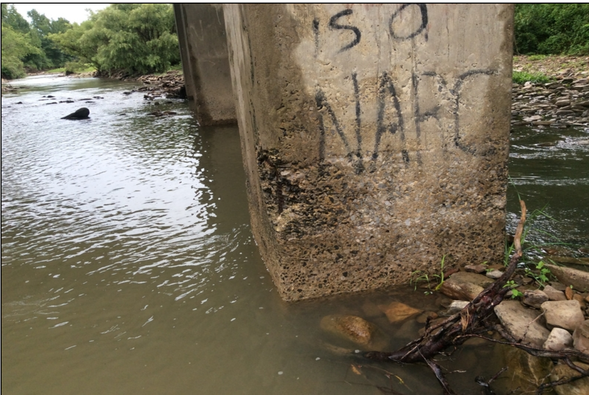
Bent 2 Column 1 ahead side spalling with steel exposed.
