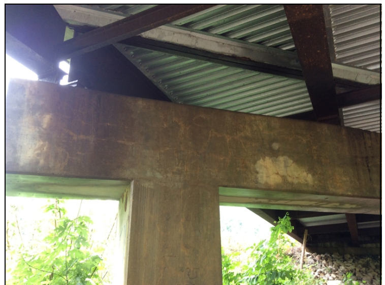
Bent 4 cap mapcracking.
