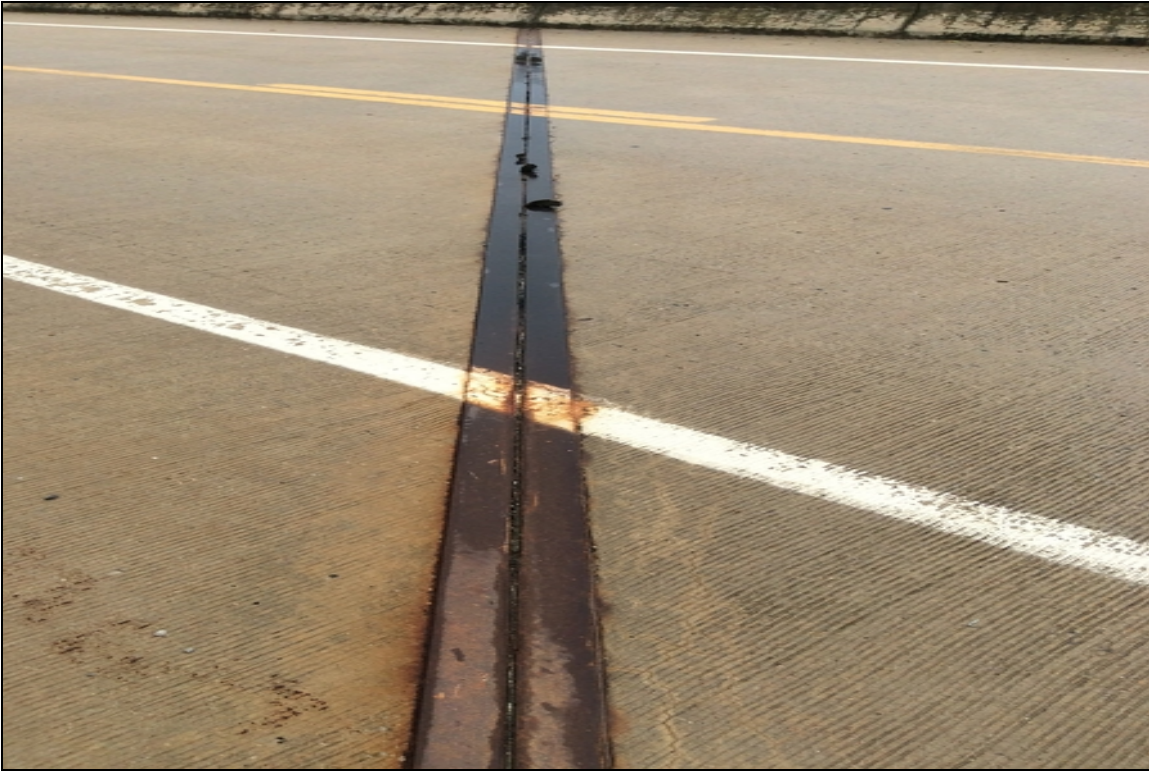
Bent 4 compression joint material being pushed out of joint due to excessive compression.
