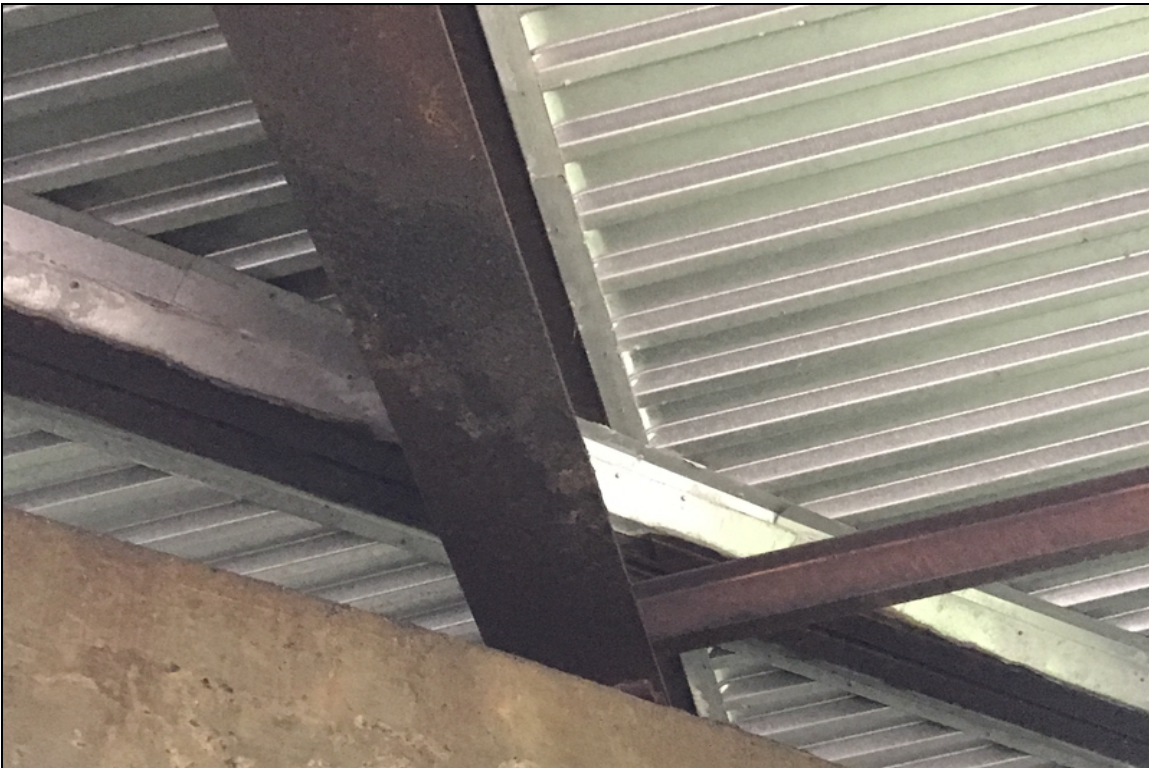
Typical condition of beams ends with minor flaking rust.
