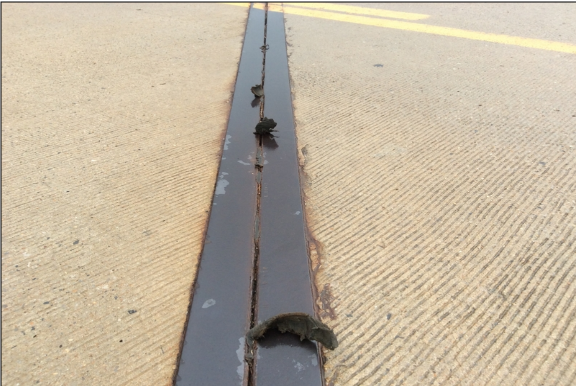
Bent 4 minimal space between road irons.
