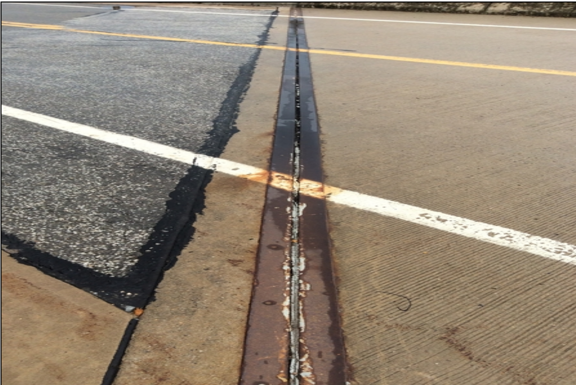
Abutment 2 joint.
