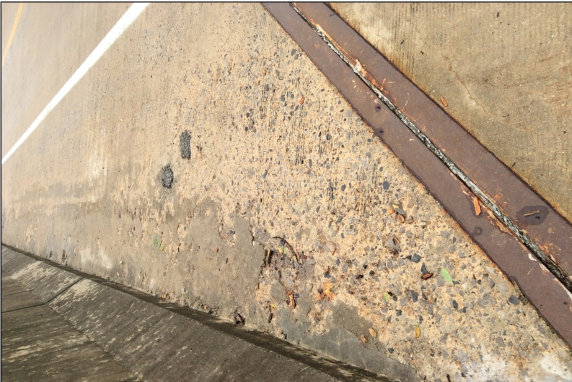
Span 1 right adjacent bent 1 large area of spalling.
