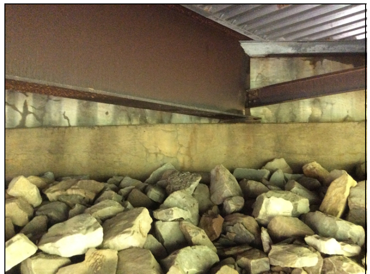
Abutment 2 bridge seat areas of map cracking.
