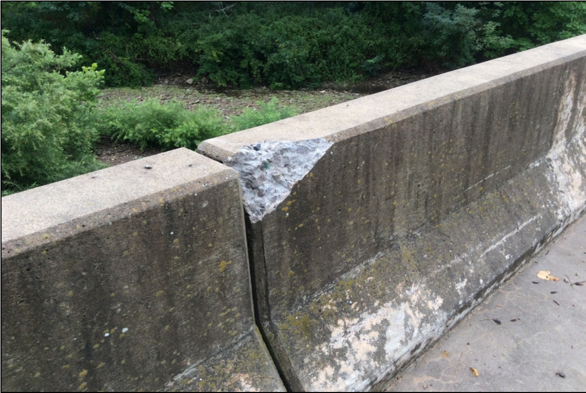
Span 3 right railing adjacent Bent 3 spalling to the top of parapet wall with steel exposed.
