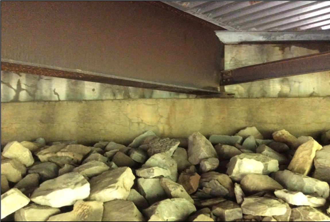
Abutment 2 bridge seat areas of map cracking.
