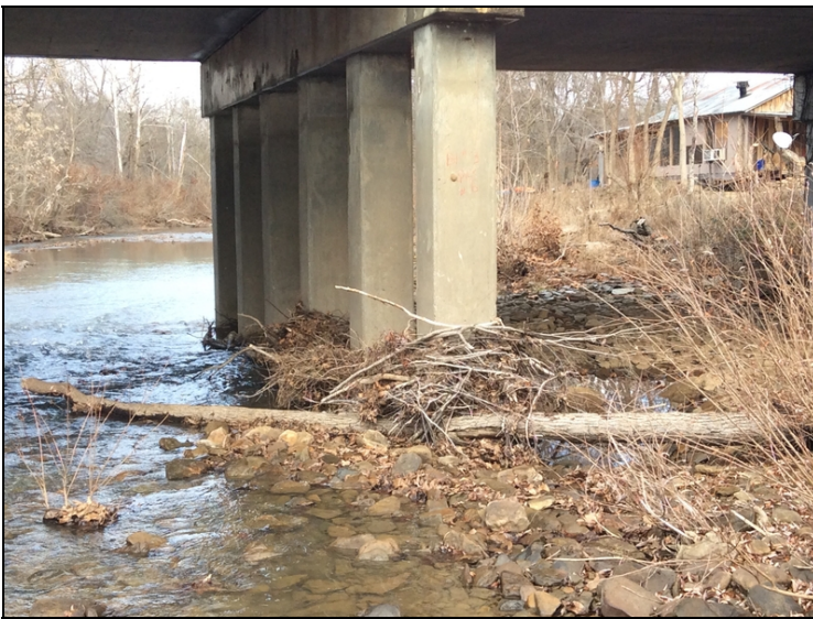
Channel has light drift at bent #3.
