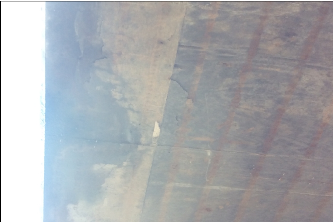
Delaminated area on undersurface of span 4 right side.
