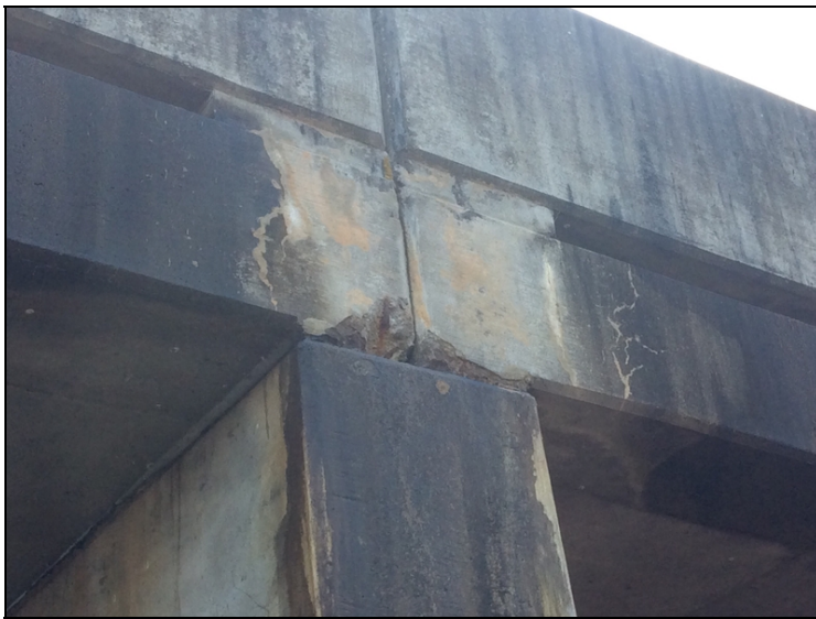
Span #3 has an area of spalling with exposed reinforcing steel to the left exterior face of slab over bent #2.
