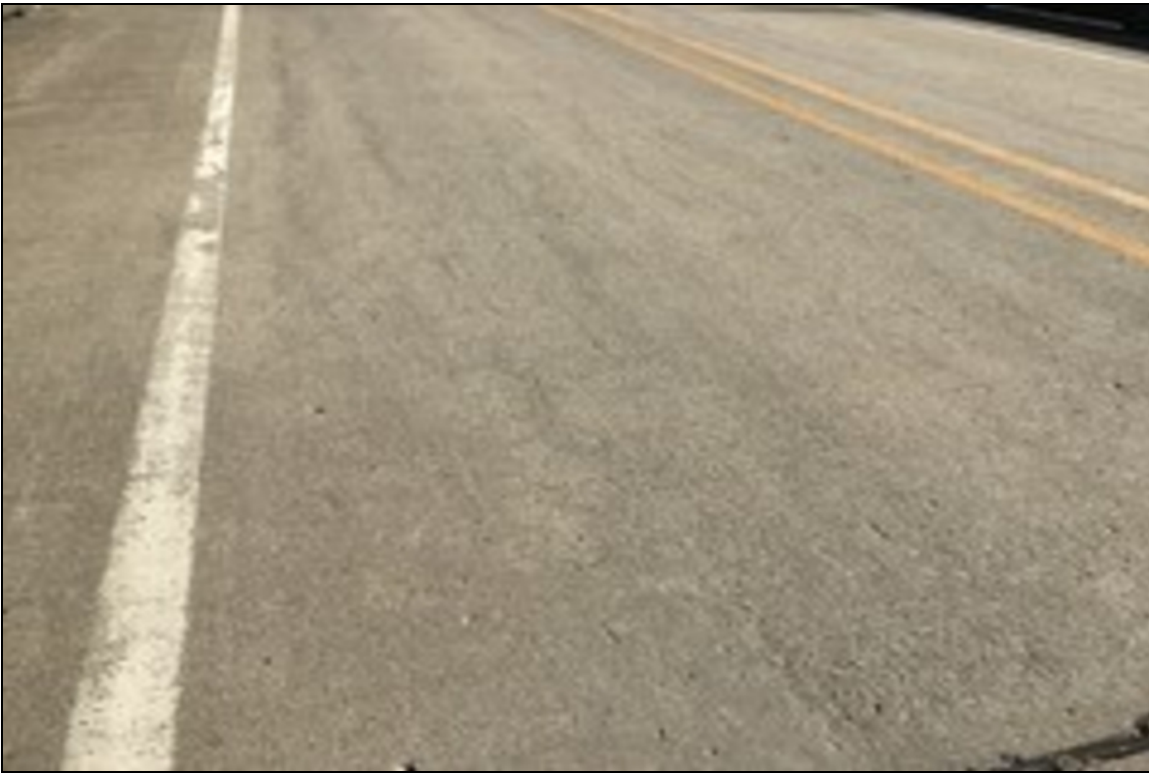
Typical longitudinal deck cracking.
