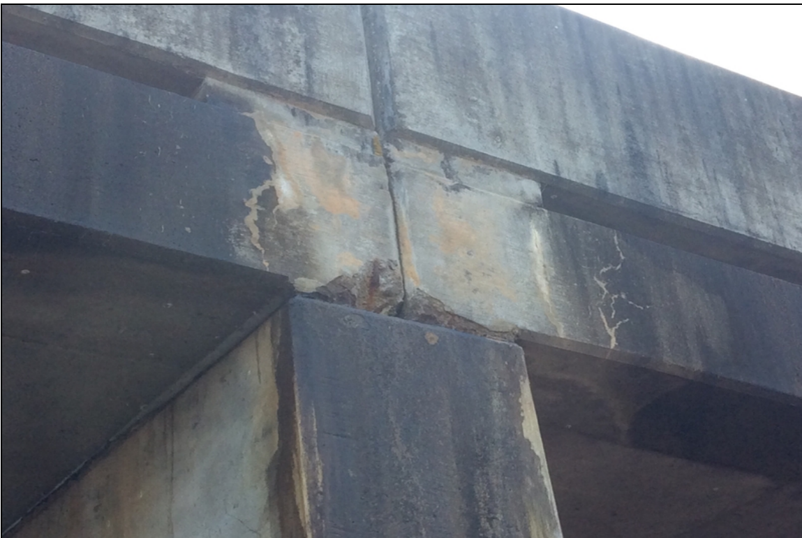
Span 3 over bent 2 spalling to left side with exposed reinforcing steel.
