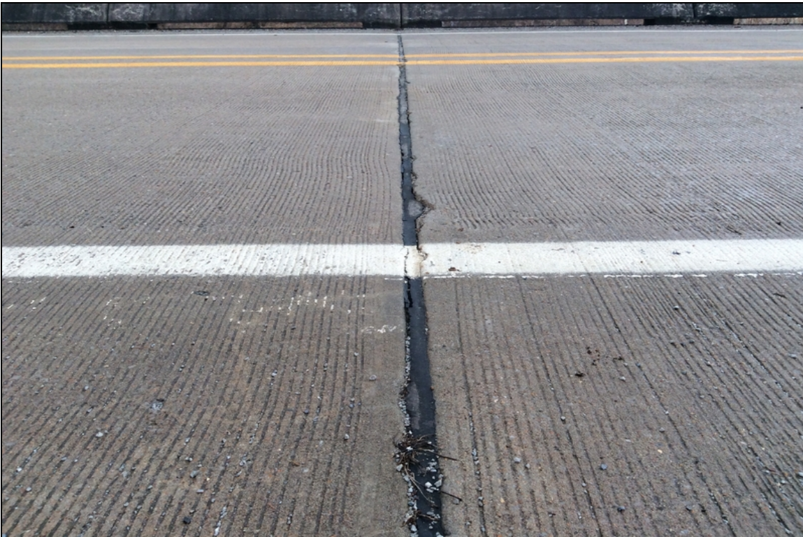
Deck joint seal at bent 1 has
