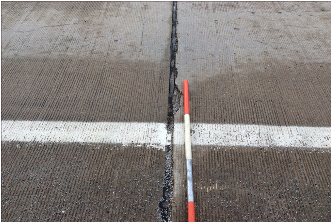
Slab spalled areas along expansion joints.
