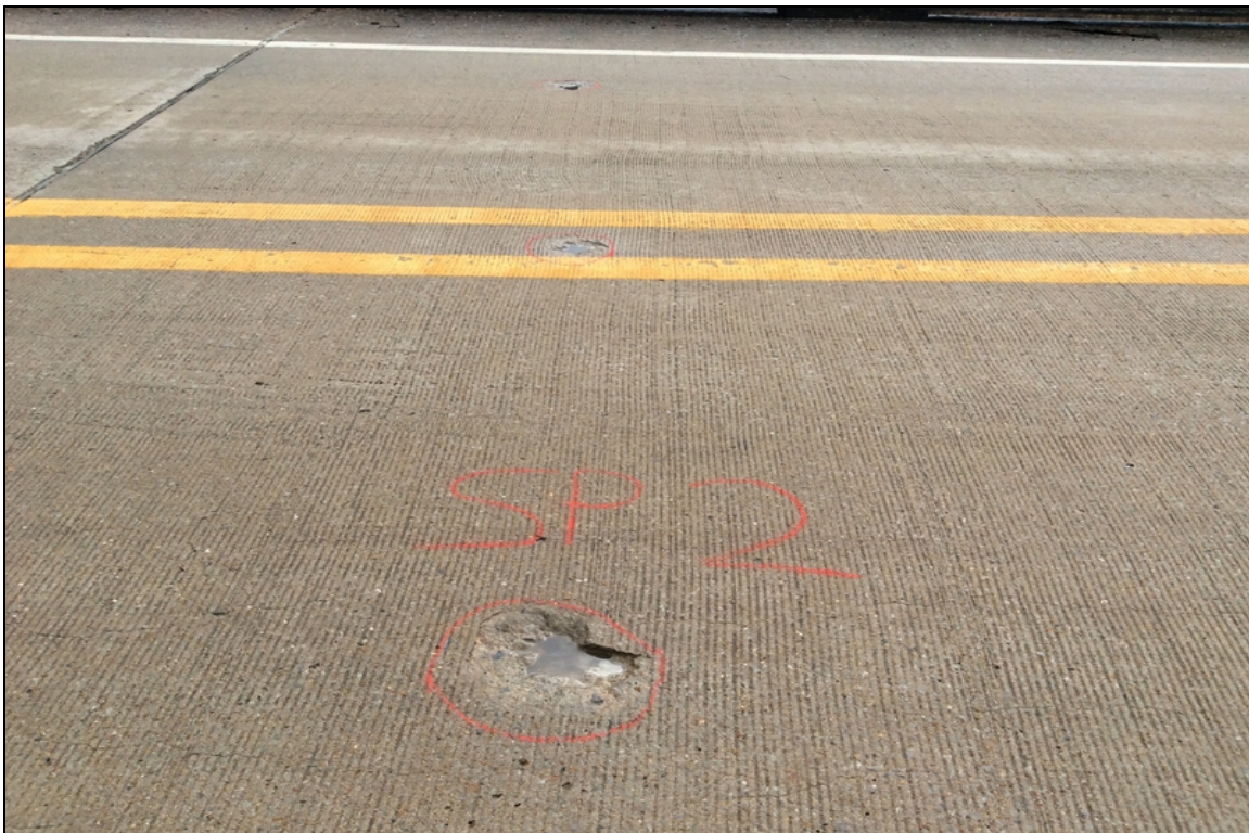
Span 2 spalling approximately 5' from bent 2.
