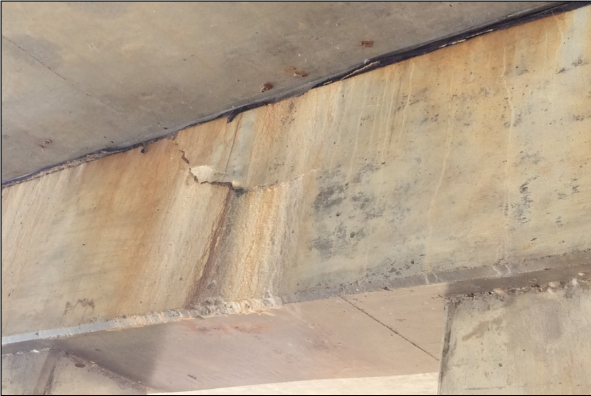
Bent 2 cap ahead side delaminated area in bay 4.
