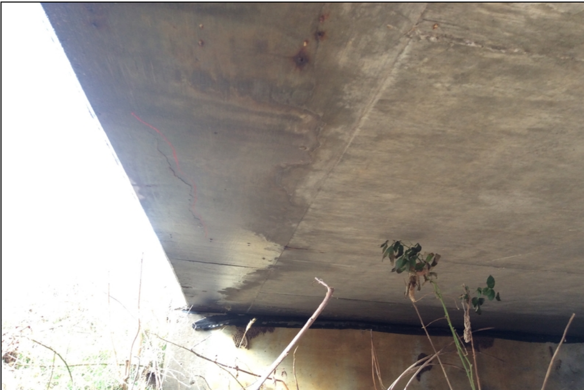
Longitudinal cracking in undersurface span 1 right side.
