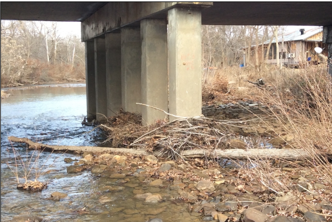
Channel has light drift at bent 3
