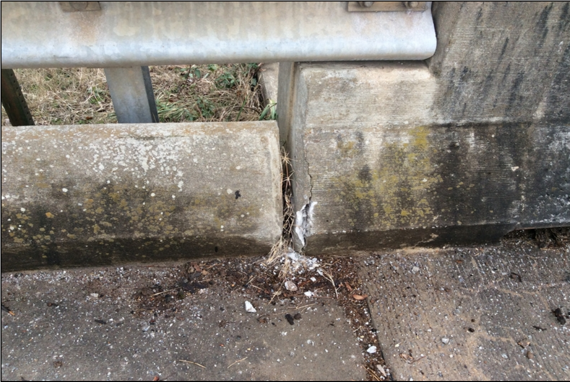
Spall at abutment 2 right side of bridge railing
