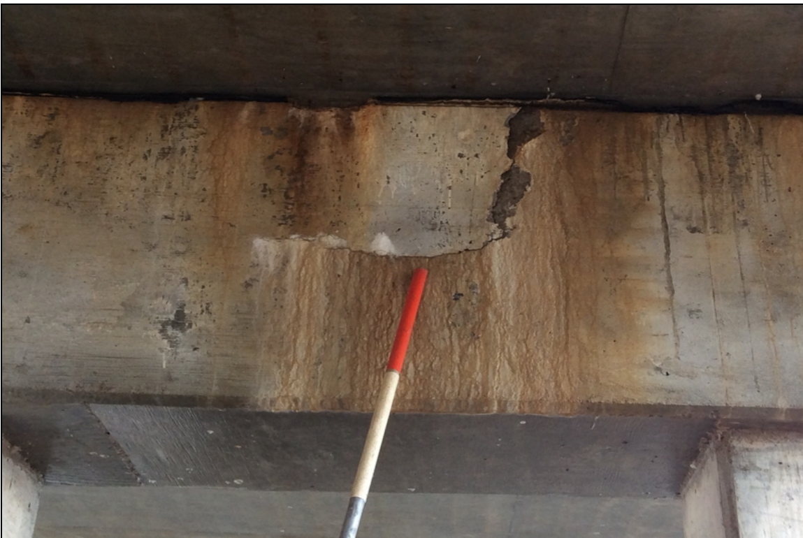
-Bent3 cap ahead side delaminated area in bay 2
