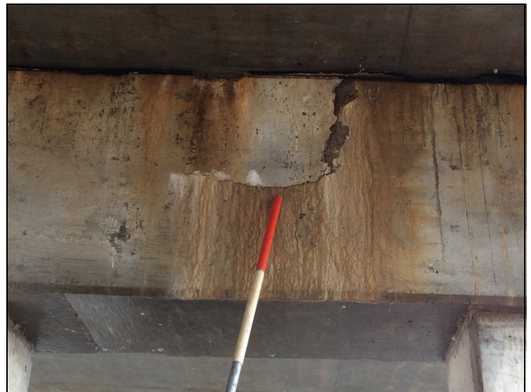
-Bent3 cap ahead side delaminated area in bay 2
