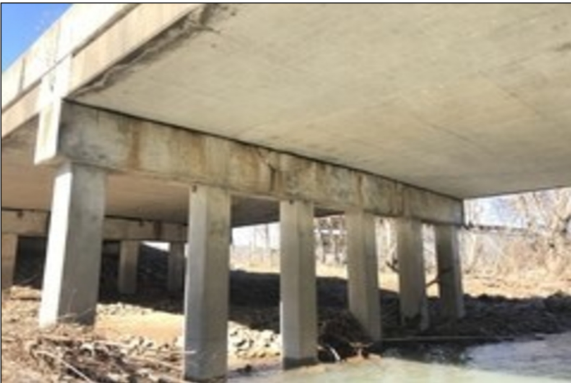
Bent #2 cap ahead side delaminated area around Keyways.
