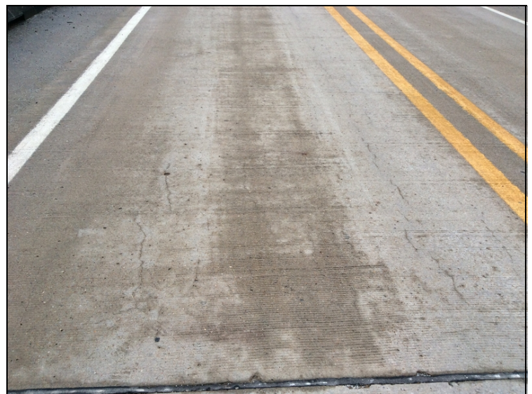
Typical of deck cracking in all spans.
