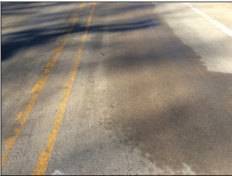
Deck - sealable longitudinal cracks located in the driving surface.
