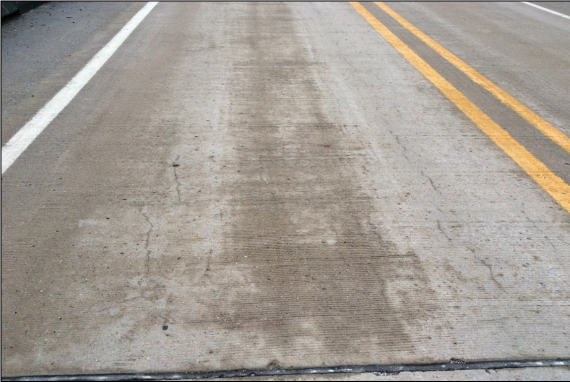
General view of deck cracking
