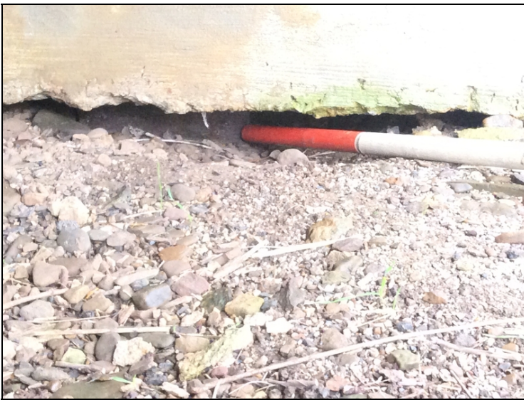
Abutment 1, Left side-piling exposed.
