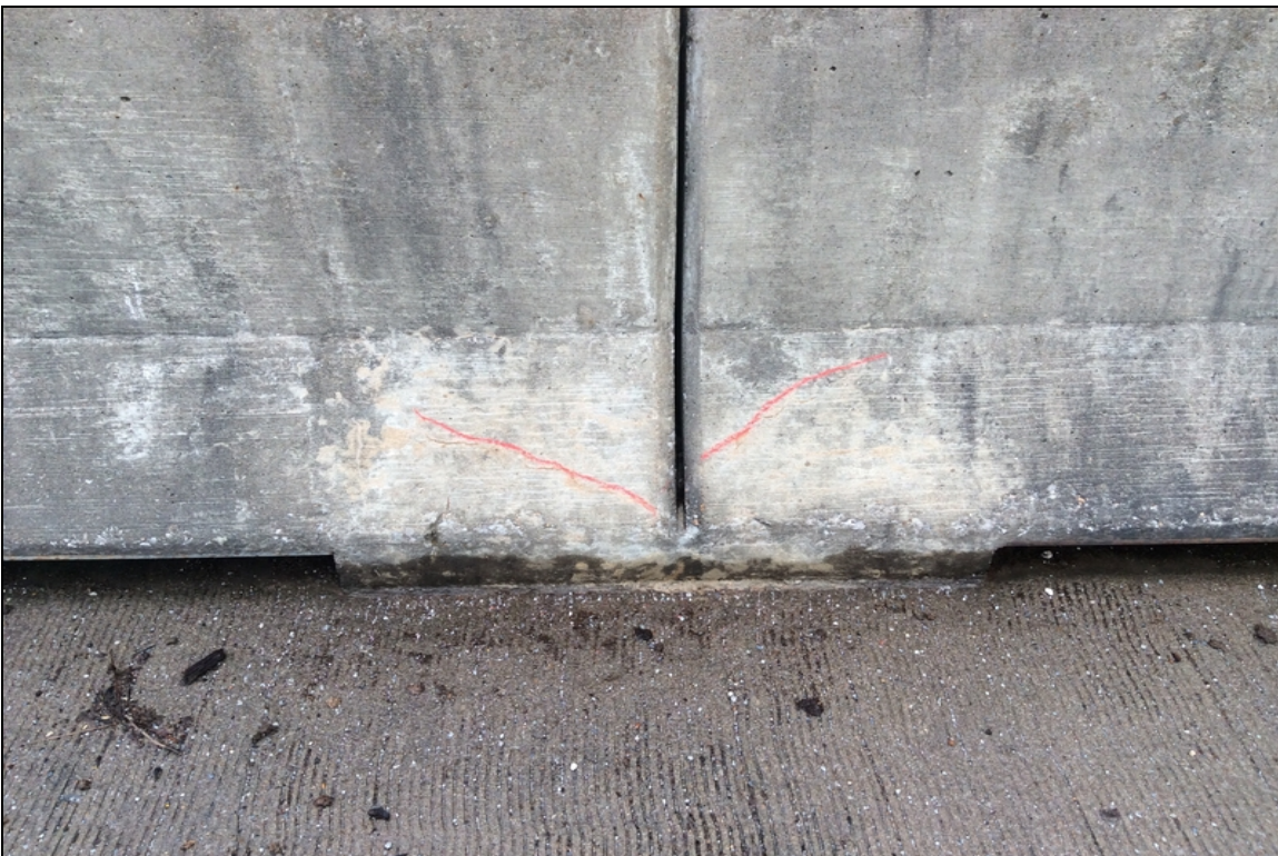
Cracking
