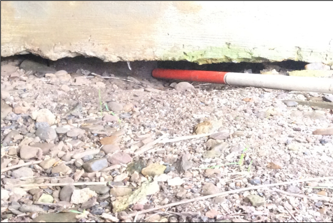
Abutment 1, Left side-piling exposed.
