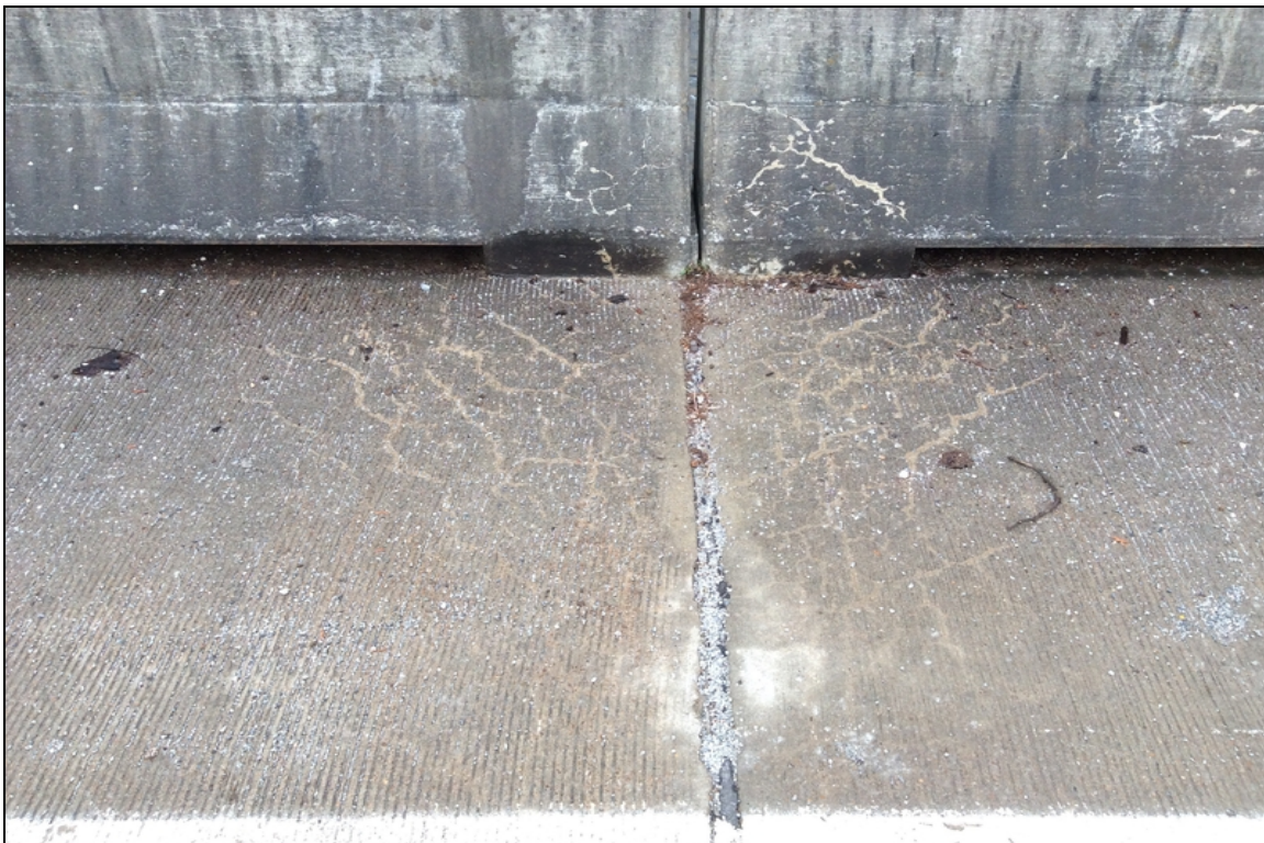
General view of map cracking
