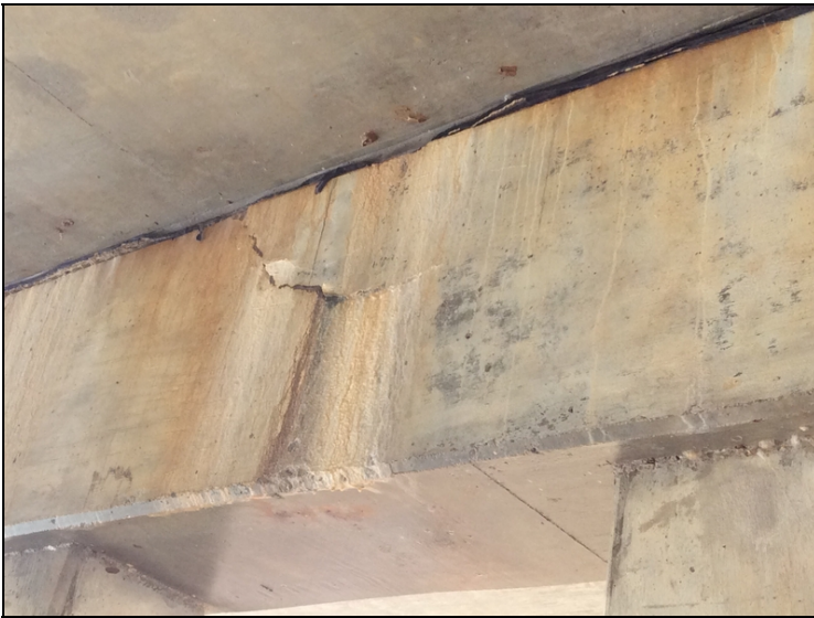
Bent 2 cap ahead side delaminated area in bay 4.
