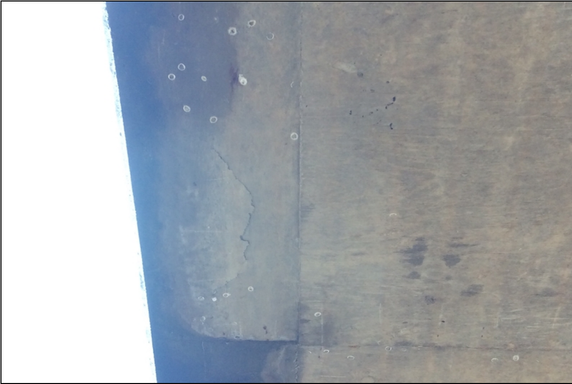
Span 3 Left side delaminated area in undersurface
