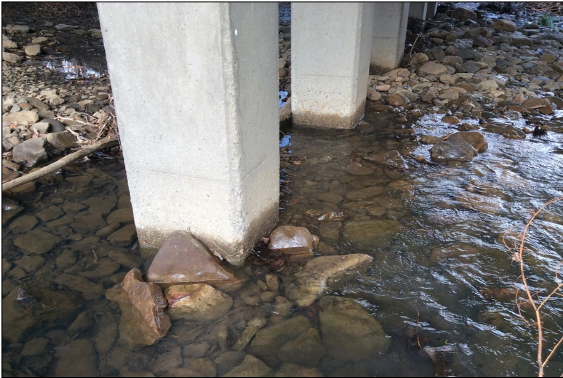
Abrasion at bent 2
