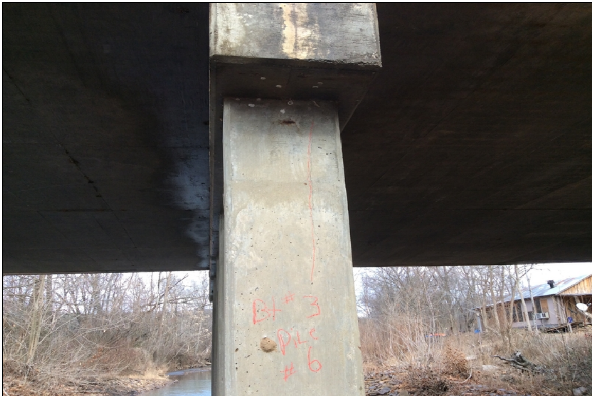
Concrete coating for pile 6 bent 3 has vertical cracking in top.
