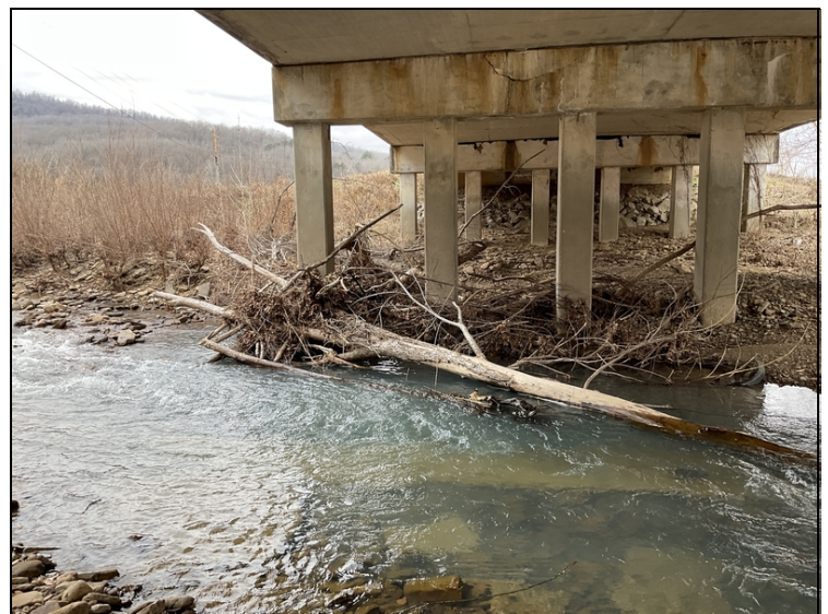
Drift has accumulated at bent #2 causing localized scour.
