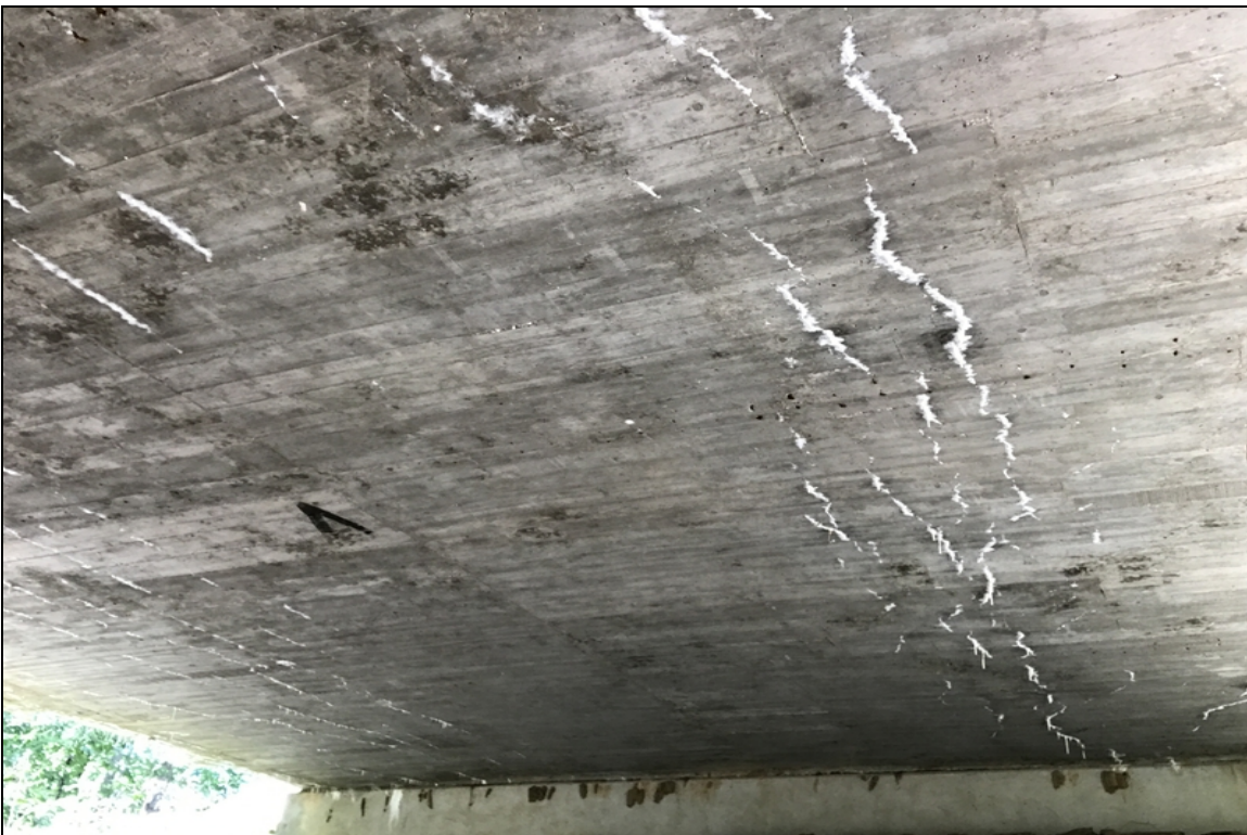
Span 1 typical cracking with efflorescence.
