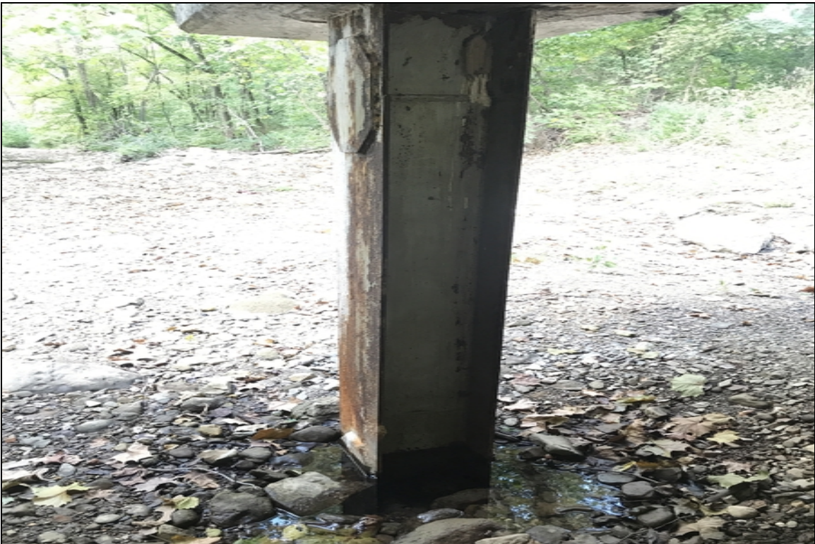
Typical repair to steel piling.
