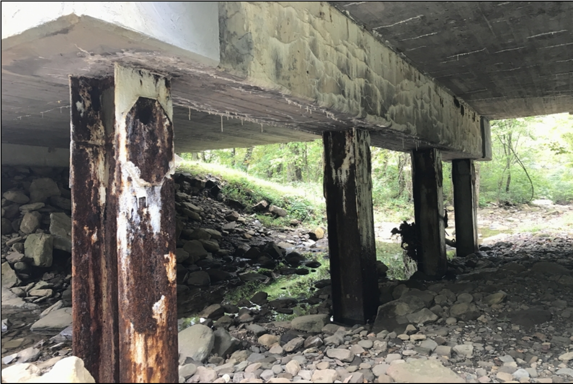
Typical view of steel piling and cap at bent #1.
