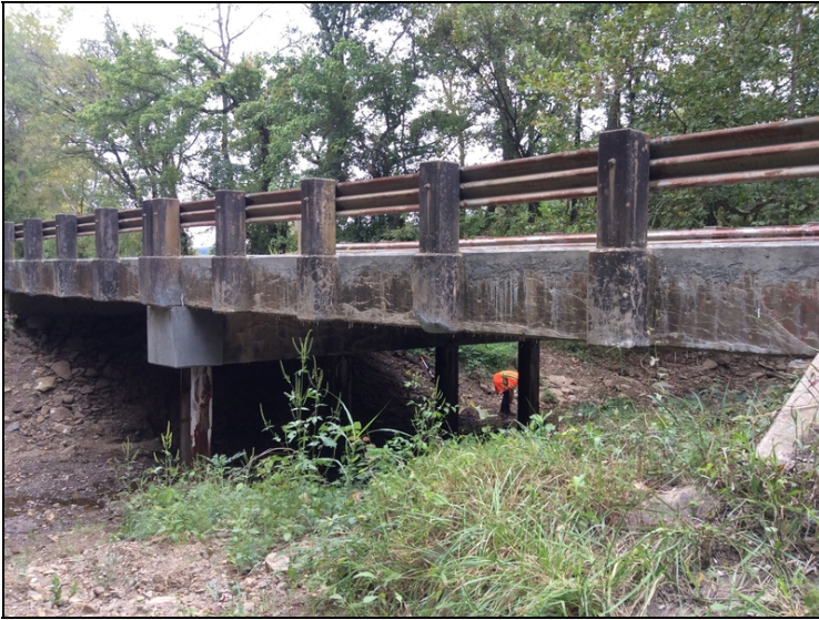
General view of side of bridge showing cracking and efflorescence.
