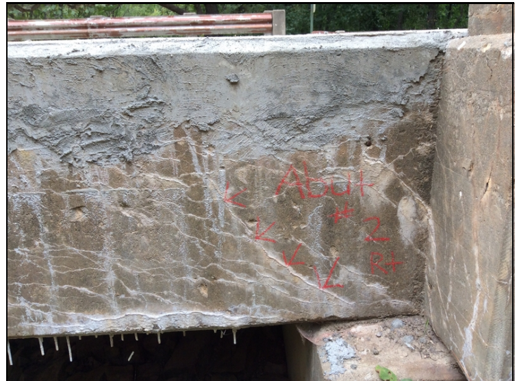
Right side of deck at abutment #2 - shear type crack.
