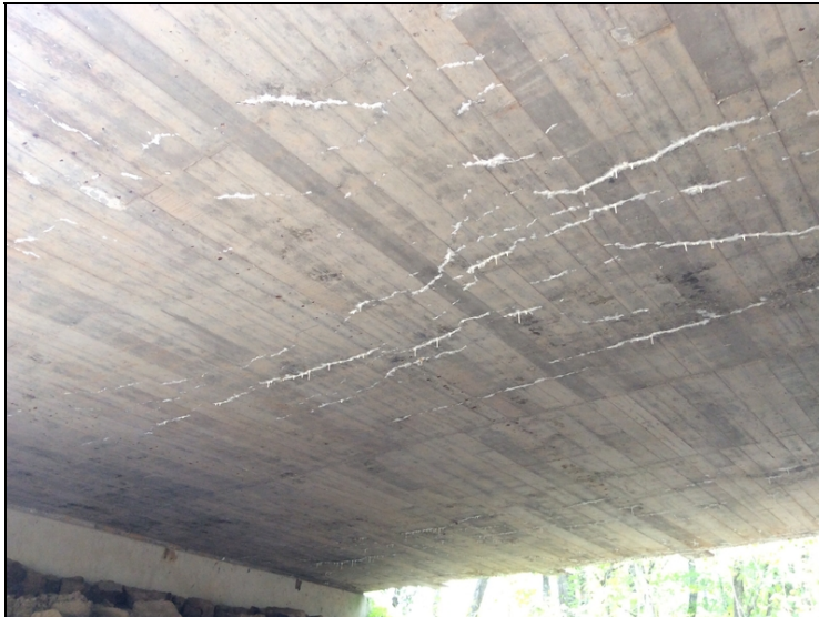
Deck undersurface Span #1 typical view of cracking with efflorescence.
