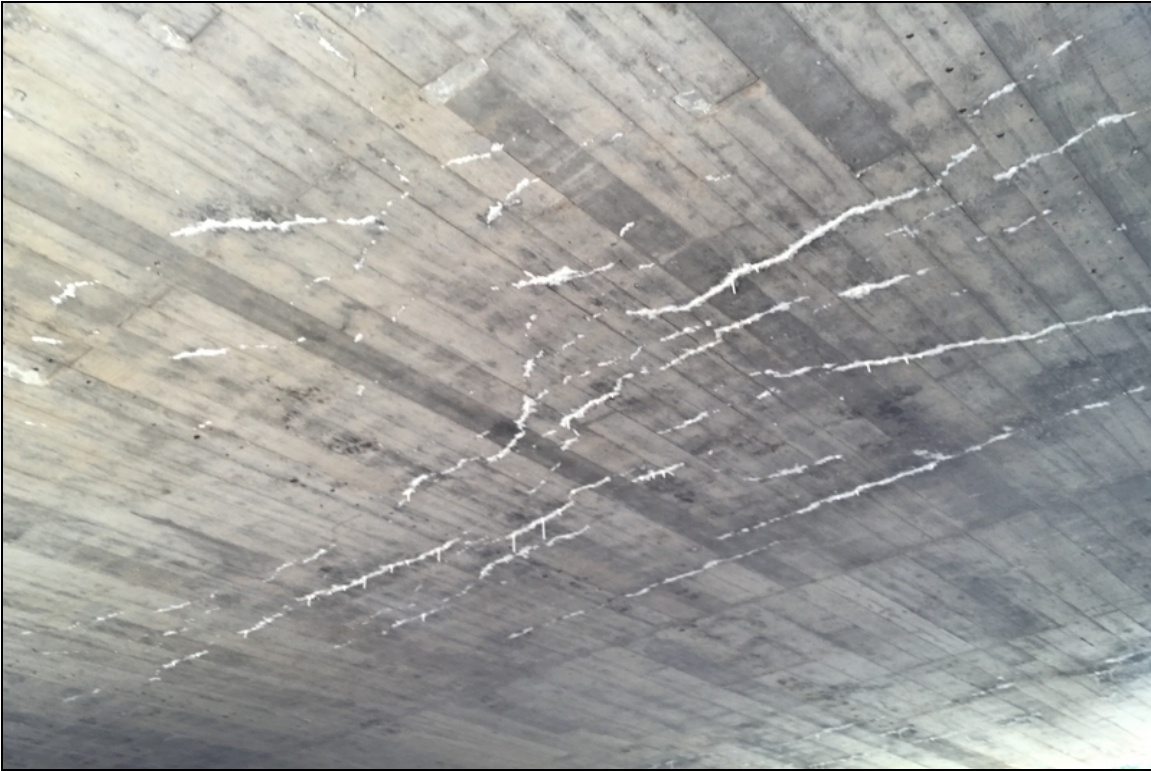
Span 1 typical cracking with efflorescence.
