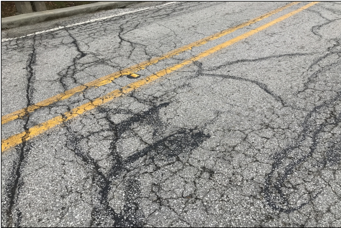
Typical cracking of asphalt wearing surface.
