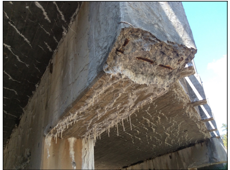
Spalling with exposed reinforcing steel in cap.
