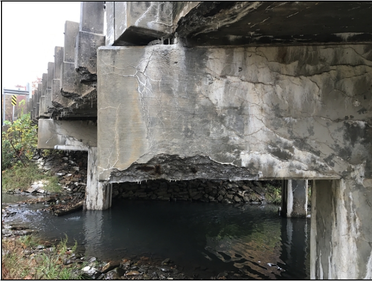
Bent #2 left behind side spalling with steel exposed.
