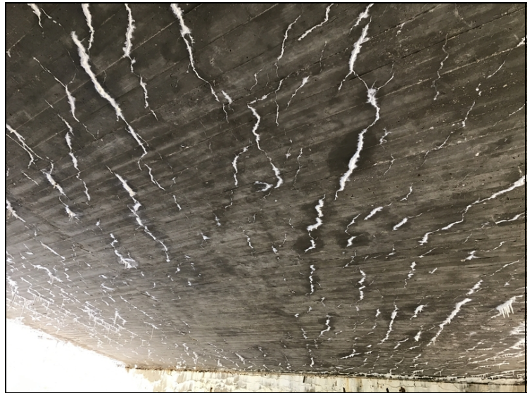
Span #2 typical view of efflorescence and and cracking to undersurface of deck.
