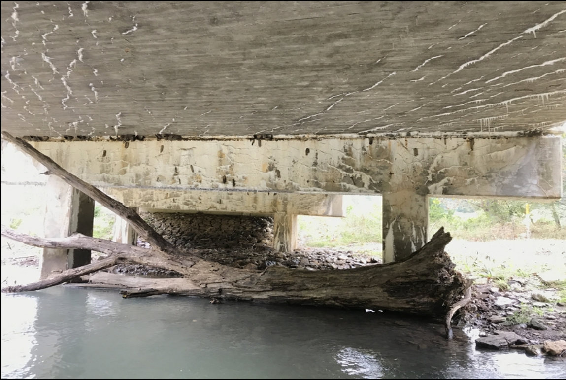
Bent #2 large tree drift accumulation.
