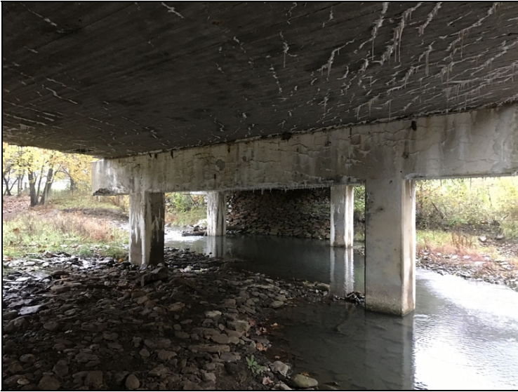
Bent #2 behind side Cracking with heavy efflorescence.
