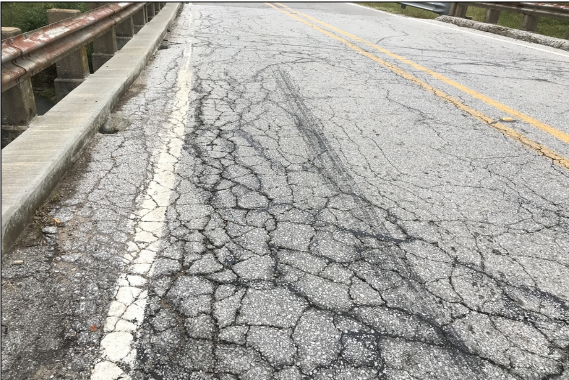
Asphalt wearing surface left lanes has almost rubblized due to traffic.
