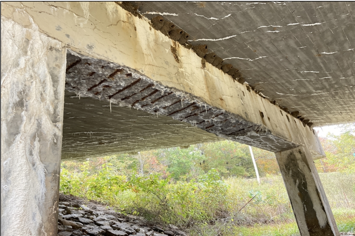
View of bent #3 cap underneath steel exposed.
