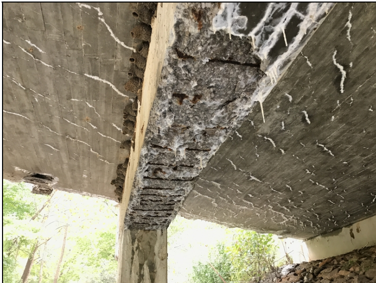
Bent #3 cap underneath deep spalling with steel exposed.
