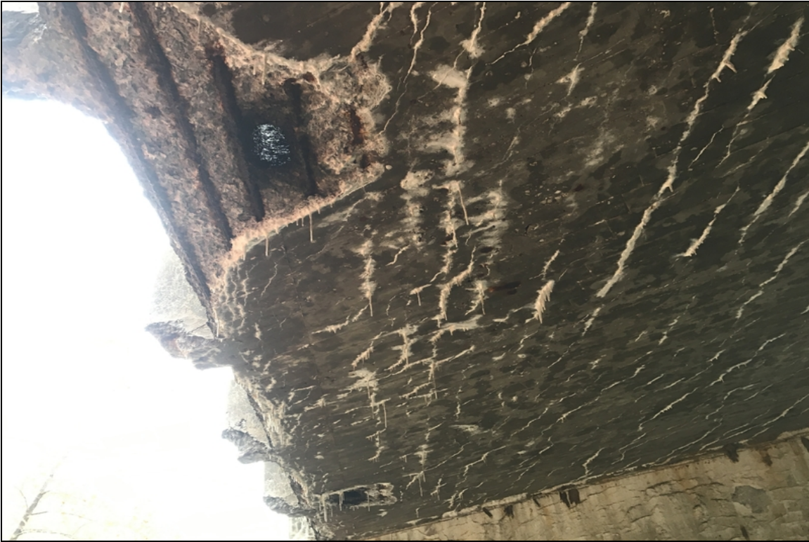
Span #2 left side steel exposed around drains.
