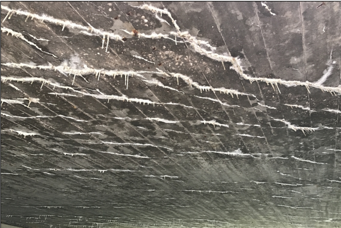
View of Span #4 undersurface.
