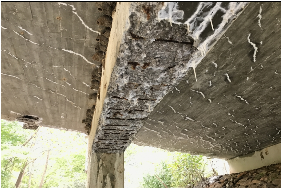
Bent #3 cap underneath deep spalling with steel exposed.
