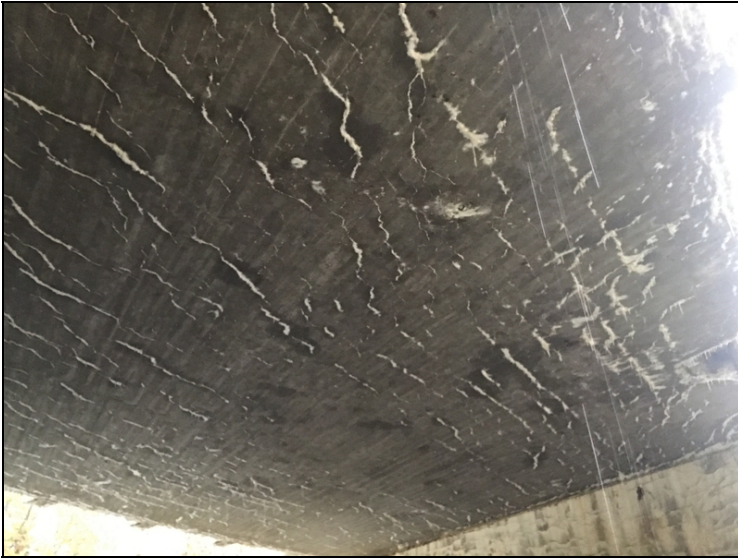
Span #2 cracking with efflorescence.
