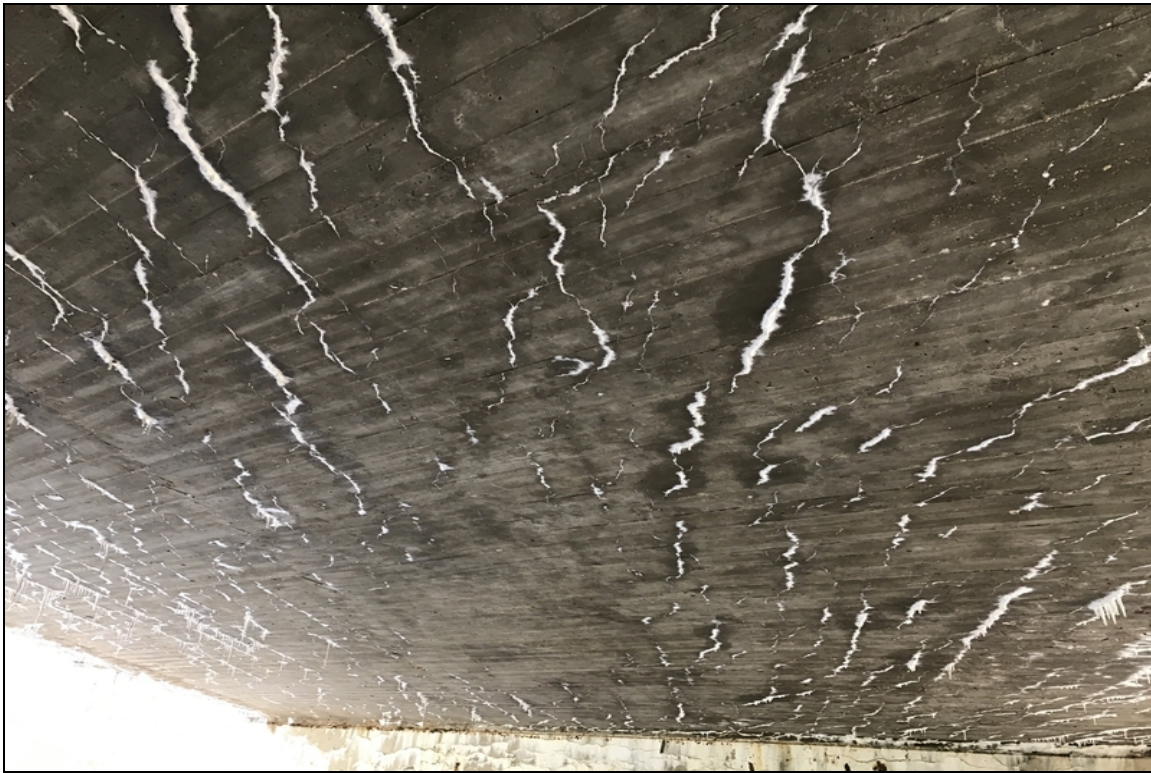
Span #2 typical view of efflorescence and cracking to undersurface of deck.
