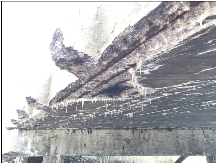
Span #2 left side typical steel exposed around deck drains and left edge
