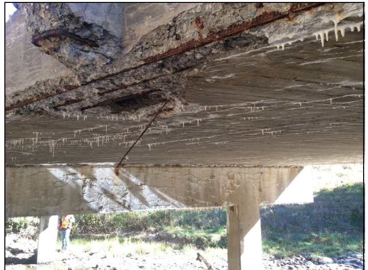
Soffit span 2 left - heavy cracking with efflorescence and spalling with exposed reinforcing steel around drain.
