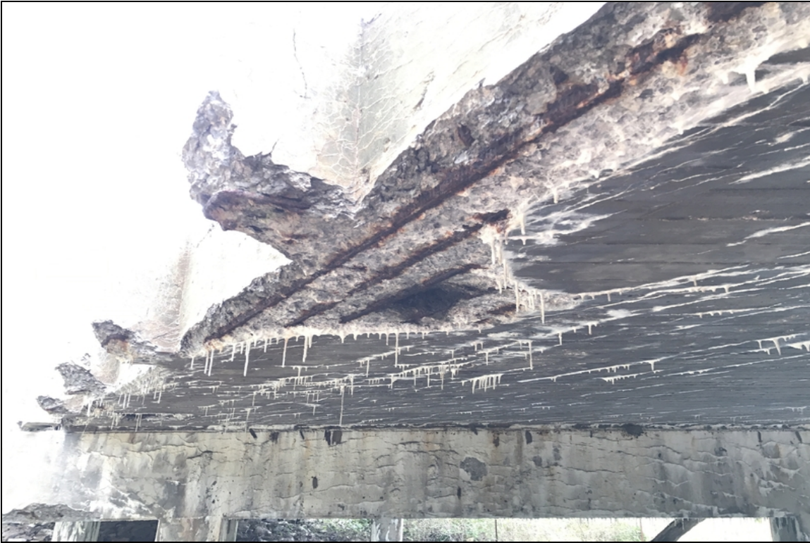
Span #2 left side typical steel exposed around deck drains and left edge
