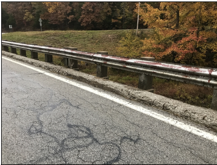
Concrete curb right spalling with steel exposed.
