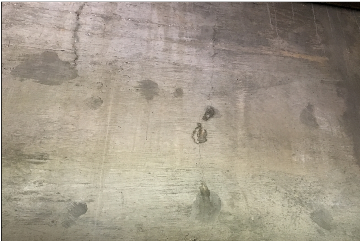
Bay #4 vertical face of backwall typical vertical cracking.
