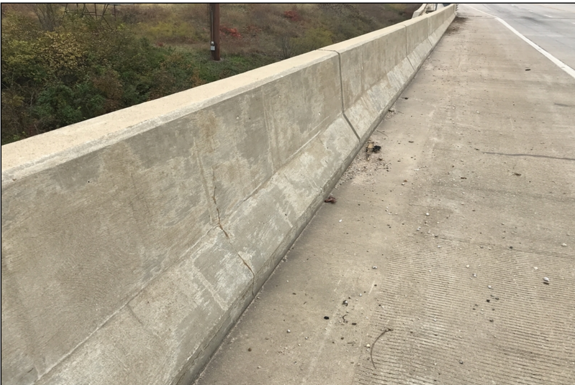
Left parapet vertical cracking
