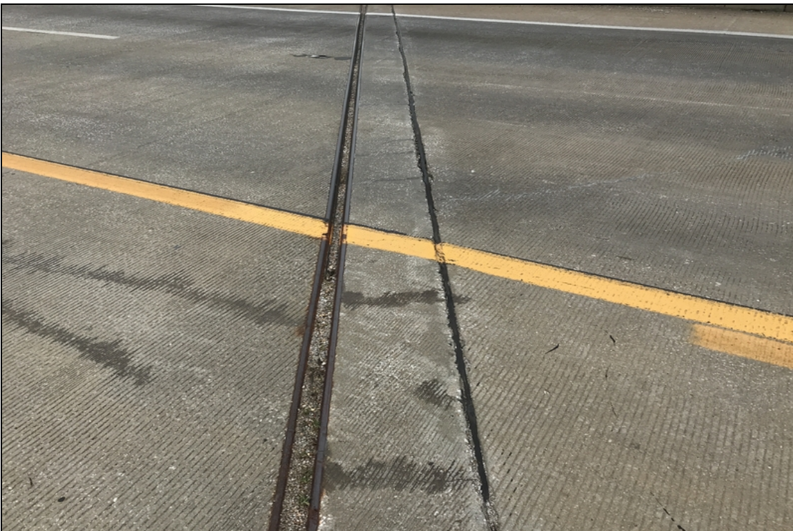
Top of abutment #1 backwall has sealed cracking.
