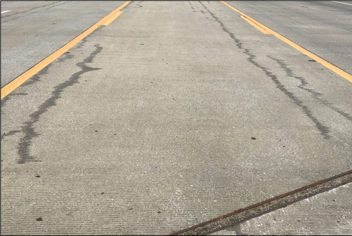
Turning lane typical view of sealed cracking .
