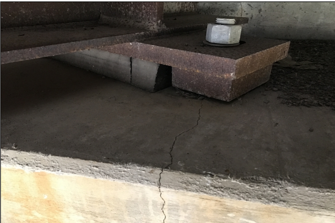
Wide cracking in bridge seat propagating from anchor bolt at bearing #5.
