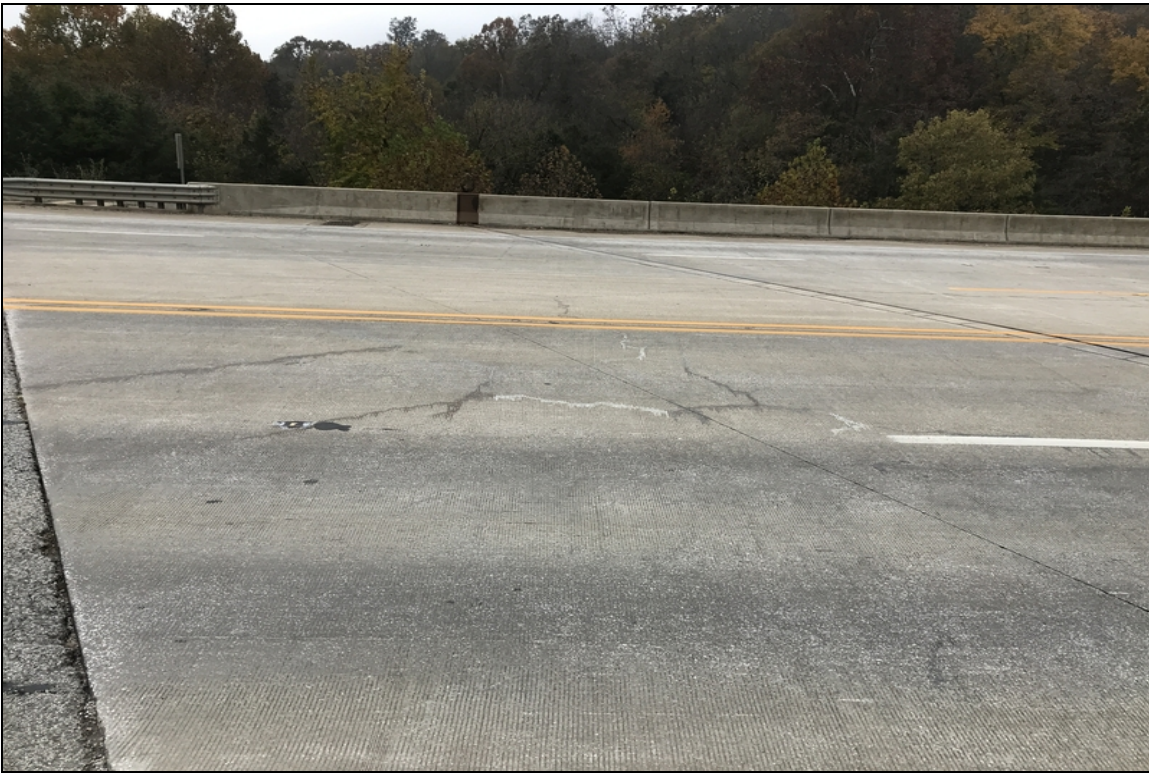
View of sealed cracking in south approach slab
