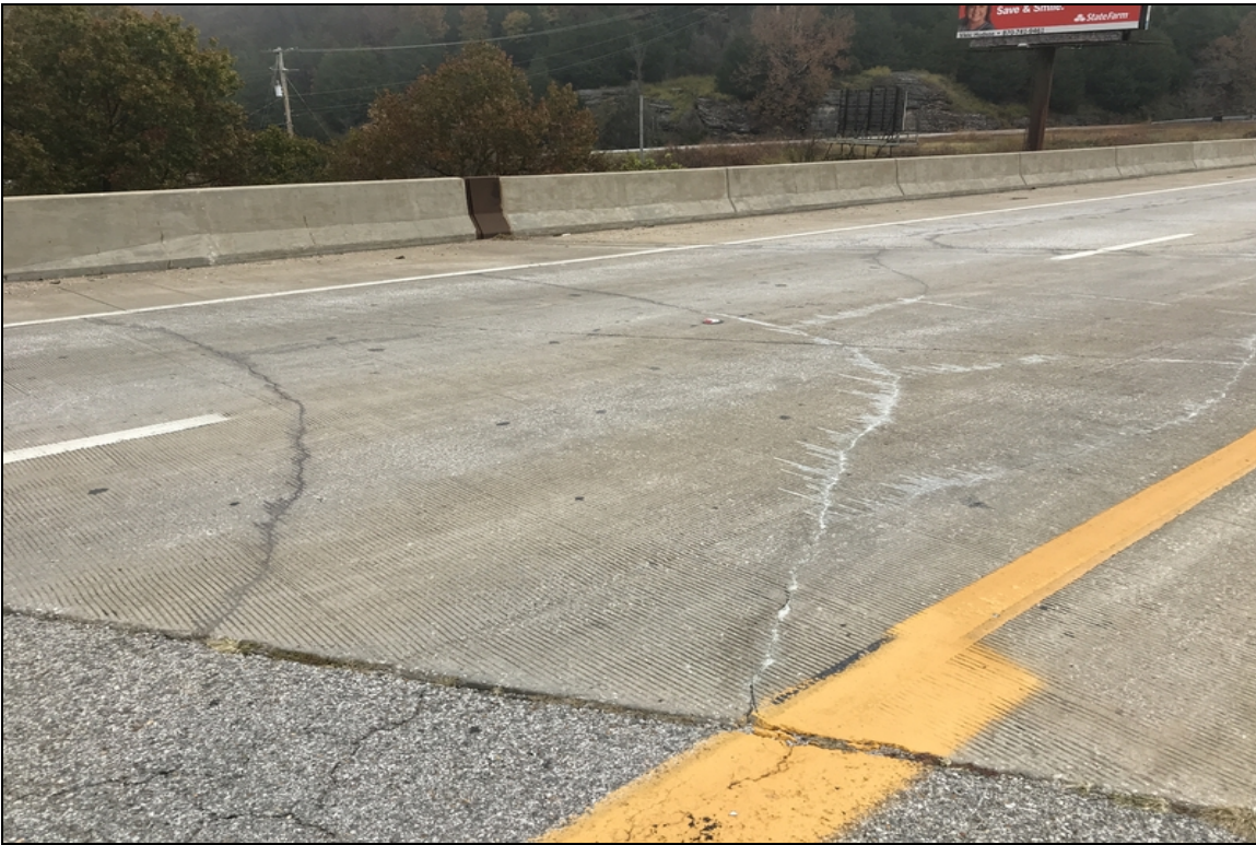
Cracking in north approach slab in the north bound lanes has been sealed.
