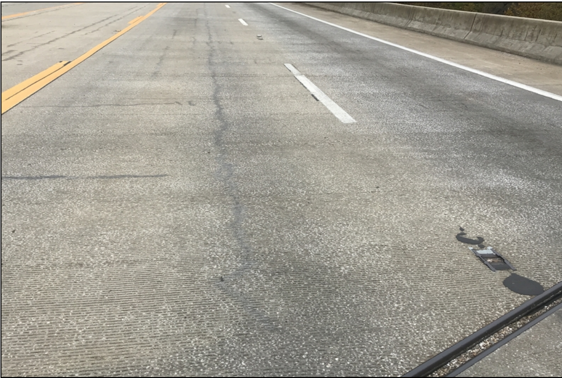
South bound lanes typical view of sealed cracking .
