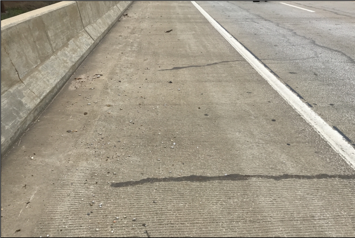
Left gutter line typical sealed cracking.
