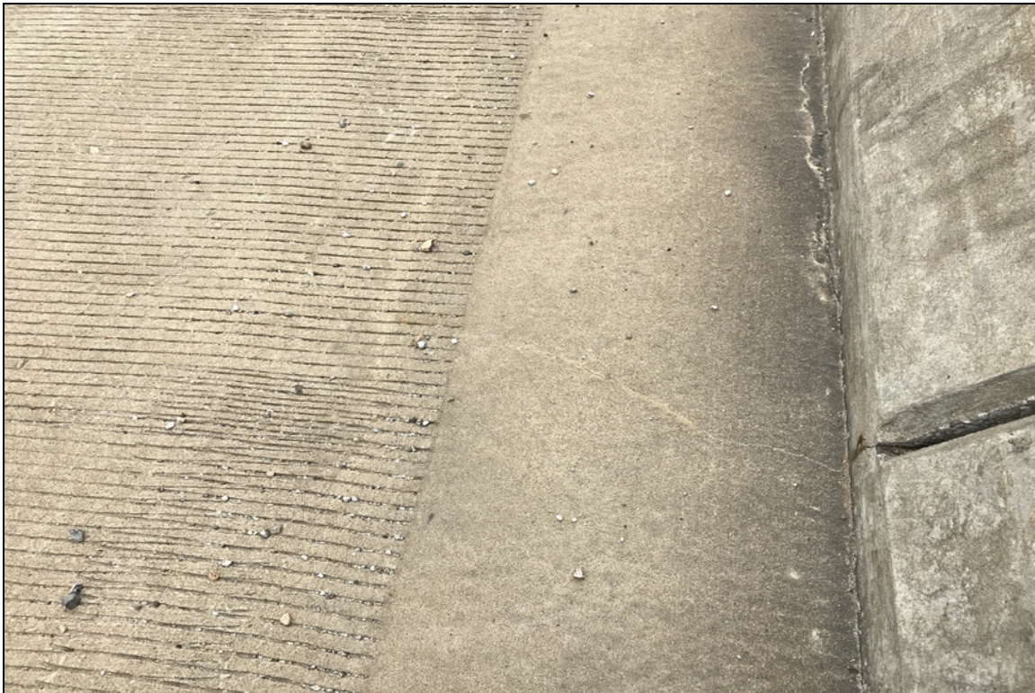
Typical cracking in left and right gutterlines.
