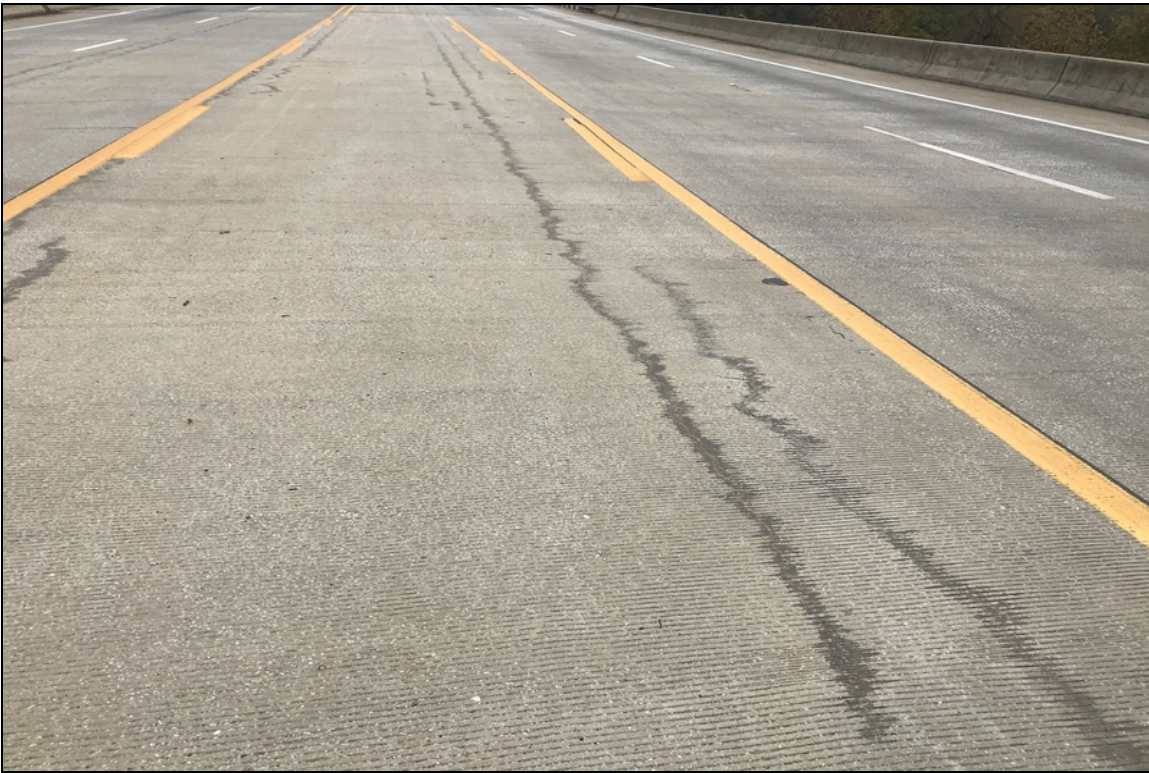
Deck driving surface has sealed full length longitudinal cracking.
