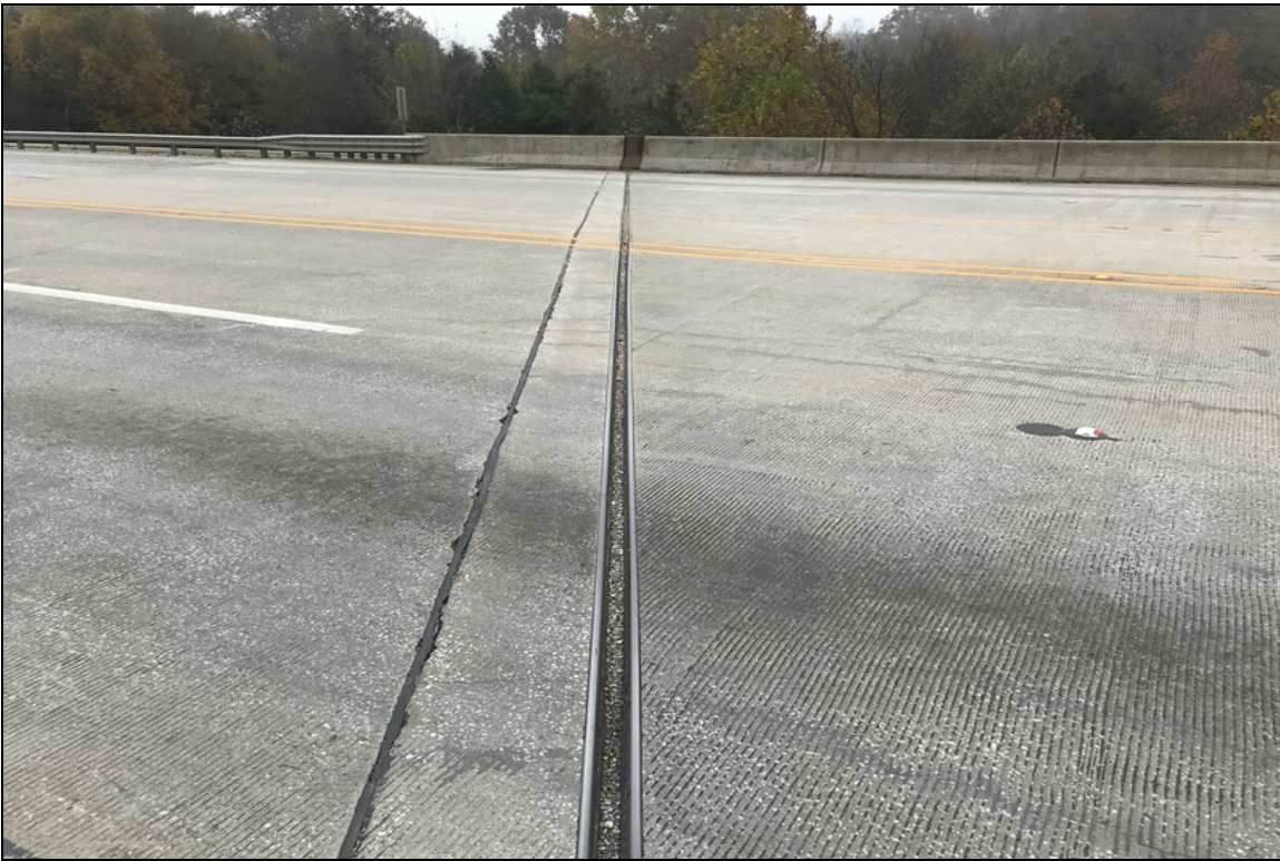
Abutment #2 compression joint seal debris impaction.
