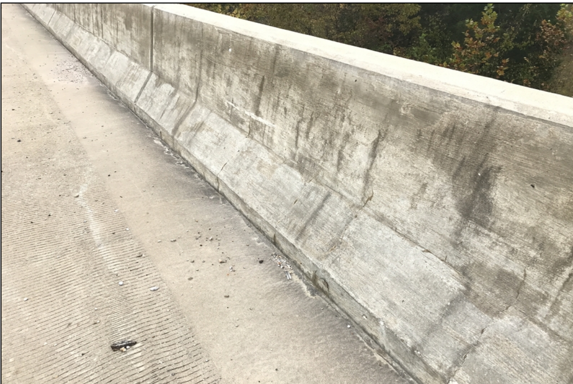
Right parapet wall has vertical cracking.
