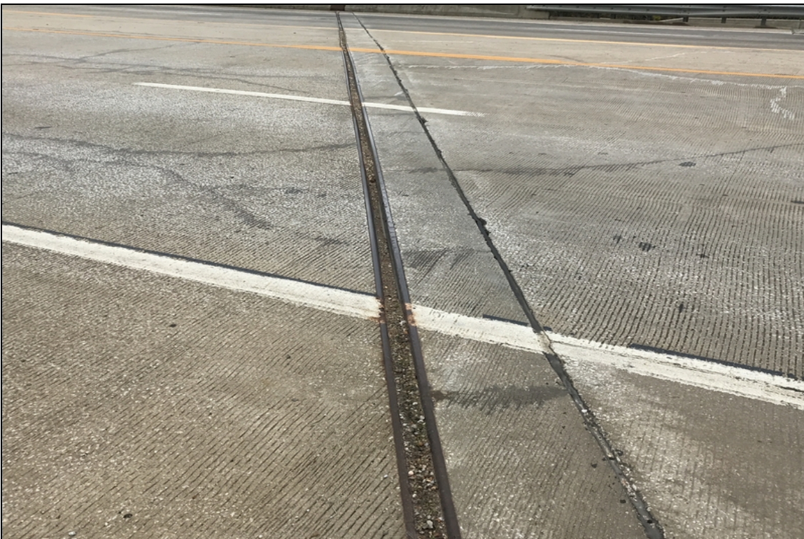
Debris impaction to joint seal at abutment #1.
