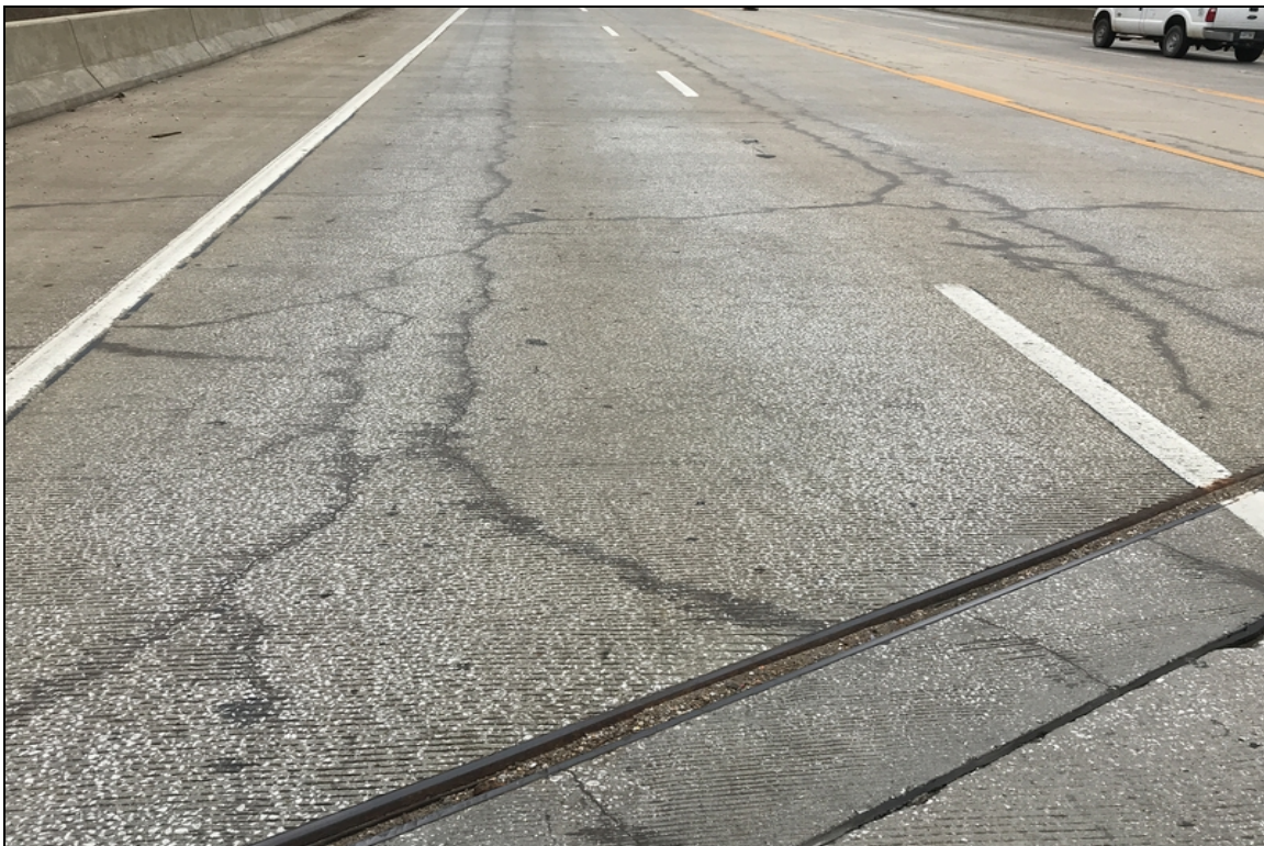
Northbound lanes typical view of sealed cracking .
