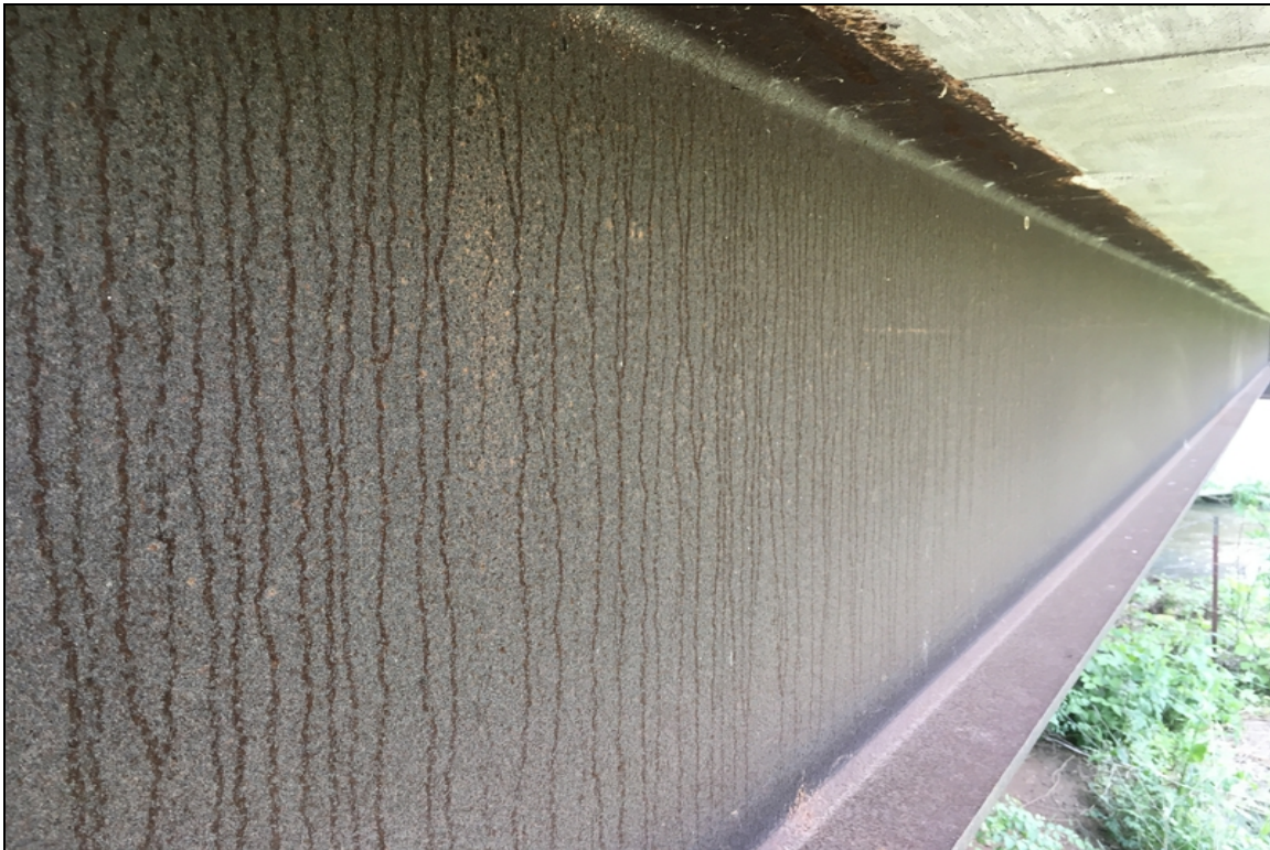
Typical weathering steel protective coating condition.
