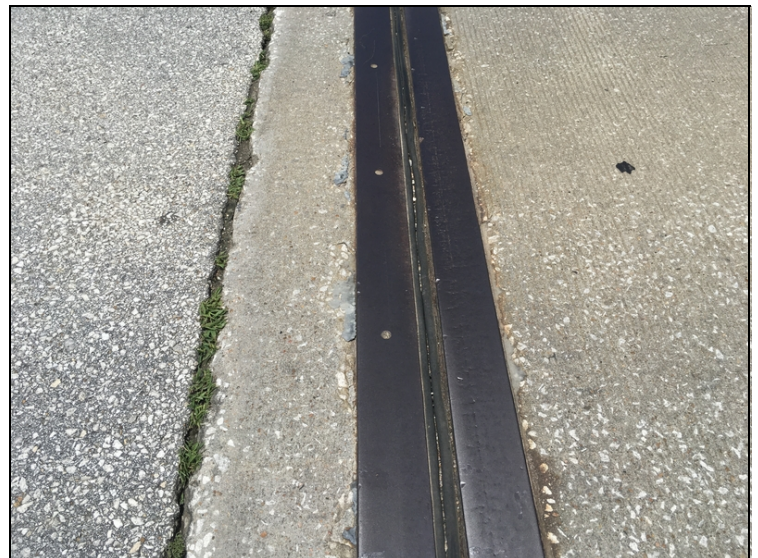
Abutment 1 joint seal showing pack rust.
