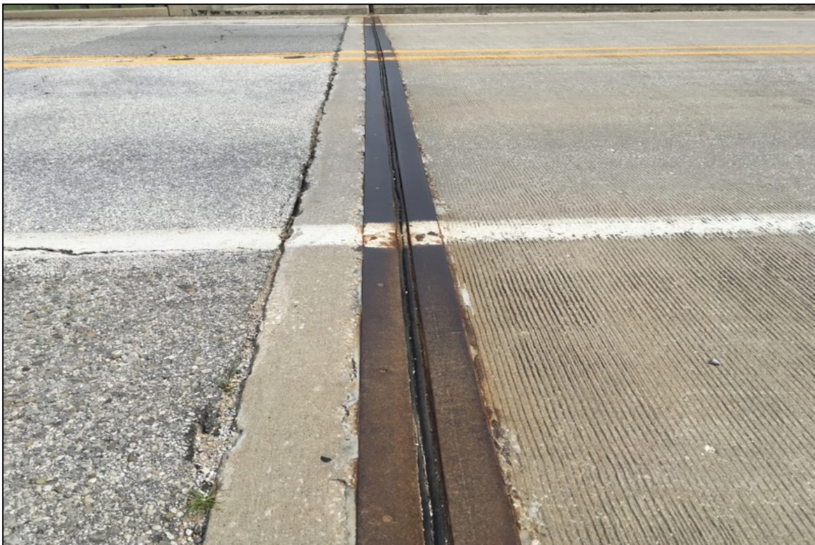
Condition of compression joint seal at abutment #1.
