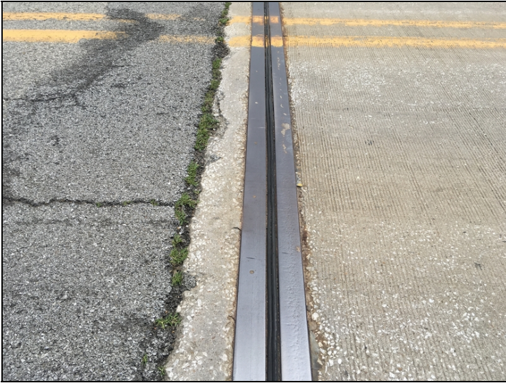
Abutment 2 joint seal condition.
