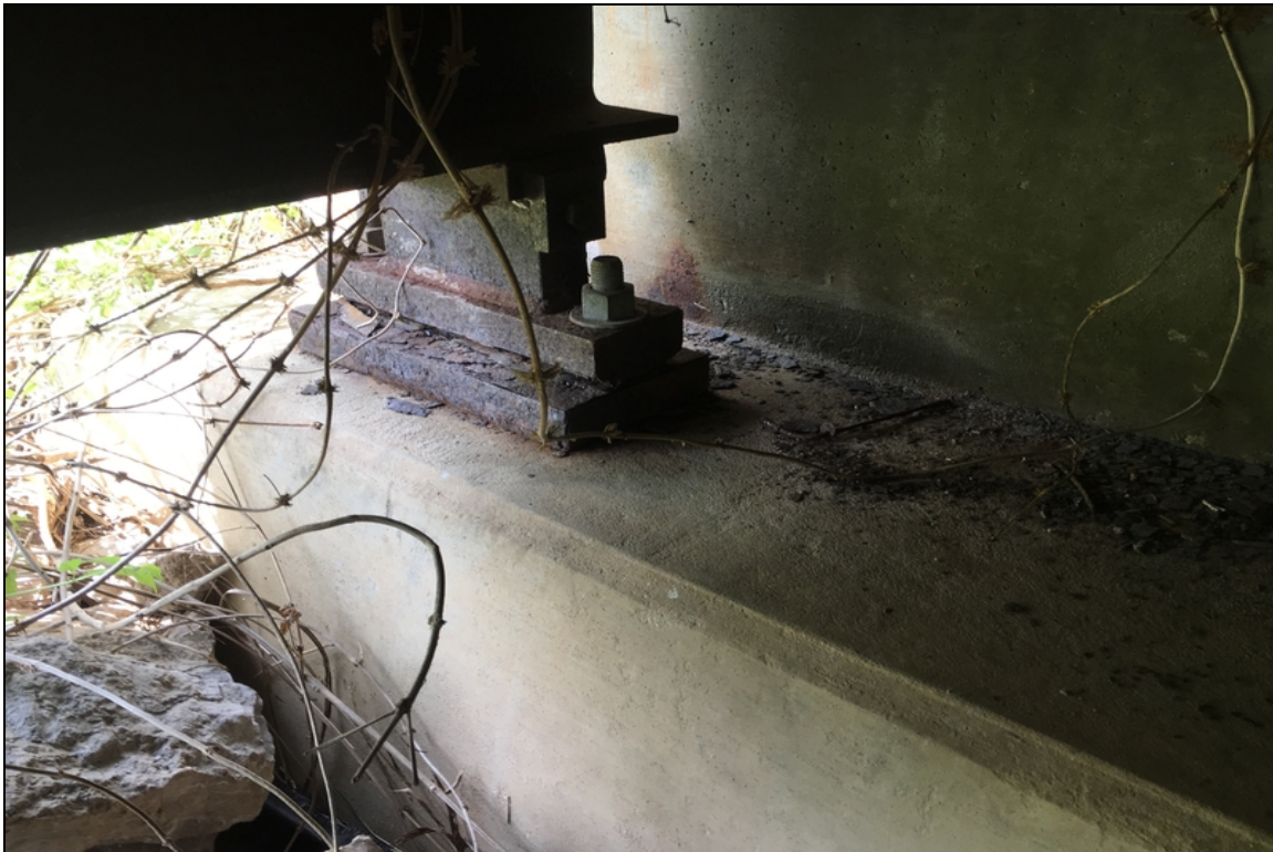
Condition of bearings 1,4,5,6 at abutment #1.
