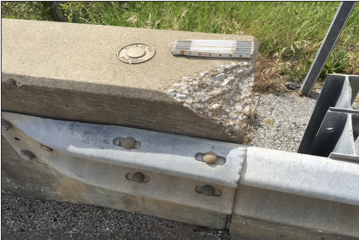
Spall with no rebar exposed at the top edge of the beginning of the right parapet.
