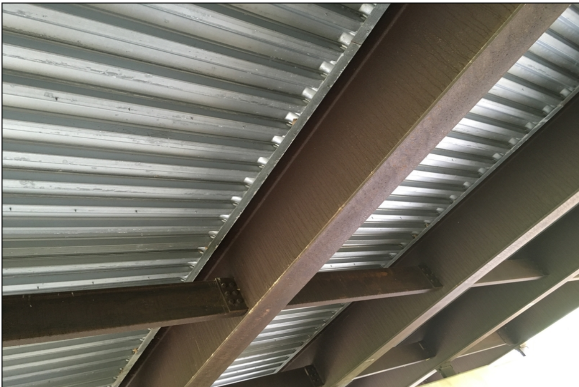
Typical view of the protective coating condition.
