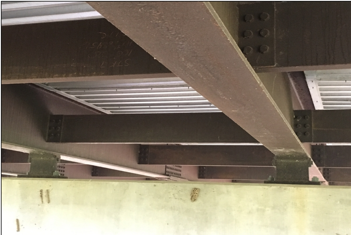
Bearing condition at pier #2. Typical of all 6 at this location.
