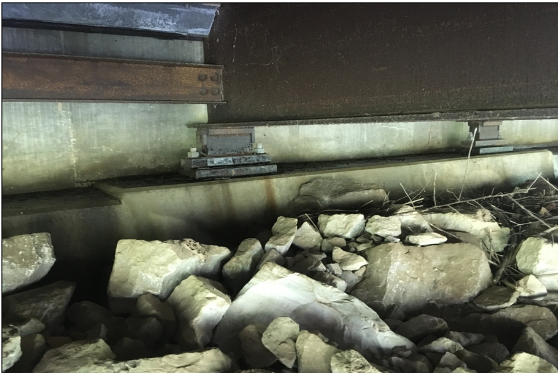
Bearing 4 at abutment 1 showing corrosion with flaking rust. Typical of other locations.
