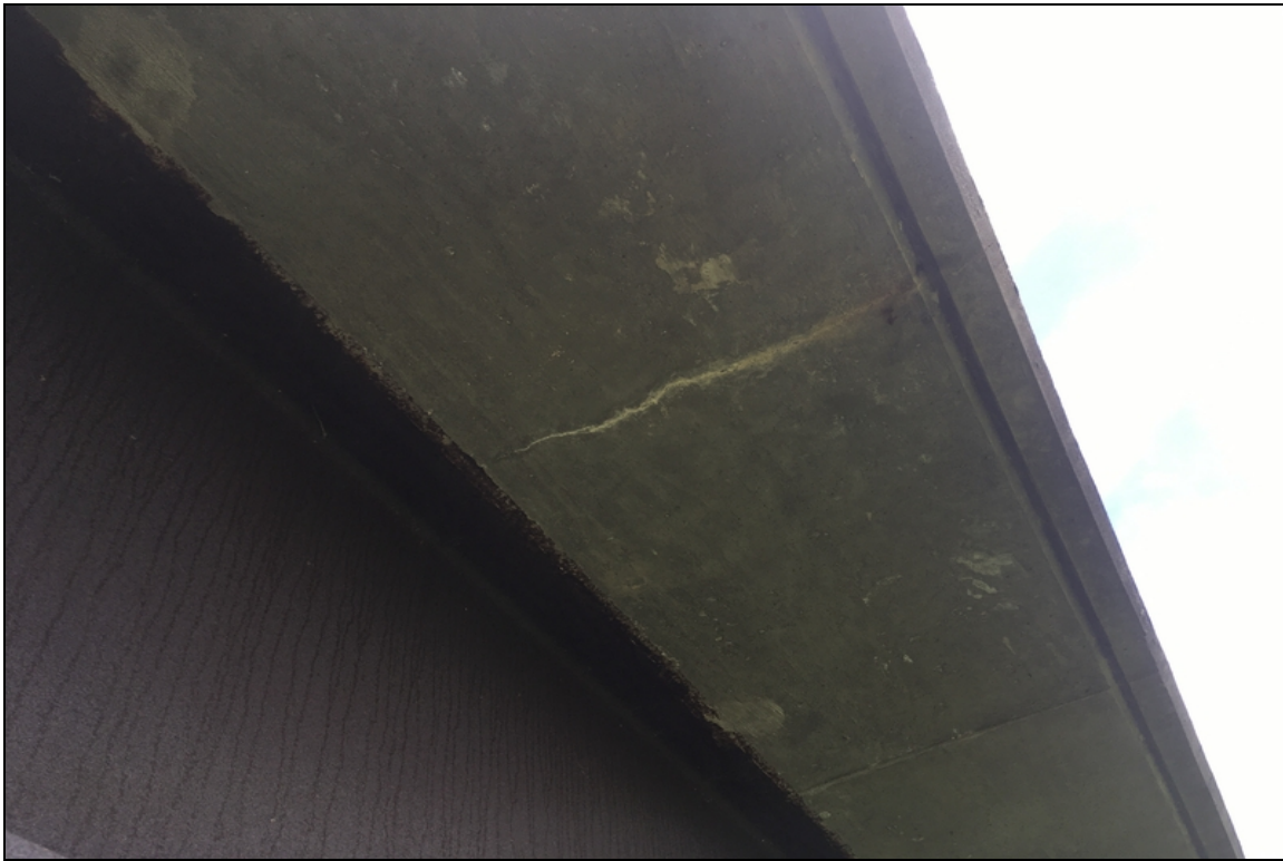
Typical efflorescence in the deck overhangs.
