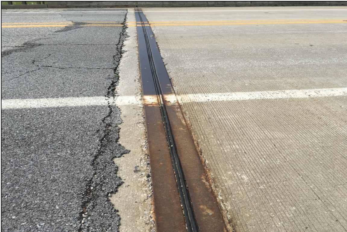
Condition of compression joint seal at abutment #2.
