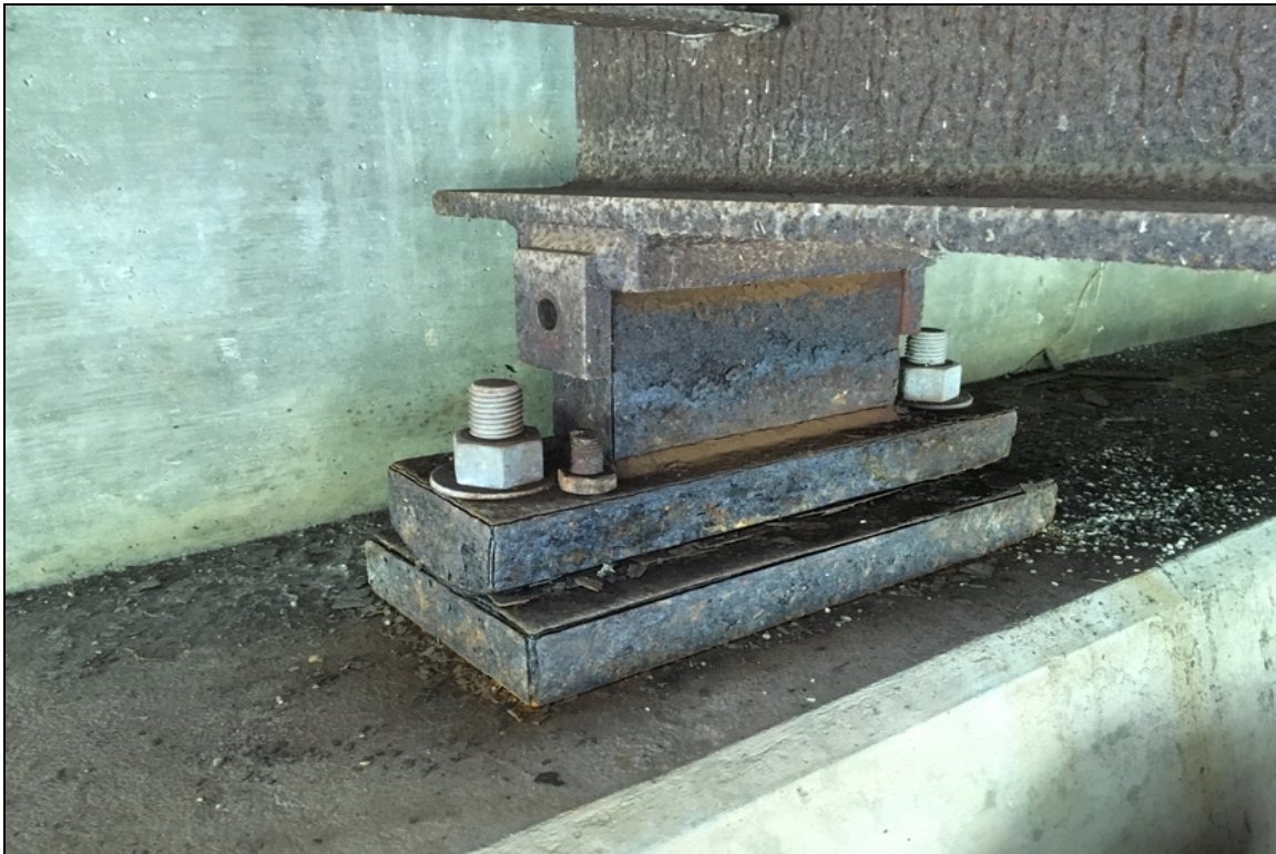
Sole plate connection bolt is sheared off at bearing #5 at abutment #1.
