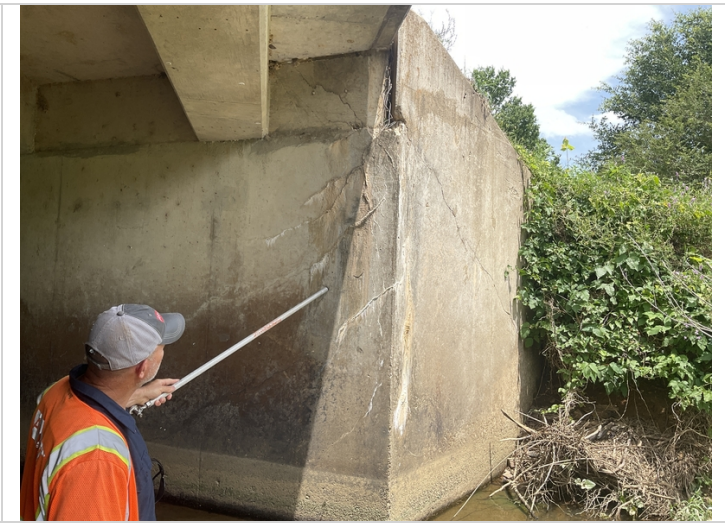
Abutment 2, right side-Cracking with efflorescence
