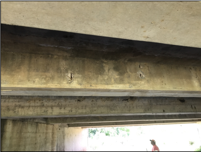
Girder # 3 has 4 small diameter shallow spalls with exposed reinforcing steel in the left vertical face of girder. Exposed reinforcing steel has no apparent noteworthy section loss during this inspection.
