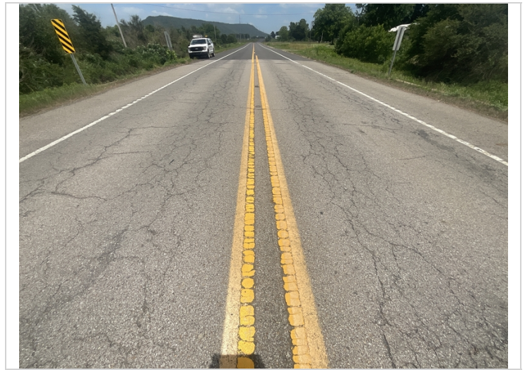
Driving surface-Mapcracking
