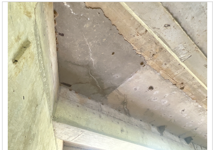
Deck undersurface, bay 5-Diagonal cracking with efflorescence
