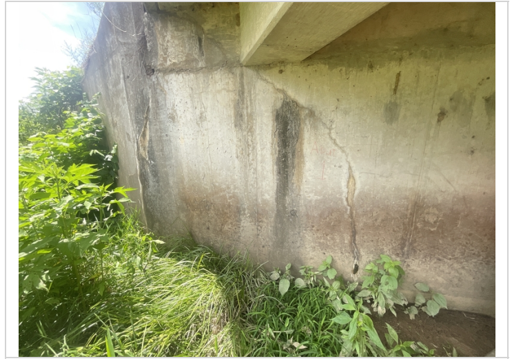
Abutment 1, right side-Diagonal cracking
