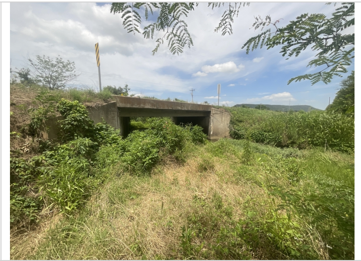
Vegetation and streambed material accumulation restricting channel
