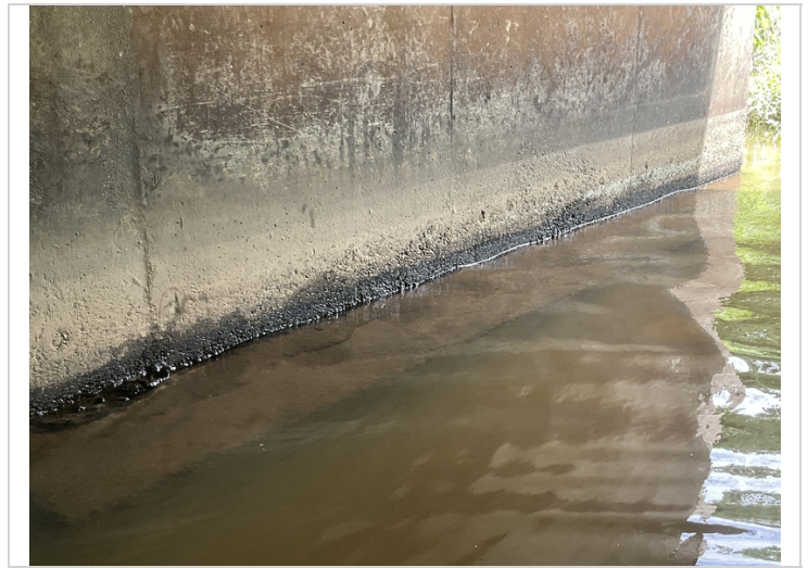
Abutment 2-Light abrasion
