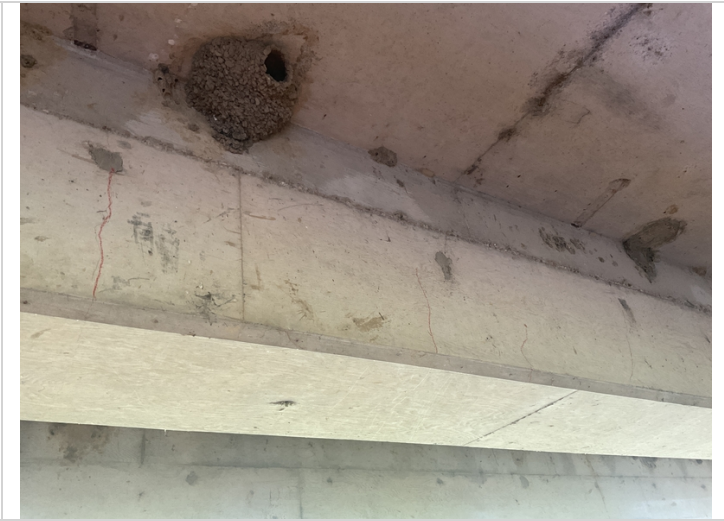
Girder 3-Hairline vertical flexure cracks
