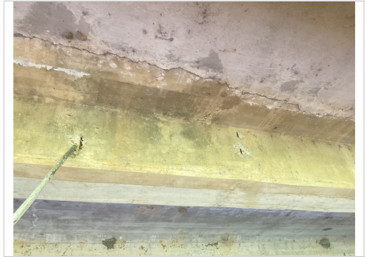
Girder 3, left vertical face-Shallow spalls with exposed reinforcing steel
