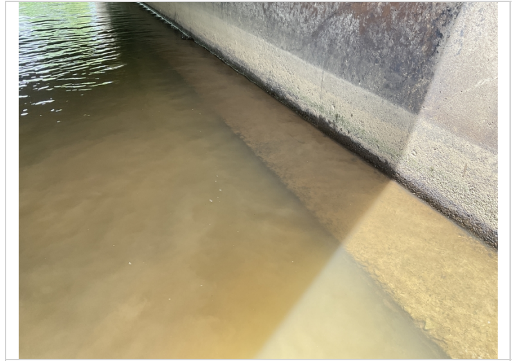
Abutment 2 footing exposed
