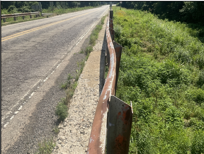
Span 8 right railing at bent 9-Collision damage
