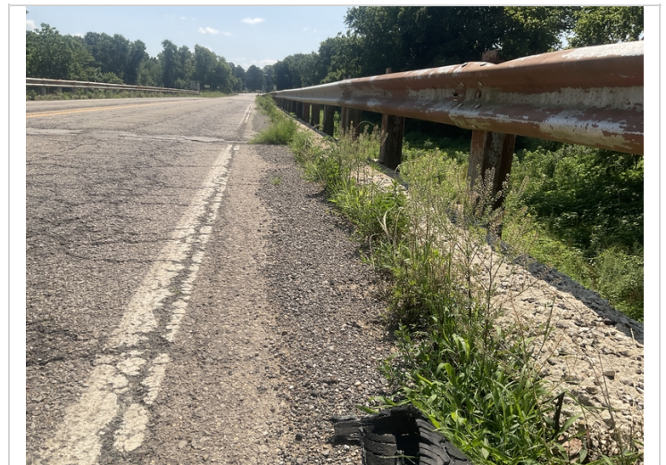
Dirt, debris with vegetation growing in shoulders
