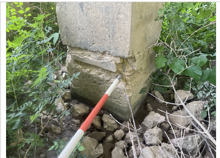
Bent 9, column 4-Spalling with exposed reinforcing steel
