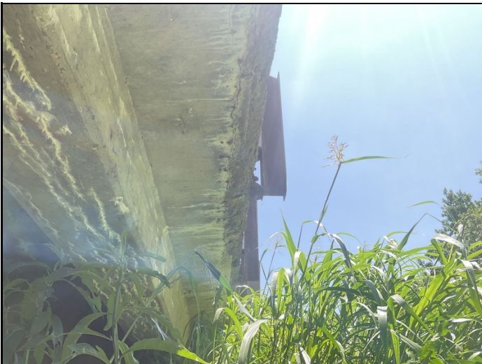
Span 10, girder 5-Mapcracking with efflorescence.
