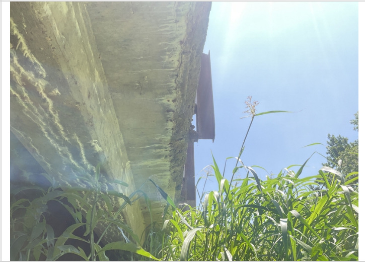
Span 10, right exterior edge of deck-Concrete deteriorating / spalling
