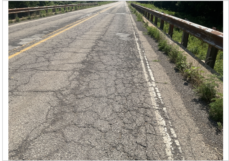
Mapcracking in wheel paths
