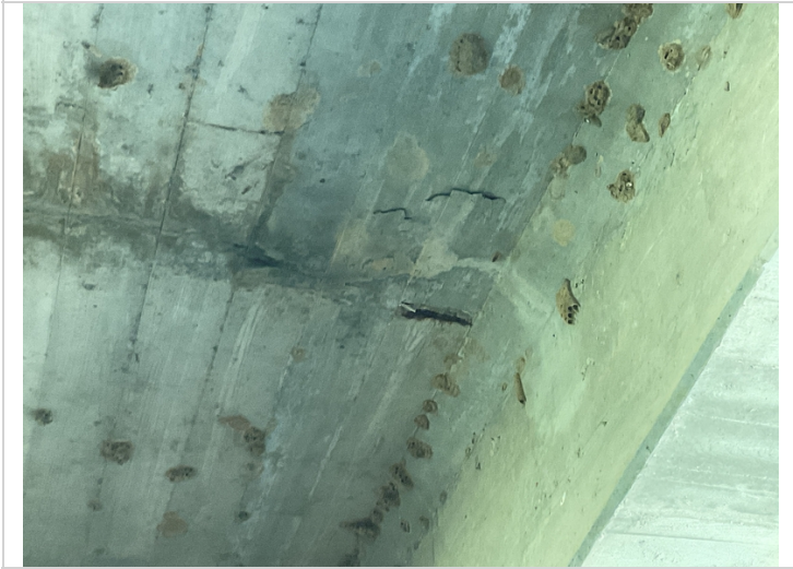
Span 1, bay 3-Delaminated areas and shallow spall with exposed reinforcing steel
