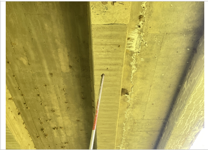
Span 8, girder 4 undersurface has a narrow width longitudinal crack that begins approximately 4' from bent 8 and extends approximately 5' towards mid-span.
