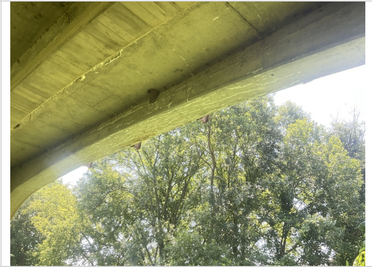
Span 2, girder 5-Mapcracking with efflorescence
