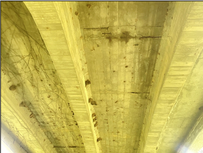
Span 2, bays 2 and 3 have shallow spalling with exposed reinforcing steel in deck undersurface
