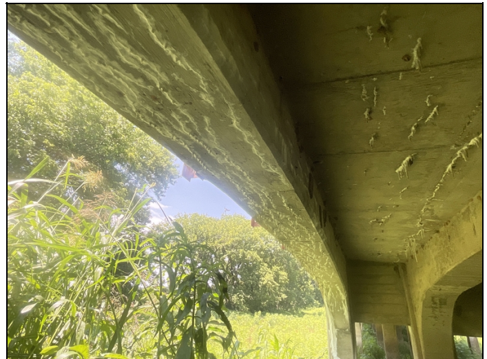
Span 10, girder 5-Mapcracking with efflorescence.
