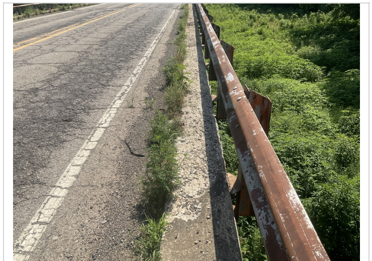
Span 2 right curb-Concrete deterioration
