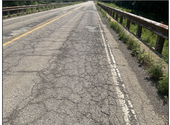
Mapcracking in wheel paths
