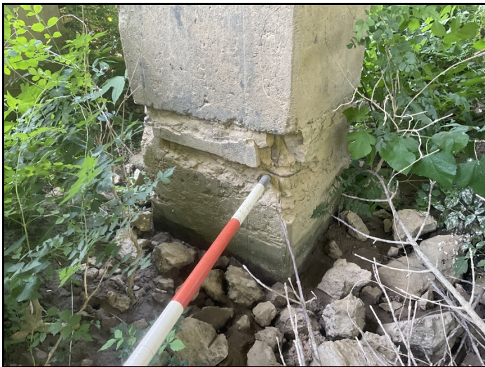
Bent 9, column 4-Spalling with exposed reinforcing steel.
