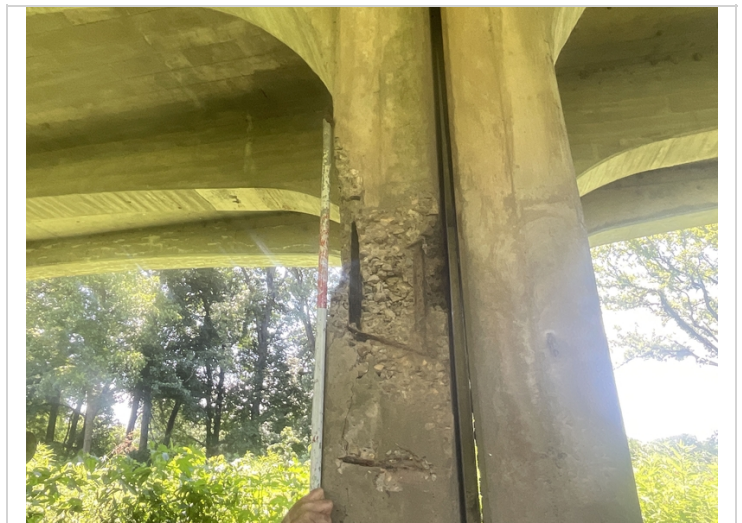
Bent 8, column 3 of span 8-Spalling with concrete section loss and exposed primary reinforcing steel. Exposed reinforcing steel has measurable section loss.
