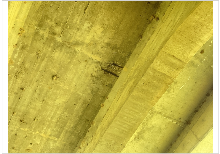
Span 3, bay 3-Spall with exposed reinforcing steel
