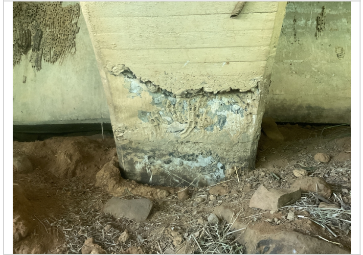
Span 1, girder 4 at abutment 1-Spalling in haunch portion of girder
