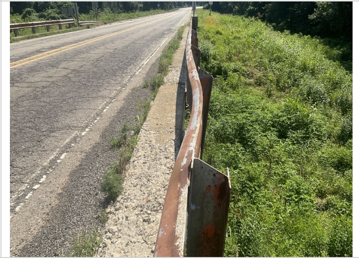
Span 8 right railing at bent 9-Collision damage
