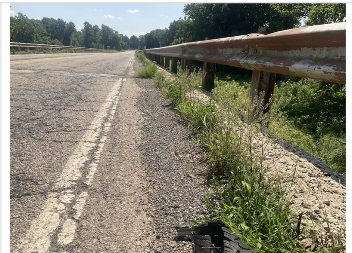
Dirt, debris with vegetation growing in shoulders
