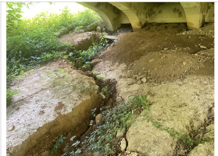
East embankment at abutment 2 has erosion
