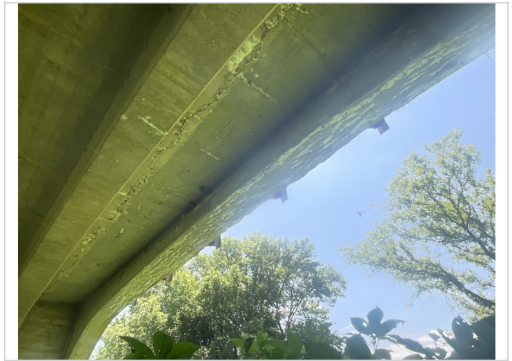
Span 6, girder 5-Mapcracking with efflorescence
