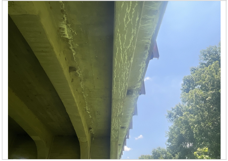
Span 8 right side-Mapcracking with efflorescence in girder 5 and deck undersurface
