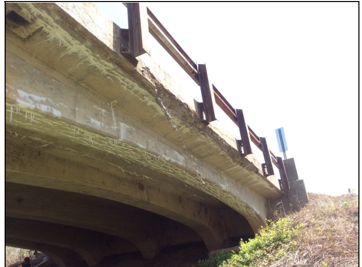
Span # 10 Right concrete deterioration with exposed reinforcing steel.
