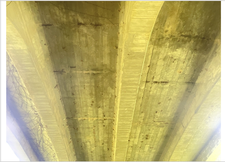
Span 5 deck undersurface-Shallow spalling with exposed reinforcing steel
