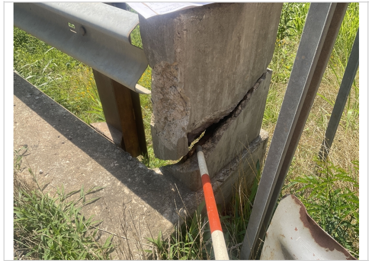
Abutment 1 right end post fractured
