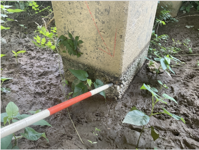
Bent 7, column 2 has light abrasion with a 4" area of concrete deterioration approximately 1" deep at base of column.
