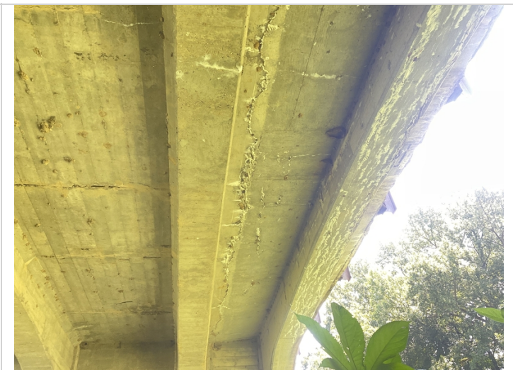
Span 6, bay 4-Efflorescence along longitudinal construction joint
