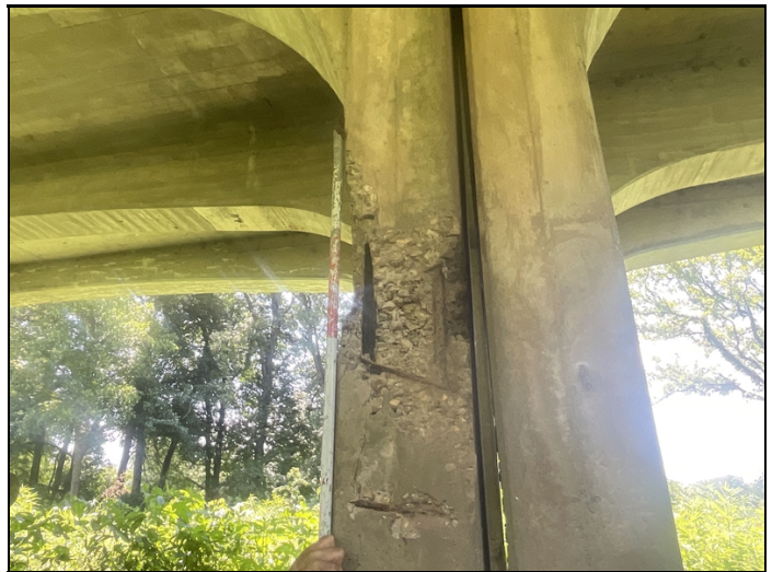
Bent 8, column 3 of span 8-Spalling with concrete section loss and exposed primary reinforcing steel. Exposed reinforcing steel has measurable section loss.
