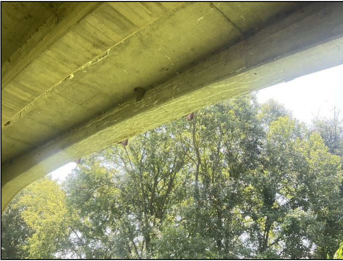
Span 2, girder 5-Mapcracking with efflorescence.
