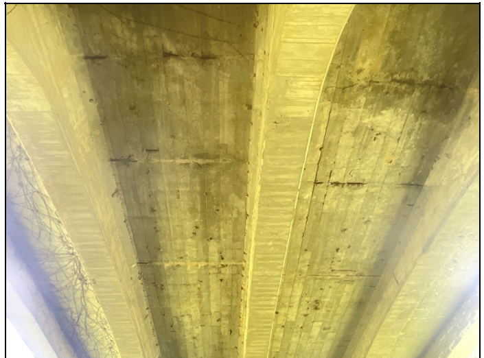
Span 5 deck undersurface-Shallow spalling with exposed reinforcing steel
