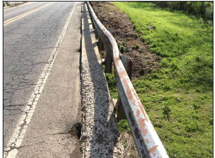
Span # 8 RT collision damage in the bridge rail and concrete deterioration in the curbs with exposed reinforcing steel.
