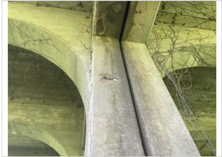
Bent 4, span 4, column 2-Shallow spall with exposed reinforcing steel
