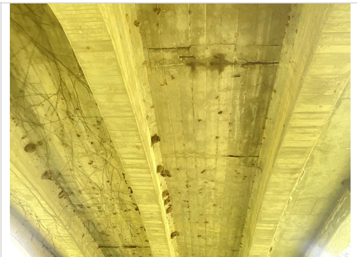
Span 2, bays 2 and 3 have shallow spalling with exposed reinforcing steel in deck undersurface
