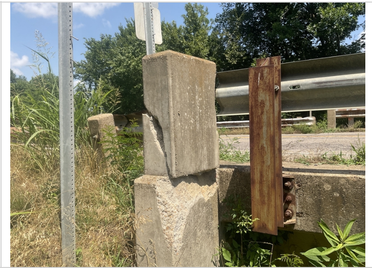
Abutment 1 right end post-Fractured
