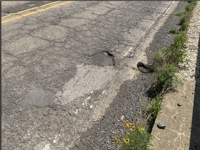
Span # 8, right lane-Failing repair.
