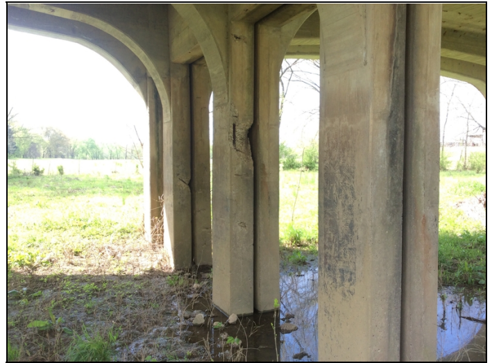
Bent # 7 Columns # 3 & 4 spalling with exposed reinforcing steel.
