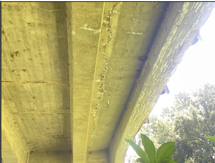
Span 6, bay 4-Efflorescence along longitudinal construction joint
