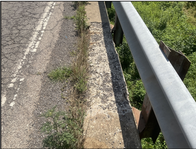
Curbs on both sides of the bridge has multiple areas of soft deteriorated concrete with exposed reinforcing steel. Span # 5, right curb pictured.
