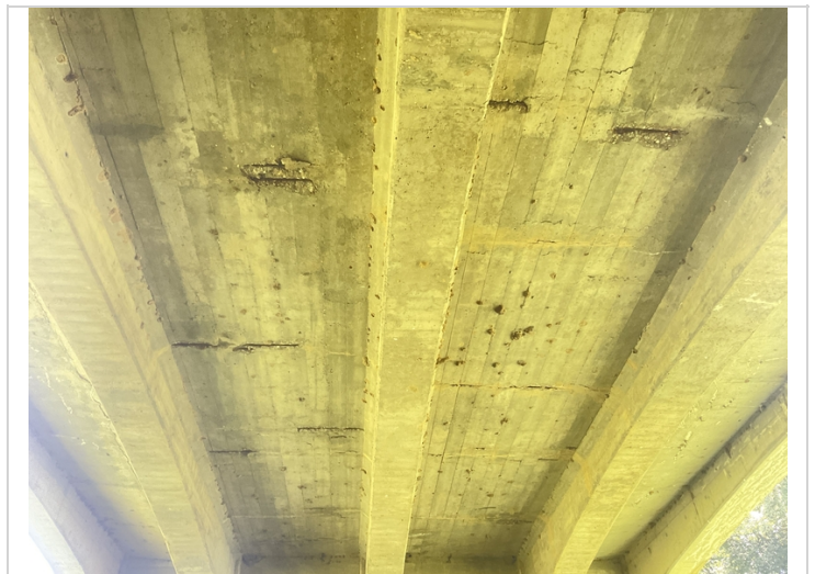
Span 6 undersurface-Shallow spalling with exposed reinforcing steel
