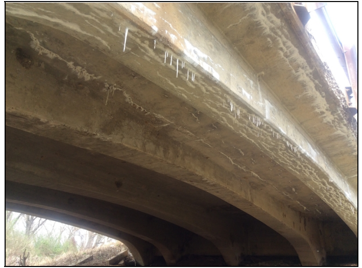
Span 11 right map cracking with efflorescence and leaching.
