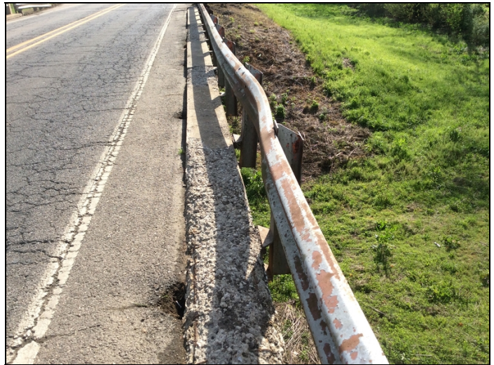
Concrete deterioration in the curbs with exposed reinforcing steel.
