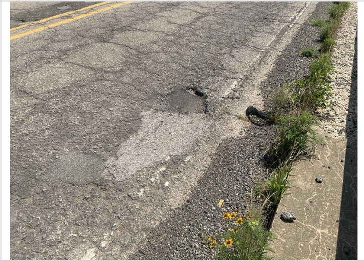
Span 8, right lane-Failing repair
