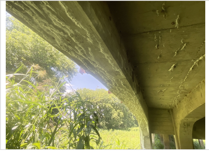
Span 10, girder 5-Mapcracking with efflorescence
