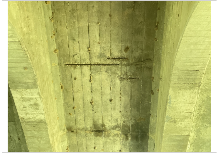
Span 9, bay 3 deck undersurface at bent 9-Spalling with exposed reinforcing steel
