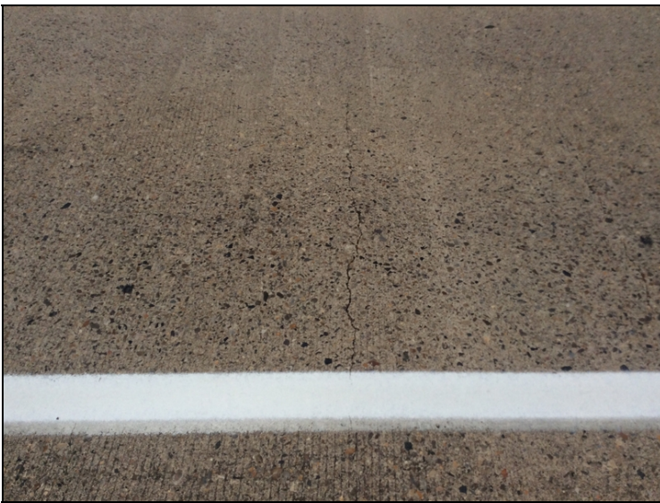
Moderate unsealed cracks.
