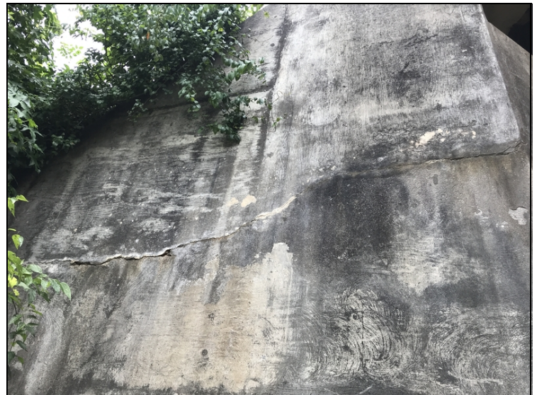
Abutment 4, Left, Wing Wall: Cracking.
