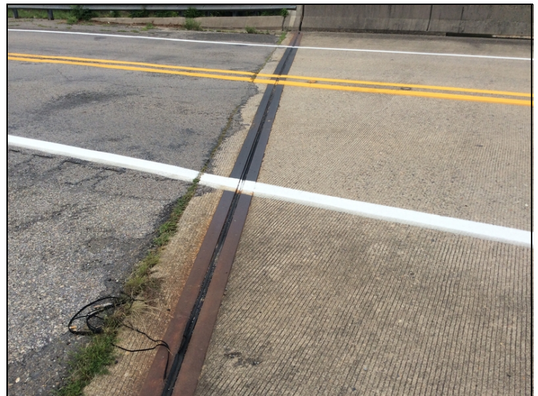
Joint #1 - deterioration of seal material.
