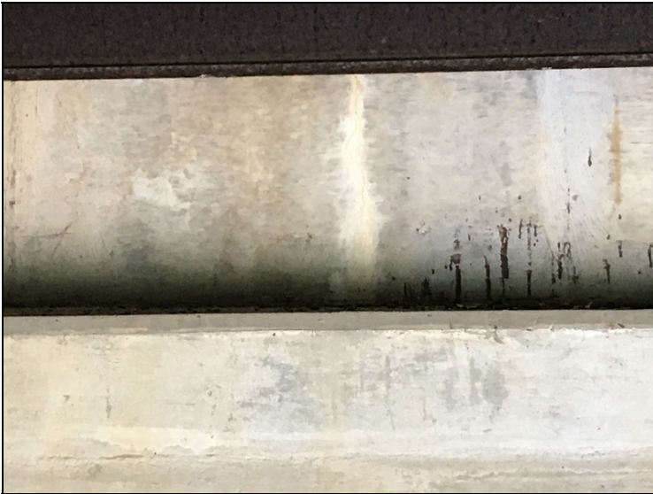
Typ. Cracking W / Efflor in Back Walls.
