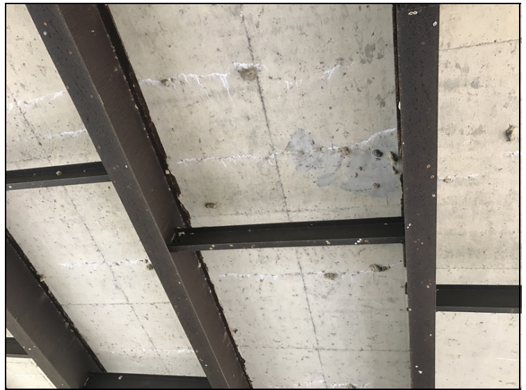
Deck, Undersurface: Typical cracking with efflorescence.
