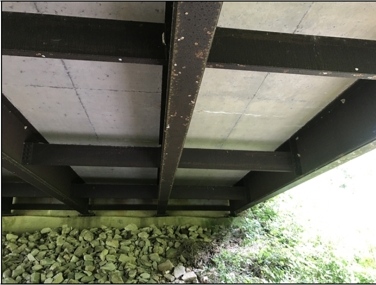
Deck, Undersurface: Cracking with efflorescence.
