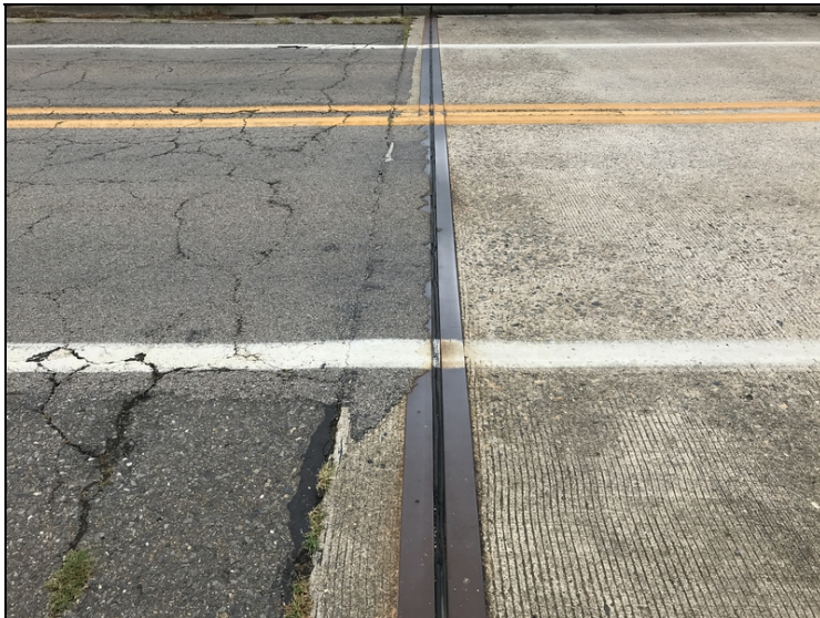
Joints: Typical damage.
