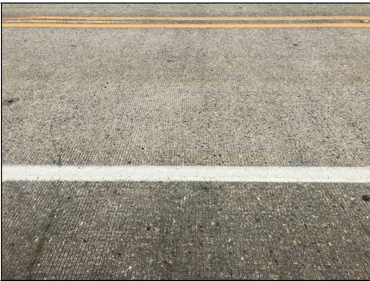
Deck: Typical moderate cracking.
