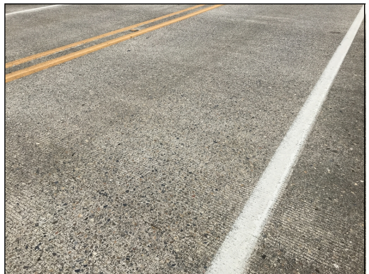
Deck: Typical minor abrasion in wheel paths.
