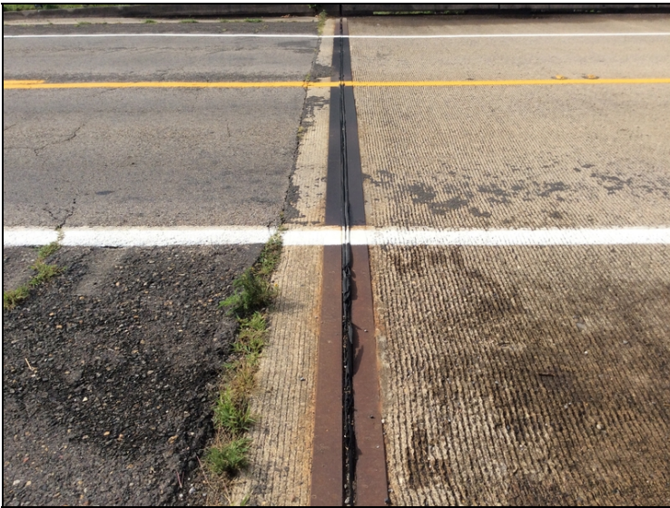
Joint #2 over abut #5 - seal material has rips and tears.
