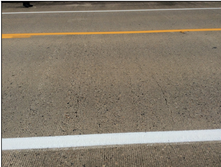
Span #3, right lane - Moderate and major transverse and longitudinal unsealed cracks, typical throughout.
