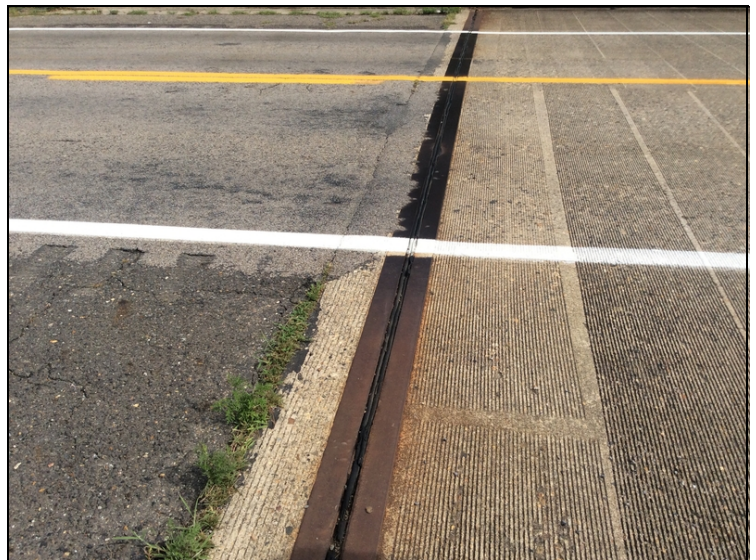
Joint #1 - moderate deterioration of seal material.
