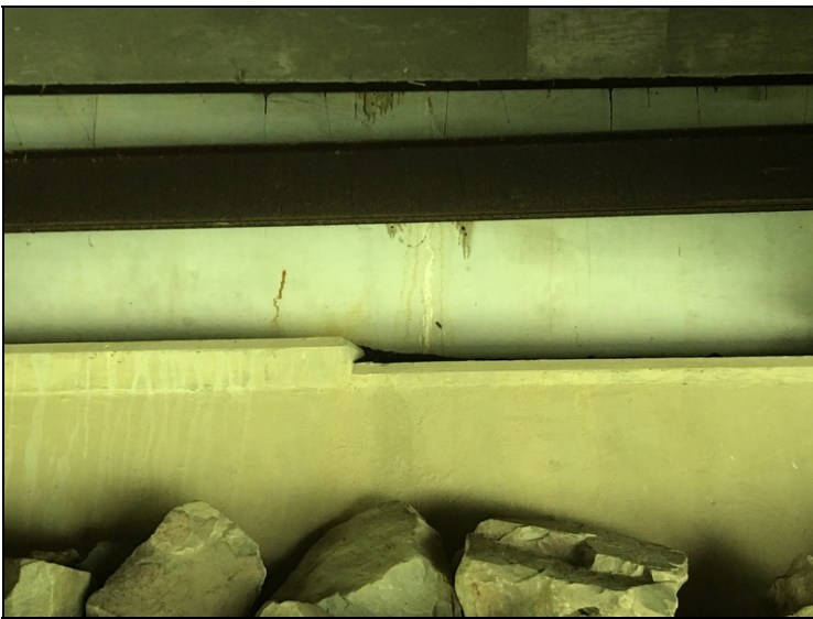
Abutment 1: Cracking with efflorescence.
