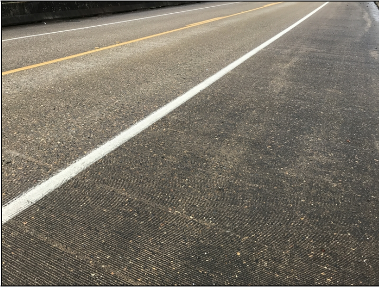
Spans 1 - 3: Minor abrasion.
