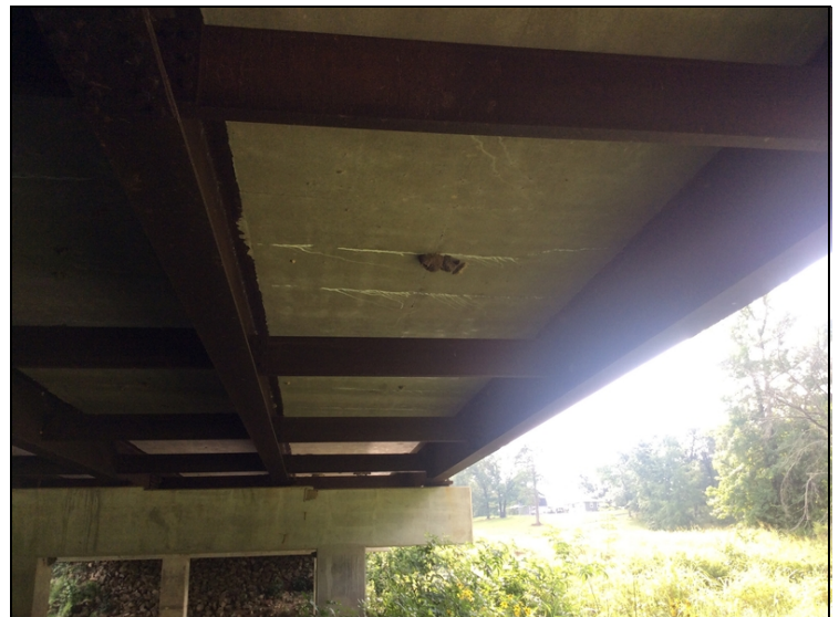
Span #2, underside - cracks with efflorescence. Typical throughout.
