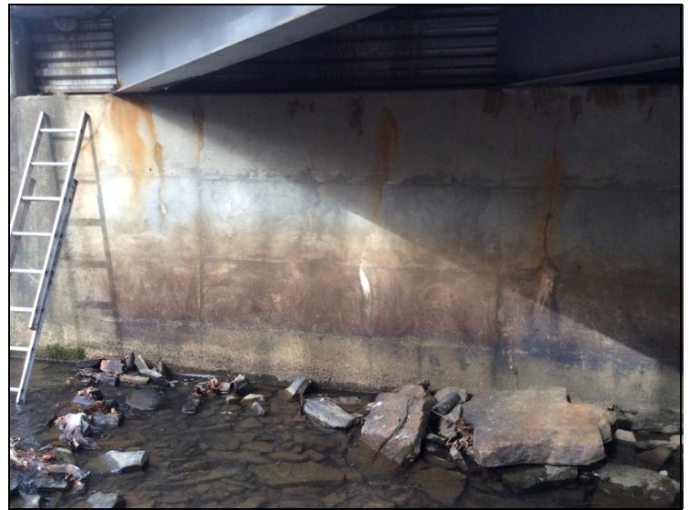
Abut #1 - Minor cracks with efflorescence in a few places throughout . 6 Lf. C2 efflorescence
