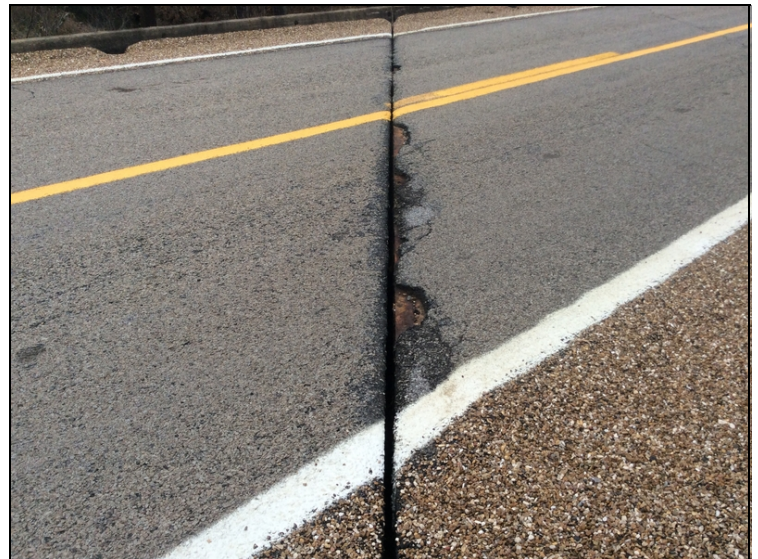
Open joint over pier #2. Asphalt overlay has some minor to moderate spalls at the joint.
