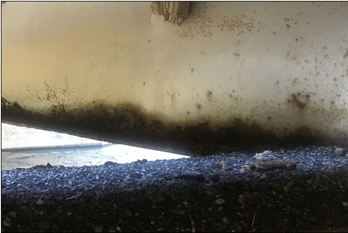
Typ. Rust on Ends of Beams.
