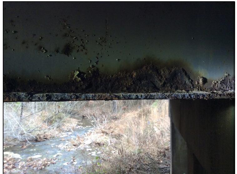
Beam #3 backside of pier #2 has moderate pack rust and moderate section loss in the lower web and the bottom flange.
