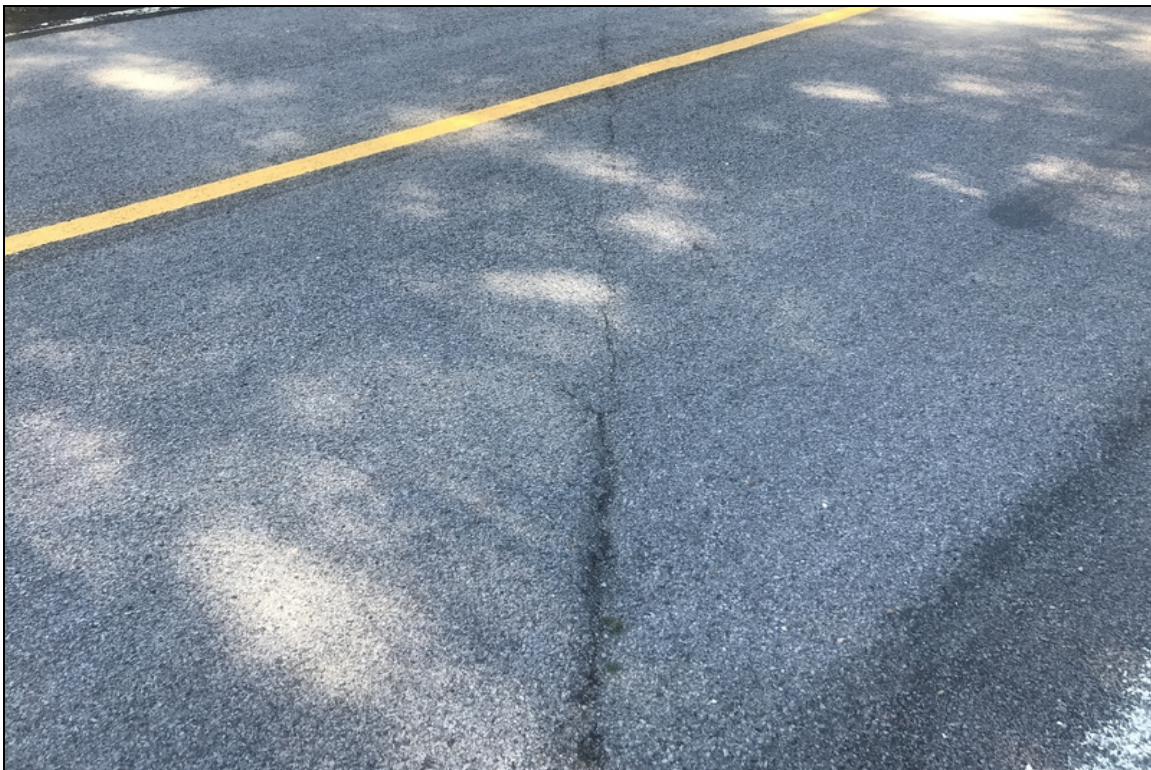
Typ. Cracking in Overlay at Abutments.
