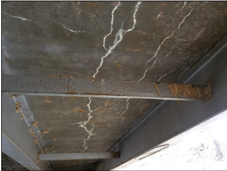
Span #1 between beams 3 and 4 minor to moderate cracks with efflorescence. Span #2 is typical.
