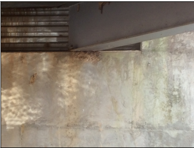
Abut. #1 - minor spall with no rebar exposed in bearing area under beam #1. Typical under beams 2 and 3.
