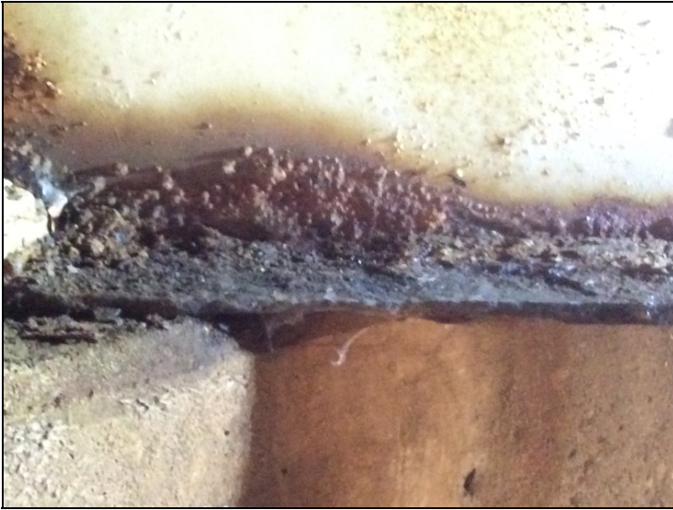
Beam #2 ahead side of pier #2 has moderate to major section loss on right side of the bottom flange.
