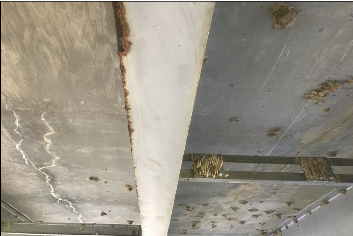
Typ. Condition of Soffit.
