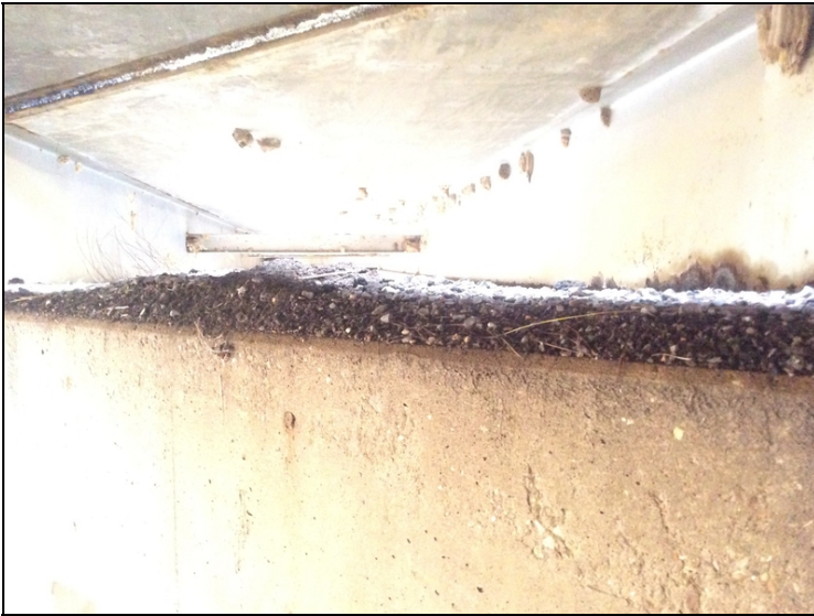
Pier #2 - Gravel, asphalt and dirt buildup on top of the cap full length.
