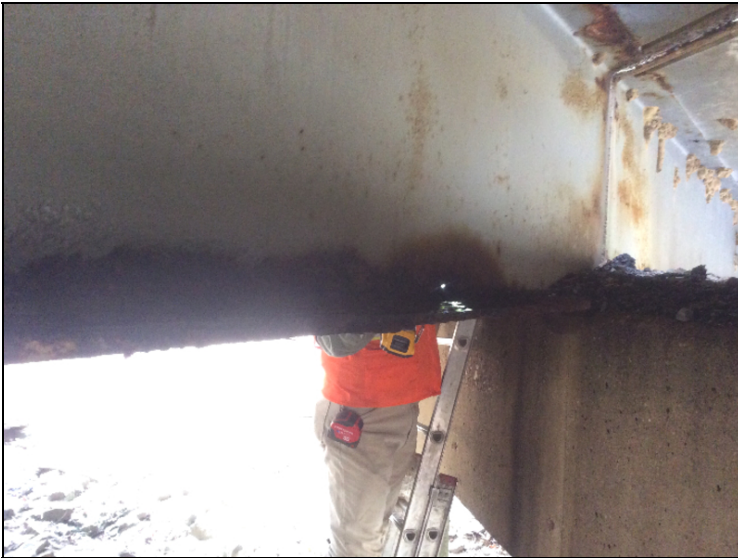
Beam #3, ahead side of pier #2 has moderate pack rust in lower web and top of the bottom flange. There is complete section loss (hole) in the lower web approx. 2' back from the end of the beam.
