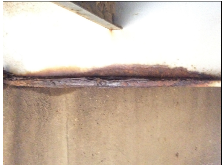
Beam #3, ahead side of pier #2 has some minor pack rust with minor section loss in the top of the bottom flange and moderate rust in the lower web.
