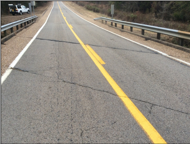
Minor to moderate cracks in overlay in span #3.
