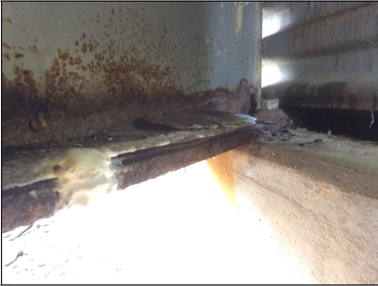
Beam #4 at abut. #1 - moderate to heavy pack rust with minor section loss.
