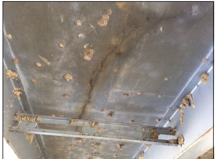
Span #1 between beams 2 and 3 has moderate crack. Approximately 15 sf. C2 cracks
