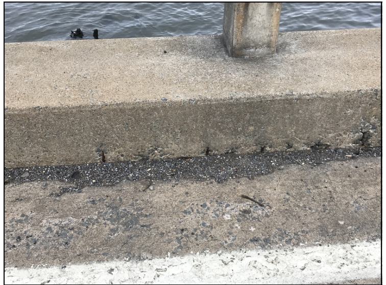
Minor Spalling in Bt. of Curb at Deck due to Rebar to close too Surface.
