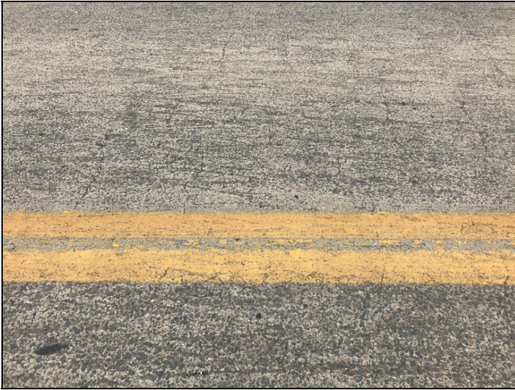
Typ. Cracking in Deck.
