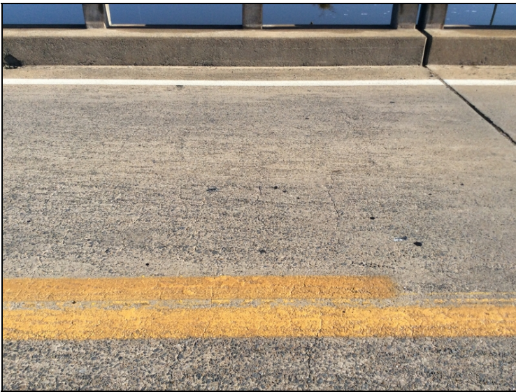
Span #2 - unsealed cracks.
