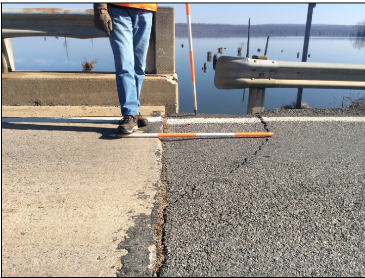
Abut #1 (SE end of bridge) Roadway settling.
