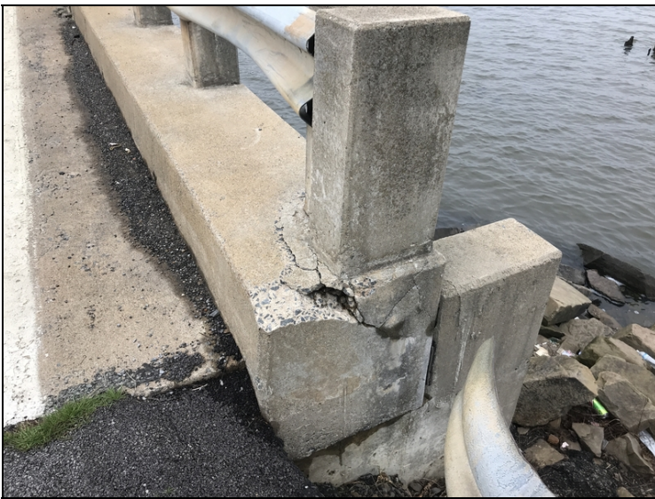
Post Broken at Abutment 1 Rt. Side.
