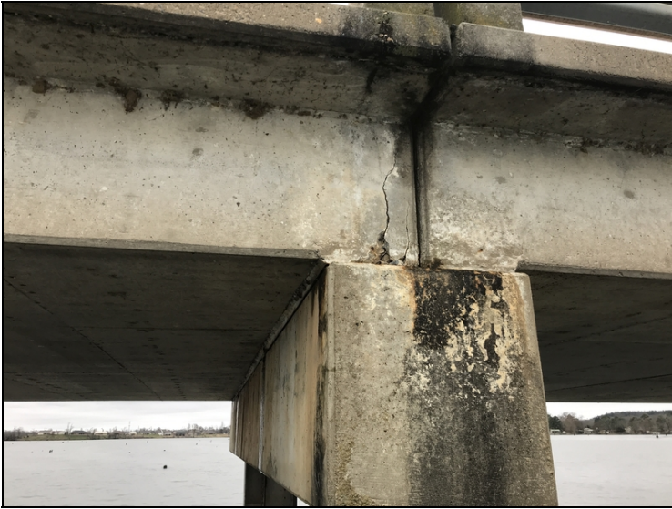
Delam, Cracking & Spalling in Side of Slab in Span 3 at Pier 4.
