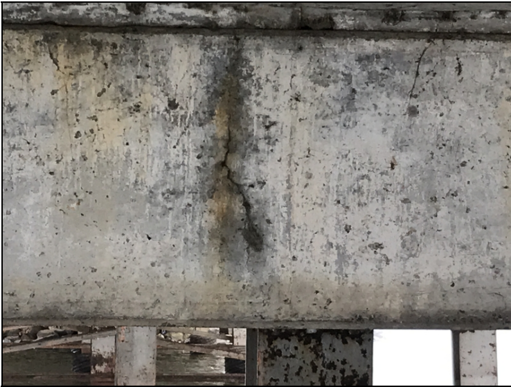
Typ. Vertical Cracking in Caps.
