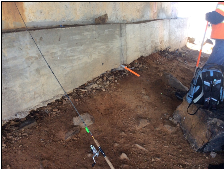
Abut. #1 - undermining full length of abut. Extends back under abutment approx. 3 ft in places.
