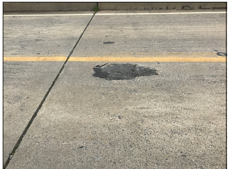
Typ Spalling in Deck.
