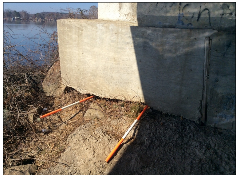
Abut. #7 - minor undermining on the left end approx. 7 ft.
