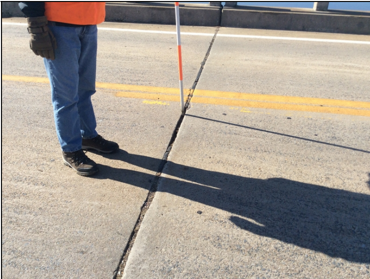
Joint at beginning of span 6 - 12 ft missing joint material
