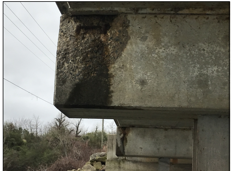
Typ. Spalling in Caps.
