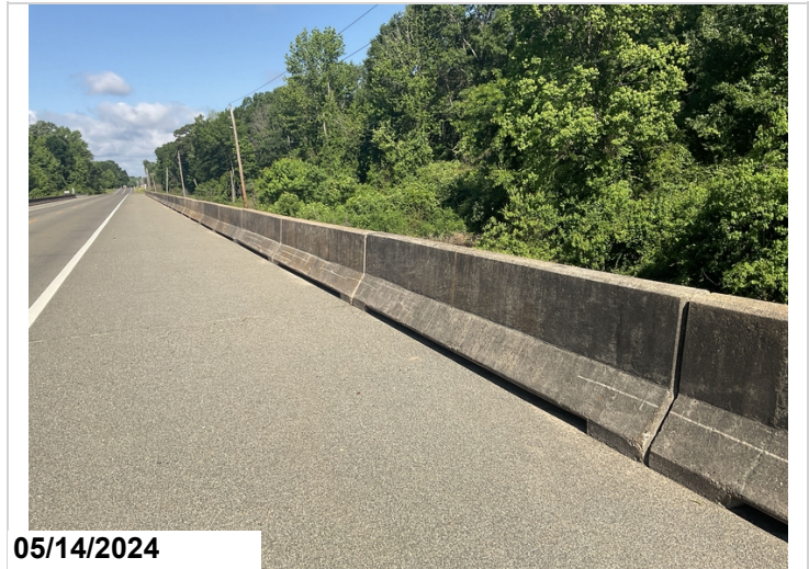
Right side, all spans have upto 1/2" creep.
