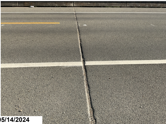
Typical of all joints, joint rehab has been performed and expansion material is in good condition.
