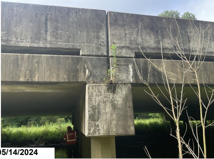
Spans 2 and 3 right side at bent 3 cracks with efflorescence, typical at both sides of all spans.
