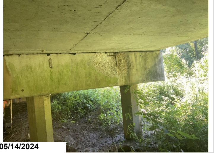
Bent 9 Ahead side 4' right of the left end, 30" x 24" x 3" spall with exposed rebar.
