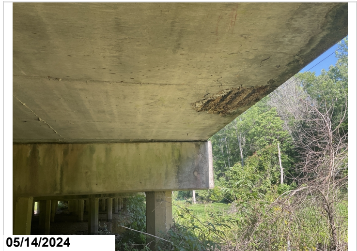
Span 11 Under surface, right side 6' back of Bent 12, 30" x 20" x 3" spall with exposed rebar, rebar has minor section loss. 6SF exposed rebar CS3
