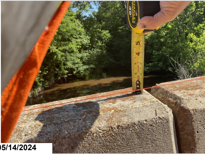
Span 4, right side, 1/2" creep at mid span. All spans have creep, span 4 is the worst.
