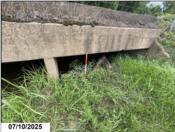
07/10/2025 Barrel 2, sediment built up to 1'-6" deep in the bottom of the culvert.
