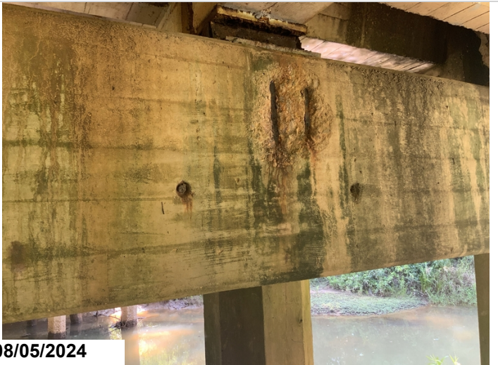
Bent 3 cap back exposed rebar
