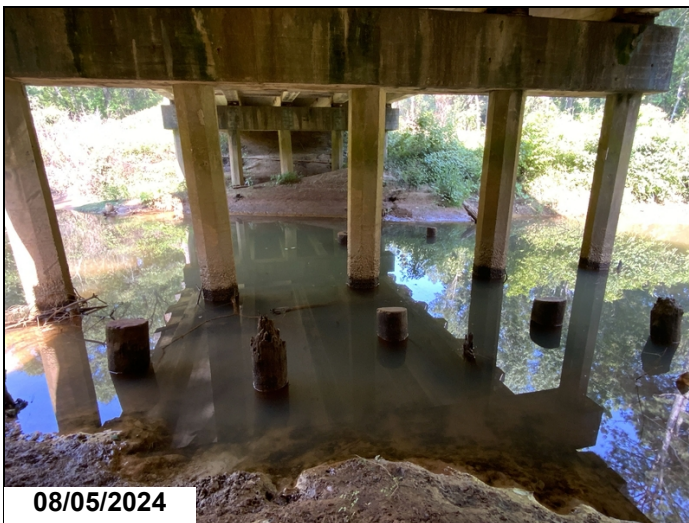
Bent 3 abrasion to piles.
