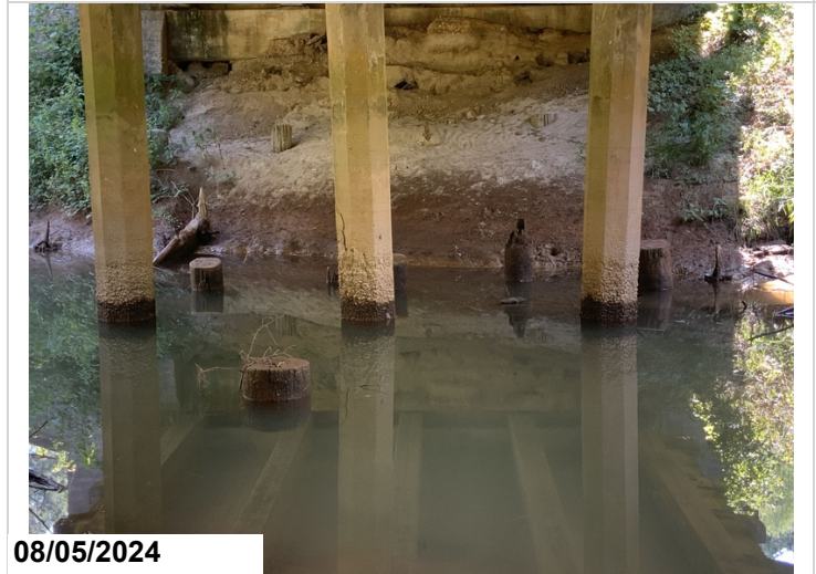
Bent 3 pile 3 delam.
