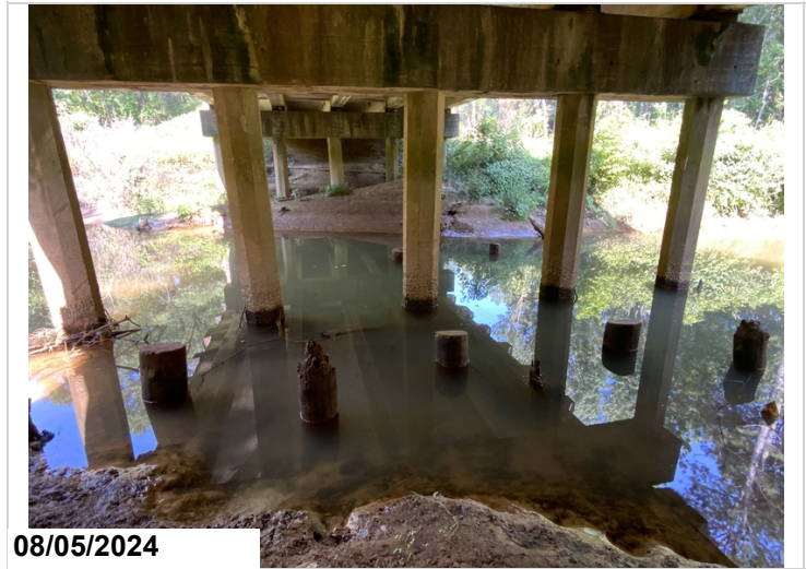
Bent 3 abrasion to piles.
