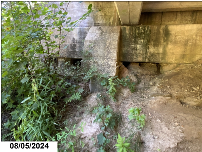
Bent 2 abutment left side scour
