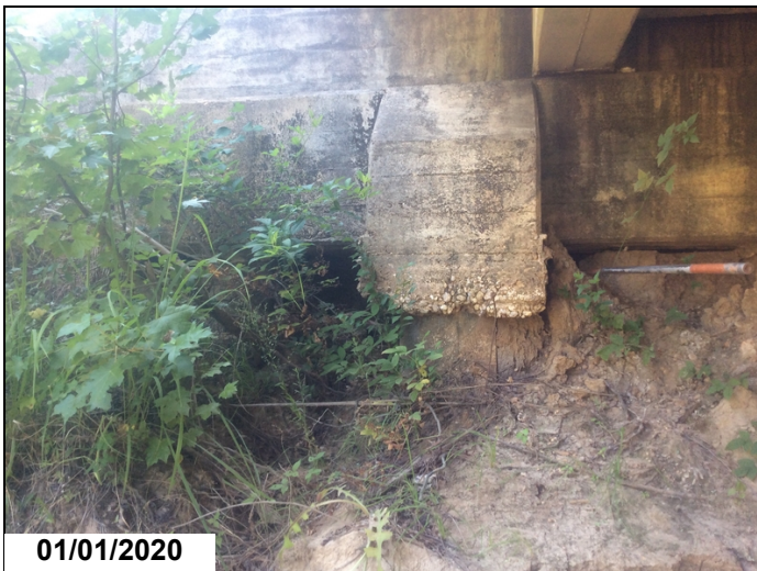
Abutment 2 Lt. side there is a large scour hole that goes back under the abutment cap from edge of wingwall & goes Rt. Just past girder 1.
