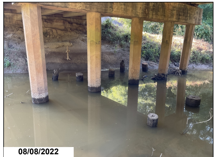
Bt. 3, looking ahead, abrasion to the piles & pile 3 has cracks & delams.
