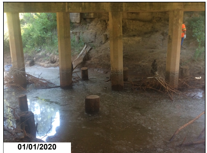
Bent 3 piles abrasion and wear pile 3 has a crack
