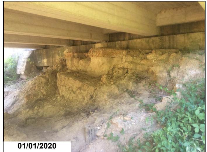
Abutment 2 slope has significant scouring & lateral stream migration.
