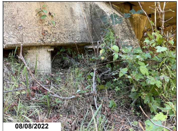
Bt. 4, left side of the abutment, erosion below the cap of the abutment.
