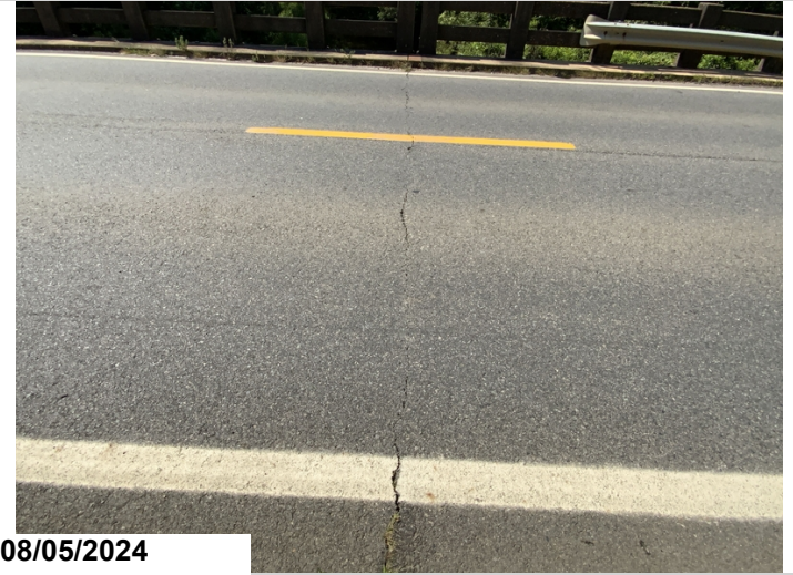
Cracks over joints in wearing surface
