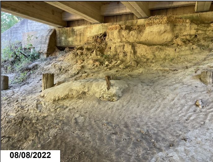
Bt. 4, abutment, scour action from the stream is removing the embankment.
