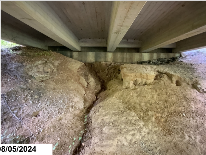
Abutment 1 slope erosion.
