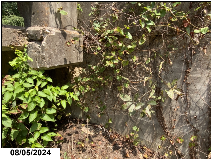
Abutment 2 right side large spall from impact damage.
