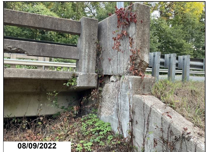
Bt. 5, right end of the abutment damage.
