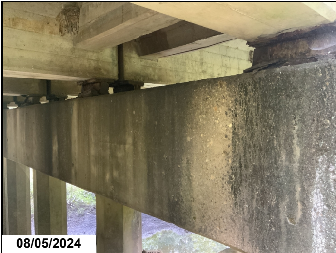
Bent 2 bearings active corrosion common all bents
