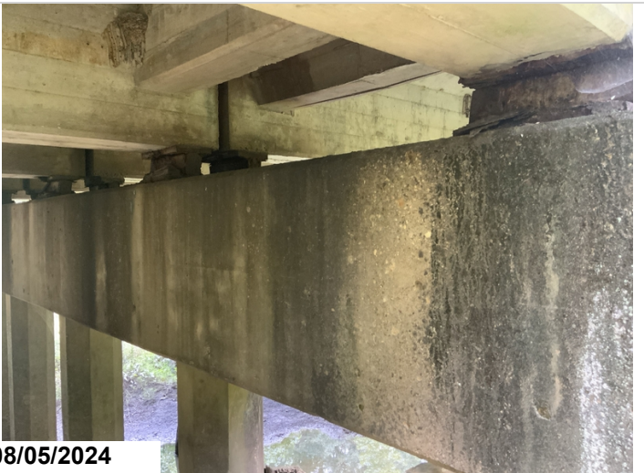
Bent 2 bearings active corrosion common all bents
