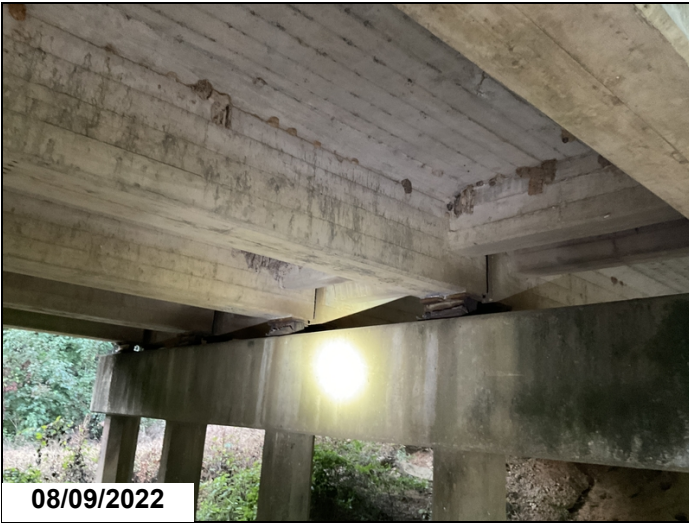
Bt. 2, bearing masonry plates have layering rust, all bearings have corrosion.
