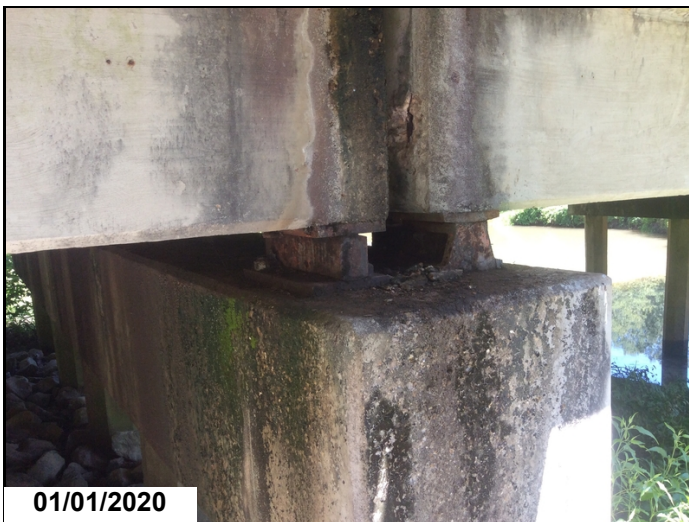
Bearings and plates all bents active corrosion
